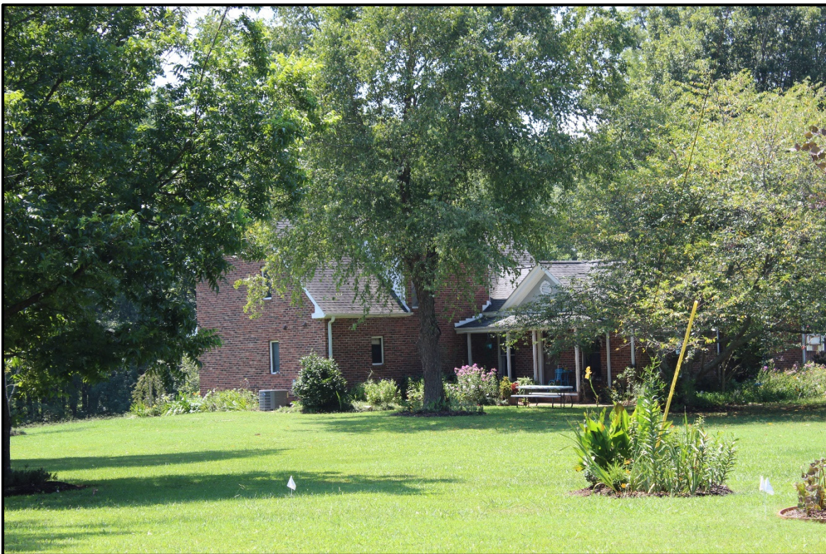
Figure 2.2. Architectural resource AM2655; view is southwest featuring the main entrance to the house located on the modern addition.
