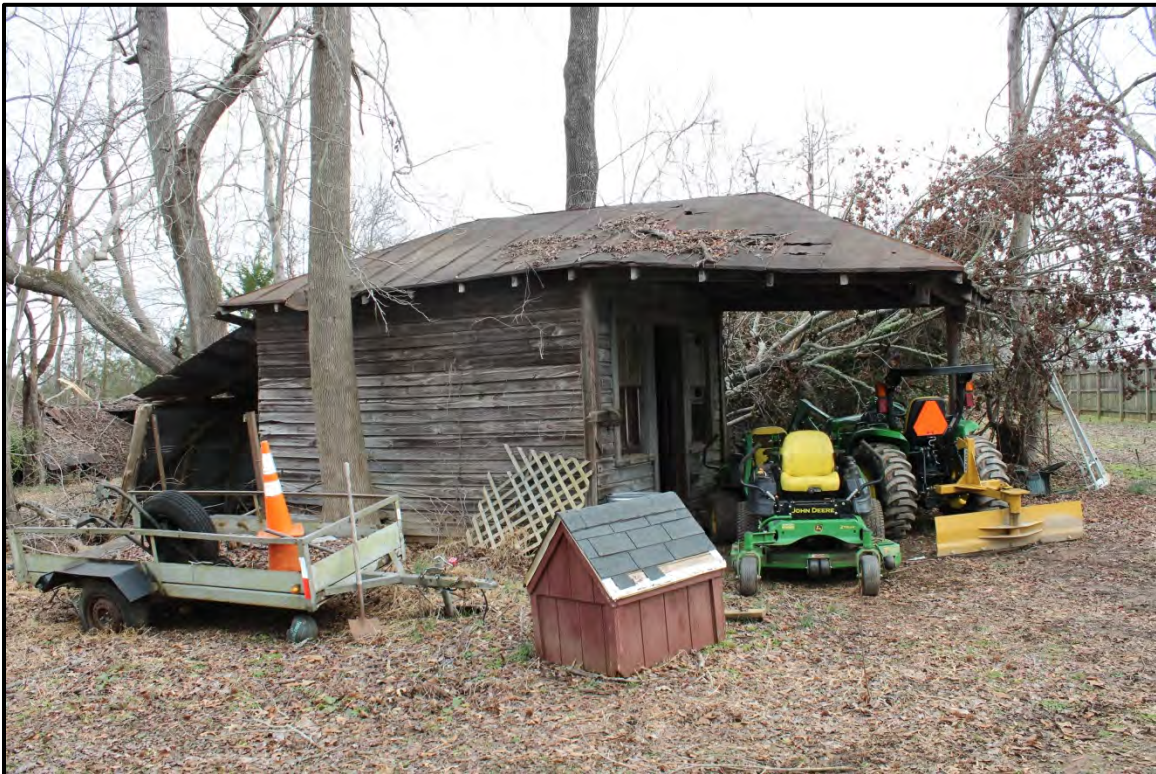
Figure 2.91. Architectural resource RK1819; view is east and features the agricultural office building.
