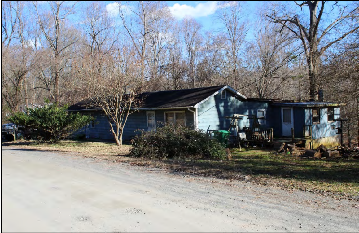
Figure 2.46. Architectural resource RK1793; view is northeast featuring the façade and southwest elevation.
