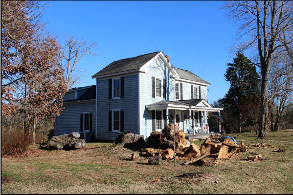
Figure 2.58. Architectural resource RK1796; view is east featuring the façade and west elevation.
