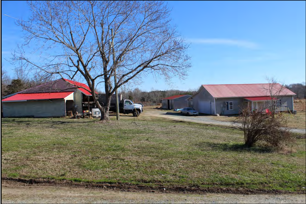
Figure 4.131. Architectural resource AM2634; view is east featuring the vehicle maintenance shop.
