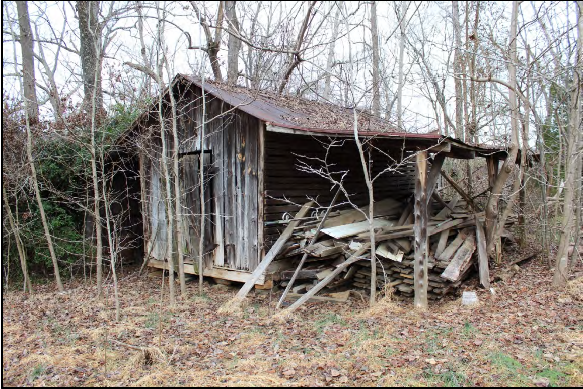
Figure 2.92. Architectural resource RK1819; view is northwest and features the storage shed.
