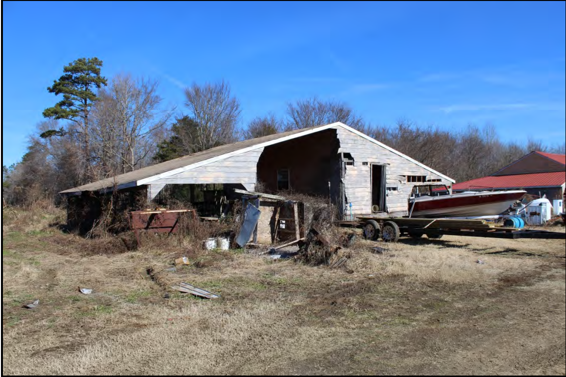
Figure 4.133. Architectural resource AM2634; view is east featuring the equipment shed.
