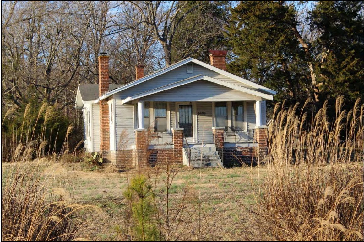
Figure 3.8. Architectural resource GF9109; view is north featuring the façade.
