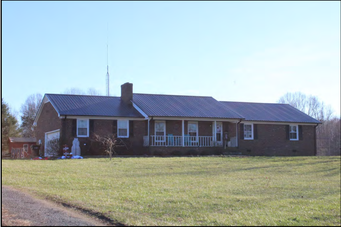
Figure 4.37. Architectural resource AM2627; view is southwest featuring the façade and east elevation garage. The modern shed is located in the background.
