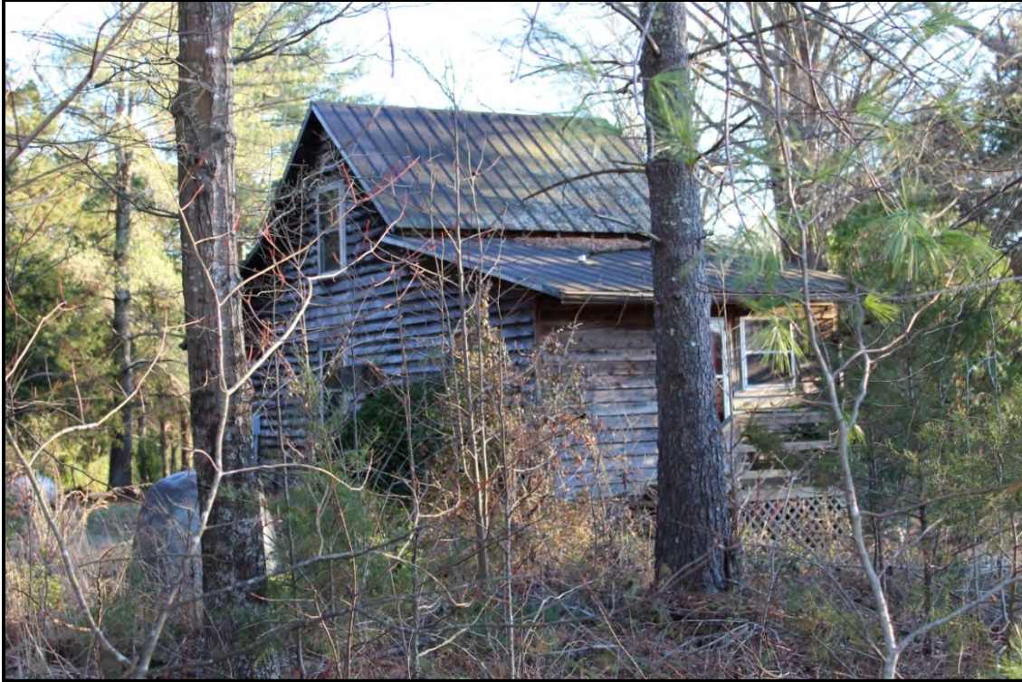
Figure 2.96. Architectural resource RK1800; view is southwest featuring the façade and east elevation.
