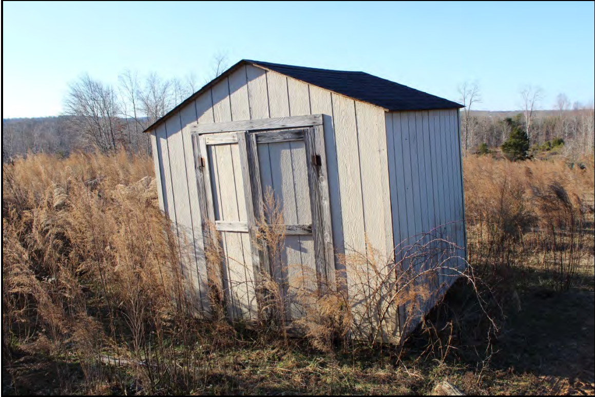
Figure 2.41. Architectural resource RK1792; view is southwest featuring the late twentieth century storage shed.
