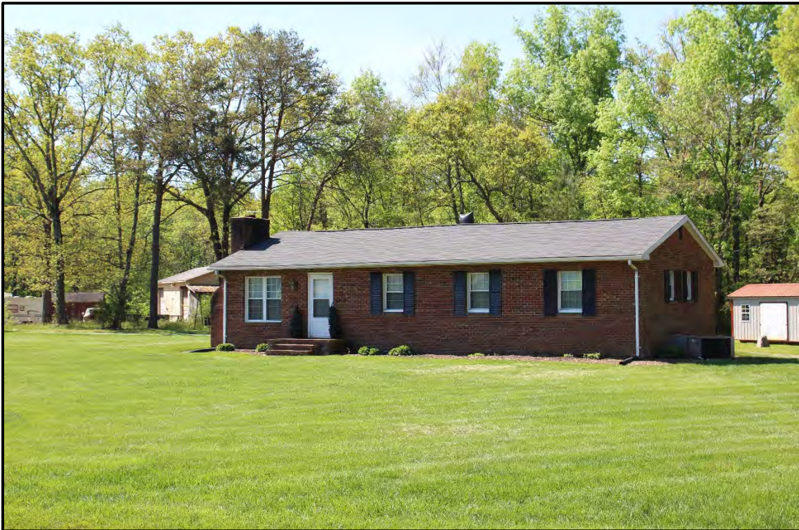
Figure 4.16. Architectural resource AM2654; view is south featuring the façade and northwest elevation.
