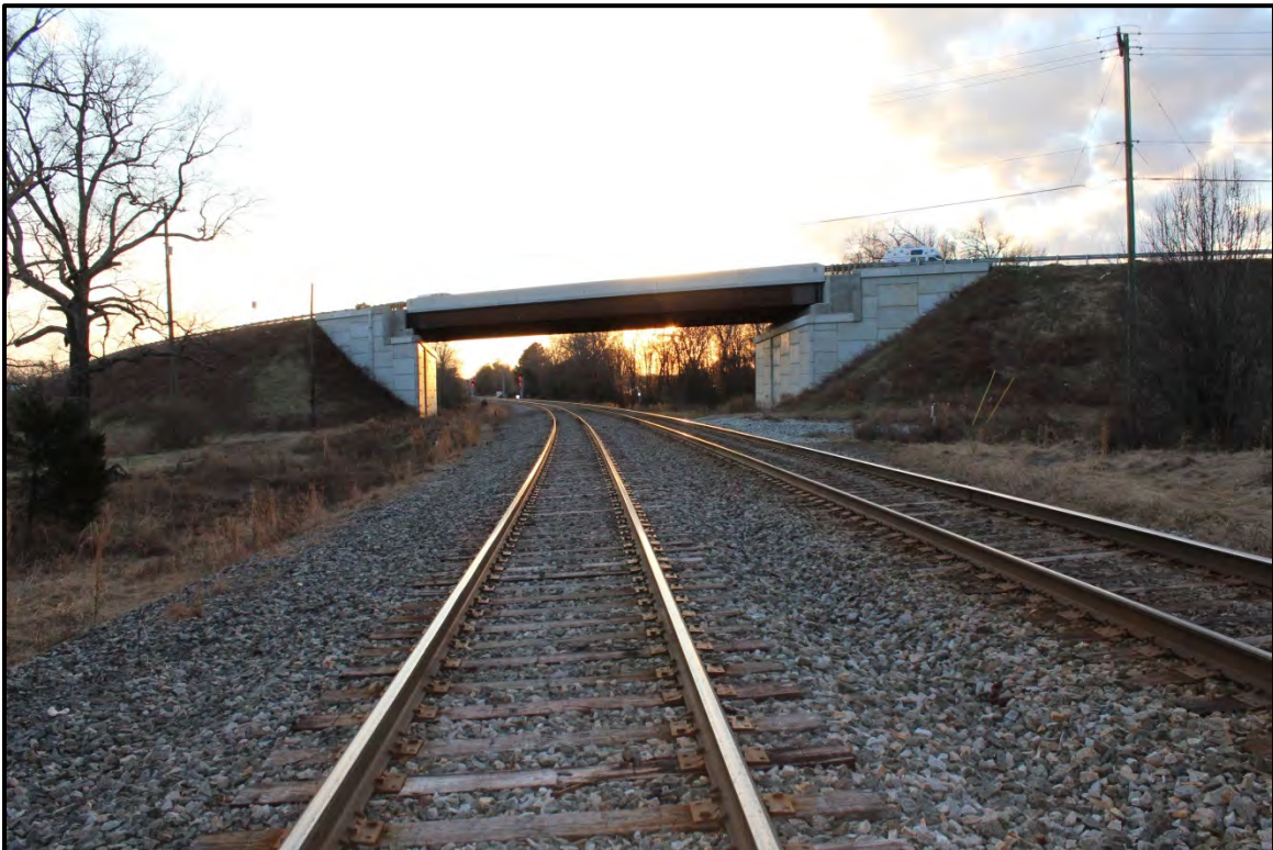
Figure 3.25. Architectural resource GF9116 along the eastern border of CY-09; view is southwest.
