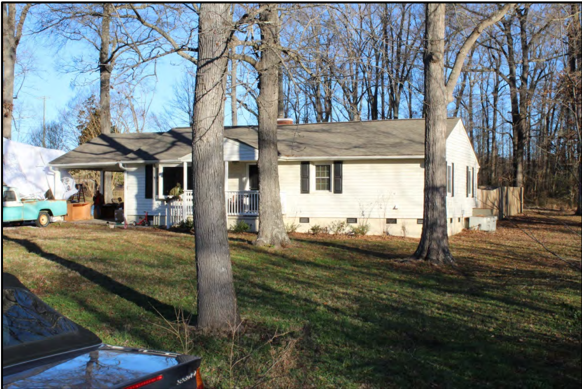
Figure 3.36. Architectural resource GF9119; view is northeast featuring the façade and west elevation.
