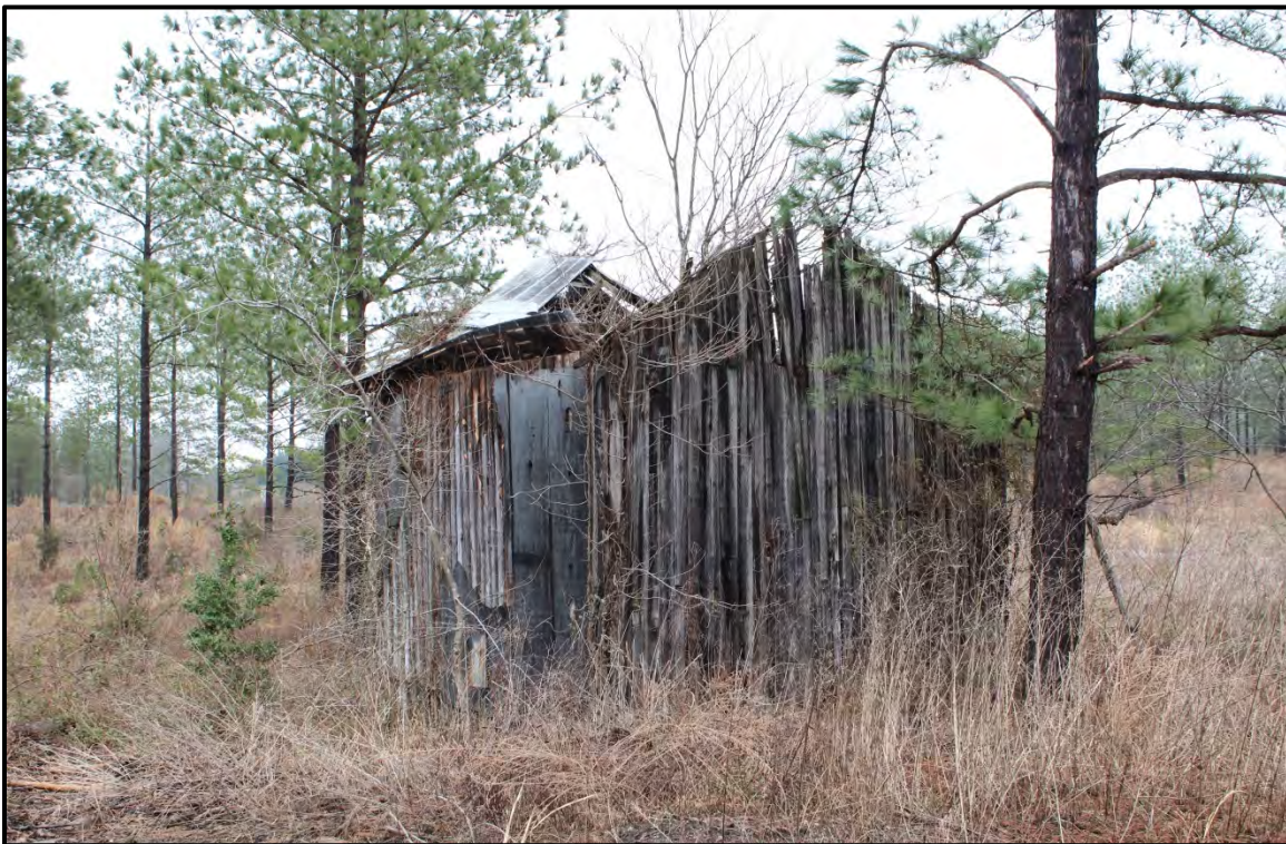
Figure 2.4. Architectural resource RK1086; view is southeast featuring the north (primary) and west elevations.
