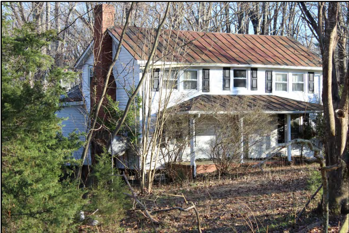
Figure 2.68. Architectural resource RK1798; view is southeast featuring the façade and north elevation.
