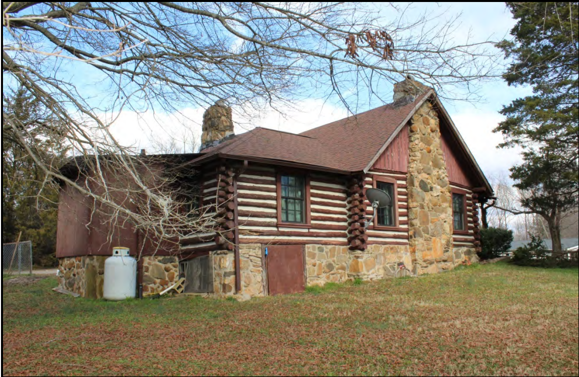
Figure 2.61. Architectural resource RK1820; view is northeast and features the façade and south elevation.
