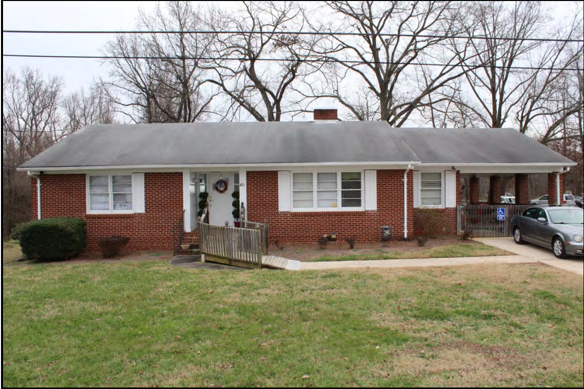
Figure 2.151. Architectural resource RK1815; view is east and features the façade.
