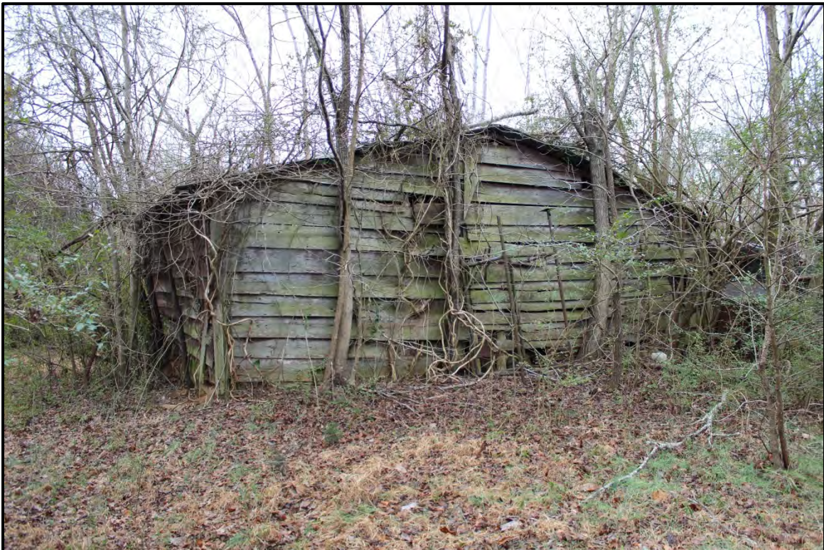
Figure 2.86. Architectural resource RK1818; view is northwest featuring the equipment shed.
