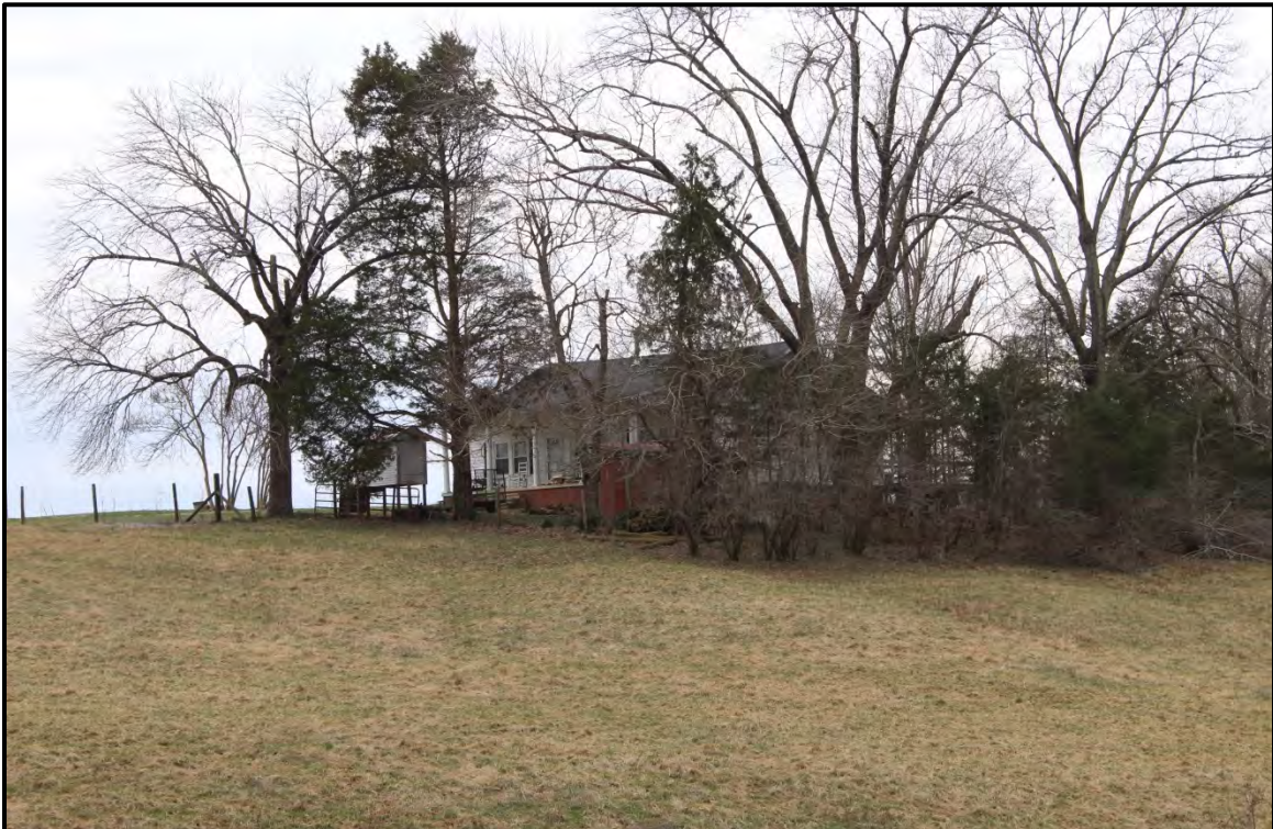
Figure 4.167. Architectural resource AM2650; view is southwest featuring the façade and north elevation of the primary residence.
