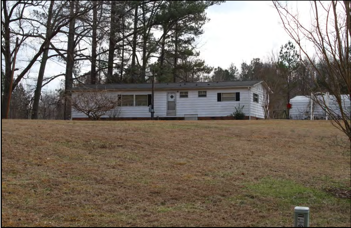
Figure 4.58. Architectural resource AM2629; view is south featuring the north and west (rear) elevations of the ca. 1952 house.
