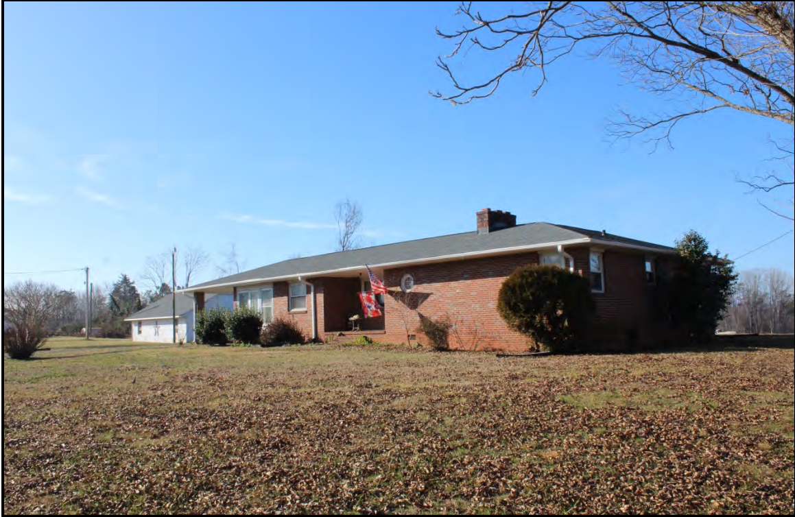
Figure 2.69. Architectural resource RK1799; view is northeast featuring the façade and south elevation.
