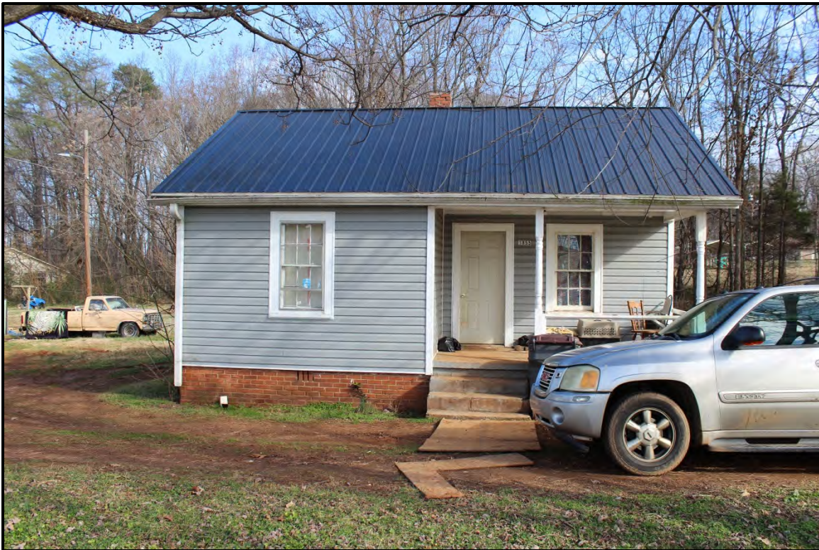
Figure 2.124. Architectural resource RK1807; view is east and features the façade.
