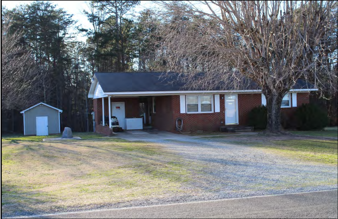
Figure 4.56. Architectural resource AM2643; view is northwest featuring the façade and south elevation of the house and associated storage shed.
