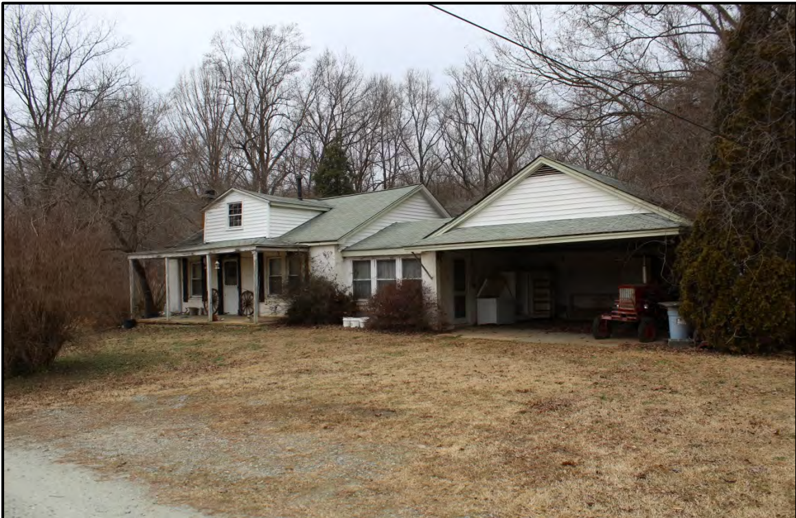
Figure 4.139. Architectural resource AM2645; view is northwest featuring the façade and east elevation garage wing.
