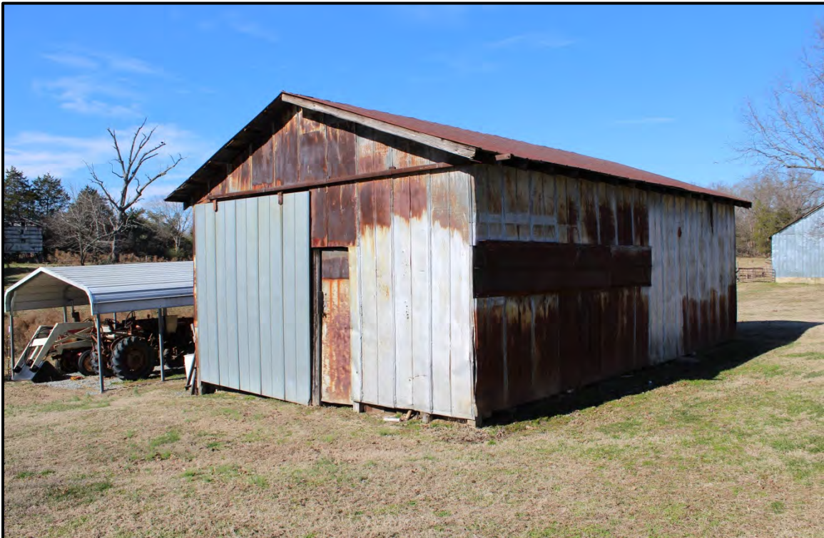
Figure 4.113. Architectural resource AM2635; view is northwest featuring the tractor shed and a modern carport.
