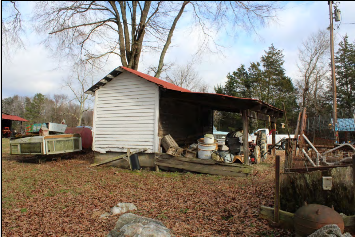
Figure 4.86. Architectural resource AM2631; view is northeast featuring the west (rear) of the single-bay garage and the open shed-roof extension attached to the south elevation.
