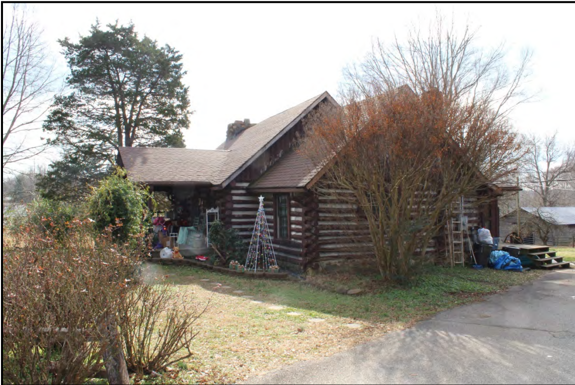
Figure 2.60. Architectural resource RK1820; view is southeast and features the façade and north elevation.
