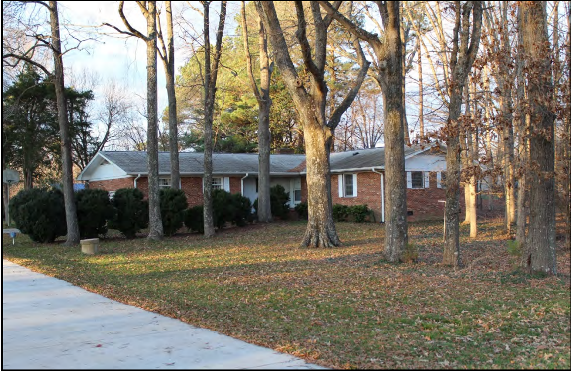
Figure 3.16. Architectural resource GF9112; view is northeast featuring the façade and west elevation.
