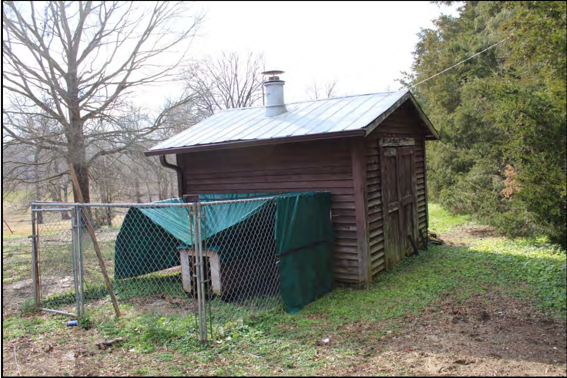
Figure 2.63. Architectural resource RK1820; view is east and features the ca. 1985 storage shed.
