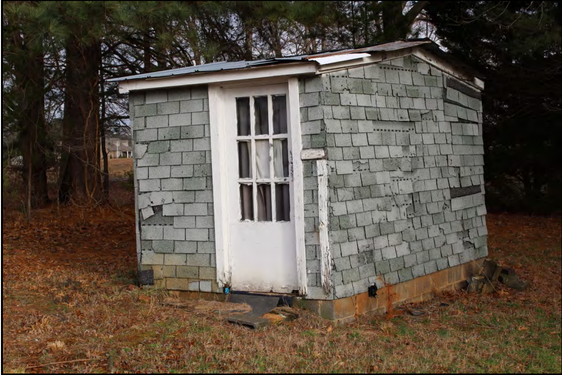
Figure 4.96. Architectural resource AM2631; view is northeast featuring the west and south elevations of the modern well house.
