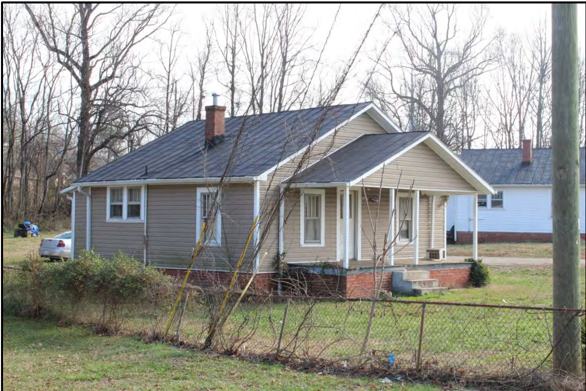
Figure 2.119. Architectural resource RK1805; view is southeast and features the façade and north elevation.
