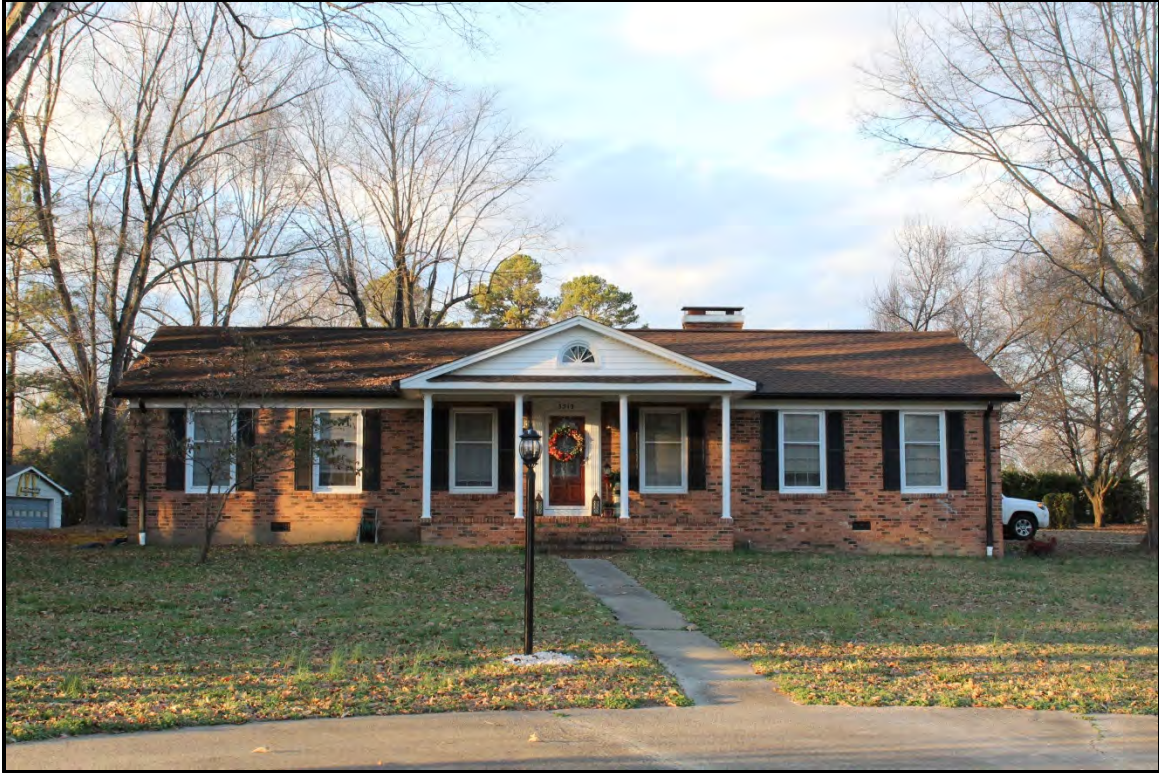
Figure 3.18. Architectural resource GF9113; view is north featuring the façade.
