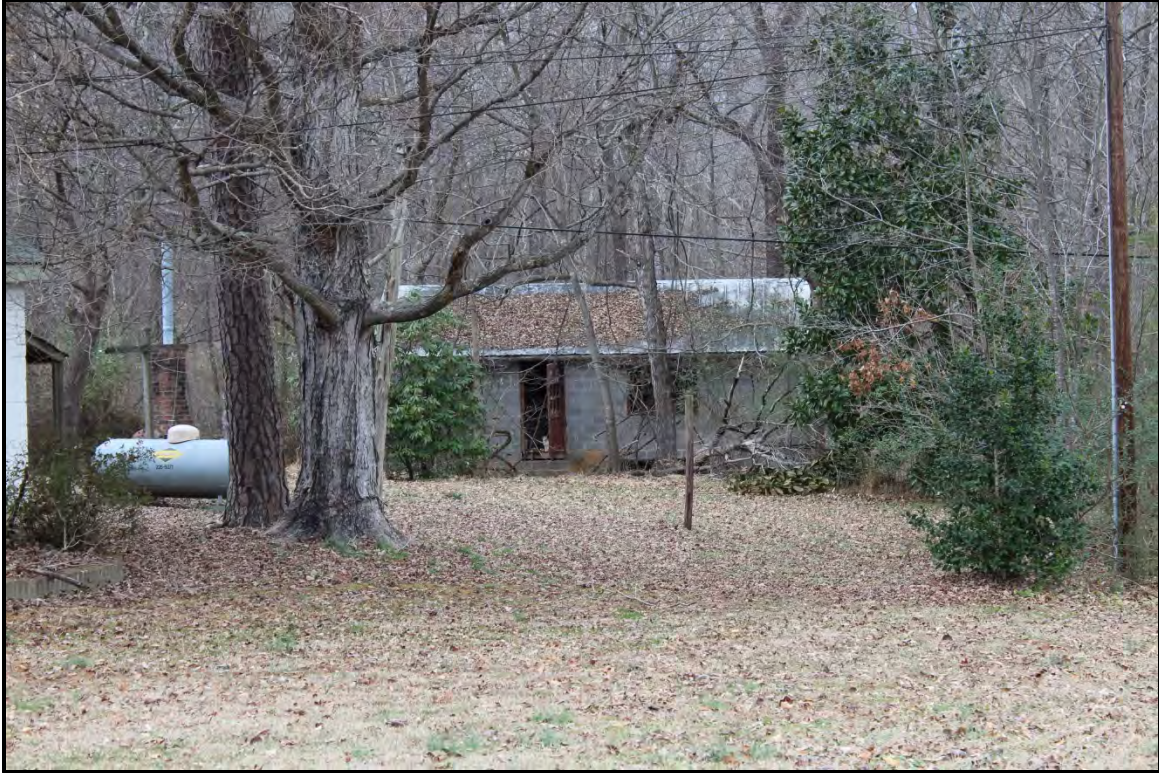
Figure 4.140. Architectural resource AM2645; view is north featuring the concrete block utility building.
