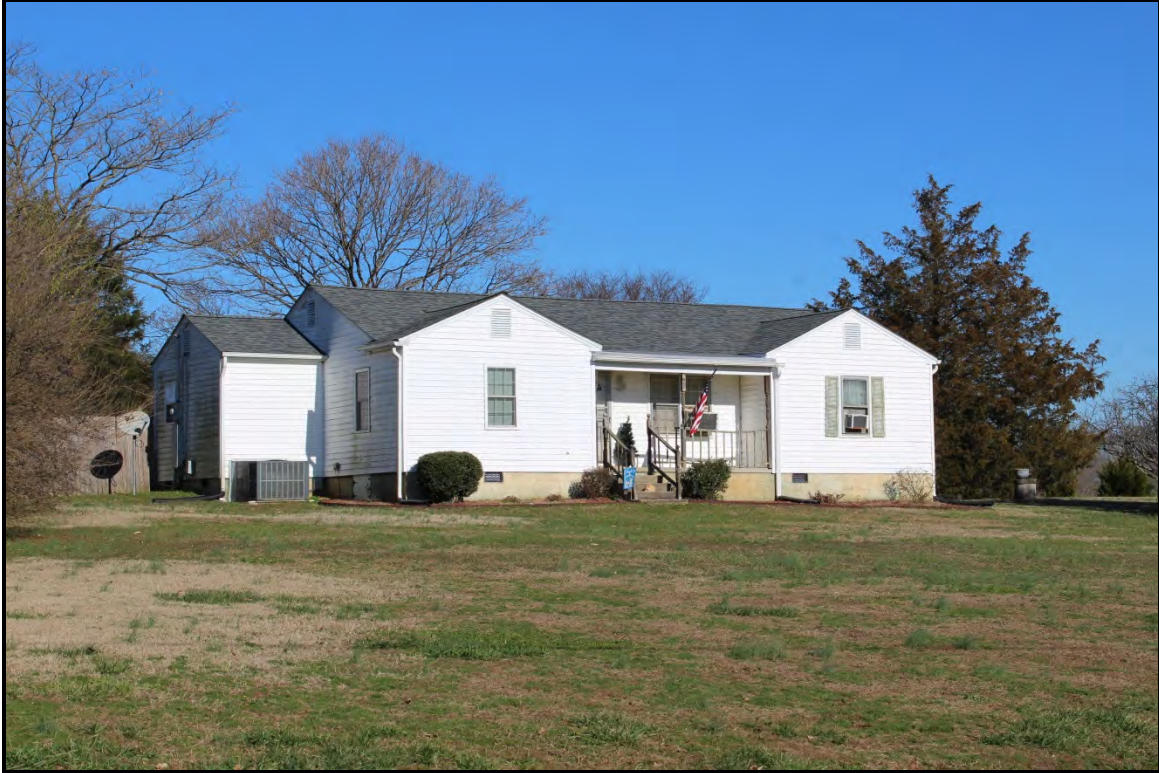
Figure 4.20. Architectural resource AM2623; view is southeast featuring the façade.
