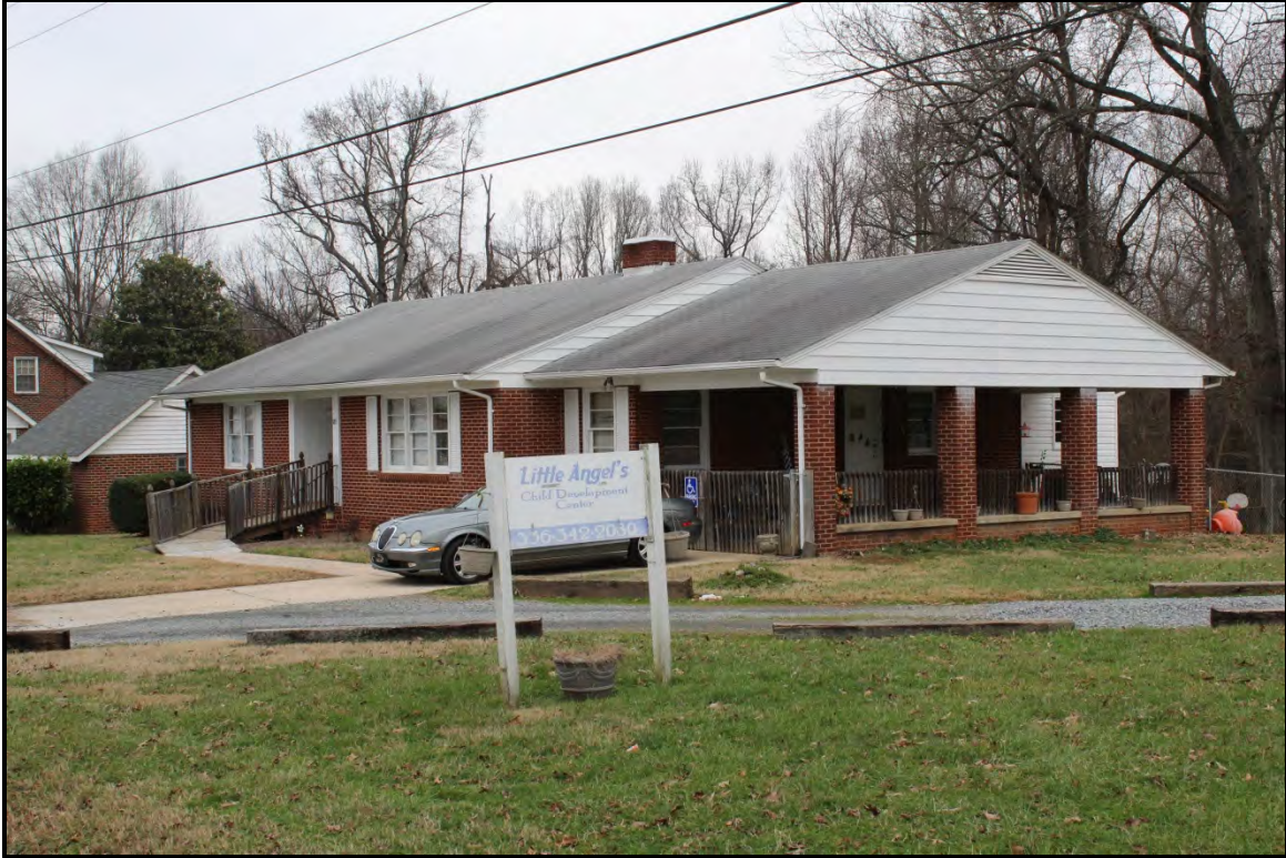
Figure 2.153. Architectural resource RK1815; view is northeast and features the façade and south elevation.
