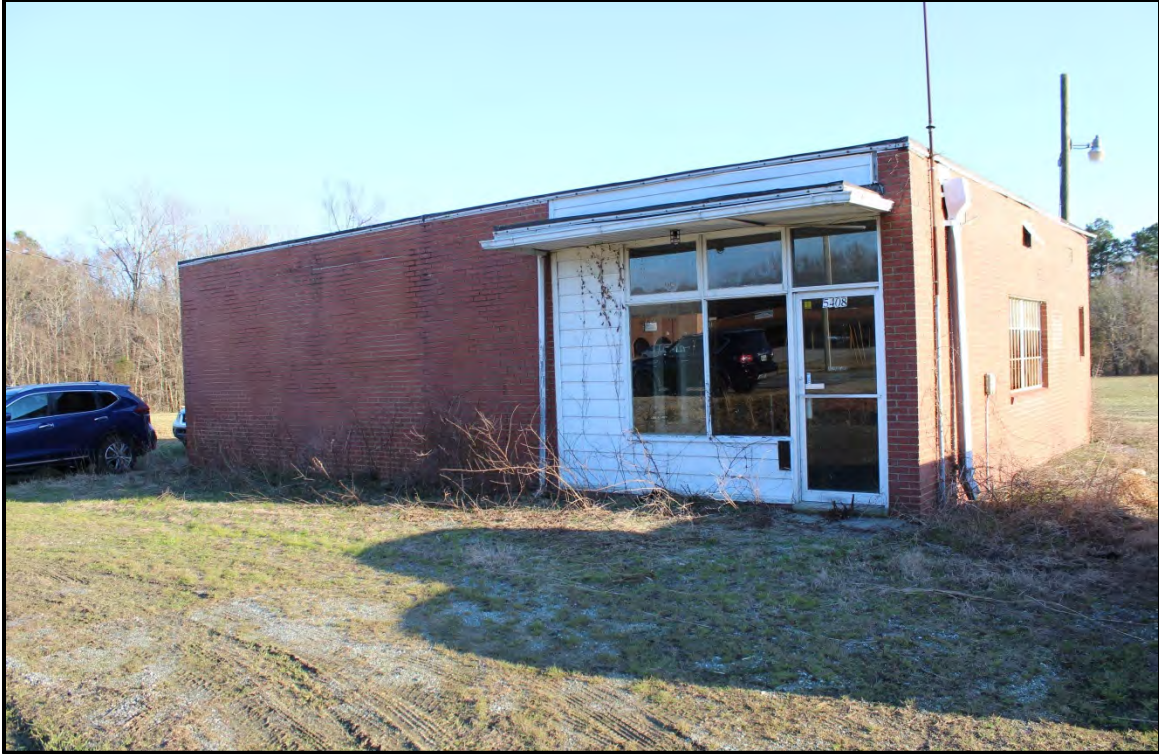
Figure 3.22. Architectural resource GF9115; view is southeast featuring the façade and west elevation.
