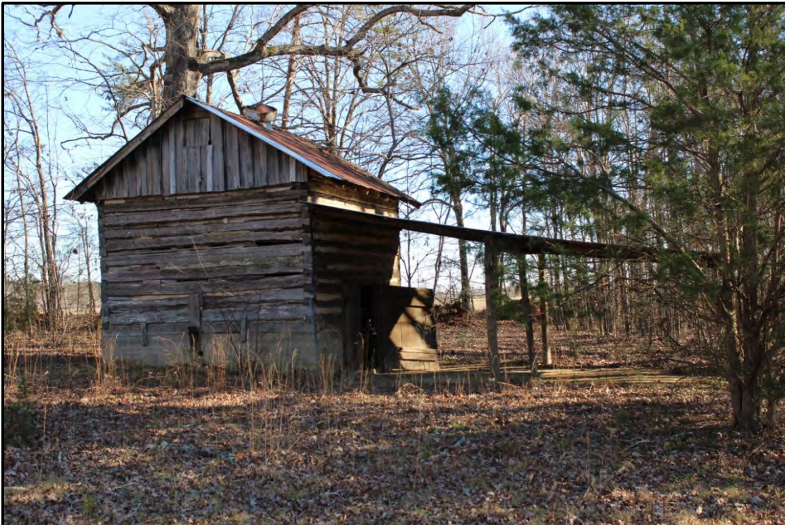
Figure 4.33. Architectural resource AM0209; view is northwest featuring the east and south elevations of the tobacco barn.
