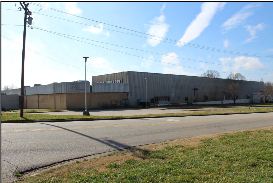
Figure 2.111. Architectural resource RK1803; view is southwest and features the north elevation of the manufacturing building.
