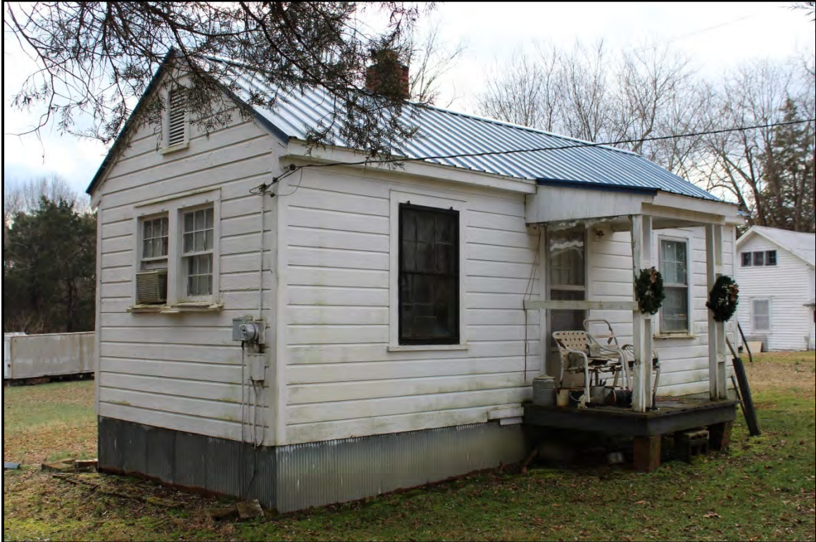
Figure 4.81. Architectural resource AM2631; view is southwest featuring the façade and east elevation of the ca. 1957 side-gabled house.
