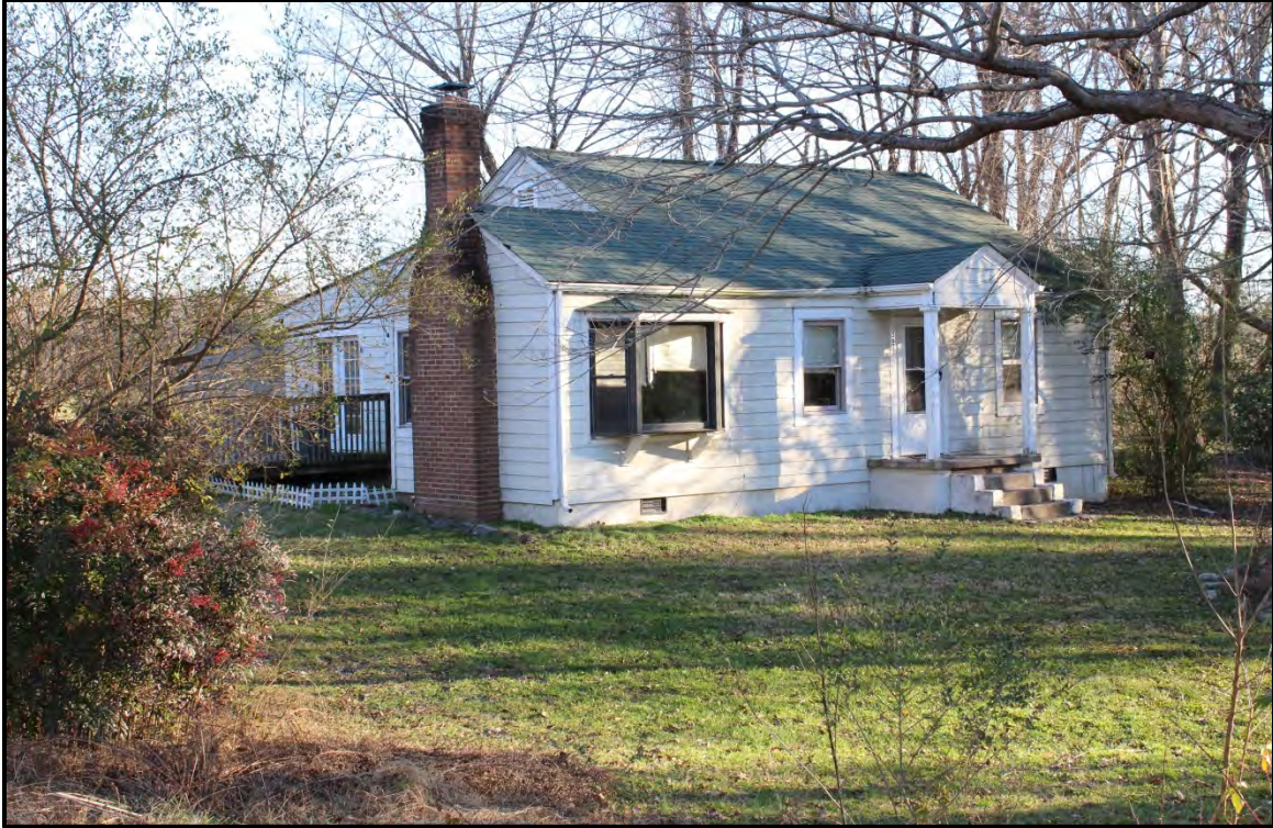
Figure 3.28. Architectural resource GF9117; view is northeast featuring the façade and west elevation.
