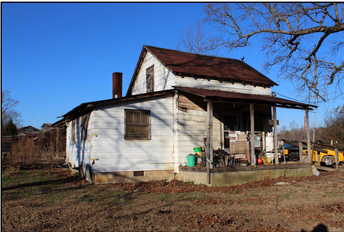
Figure 2.32. Architectural resource RK1792 farmhouse; view is northwest featuring the façade and south elevation.
