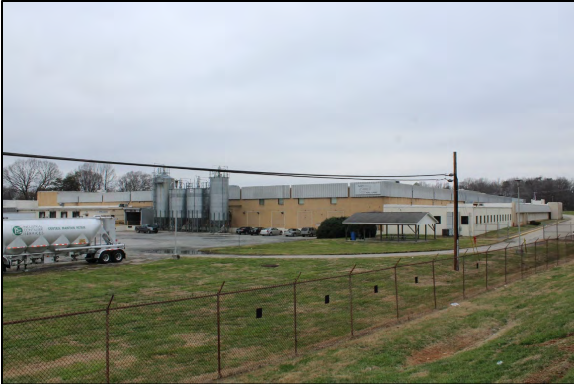
Figure 2.112. Architectural resource RK1803; view is northwest and features the south elevation of the manufacturing building, the storage silos, and the picnic shelter.
