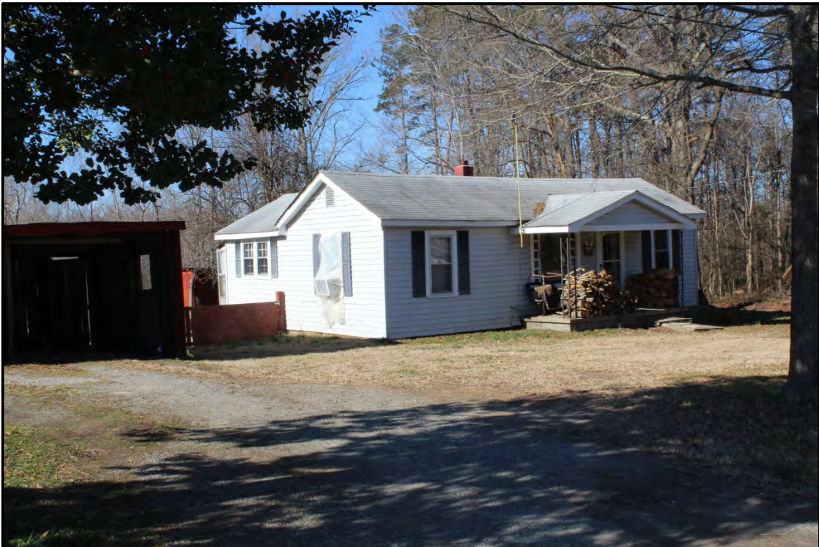
Figure 2.9. Architectural resource RK1785; view is northwest featuring the façade and the south elevation.
