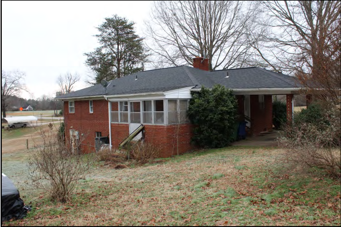
Figure 2.75. Architectural resource RK1818 farmhouse; view is southeast featuring the east and north (rear) elevations.
