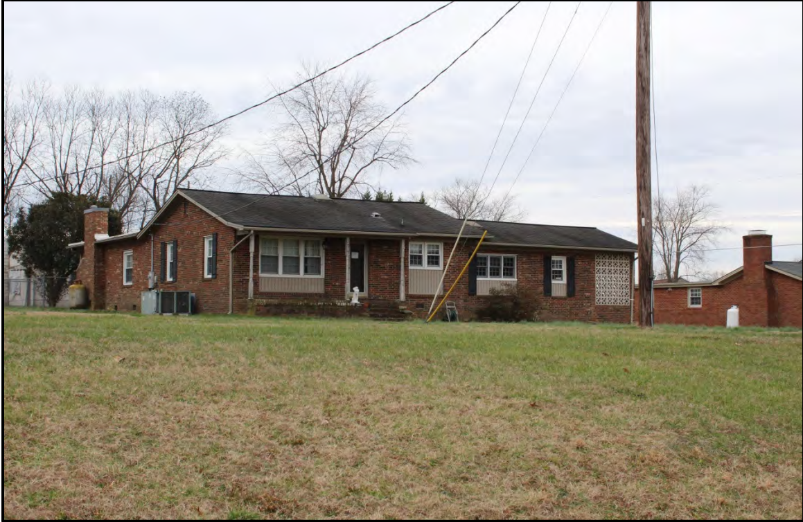
Figure 4.50. Architectural resource AM2640; view is southwest featuring the façade and east elevation.
