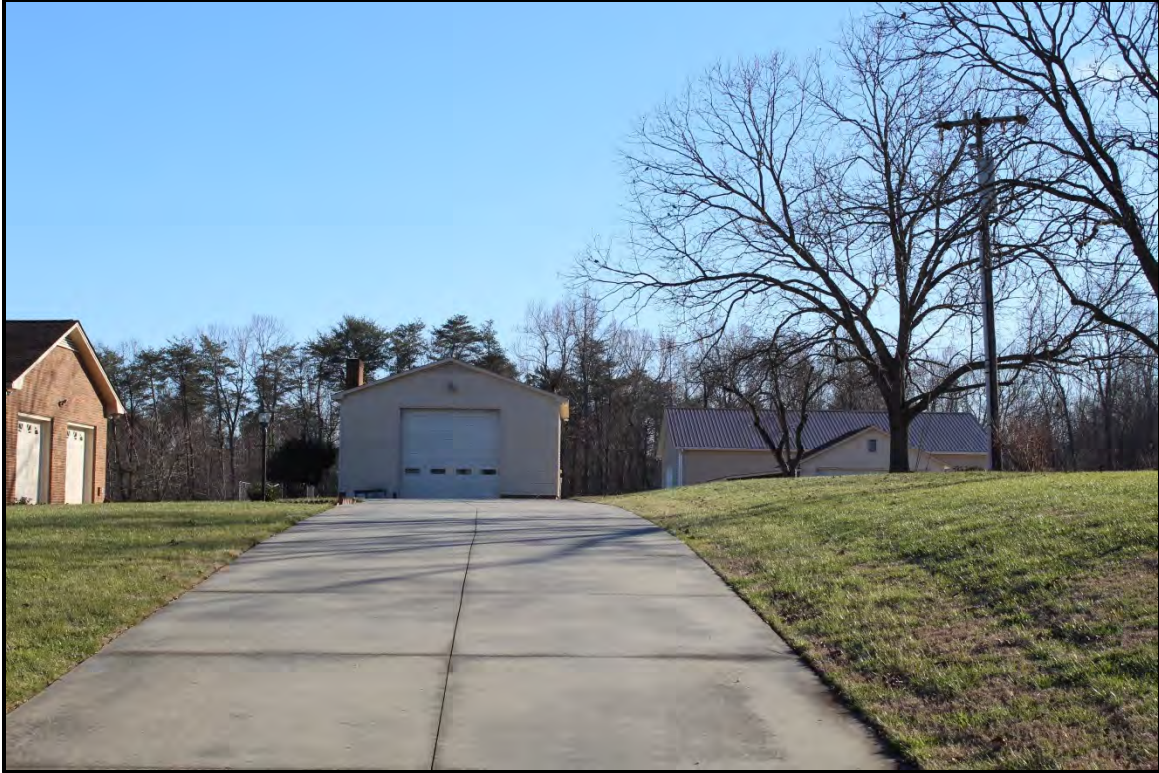
Figure 4.36. Architectural resource AM2626; view is south featuring the modern garage and workshop building.
