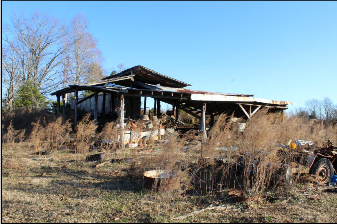
Figure 2.37. Architectural resource RK1792 ca. 1970 pole shed; view is north.
