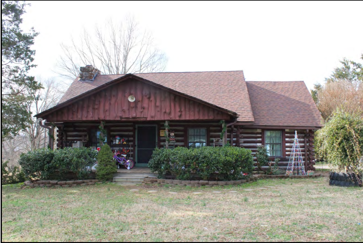
Figure 2.59. Architectural resource RK1820; view is east and features the façade.
