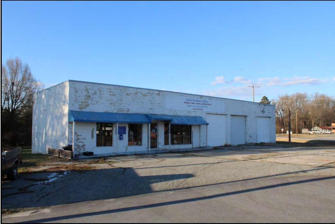
Figure 3.5. Architectural resource GF9108; view is southeast featuring the façade and west elevation.
