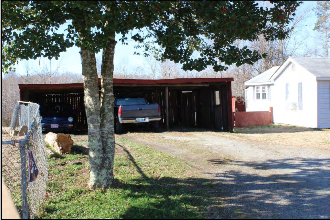
Figure 2.10. Architectural resource RK1785; view is west featuring the vehicle shed.
