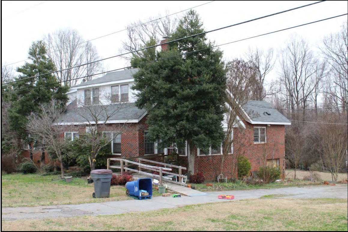
Figure 2.156. Architectural resource RK1816; view is northeast and features the façade and south elevation.
