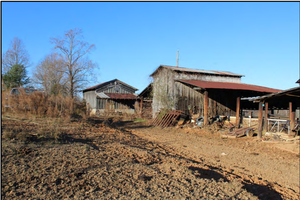
Figure 2.38. Architectural resource RK1792; view is west featuring the mid-twentieth century storage building.
