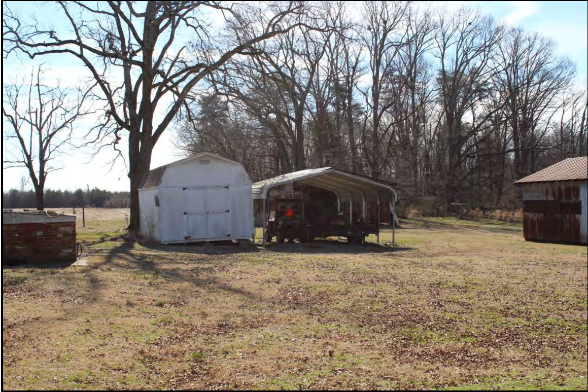
Figure 4.110. Architectural resource AM2635; view is west featuring a modern carport, a prefabricated storage shed, and the pump shed.
