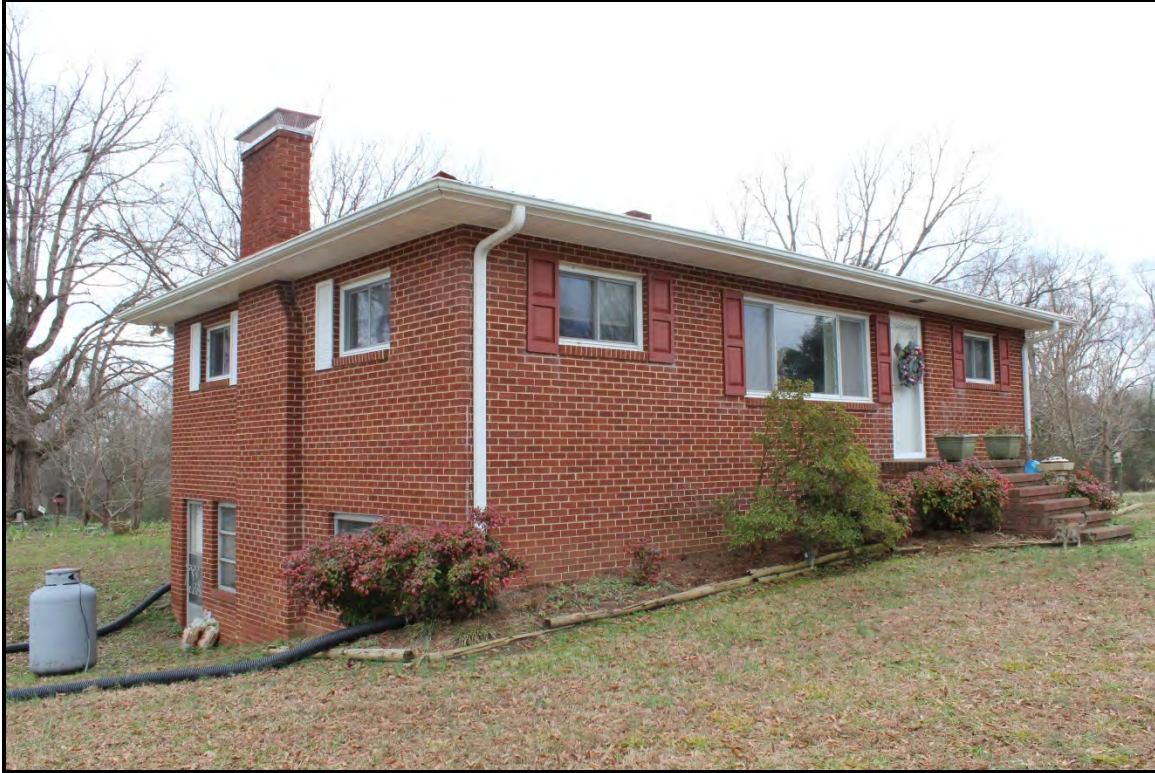
Figure 4.98. Architectural resource AM2652; view is southwest featuring the façade and east elevation of the farmhouse.
