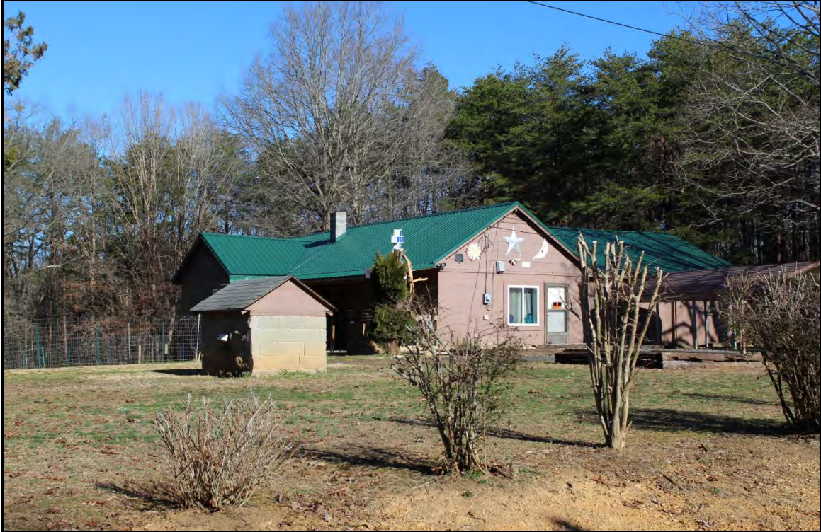
Figure 2.20. Architectural resource RK1788; view is northeast featuring the façade and the south elevation of the house with the pump shed in the foreground.
