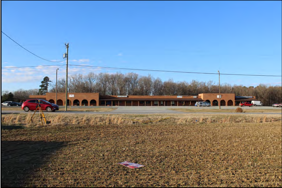
Figure 3.1. Architectural resource GF1536; view is north featuring the primary façade.
