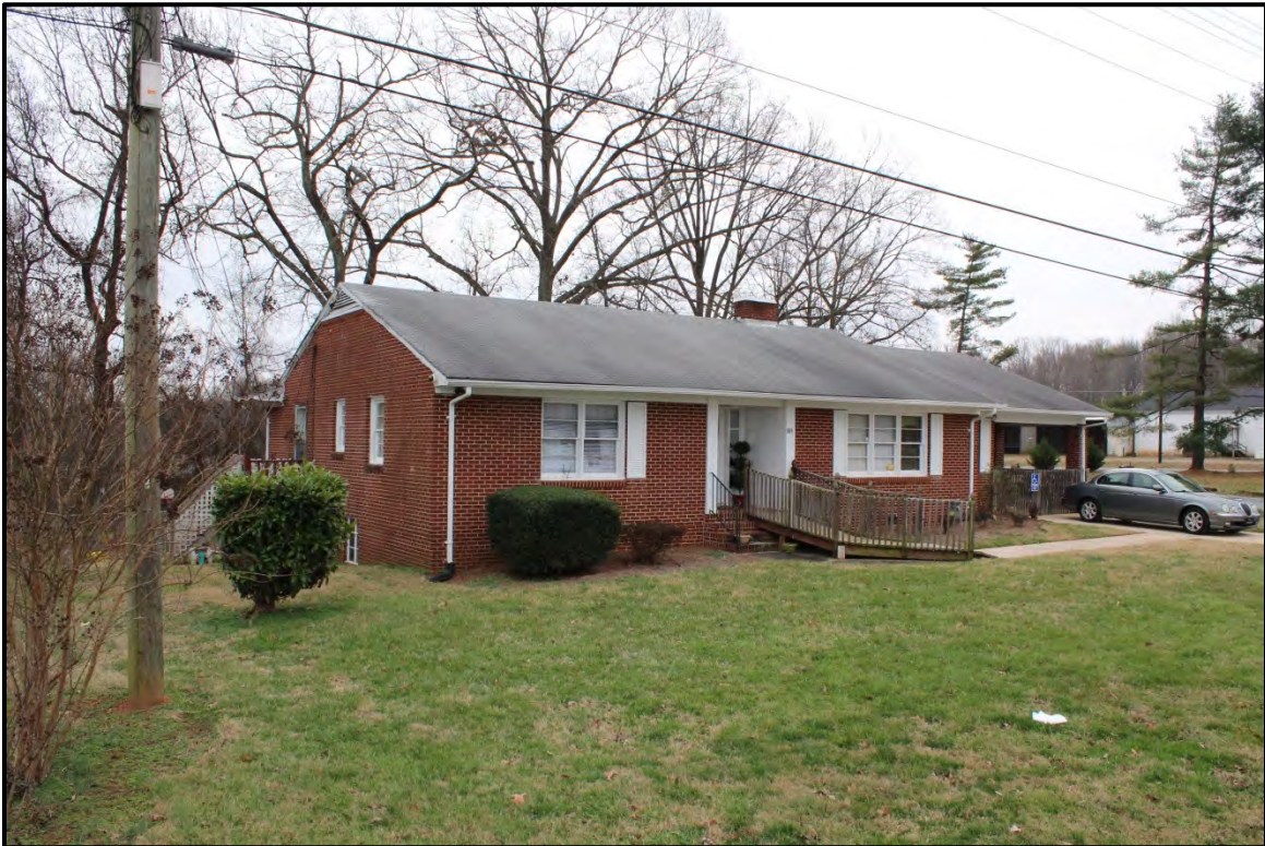
Figure 2.152. Architectural resource RK1815; view is southeast and features the façade and north elevation.
