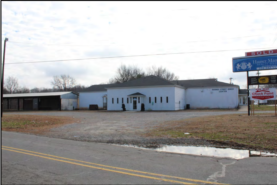
Figure 2.149. Architectural resource RK1814; view is south and features the hipped-roof addition to the north elevation.
