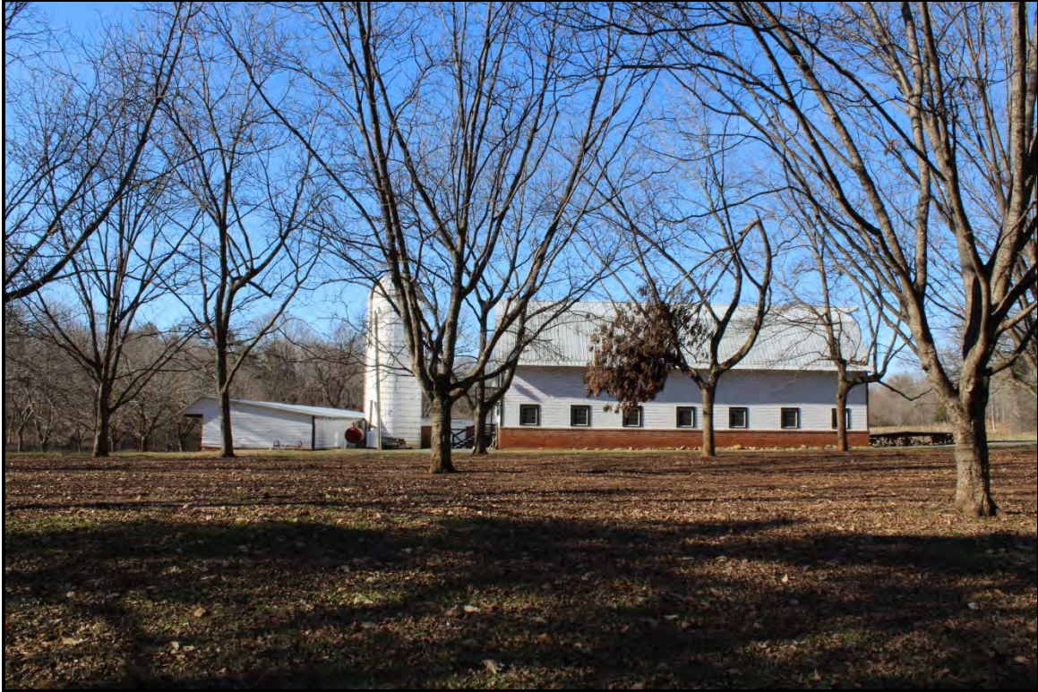
Figure 2.104. High Rock Farm; view is west featuring a barn, silo, and equipment shed.
