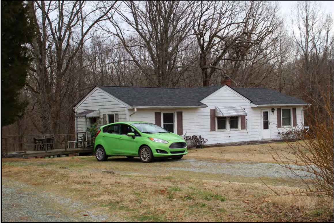
Figure 4.158. Architectural resource AM2647; view is southeast featuring the façade and north elevation.
