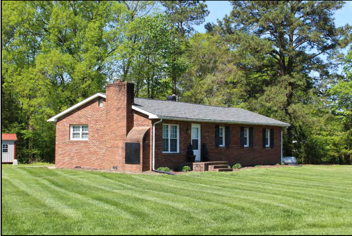
Figure 4.15. Architectural resource AM2654; view is west featuring the façade and southeast elevation.
