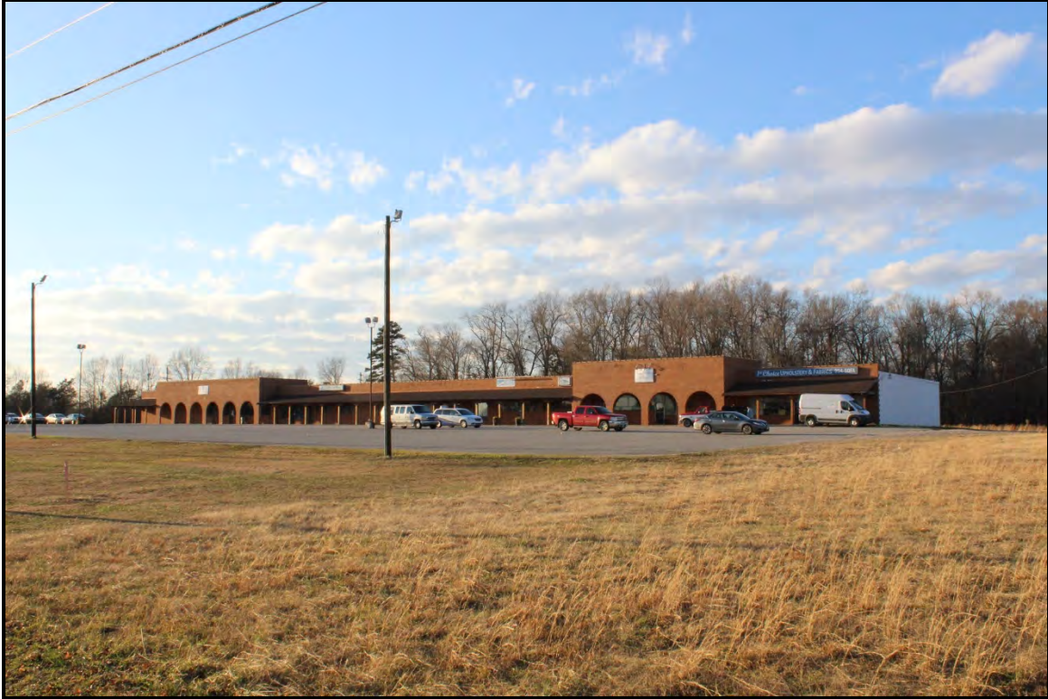
Figure 3.3. Architectural resource GF1536; view is northwest featuring the façade and east elevation wing.
