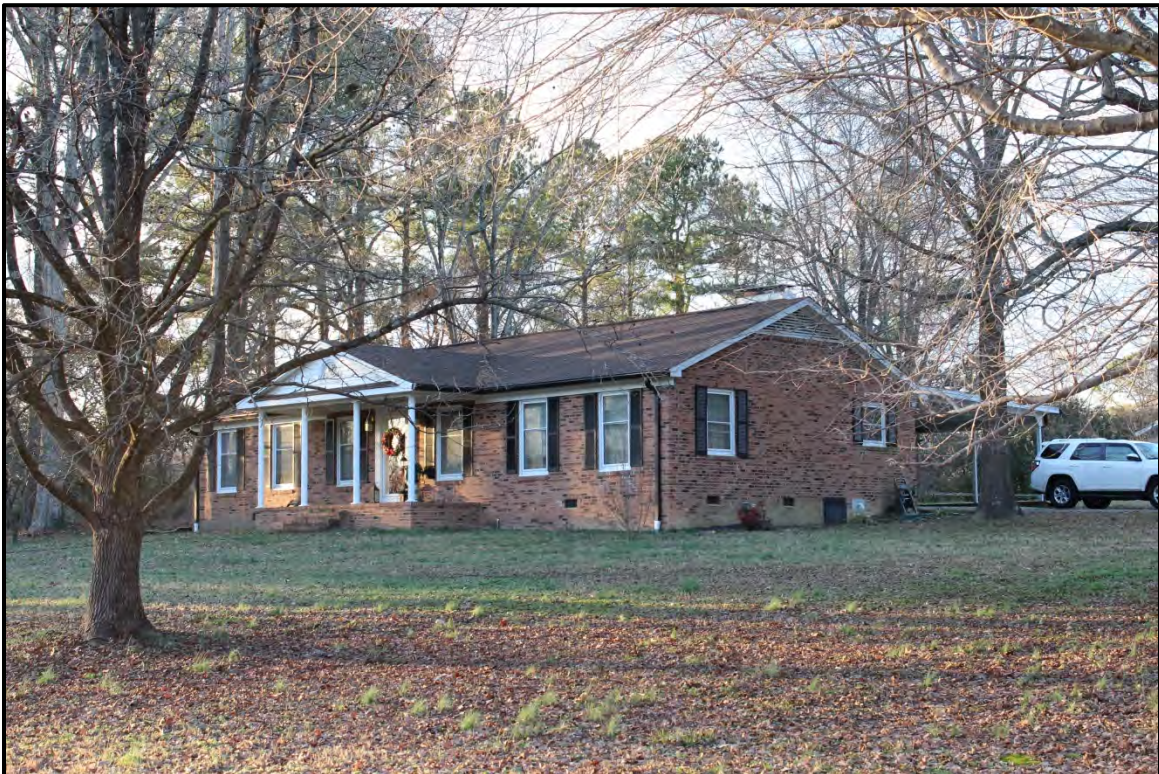
Figure 3.19. Architectural resource GF9113; view is northwest featuring the façade and east elevation.
