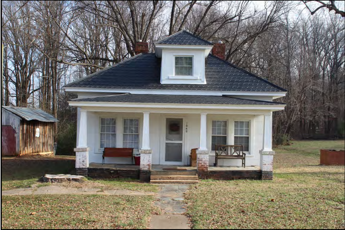
Figure 2.131. Architectural resource RK1809; view is east and features the façade and associated garage to the left.
