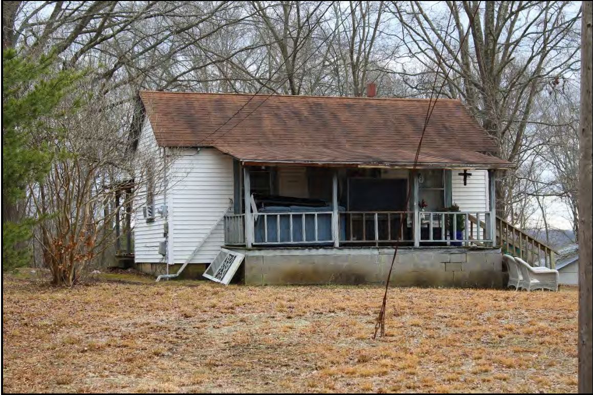
Figure 2.11. Architectural resource RK1821; view is southeast and features the façade and the northeast elevation.
