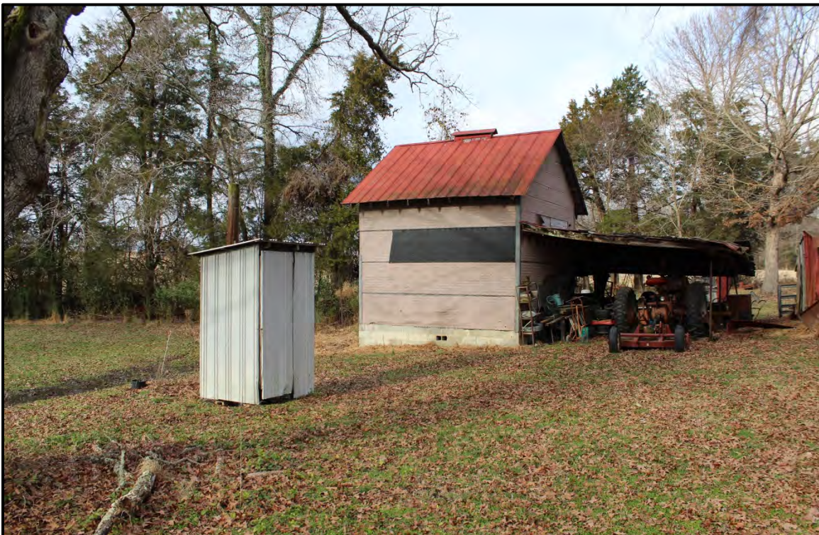
Figure 4.87. Architectural resource AM2631; view is northwest featuring the modern privy and the south and east elevations of the mid- to late twentieth century tobacco barn.
