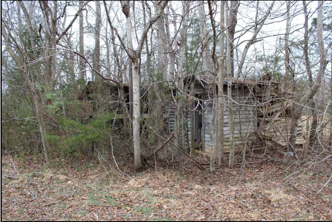
Figure 2.94. Architectural resource RK1819; view is northeast and features the equipment shed.
