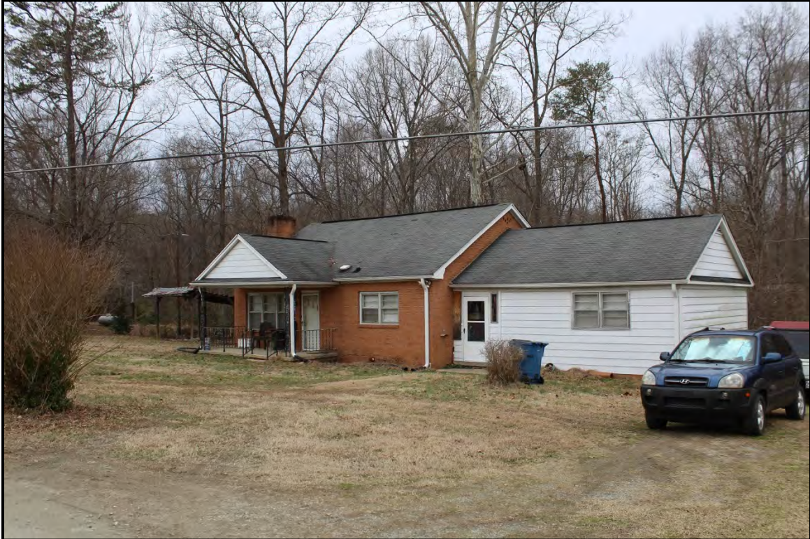
Figure 4.137. Architectural resource AM2646; view is northwest featuring the façade and east elevation garage wing.
