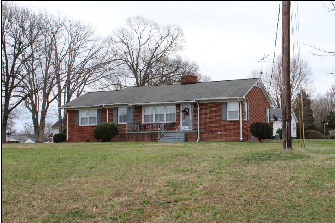
Figure 4.48. Architectural resource AM2639; view is southeast featuring the façade and west elevation.
