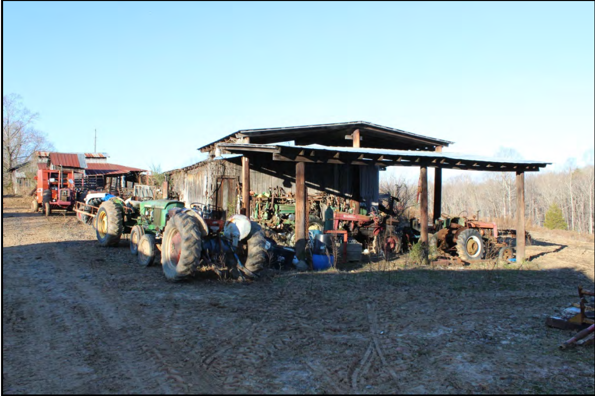
Figure 2.45. Architectural resource RK1792; view is west featuring the mid-twentieth century workshop and equipment shed.
