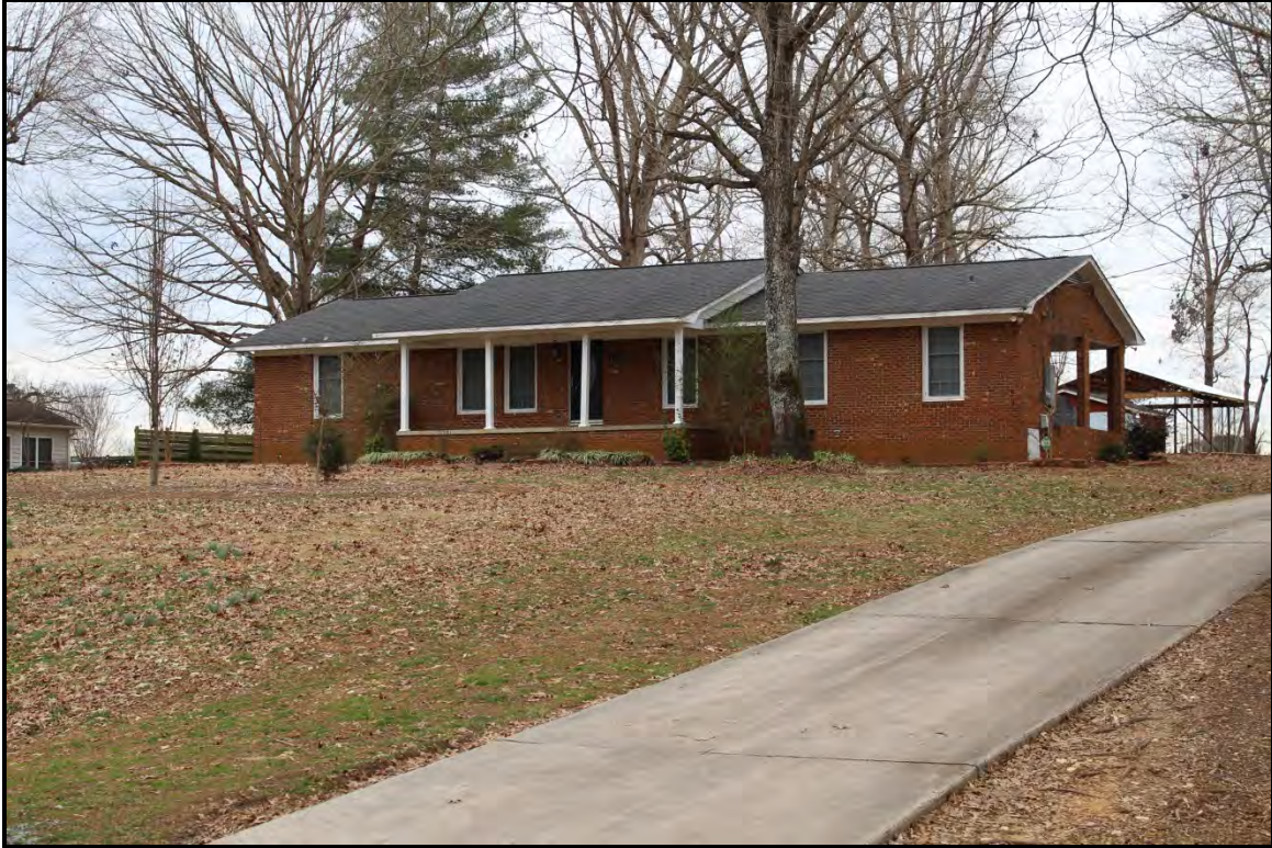
Figure 4.70. Architectural resource AM2637; view is southeast featuring the façade and west elevation.
