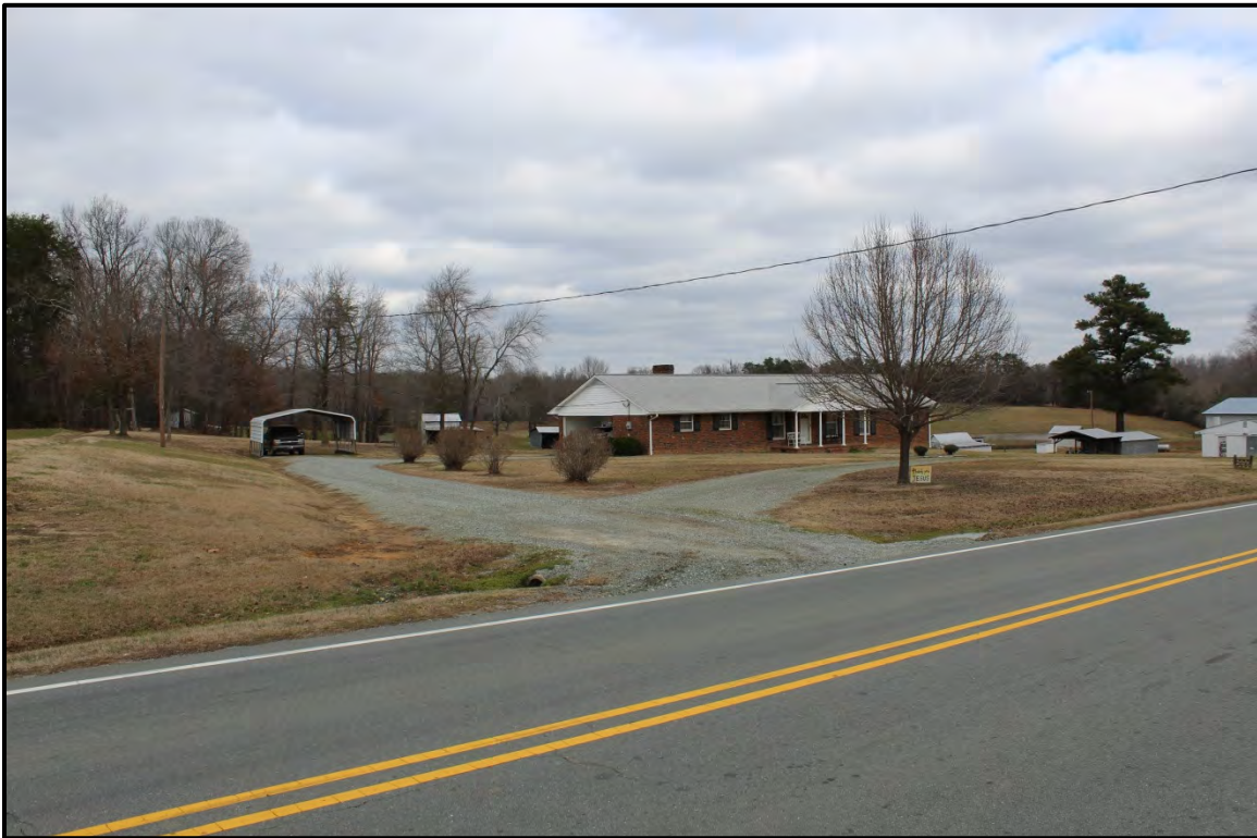
Figure 4.121. Architectural resource AM2633; view is northeast featuring the façade and west elevation of the residence and the modern carport.
