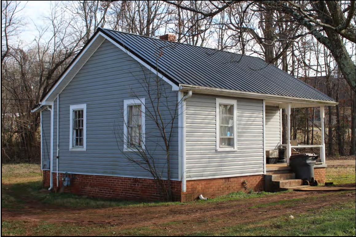
Figure 2.125. Architectural resource RK1807; view is southeast and features the façade and north elevation.
