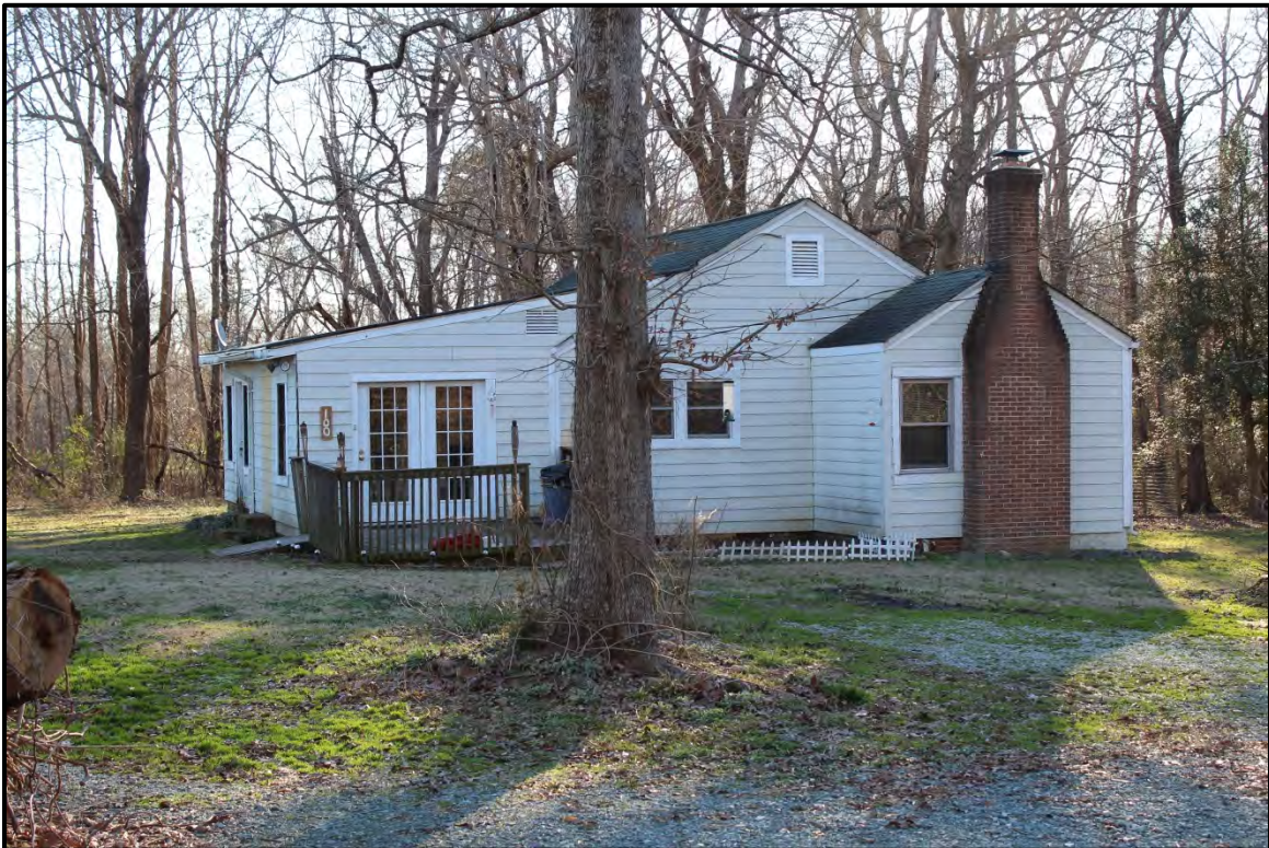
Figure 3.29. Architectural resource GF9117; view is southeast featuring the west and north (rear) elevations.
