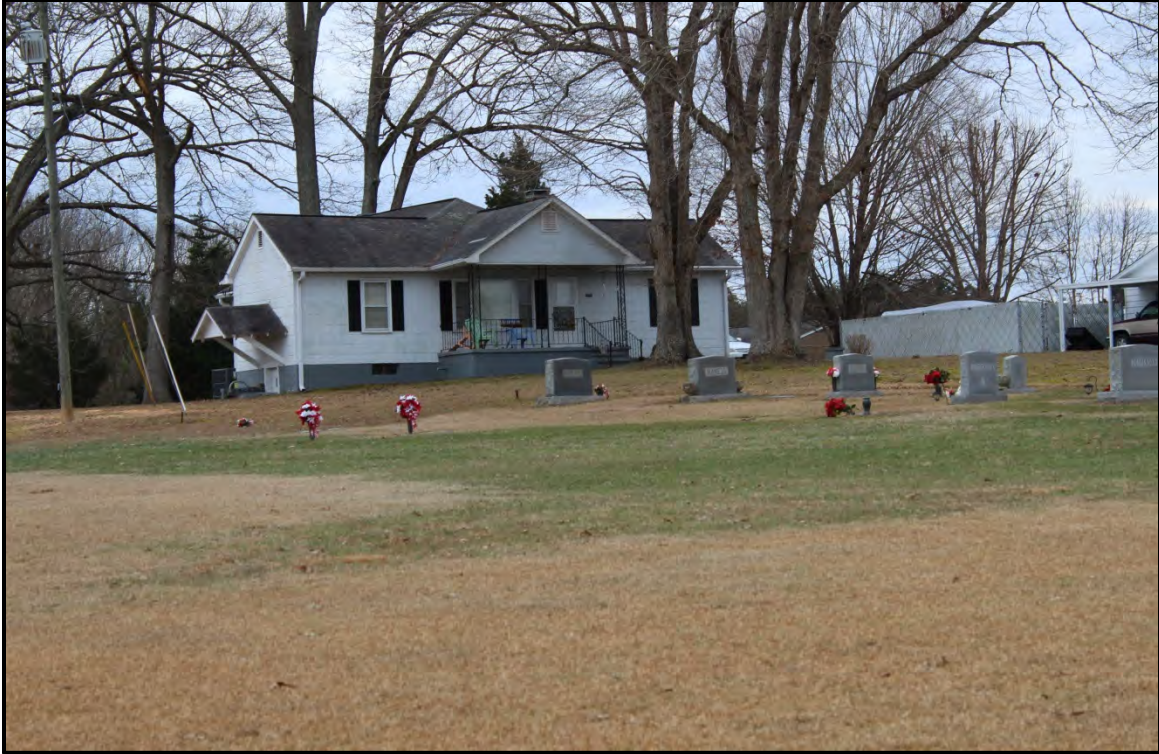
Figure 4.45. Architectural resource AM2638; view is southwest featuring the façade and east elevation.
