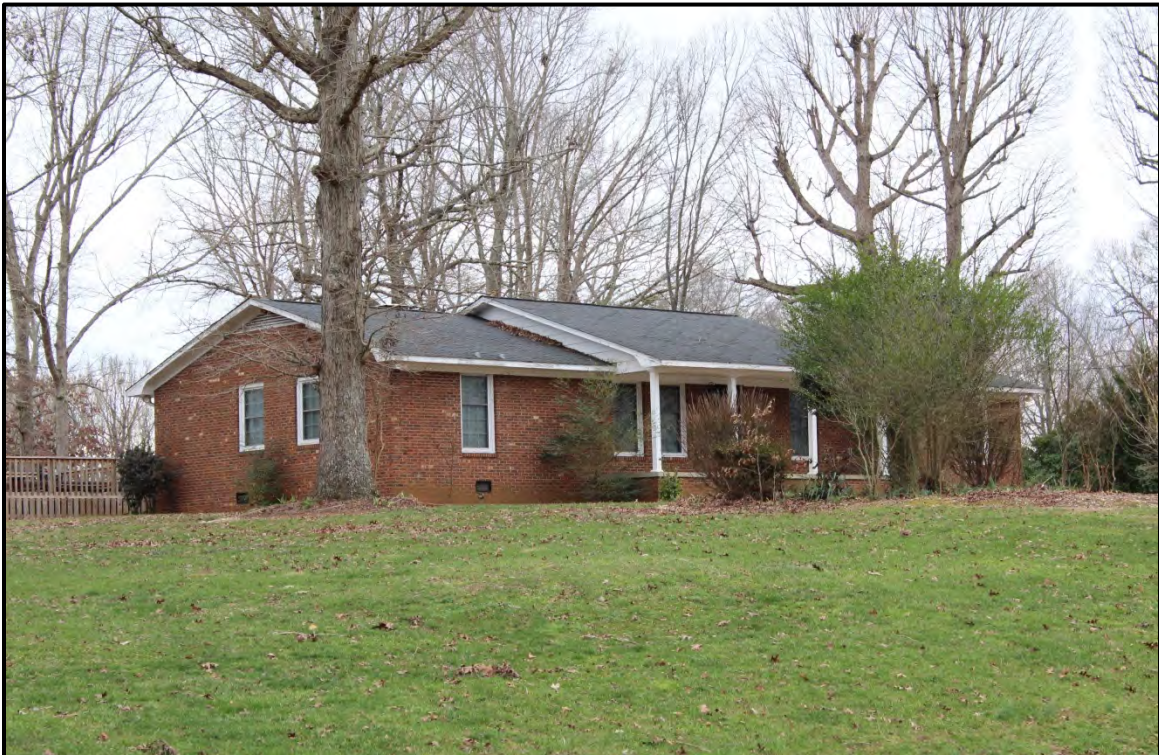
Figure 4.71. Architectural resource AM2637; view is southwest featuring the façade and east elevation.
