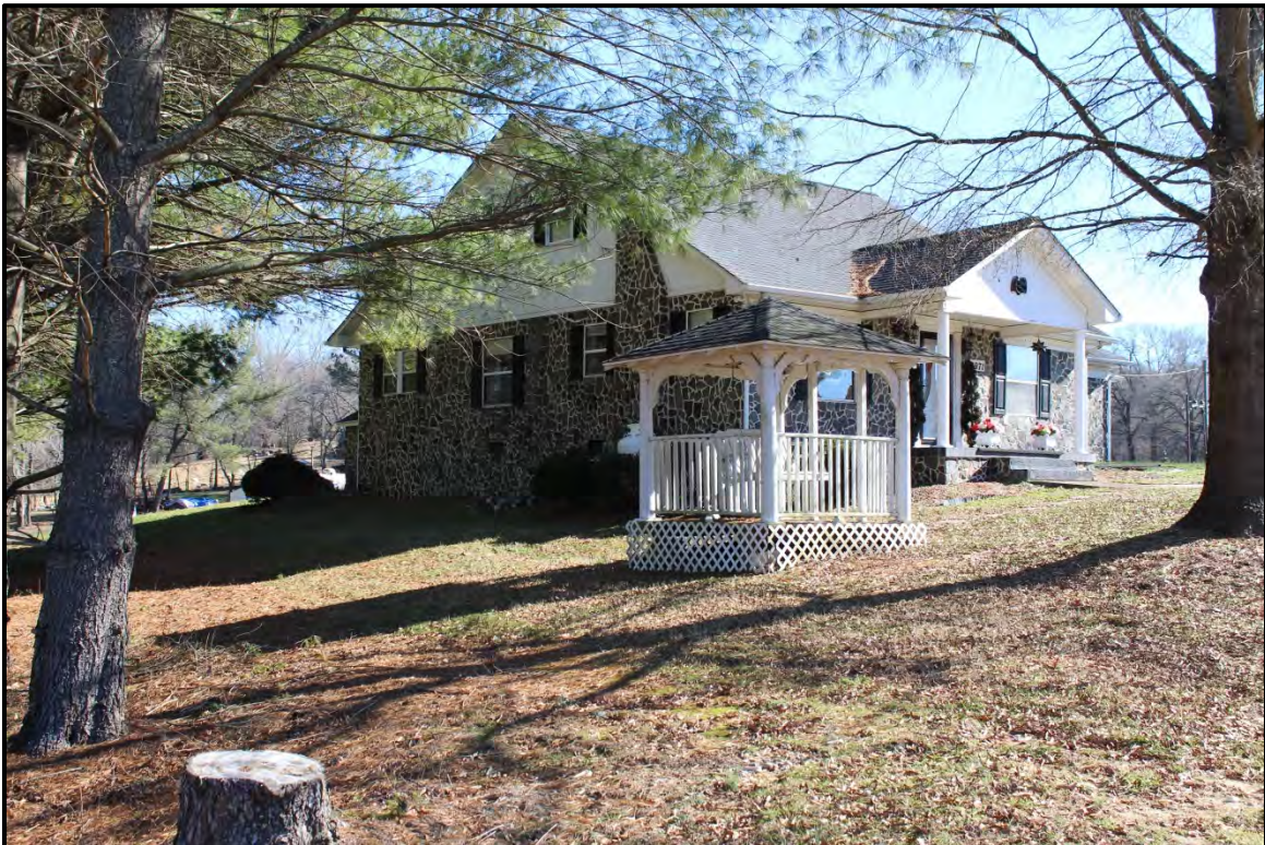
Figure 2.26. Architectural resource RK1790; view is southeast featuring the façade and the north elevation.
