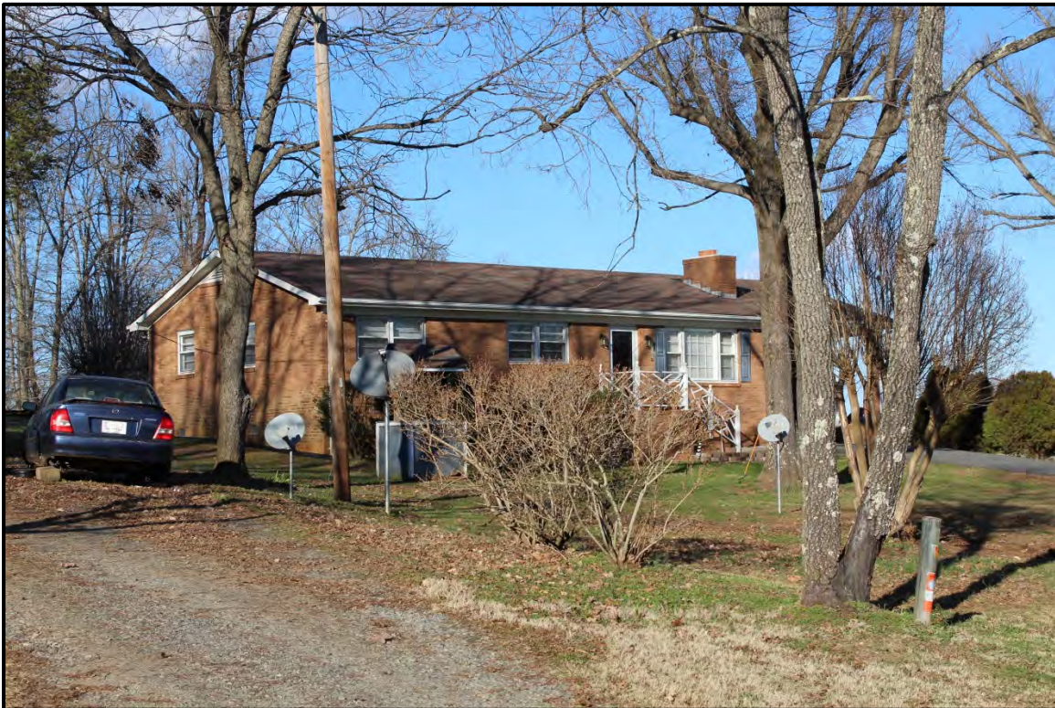
Figure 2.66. Architectural resource RK1797; view is northeast featuring the façade and west elevation.
