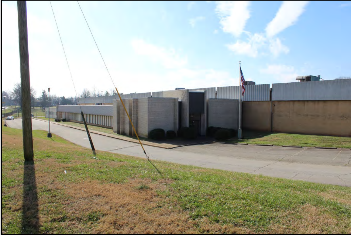
Figure 2.110. Architectural resource RK1803; view is southwest and features the office wing.
