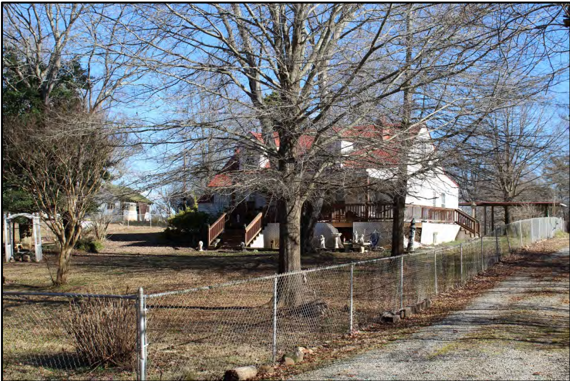
Figure 2.30. Architectural resource RK1791; view is northeast featuring the façade and the south elevation.
