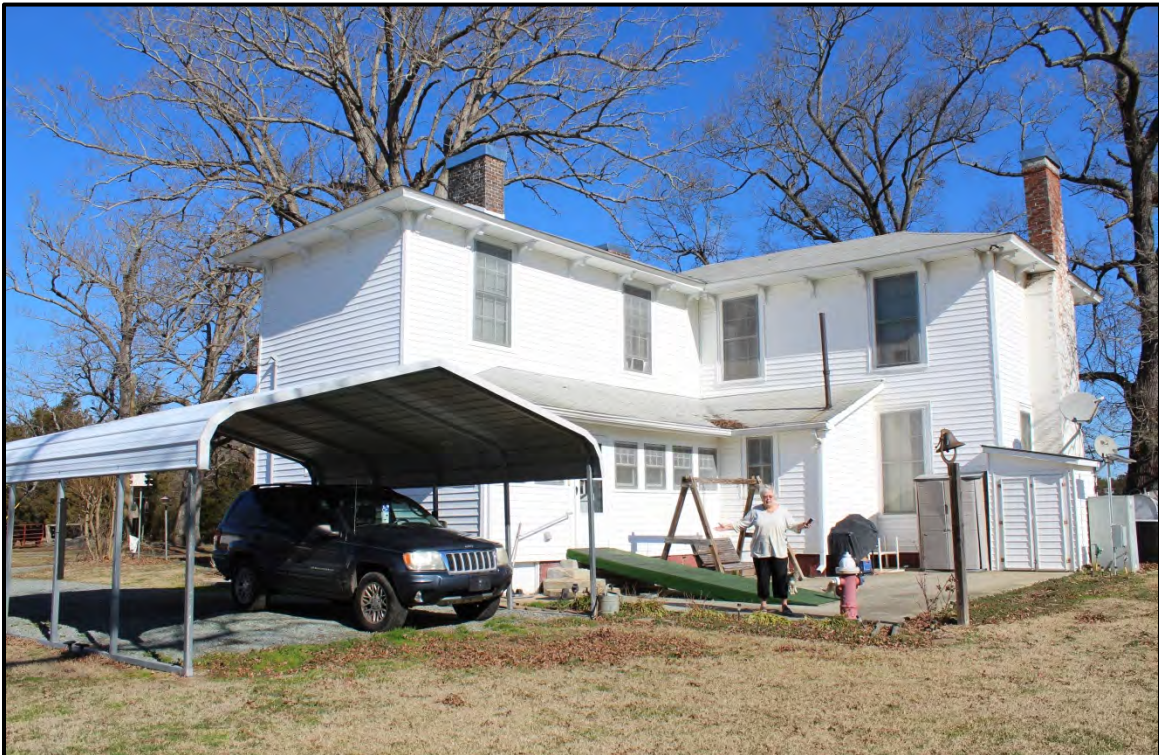
Figure 4.109. Architectural resource AM2635; view is northeast featuring the west (rear) elevation and a modern carport.
