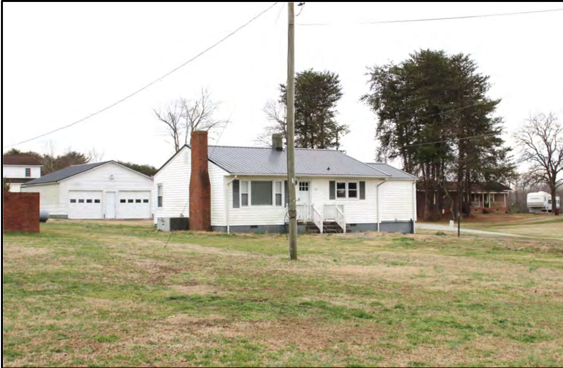
Figure 4.54. Architectural resource AM2642; view is southwest featuring the façade and east elevation of the house and associated garage.
