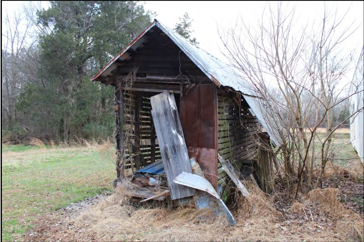
Figure 4.79. Architectural resource AM2631; view is southwest featuring the mid-twentieth century storage crib.
