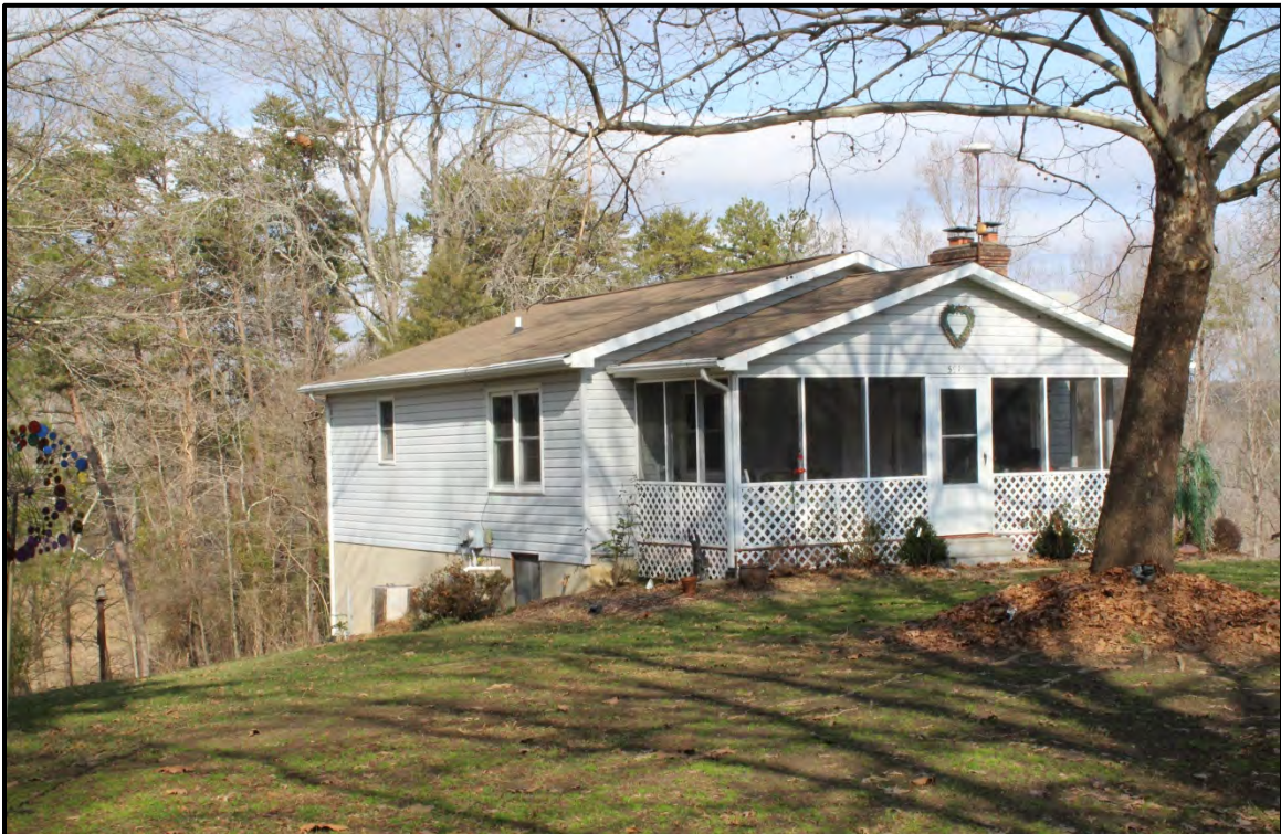
Figure 2.49. Architectural resource RK1794; view is northeast featuring the façade and the west elevation.
