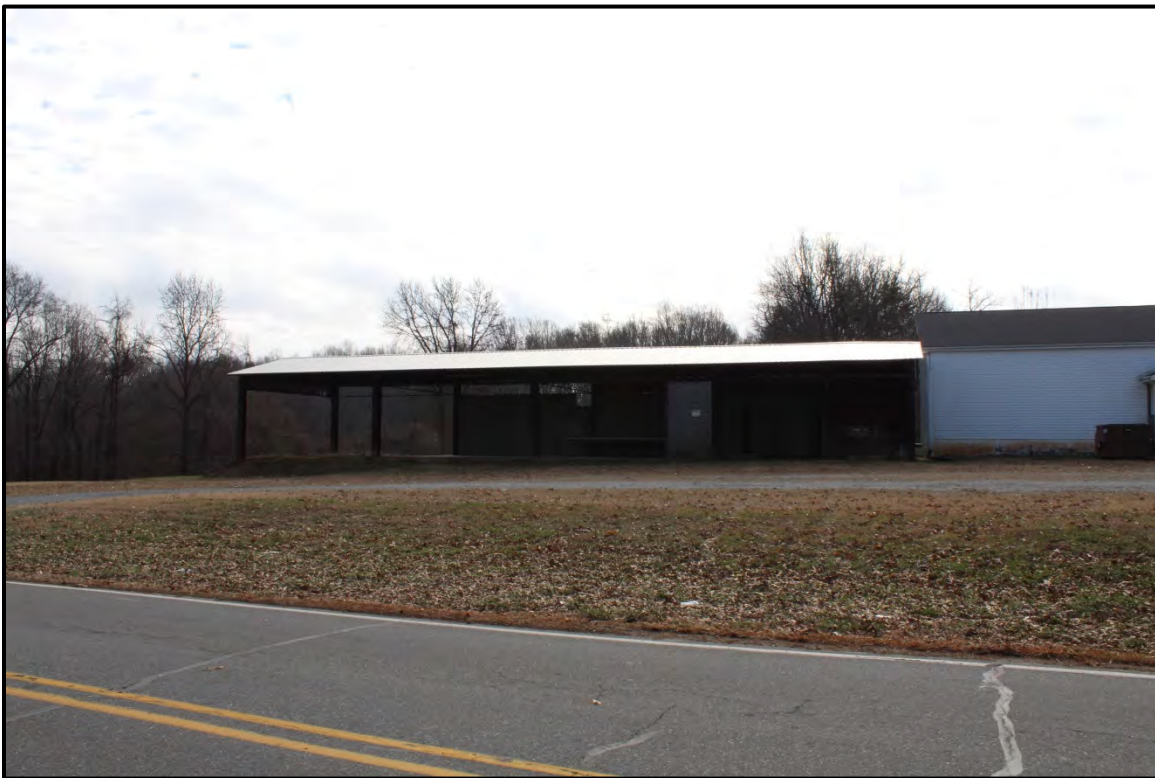
Figure 2.150. Architectural resource RK1814; view is southeast and features the equipment shed.
