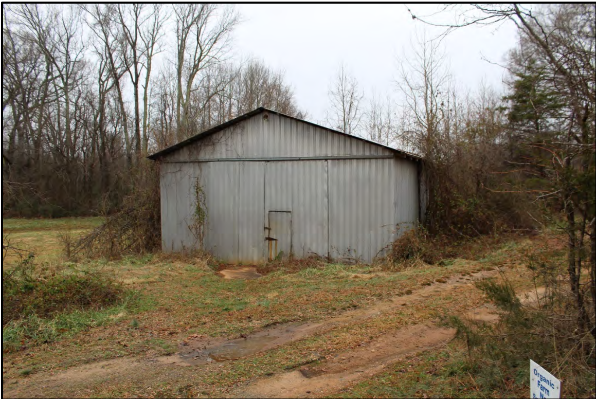
Figure 2.78. Architectural resource RK1818; view is west featuring the 1981 agricultural storage building.
