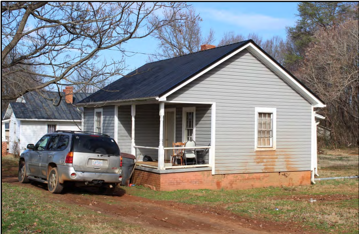
Figure 2.126. Architectural resource RK1807; view is southeast and features the façade and north elevation.
