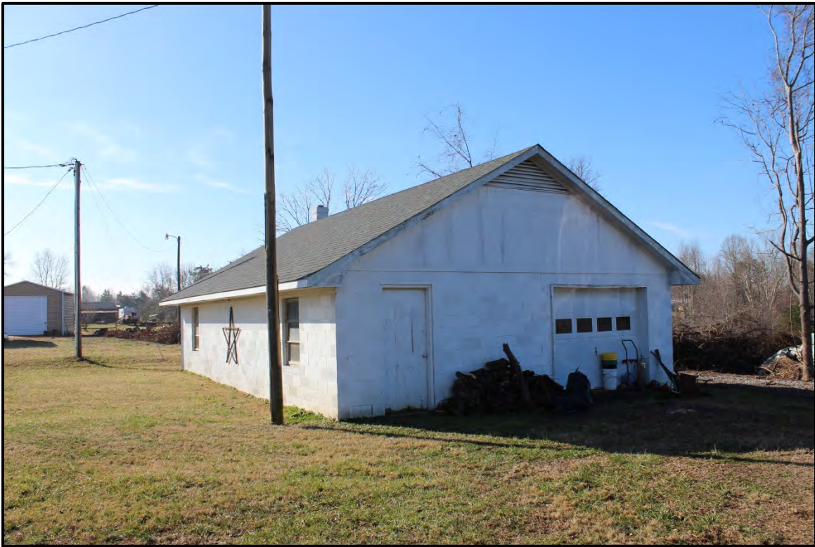
Figure 2.72. Architectural resource RK1799; view is southwest featuring the maintenance garage.
