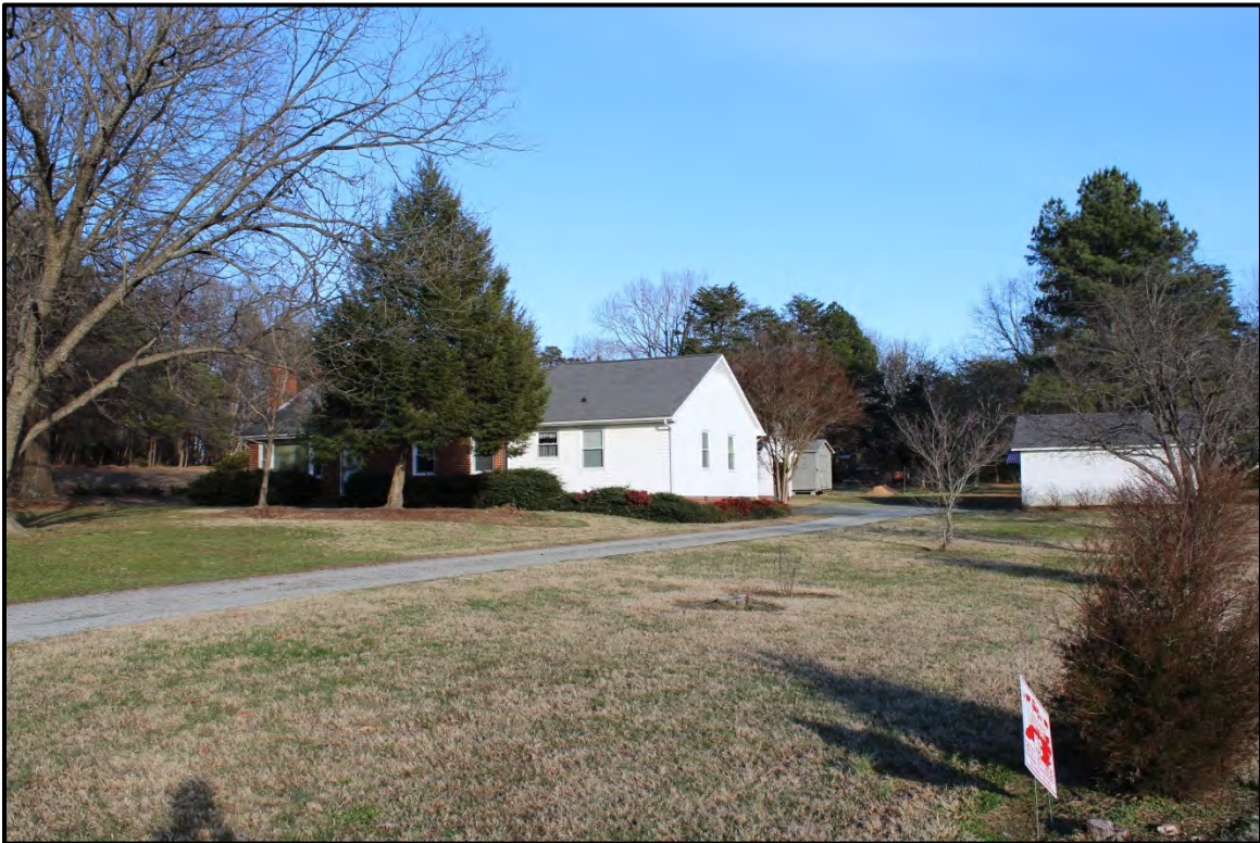
Figure 4.7. Architectural resource AM2620; view is northeast featuring the modern addition attached to the south elevation and associated outbuildings.
