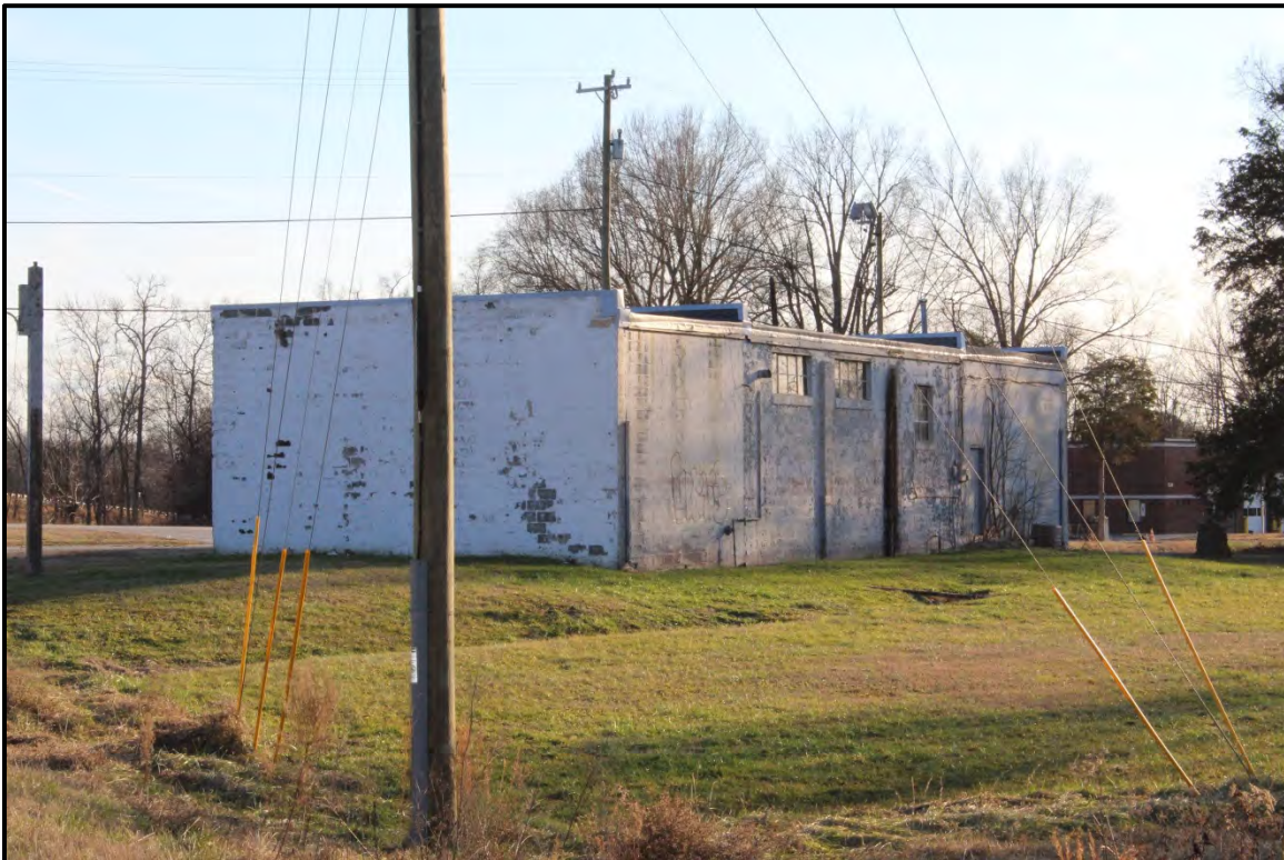
Figure 3.6. Architectural resource GF9108; view is northwest featuring the south (rear) and east elevations.
