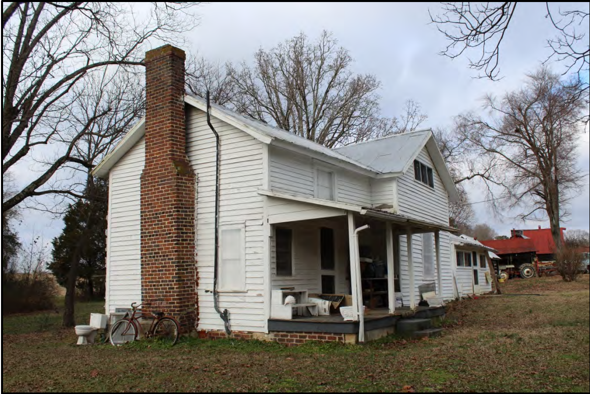
Figure 4.74. Architectural resource AM2631; view is north featuring the façade and southwest elevation of the ca. 1893 log-frame house.
