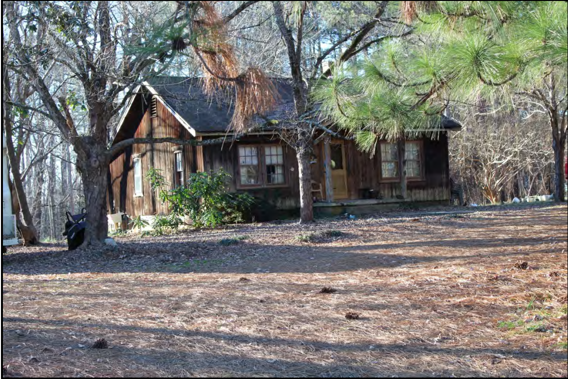
Figure 4.39. Architectural resource AM2628; view is northwest featuring the façade and south elevation.
