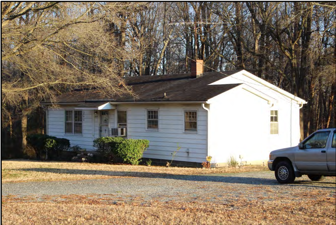
Figure 3.21. Architectural resource GF9114; view is southeast featuring the façade and west elevation.
