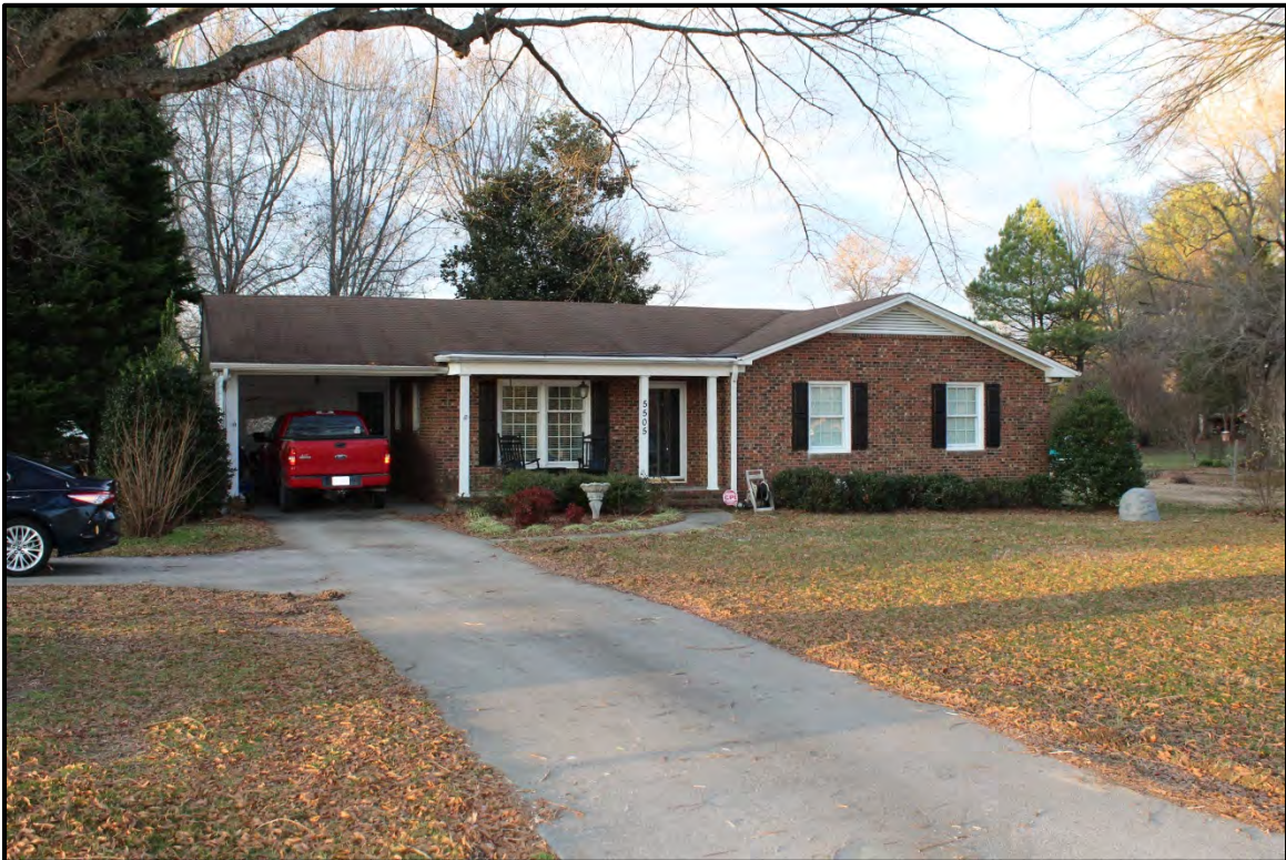
Figure 3.15. Architectural resource GF9111; view is northeast featuring the façade and west elevation.
