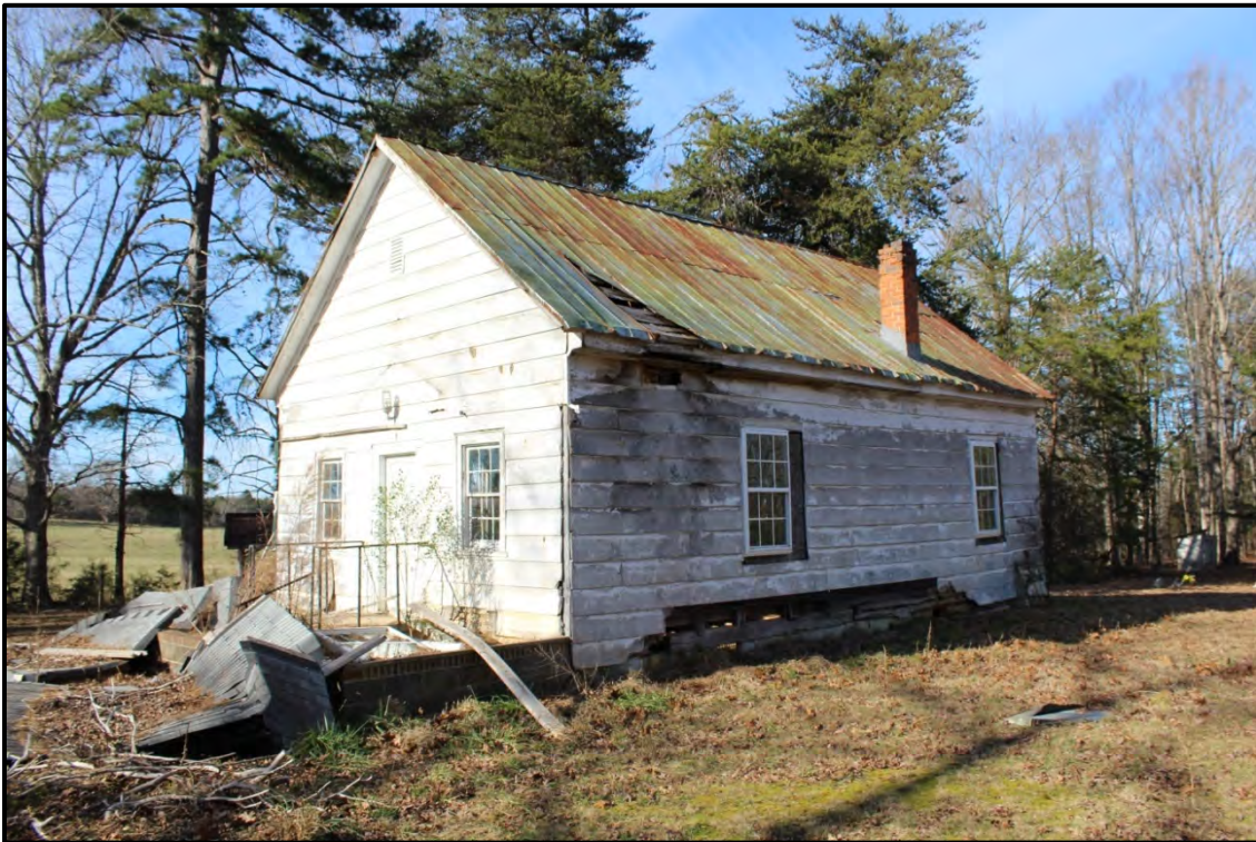
Figure 4.61. Architectural resource AM1603; view is northwest featuring the façade and east elevation.
