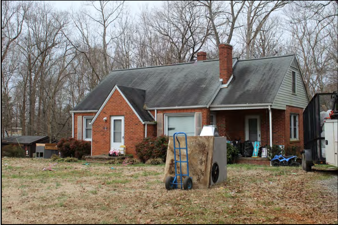
Figure 4.160. Architectural resource AM2648; view is southeast featuring the façade and north elevation.
