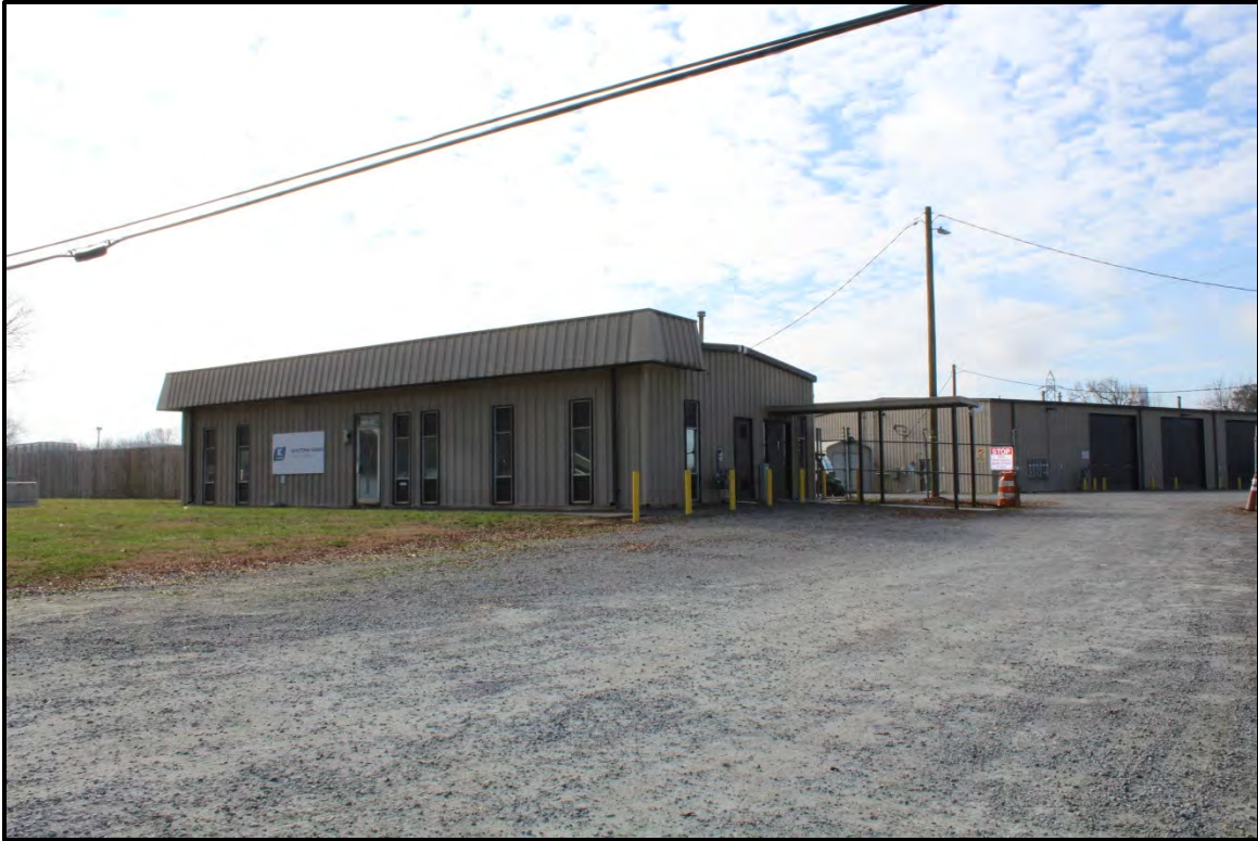
Figure 2.115. Architectural resource RK1804; view is southwest and features the office building.
