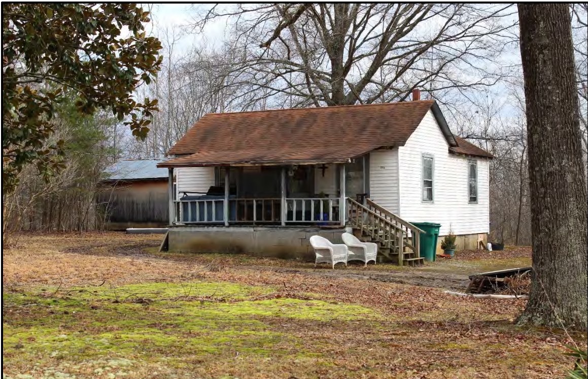
Figure 2.12. Architectural resource RK1821; view is north and features the façade and southeast elevation.
