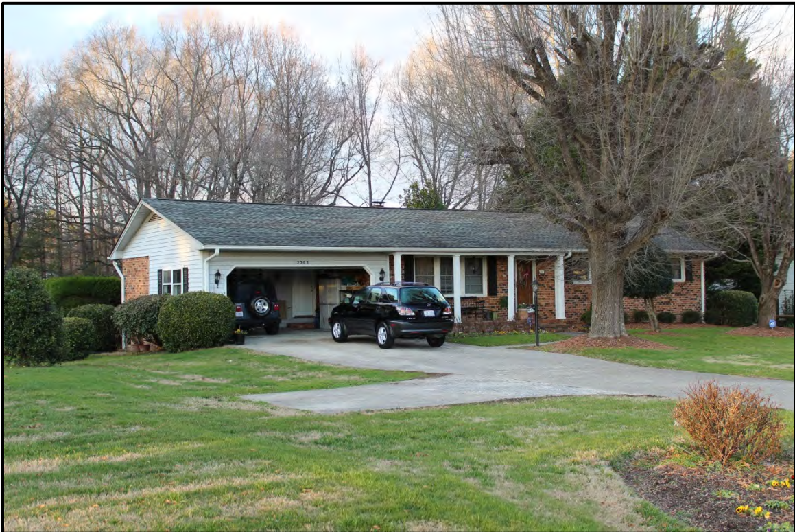
Figure 3.13. Architectural resource GF9110; view is northeast featuring the façade and west elevation.
