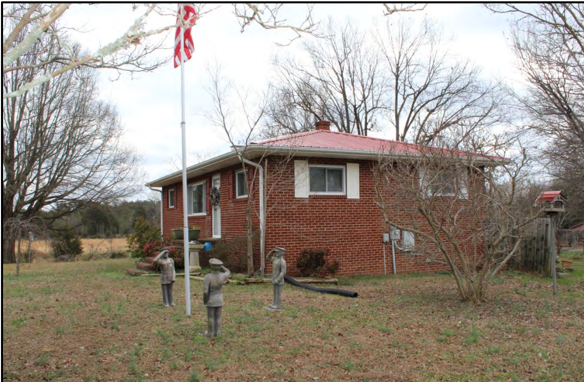
Figure 4.99. Architectural resource AM2652; view is southeast featuring the façade and west elevation of the farmhouse.
