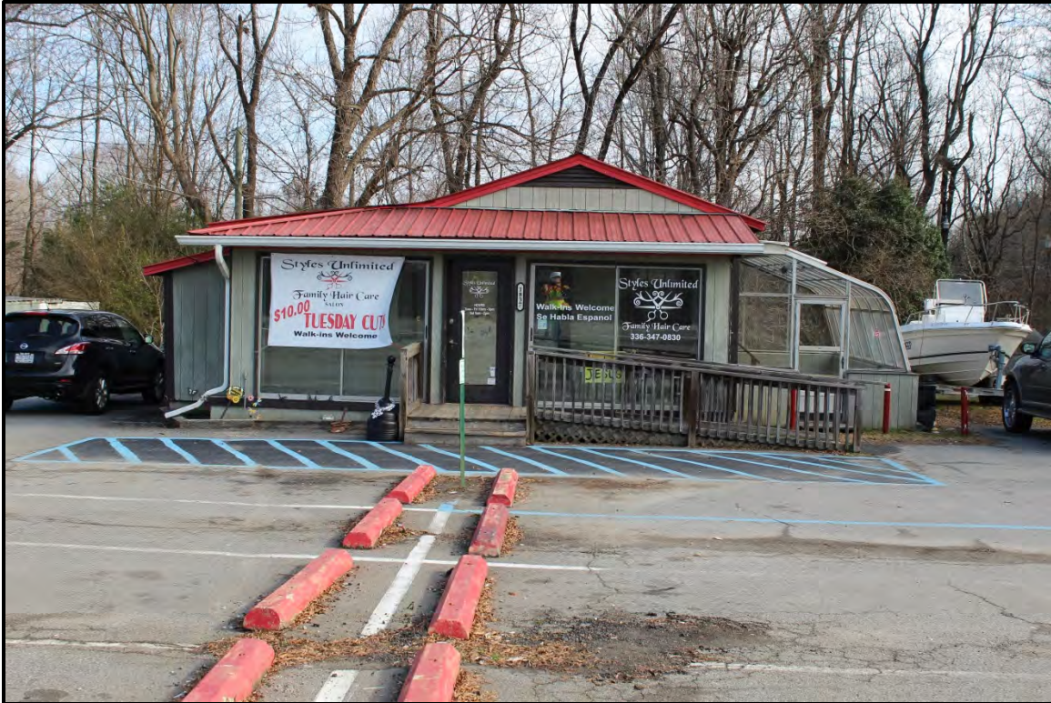
Figure 2.137. Architectural resource RK1811; view is east and features the façade.
