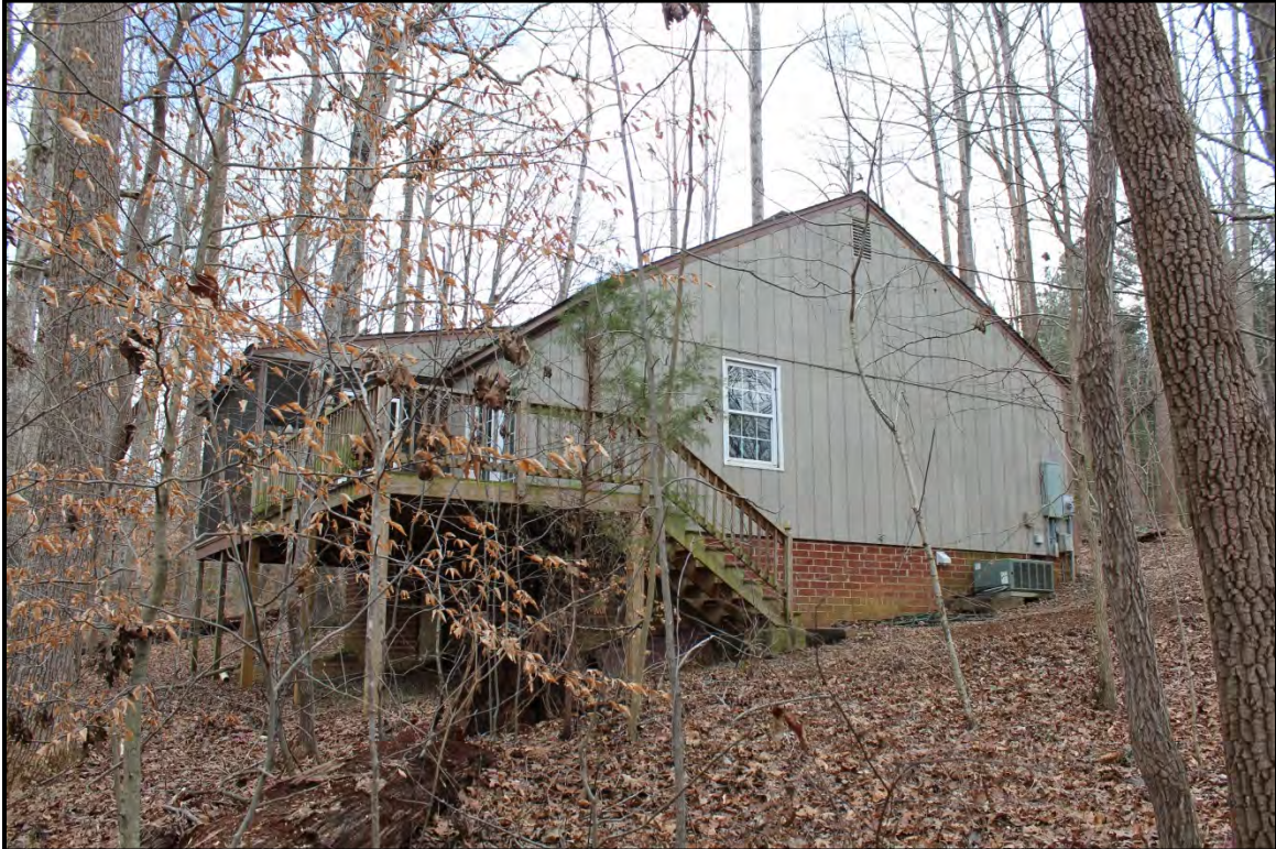
Figure 4.164. Architectural resource AM2649; view is east featuring the northwest (rear) and southwest elevations.
