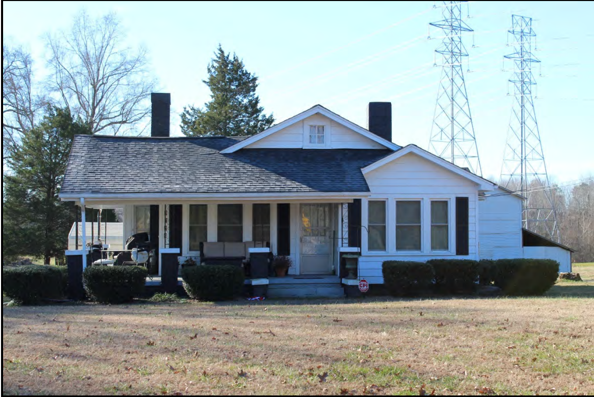
Figure 4.10. Architectural resource AM2621; view is south featuring the façade.
