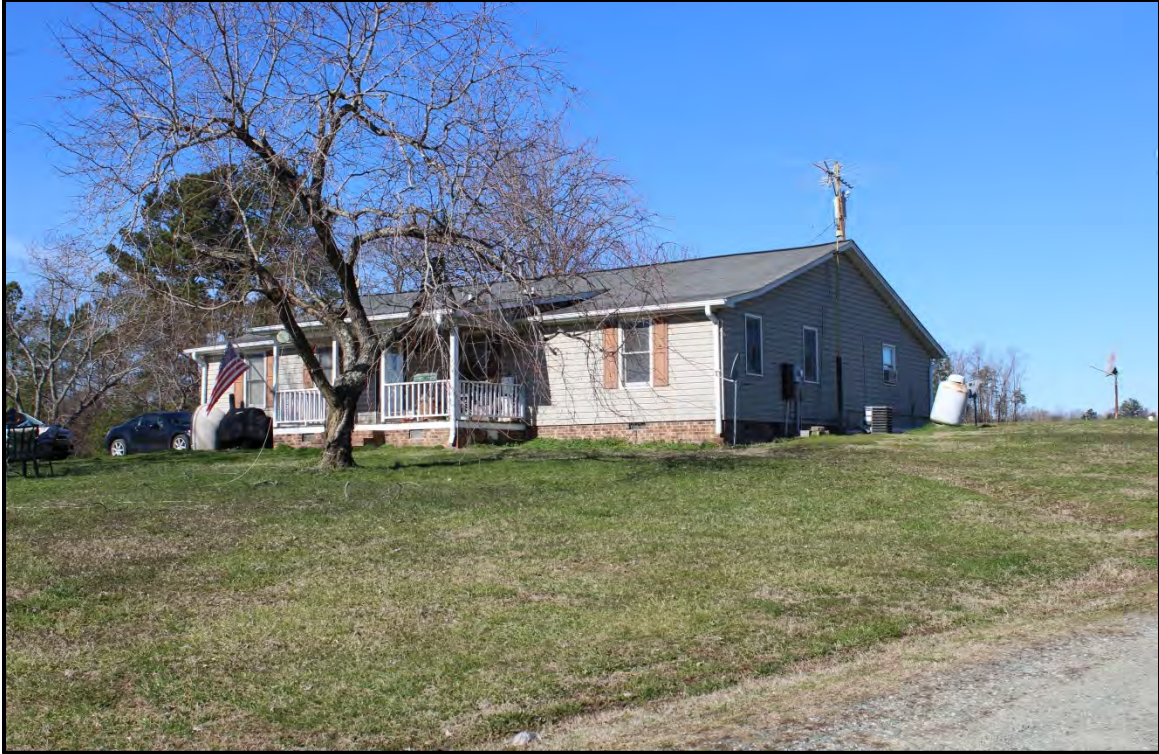
Figure 4.129. Architectural resource AM2634 farmhouse; view is northwest featuring the façade and east elevation.
