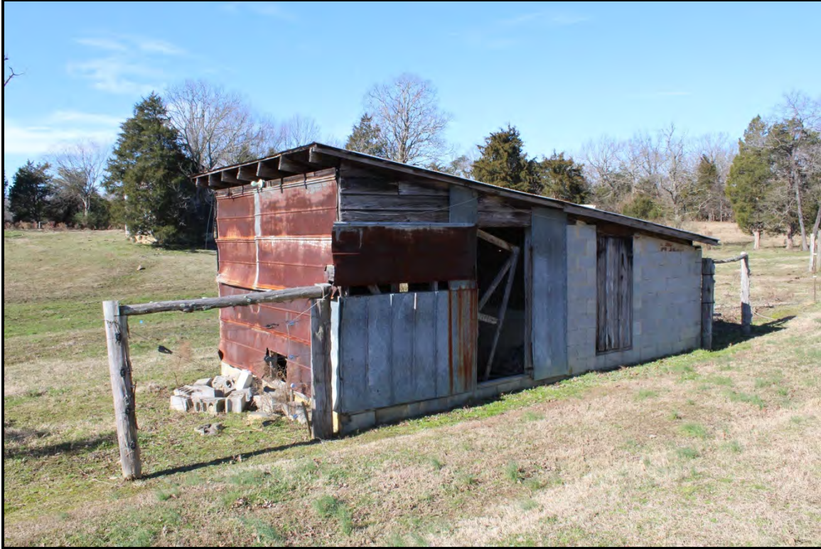
Figure 4.112. Architectural resource AM2635; view is northwest featuring the concrete block storage shed.
