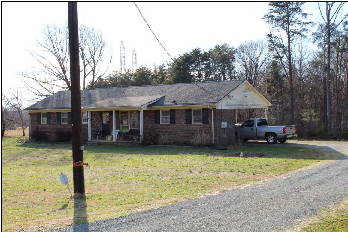
Figure 4.4. Architectural resource AM2618; view is southwest featuring the façade and north elevation.
