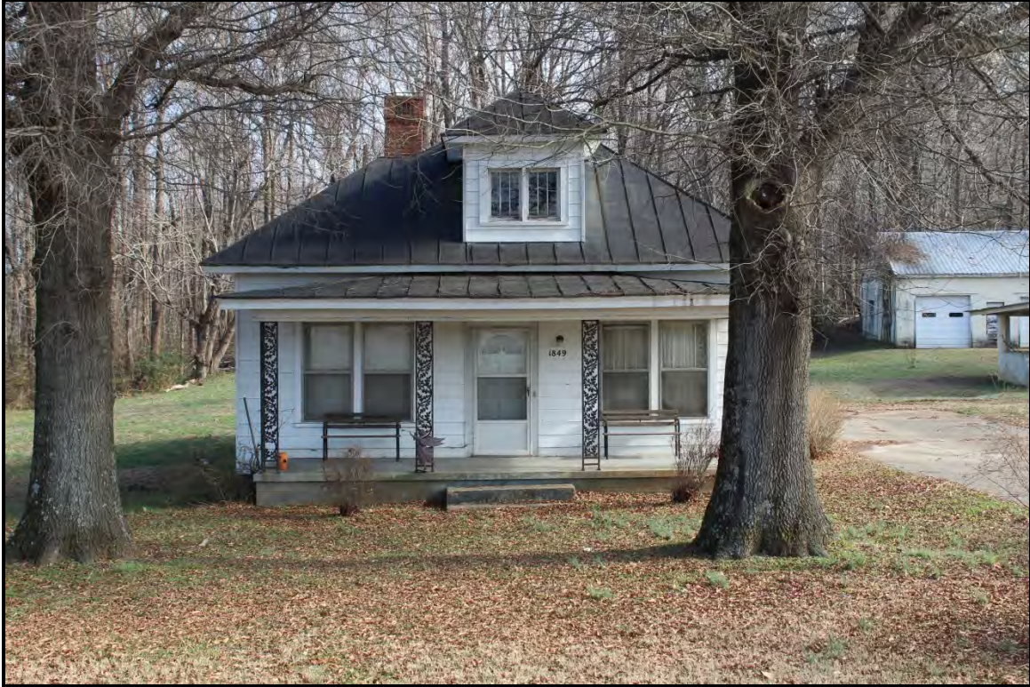
Figure 2.127. Architectural resource RK1808; view is east and features the façade.
