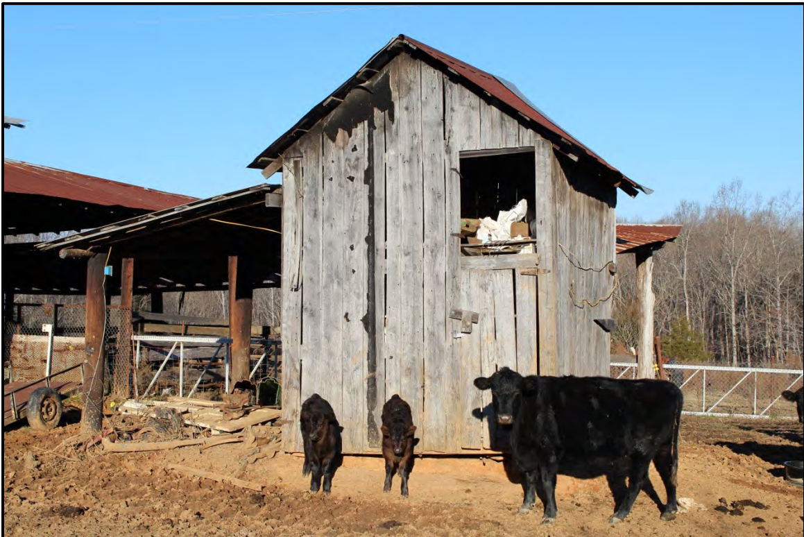
Figure 2.36. Architectural resource RK1792 ca. 1970 storage shed; view is east.
