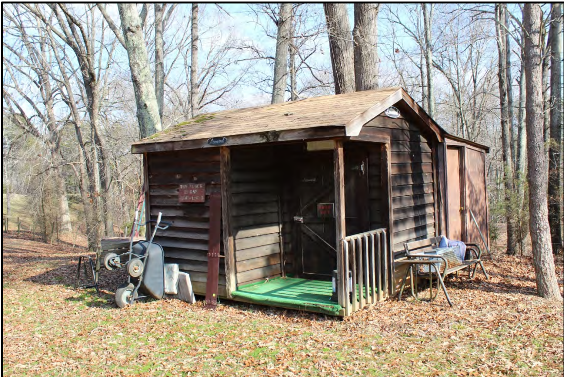
Figure 2.51. Architectural resource RK1794; view is northeast featuring the storage shed.
