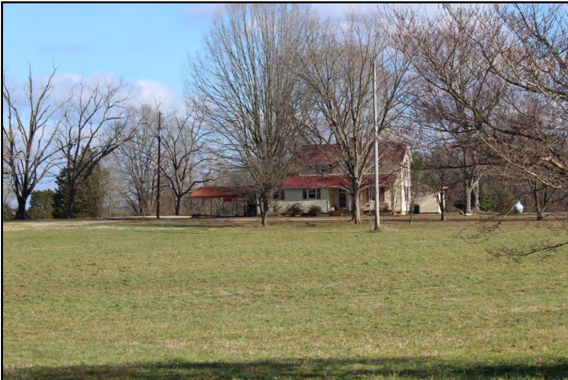
Figure 4.29. Architectural resource AM1536; view is northeast featuring the façade and modern carport.
