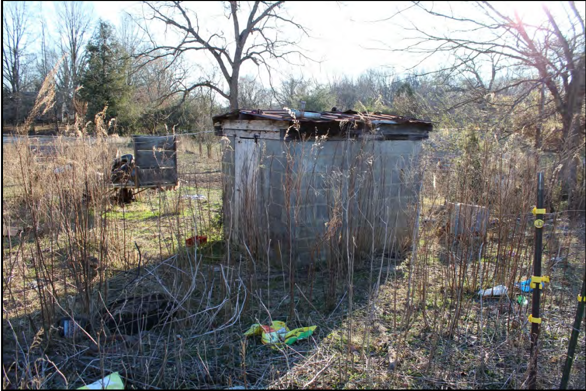
Figure 2.35. Architectural resource RK1792 water pump shed; view is southwest.
