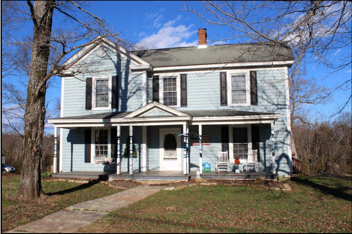
Figure 2.56. Architectural resource RK1796; view is northeast featuring the façade.
