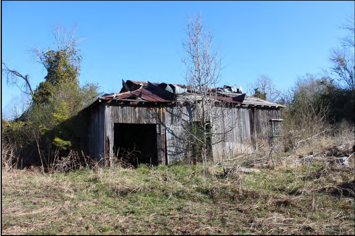
Figure 2.73. Architectural resource RK1799; view is northeast featuring the tractor barn.
