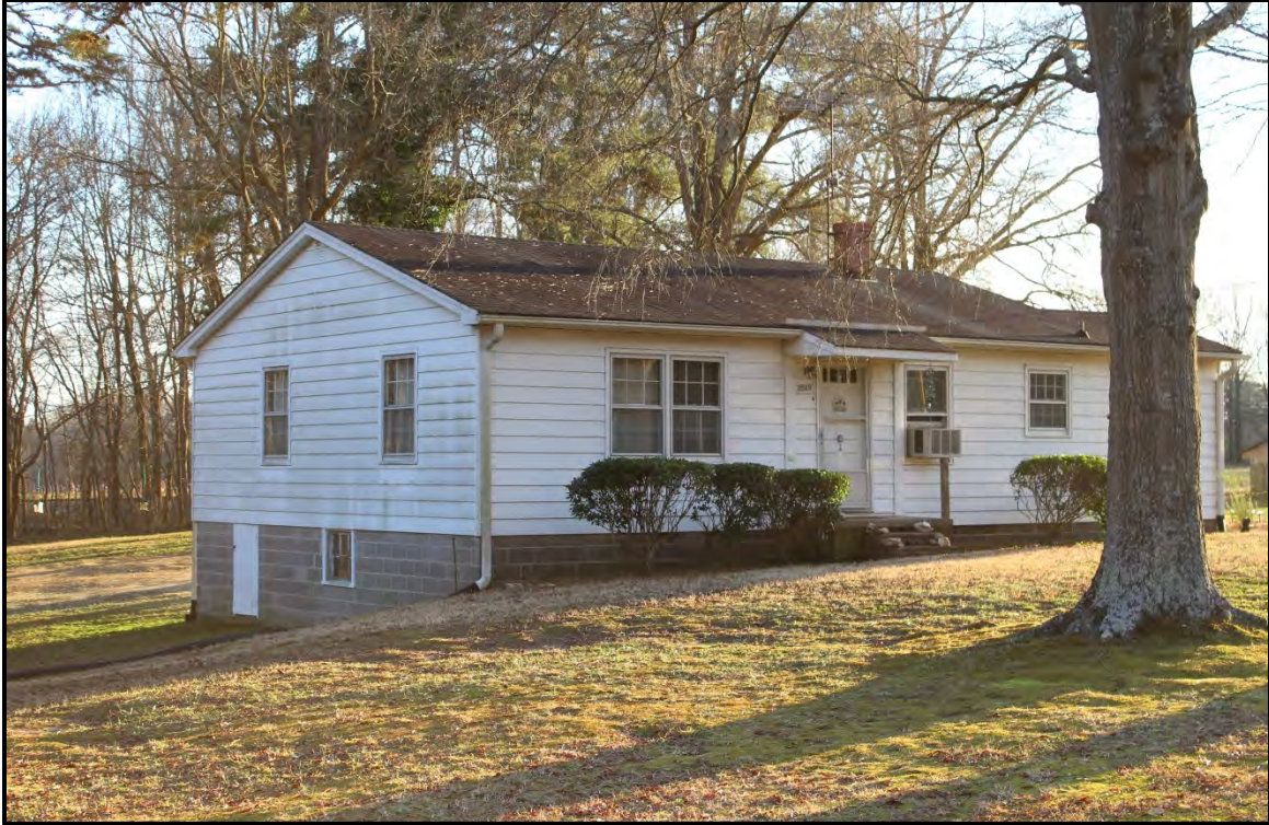
Figure 3.20. Architectural resource GF9114; view is southwest featuring the façade and east elevation.
