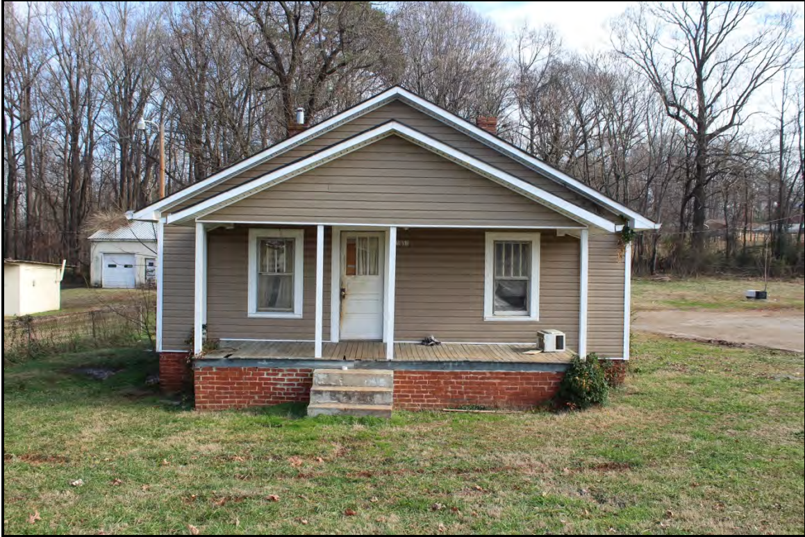
Figure 2.118. Architectural resource RK1805; view is east and features the façade.
