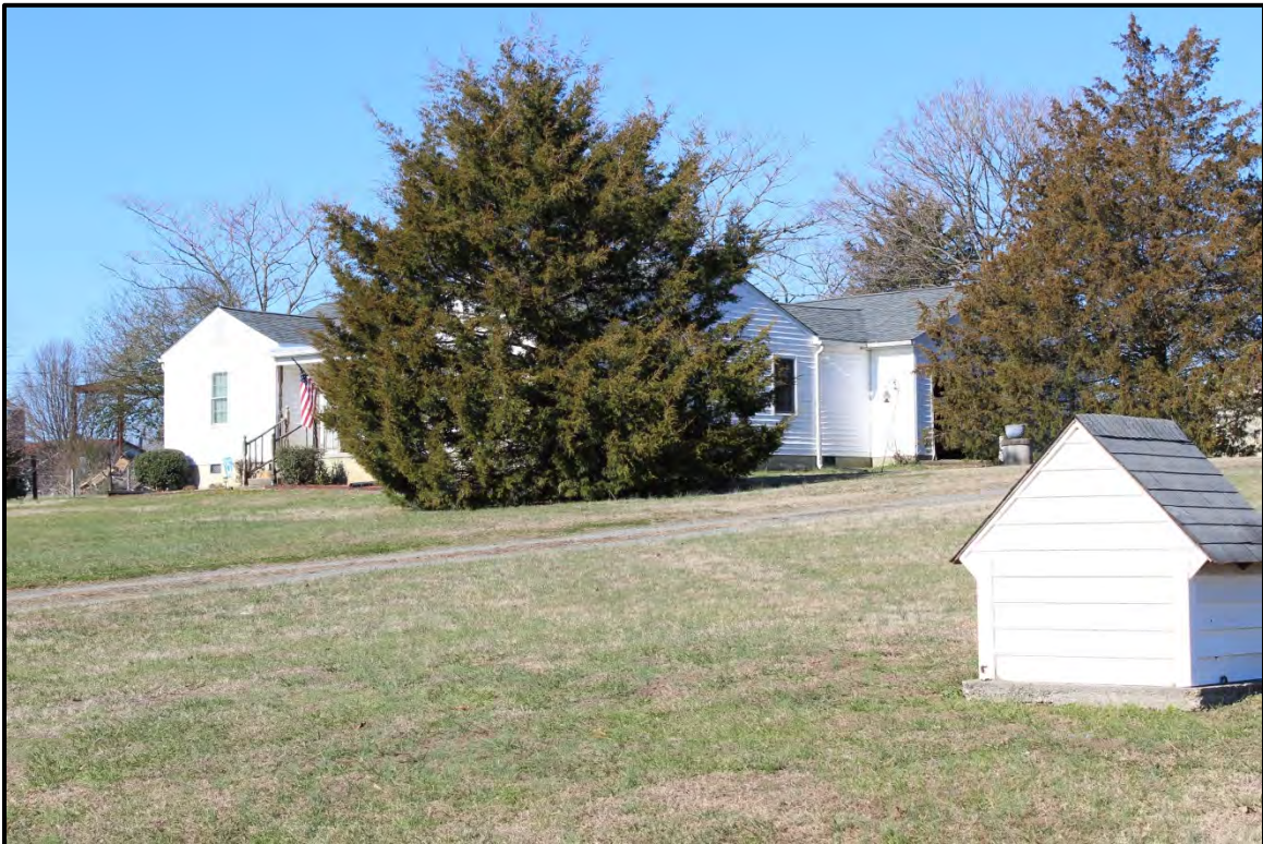
Figure 4.21. Architectural resource AM2623; view is east featuring the west elevation and the early twentieth century garage.
