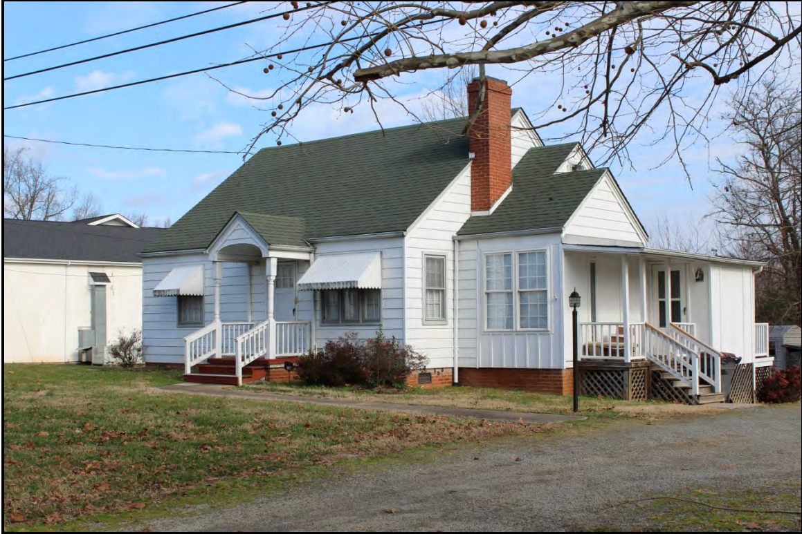
Figure 2.146. Architectural resource RK1813; view is northeast and features the façade and south elevation.
