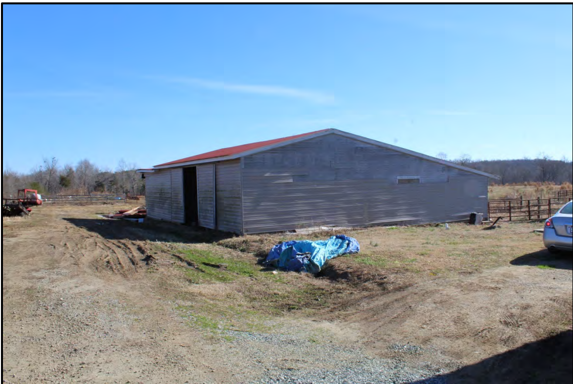
Figure 4.132. Architectural resource AM2634; view is east featuring the storage building.
