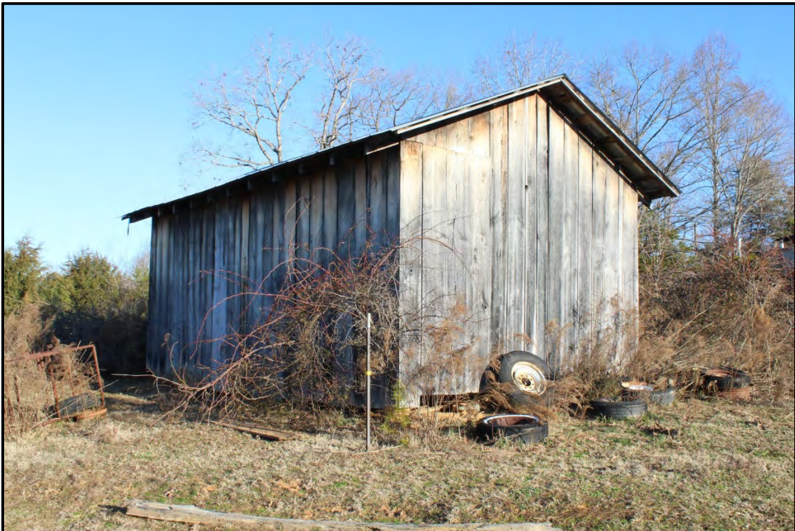
Figure 2.40. Architectural resource RK1792; view is north featuring the late twentieth century equipment shed.
