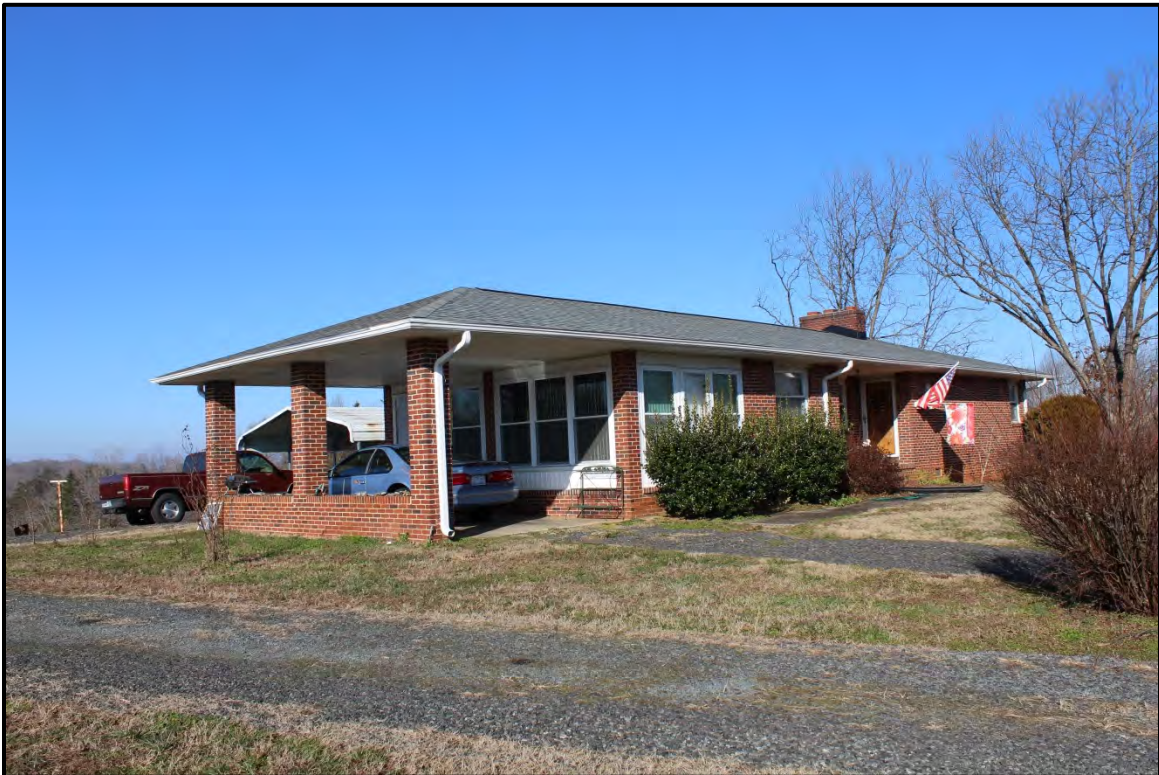
Figure 2.70. Architectural resource RK1799; view is southeast featuring the façade and north elevation.
