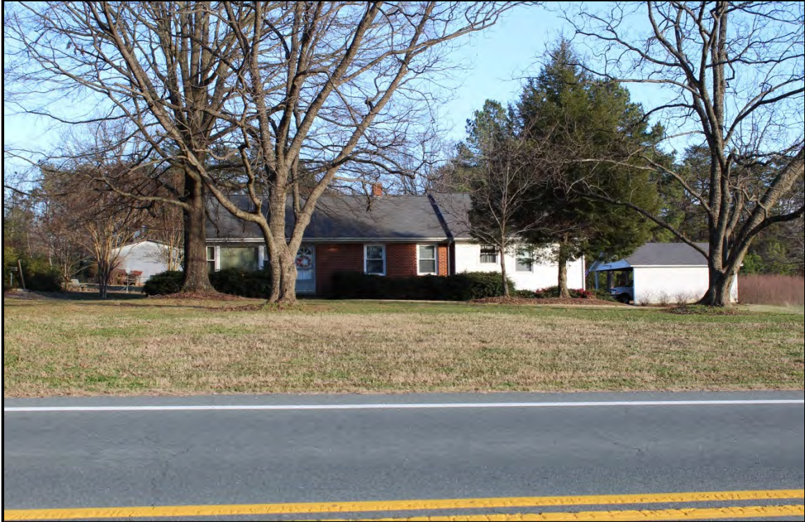
Figure 4.6. Architectural resource AM2620; view is east featuring the façade and associated outbuildings.
