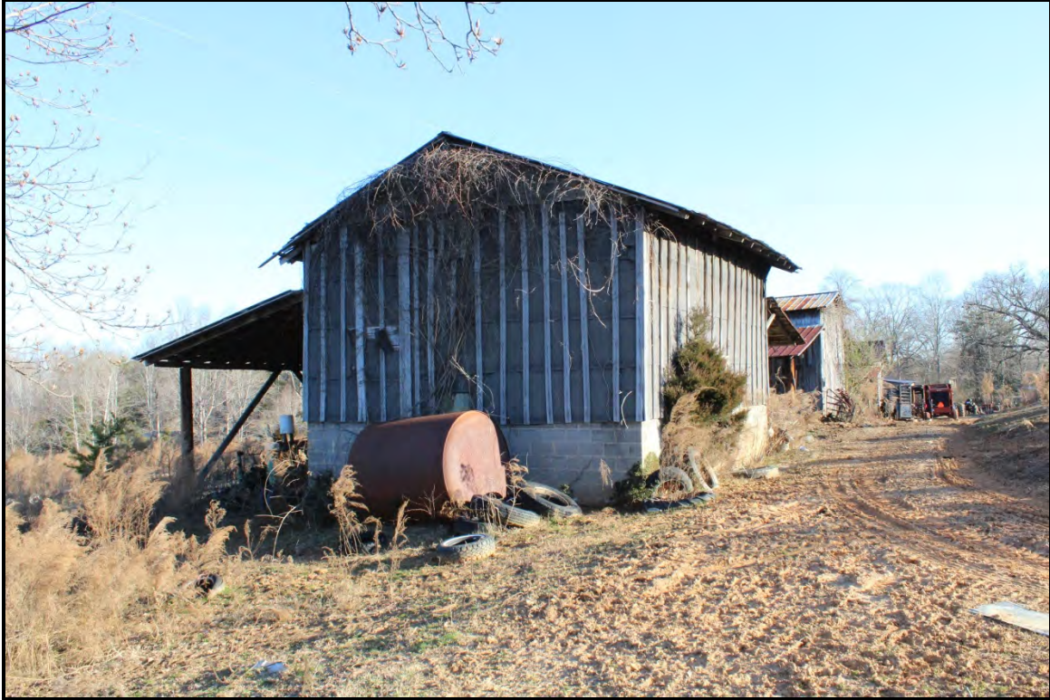
Figure 2.39. Architectural resource RK1792; view is east featuring the ca. 2000 tractor barn.
