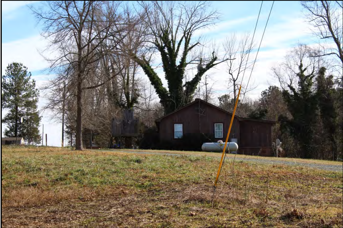
Figure 4.59. Architectural resource AM2629; view is southeast featuring the façade and west elevation of the ca. 1968 residence with the modern carport in the background.
