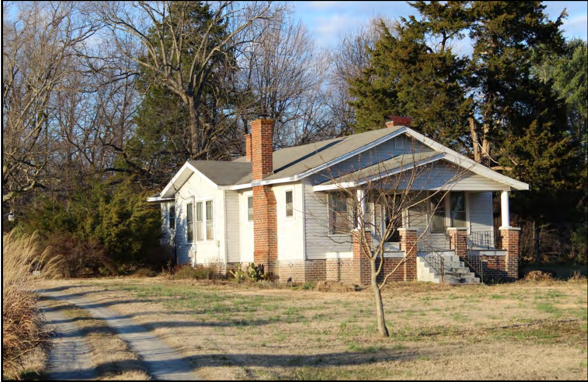
Figure 3.10. Architectural resource GF9109; view is northeast featuring the façade and west elevation.
