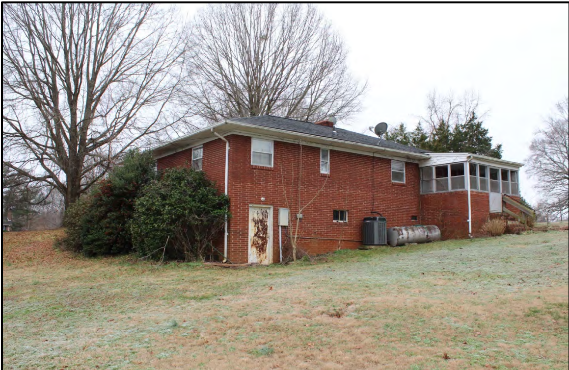
Figure 2.76. Architectural resource RK1818 farmhouse; view is southwest featuring the north (rear) and east elevations.
