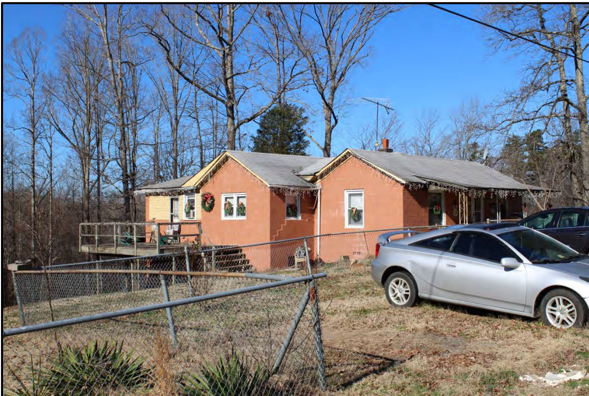
Figure 2.7. Architectural resource RK1784; view is northwest featuring the façade and the side-gabled extension to the west (rear) elevation.
