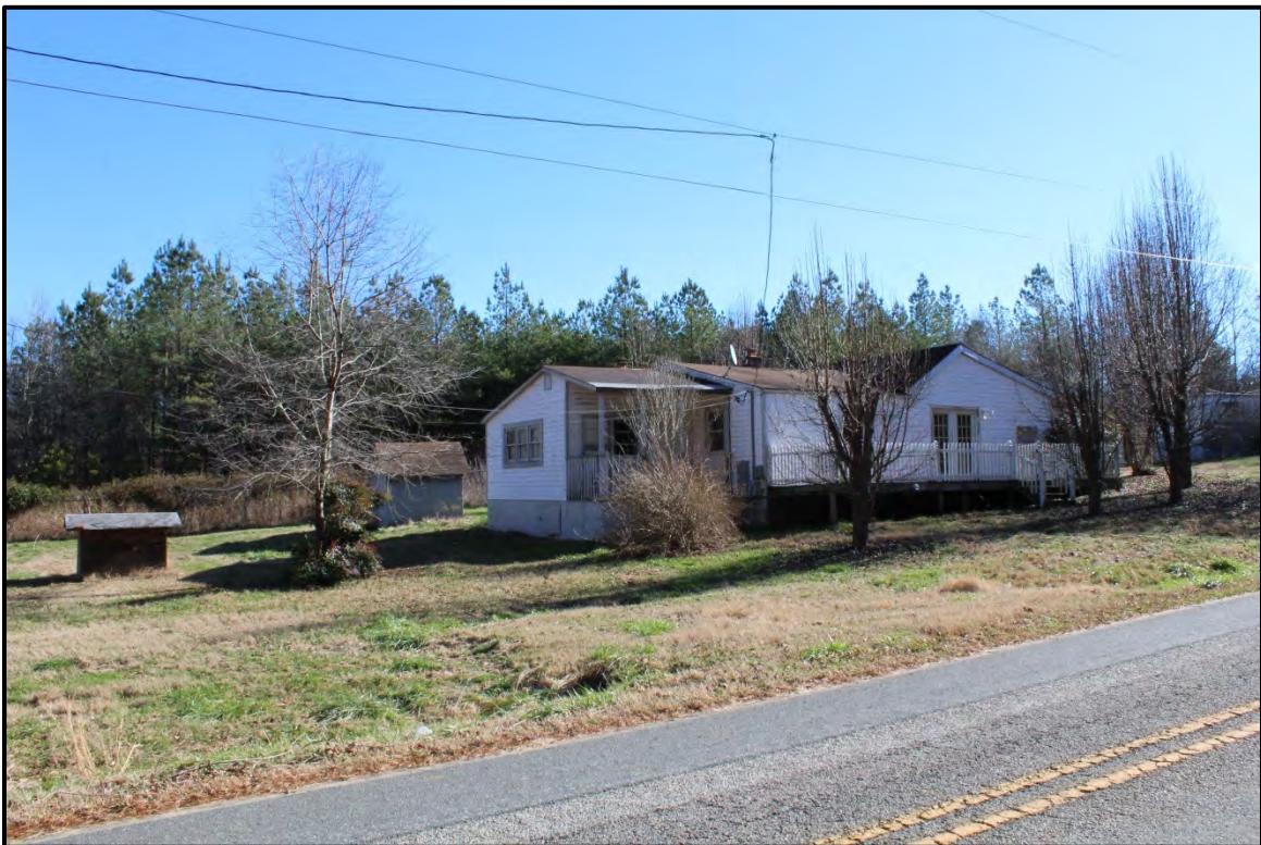
Figure 2.2. Architectural resource RK1786; view is southeast featuring the façade and the north elevation of the house with associated the pump shed and concrete storage shed.
