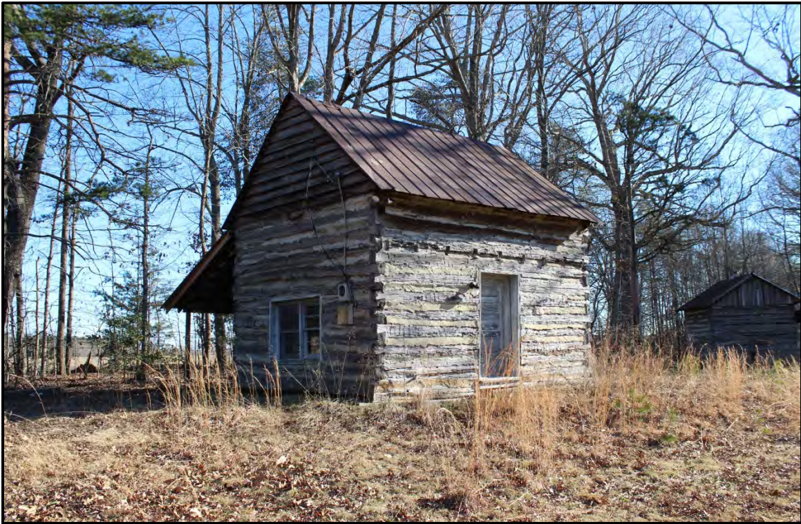
Figure 4.31. Architectural resource AM0209; view is southeast featuring the façade and north elevation with non-historic window sash.
