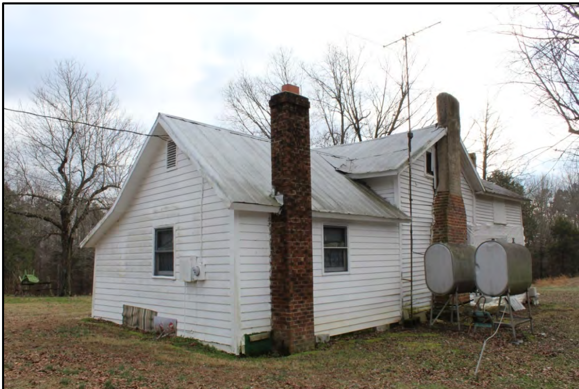
Figure 4.77. Architectural resource AM2631; view is south featuring the northeast and northwest (rear) elevations of ca. 1940 wood-frame wing addition.
