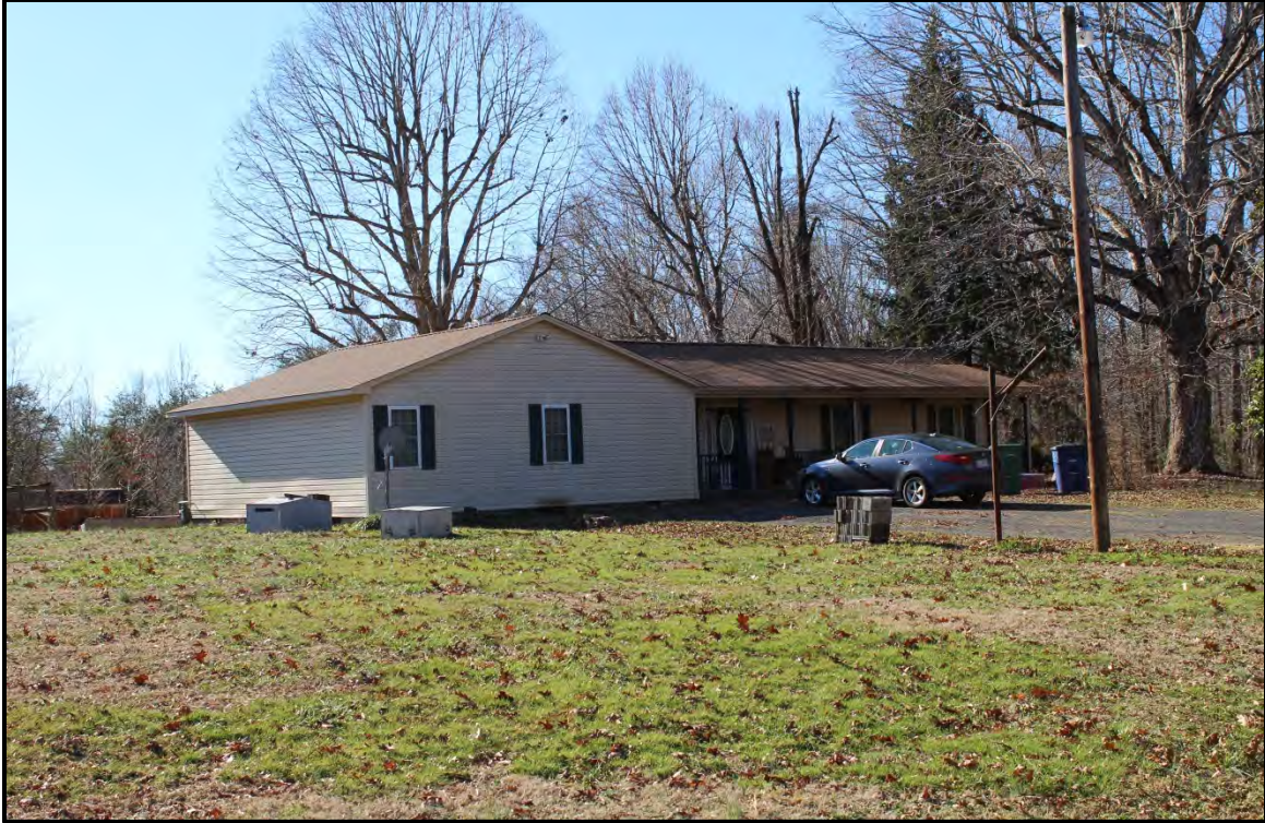
Figure 2.22. Architectural resource RK1789; view is southwest featuring the façade and the modern addition attached to the west elevation.
