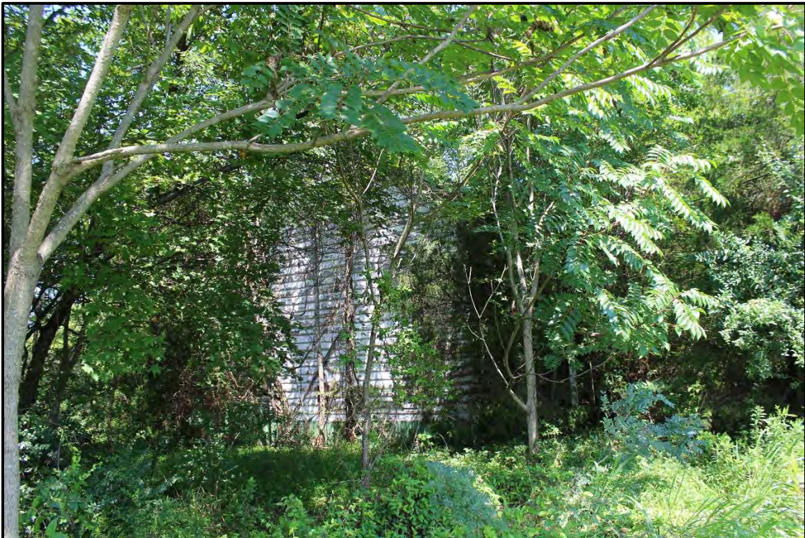
Figure 2.2. Property RK1822; view is northwest and features the south elevation.
