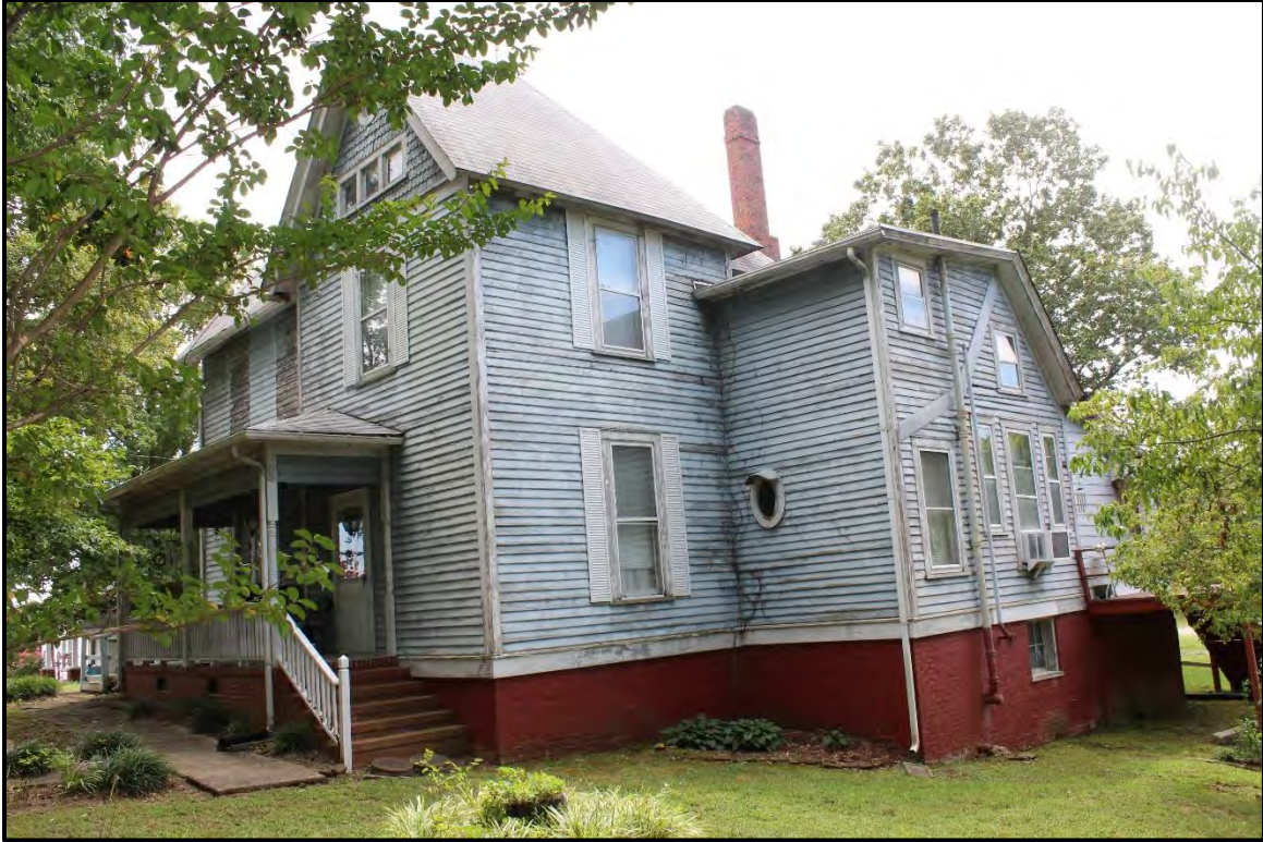
Figure 3.13. Architectural resource AM0447; view is southwest featuring the east and north (rear) elevations.
