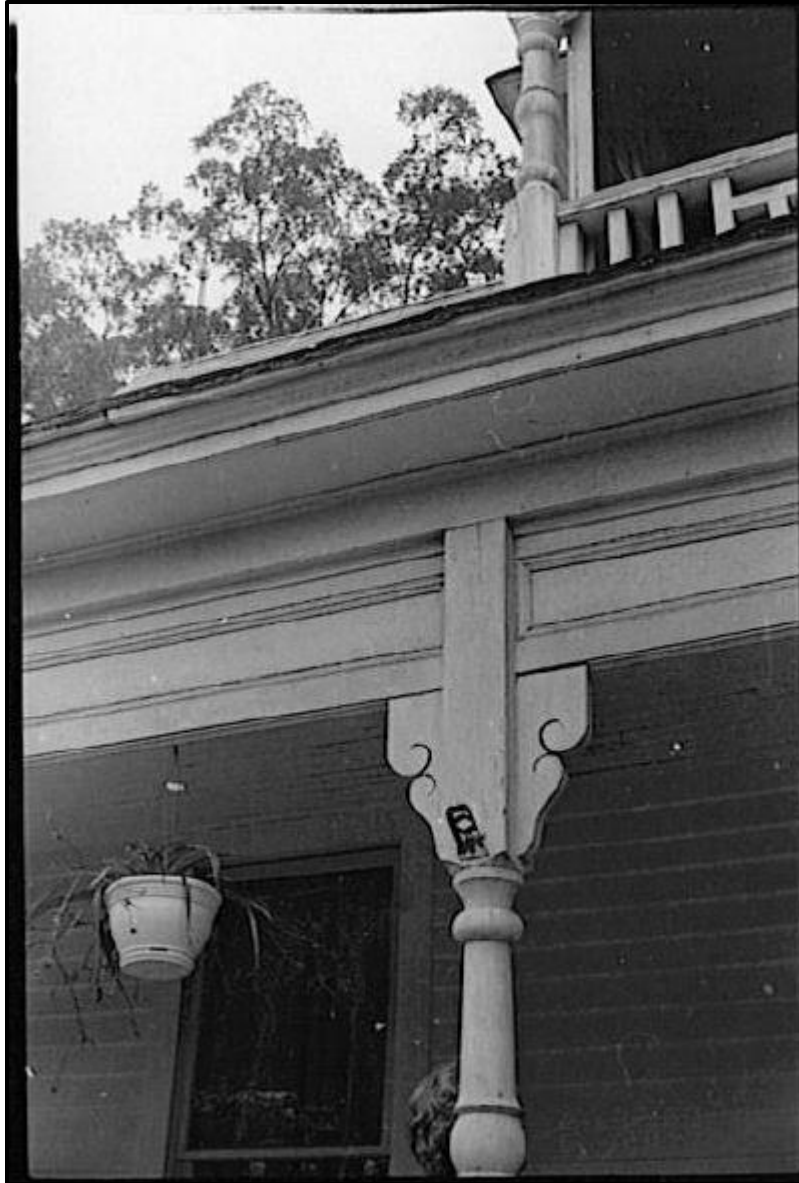
Figure 3.18. Photo of architectural resource AM0447 taken in 1978 depicting an original porch bracket and column on the façade porch (Image courtesy of Lounsbury 1978).
