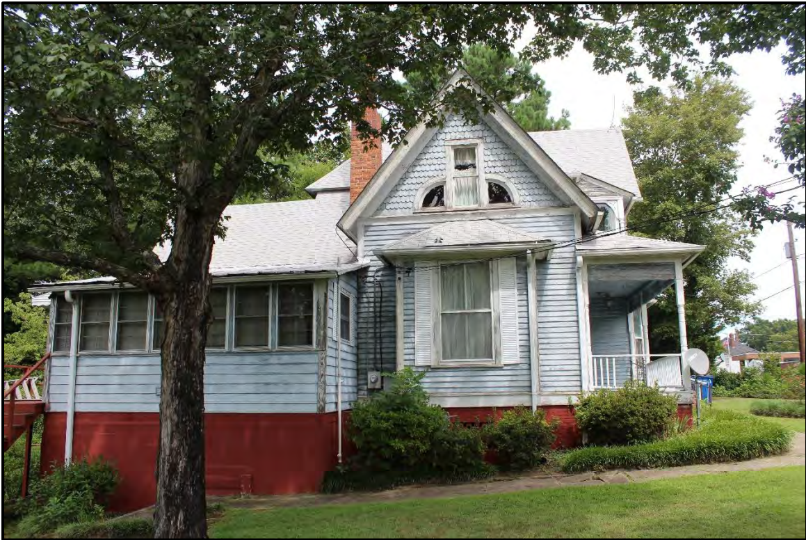
Figure 3.16. Architectural resource AM0447; featuring the west elevation, view is east.
