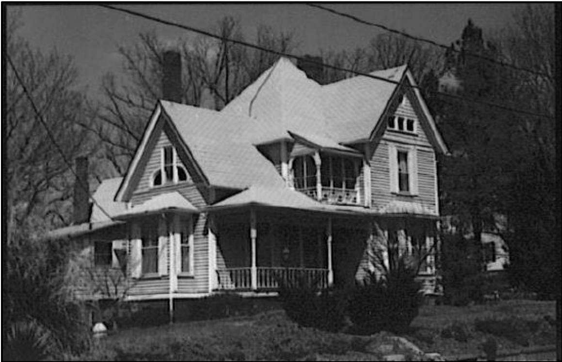
Figure 3.12. 2002 photo of AM0447. Note original sleeper porch balustrade (Image courtesy of Barkham 2002).
