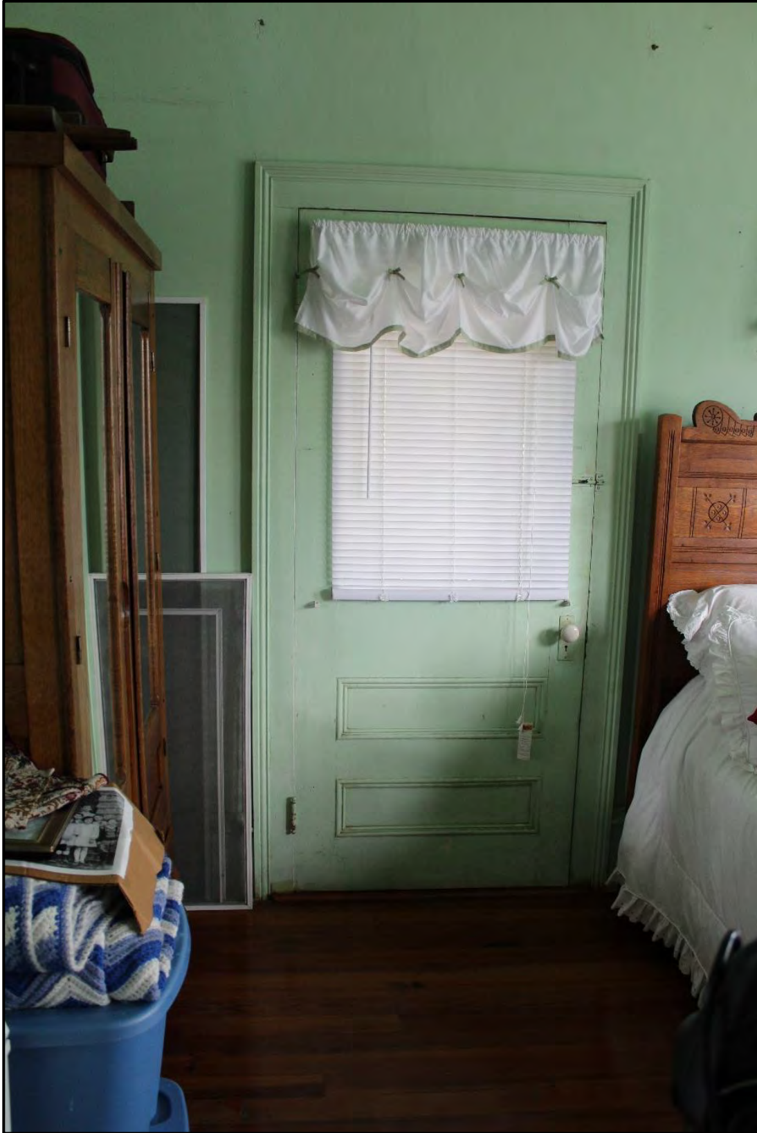
Figure 3.28. Architectural resource AM0447; east parlor door detail, view is east.
