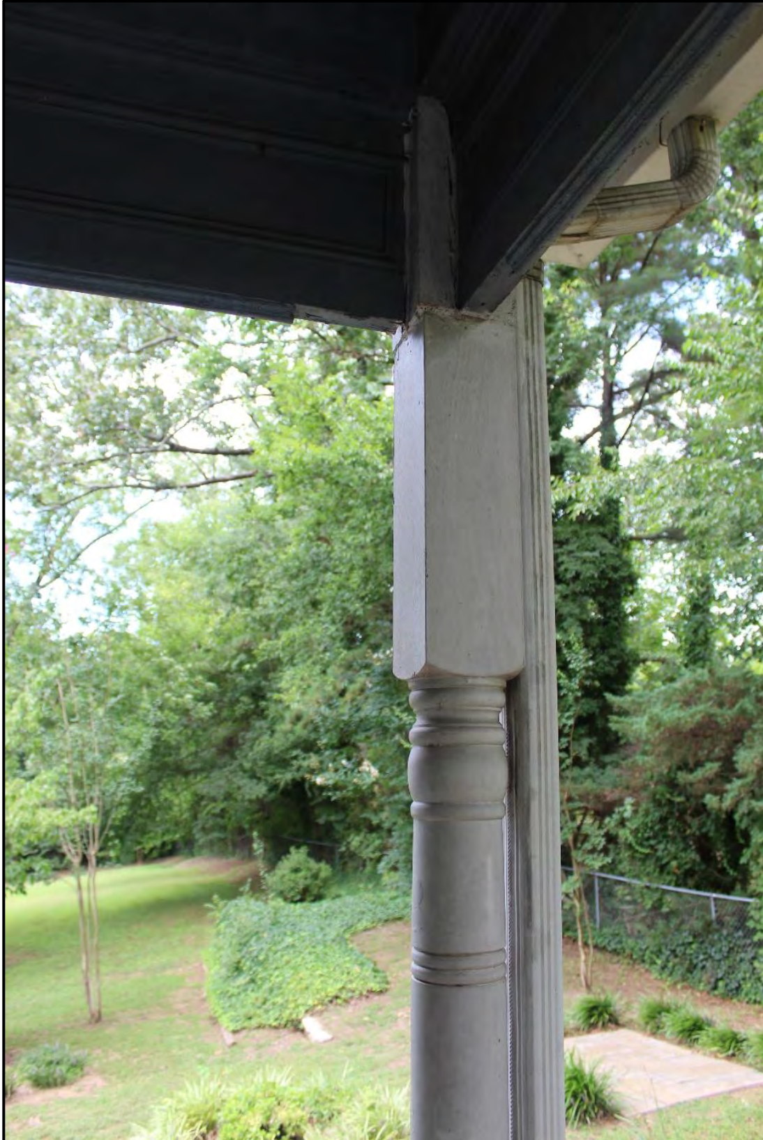
Figure 3.19. Architectural resource AM0447; porch detail showing butt joint connecting the frieze to the replacement column.
