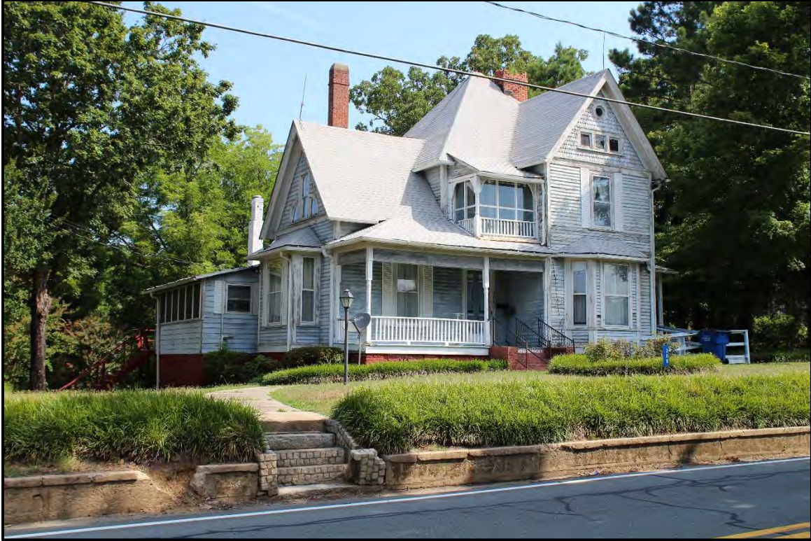
Figure 3.11. Architectural resource AM0447; view is northeast featuring the façade and west elevation.
