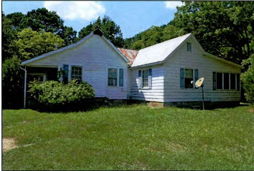
Fig. 2 The east elevation of the Lemuel Morgan Farm
