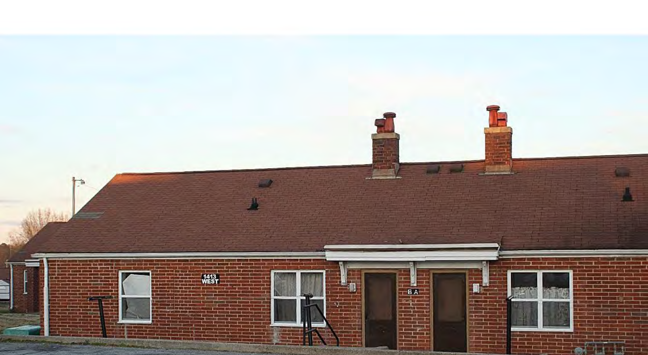
Development: Daniel Brooks Homes Building Number: 1413 West Ave. Description: Unit Type C Photographer: High Point Housing Authority Date Taken: June 14, 2019 Digital Photo: 1413 West Ave. Unit Type C3
