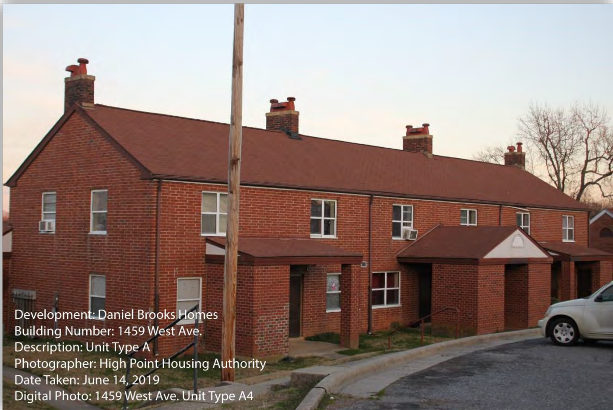
Development: Daniel Brooks Homes Building Number: 1459 West Ave. Description: Unit Type A Photographer: High Point Housing Authority Date Taken: June 14, 2019 Digital Photo: 1459 West Ave. Unit Type A3
