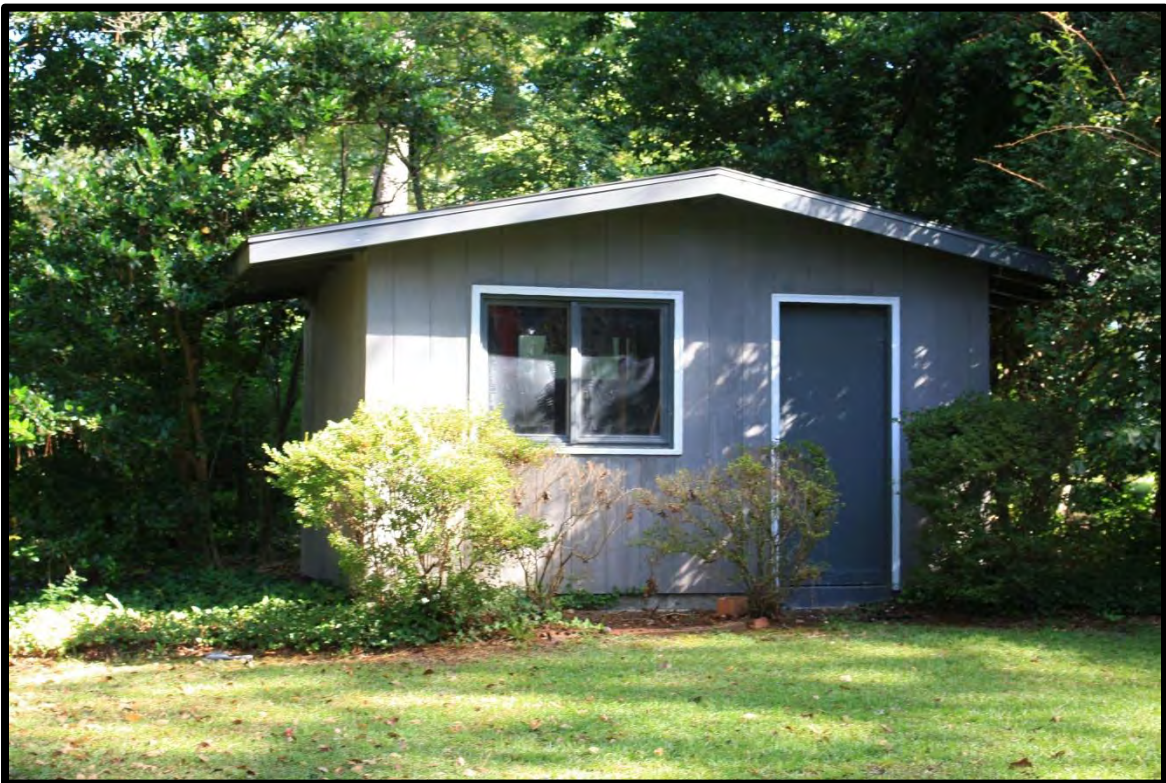
Figure 31: Garden Shed, Looking North.
