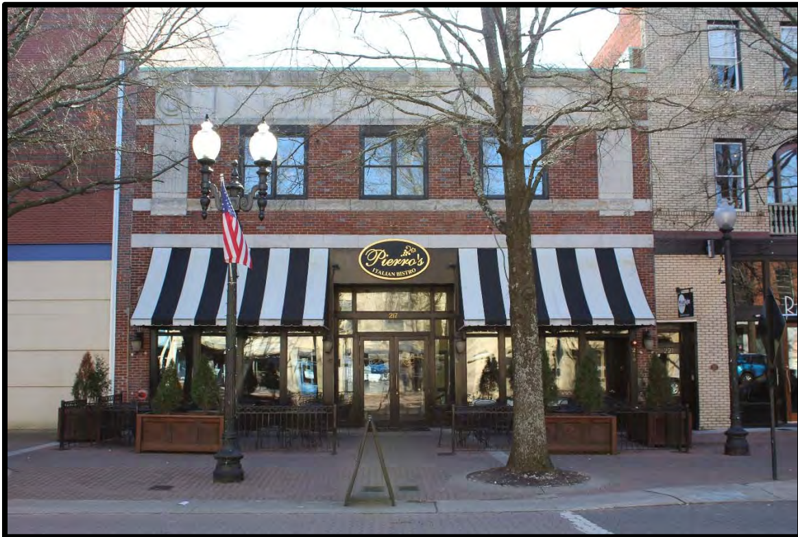
Figure 87: 217 Hay Street, Ca. 1935 Commercial Building.
