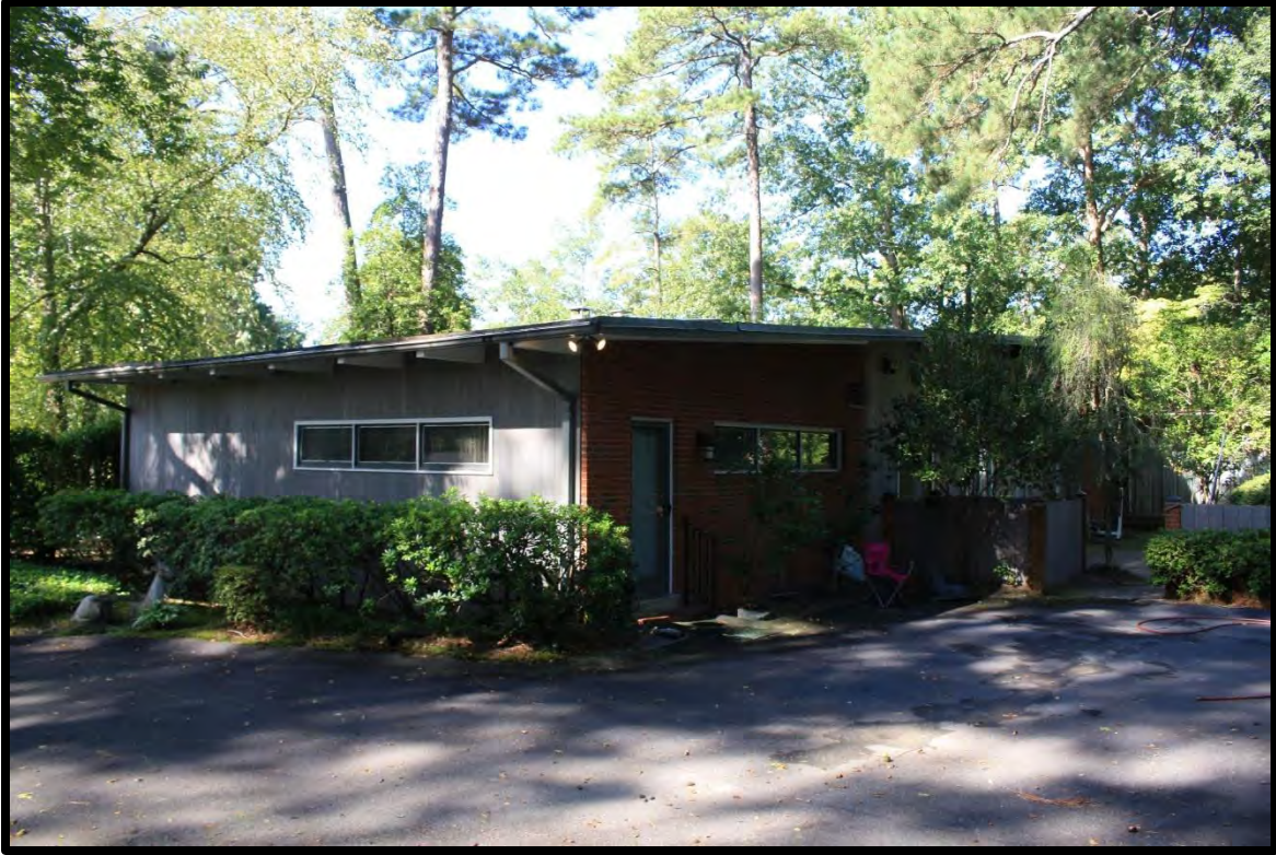
Figure 34: Fleishman House, Looking Southwest.
