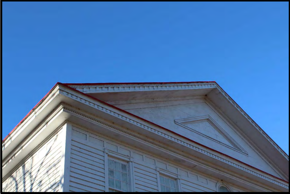
Figure 78: Old Bluff Church Detail, Looking Northwest.
