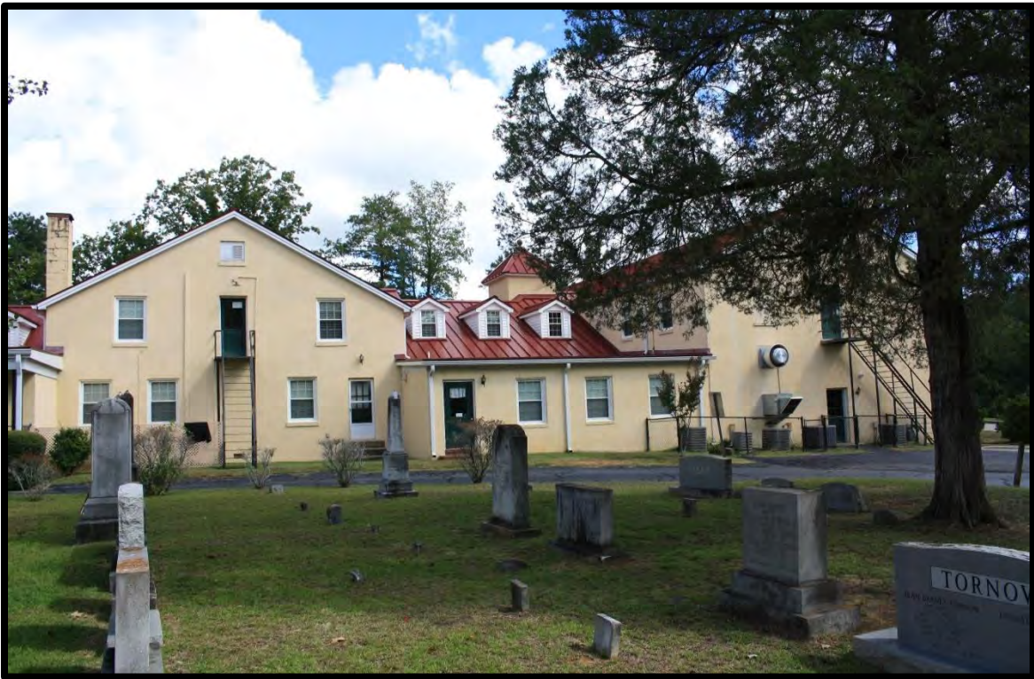
Figure 56: MacPherson Presbyterian Church, Education Wing, Hyphen, Fellowship Hall, Looking North-Northeast.
