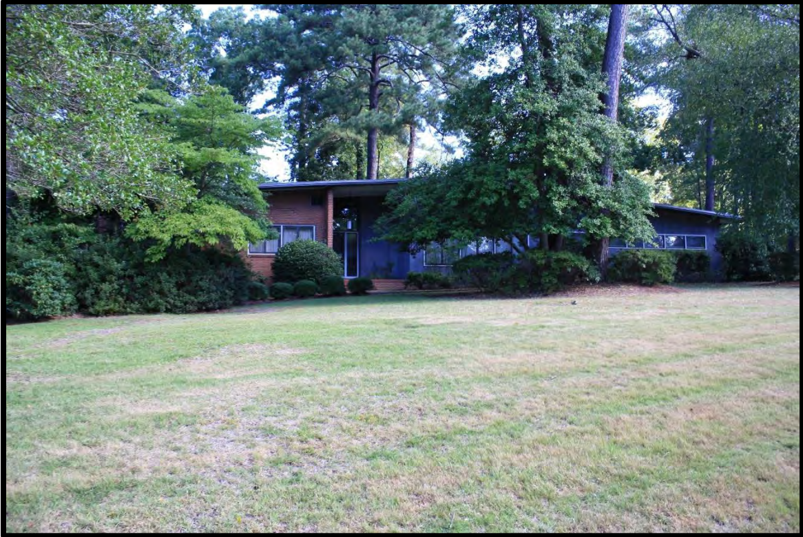
Figure 26: Fleishman House, Looking North.
