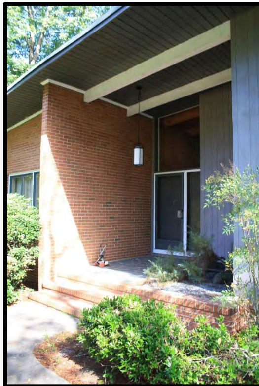
Figure 32: Entry Vestibule, Looking Northwest.
