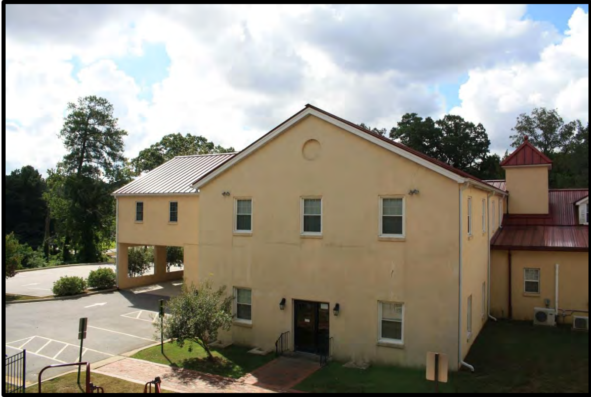
Figure 58: MacPherson Presbyterian Church, Fellowship Hall, Looking Southeast.
