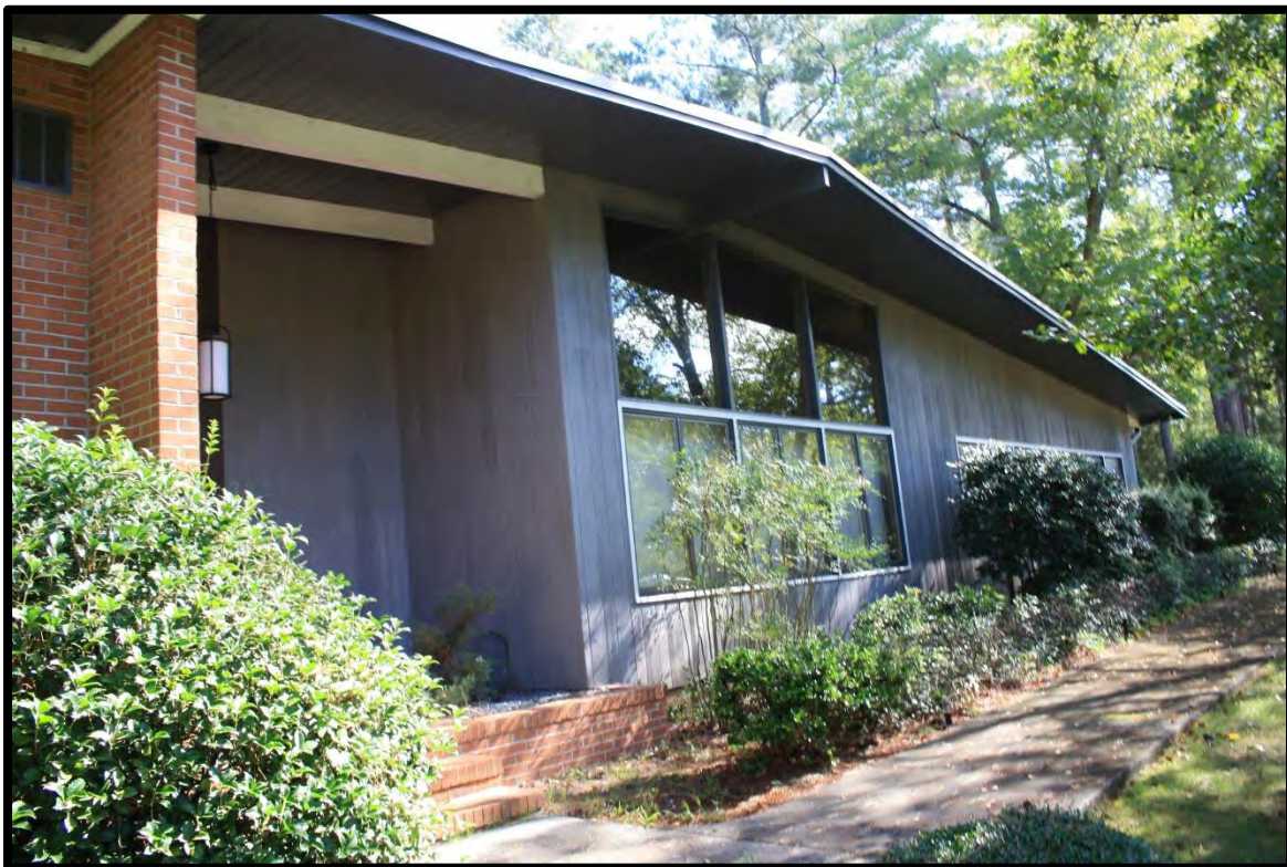
Figure 33: Façade Fenestration Detail, Looking North-Northeast.
