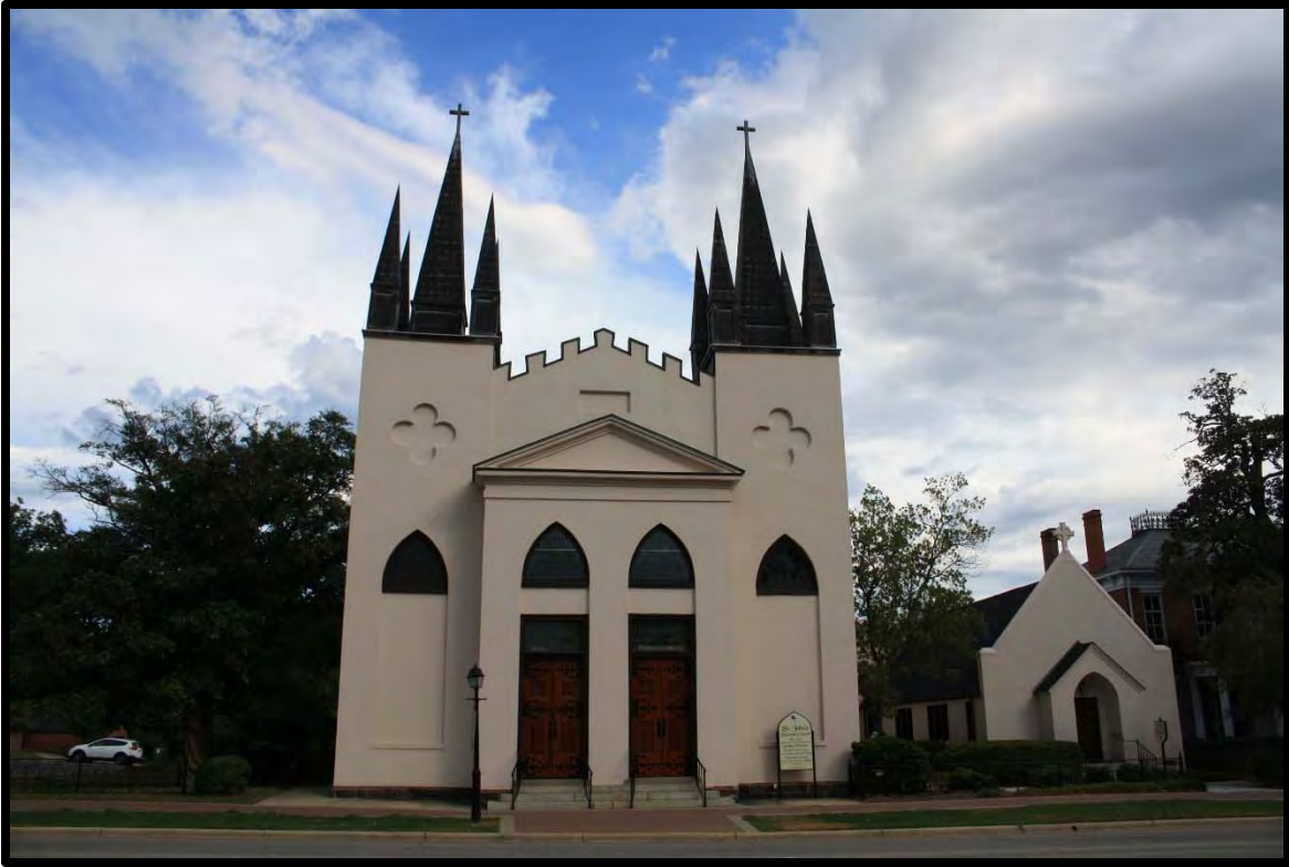
Figure 76: St. John's Episcopal Church (CD0011), Looking East.
