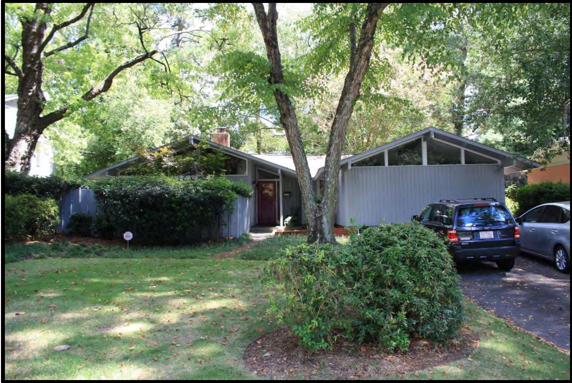
Figure 40: 1437 Pine Valley Loop, Looking East.
