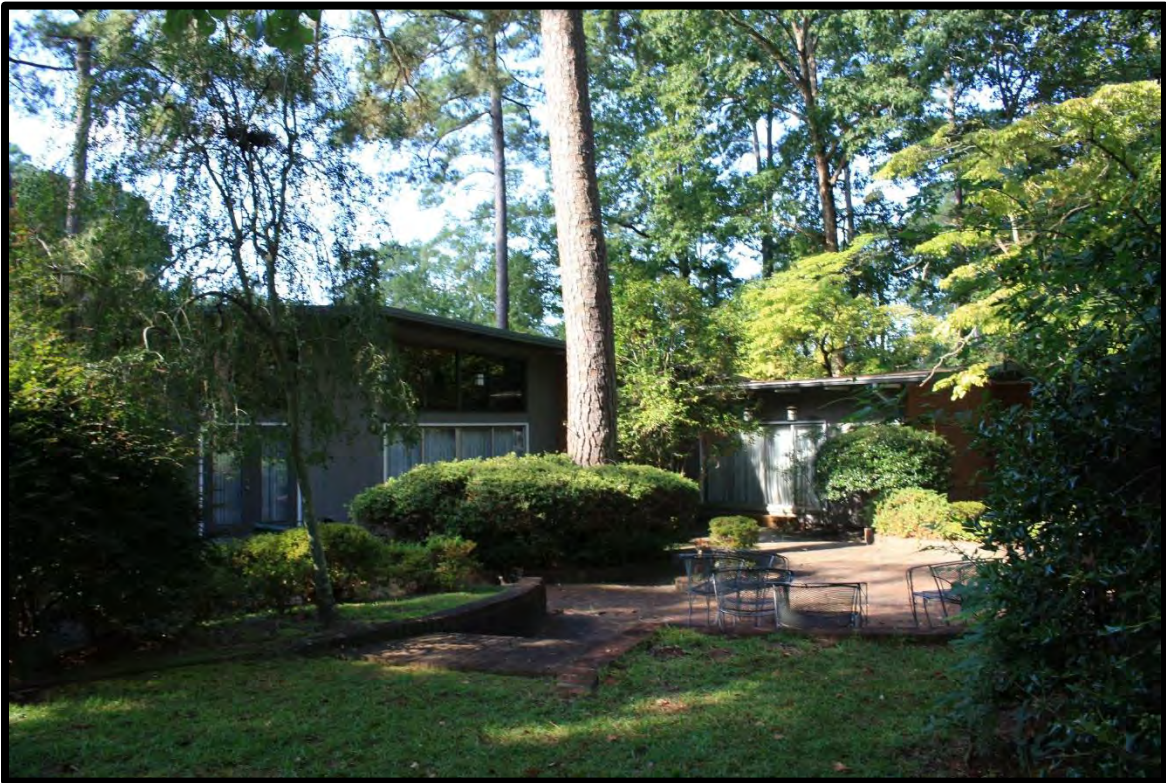
Figure 35: Fleishman House, Looking Southwest.
