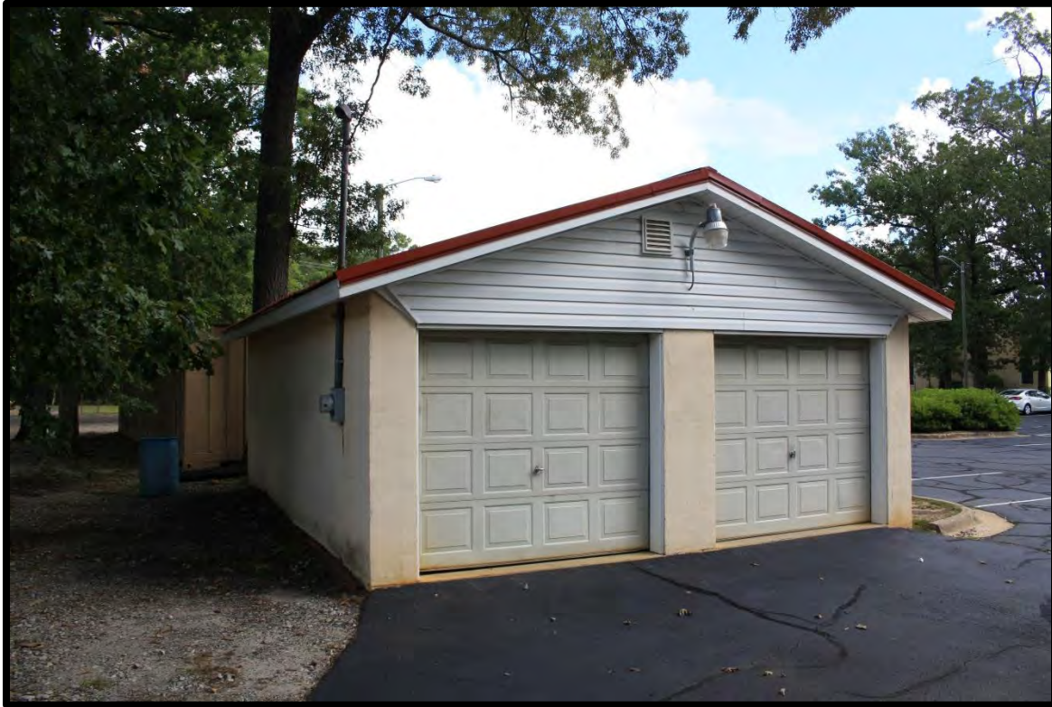
Figure 67: Garage, Looking Northeast.
