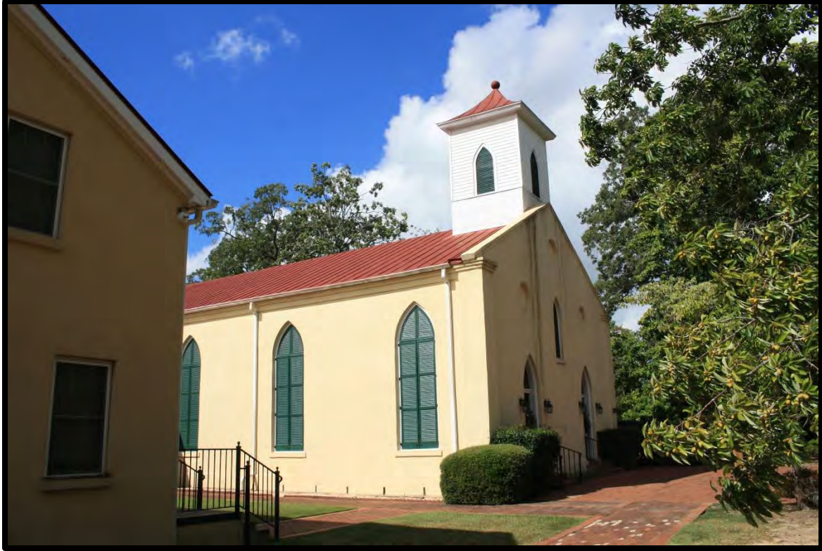
Figure 49: Nave, Looking Southwest.
