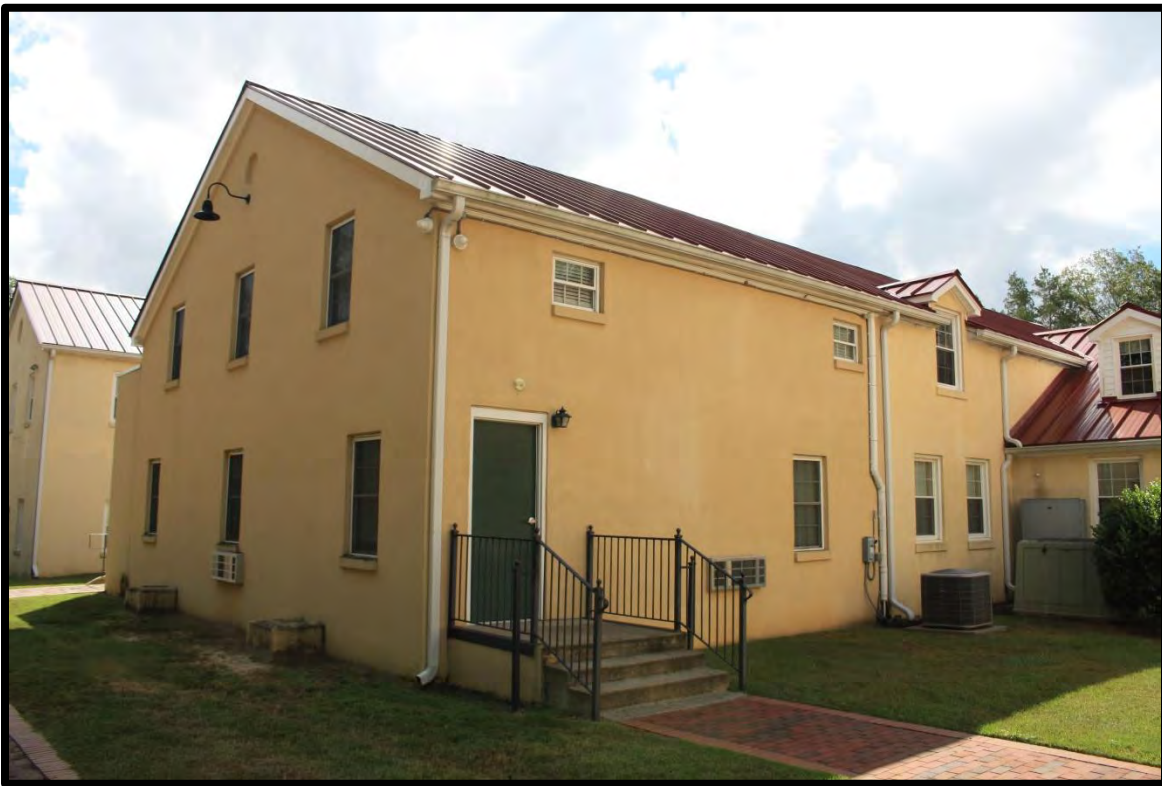
Figure 54: MacPherson Presbyterian Church, Education Wing, Looking Southeast.
