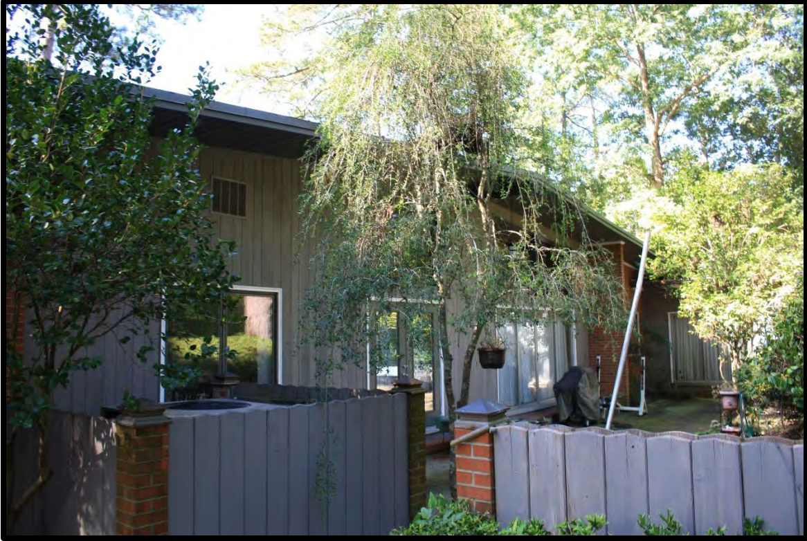
Figure 28: Concrete Patio, Looking Southwest.
