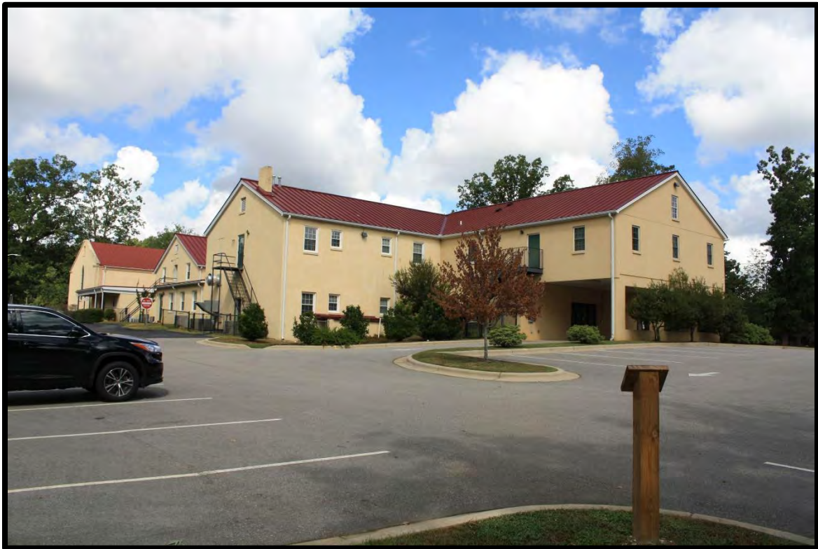
Figure 59: MacPherson Presbyterian Church, Fellowship Hall, Looking Northwest.
