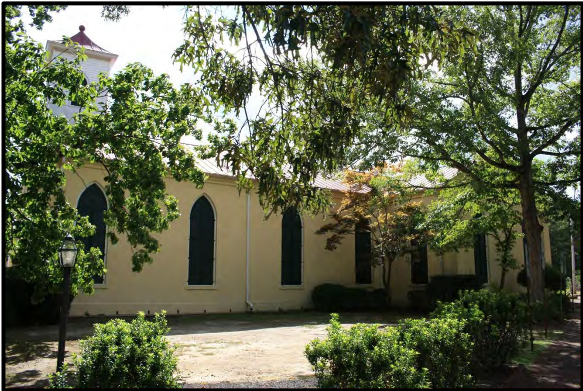
Figure 50: Nave, Looking Southeast.
