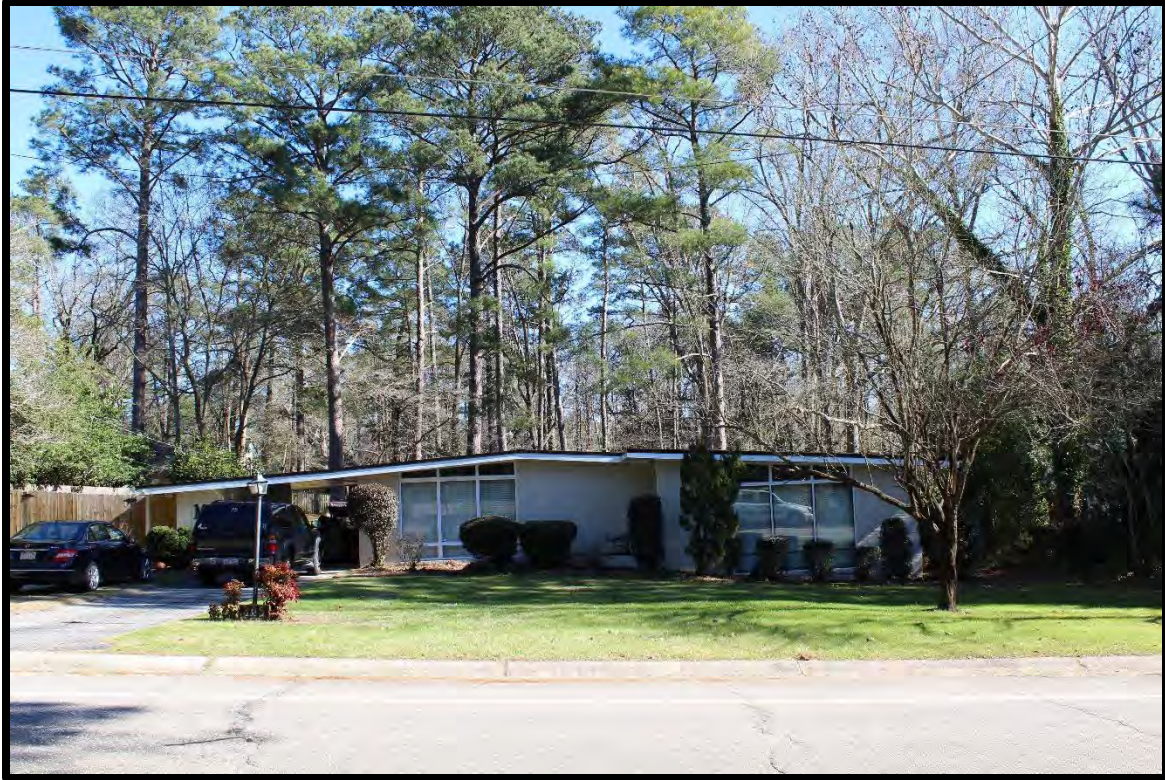
Figure 38: 305 Murray Hill Road, Looking East-Southeast.
