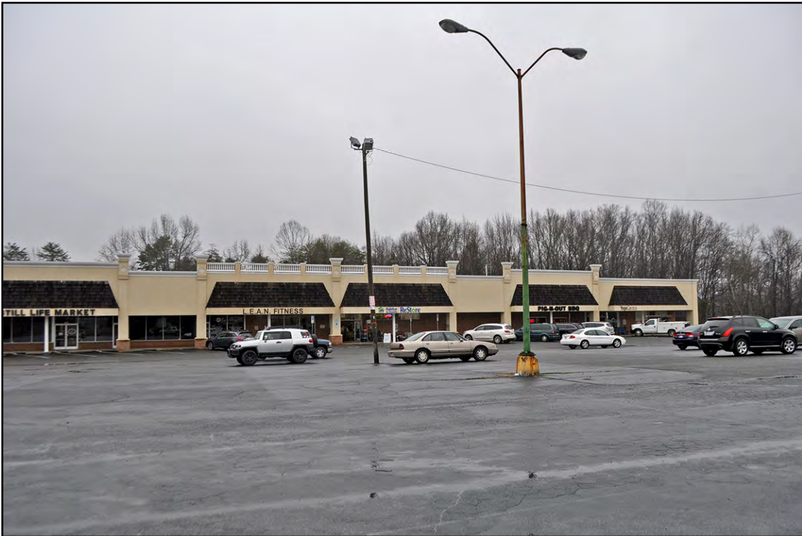
PLATE 42: Shopping Plaza Building Sharing Parcel with Lewis Laugenour House, South Elevation, Forsyth County, North Carolina
