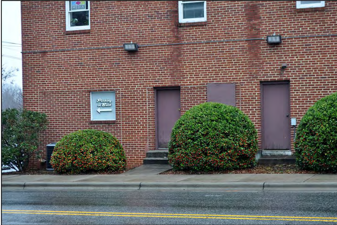
PLATE 25: Jennings Building (FY9063), Detail of Bricked-over Garage Openings, Looking East, Forsyth County, North Carolina
