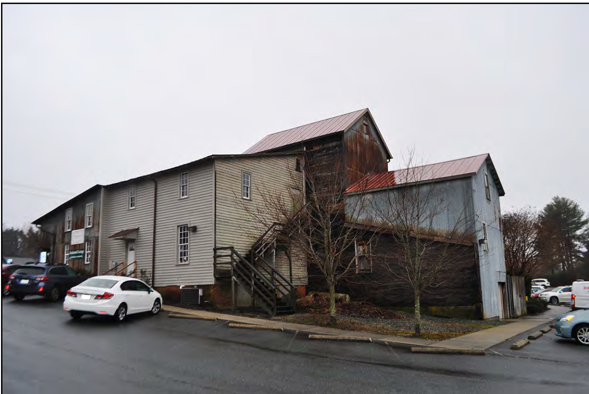
PLATE 13: Lewisville Roller Mills (FY1446), Oblique View of East and North Elevations, Looking Southwest, Forsyth County, North Carolina
