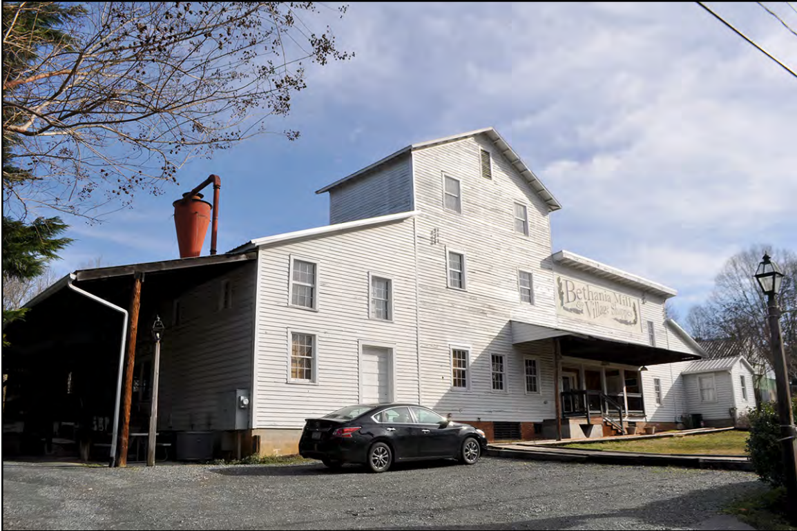
PLATE 18: The Former Lehman and Butner Roller Mill (now Bethania Mill & Village Shoppes) (FY0067), Looking Northeast, Forsyth County, North Carolina
