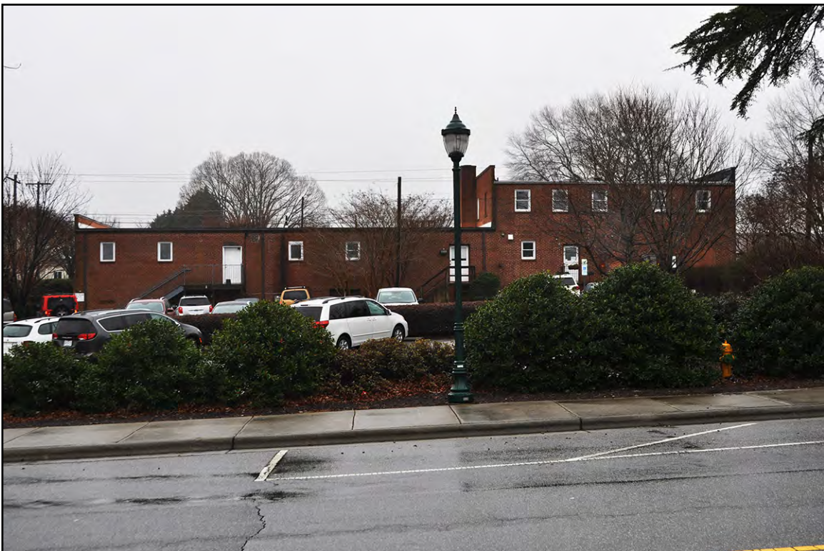
PLATE 23: Jennings Building (FY9063), North Elevation, Looking South, Forsyth County, North Carolina
