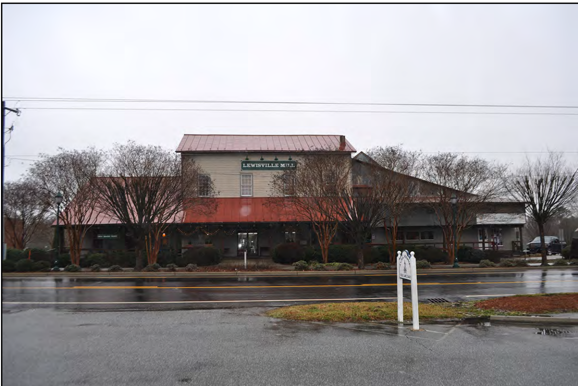
PLATE 11: Lewisville Roller Mills (FY1446), South Elevation, Looking North, Forsyth County, North Carolina
