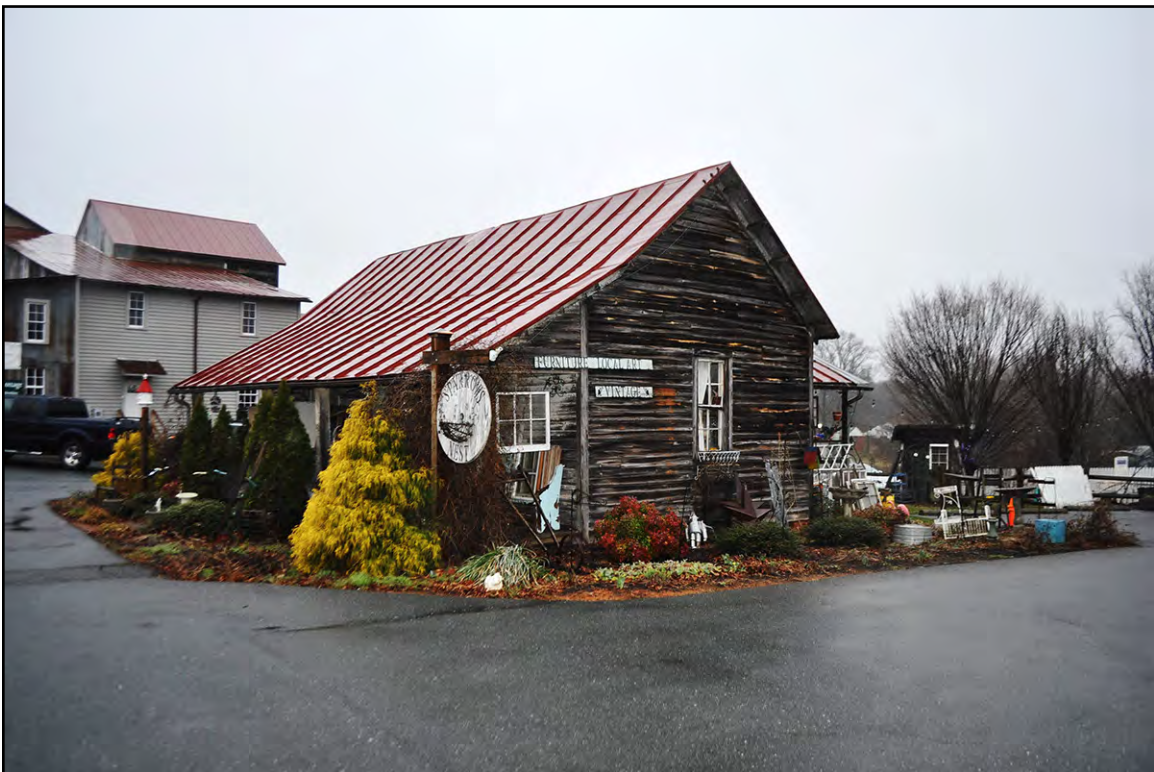
PLATE 4: Sprinkle-Jennings House (FY9060), Oblique View of South and East Elevations, Looking Northwest, Forsyth County, North Carolina
