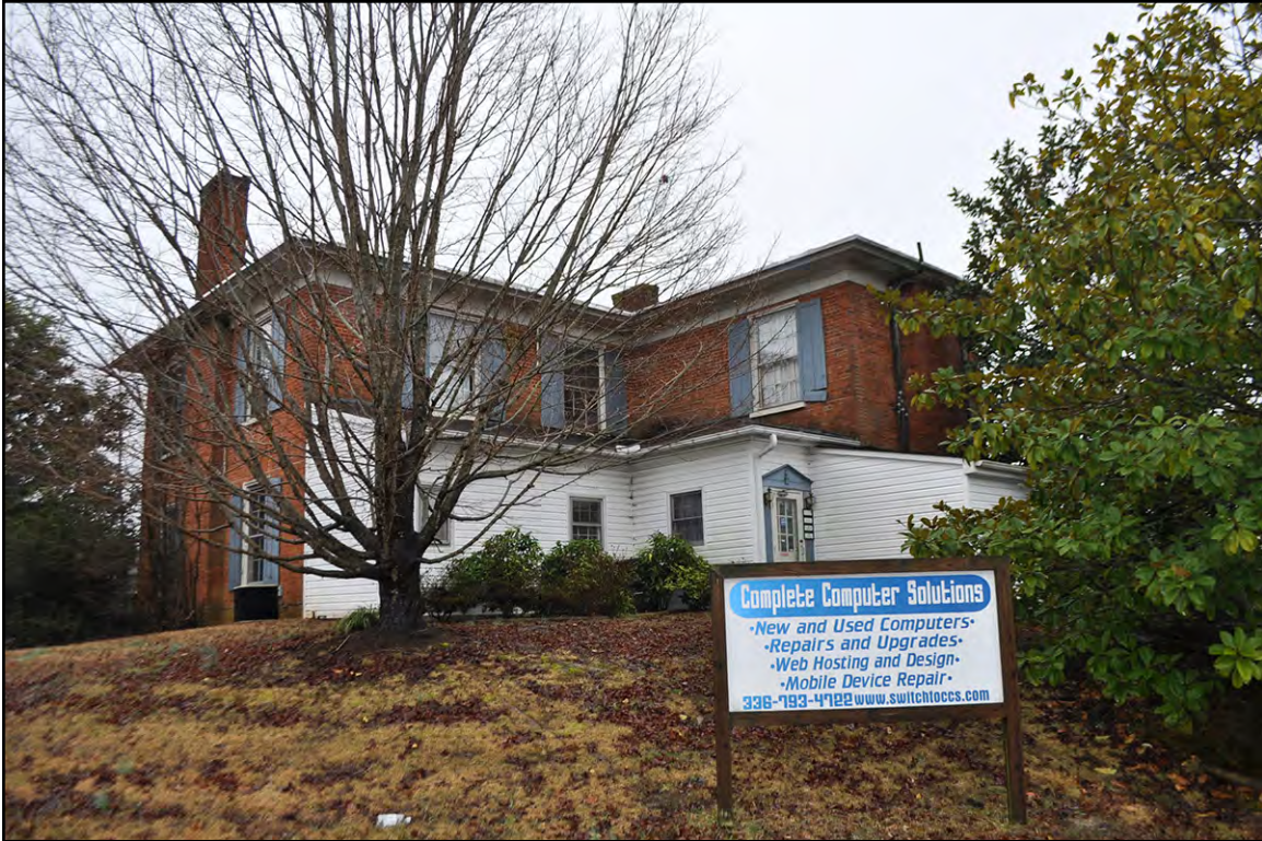
PLATE 38: Lewis Laugenour House (FY0134), Oblique View of North and East Elevation, Looking Southwest, Forsyth County, North Carolina
