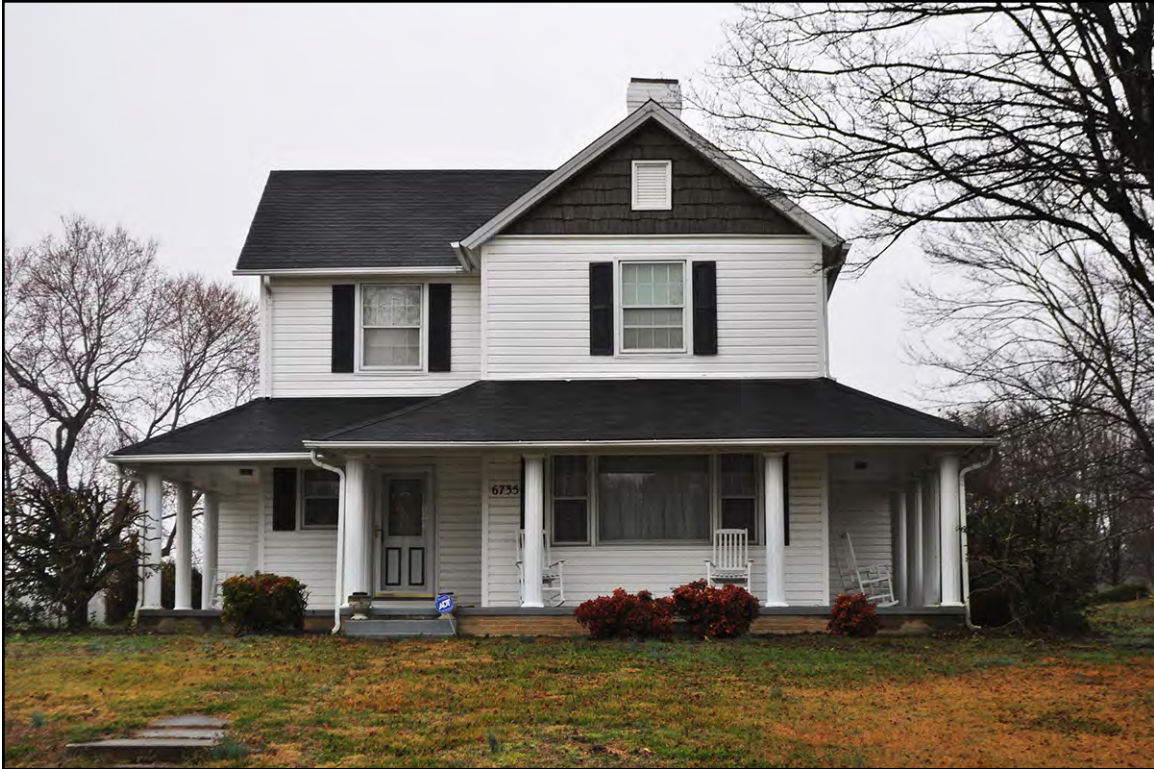
PLATE 46: Charles L. Spough House (FY9085), South Elevation, Looking North, Forsyth County, North Carolina
