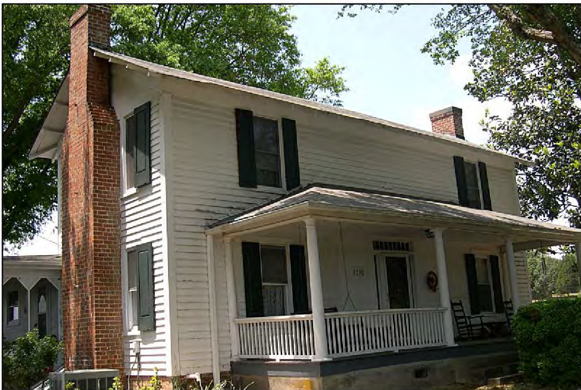
PLATE 34: Theophilus Kimel House (FY0236), Oblique View of West and South Elevations, Forsyth County, North Carolina (NC HPOweb 2019)
