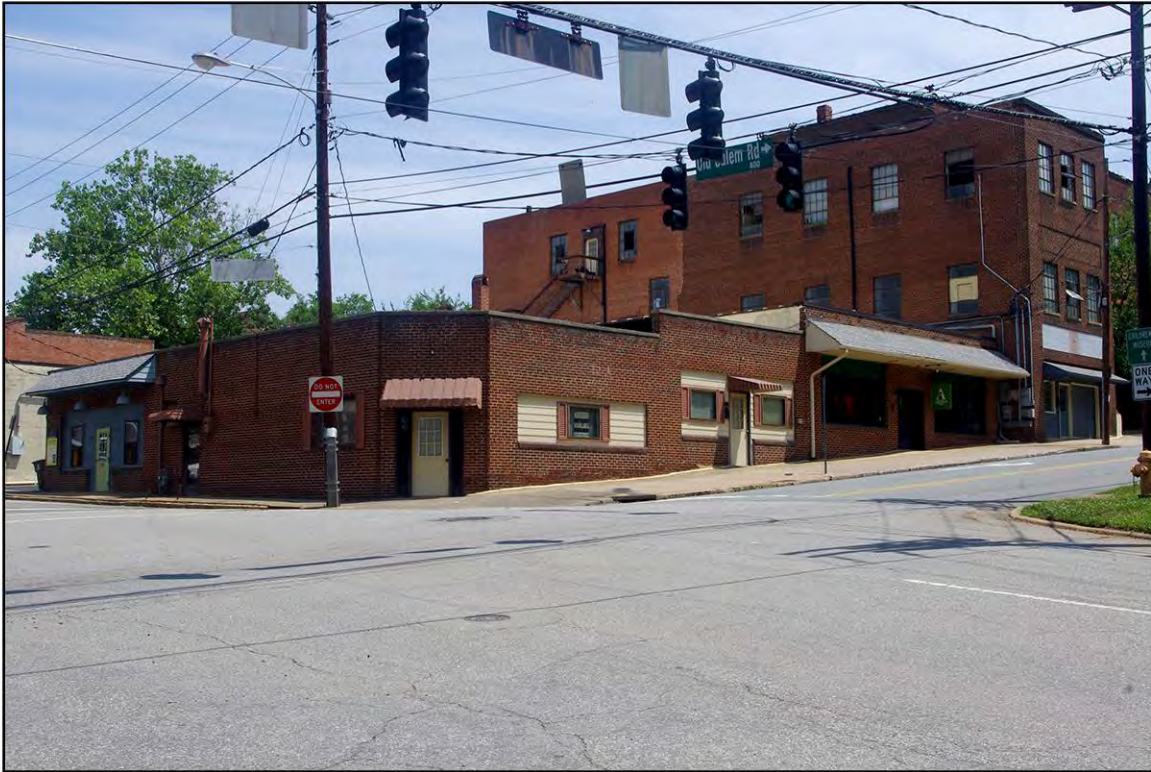
PLATE 28: Commercial Building (FY4262), Oblique View of South Elevation, Forsyth County, North Carolina
