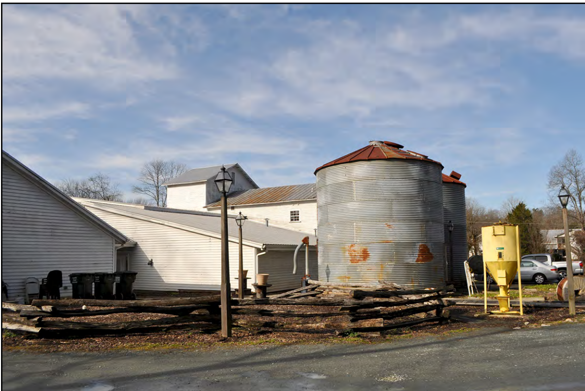
PLATE 19: Silos North of the Former Lehman & Butner Roller Mill (now Bethania Mill & Village Shoppes) (FY0067), Looking Southwest, Forsyth County, North Carolina
