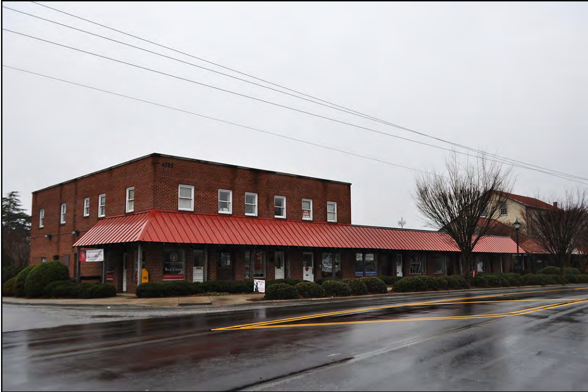
PLATE 22: Jennings Building (FY9063), Oblique View of South and West Elevations, Looking North, Forsyth County, North Carolina
