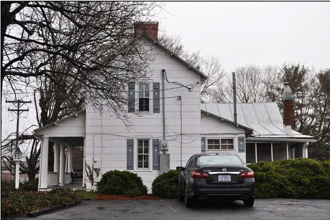
PLATE 31: Omer and Fannie Fulk Conrad House (FY0135), West Elevation, Looking East, Forsyth County, North Carolina
