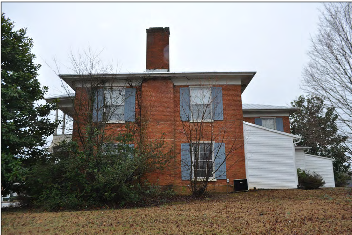
PLATE 39: Lewis Laugenour House (FY0134), East Elevation, Looking West, Forsyth County, North Carolina
