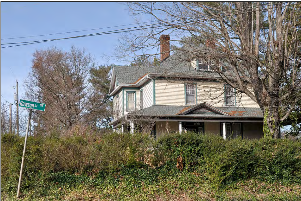
PLATE 52: House (FY1205), East Elevation, Looking Northwest, Forsyth County, North Carolina
