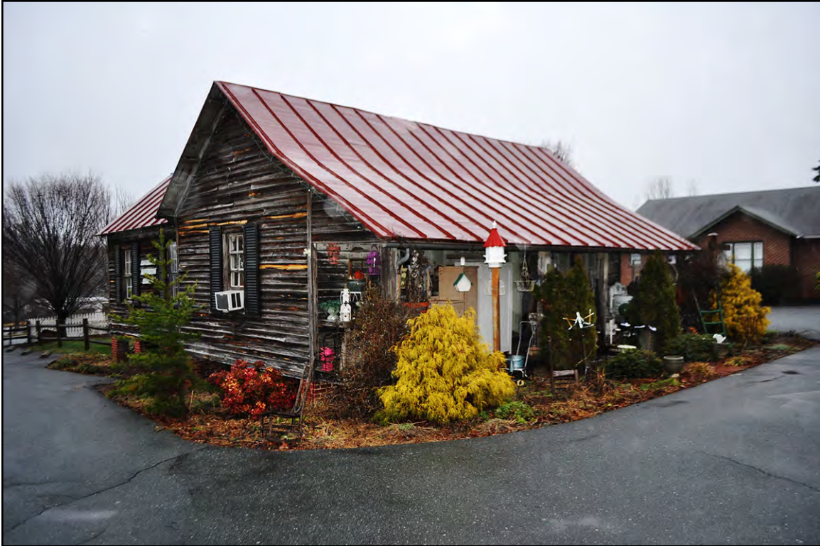
PLATE 1: Sprinkle-Jennings House (FY9060), Oblique View of South and West Elevations, Looking Northeast, Forsyth County, North Carolina
