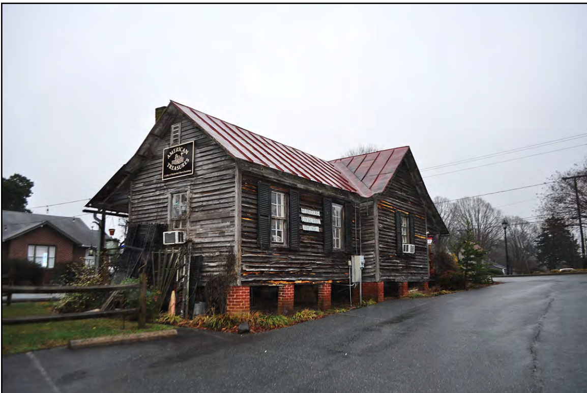
PLATE 2: Sprinkle-Jennings House (FY9060), Oblique View of West and North Elevations, Looking Southeast, Forsyth County, North Carolina
