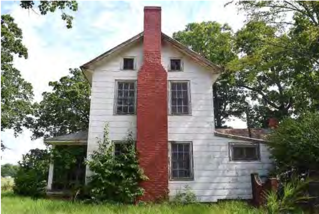
Alexander Farm, Alexander House, South Gable End, Looking North.
