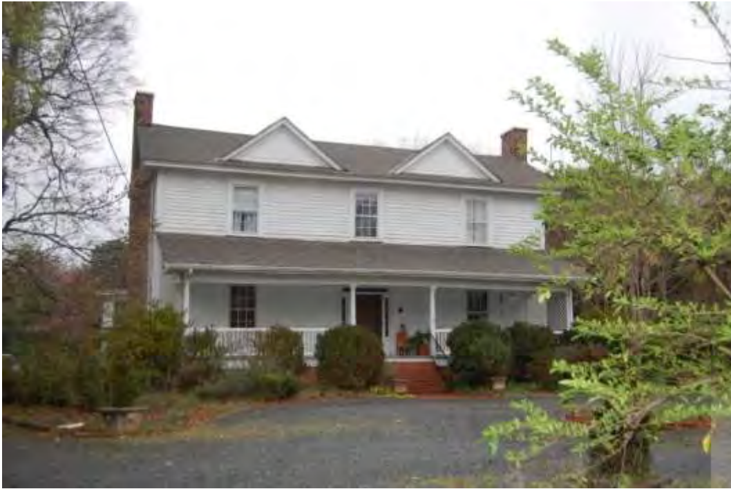
John Hunter House, ca. 1869, 5607 Sardis Road, Looking North.
