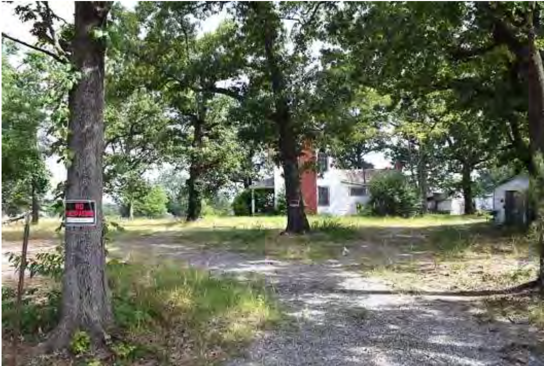
Alexander Farm, Overall View of House Site, Looking North from Westmoreland Road.
