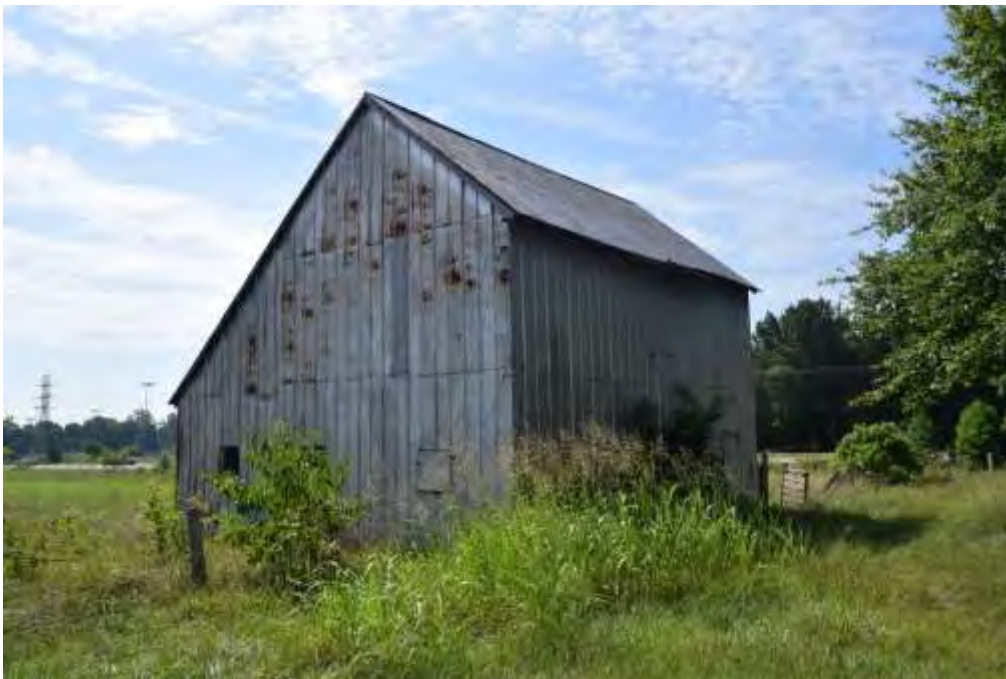
Alexander Farm, Barn No. 2, Looking Southeast.
