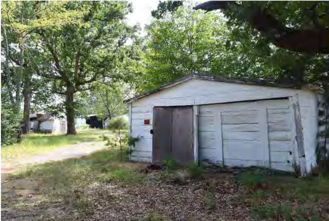
Alexander Farm, Garage (Foreground), Shed, and Equipment Shed (Background), Looking East.
