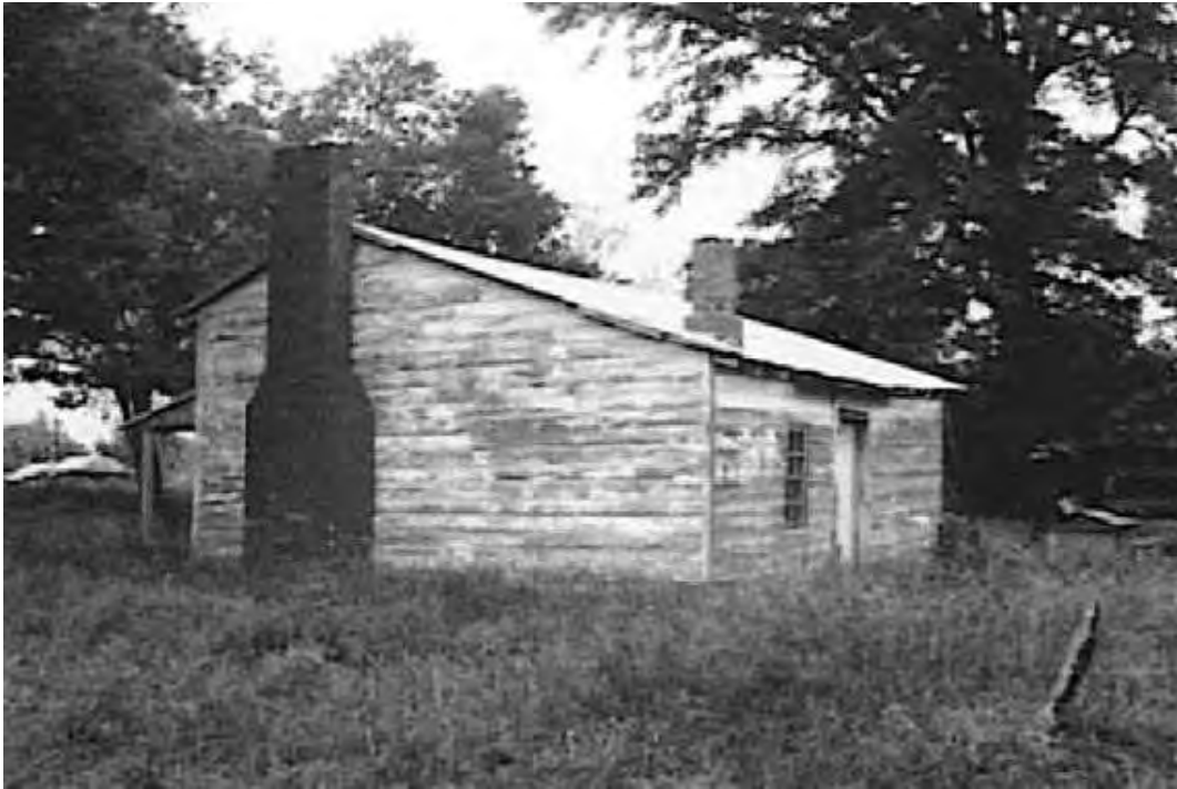
Alexander Farm Tenant House, Side (South) and Rear (East) Elevations. Source: HPO File Photograph, 2002.
