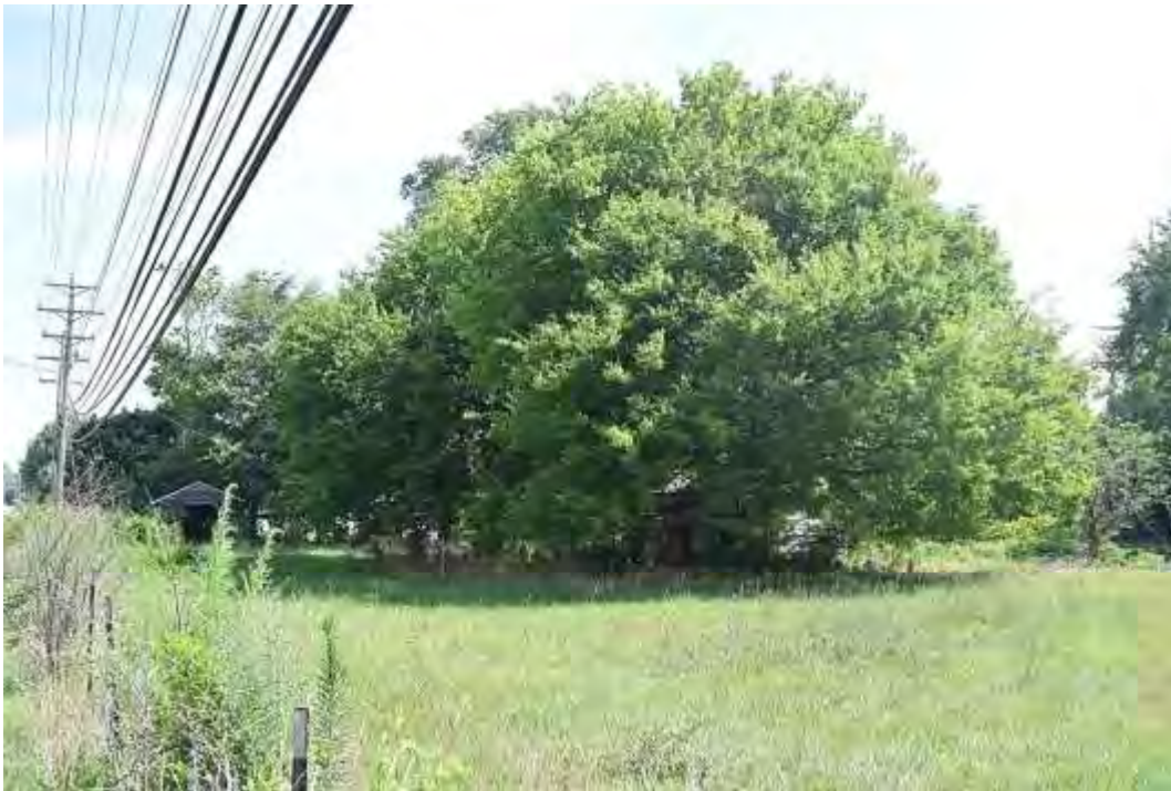
Alexander Farm Tenant House, House and Setting, House Shaded by Pecan Trees and Garage in Left Background, Looking North Along West Catawba Avenue.
