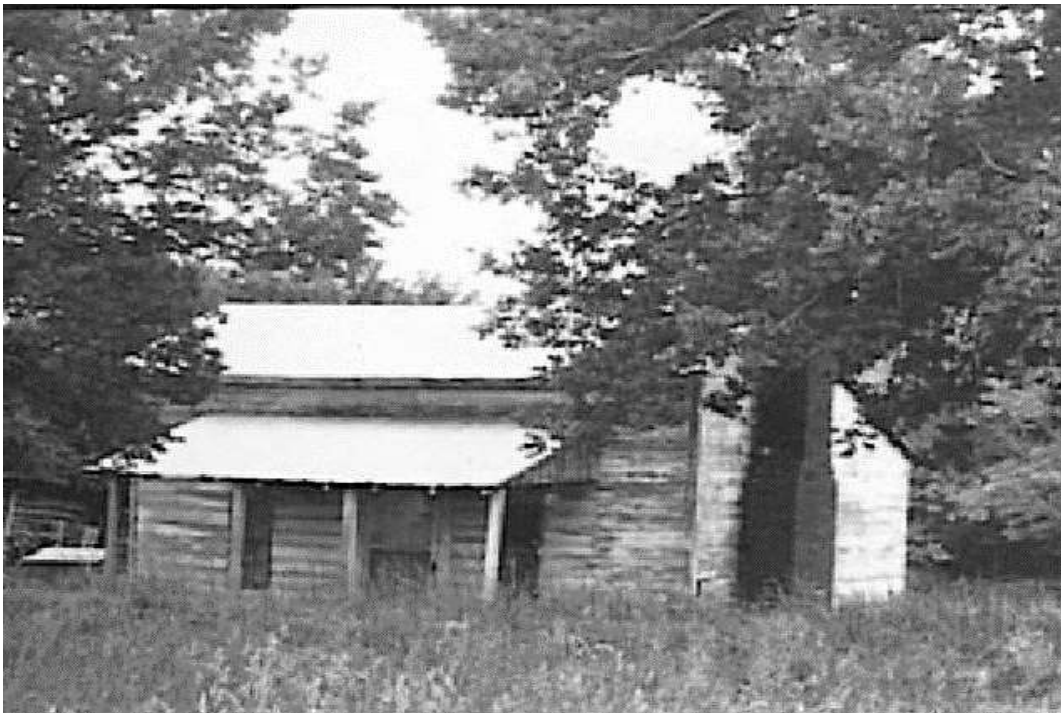
Alexander Farm Tenant House, Façade. Source: HPO File Photograph, 2002.
