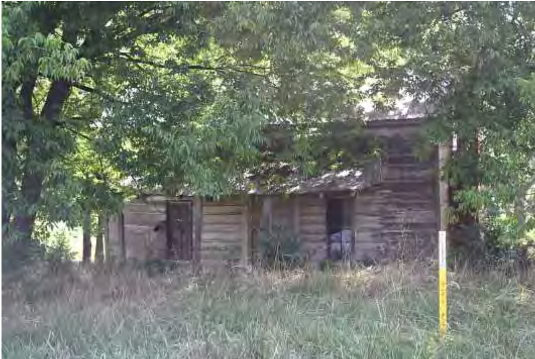
Alexander Farm Tenant House, Façade (West Elevation), Looking East from West Catawba Avenue.
