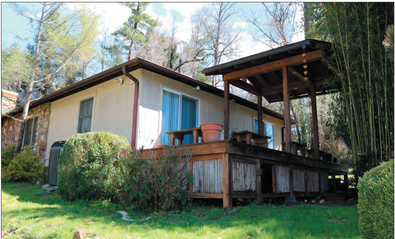
Figure 4.7. Johnson House, Bunk House Wing, South Elevation, Facing Northeast
