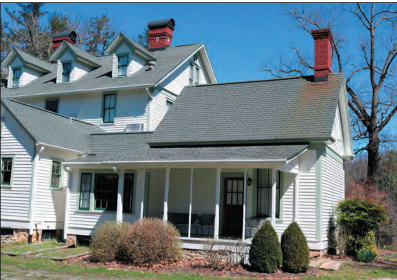
Figure 3.11. W.J. Davis House, Attached Kitchen or Servants' Quarters
