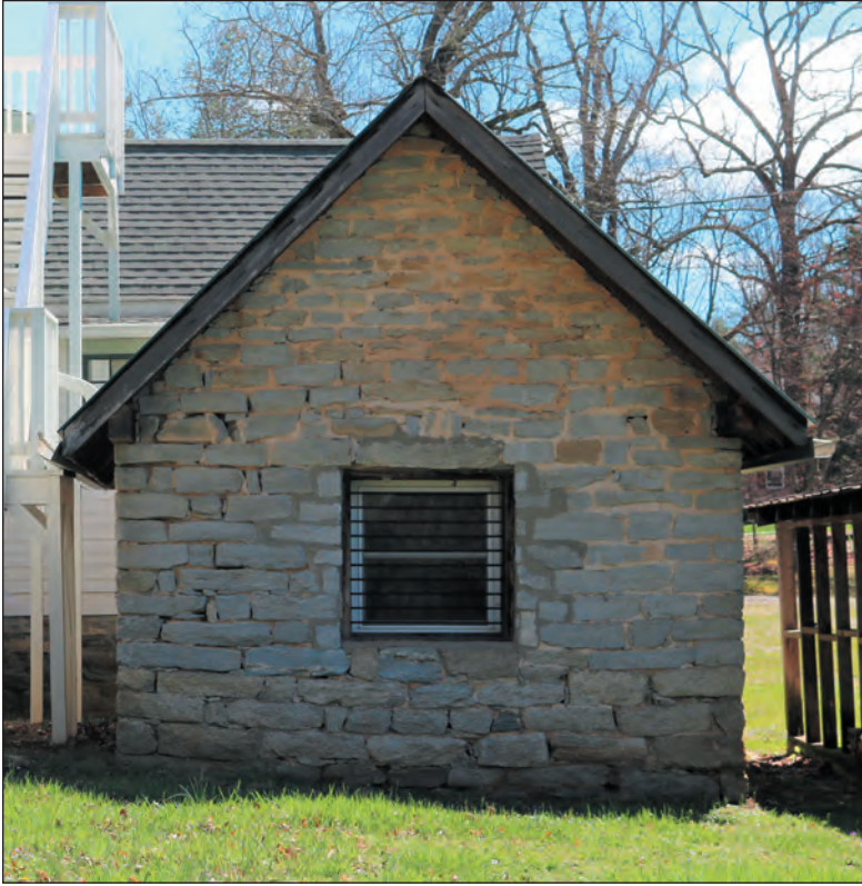
Figure 3.19. Icehouse, Facing East
