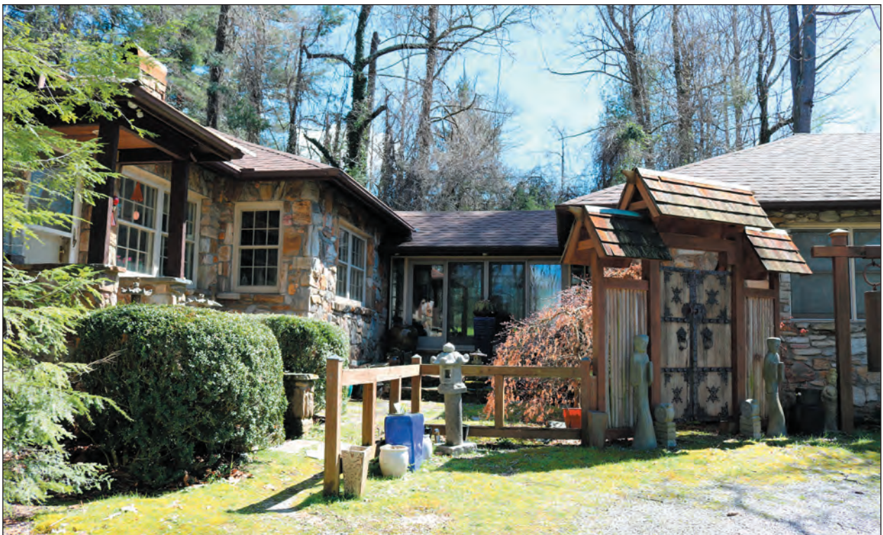
Figure 4.4. Johnson House, Courtyard, Facing Northeast
