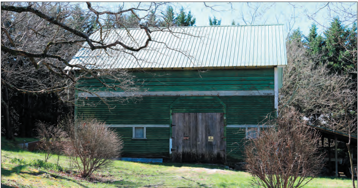
Figure 3.23. Barn, Facing Southeast
