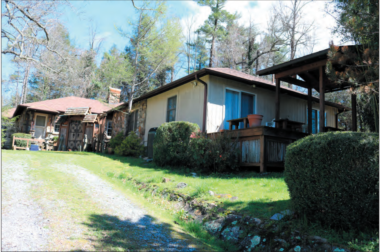
Figure 4.3. Johnson House, Façade and South Elevation, Facing Northeast
