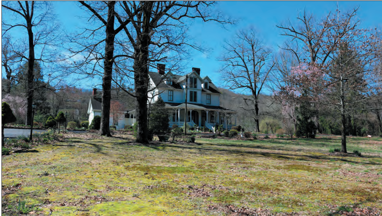
Figure 3.1. W.J. Davis House, Façade and Setting, Facing Southwest.
