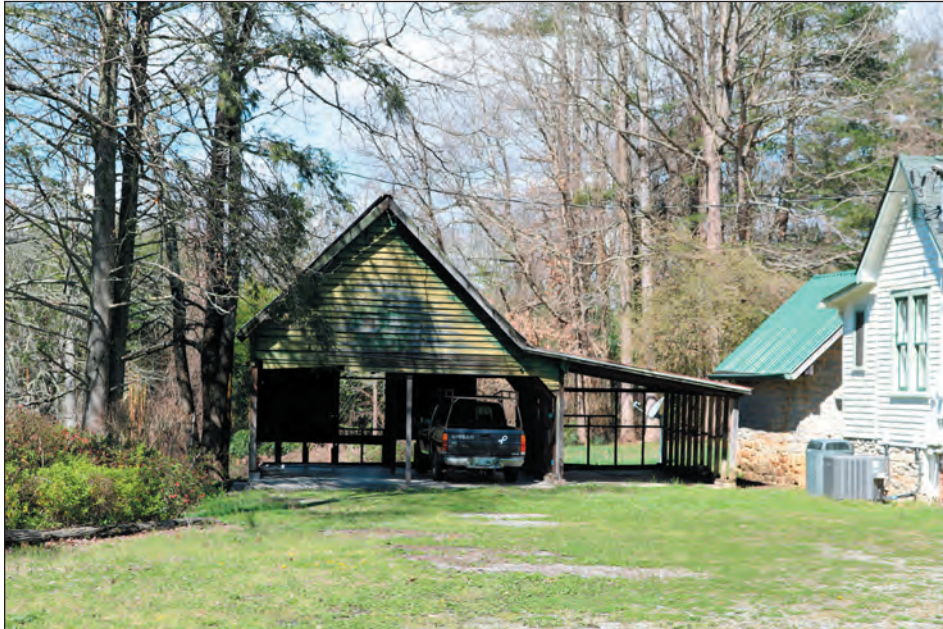
Figure 3.21. Garage, Facing West
