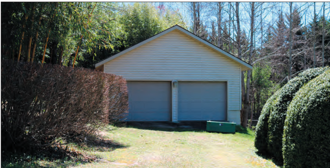
Figure 4.9. Garage, Facing Southeast
