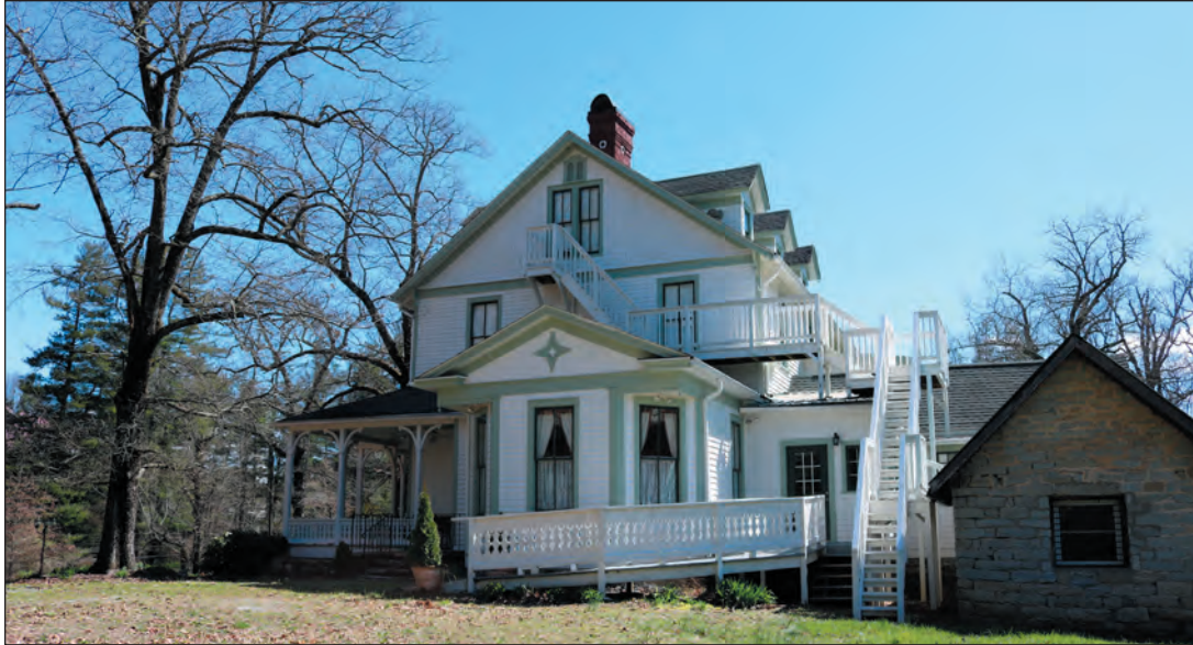
Figure 3.7. W.J. Davis House, West Elevation and Egress at Southwest Corner
