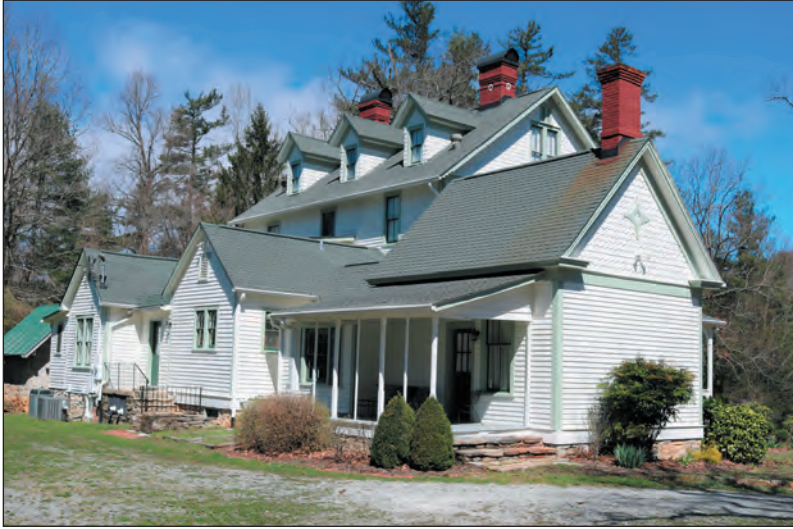
Figure 3.9. W.J. Davis House, South Elevation, Facing Northwest
