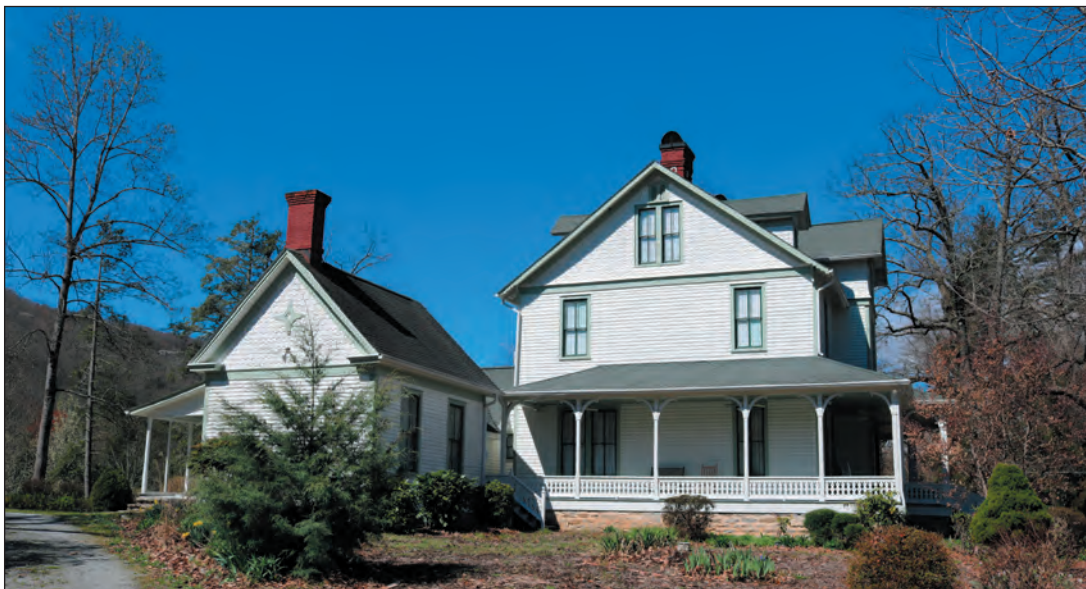
Figure 3.8. W.J. Davis House, East Elevation
