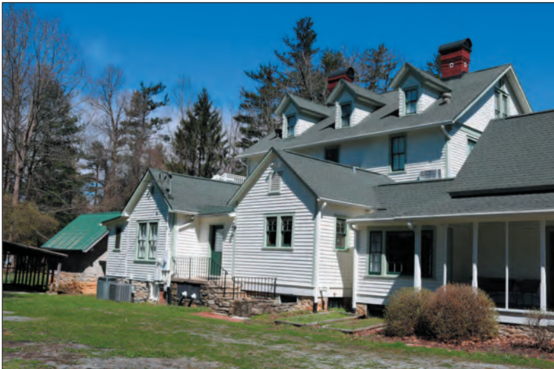
Figure 3.10. W.J. Davis House, South Elevation, West End
