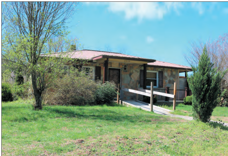
Figure 4.13. 2400 East Morningside Drive, Facing Southwest
