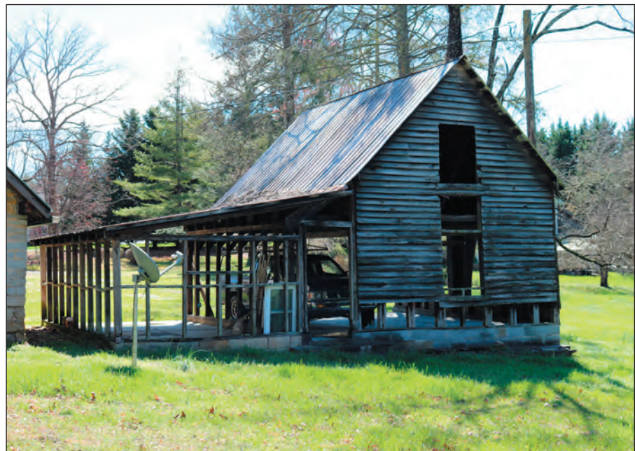
Figure 3.22. Garage, Facing Southeast
