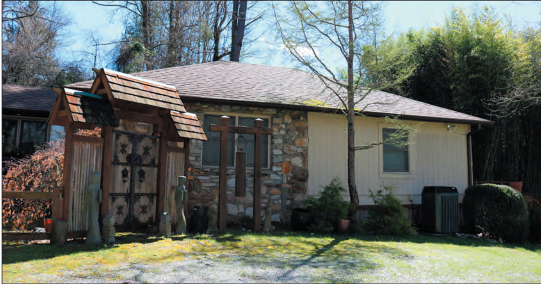
Figure 4.8. Johnson House, Bunk House Wing, Facing Southeast
