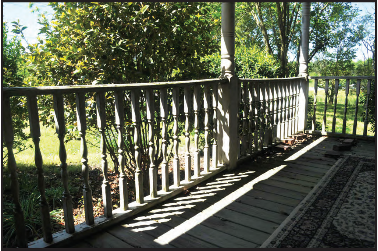
Figure 15. Replacement Posts and Balustrade on Front Porch.
