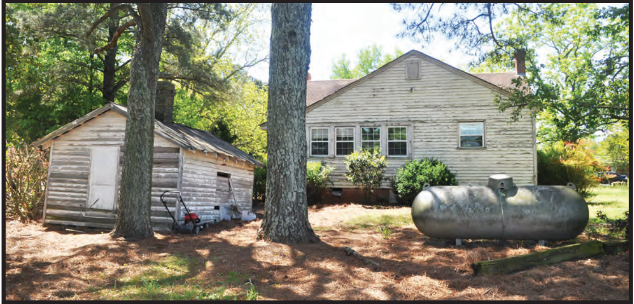
Figure 5. View of Rear Yard Looking South
