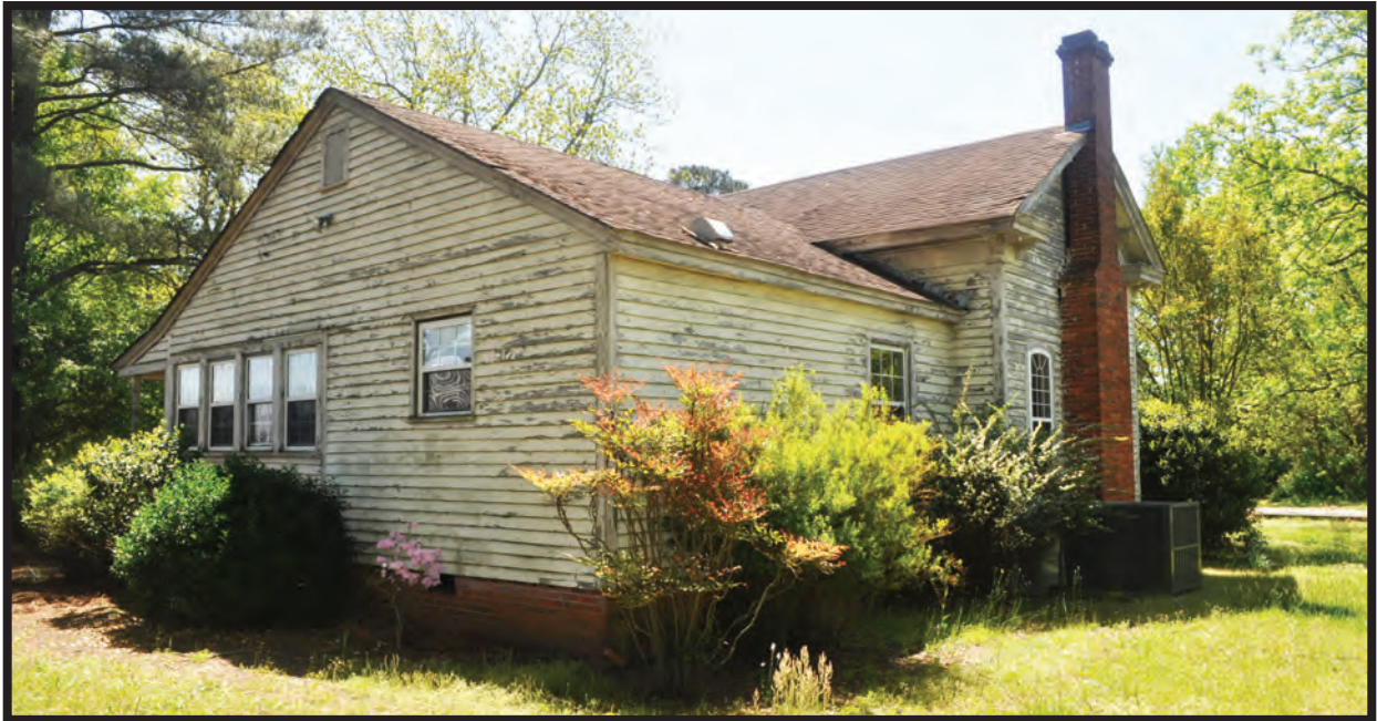
Figure 12. Rear/North and West Side
