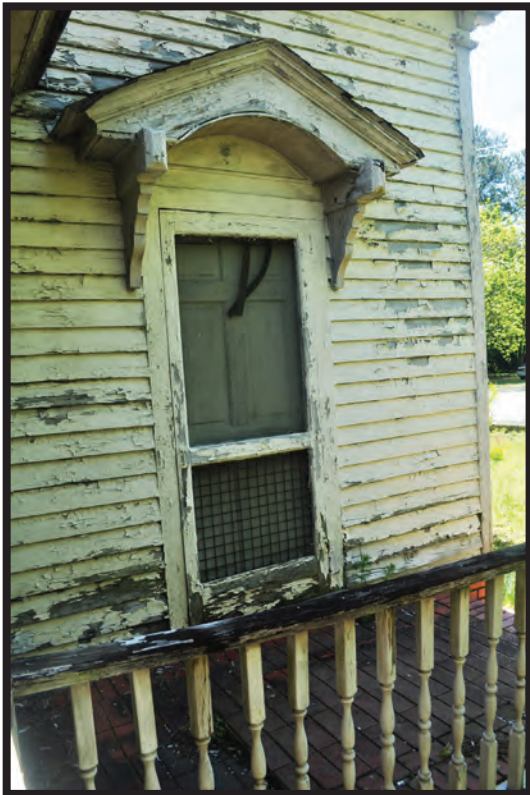
Figure 18. Circa 1940s Entry on West Side of Front Wing
