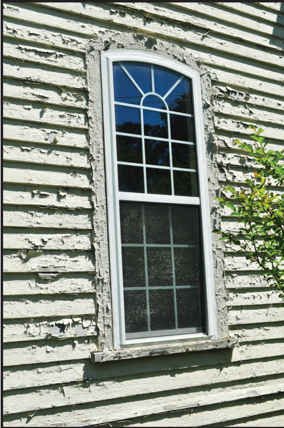
Figure 14. Typical Vinyl Replacement Window on Circa 1885 Section
