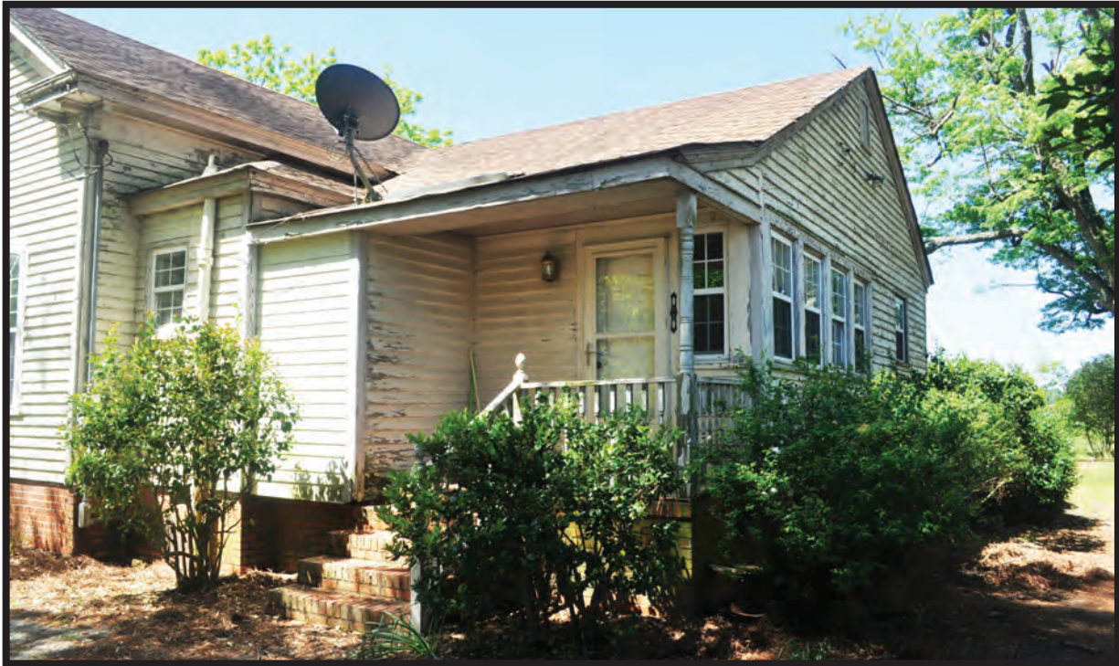
Figure 10. West Side of 1940s Kitchen Addition
