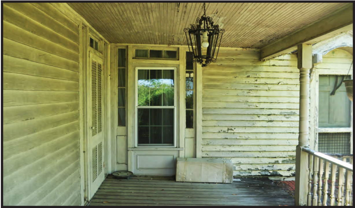
Figure 17. Original West Entry of Front Wing, altered in 2002.
