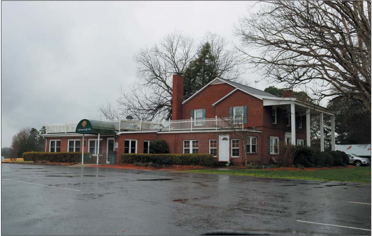
Figure 48. The Lakewood Golf Course and Clubhouse, Facing East
