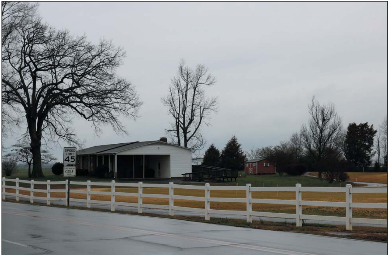
Figure 38. The Jessica Keel House, Facing Northwest
