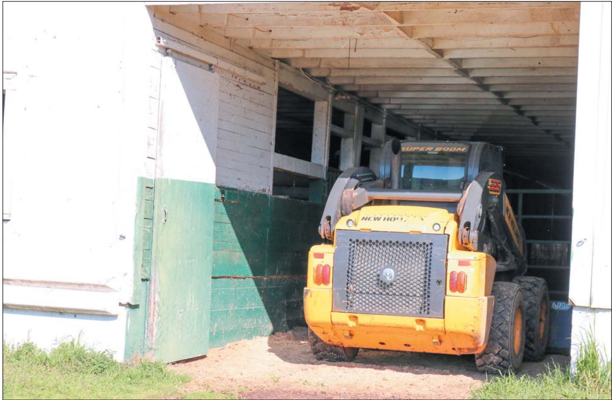
Figure 15. Stamey Farm Barn Interior View Through Center Aisle Doors, Facing North
