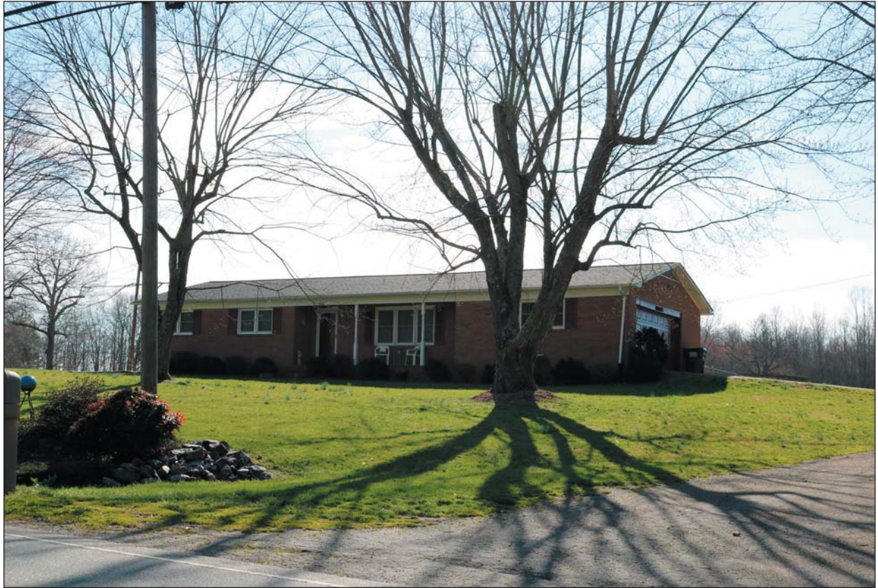
Figure 25. Jeffrey L. Morrow House, Northwestern Oblique
