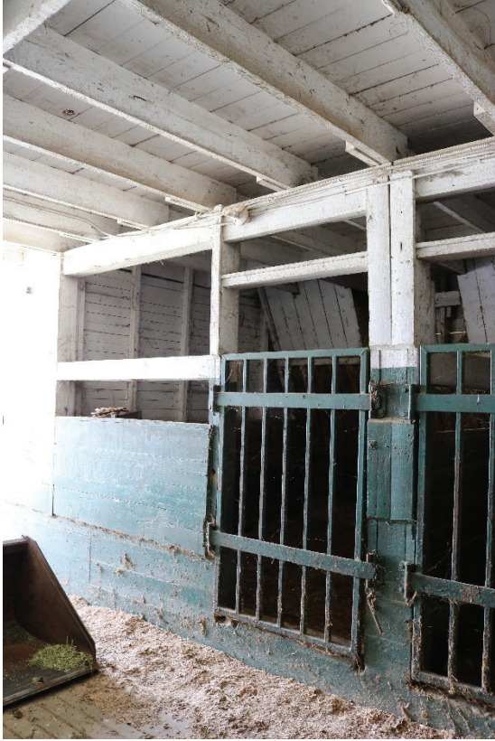
Figure 3. Stamey Barn Original Stalls
