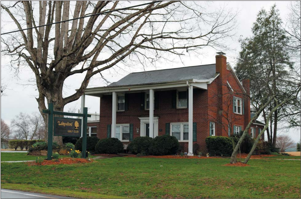
Figure 51. Northwestern Elevation of the Lakewood Golf Course Clubhouse
