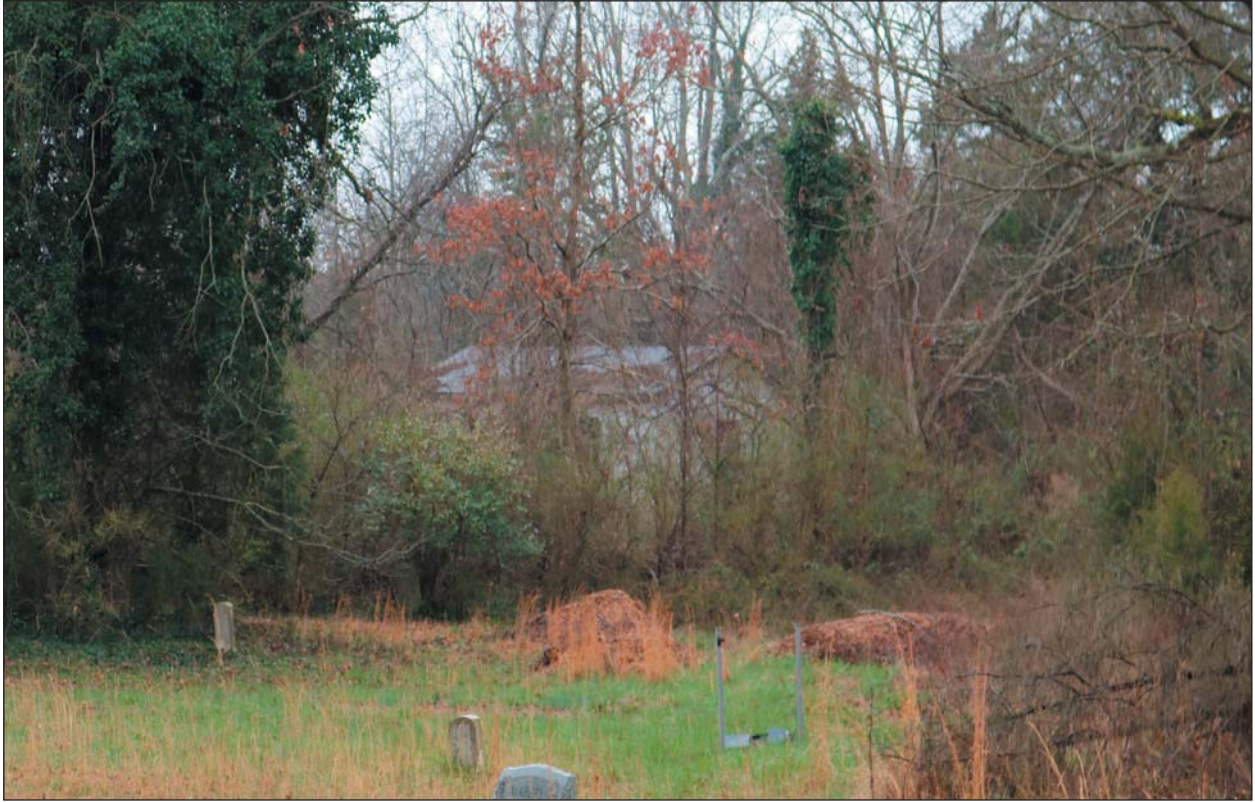
Figure 36. Dilapidated House on John Wayne Tatum's Parcel, Facing South
