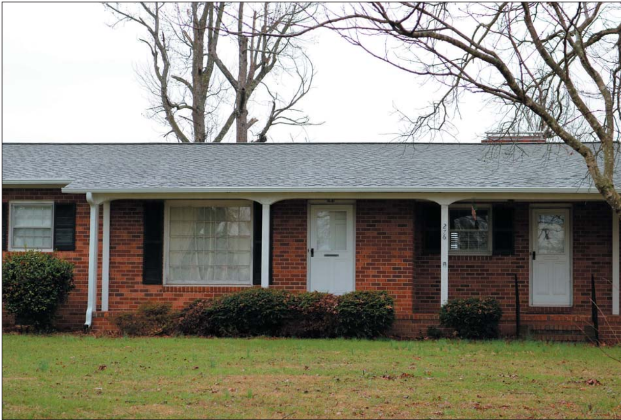
Figure 40. The Jessica Keel House, Façade Detail
