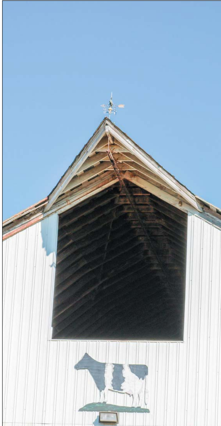
Figure 16. Stamey Farm Barn Interior Through Third-story Hay Loft Access
