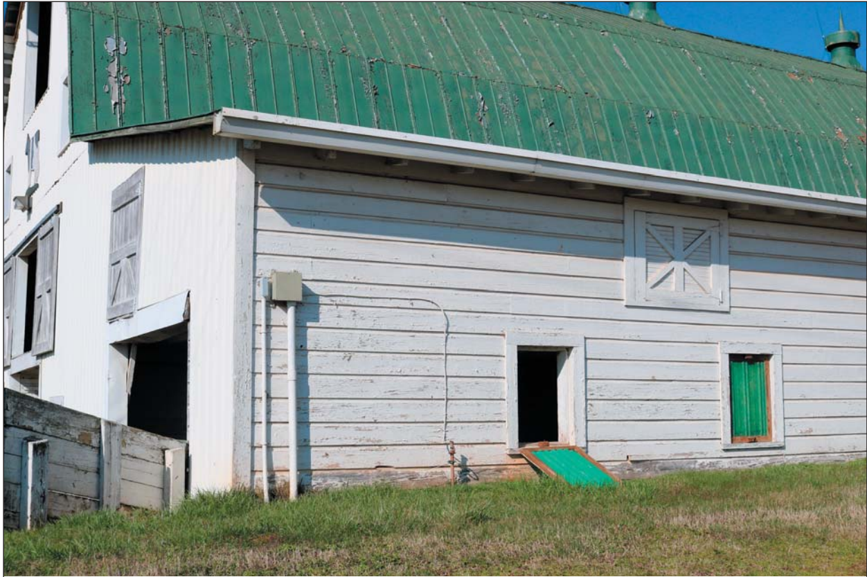
Figure 9. Stamey Farm Barn, Detail of Southeastern Elevation's Cladding and Shuttered Windows
