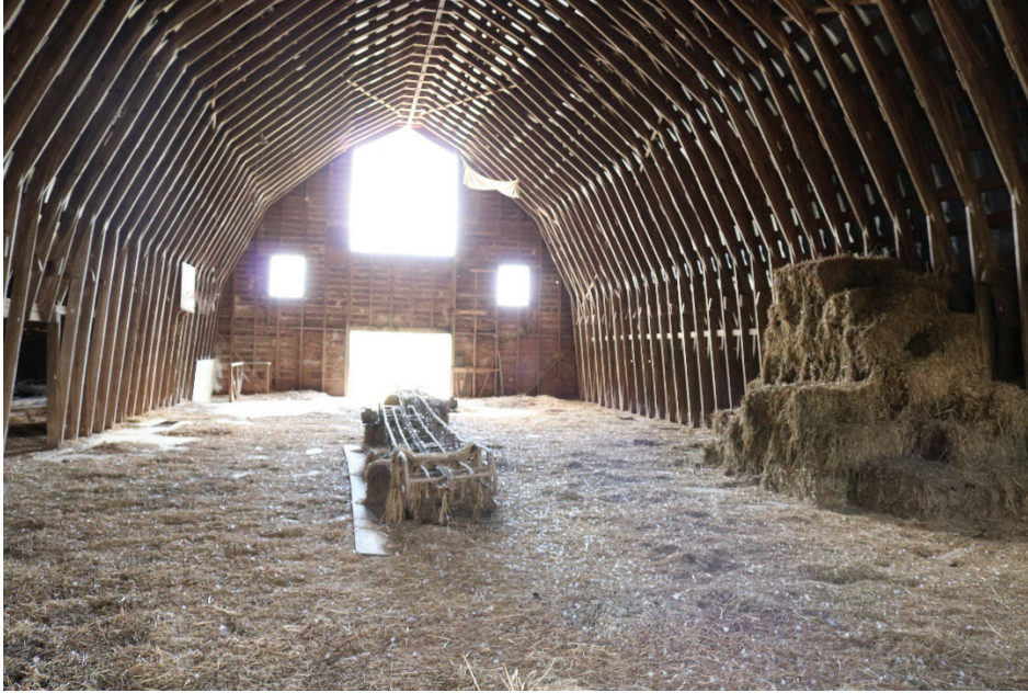
Figure 1. Stamey Barn Upper Loft
