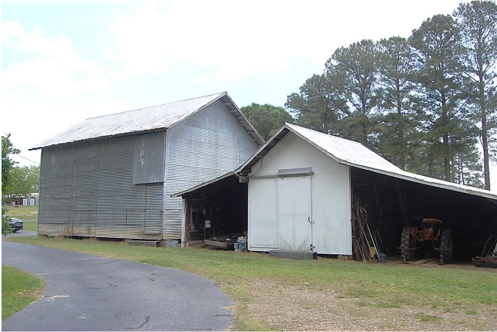
Adams Family House, Packhouse and Prefabricated Shed, Looking East.
