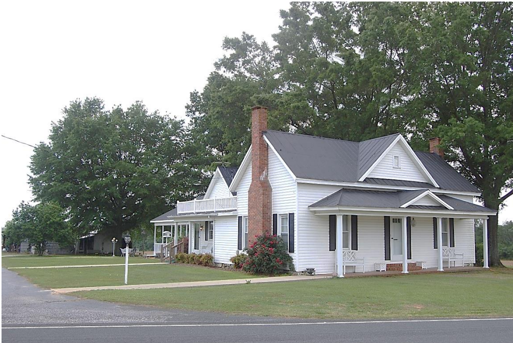
Adams Family House, Overall View, Looking South.
