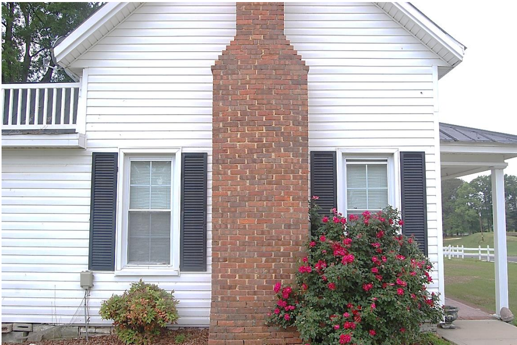
Adams Family House, Side (East) Elevation, Chimney and Replacement Windows, Looking West.
