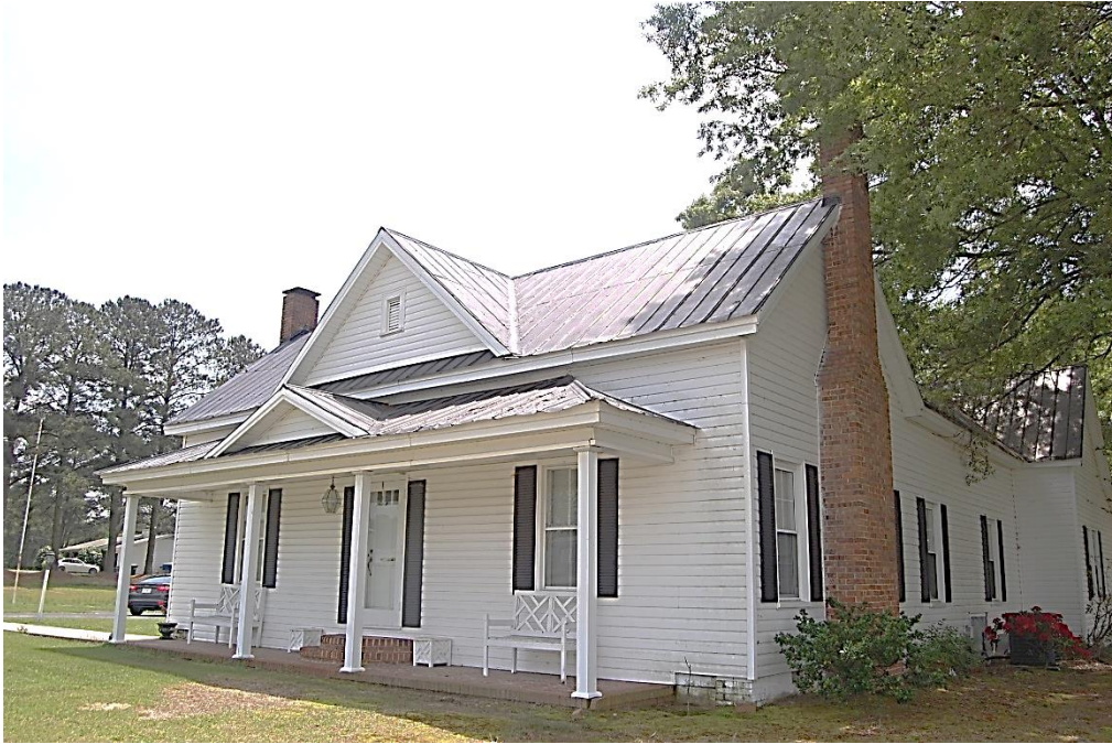
Adams Family House, Façade, Looking Southeast.
