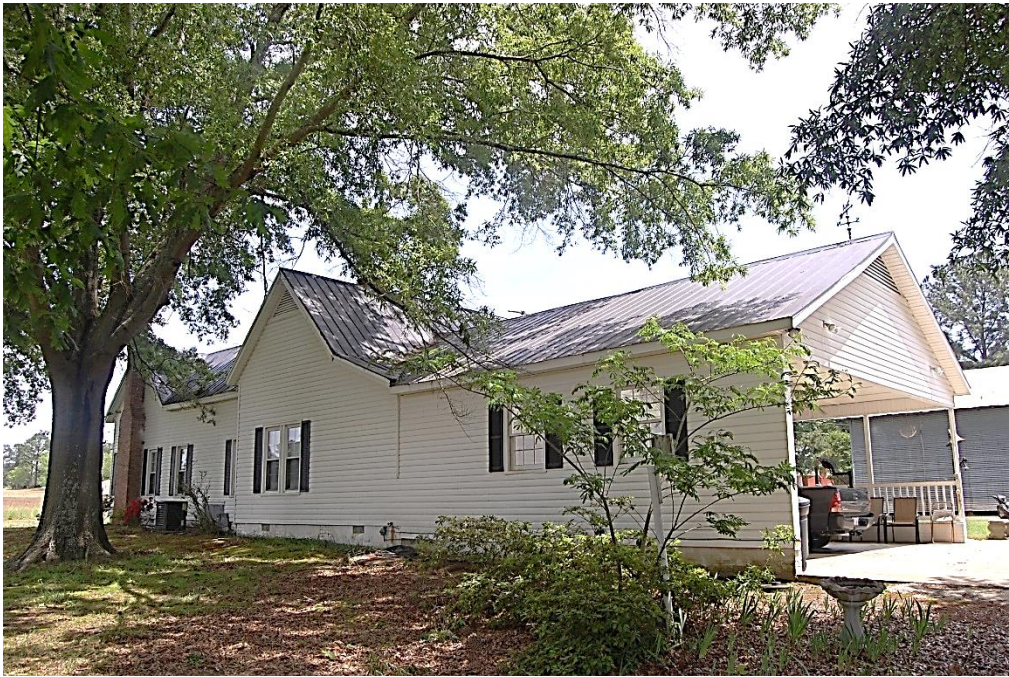
Adams Family House, Side (West) Elevation and Carport, Looking Northeast.
