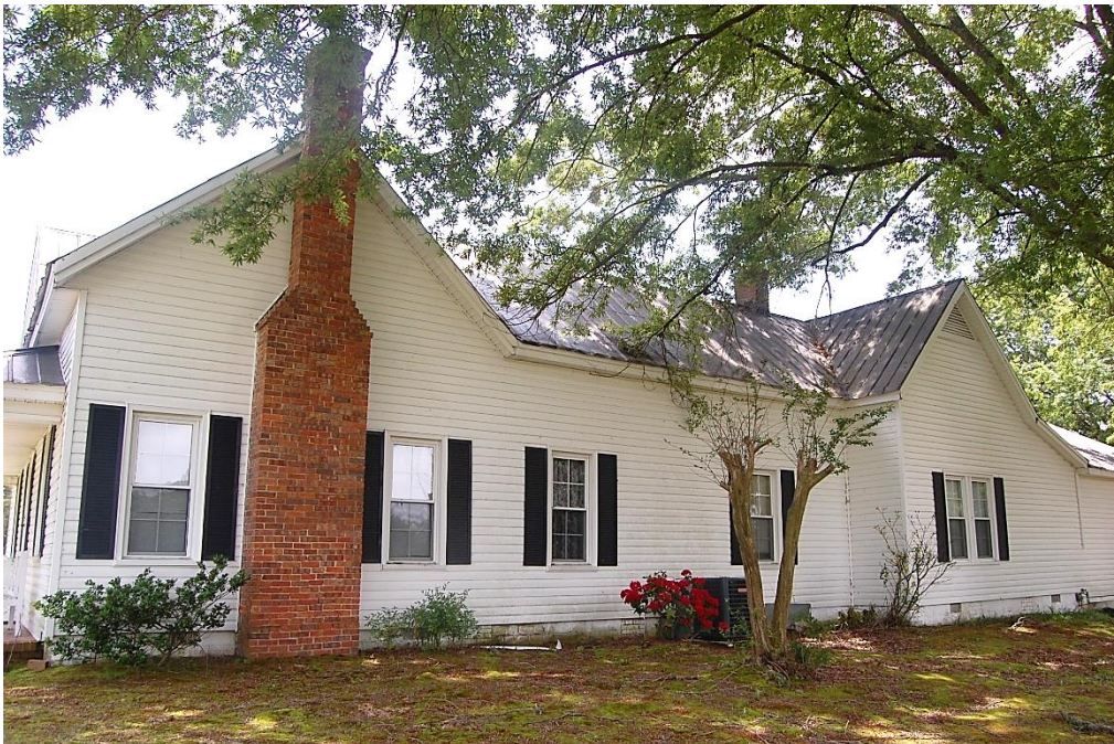
Adams Family House, Side (West) Elevation, Looking Southeast.
