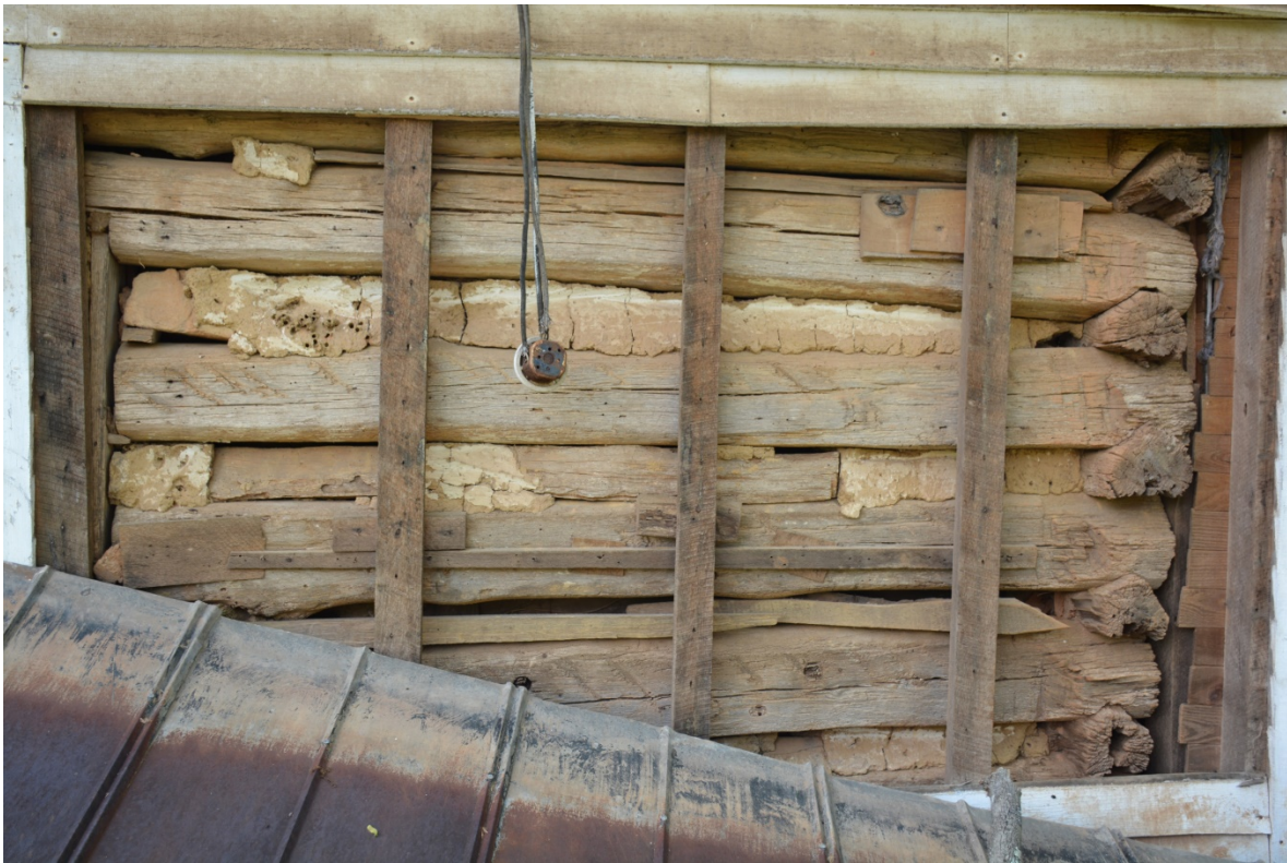
Herbin-Troxler House, mid-nineteenth century log section, east elevation
