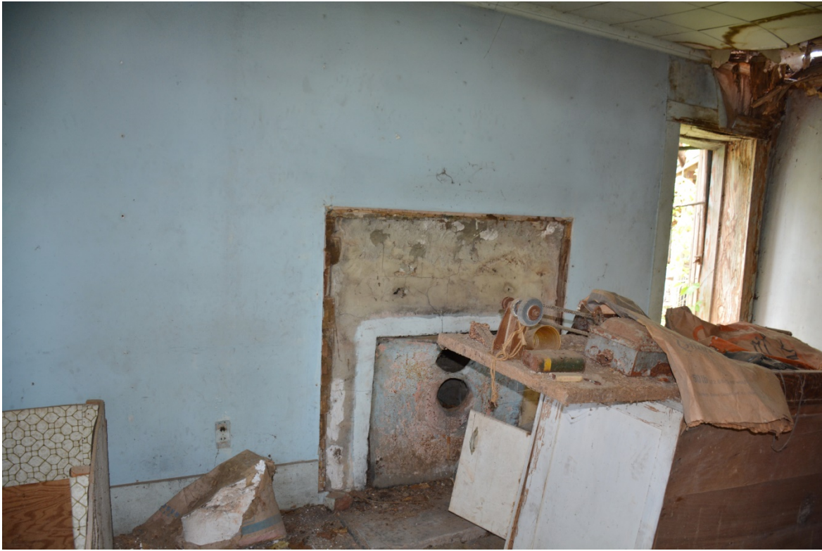
Mid-nineteenth-century log dwelling, south elevation
