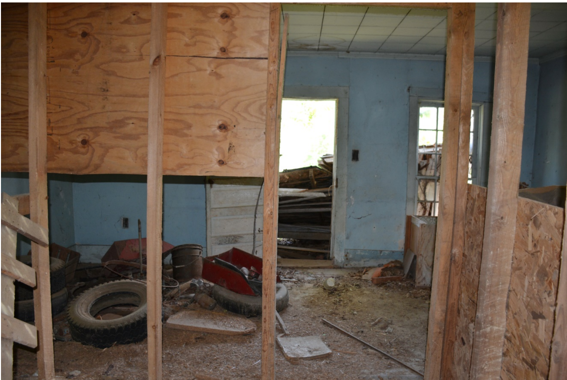
Mid-nineteenth-century log dwelling, looking east
