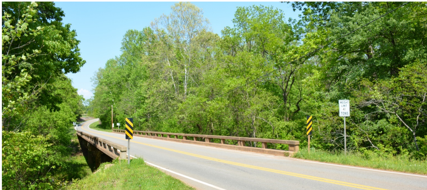
Bridge No. 184 over the Haw River
