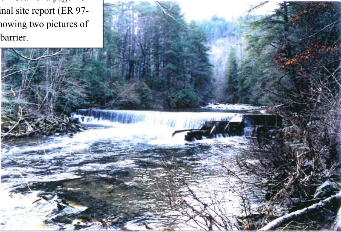
OVERALL VIEW OF DAM, FACING WEST
