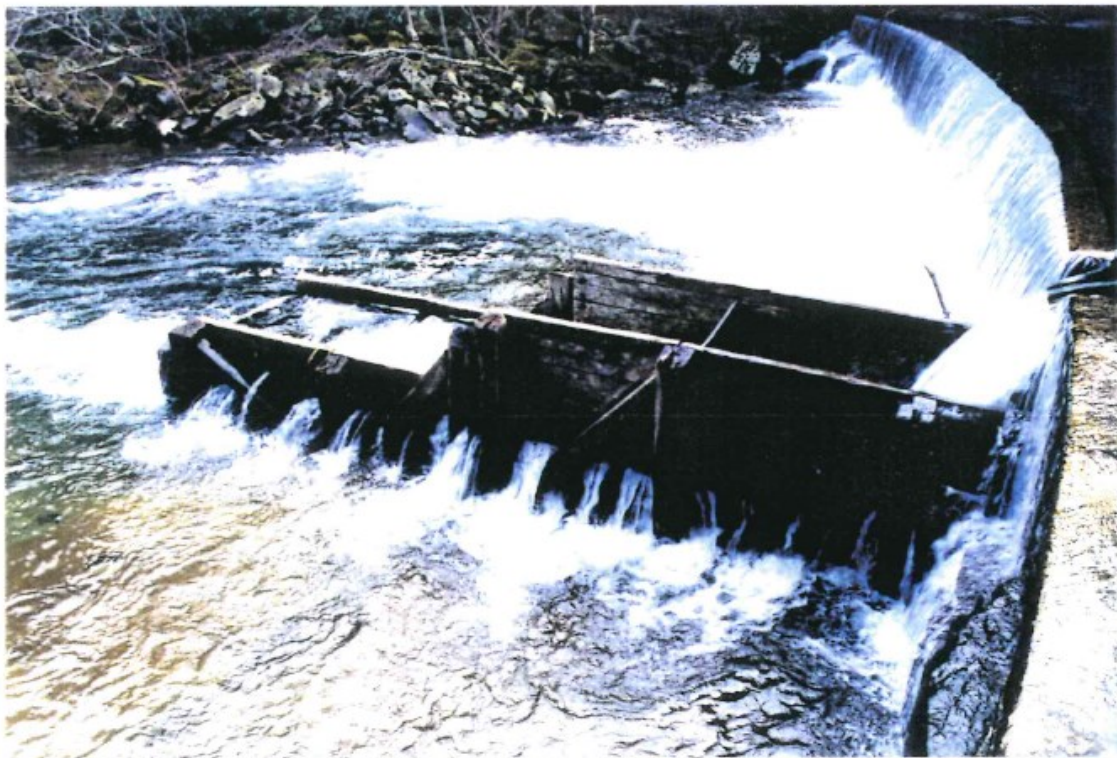
DETAIL OF STEP BOX, FACING SOUTH
