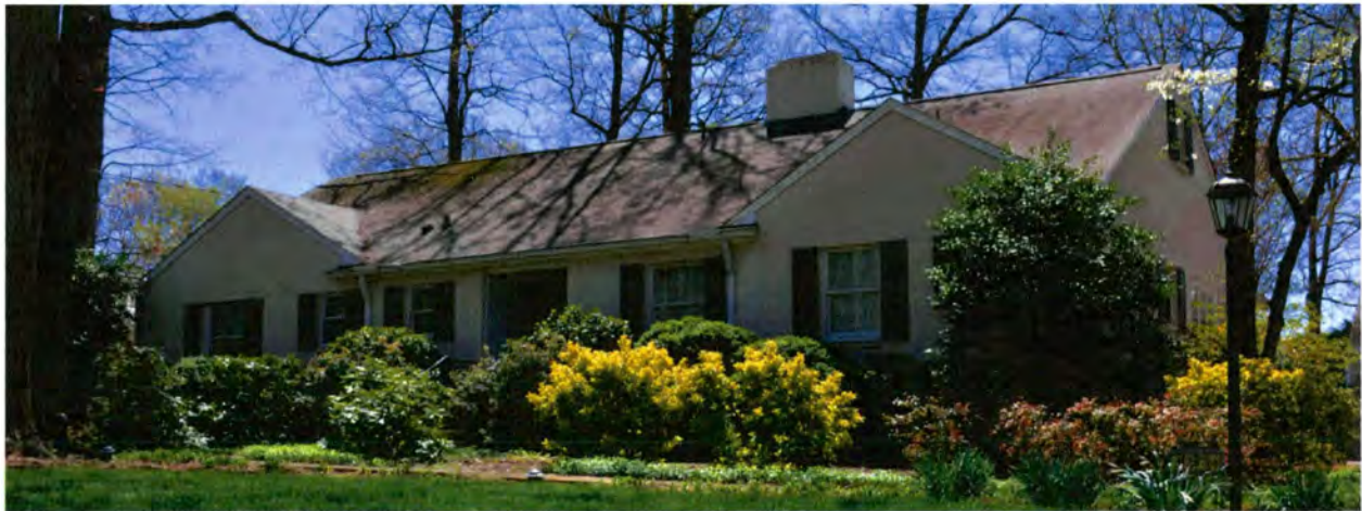
Residence, 1952, 3274 Nottingham Road (within B-5148 APE)
