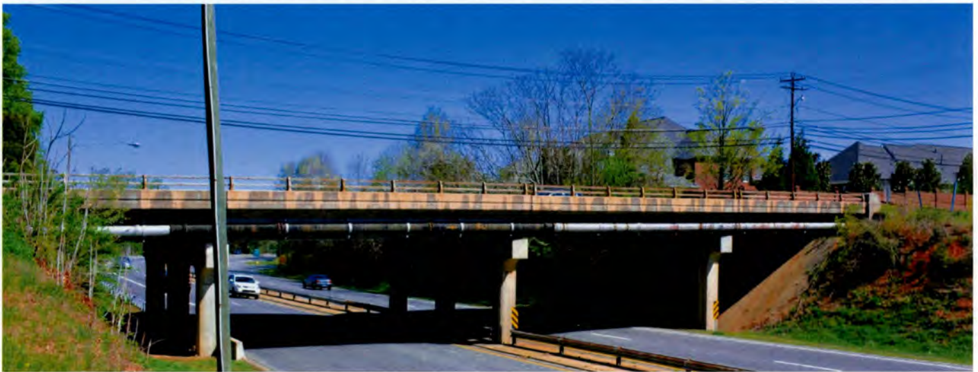
Bridge No. 276 over Silas Creek Parkway
