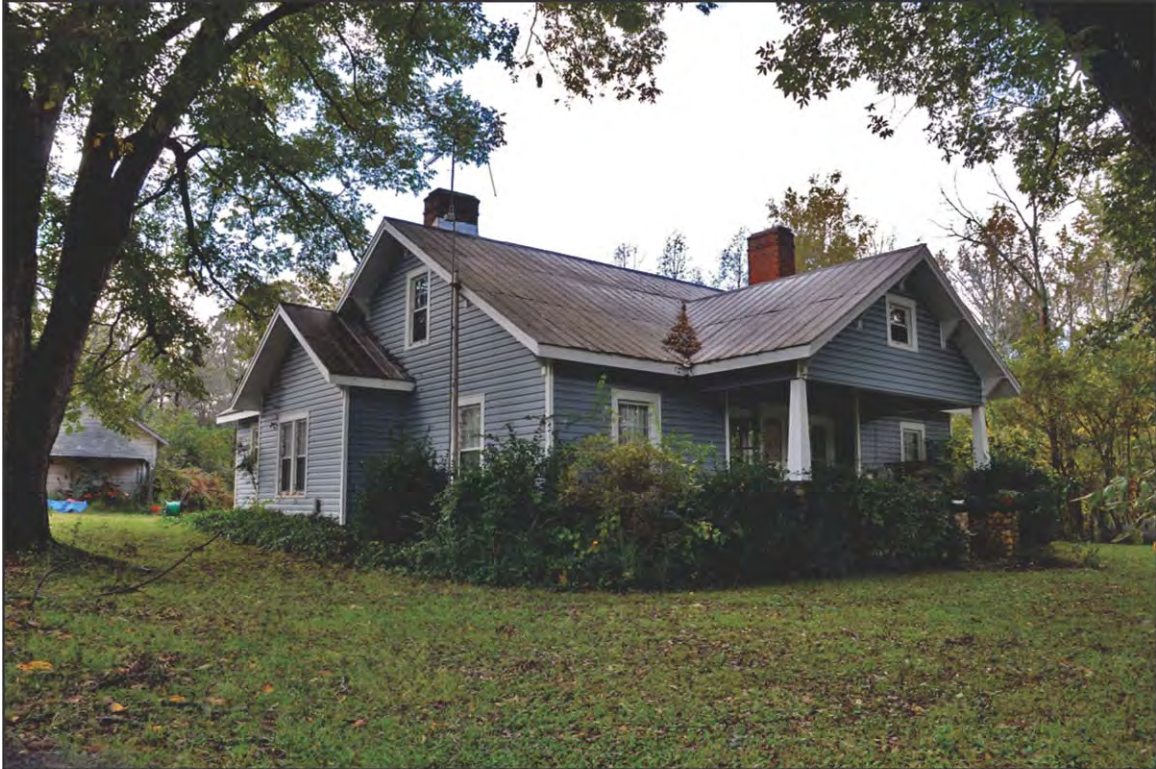
FIGURE 5: Reitzel House, East Corner, Looking Southwest
