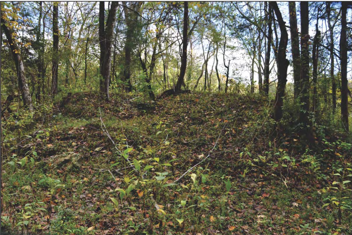
FIGURE 16: Remains of Southeast Sidewall of Dam, Looking South
