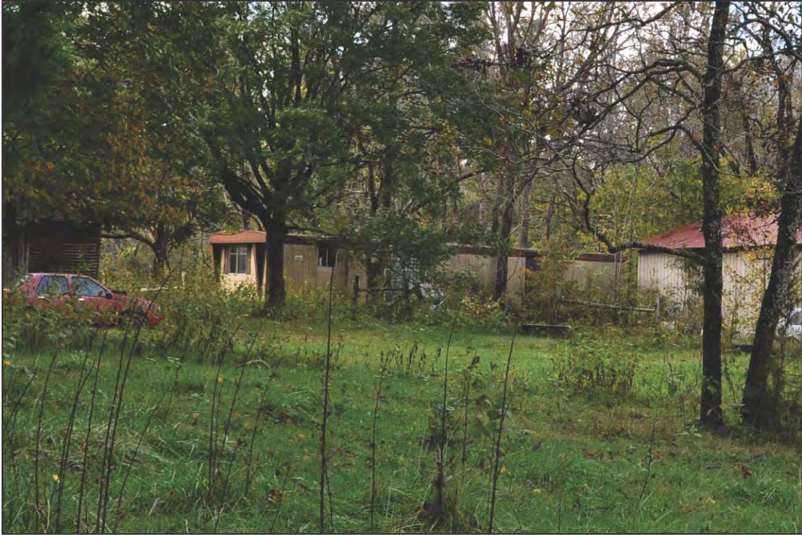
FIGURE 13: Mobile Home, Northeast Elevation
