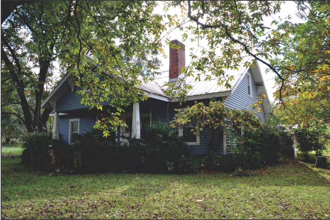
FIGURE 7: Reitzel House, West Corner, Looking Southeast
