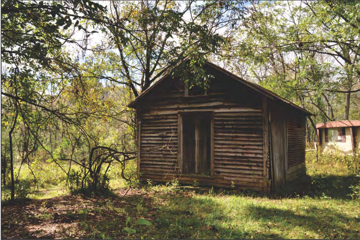
FIGURE 10: Outbuilding, Southeast Elevation
