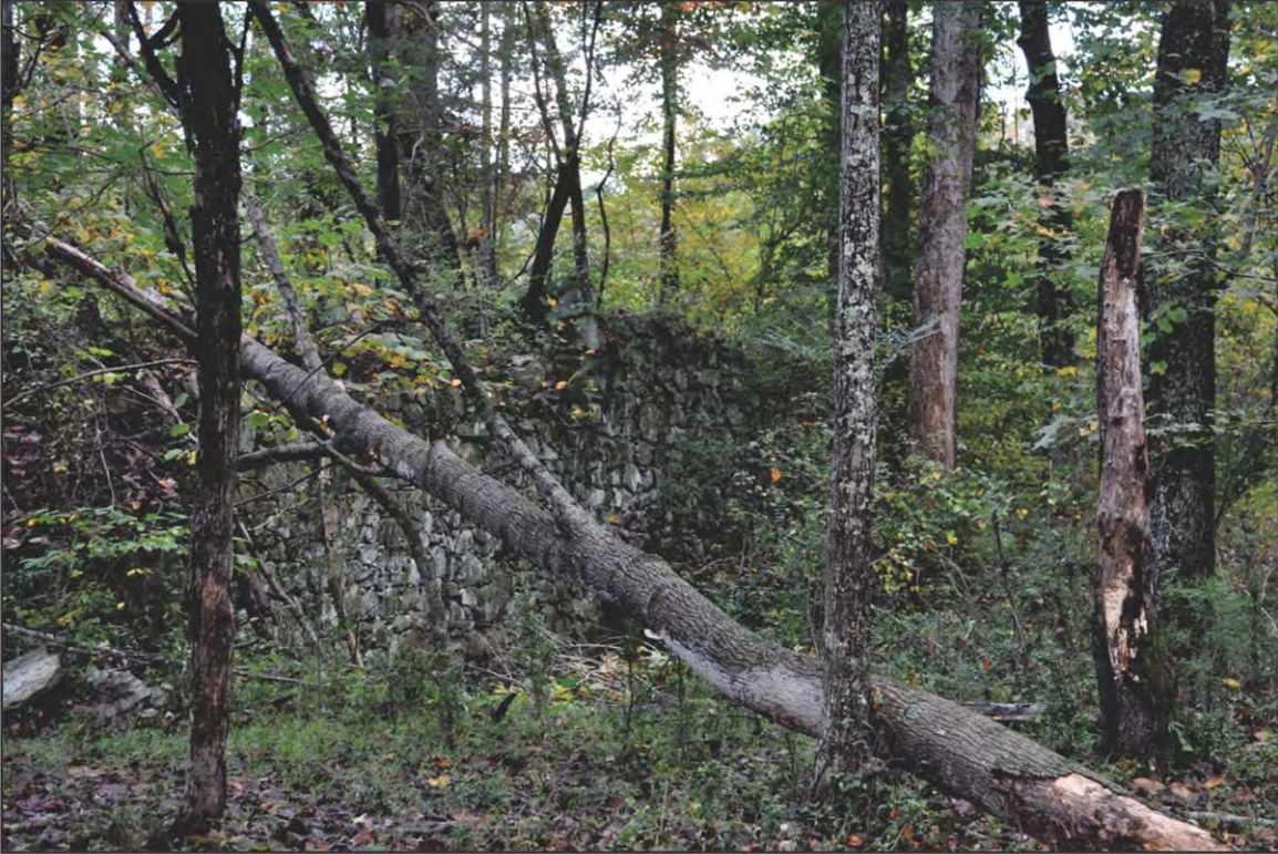
FIGURE 15: Remains of Northwest Sidewall of Dam, Looking West
