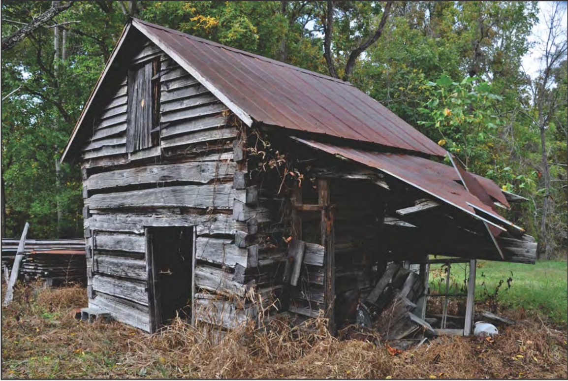
FIGURE 12: Log Outbuilding, Southeast Corner, Looking Northwest
