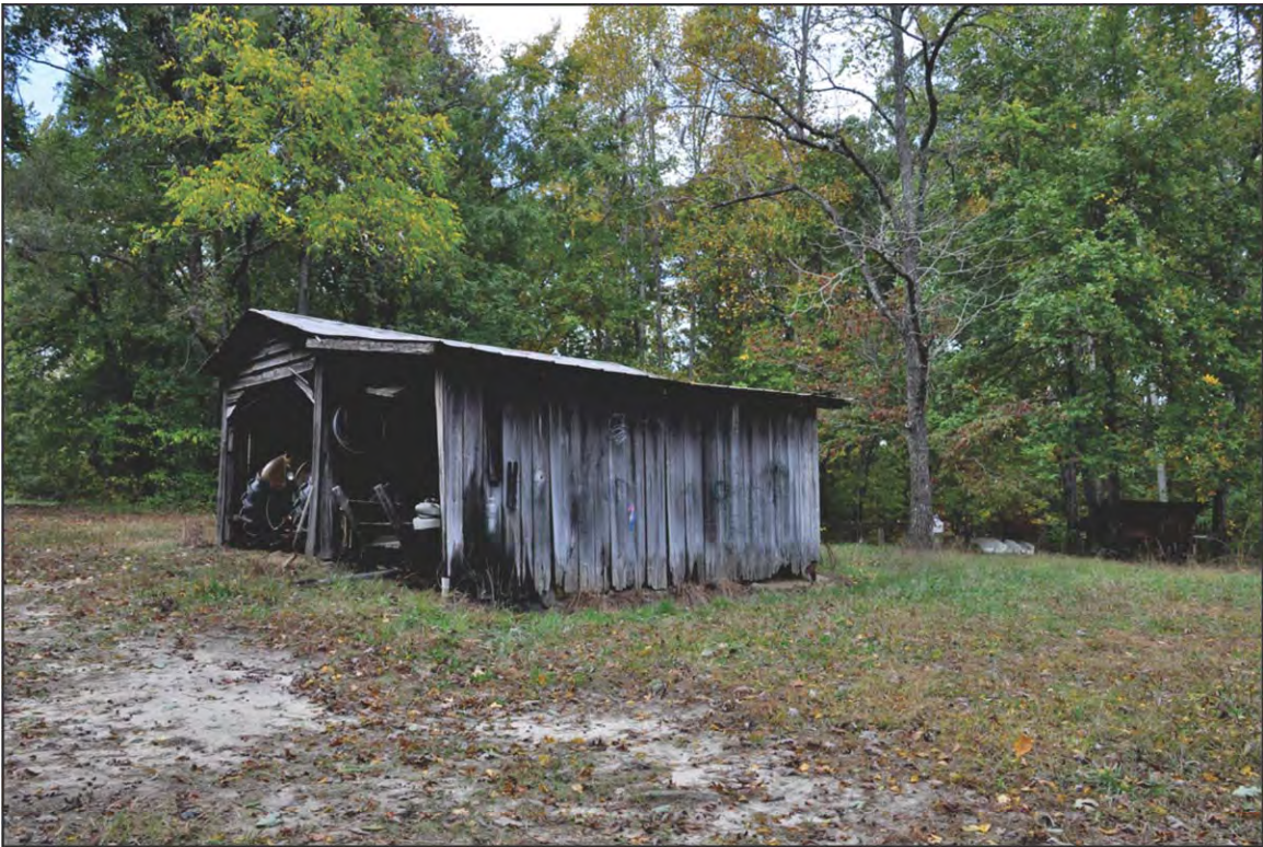
FIGURE 13: Machine Shed, Looking Northwest
