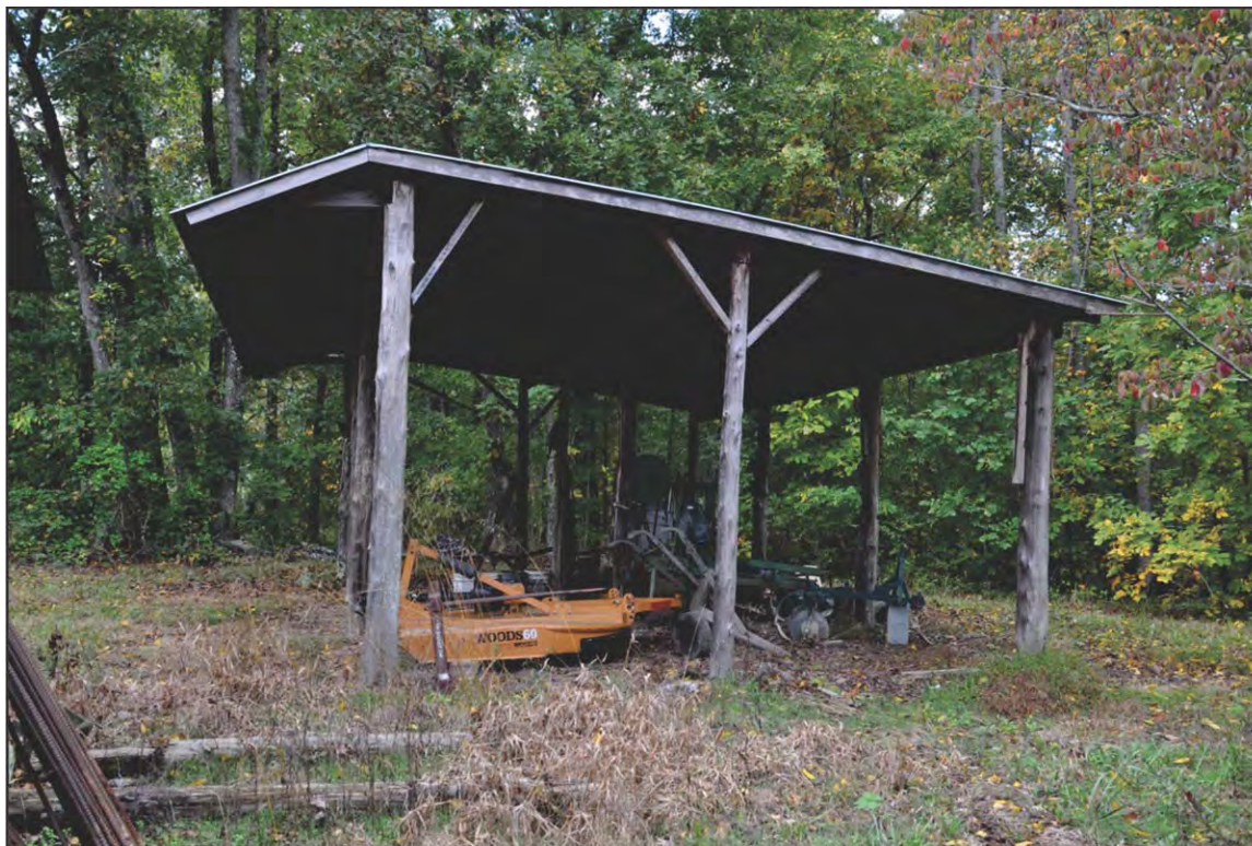
FIGURE 14: Machine Shed, Looking Northwest
