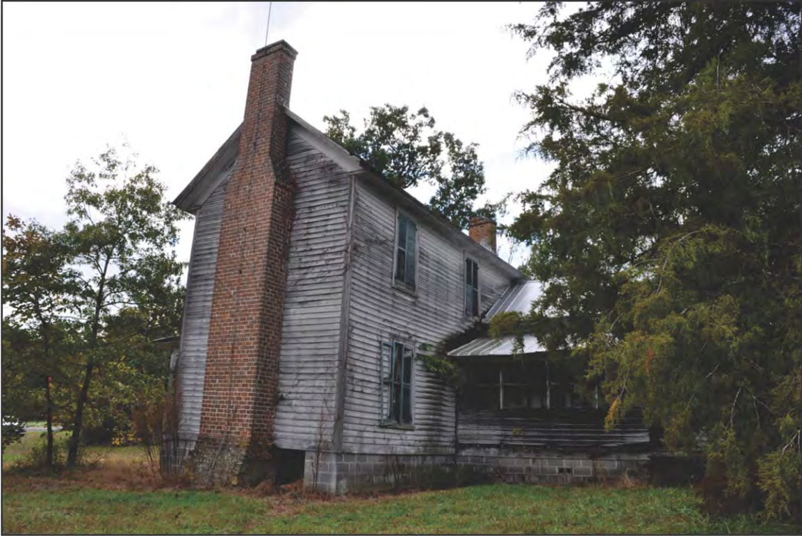
FIGURE 7: Thomas R. Greeson House, North and East Elevations
