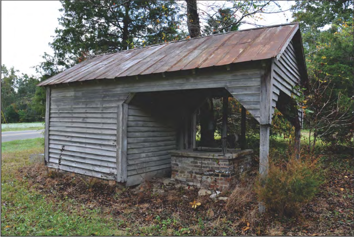
FIGURE 11: Well House, Looking West
