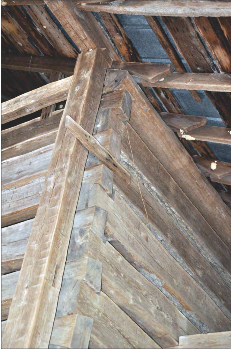
FIGURE 21: Log Barn, Showing Notching
