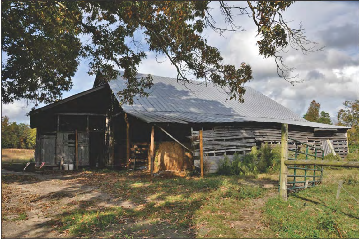
FIGURE 19: Barn, Looking North
