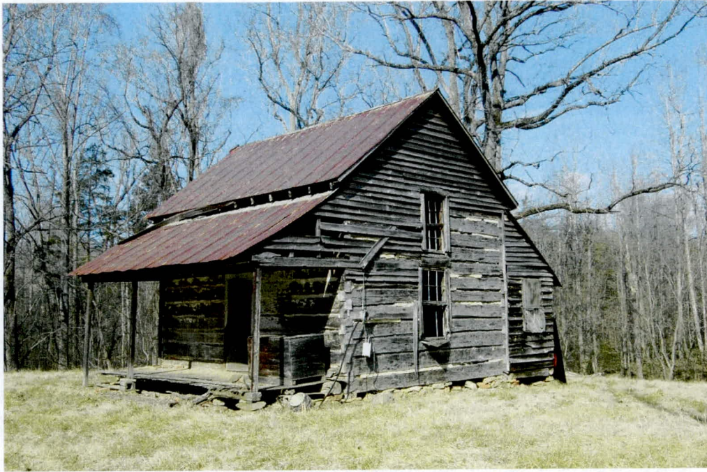
Clapp Family Log House, Façade (South Elevation) and Side (East) Elevation, Looking Northwest.
