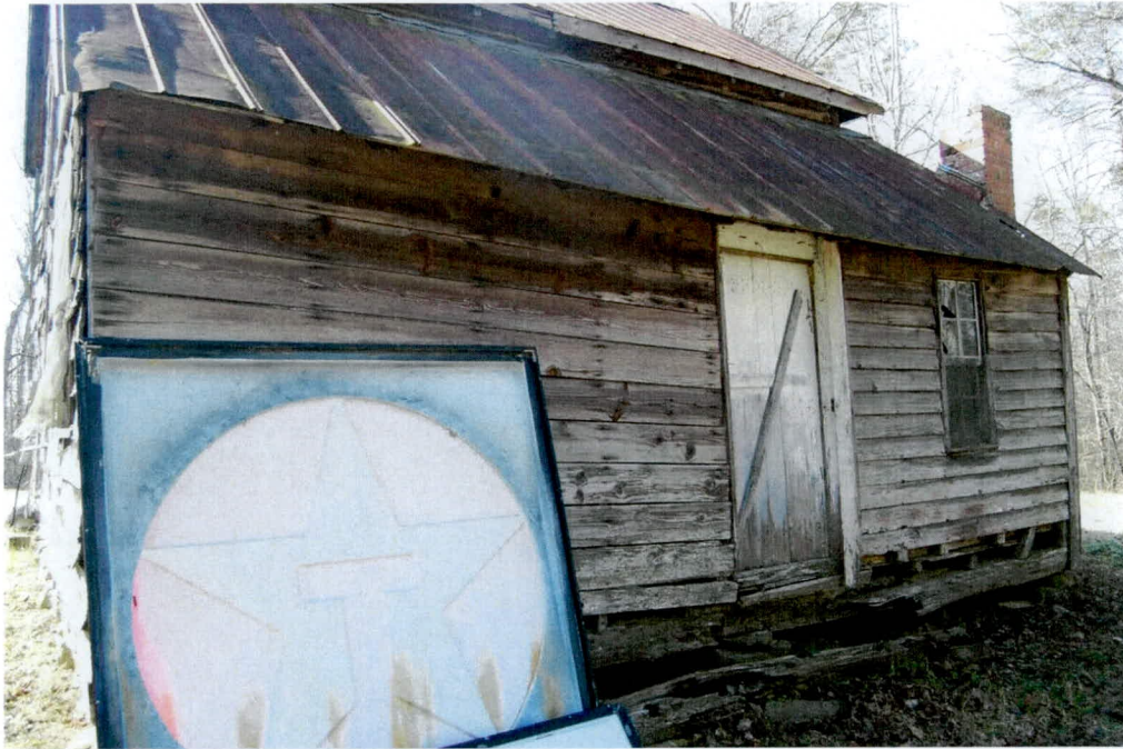
Clapp Family Log House, Rear Shed, Looking South.
