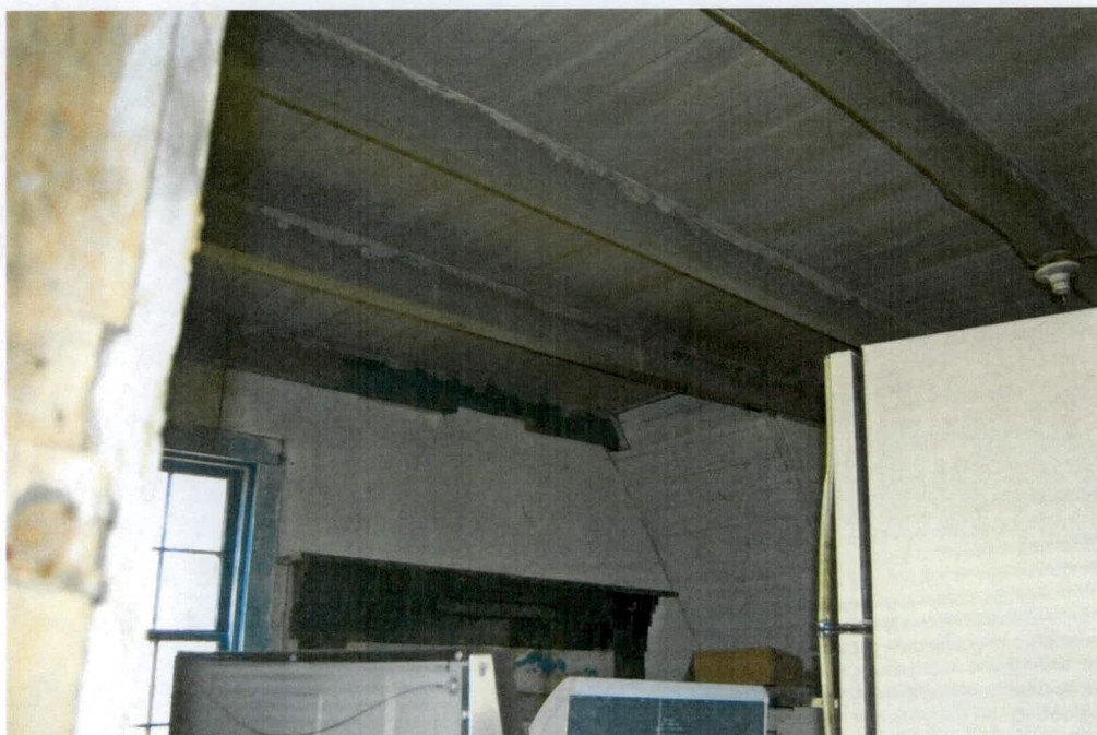
Clapp Family Log House, Interior, Mantel and Staircase in Lower Background.
