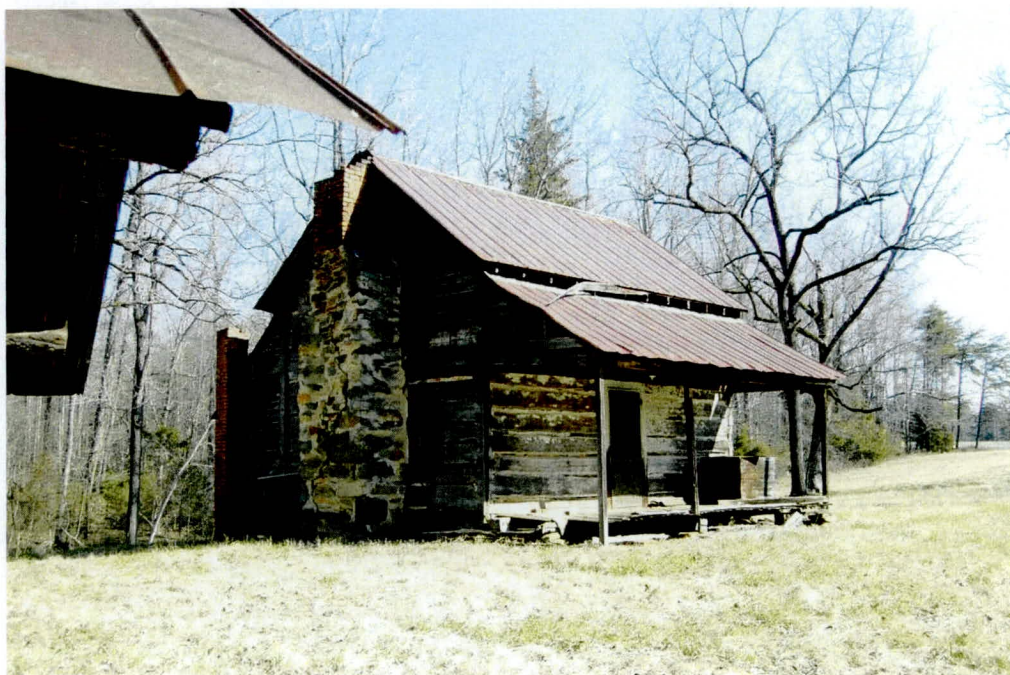
Clapp Family Log House, Looking Northeast from Corncrib.
