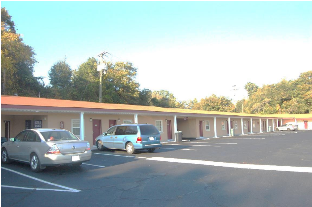
Plate 87. Holiday Motel, Office, Motel Rooms, Looking Northeast.
