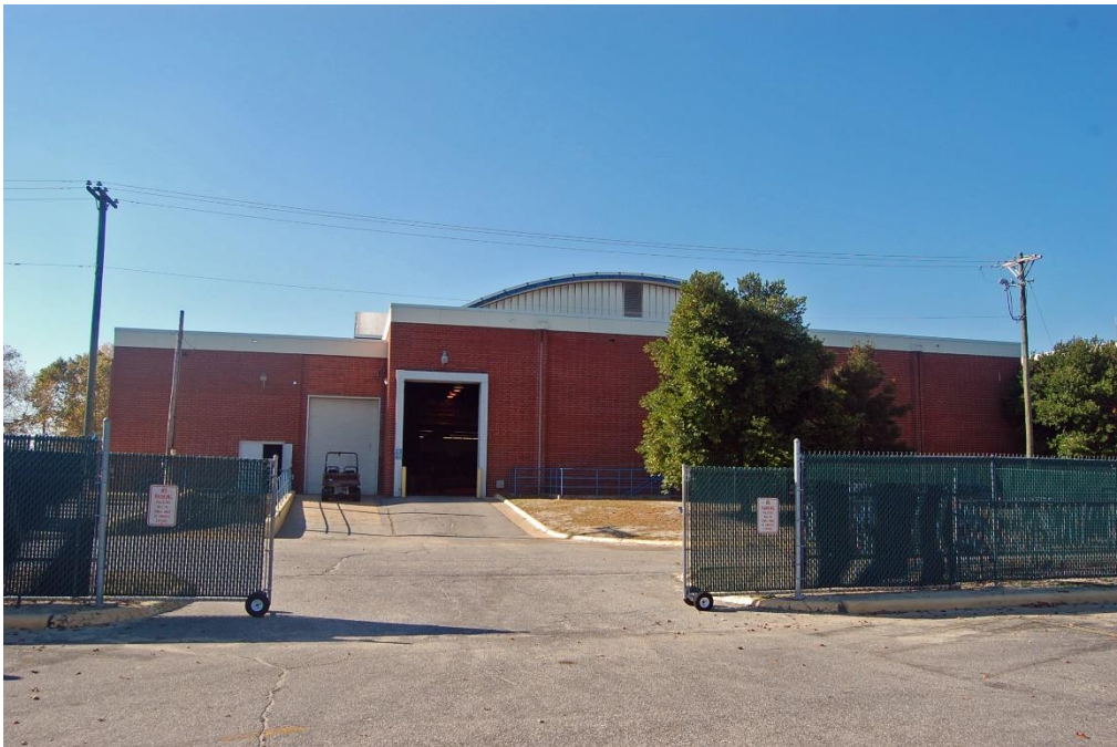
Plate 53. Cumberland County Memorial Auditorium/Exhibit Hall, Exhibit Hall/Arena, Rear (East) Elevation.
