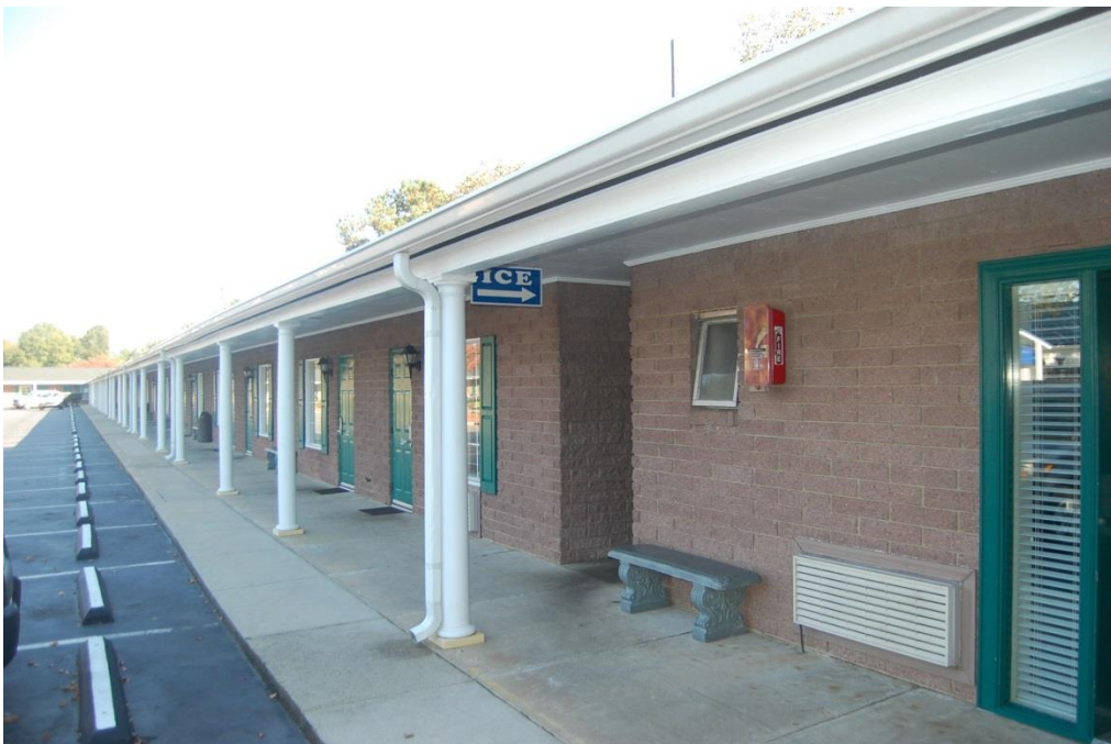
Plate 60. Ambassador Motel and Pancake House Restaurant, South Row of Rooms, Looking East.
