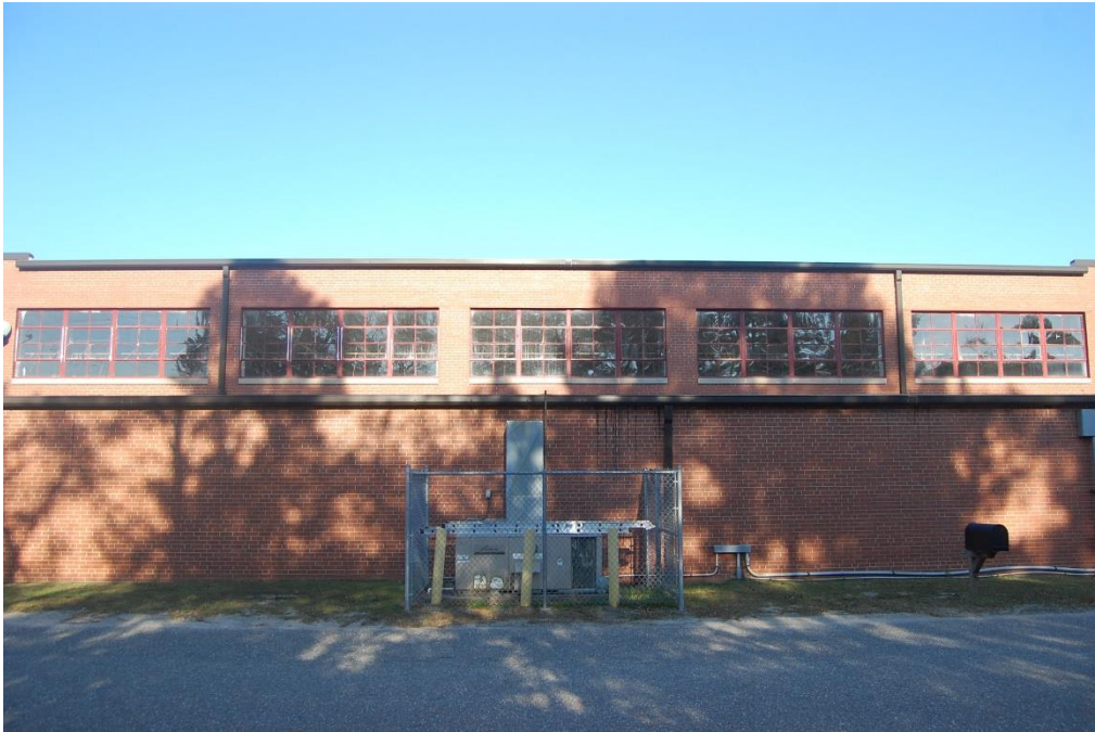
Plate 80. North Carolina National Guard Armory, Side (South) Elevation, Looking East.
