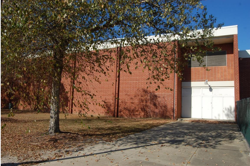
Plate 52. Cumberland County Memorial Auditorium/Exhibit Hall, Exhibit Hall/Arena, Side (South) Elevation.
