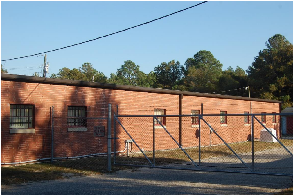
Plate 81. North Carolina National Guard Armory, Side (West) Elevation, Shooting Range, Looking East.
