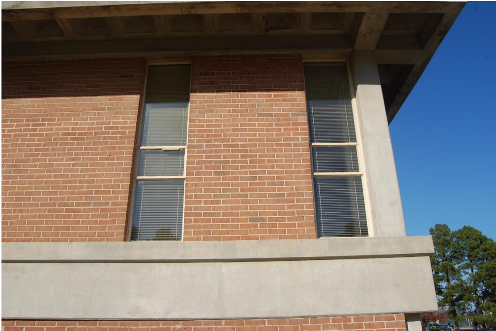
Plate 35. Cumberland County Administration Building, Facade, Original Windows, Looking North.
