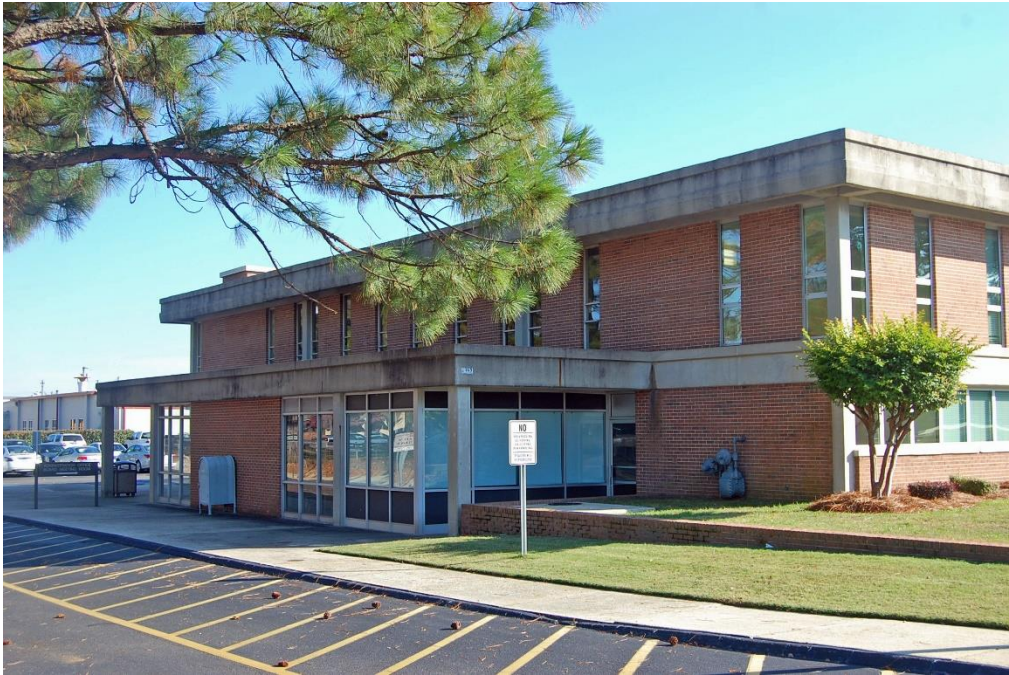
Plate 37. Cumberland County Administration Building, North Elevation, Looking Southeast.
