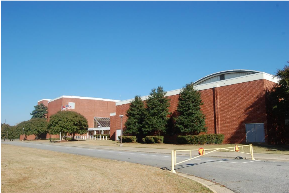
Plate 48. Cumberland County Memorial Auditorium/Exhibit Hall, Front (West) Elevation of Arena (Exhibit Hall), Looking Northeast.
