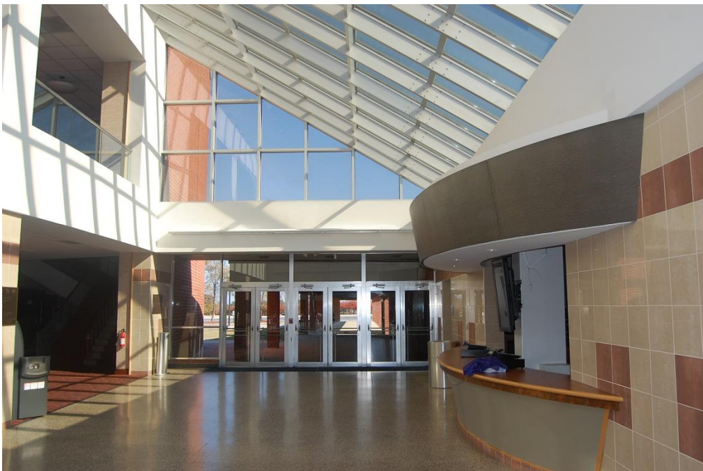
Plate 57. Cumberland County Memorial Auditorium/Exhibit Hall, Center Lobby, Interior, Skylight and Modern Snack Bar, Looking East.
