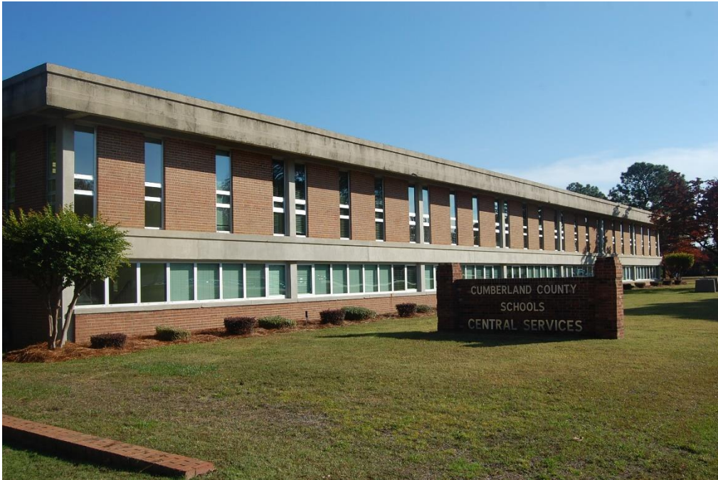
Plate 33. Cumberland County Administration Building, West Elevation, Looking Southeast.
