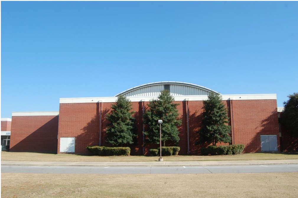
Plate 51. Cumberland County Memorial Auditorium/Exhibit Hall, Exhibit Hall/Arena, Front (West) Elevation.
