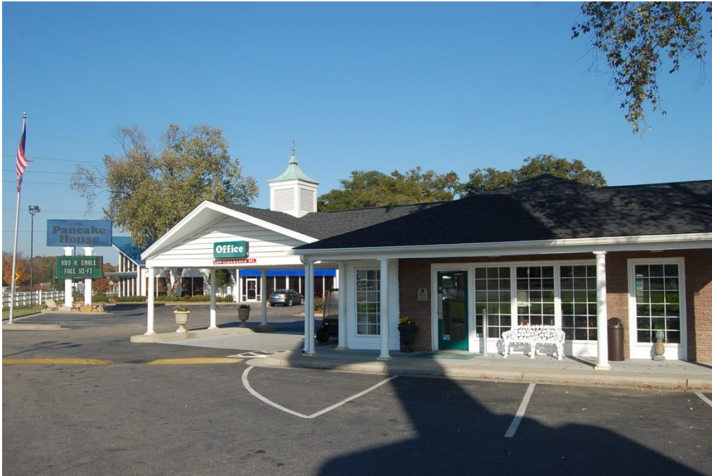
Plate 58. Ambassador Motel and Pancake House Restaurant, Office and Pancake House Restaurant (Background), Looking Northeast.
