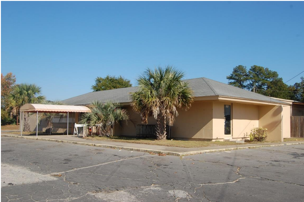
Plate 14. Howard Johnson's Motor Lodge, Restaurant, Looking East.
