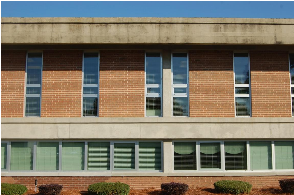
Plate 34. Cumberland County Administration Building, West Elevation, Looking East.
