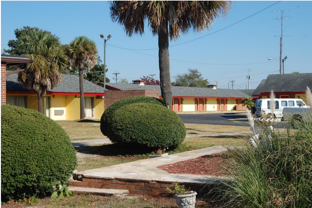
Plate 20. Americana Motor Lodge, Infilled Wading Pool (Foreground) and North Units, Looking Northeast.
