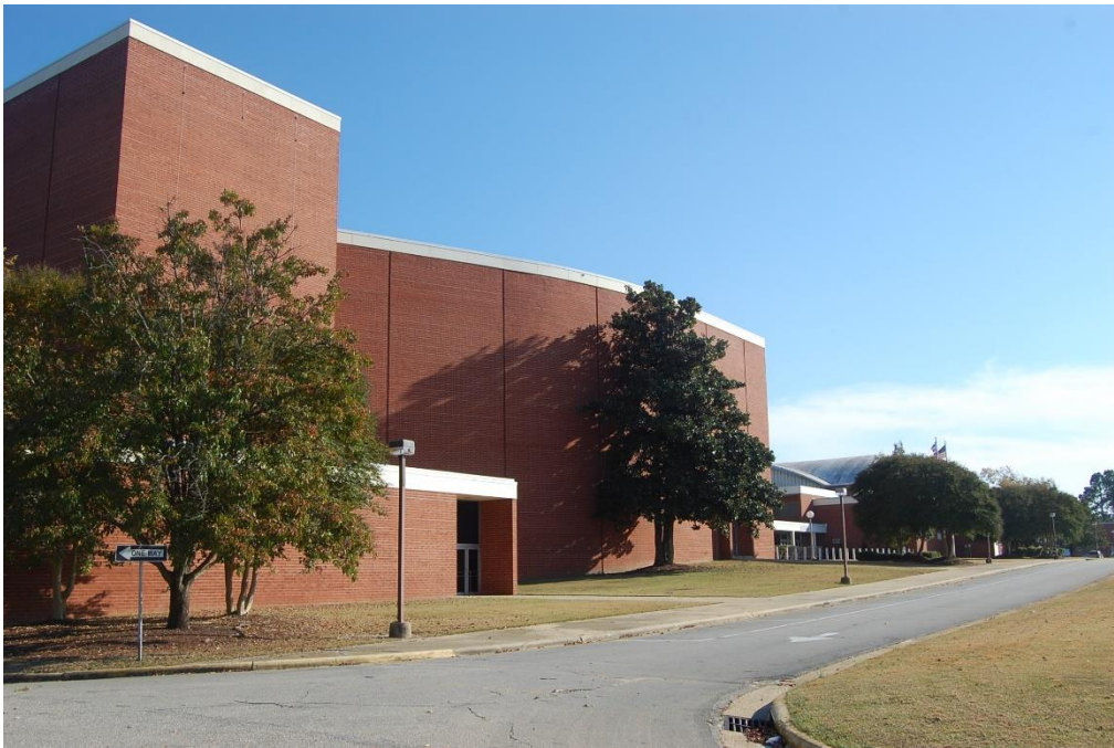
Plate 47. Cumberland County Memorial Auditorium/Exhibit Hall, Front (West) Elevation of Auditorium, Looking South.
