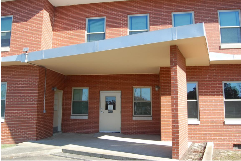
Plate 45. North Carolina Highway Patrol Building, Entrance Detail.
