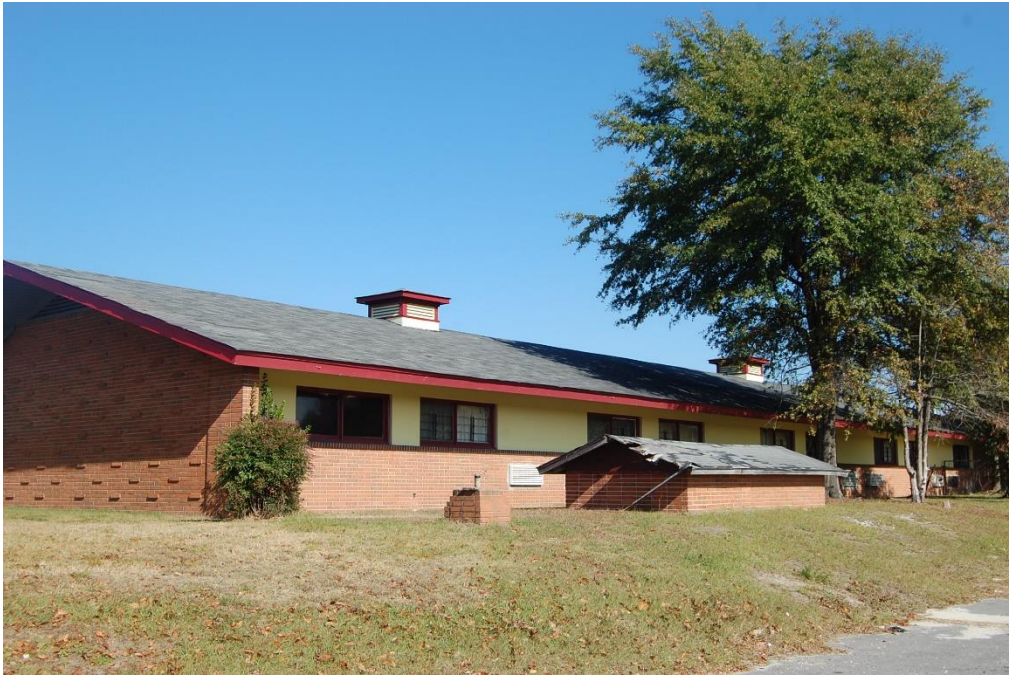
Plate 28. Americana Motor Lodge, South Units, Rear Elevation, Looking North.
