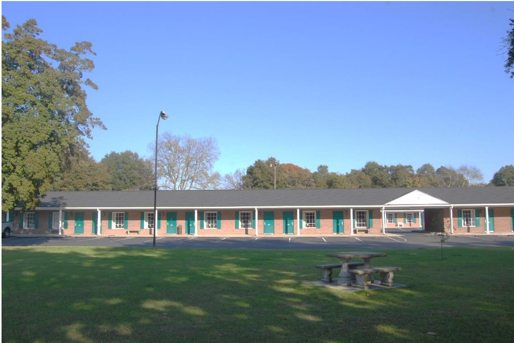
Plate 59. Ambassador Motel and Pancake House Restaurant, View Across Lawn, Looking East.
