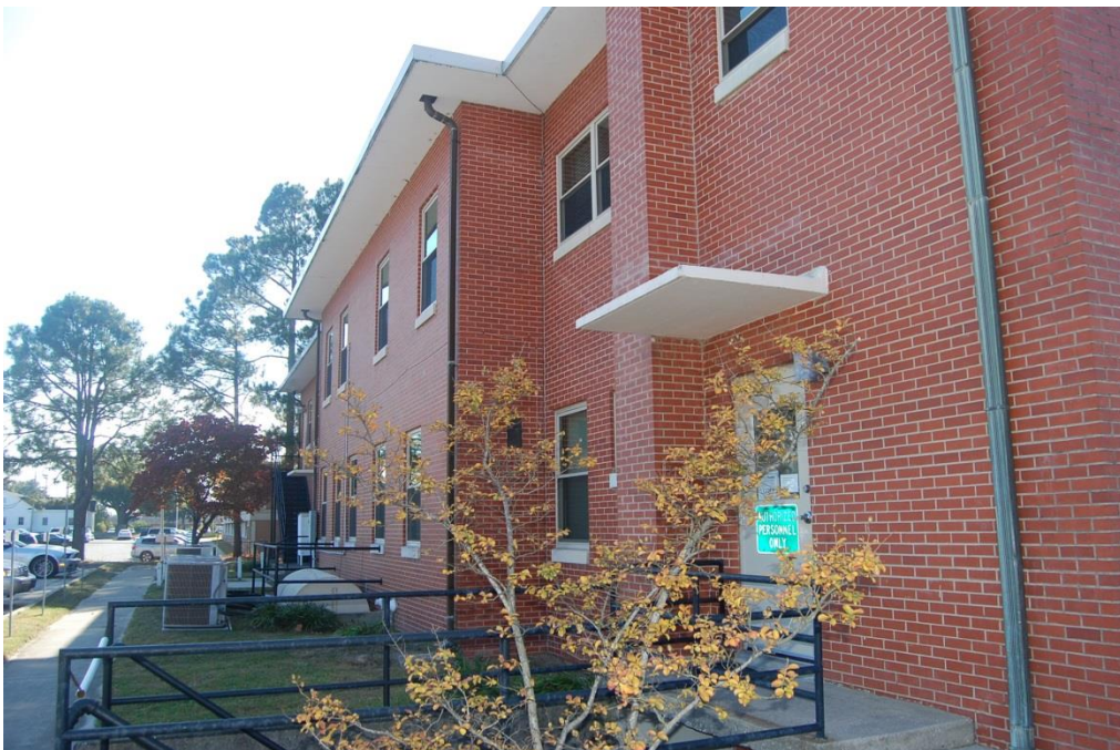
Plate 44. North Carolina Highway Patrol Building, Rear (East) Elevation, Looking South.
