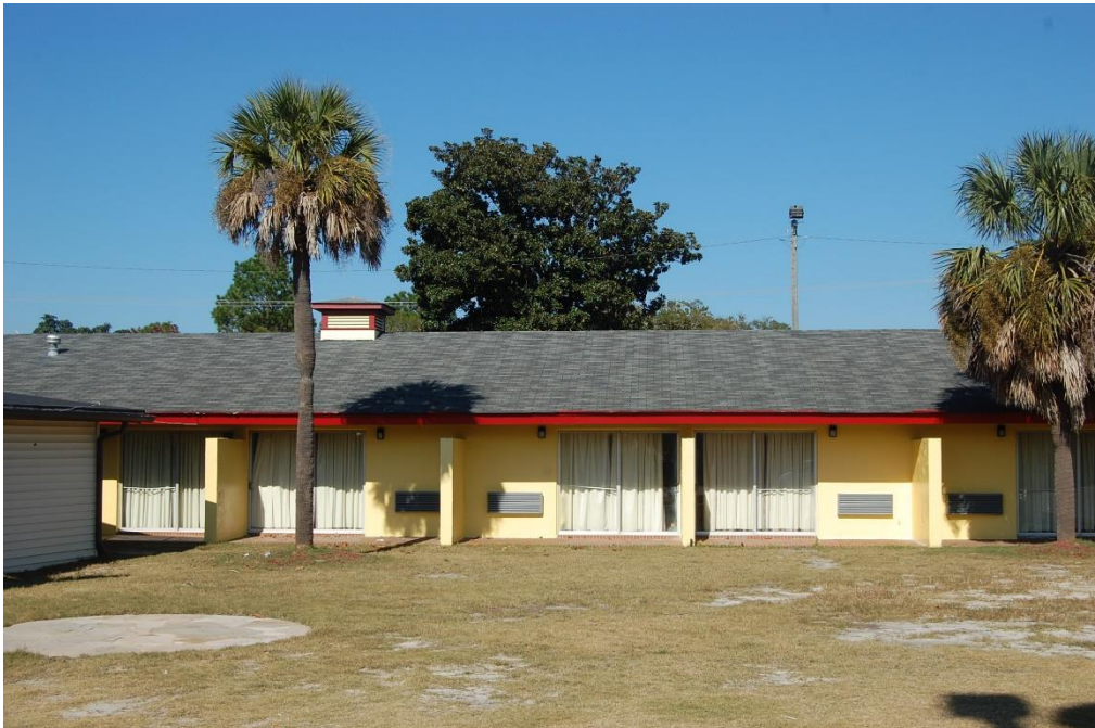
Plate 23. Americana Motor Lodge, Northwest Units (East of Office), Looking North.
