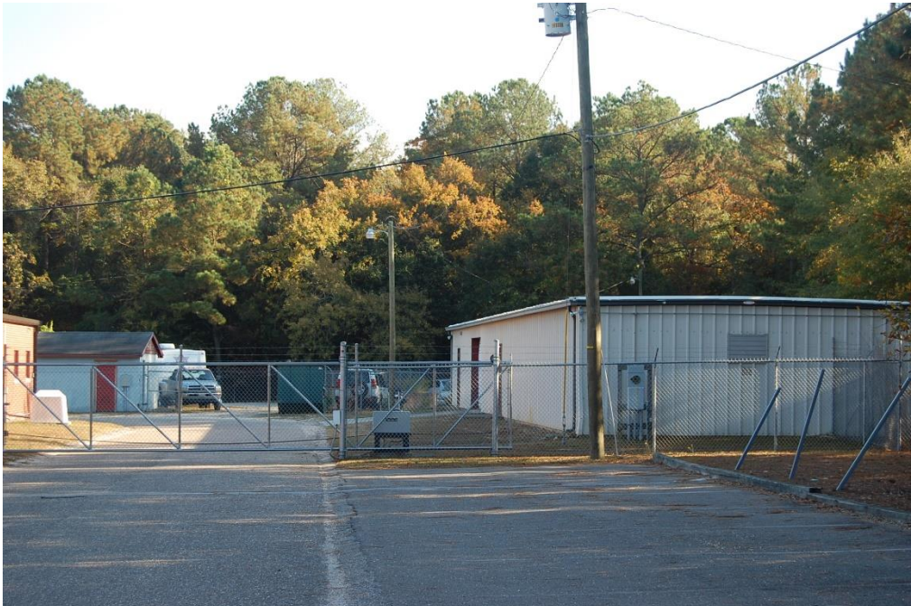
Plate 83. North Carolina National Guard Armory, Rear Maintenance Sheds, Looking South.
