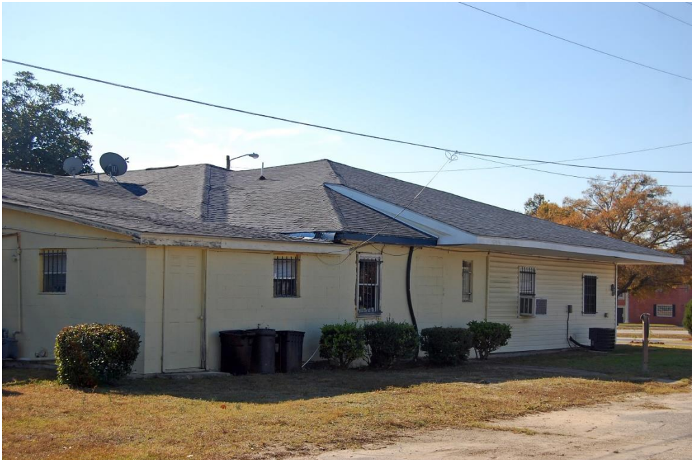
Plate 12. Howard Johnson's Motor Lodge, Office, Rear (North) Elevation, Looking Southwest.
