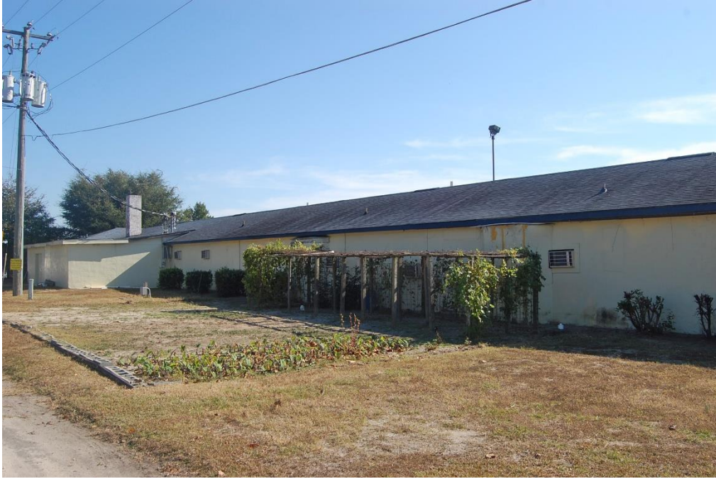
Plate 13. Howard Johnson's Motor Lodge, Rear (North) Elevation, Looking Southeast.
