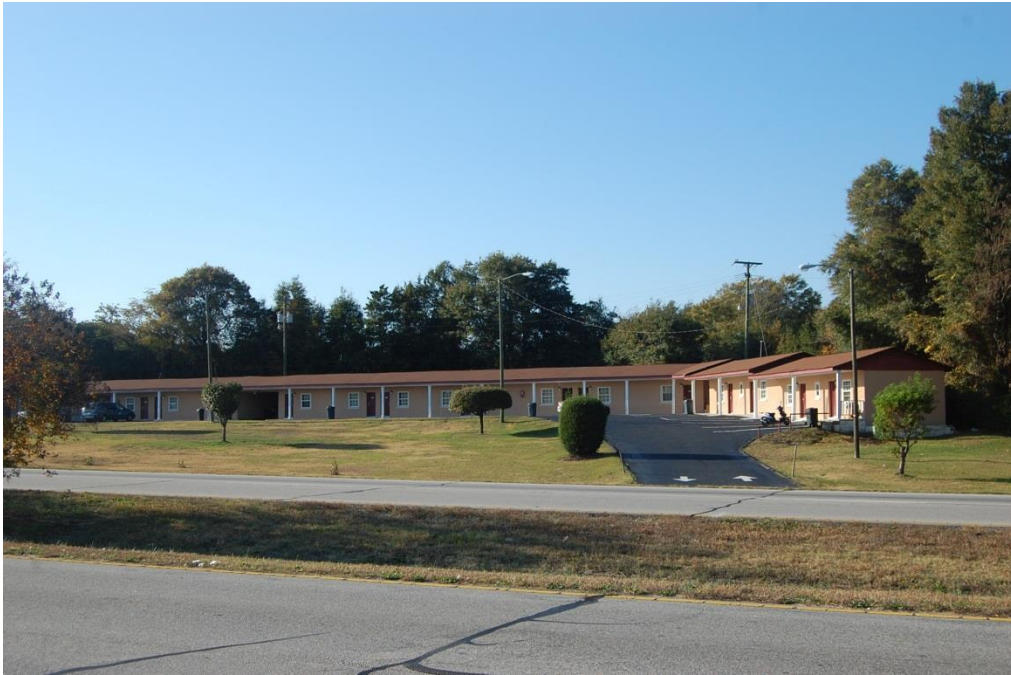
Plate 84. Holiday Motel, Overall View, Looking North.
