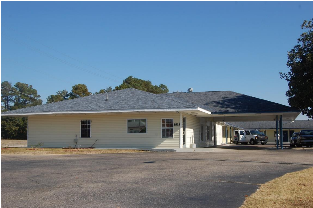
Plate 10. Howard Johnson's Motor Lodge, Office, Looking East.
