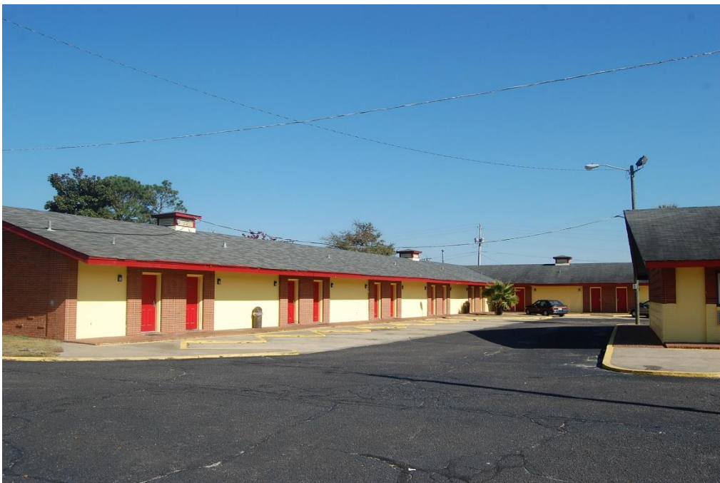
Plate 21. Americana Motor Lodge, Northwest and West Units, Looking East.
