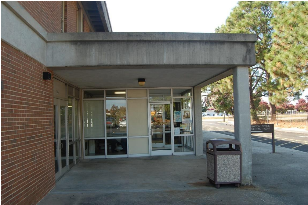
Plate 38. Cumberland County Administration Building, North Elevation, Entrance, Looking West.
