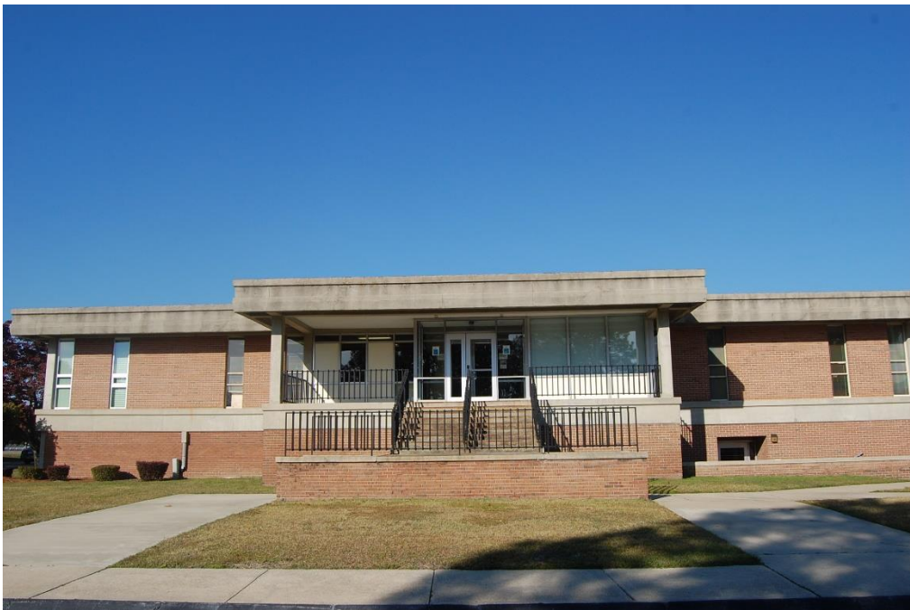
Plate 30. Cumberland County Administration Building, Façade, (South Elevation), Looking North.
