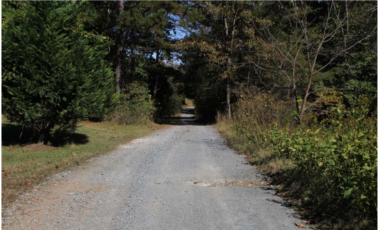
View northeast along Payne Road (SR 1601) to project end
