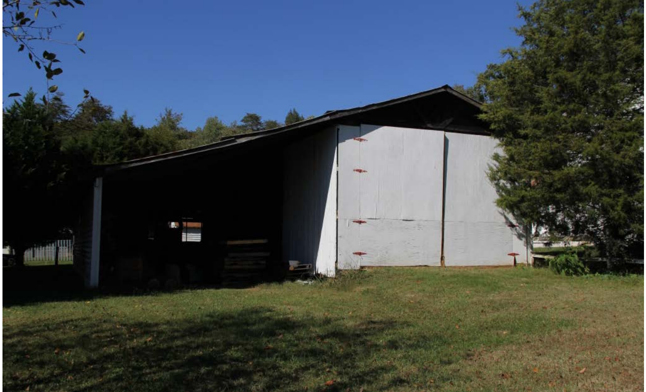
Barn, view to north
