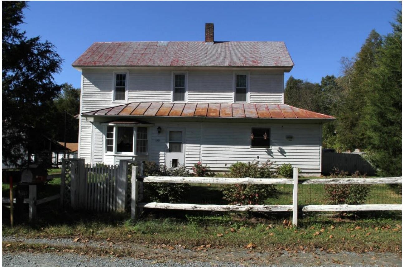
Bill Spainhour House (FY1448), 6491 Payne Road, façade, view to northwest
