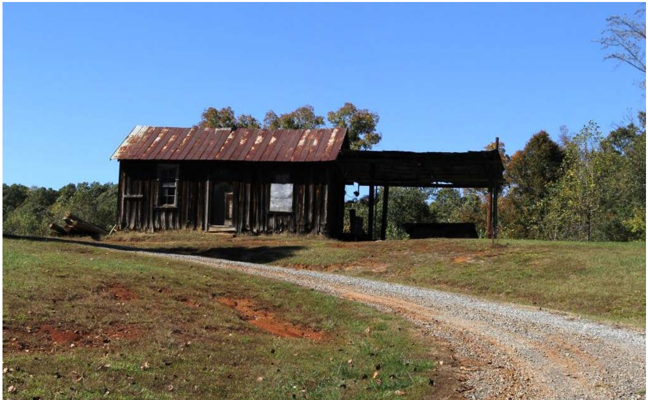
Shed, façade, view to northwest
