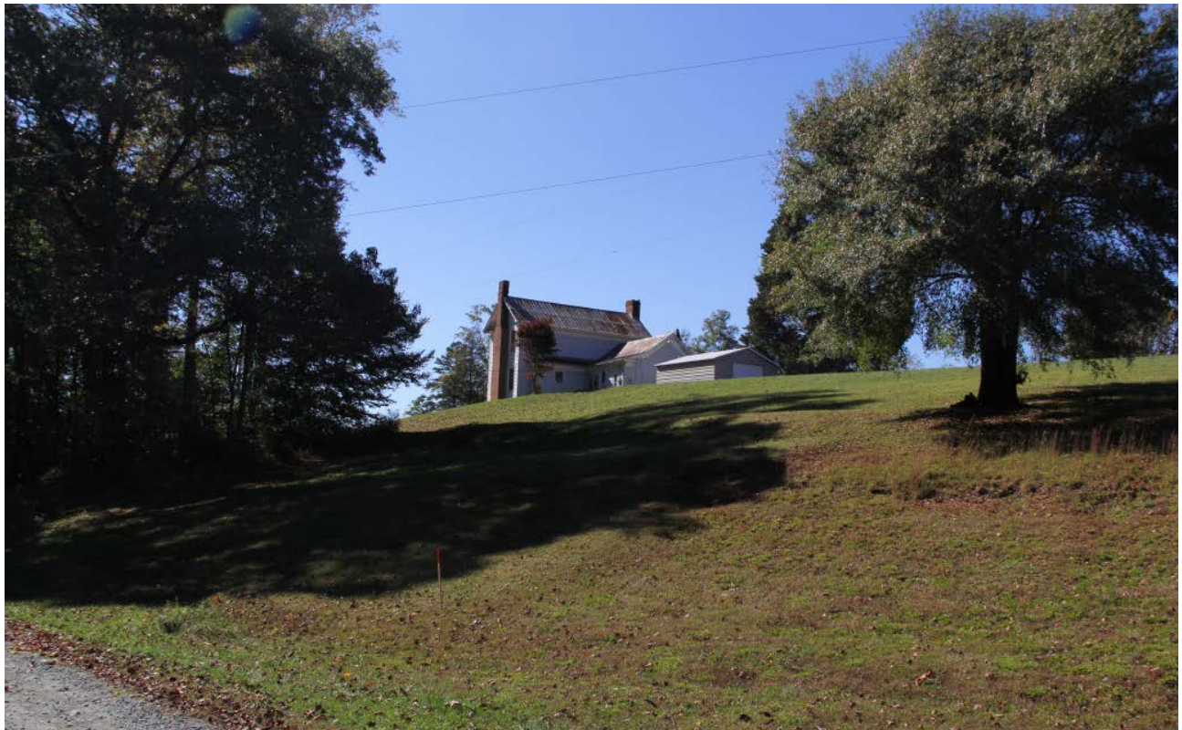
John Ward House (FY1449), 6481 Payne Road, oblique view to northwest from the west
