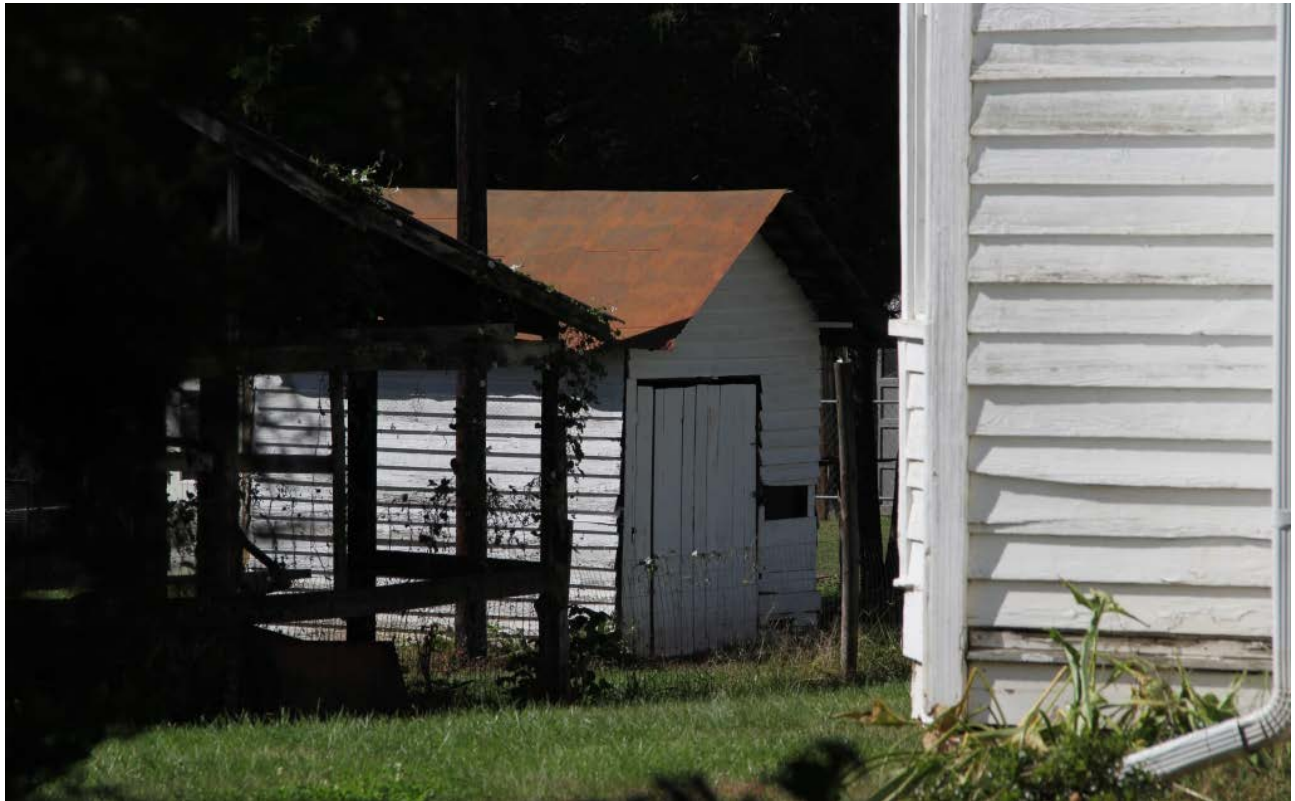
Shed, oblique front view to northwest
