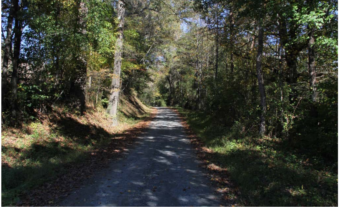
Payne Road (SR 1601), view to northeast
