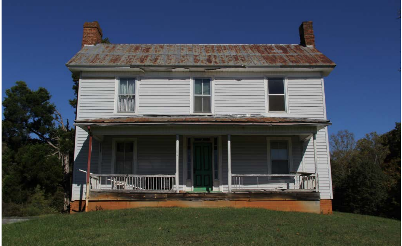
John Ward House, façade, view to northeast
