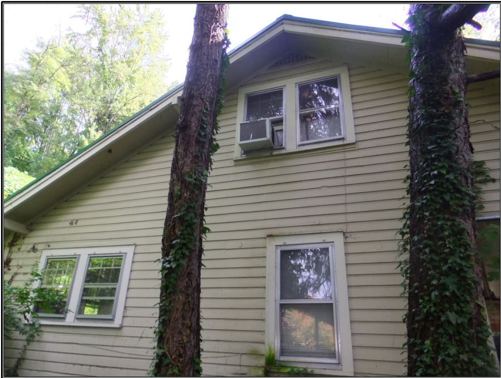
Figure 15. East-northeasterly view of the west elevation.
