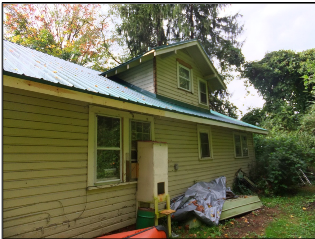
Figure 13. Southwesterly view of the rear elevation and dormer.
