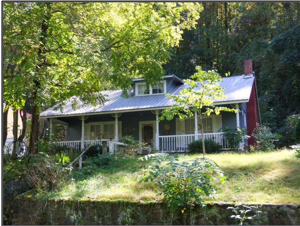
Figure 23. View of the Bungalow at 12 E. Hemlock Street in Dillsboro.
