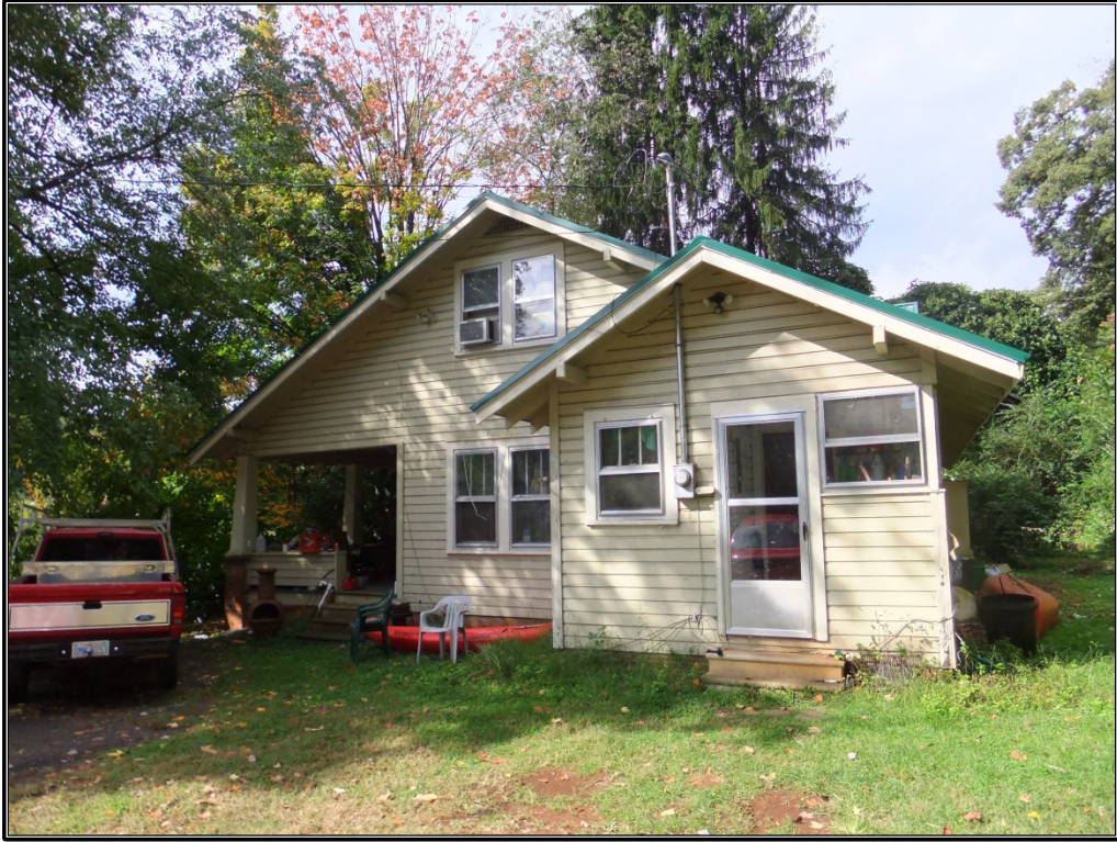
Figure 14. West-southwesterly view of the east elevation.
