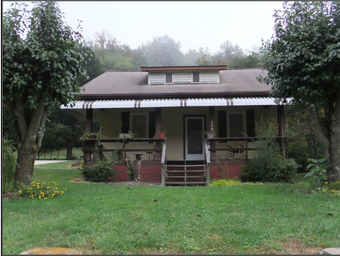
Figure 28. View of Bungalow at 574 Dillsboro Road in Sylva.
