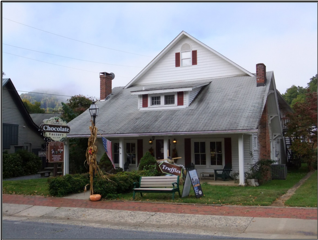
Figure 25. View of the Dillsboro Chocolate Factory at 28 Church Street in Dillsboro.
