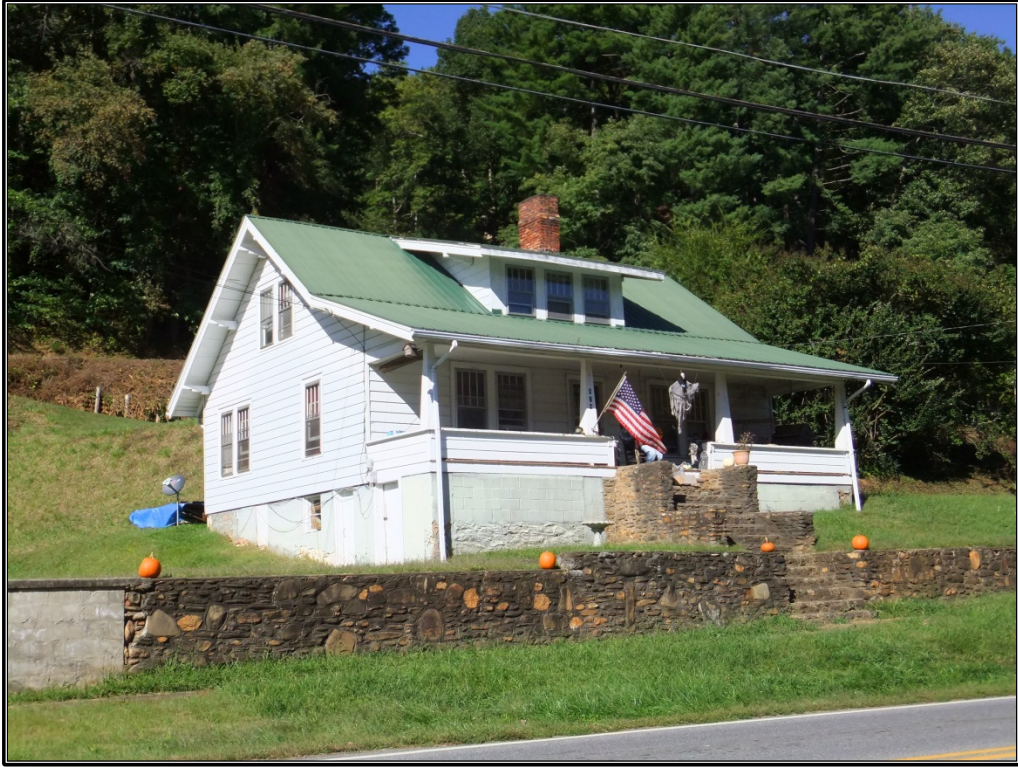
Figure 24. View of the Bungalow at 434 Haywood Road in Dillsboro.
