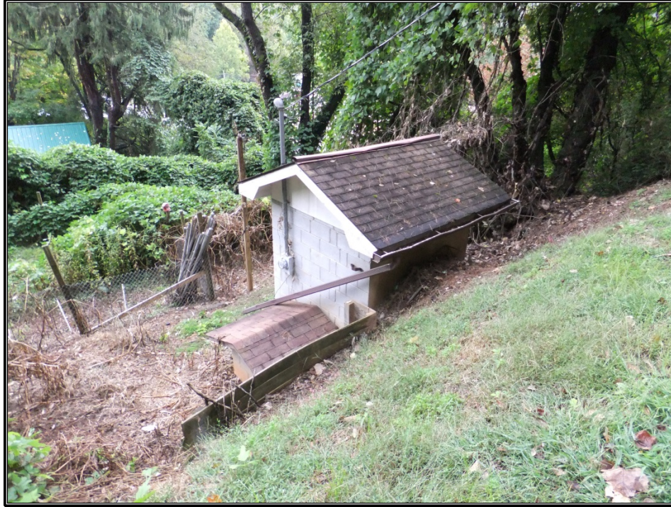
Figure 19. Southwesterly view of the pump house from Hill Street.
