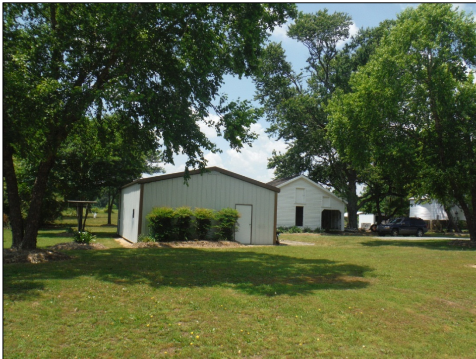
Figure 51. Outbuildings at Parrish Farms property, facing west.
