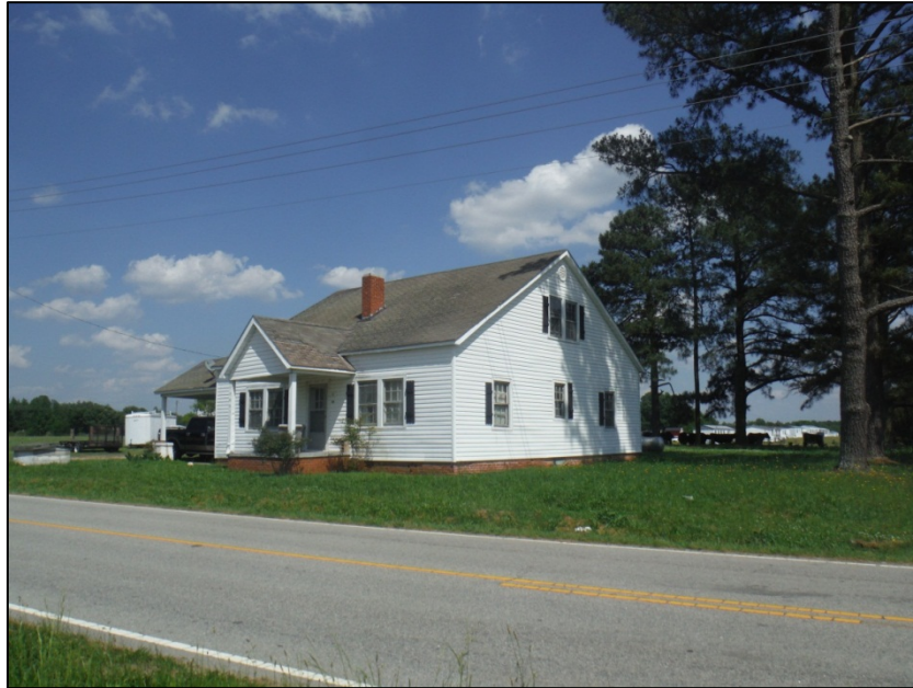
Figure 63. View of the Jones House, front elevation, facing northeast.
