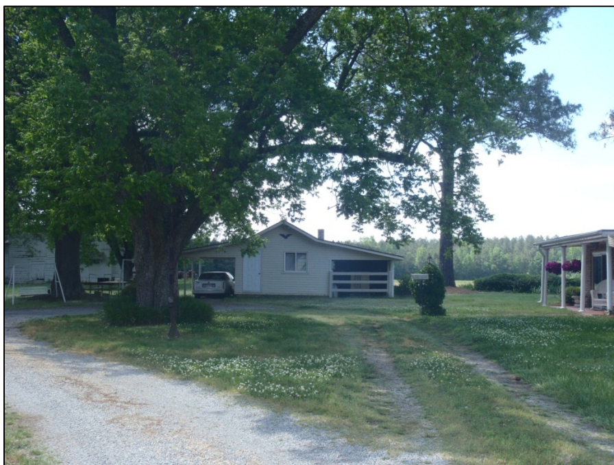
Figure 79. Carport and storage building at Langston House property, facing west.
