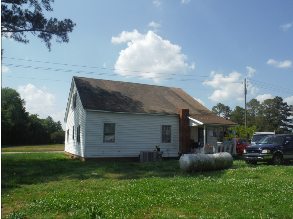
Figure 65. View of the Jones House, rear elevation, facing west.
