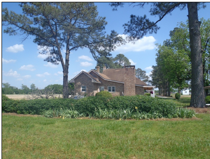
Figure 76. View of Langston House, rear elevation, facing east.
