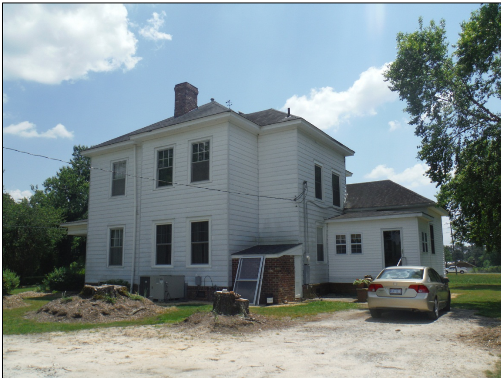
Figure 43. Oblique of Parrish Farms house, rear elevation, facing southeast.
