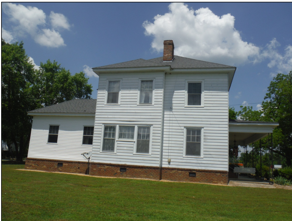
Figure 46. View of Parrish Farms house, south elevation, facing north.
