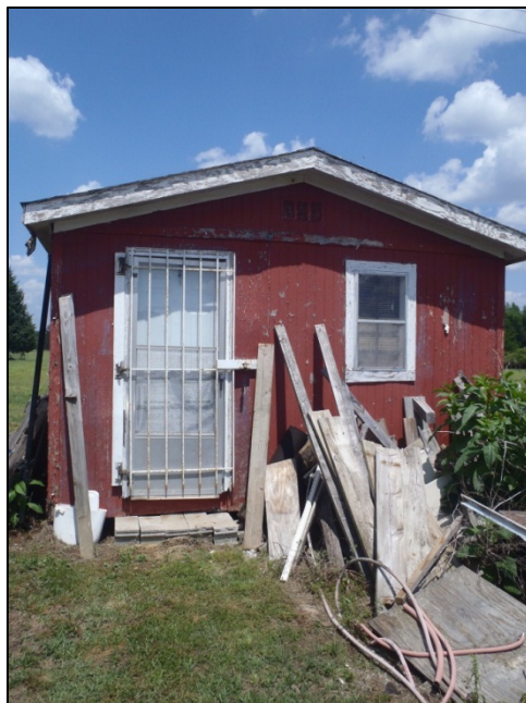
Figure 31. View of Jones Farm shed, facing north.
