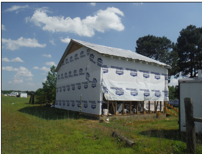
Figure 68. View of Jones House barn, facing southeast.
