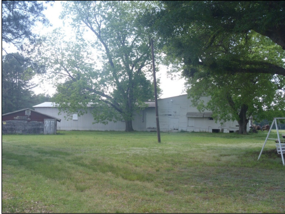
Figure 81. Barn and shed at Langston House property, facing southwest.
