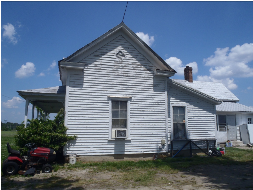
Figure 19. View of Jones Farm house, south elevation, facing north.
