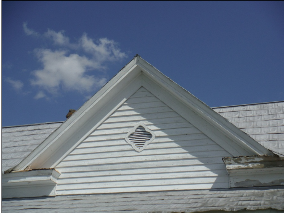
Figure 21. View of Jones Farm house, front gable detail, facing east.
