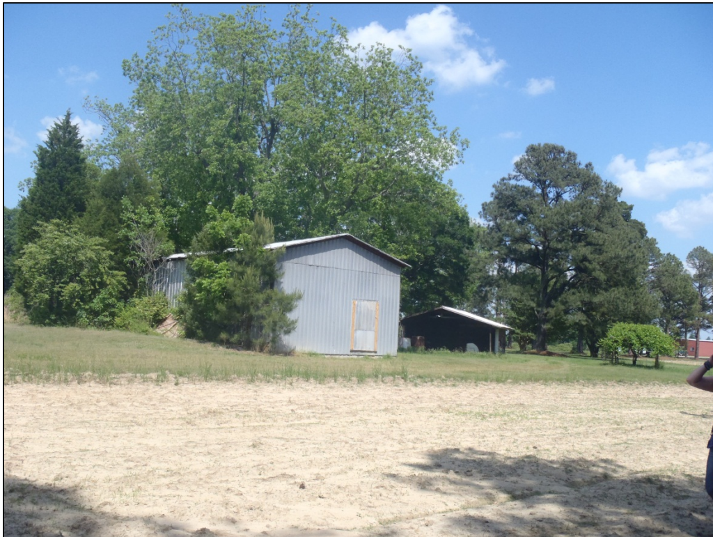
Figure 85. Barn and shed at Langston House property, facing northeast.
