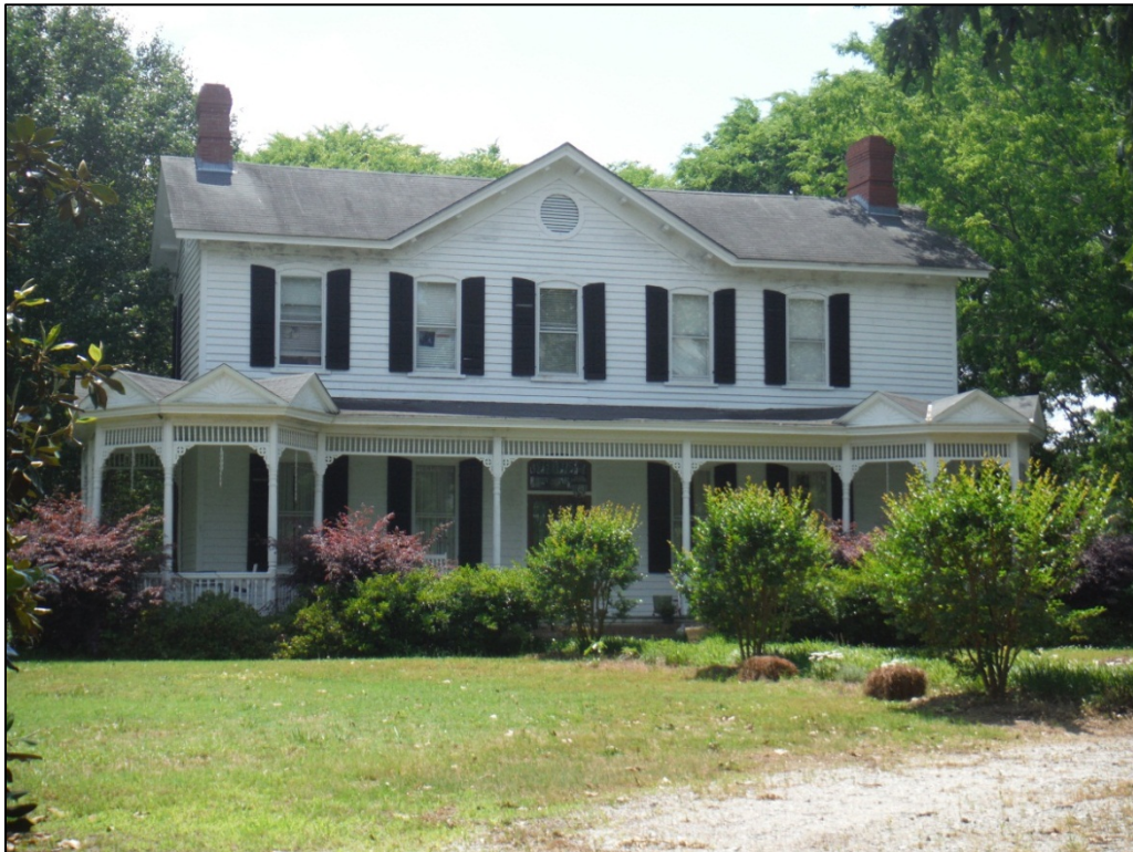
Figure 9. Parker-Wilson-Corbett House, ca. 1875, facing southwest.
