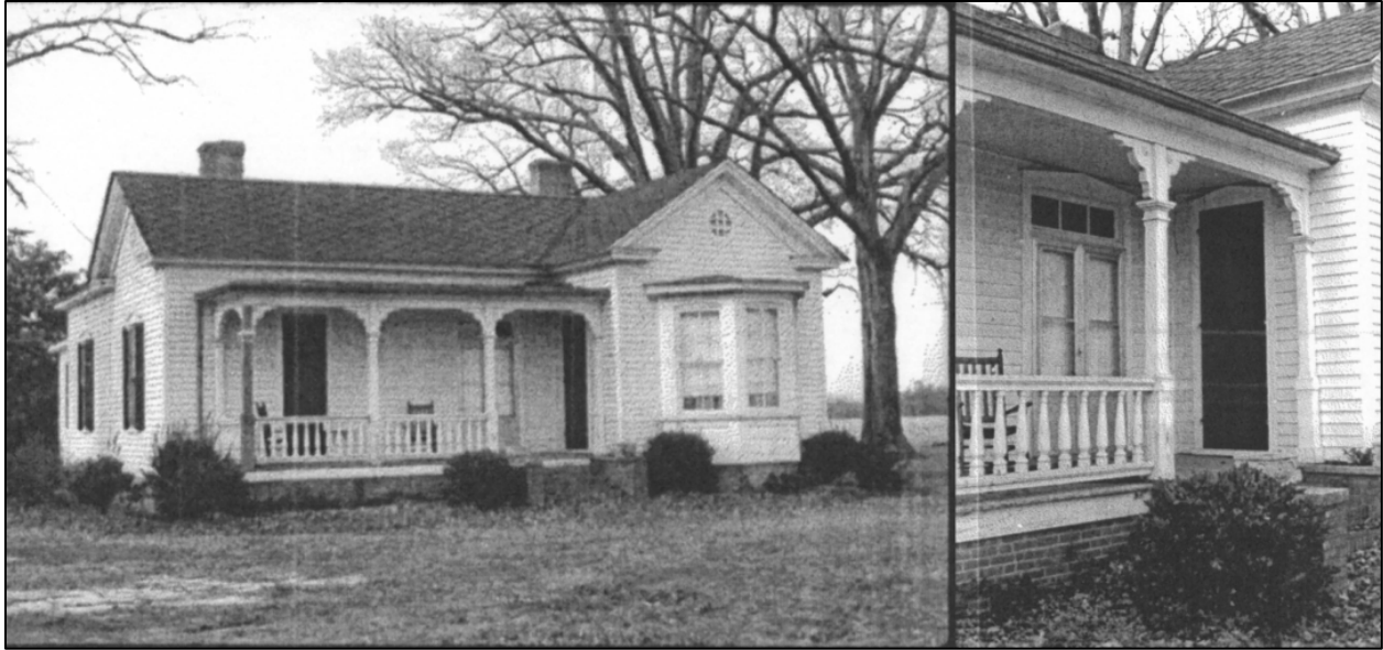
Figure 10. Robert N. Youngblood House, ca. 1890, facing south (1982 Survey Photos).
