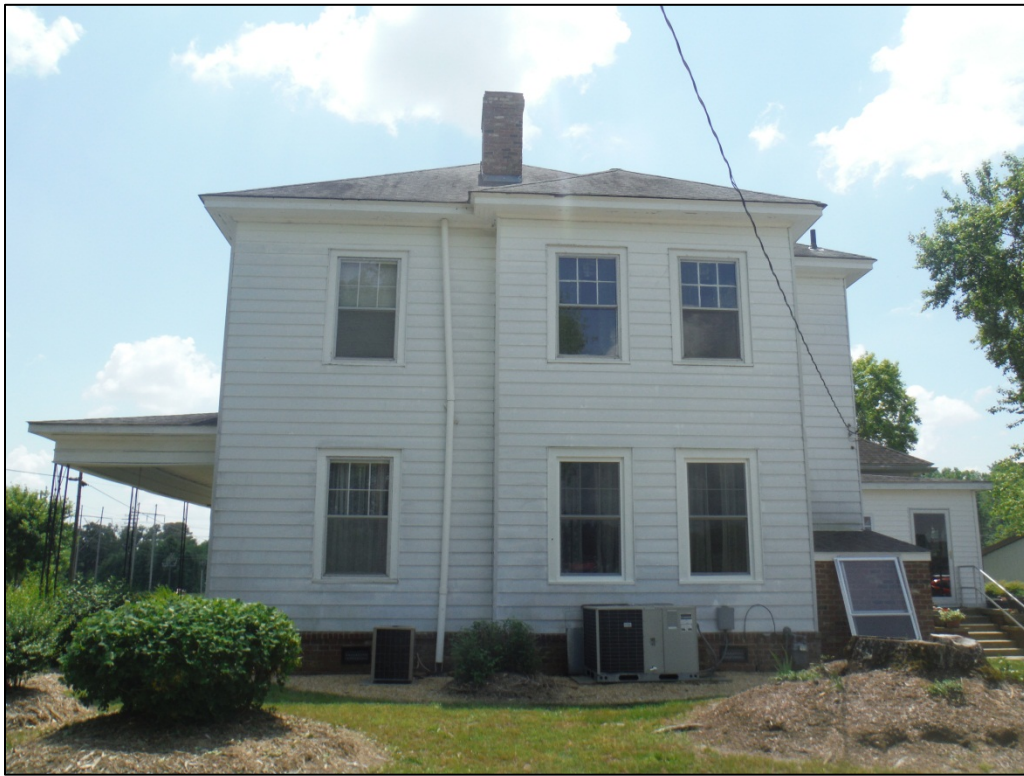
Figure 42. View of Parrish Farms house, north elevation, facing south.
