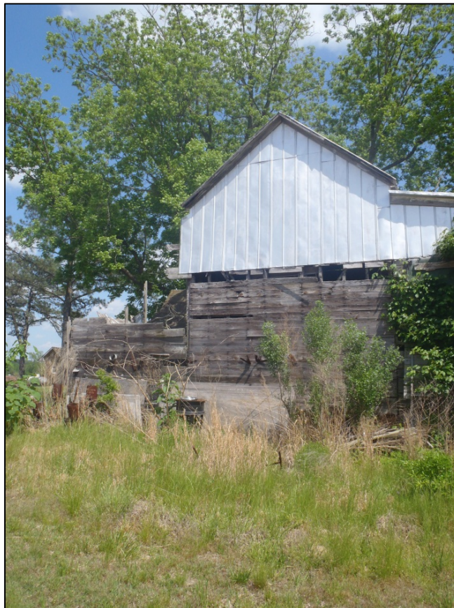
Figure 82. Barn at Langston House property, rear elevation, facing east.
