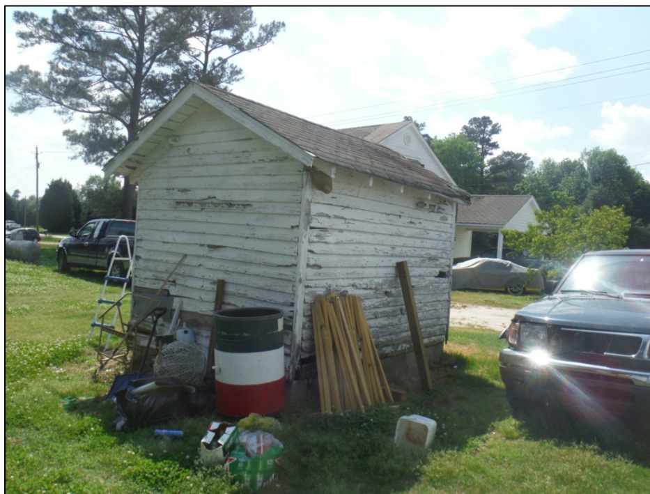
Figure 70. View of Jones House shed, facing south southwest.
