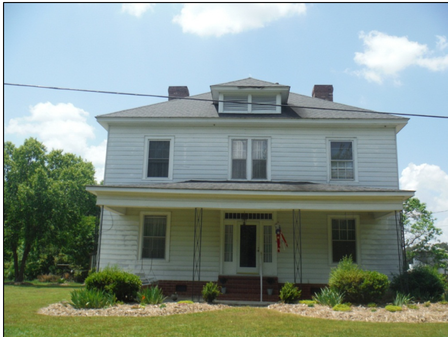
Figure 40. View of Parrish Farms house, front elevation, facing west.
