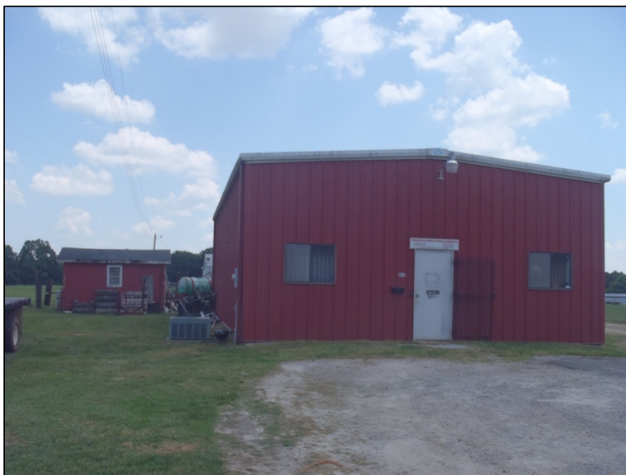
Figure 30. View of Jones Farm metal office building and shed, facing east.
