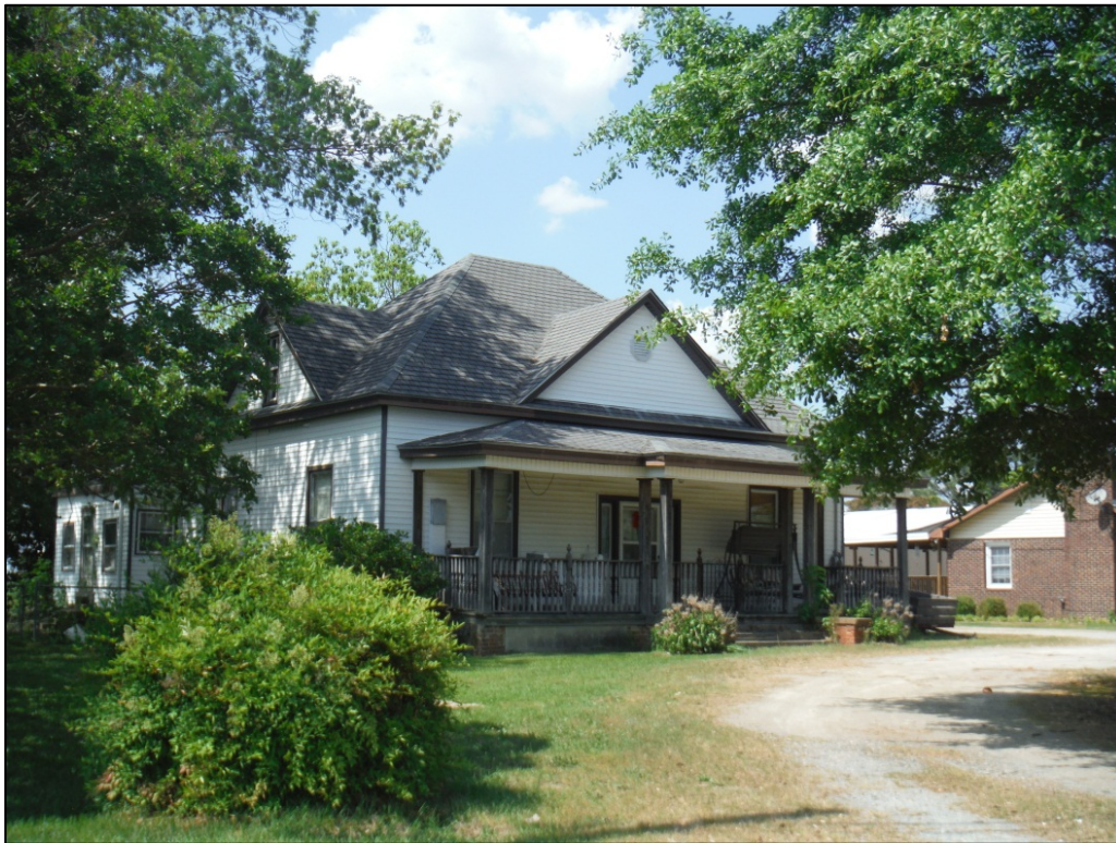
Figure 6. Photo of hipped roof, false gable style house, located along NC 210 west of Smithfield, facing northwest.
