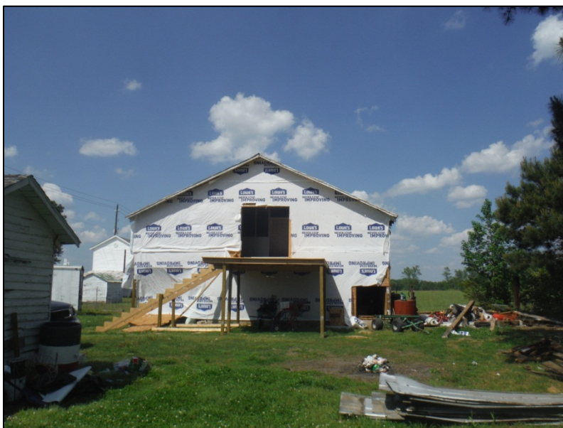
Figure 67. View of the Jones House barn, facing north.
