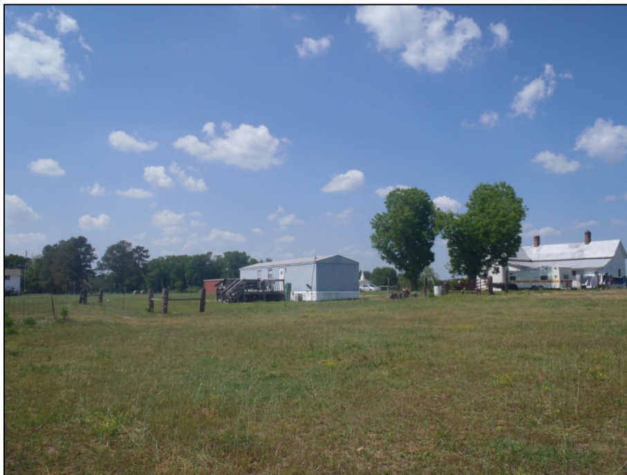
Figure 26. View of Jones Farm house, trailer, and landscape, facing northwest.
