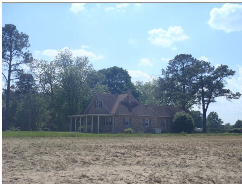
Figure 77. Oblique view of Langston House, facing southwest.
