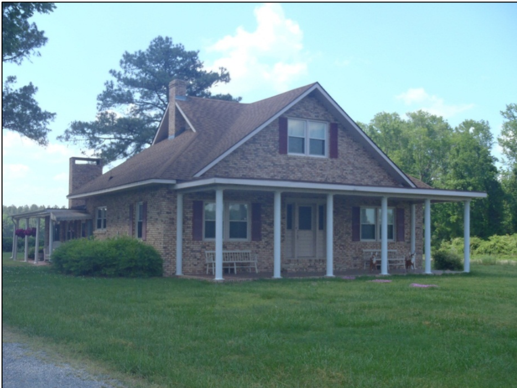
Figure 75. Oblique view of Langston House, facing northwest.
