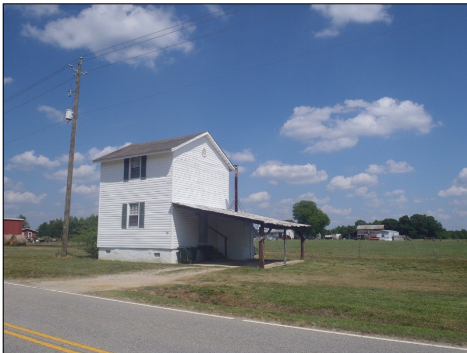
Figure 27. View of Jones Farm converted tobacco barn, facing northeast.
