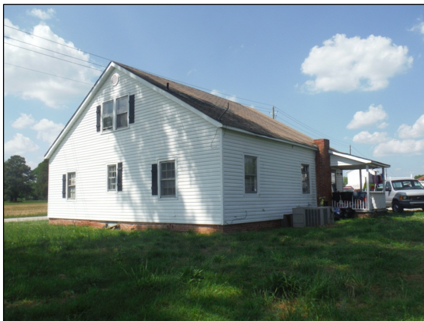
Figure 64. View of Jones House, rear oblique, facing northwest.
