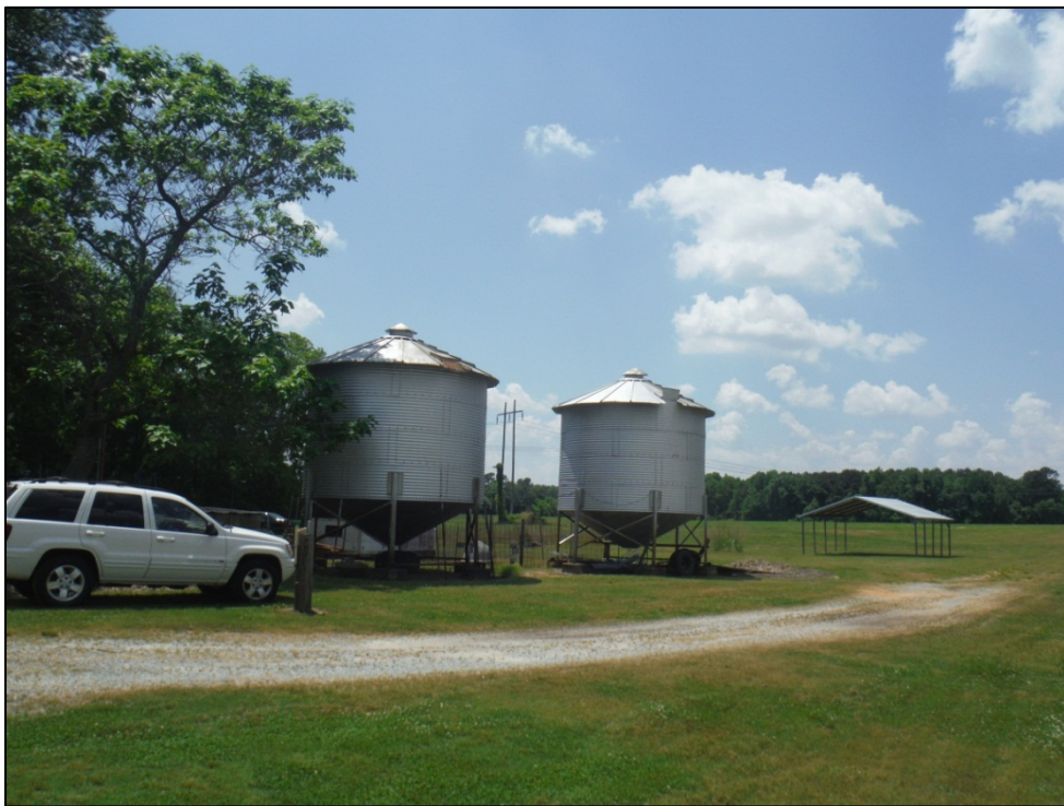
Figure 55. Silos and metal shelter at Parrish Farms property, facing southwest.
