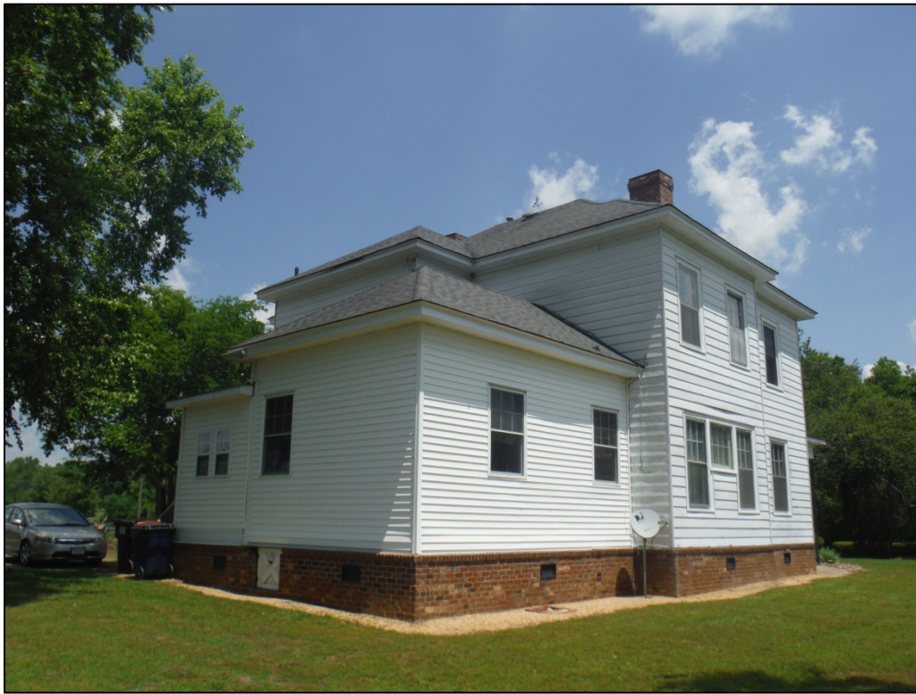
Figure 44. Oblique of Parrish Farms house, facing northeast.
