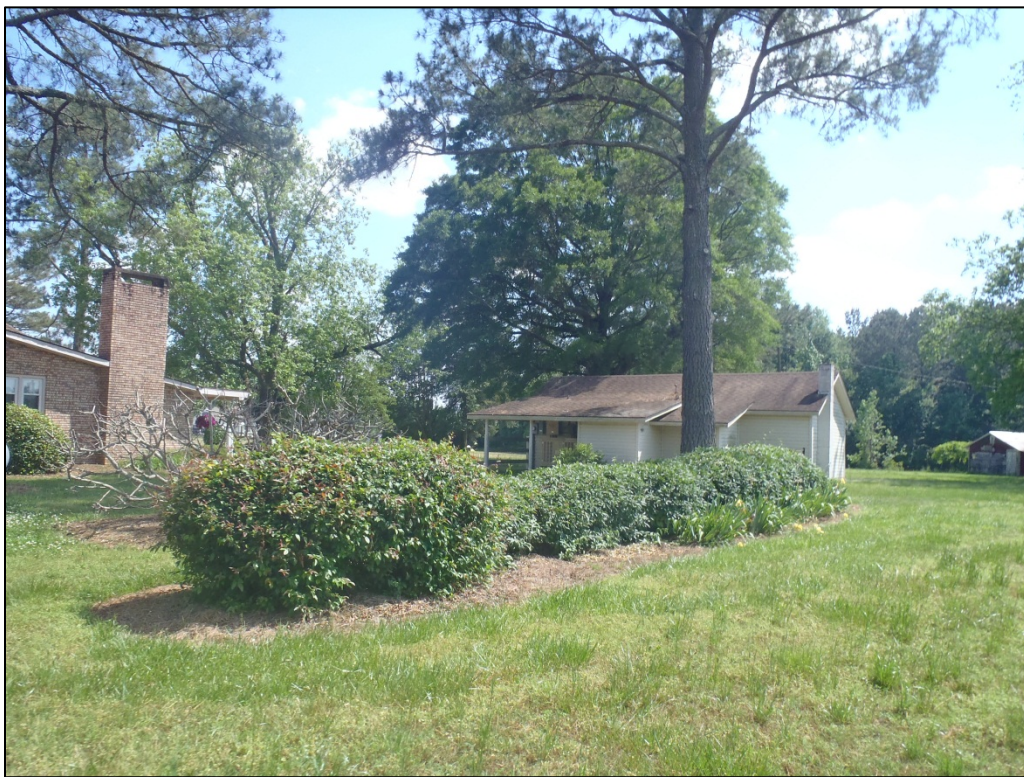
Figure 80. Garage at Langston House property, oblique view, facing east.
