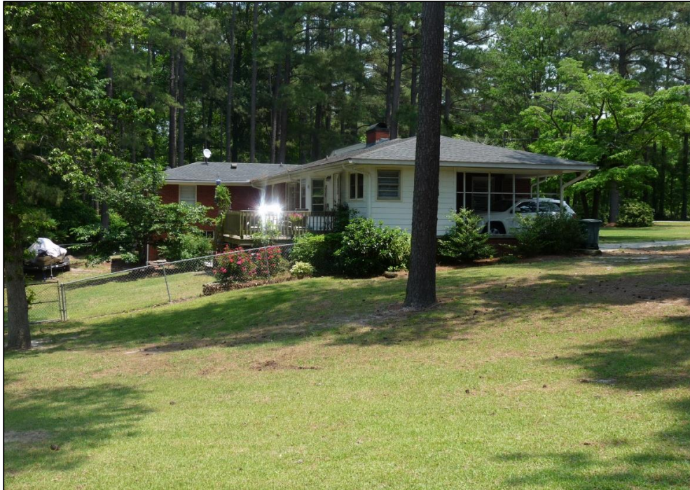
Photo 19: Northeast Oblique View of Residence. Note wooden deck and partially enclosed carport.
