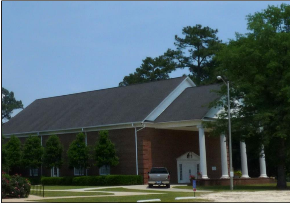
Photo 6: View of 1991 Addition, Looking Northeast.
