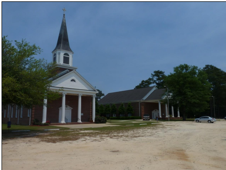
Photo 1: View of the Galatia Presbyterian Church Property, Looking Northeast from Galatia Church Road (SR 1103). Original (1960) section on left, 1991 addition on right.
