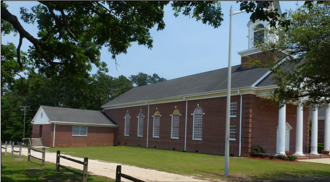
Photo 4: View of West Elevation, Looking Northeast from the Adjacent Cemetery. The sanctuary is on the right, while classrooms occupy the rear projecting wing. Both sections were built in 1960.
