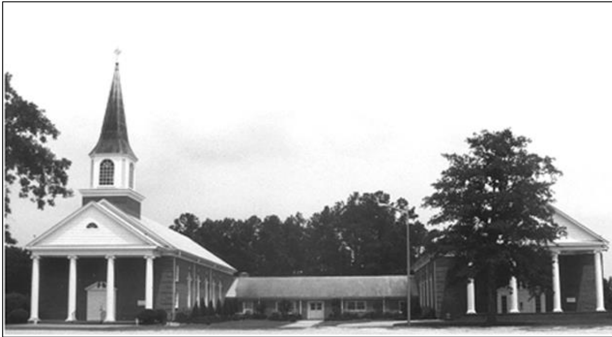
Figure 12: Undated photograph (post-1991) Showing the New Eastern Addition to the Galatia Presbyterian Church. Half of the central wing, as well as the entire eastern Fellowship Hall, were added to the original (1960) building to the left of the photograph.
