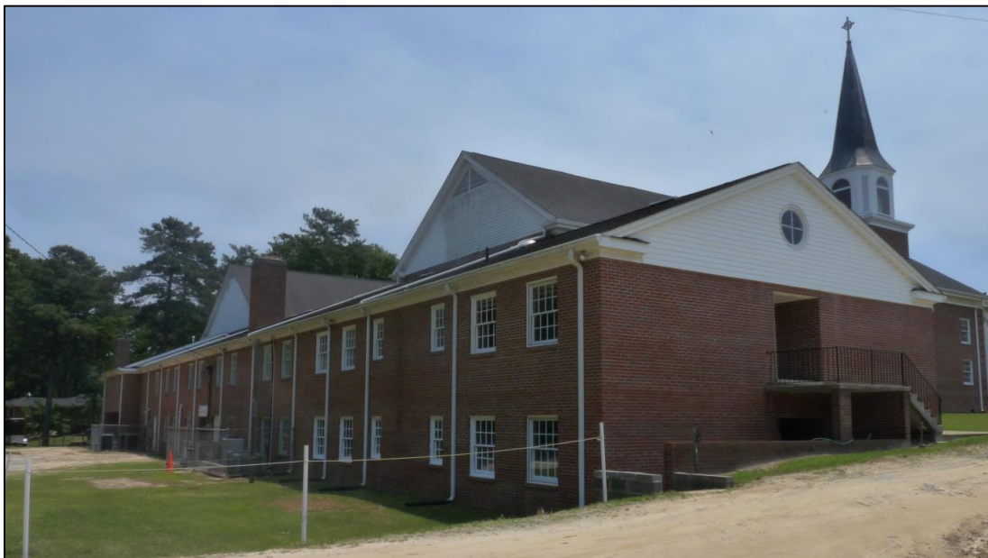
Photo 5: View of the Rear (North) Section of the Church, Looking Southeast.
