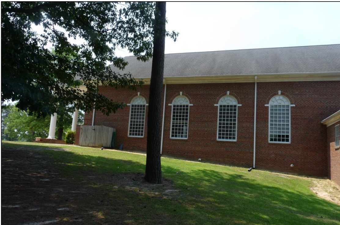
Photo 8: View of Eastern Elevation of 1991 Addition, Looking West.
