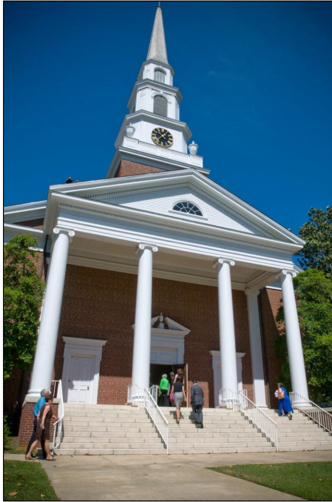
Photo 21: View of the main elevation of the Snyder Memorial Baptist Church in Fayetteville.
