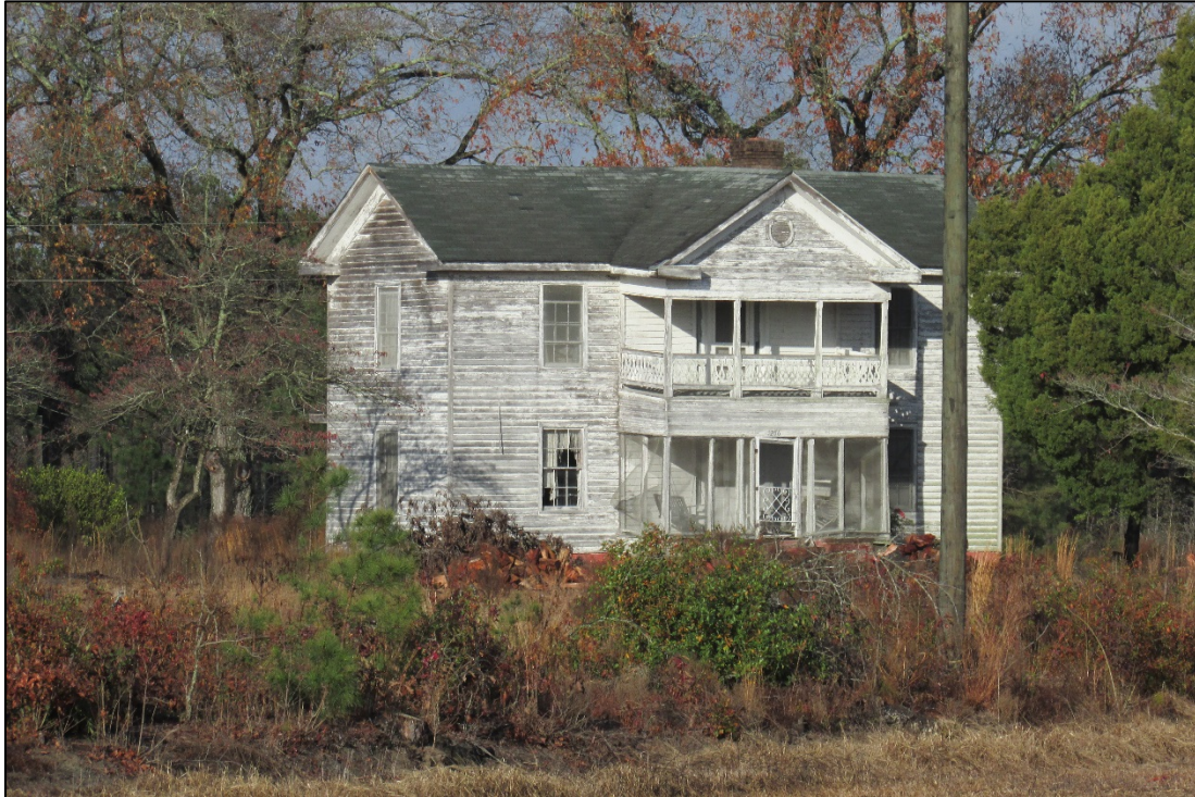
Figure 3. RB0678, dwelling house, facing northwest.
