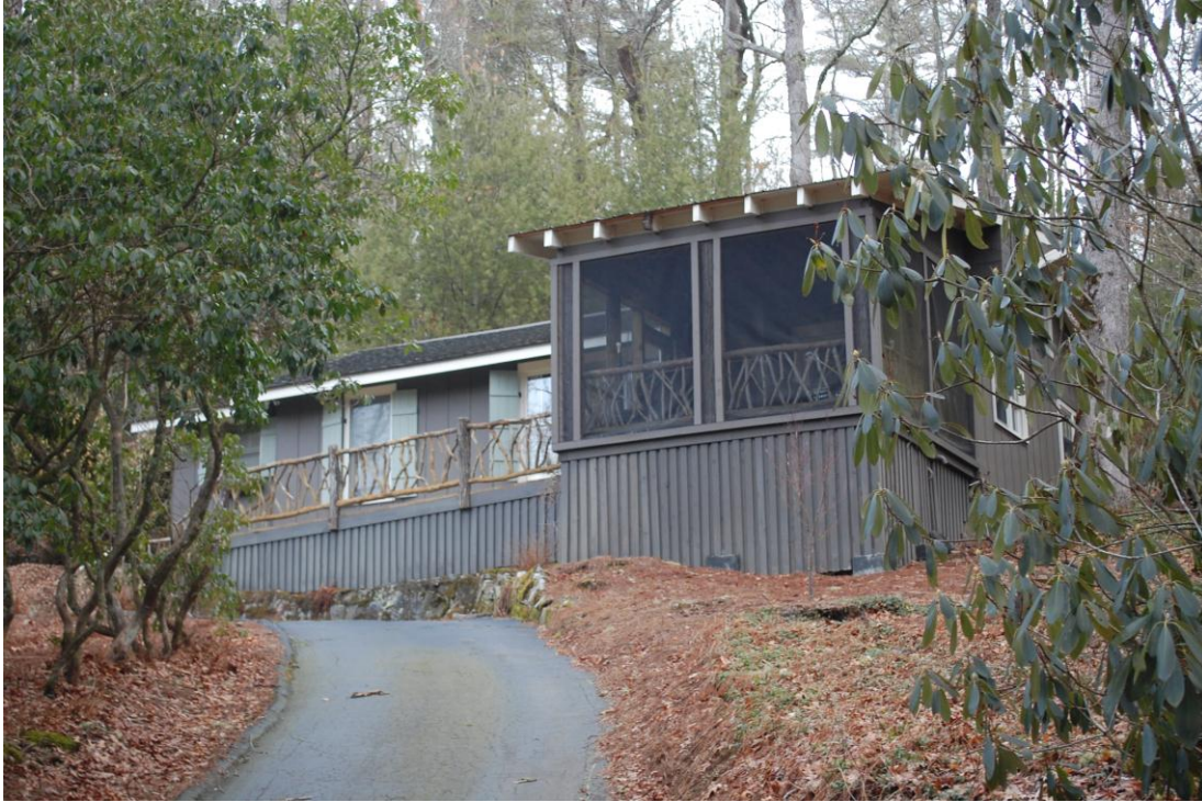
Figure 13: House at 932 Hickory Hill Road, view to the north
