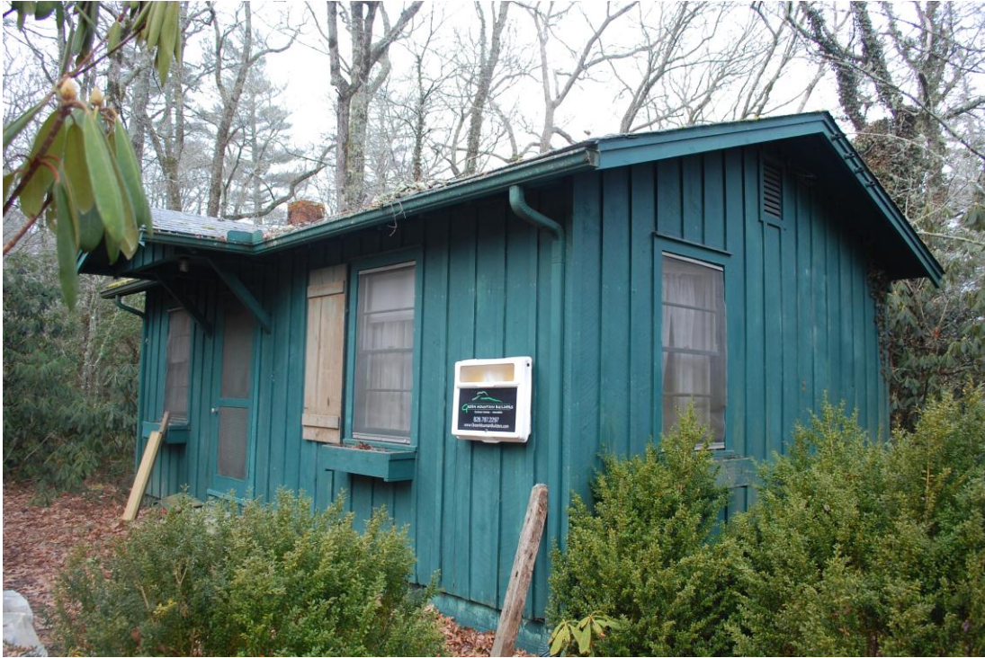
Figure 15: House at 172 Bowery Road, view to the northwest
