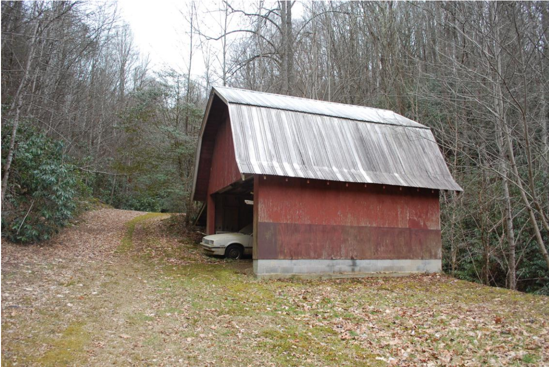
Figure 12: Barn, view to southwest
