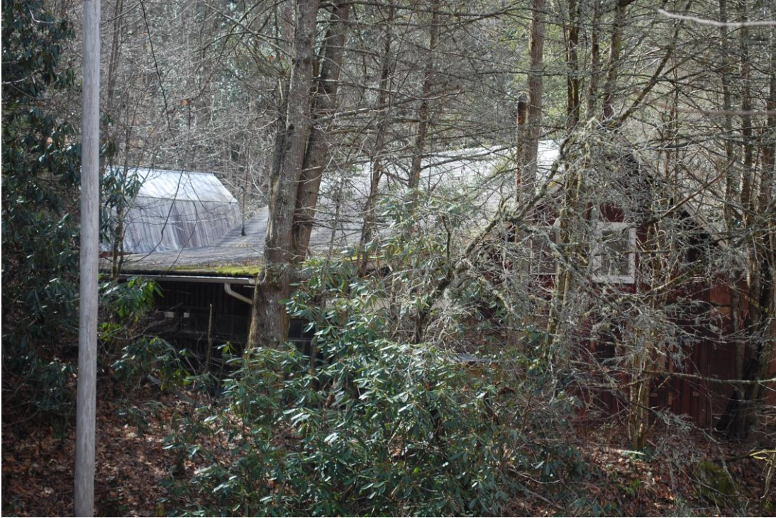
Figure 10: Secondary dwelling, northeast corner, view to the southwest
