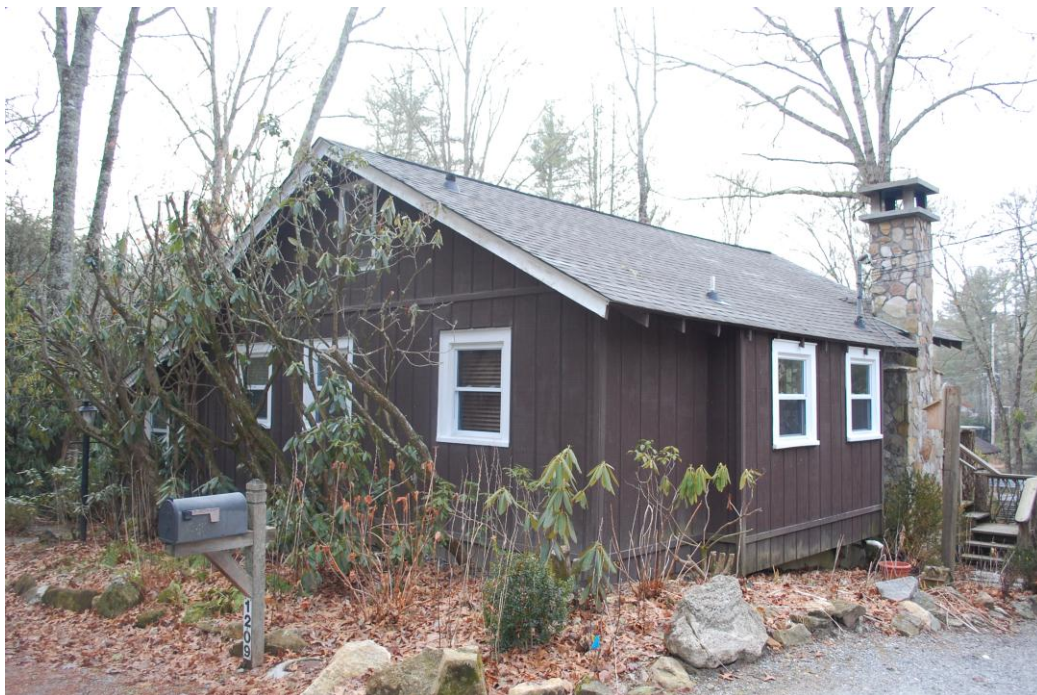
Figure 14: House at 1209 Hickory Hill Road, view to the southeast
