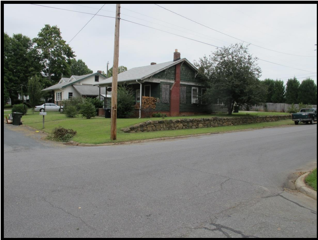
Figure 22: View of Stone Retaining Wall at the Corner of Broad Street and Second Street (now Twelfth Street), Looking Northeast.
