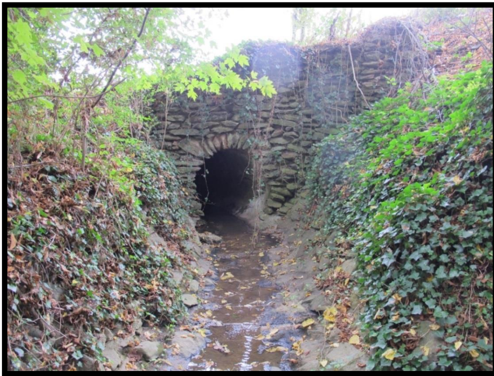
Figure 3: View of Channelized Section of Unnamed Tributary of Michael Branch and Stone-faced Headwall, Looking East.
