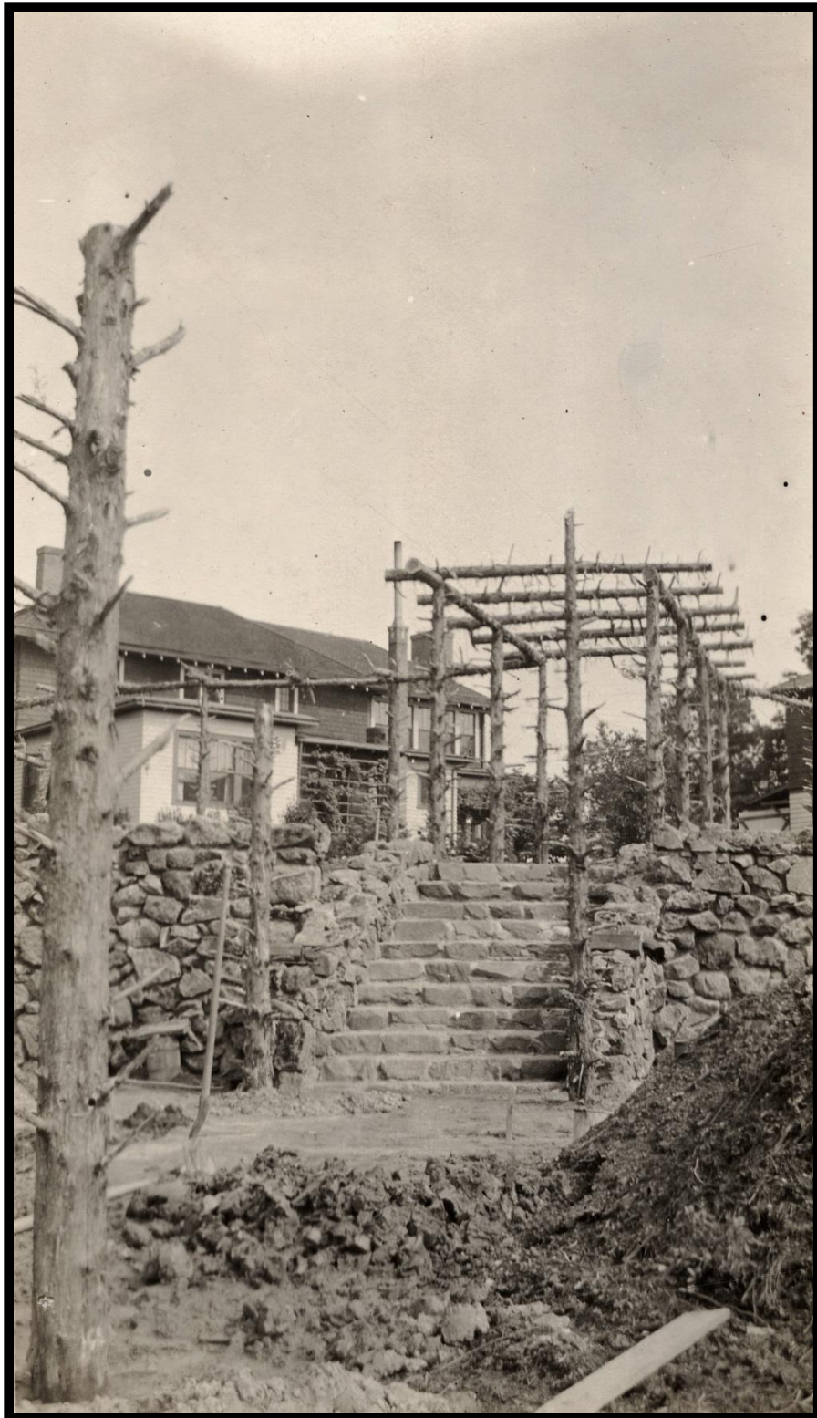
Figure 29: Undated Historic Photograph Showing the Stone Retaining Walls and Steps Leading Down to the Footpath at the Rear of the Superintendent's House, Looking Southeast (North Carolina Collection Photographic Archives 2014b).
