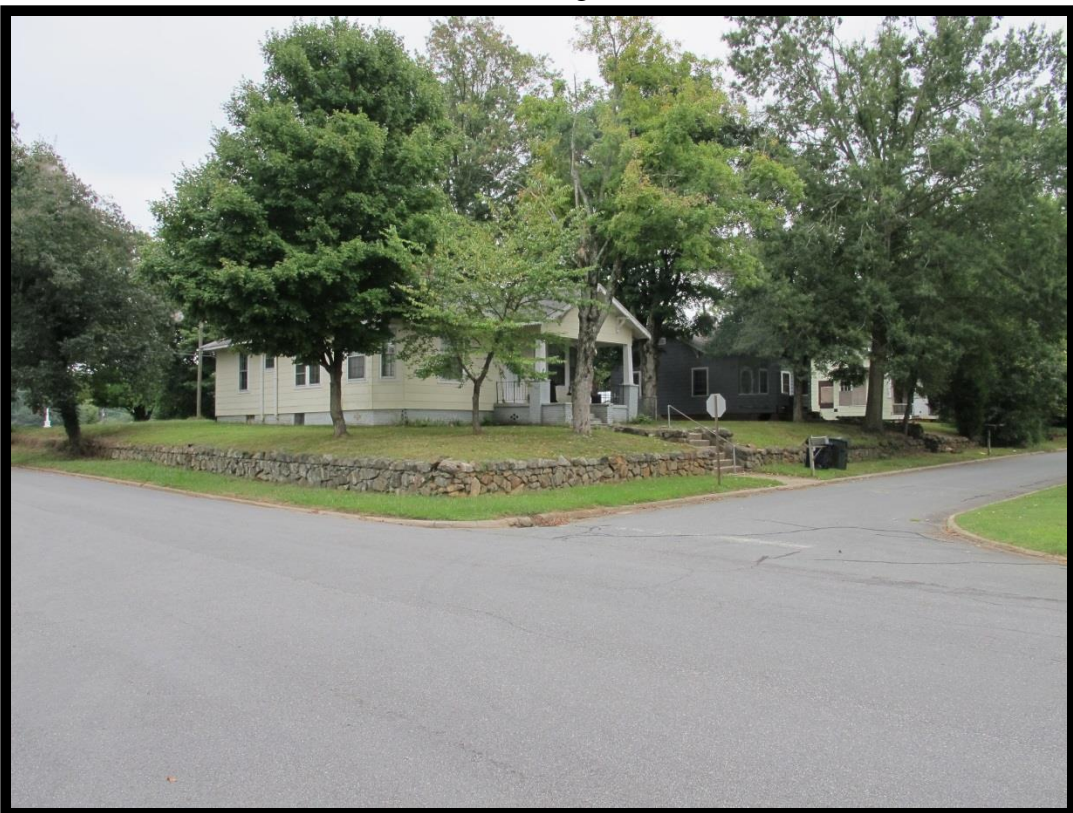
Figure 23: View of Stone Retaining Wall at the Corner of Broad Street and Second Street (now Twelfth Street), Looking Southeast.
