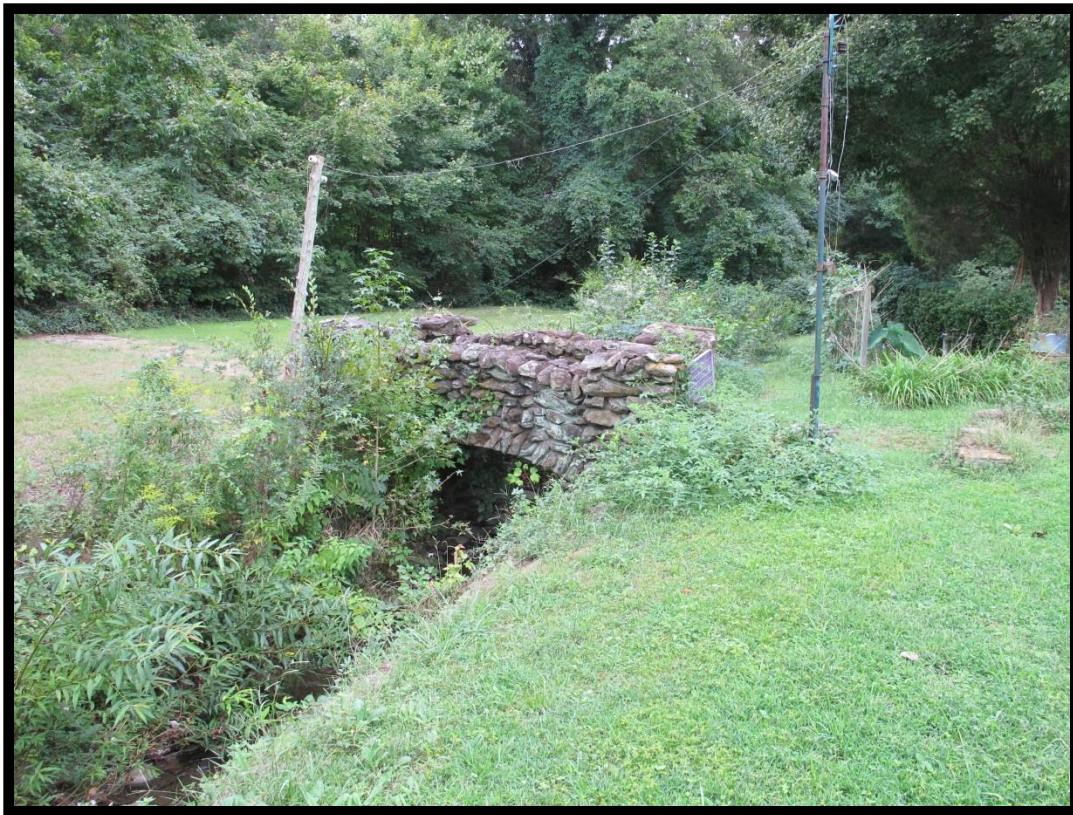
Figure 11: View of Bridge over Unnamed Tributary of Michael Branch, Looking Southwest.
