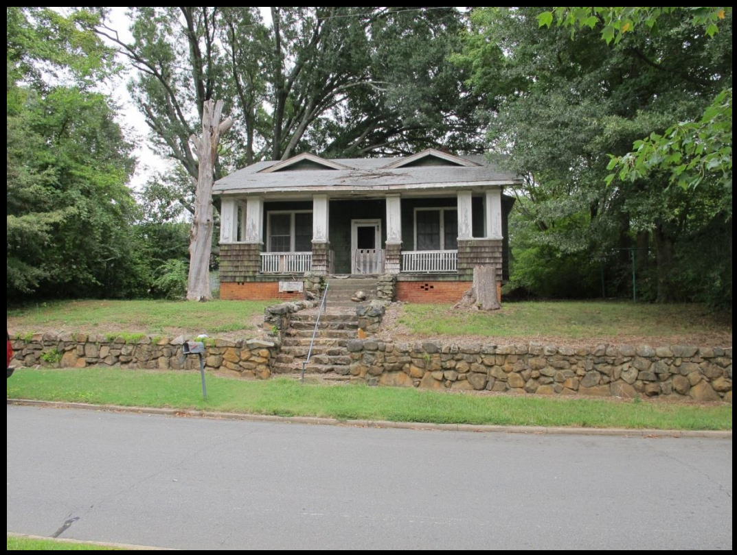
Figure 25: Detail of Stone Retaining Wall and Stone Steps in the 200-Block of Broad Street, Looking East.
