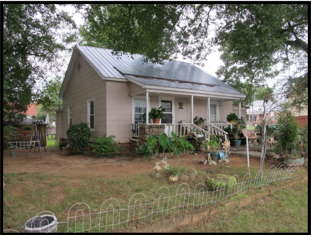
Figure 21: Mill House at 28 Church (Hames) Street, Looking Northwest.
