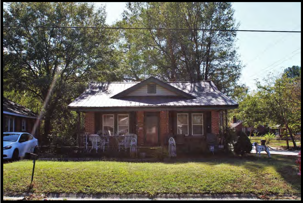
Figure 59: House, 310 Murray Street, Looking South.
