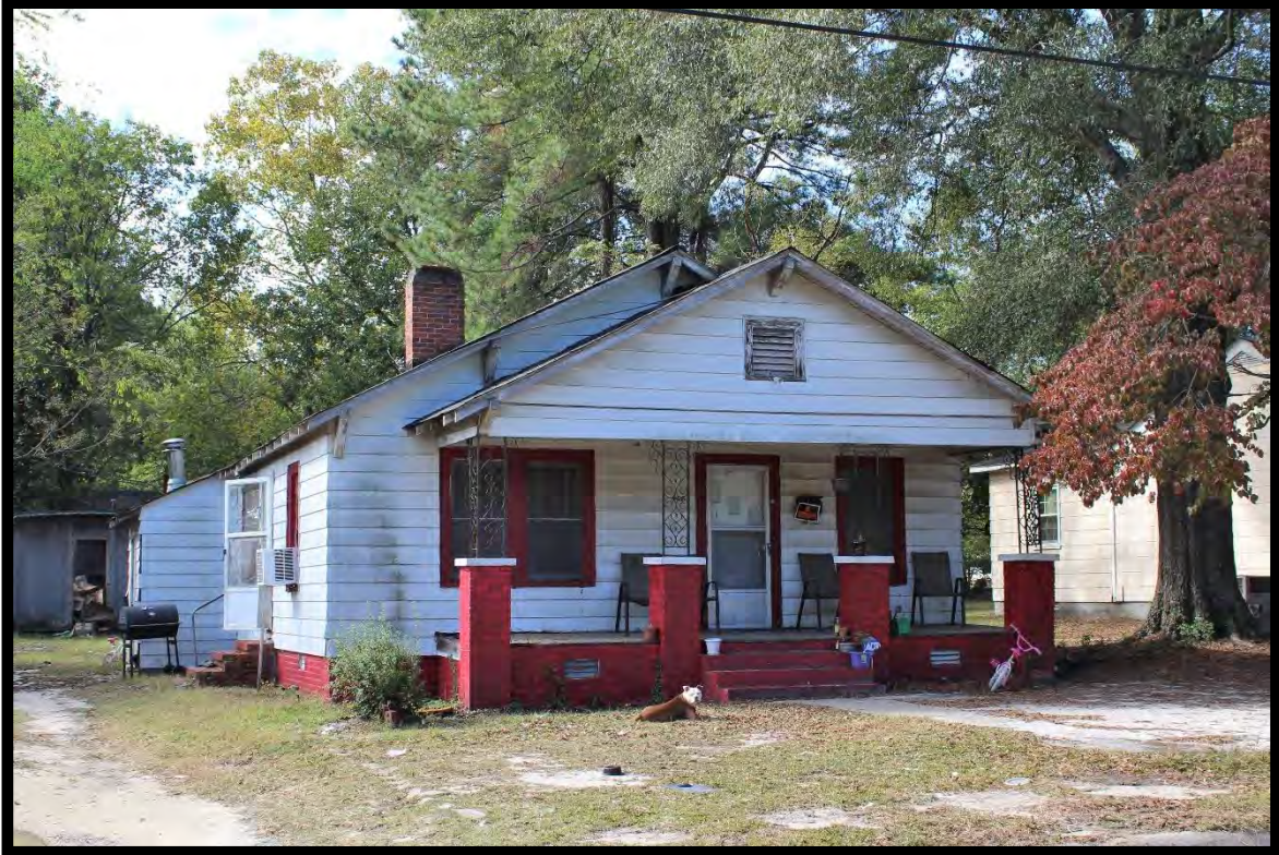
Figure 97: House, 408 Murray Street, Looking Southwest.
