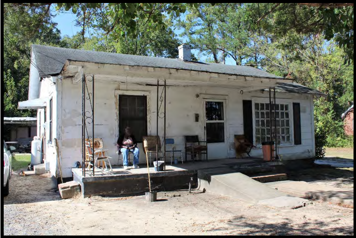
Figure 77: House, 809 North Virginia Street, Looking Northwest.
