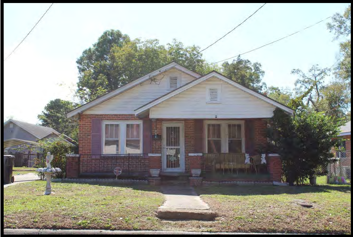
Figure 57: House, 306 Murray Street, Looking South.
