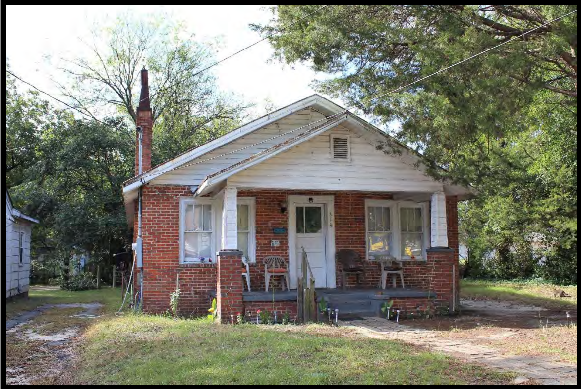
Figure 99: House, 414 Murray Street, Looking Southwest.
