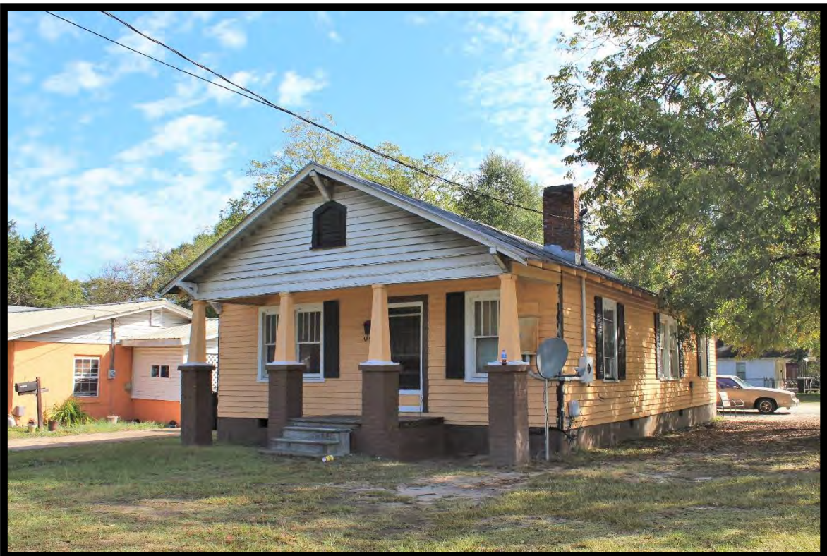
Figure 102: House, 900 North Carolina Street, Looking Northeast.
