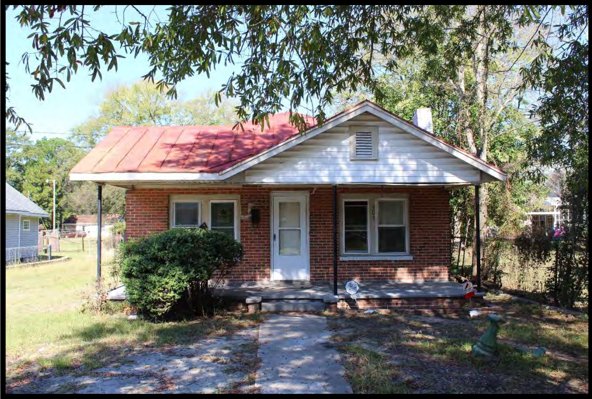
Figure 63: House, 305 Brownrigg Street, Looking North.
