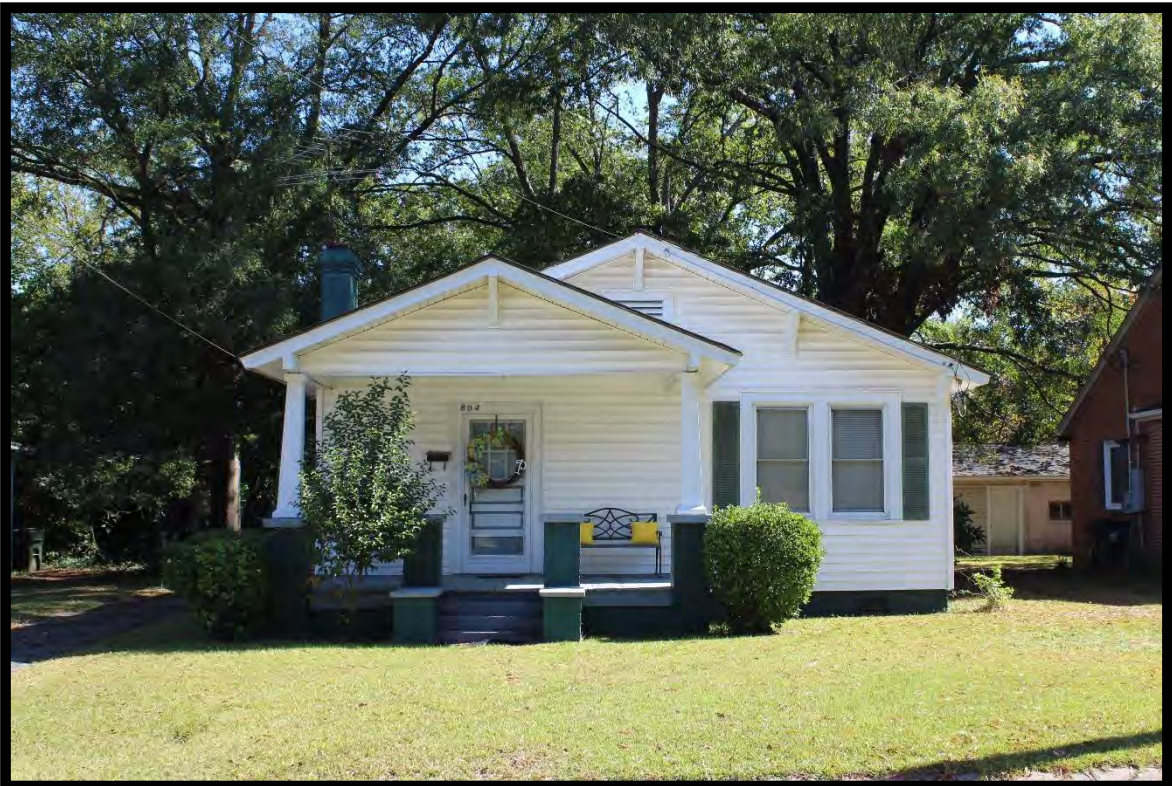
Figure 48: House, 804 North Virginia Street, Looking East.
