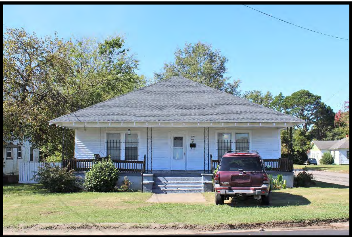
Figure 56: House, 909 North George Street, Looking West.
