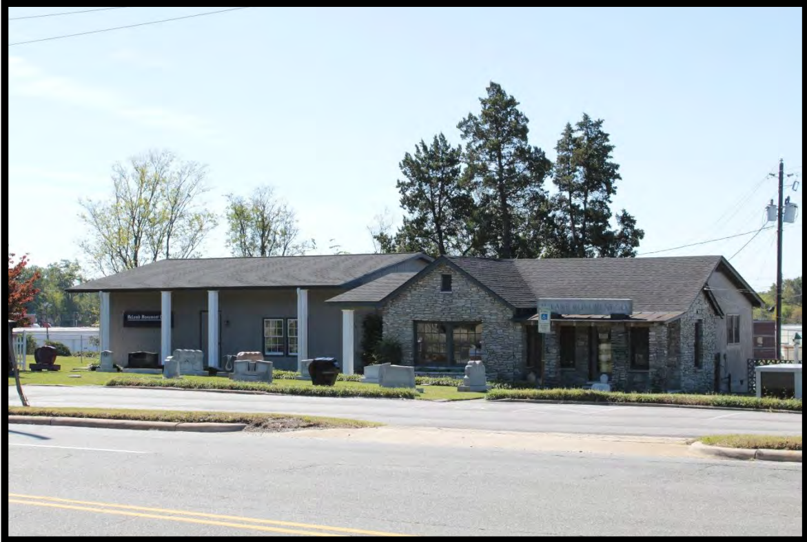
Figure 72: Commercial Building (Office and Showroom), 416 West Grantham Street, Looking South.
