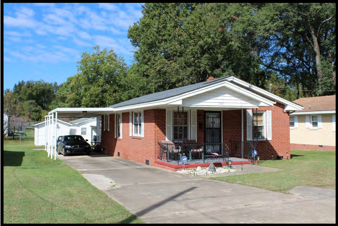
Figure 107: House, 1005 North Virginia Street, Looking Northwest.
