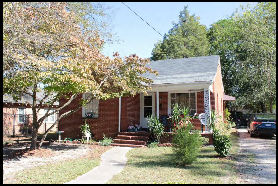
Figure 61: House, 902 North Virginia Street, Looking East.
