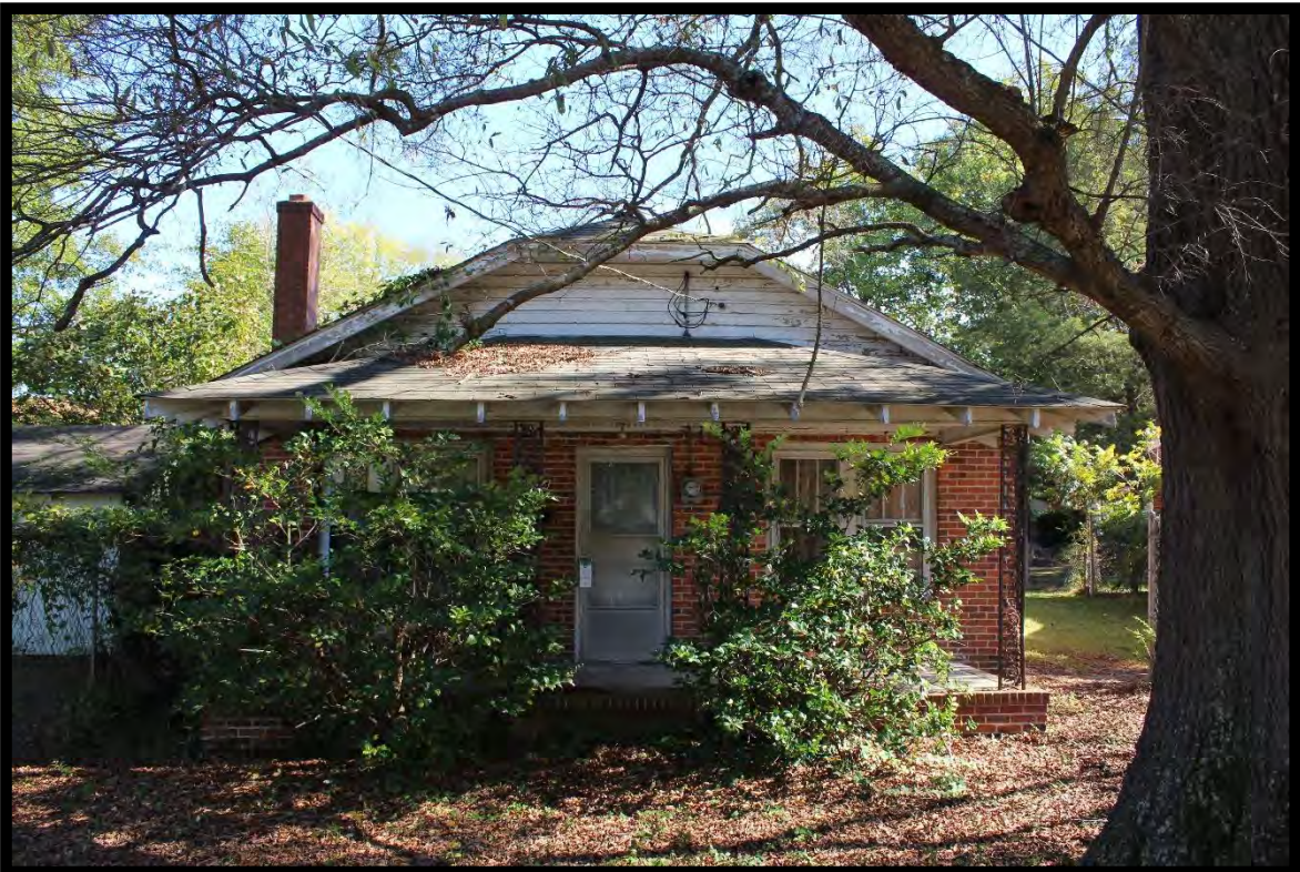
Figure 60: House, 904 North Virginia Street, Looking East.
