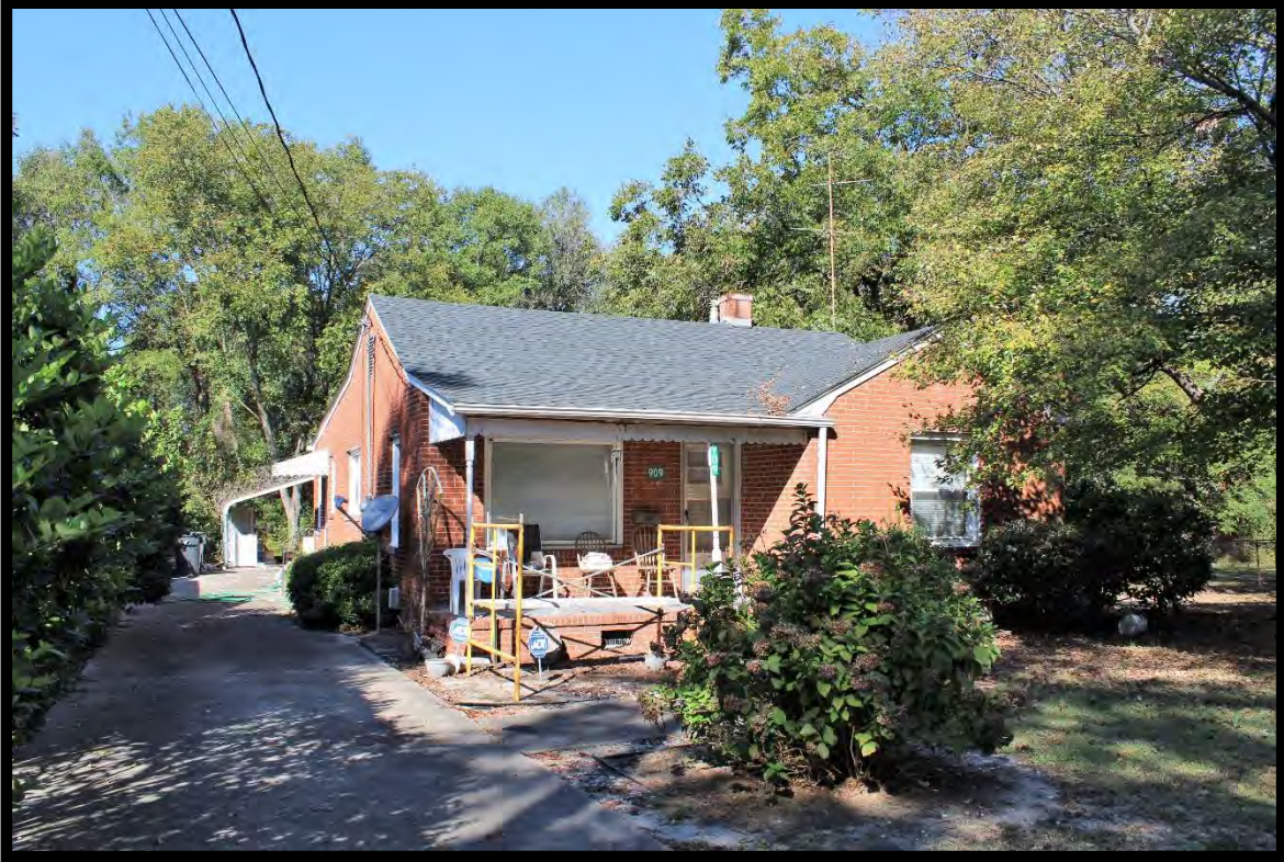
Figure 124: House, 909 North Carolina Street, Looking West.
