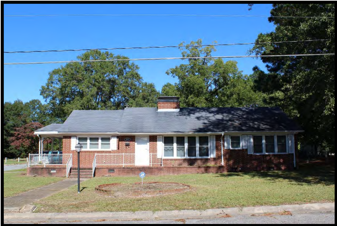
Figure 66: House, 309 Murray Street, Looking North.
