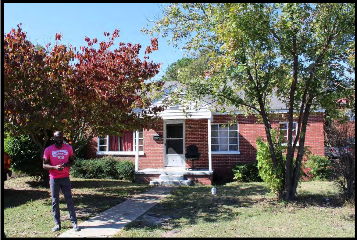
Figure 39: House, 811 North George Street, Looking West.
