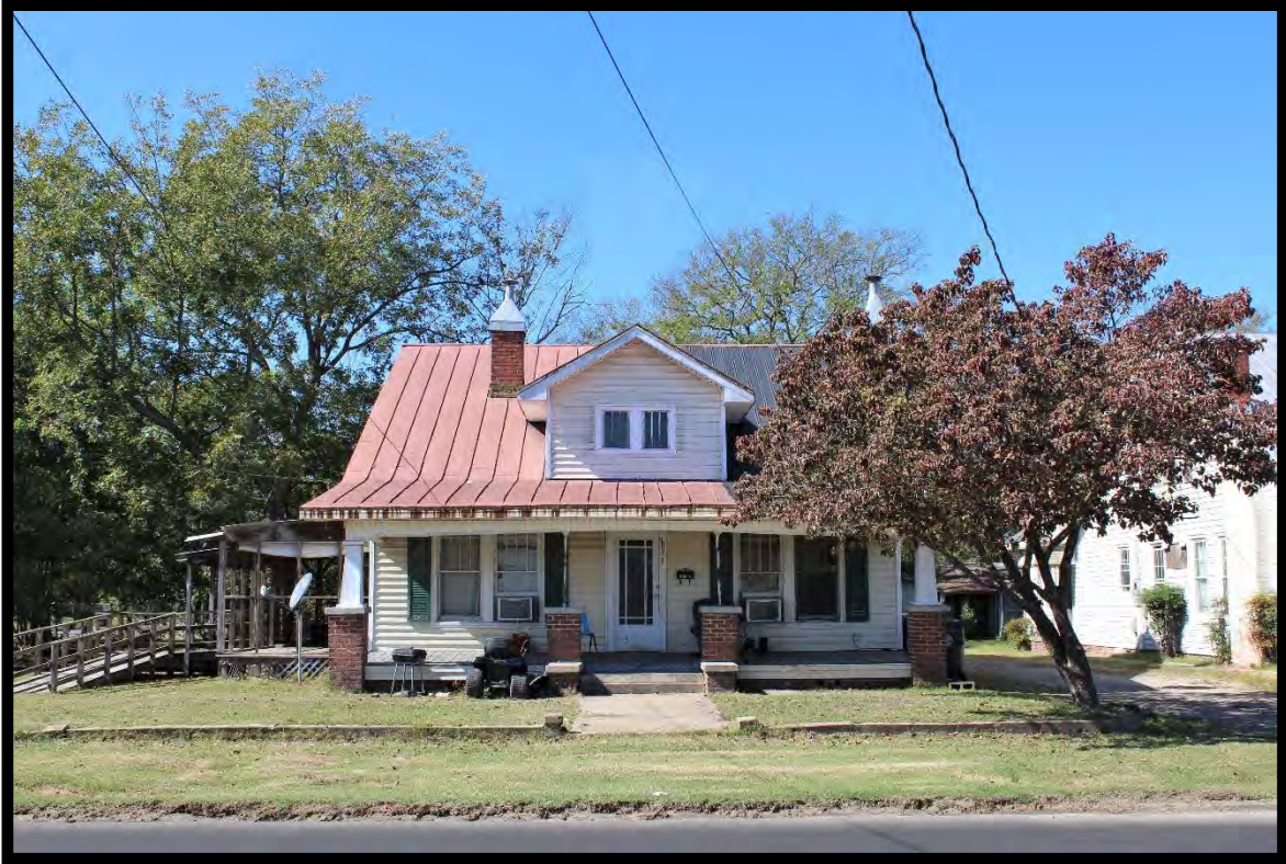
Figure 53: House, 903 North George Street, Looking West.
