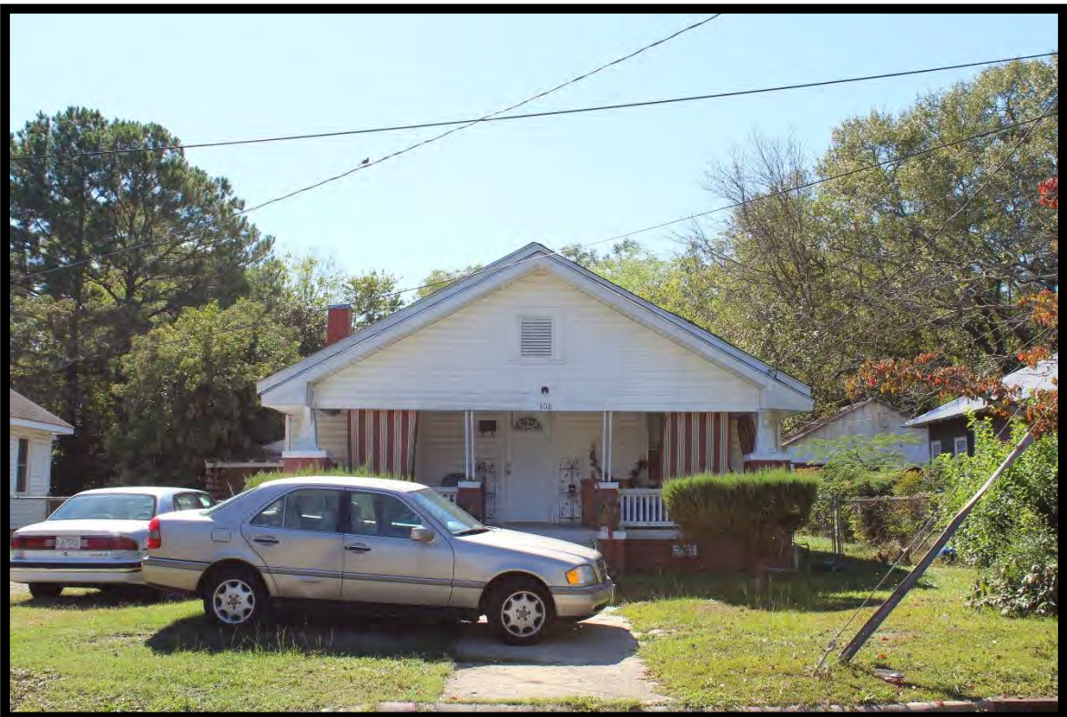
Figure 42: House, 308 Brownrigg Street, Looking South.
