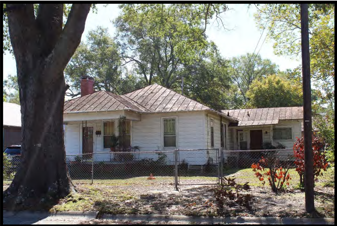
Figure 44: House, 312 Brownrigg Street, Looking Southeast.
