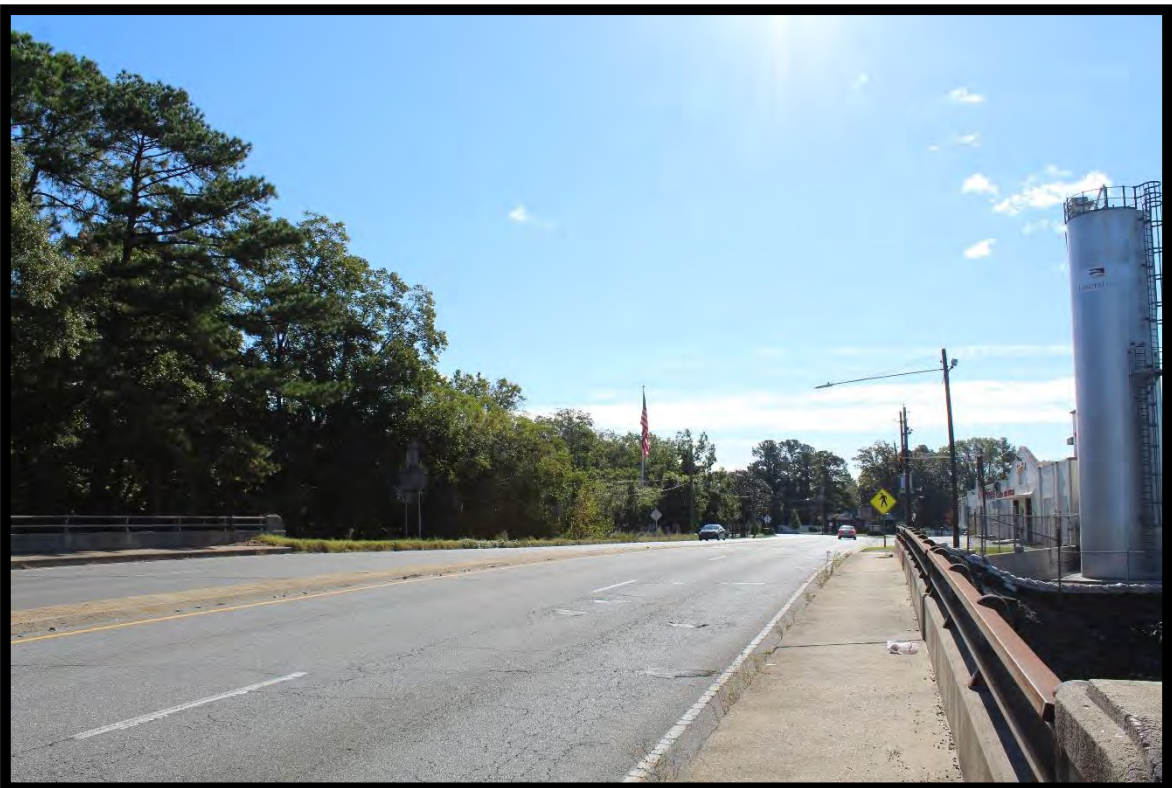
Figure 8: West Grantham Street and Bridge, Looking Southeast to Oak Heights.
