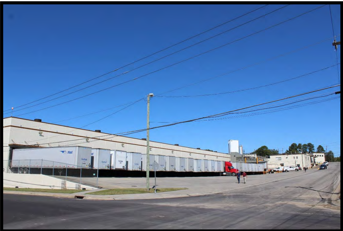
Figure 116: Franklin Baking Company, 500 West Grantham Street, Looking North.
