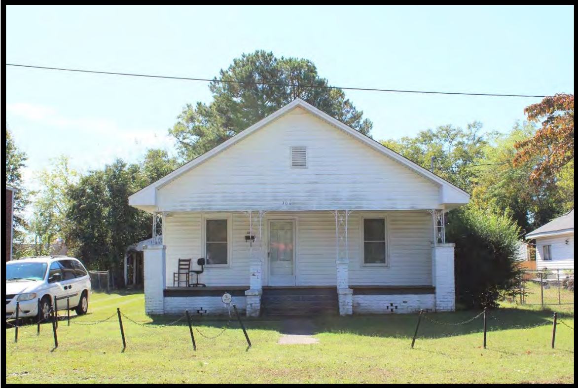
Figure 41: House, 306 Brownrigg Street, Looking South.
