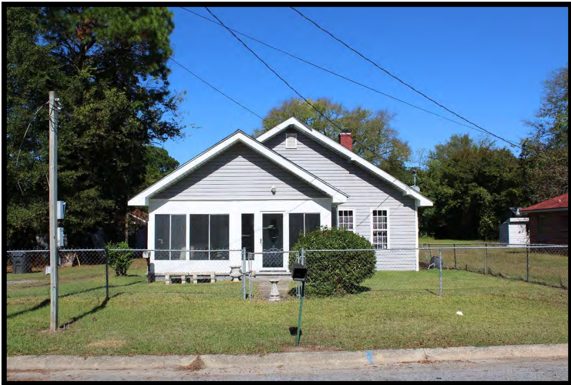
Figure 62: House, 307 Brownrigg Street, Looking North.
