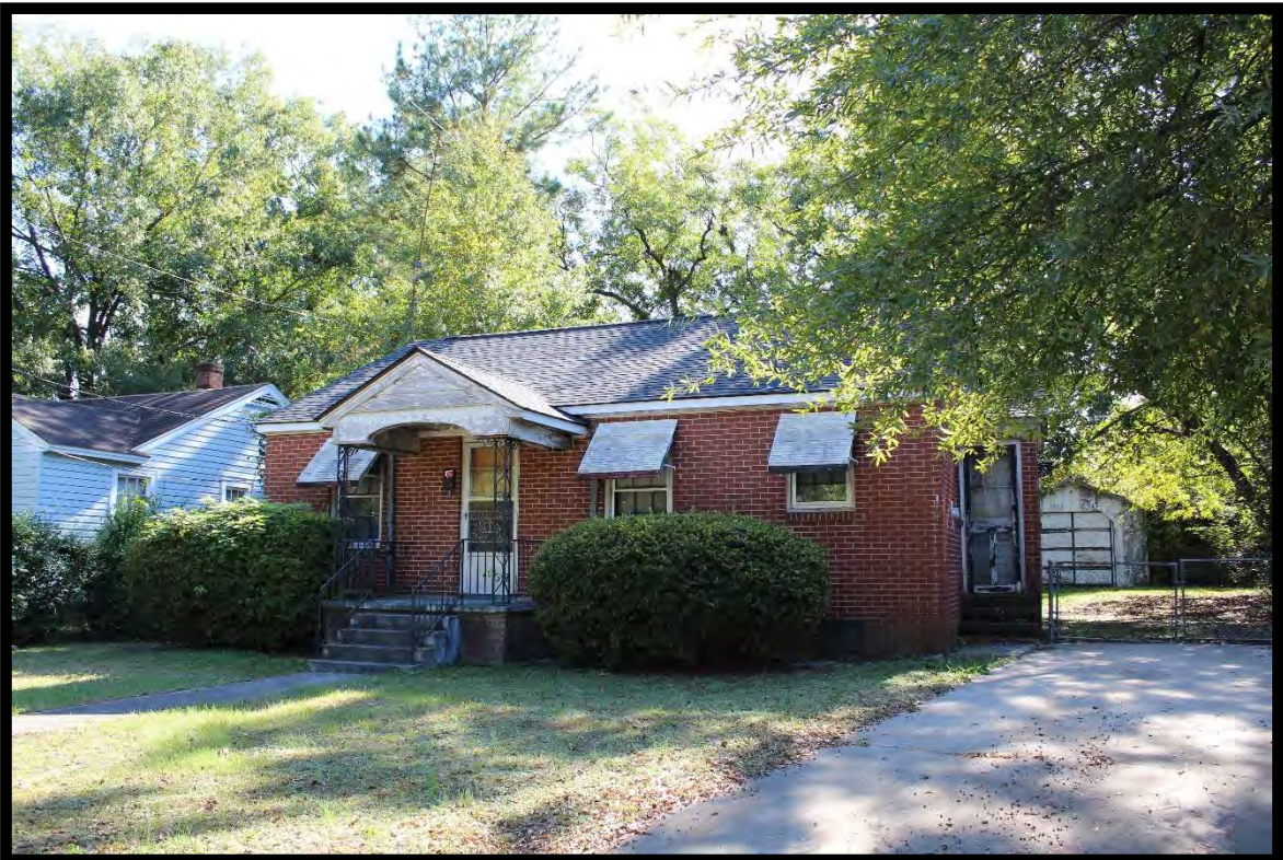
Figure 82: House, 408 Brownrigg Street, Looking South.
