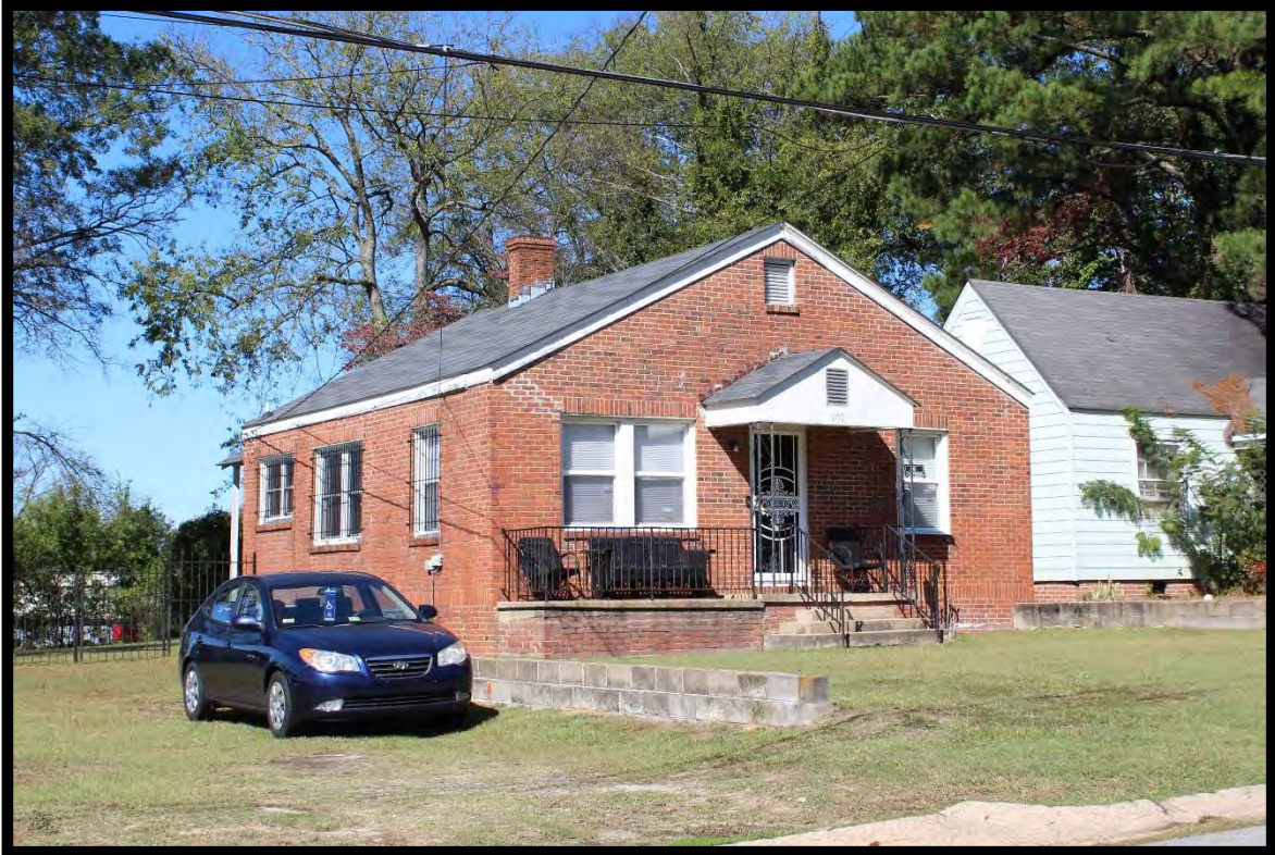
Figure 68: House, 707 North Virginia Street, Looking Northwest.
