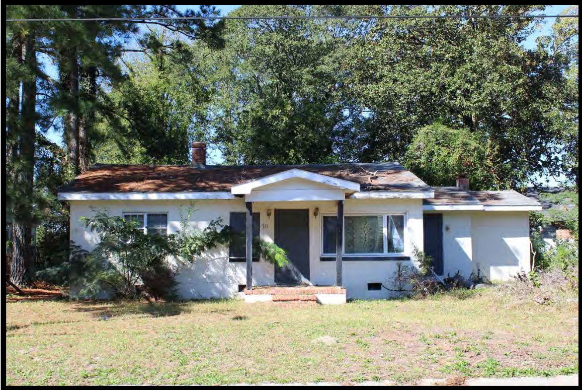
Figure 70: House, 711 North Virginia Street, Looking West.
