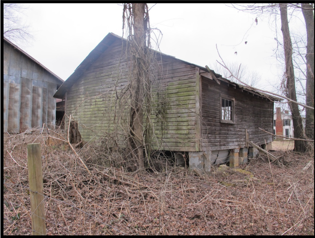
Figure 47: View of Machine Shed, Looking Southeast.
