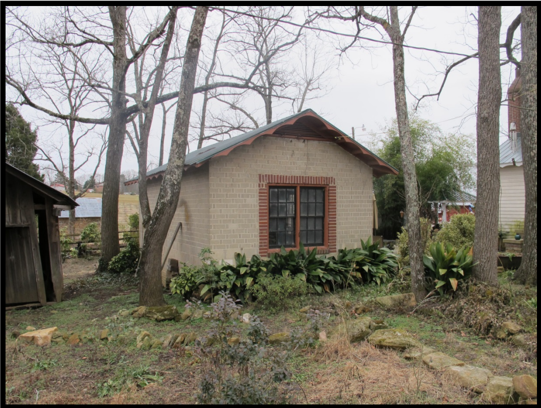
Figure 37: View of Smokehouse/Pantry, Looking South.
