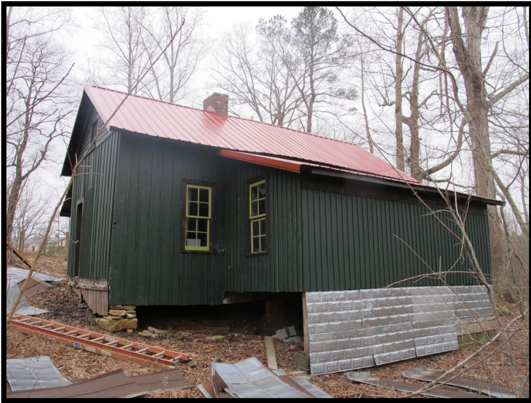
Figure 49: View of Tenant House, Looking South.
