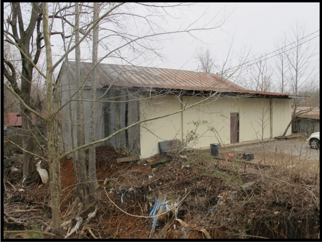
Figure 12: View of Pallet Workshop (No. 3), Looking Southwest.
