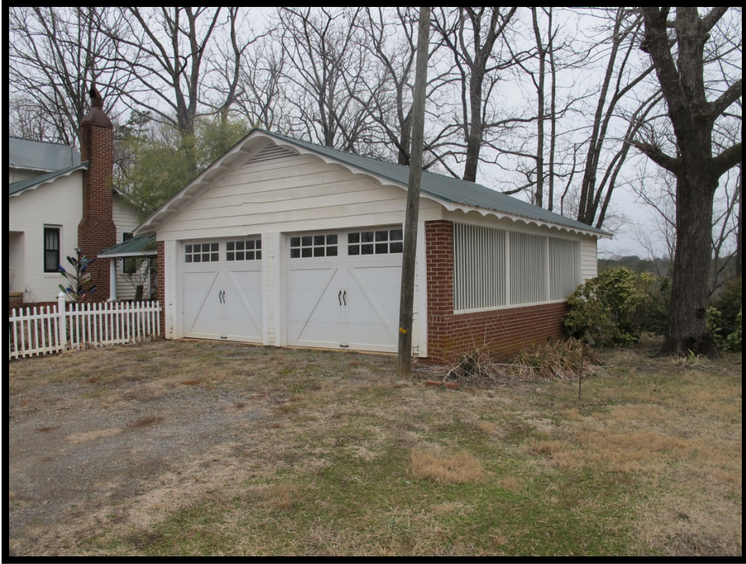
Figure 54: View of Garage, Looking Northeast.
