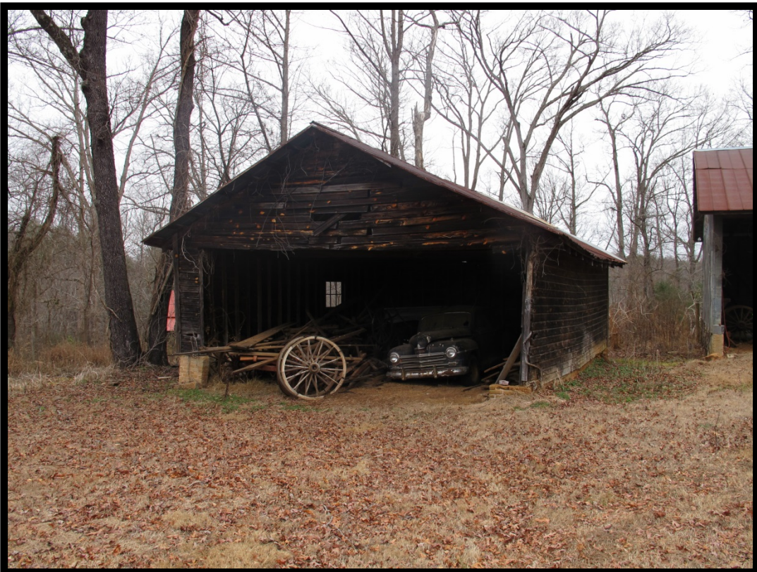
Figure 46: View of Machine Shed, Looking Northwest.
