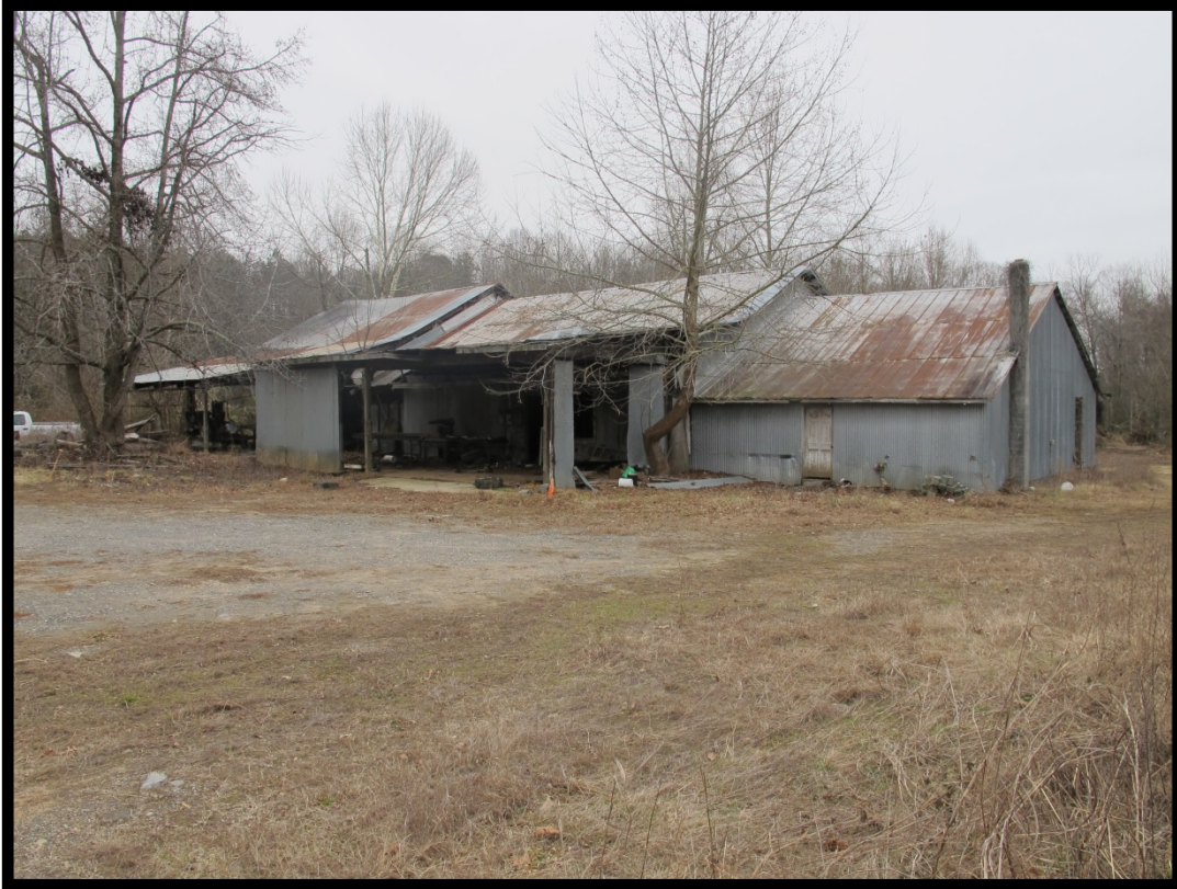
Figure 6: View of Workshops & Saw Mill (No. 1 – ca. 1903), Looking Southeast.
