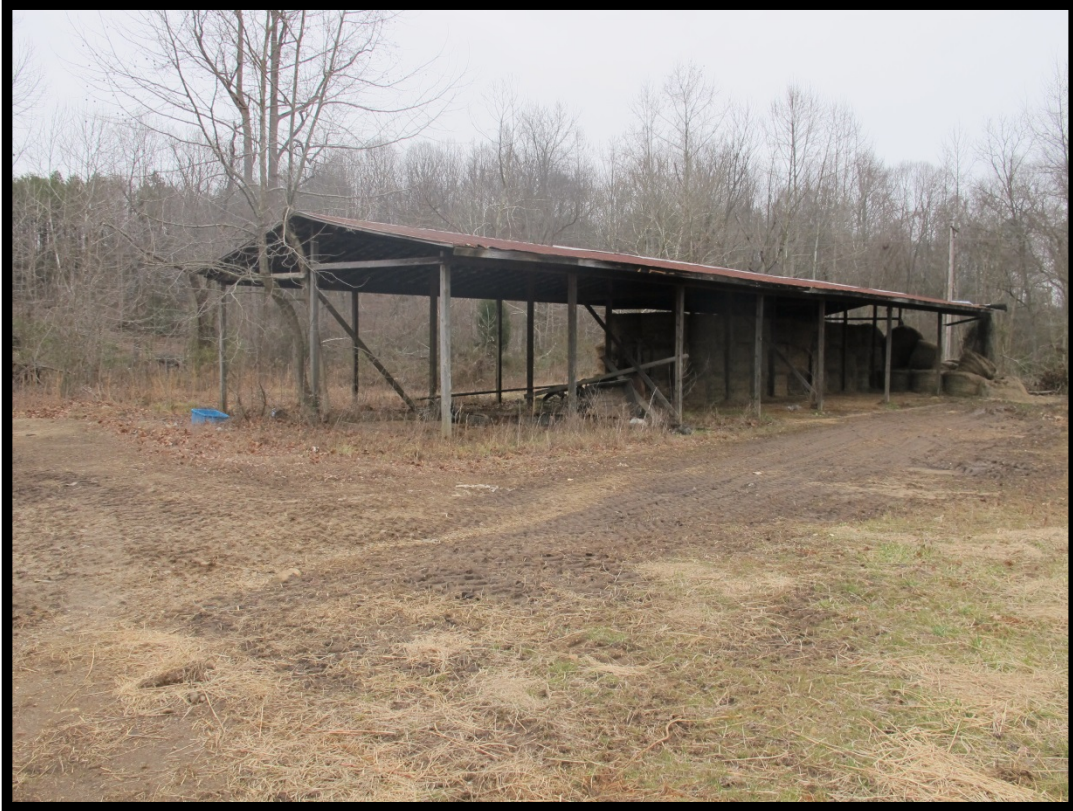
Figure 20: View of Drying Shed (No. 8) Looking Southeast.
