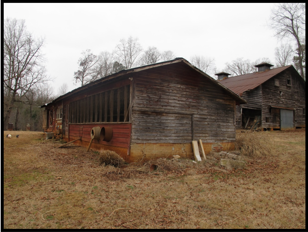
Figure 40: View of Poultry Barn, Looking Northwest.
