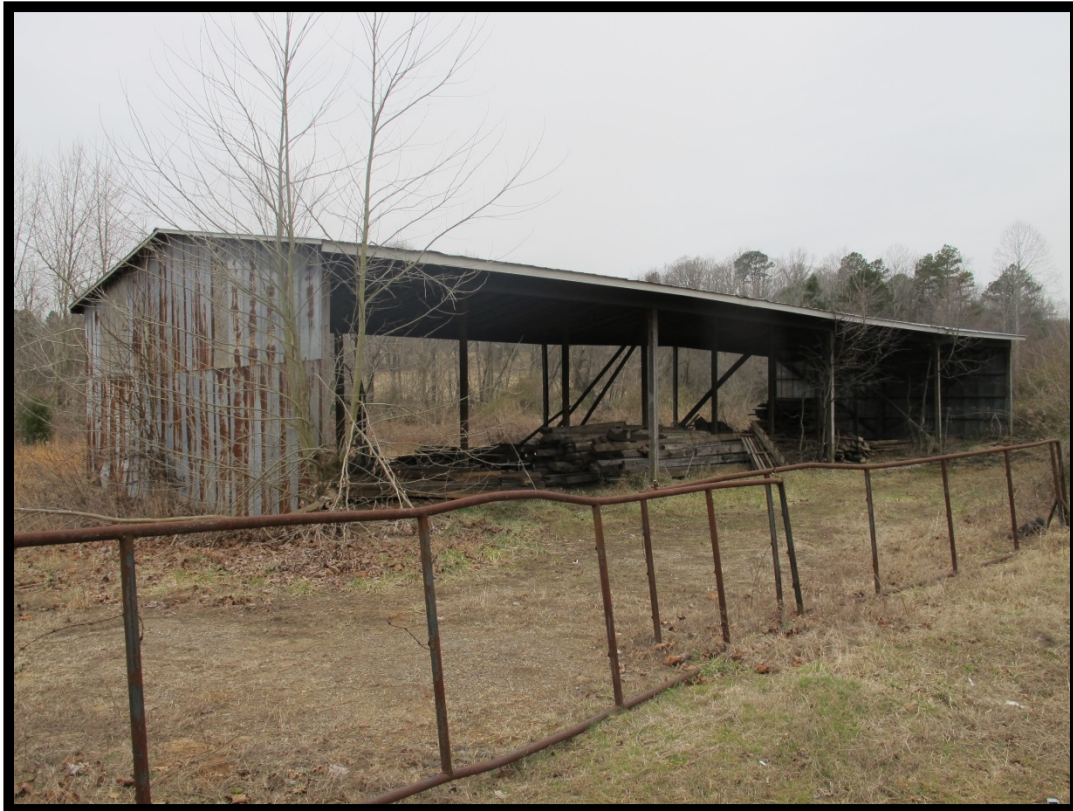
Figure 21: View of Drying Shed (No. 11), Looking Southwest.
