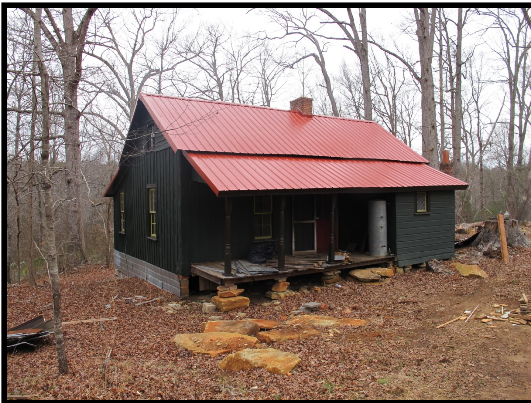
Figure 48: View of Tenant House, Looking North.
