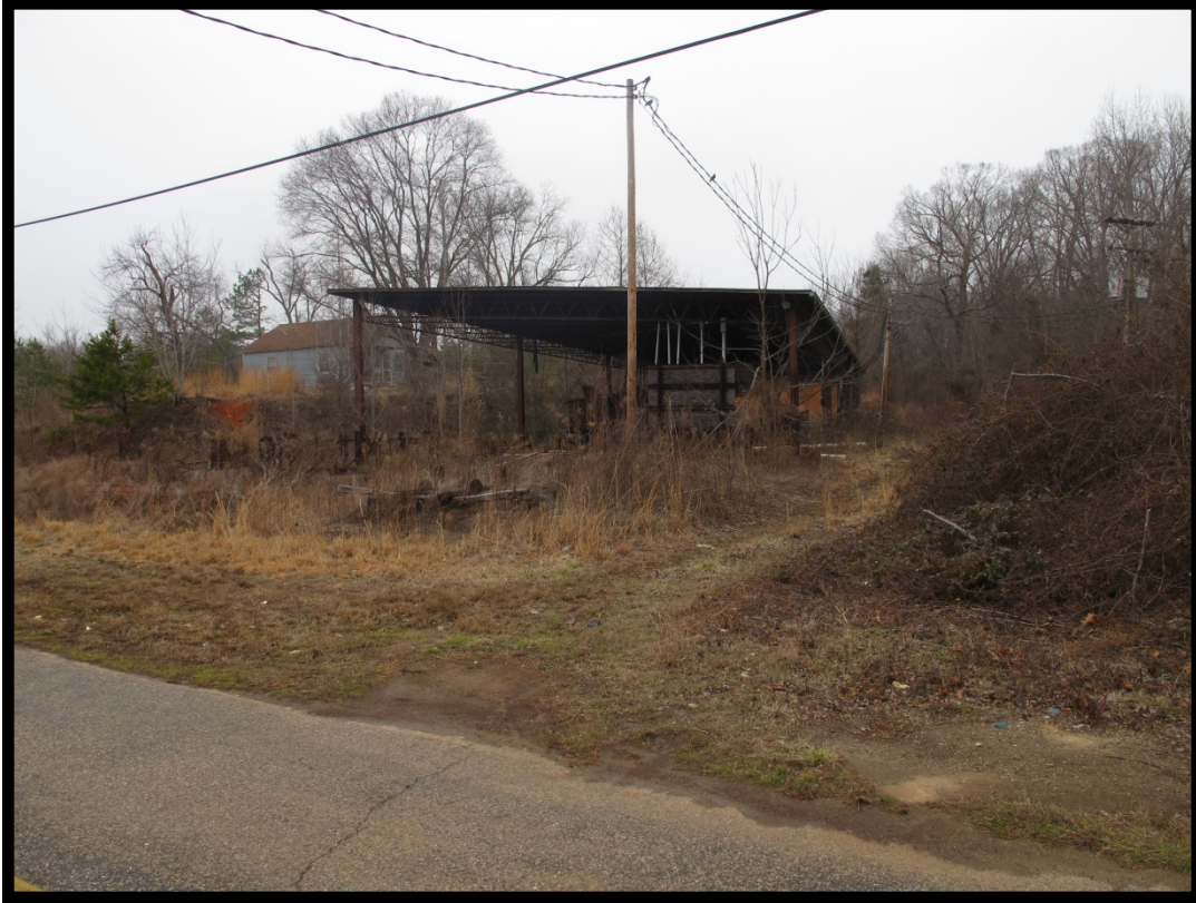
Figure 24: View Workshop (No. 12) and Dwelling (No. 13), Looking Northwest.
