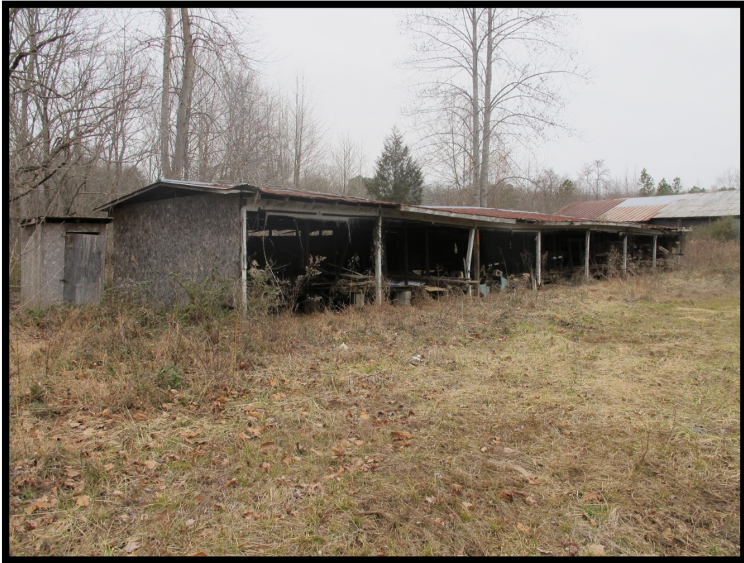
Figure 14: View of Wood Storage Shed (No. 6), Looking Northwest.
