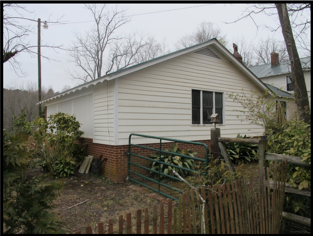
Figure 55: View of Garage, Looking Northwest.
