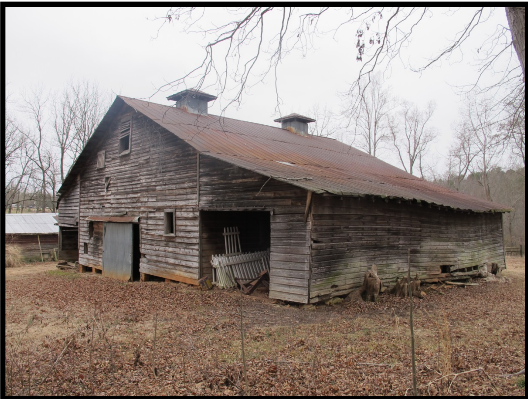
Figure 42: View of Granary, Looking Southwest.
