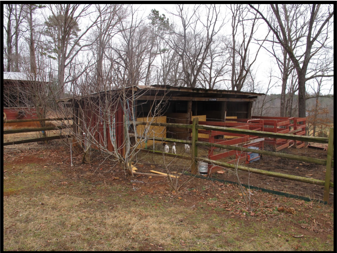
Figure 57: View of Animal Shelter, Looking Northeast.
