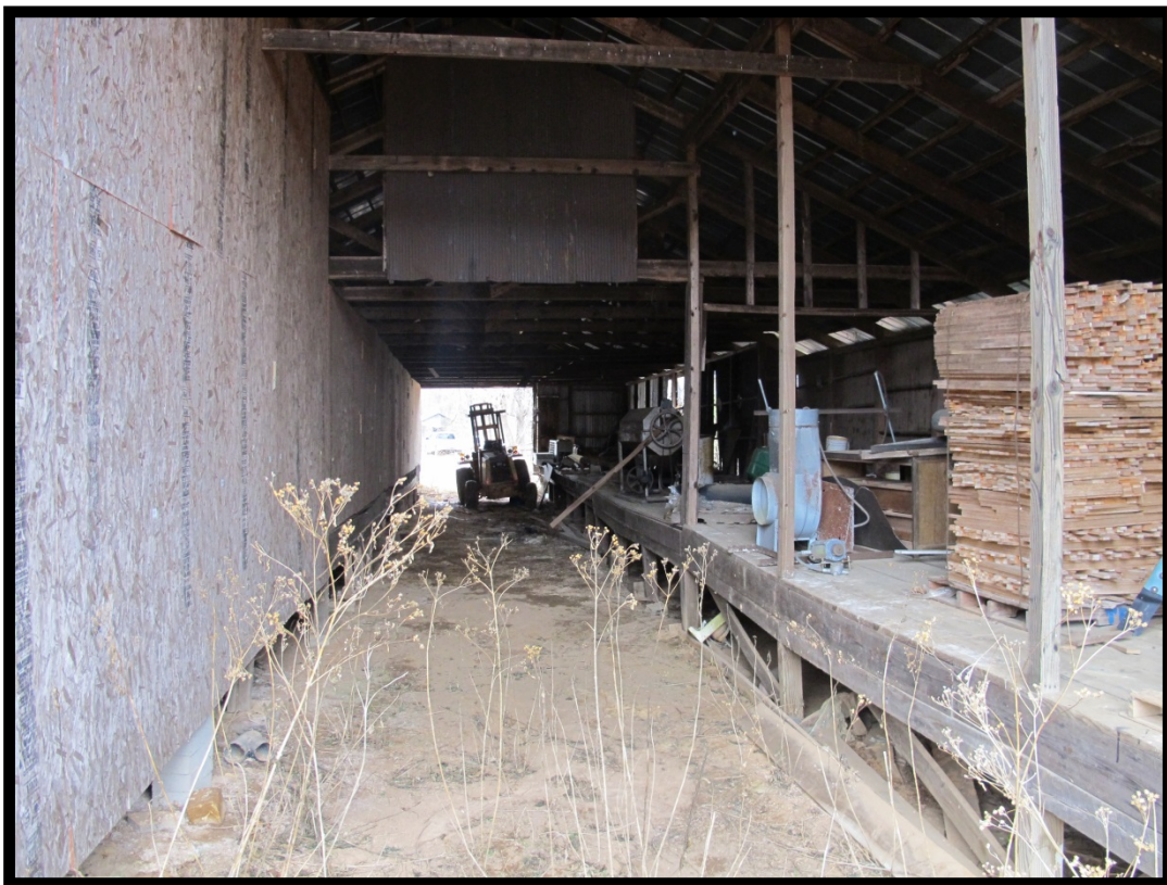
Figure 17: Interior of Storage Shed (No. 9), Looking East.
