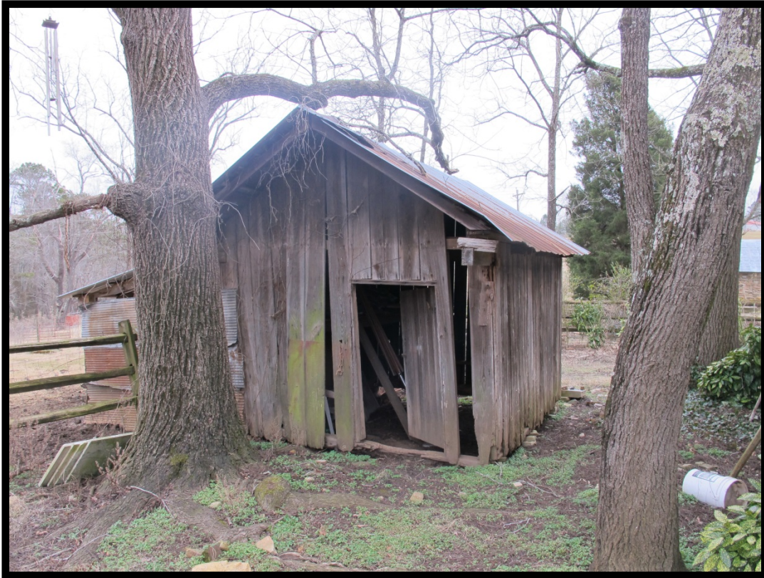
Figure 38: View of Shed, Looking Southeast.
