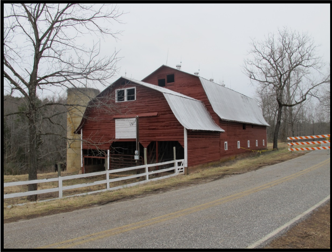
Figure 51: View of Horse/Dairy Barn, Looking Northwest.
