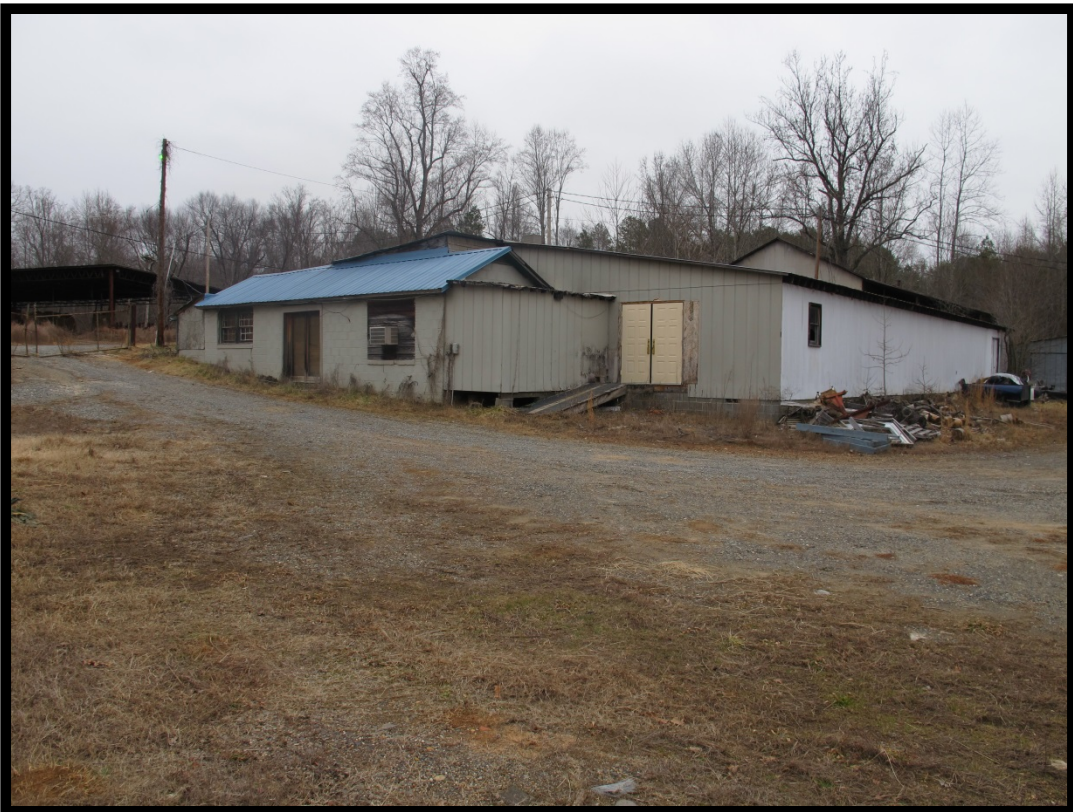
Figure 11: View of Office and Cabinet Shop (No. 2), Looking Northeast.
