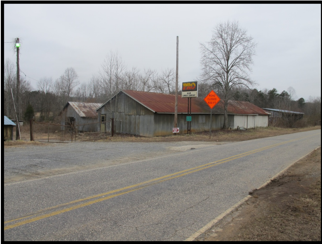
Figure 18: View of Storage Shed (No. 10), Looking Southwest.
