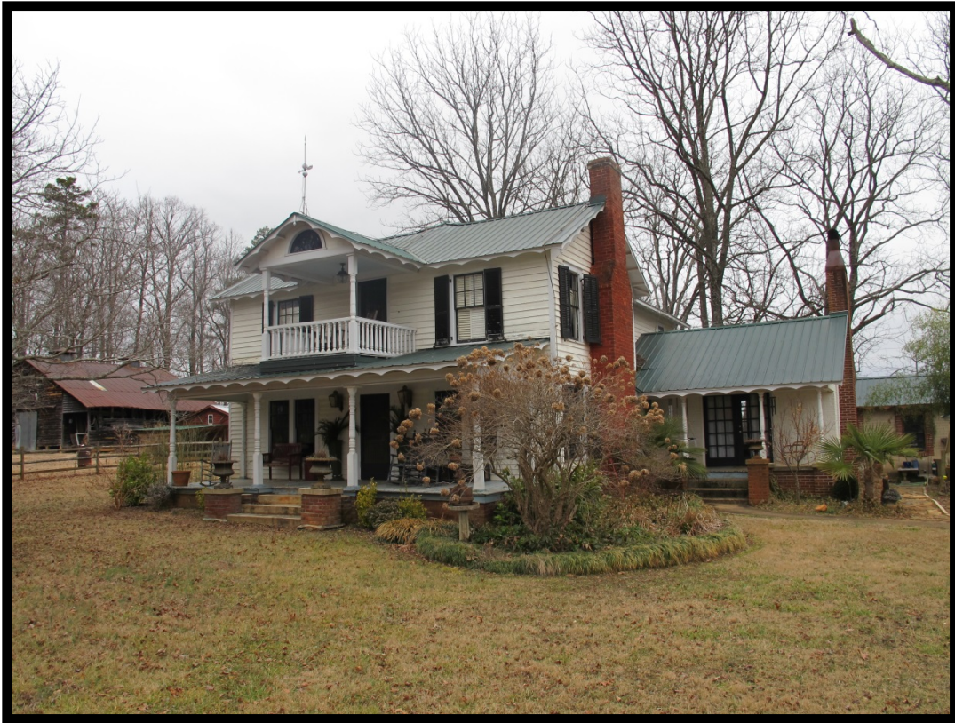
Figure 30: View the Beam House (ca. 1870), Looking Northeast.
