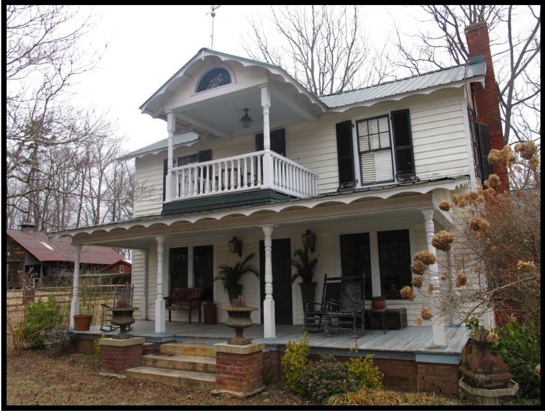
Figure 32: Detail of Porch on Beam House, Looking Northeast.
