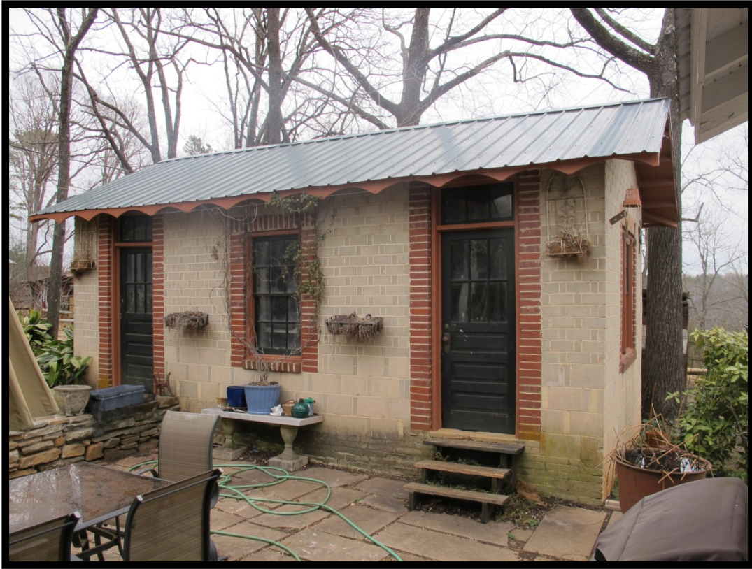
Figure 36: View of Smokehouse/Pantry, Looking Northeast.
