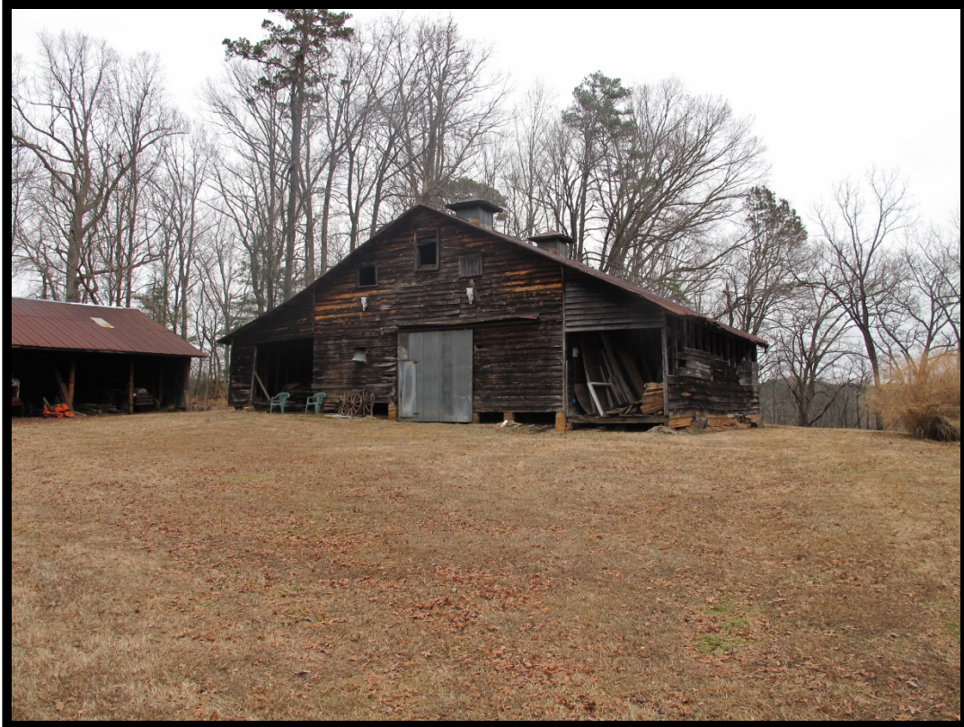
Figure 41: View of Granary, Looking Northeast.
