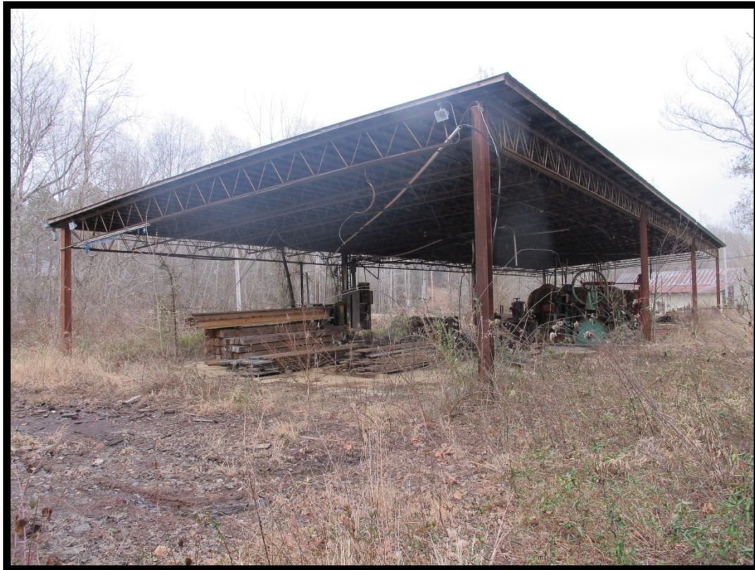
Figure 25: View of Workshop (No. 12), Looking Southeast.
