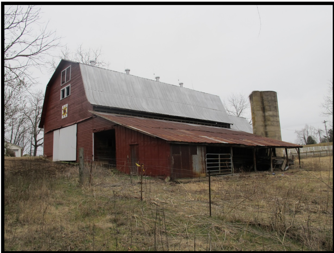
Figure 50: View of Horse/Dairy Barn, Looking Southeast.
