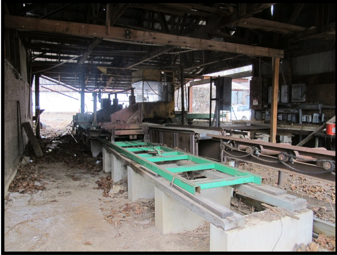
Figure 8: View of Saw Mill.
