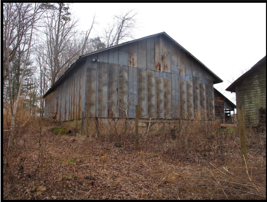
Figure 45: View of Machine Shed, Looking Southeast.
