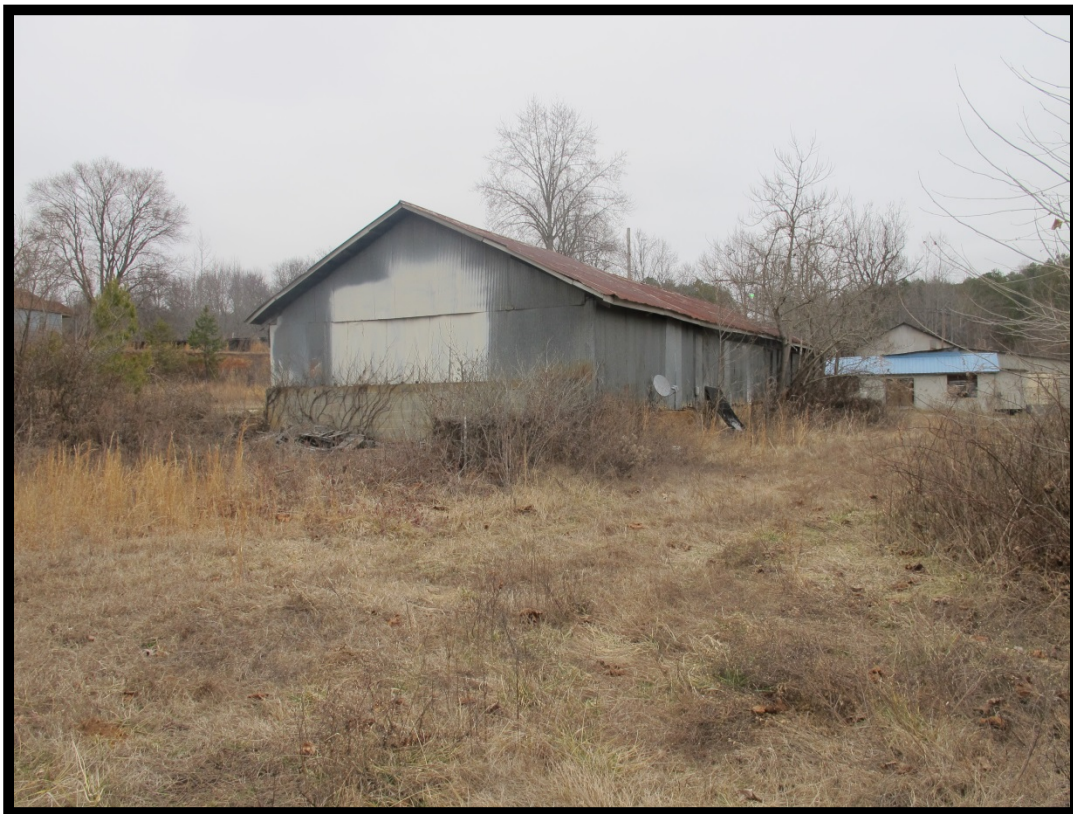
Figure 19: View of Storage Shed (No. 10), Looking Northeast.
