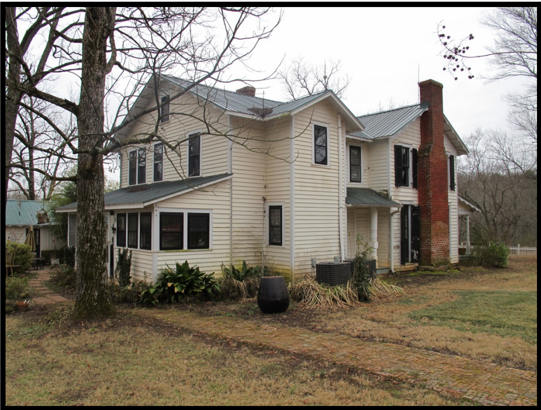
Figure 31: View the Beam House (ca. 1870), Looking Southwest.
