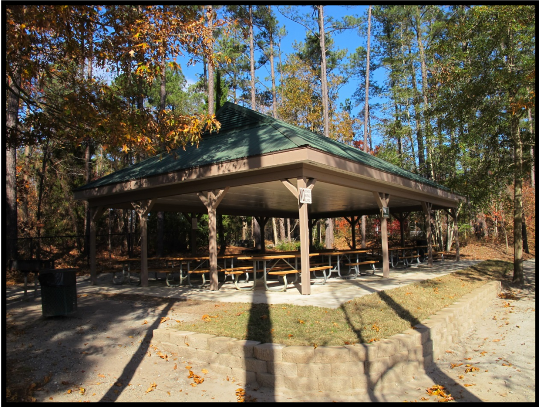
Figure 22: View of Picnic Shelter (2000) Located Southwest of Visitor's Center, Looking Northwest.
