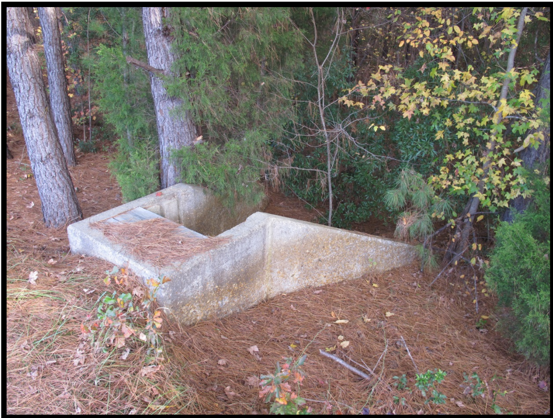
Figure 13: View of Concrete Outlet (1930s) of Abandoned Rearing Pond (ca. 1924).
