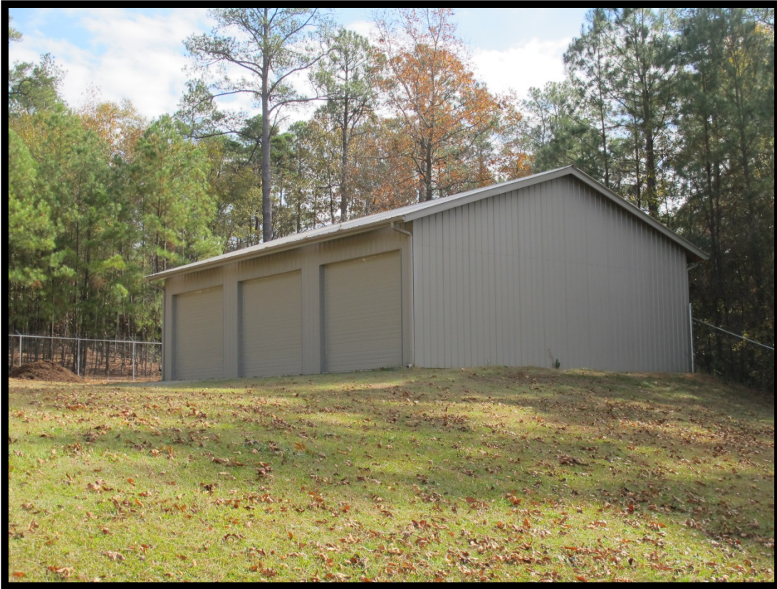
Figure 16: View of the Maintenance Building (ca. 2008) Southeast of the Education Center, Looking Southeast.
