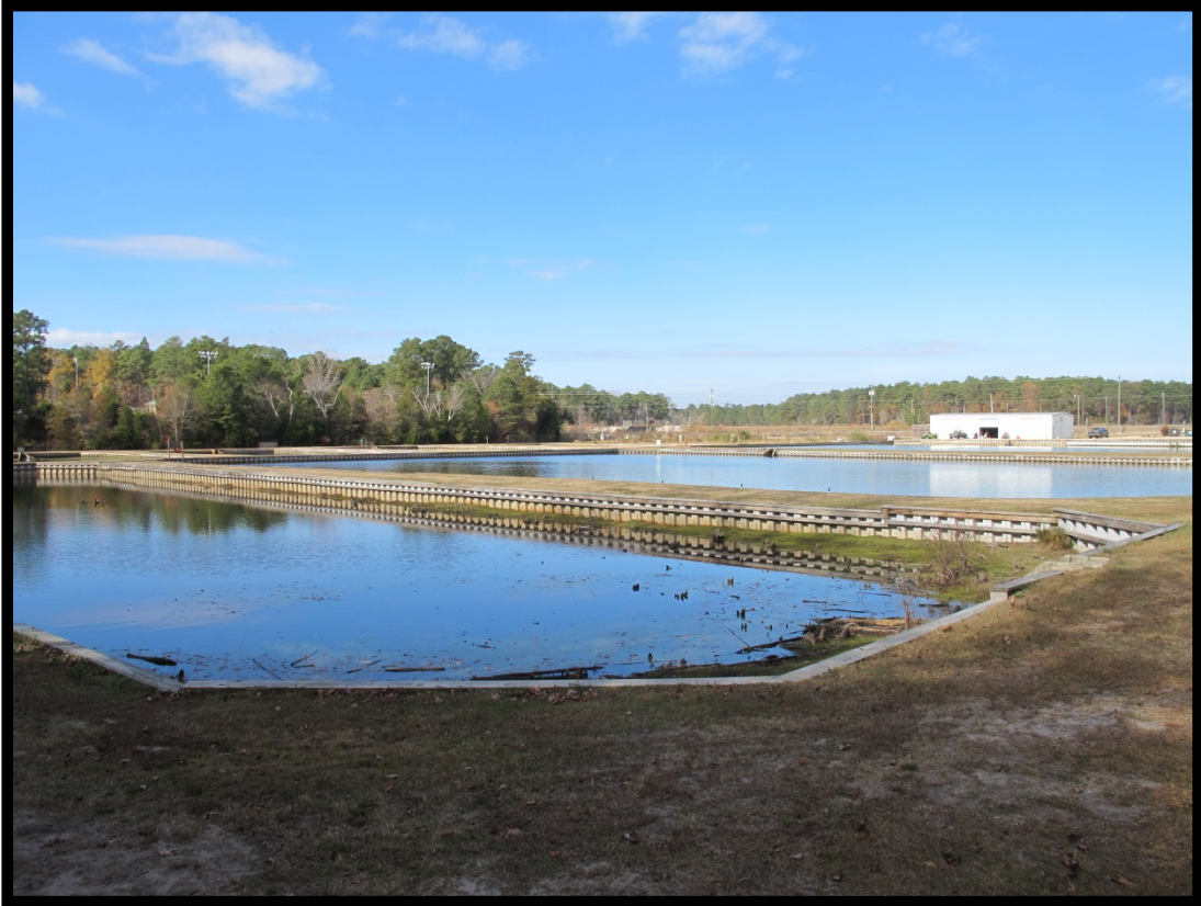
Figure 11: View of the Rearing Ponds (ca. 1924), Looking Northwest Towards the Second Maintenance Building.
