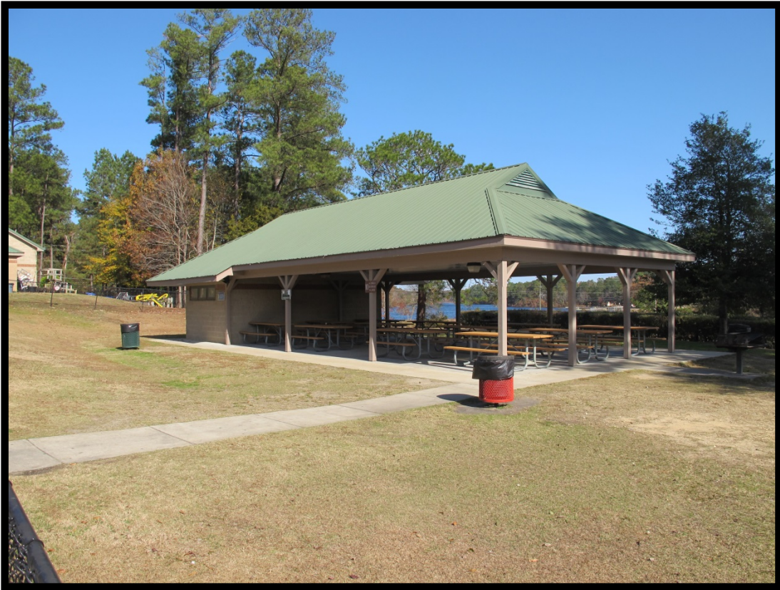
Figure 24: View of Picnic Shelter and Civil Works Administration Pavilion (2000), Looking Northeast.
