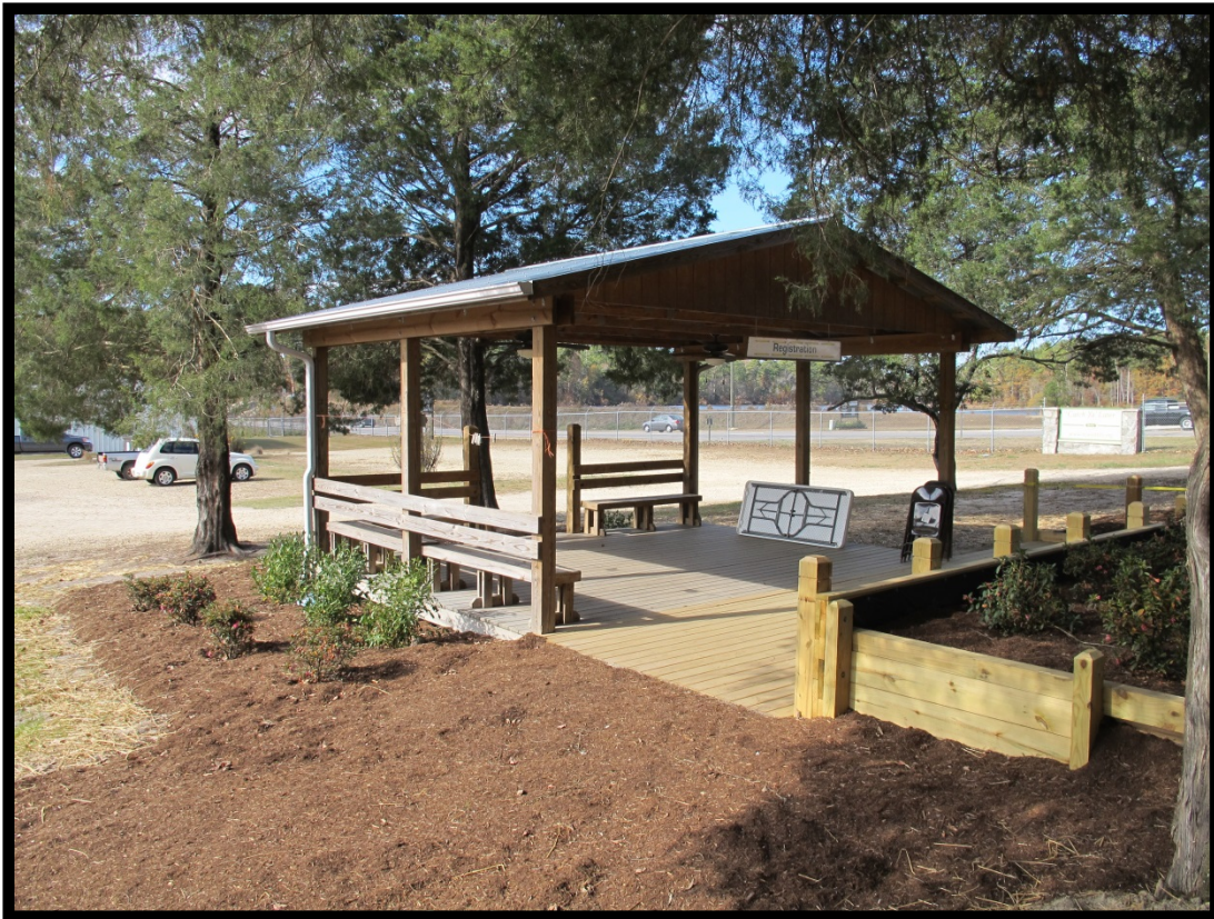
Figure 18: View of the Registration Shelter (ca. 2007), Looking Northwest.
