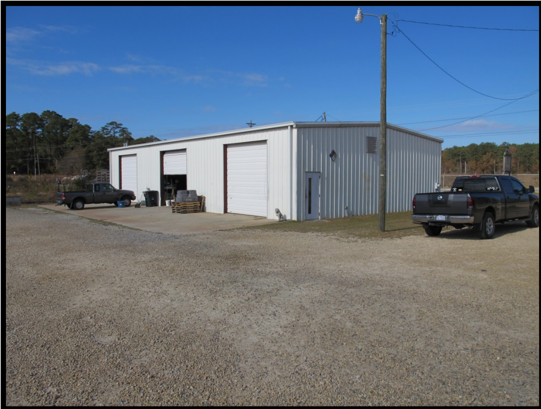
Figure 17: View of the Maintenance Building (1980s) at the Rearing Ponds, Looking Northwest.
