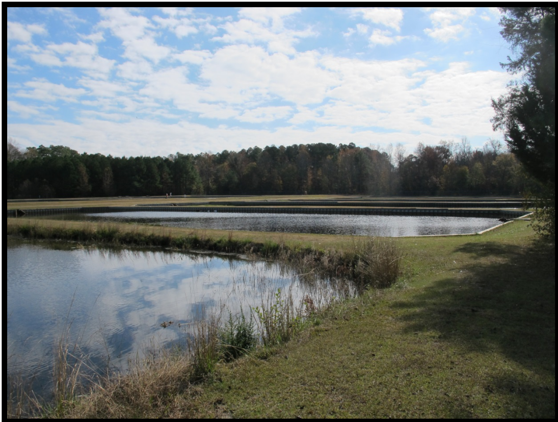
Figure 10: View of the Rearing Ponds (ca. 1924) near the North End of the Spillway, Looking Southeast.
