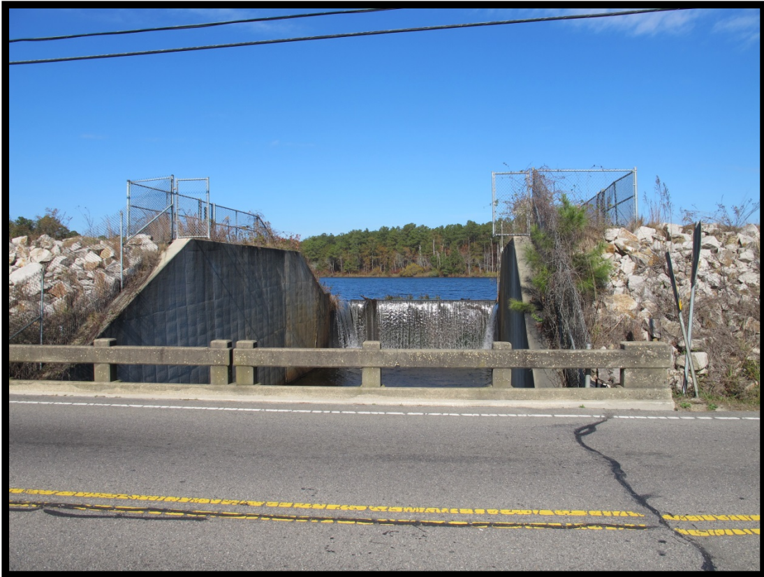
Figure 6: View of the Spillway and Lake Rim from Bridge No. 14 (ca. 1922 & 1938) on Raeford Road, Looking North.
