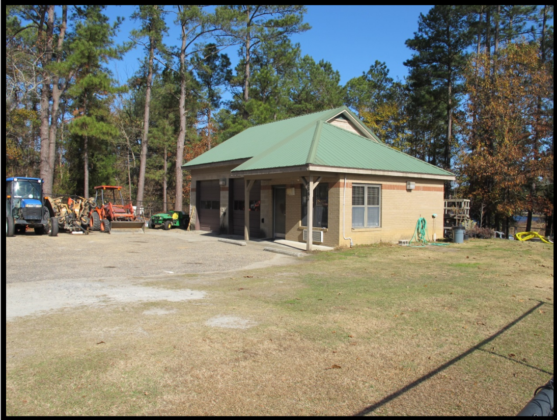
Figure 25: View of Maintenance Building (2000), Looking Northeast.
