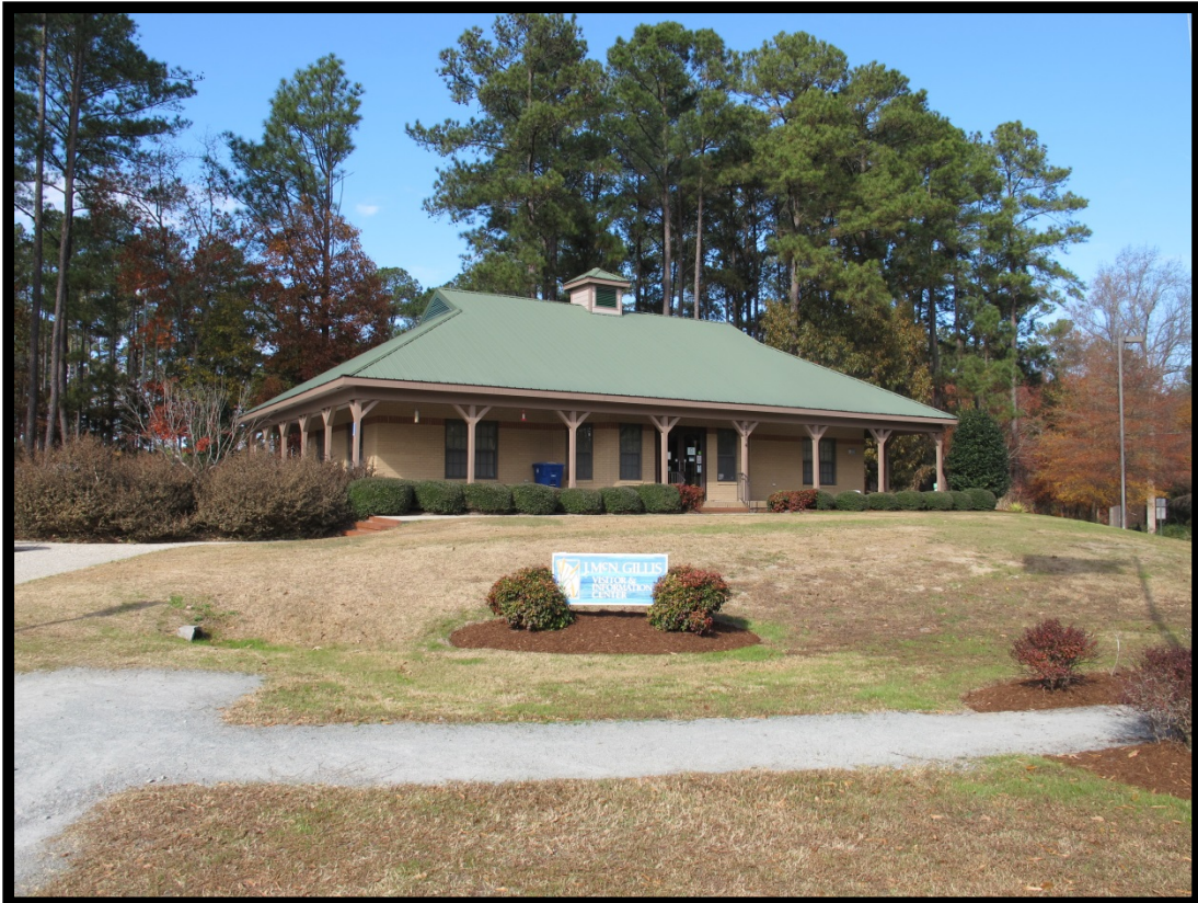
Figure 21: View of the J. McN. Gillis Visitor & Information Center (2000) at Lake Rim Park, Looking Northwest.
