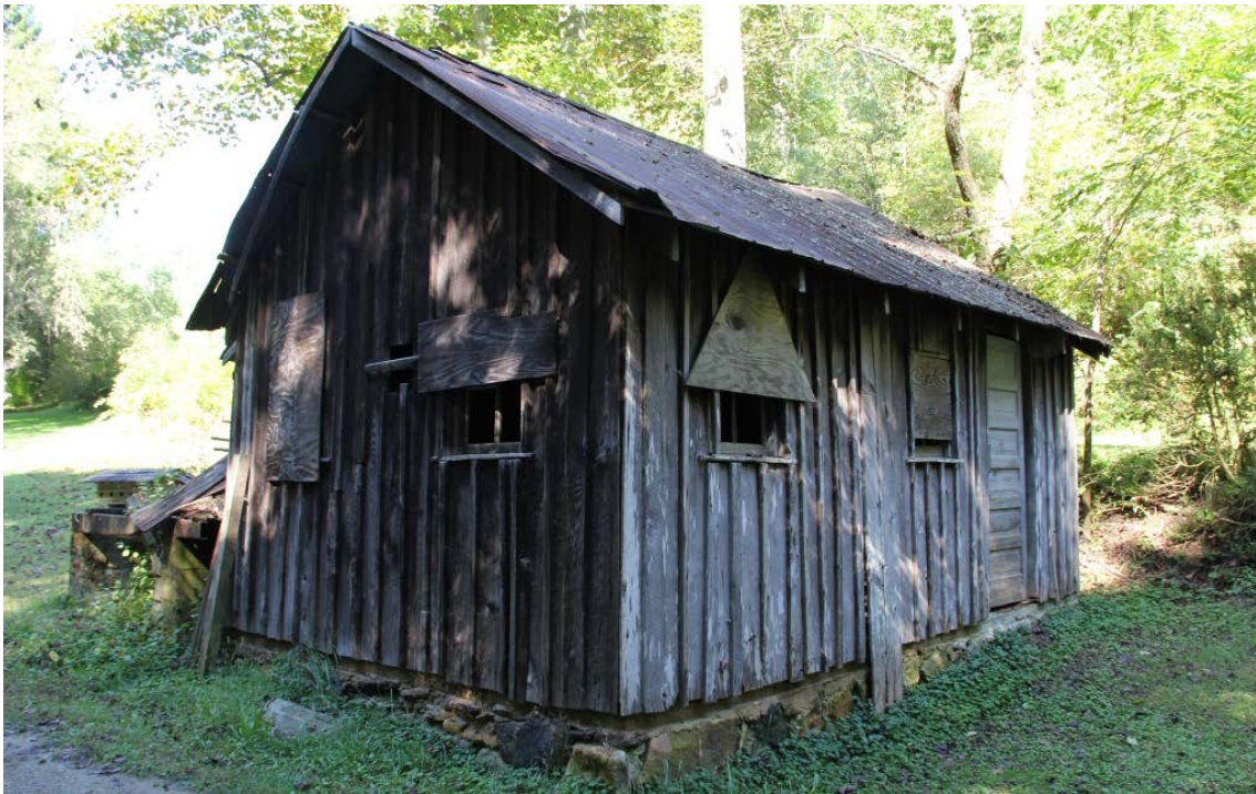
Storage shed, overall front view to southwest from Bearwallow Mountain Road
