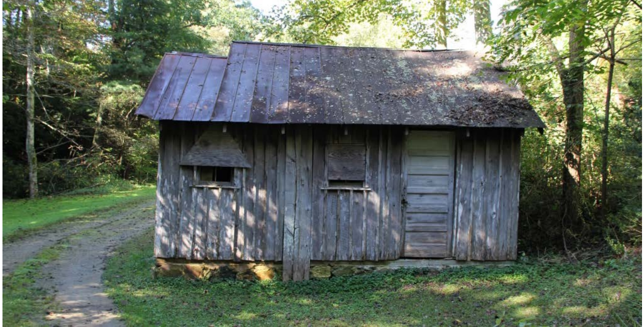
Storage shed, overall front view to southwest from Bearwallow Mountain Road
