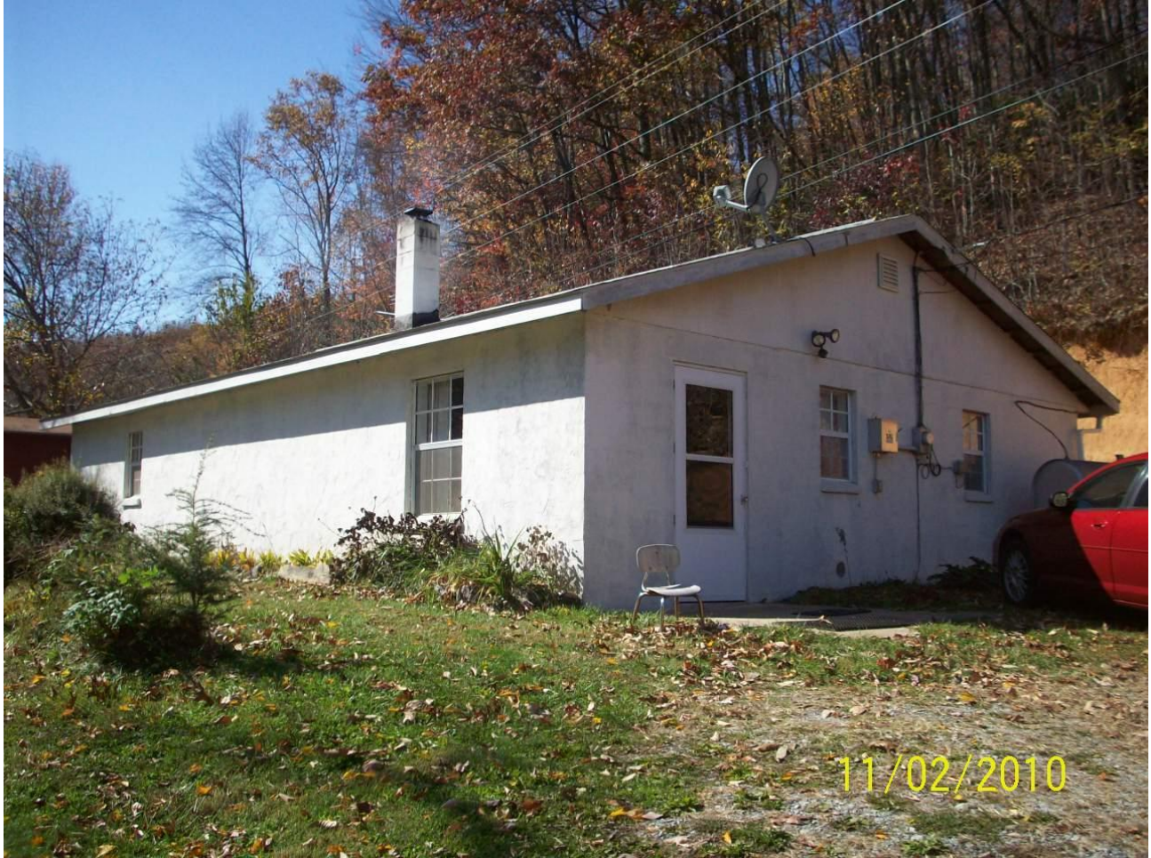
House, 6713 Bearwallow Mountain Road, oblique front view to west
