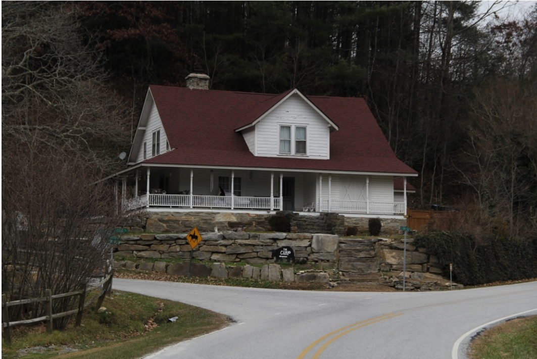
William Huntley House (HN 1179), 1444 Middle Fork Road, view to northeast
