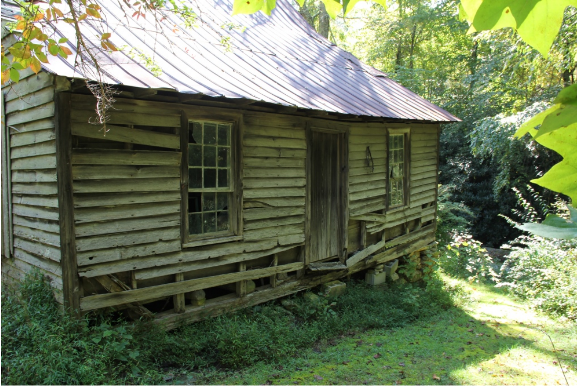
Riley Wall House, oblique rear view to southeast
