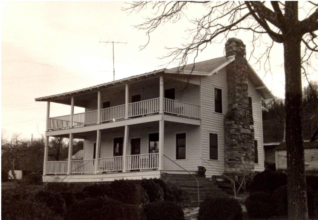
Lyda House at Bee Hive Inn (HN 1092), 417 Beehive Road, view to south, photographs by Michael Ann Williams, 1980, from collection of NC HPO
