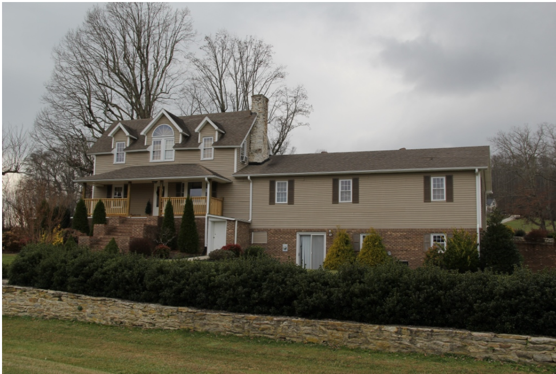
Zeb Dalton House (HN 1124), 3045 Old Clear Creek Road, view to northwest
