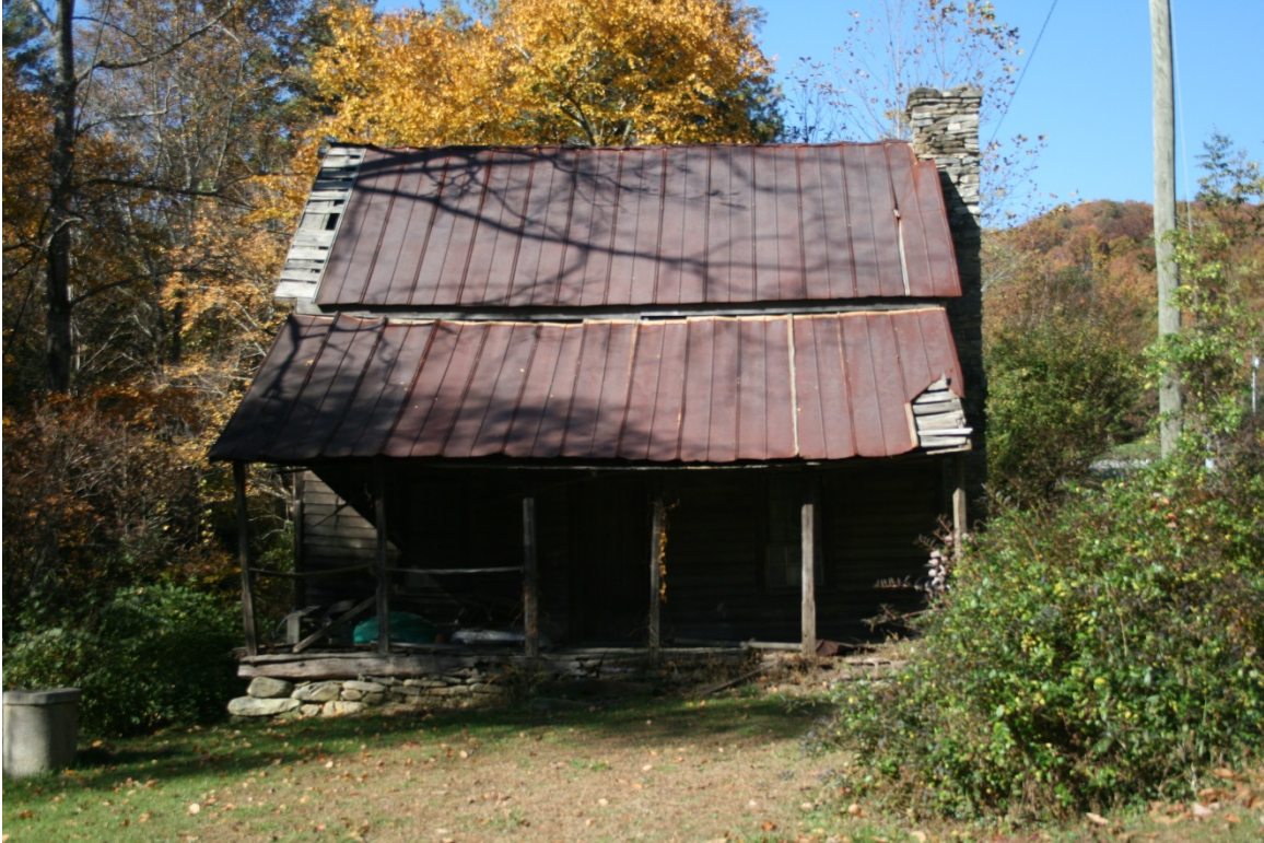
Riley Wall House (HN 1274), façade, view to west
