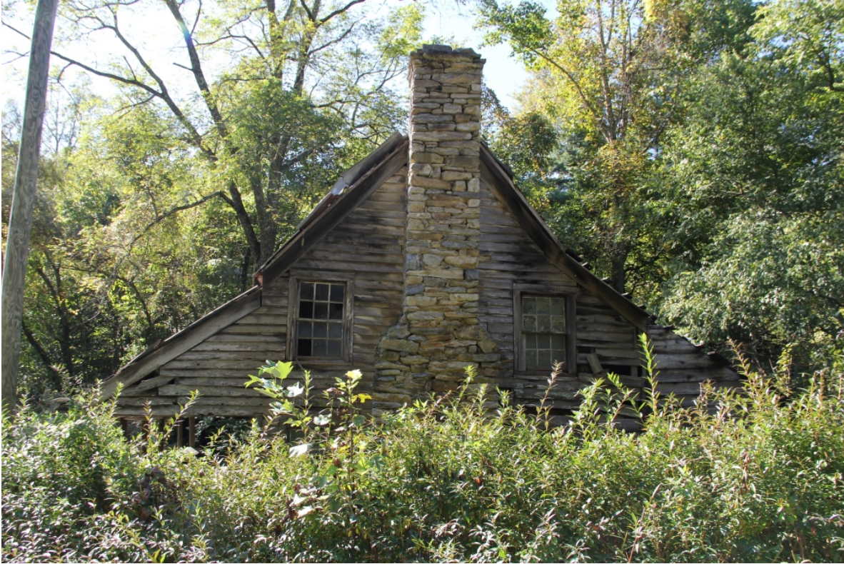
Riley Wall House, north elevation, view to south
