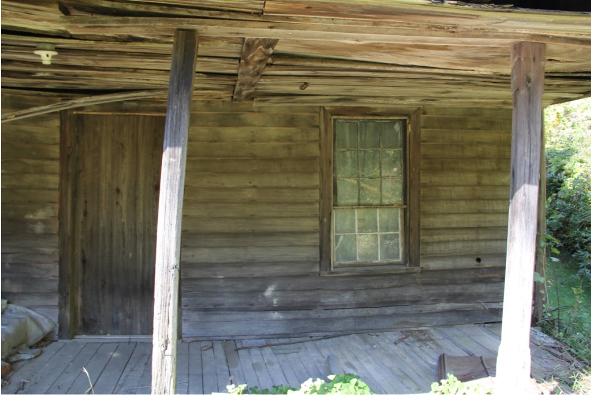
Riley Wall House, porch detail, view to west
