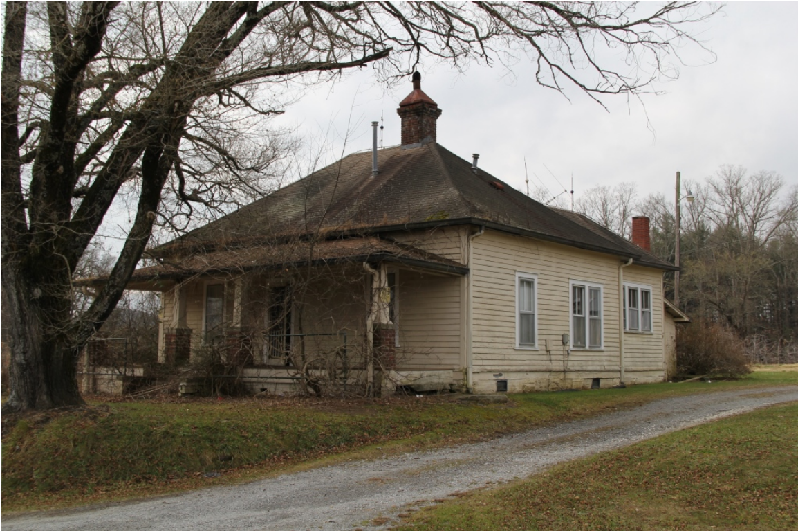
House, 1995 Pace Road, oblique view to southwest
