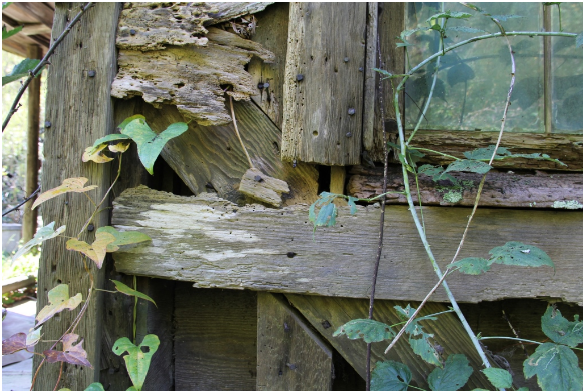
Riley Wall House, framing detail at northeast corner, view to south
