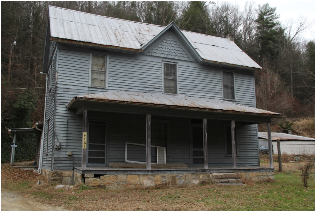
G. W. Freeman House (HN 1148), 4761 Chimney Rock Road, view to northeast
