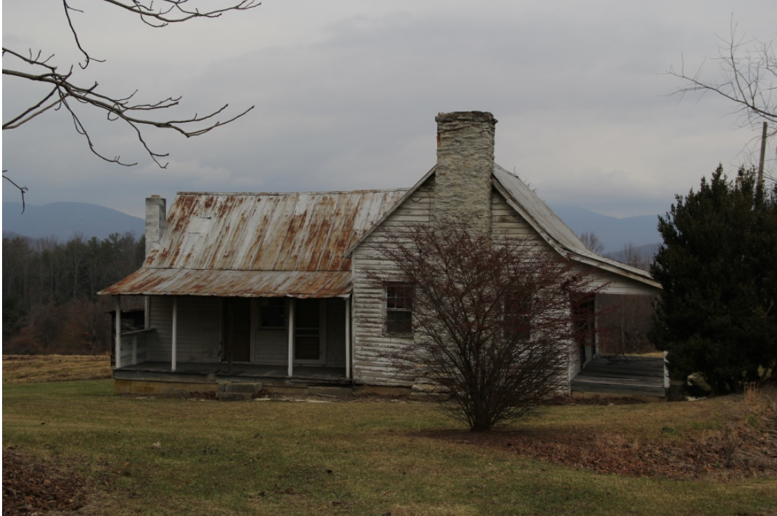
William Jones House (HN 1187), 5603 Sugarloaf Road, oblique view to north
