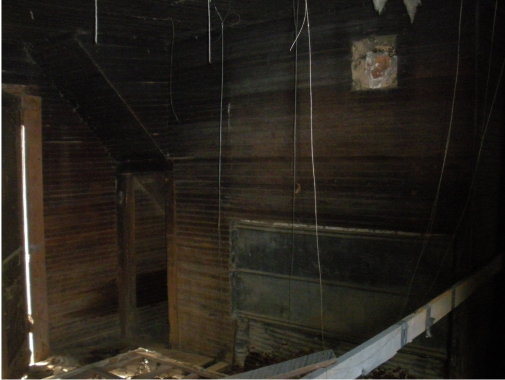
Figure 16. View west within kitchen.
