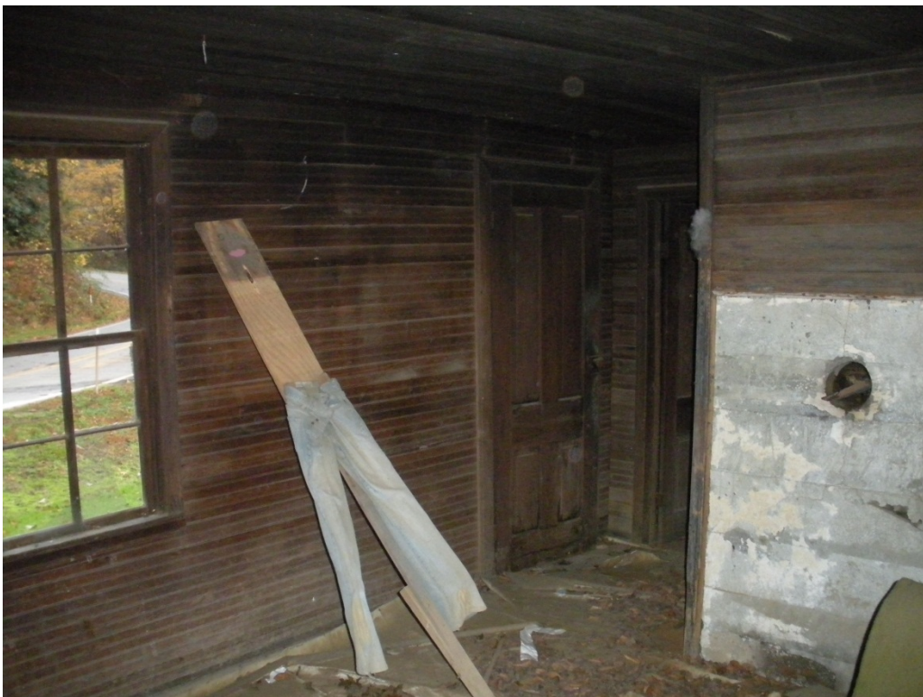
Figure 13. View northwest within main block's south parlor to main entry.
