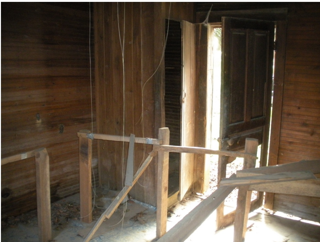
Figure 15. View south within dining room.
