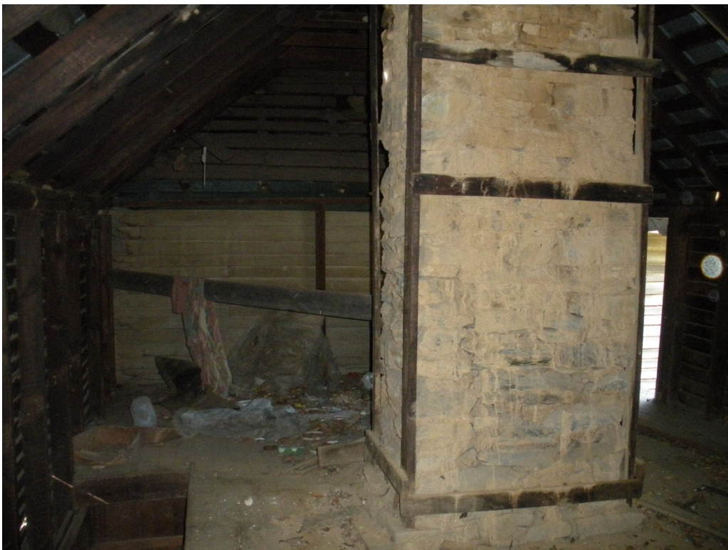
Figure 19. View west within rear ell's bedroom above dining room and kitchen.
