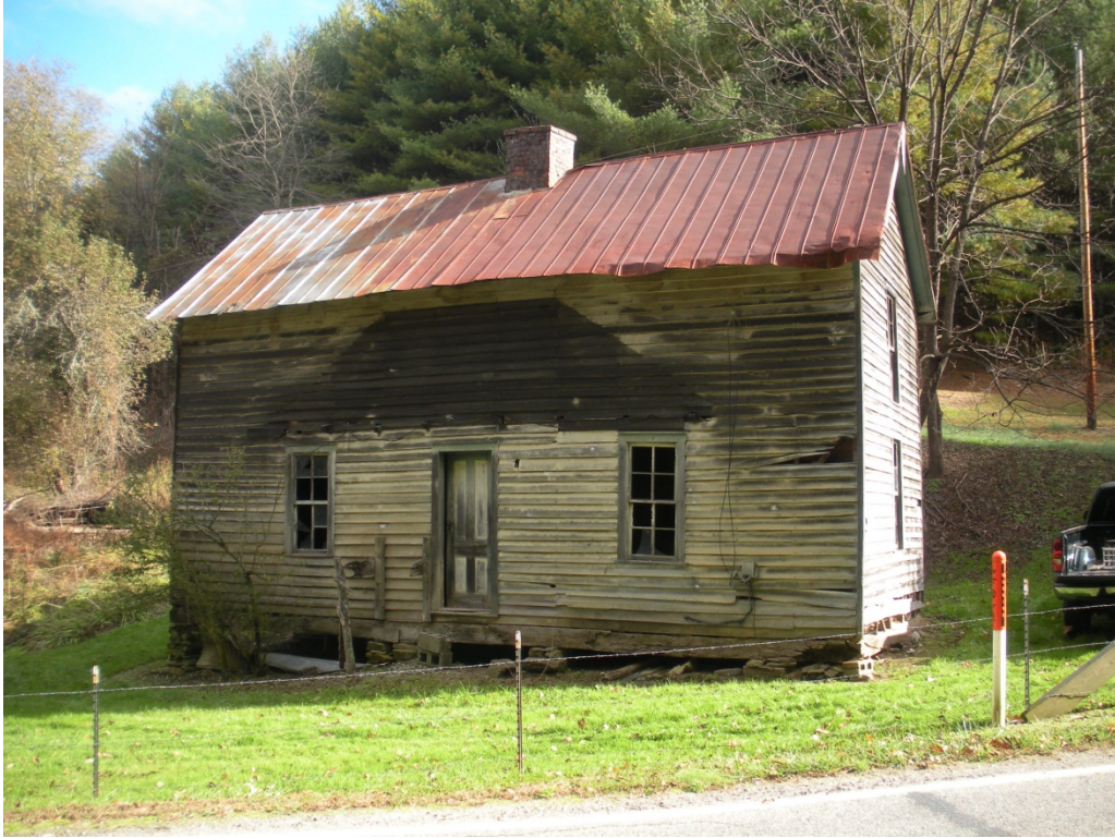
Figure 4. View northeast to west façade.
