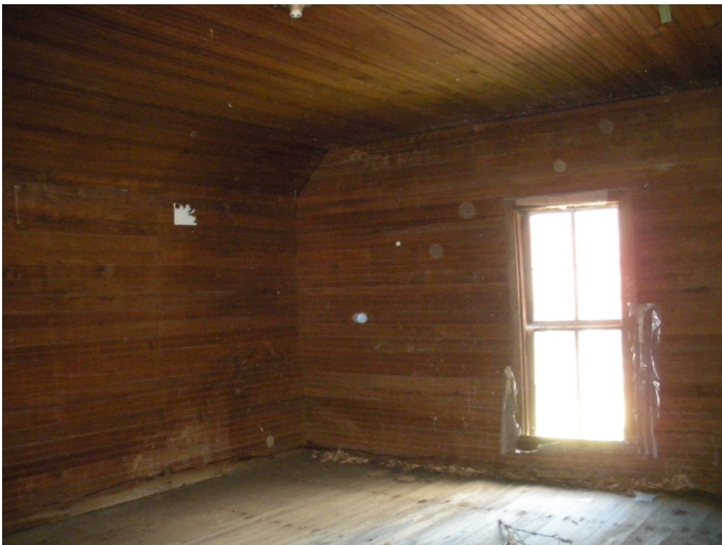
Figure 17. View northwest within bedroom above main block's north hall.
