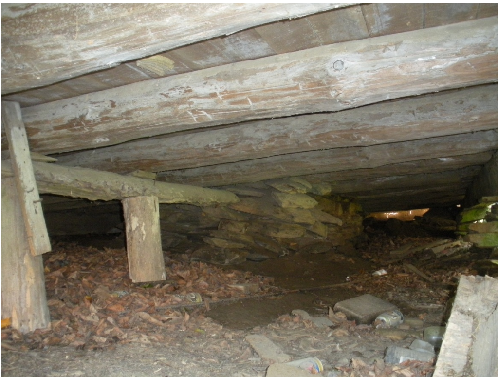
Figure 11. Representative view of main block's log floor joists.
