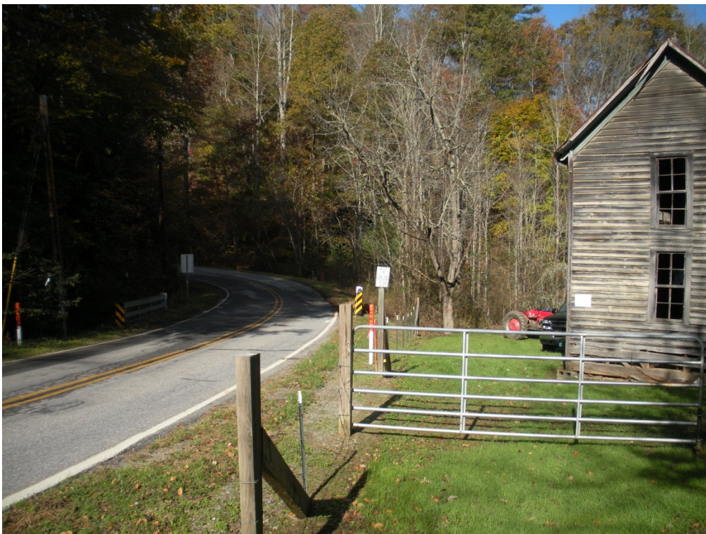
Figure 21. View west along White Oak Rd. to Bridge No. 273 and Teague House.
