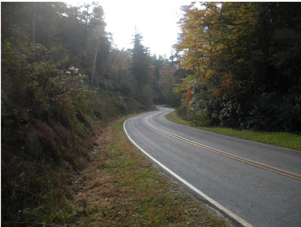
Figure 23. View southeast along White Oak Rd. from just south of Teague House.
