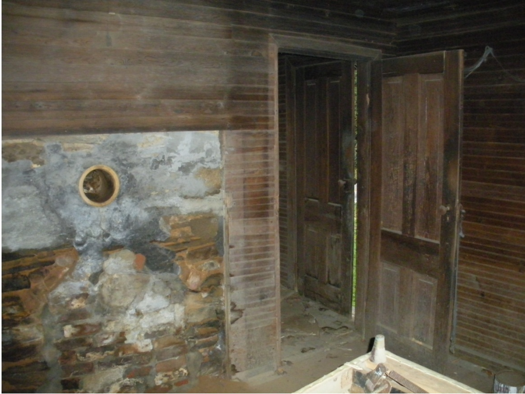
Figure 12. View southwest within main block's north hall to main entry.
