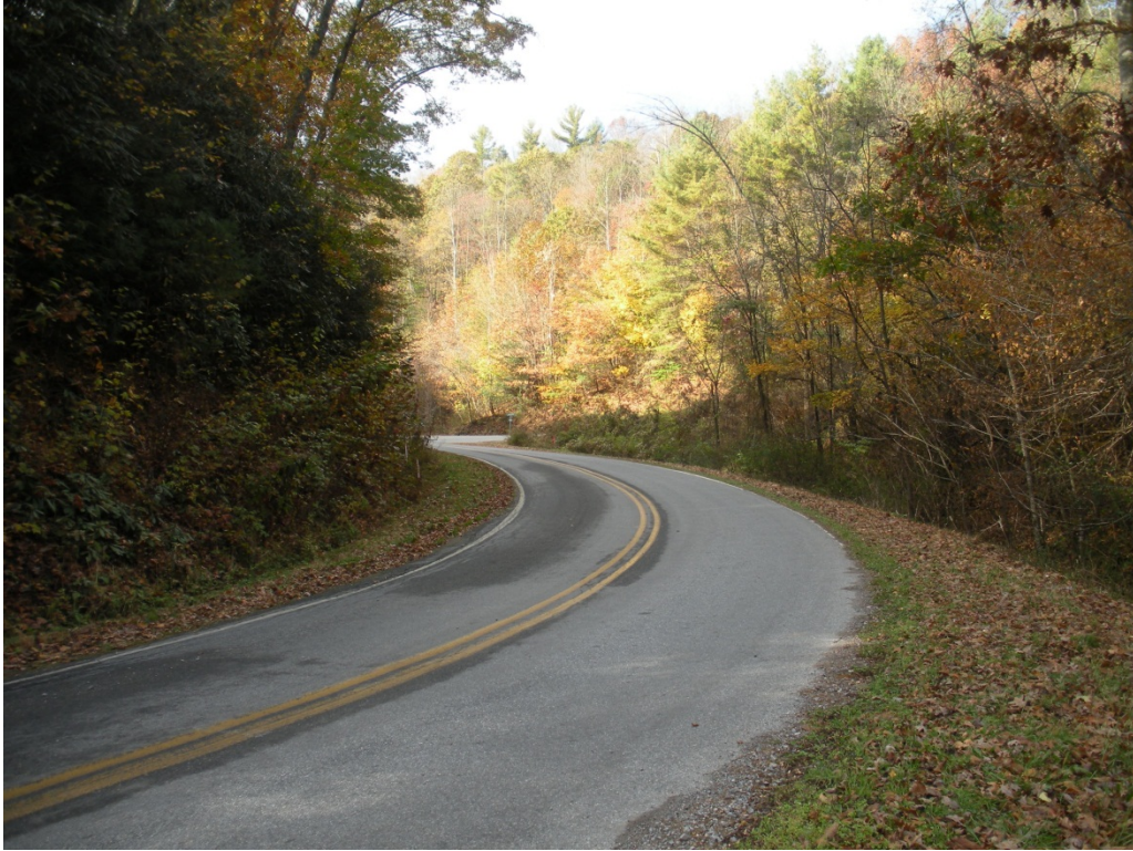
Figure 22. View west along White Oak Rd. from Bridge No. 273.
