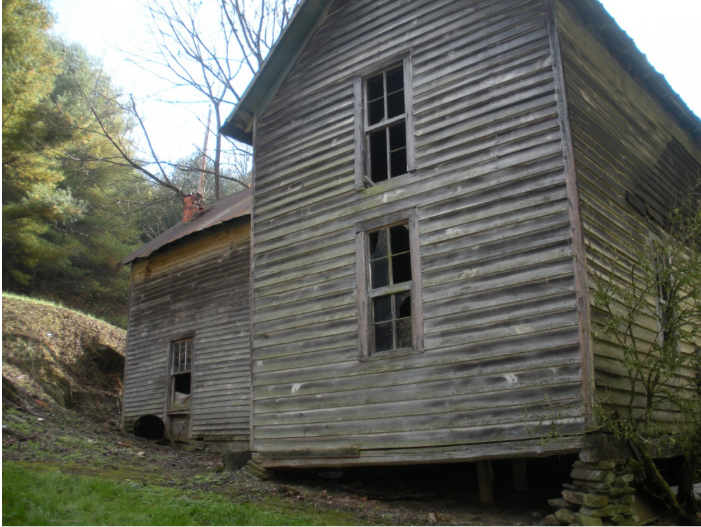
Figure 10. View southeast to north elevation.
