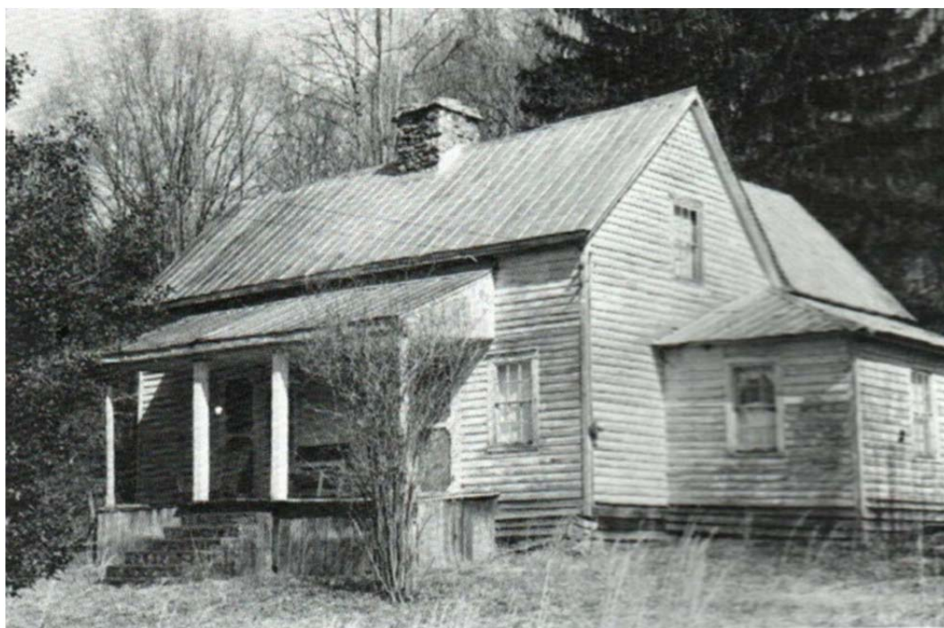
Figure 34. Comparable extant example: Smathers House, Dutch Cove vicinity (Source: Mountain Gables: A History of Haywood County Architecture )
