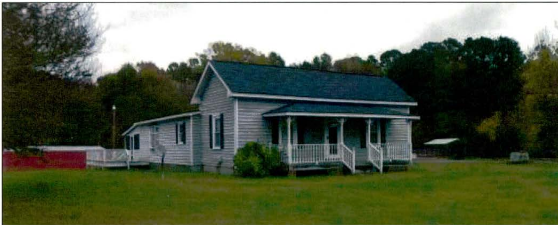
Photo 3: Southwest Oblique of Dwelling at Booth Farm.
