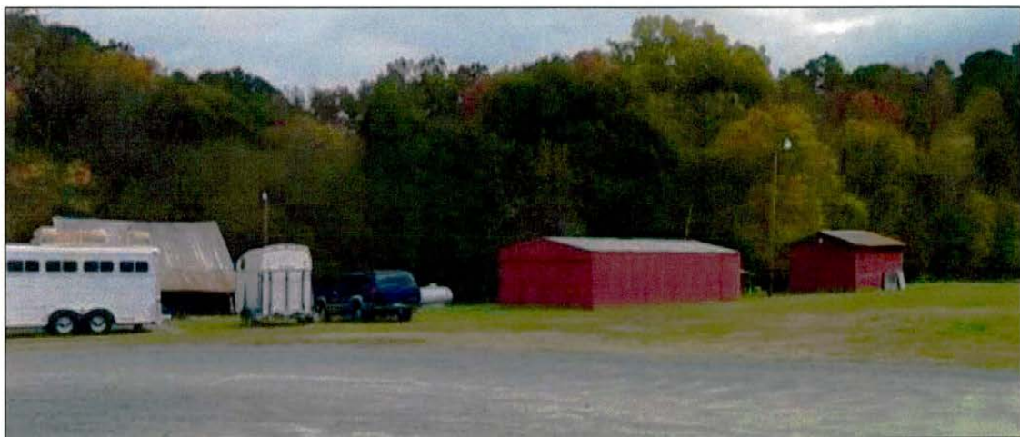
Photo 5: View of Outbuildings Associated with Booth Farm Property Looking Northeast. At right, behind the horse trailers, is a circa-1940s, multi-purpose barn.
