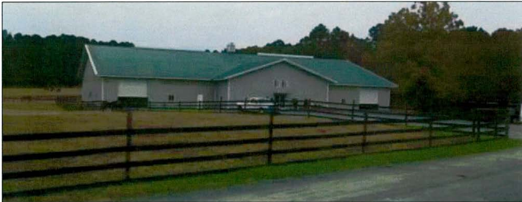
Photo 6: Southeast Oblique of Circa-2003 Equine Facility.
