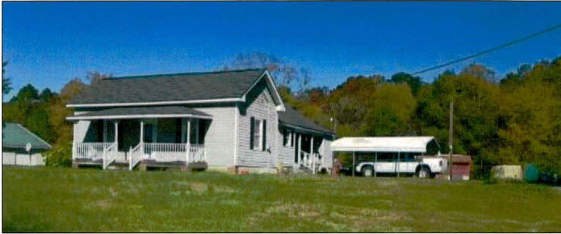
Photo 2: Southeast Oblique of Dwelling at Booth Farm. Well, carport, and outbuildings visible at right and in background.
