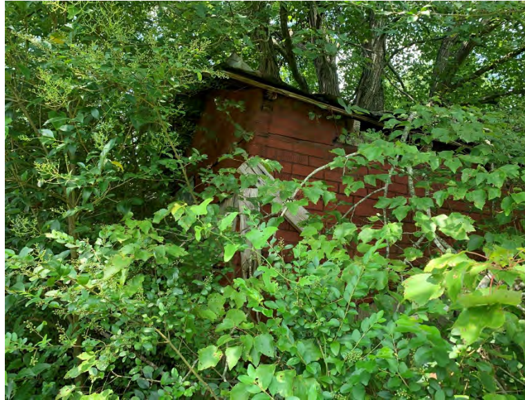
ST0910: looking southeast
