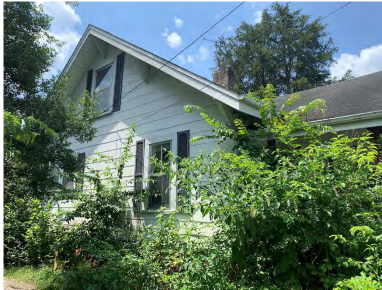
ST0910: looking southeast
