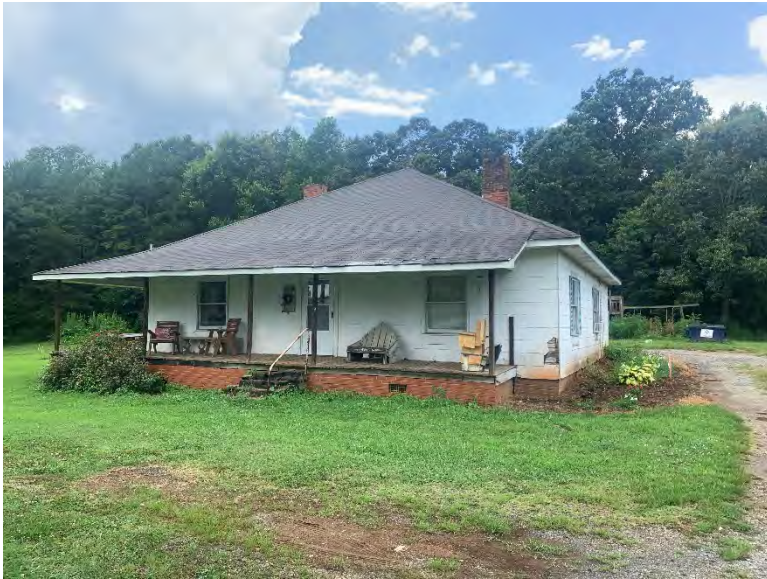
UN1223: façade (southeast elevation), looking northwest
