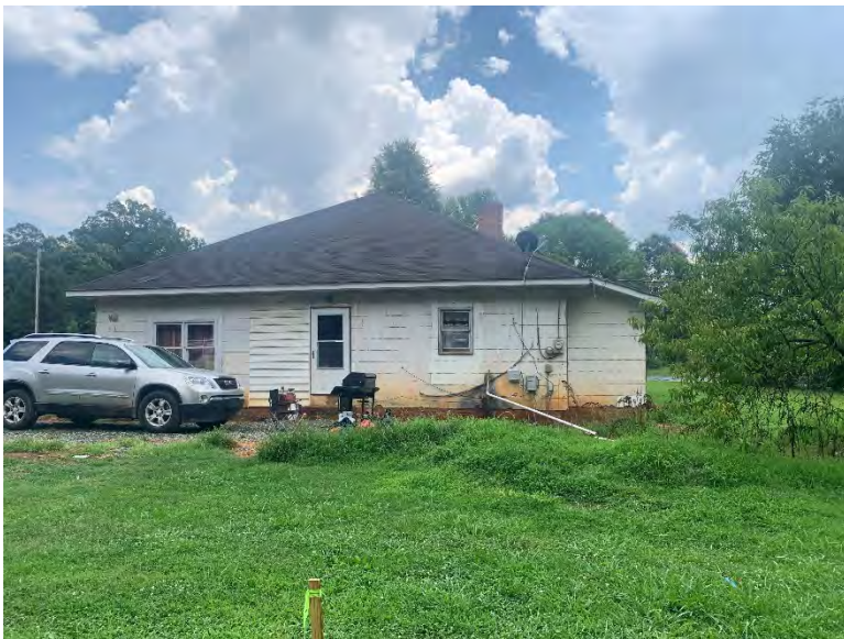
UN1223: northwest (rear) elevation, looking southeast
