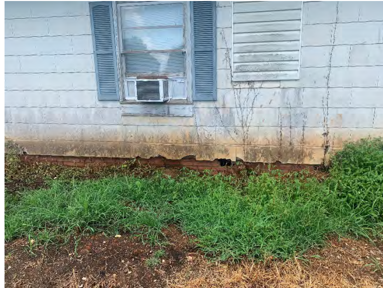
UN1223: northeast elevation, looking southwest
