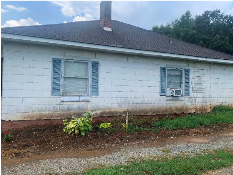
UN1223:northeast elevation, looking southwest
