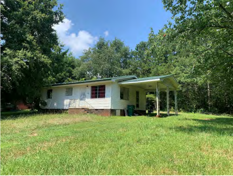
ST0909: looking west
