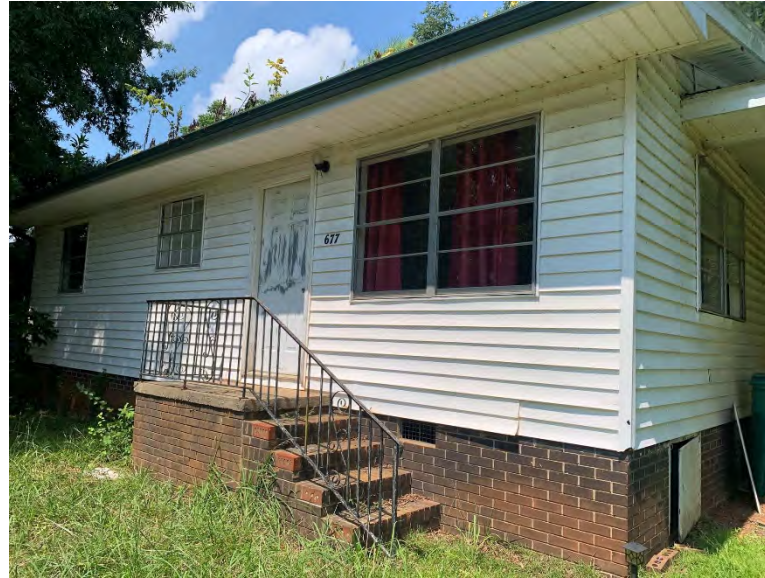
ST0909: looking west
