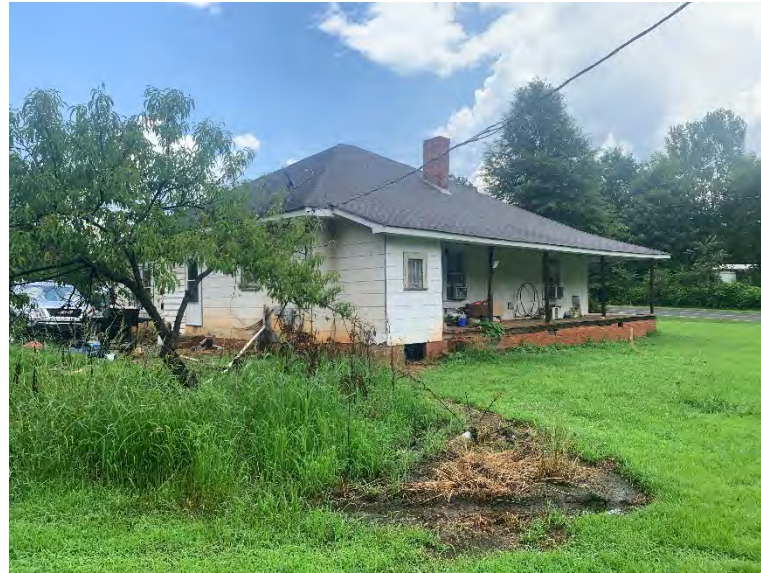
UN1223: southwest elevation (right), looking northeast
