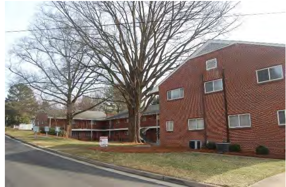
No. 4 Apartment Building (FY8776) (PIN 6825-45-5942), 1606 West Northwest Boulevard, Winston-Salem, Forsyth County
