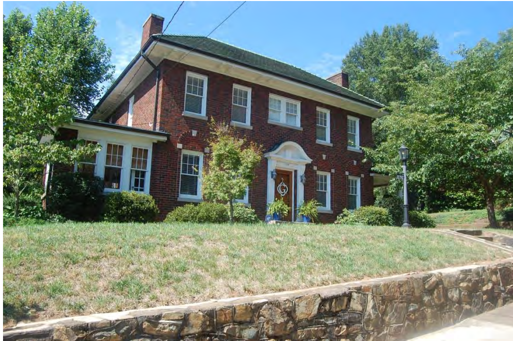
West Highlands Historic District, House, 1624 Lynwood Avenue, Looking West.
