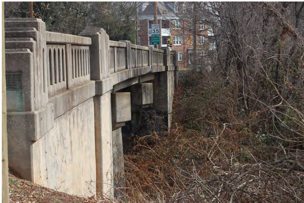
Bridge No. 296, Looking East.
