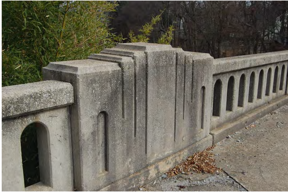
Bridge No. 296, Art Deco Bridge Wall, Looking North.
