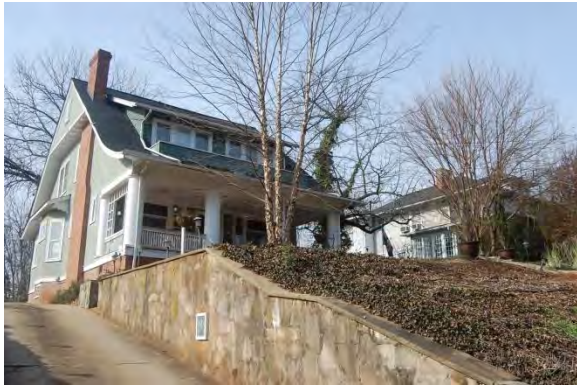
No. 9 House (PIN 6825-45-9689), 1622 West First Street, Winston-Salem, Forsyth County
