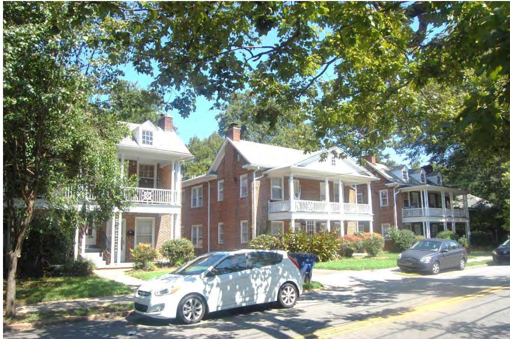
West Highlands Historic District, Apartment Buildings, 1569-1577 Northwest Boulevard, Looking Northwest.
