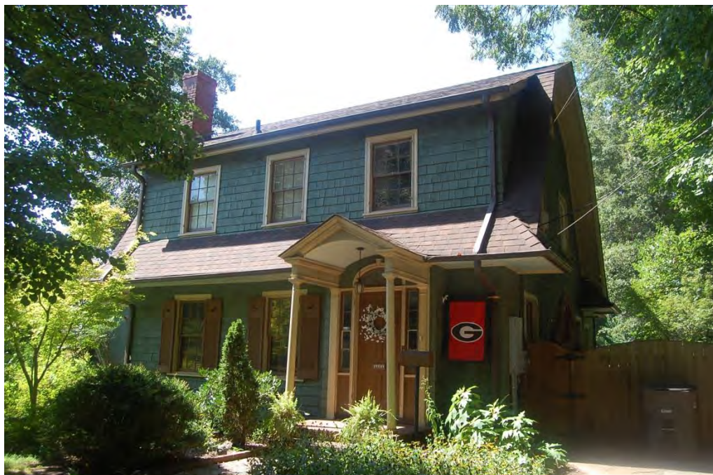
West Highlands Historic District, House, 1700 Lynwood Avenue, Looking West,
