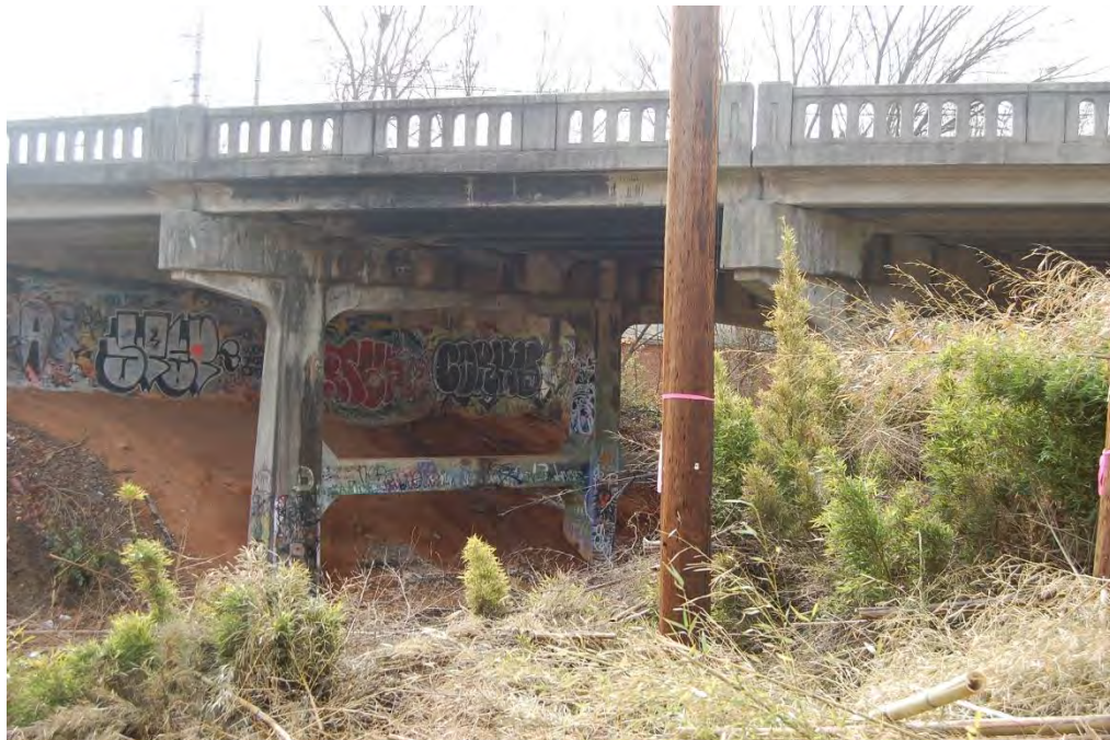
Bridge No. 296, Looking South.
