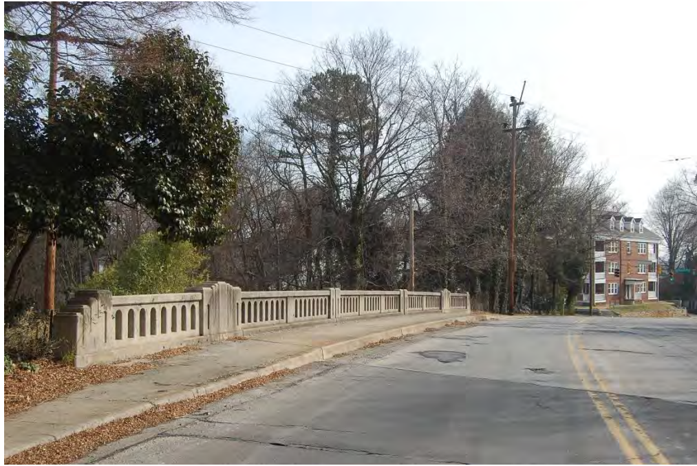
Bridge No. 296, Looking East.
