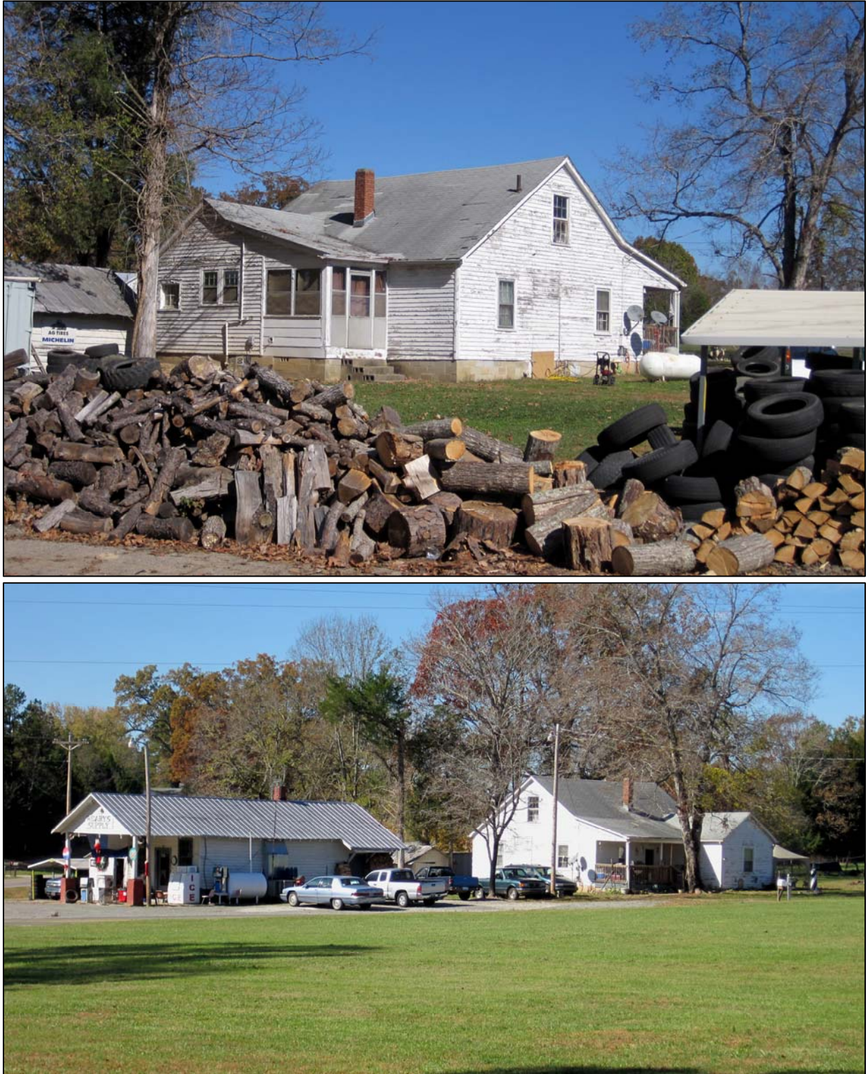
Figure 17. Single family residence at 9155 Grassy Creek Rd. Photos taken November 2012, facing northeast (top) and northwest (bottom).
