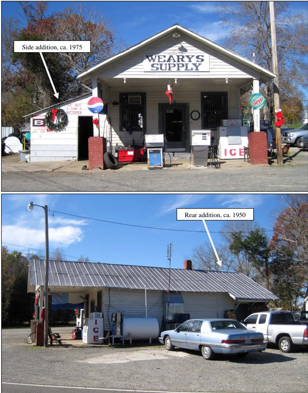
Figure 14. Weary's Supply. Photos taken November 2012, facing north (top) and west (bottom).
