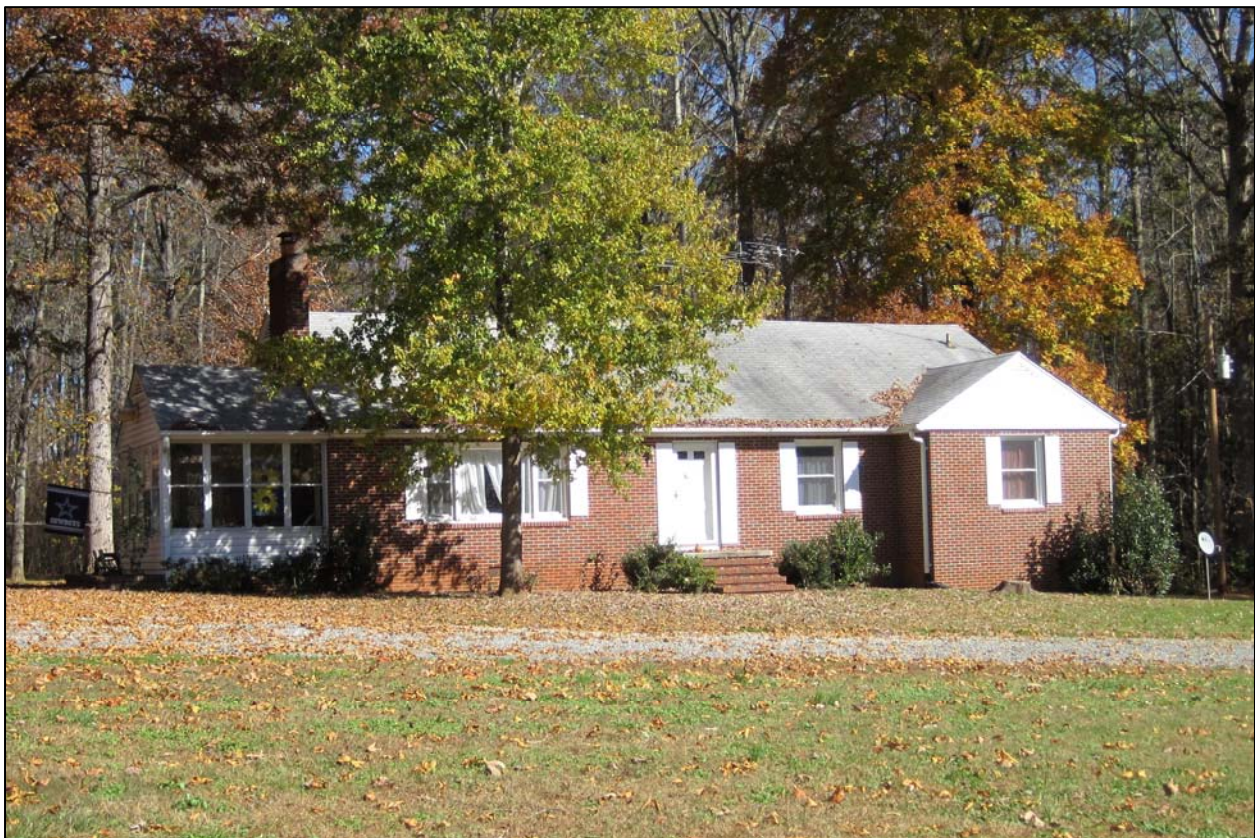
Figure 12. Grassy Creek Baptist Church Parsonage. Photos taken November 2012, facing northwest (top) and northeast (bottom).
