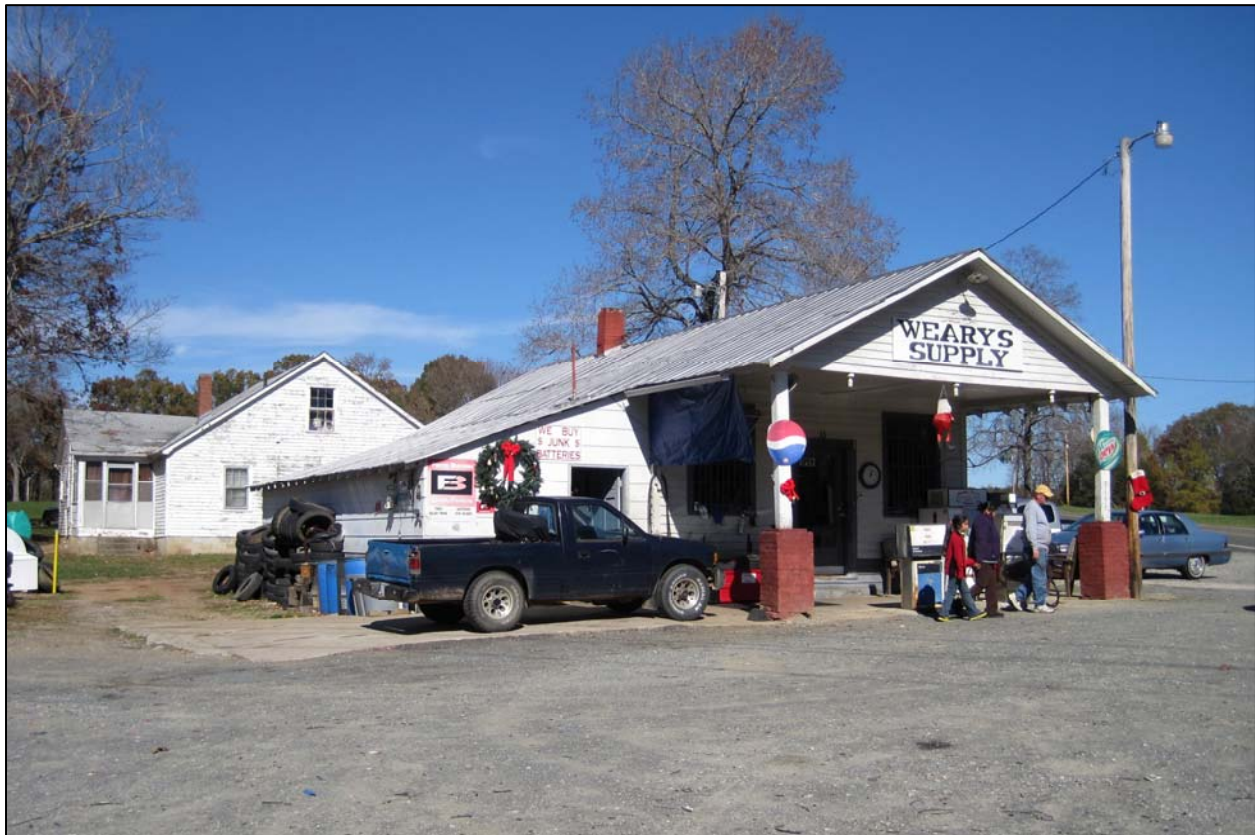
Figure 15. Weary's Supply. Photos taken November 2012, facing east (top) and northeast (bottom).
