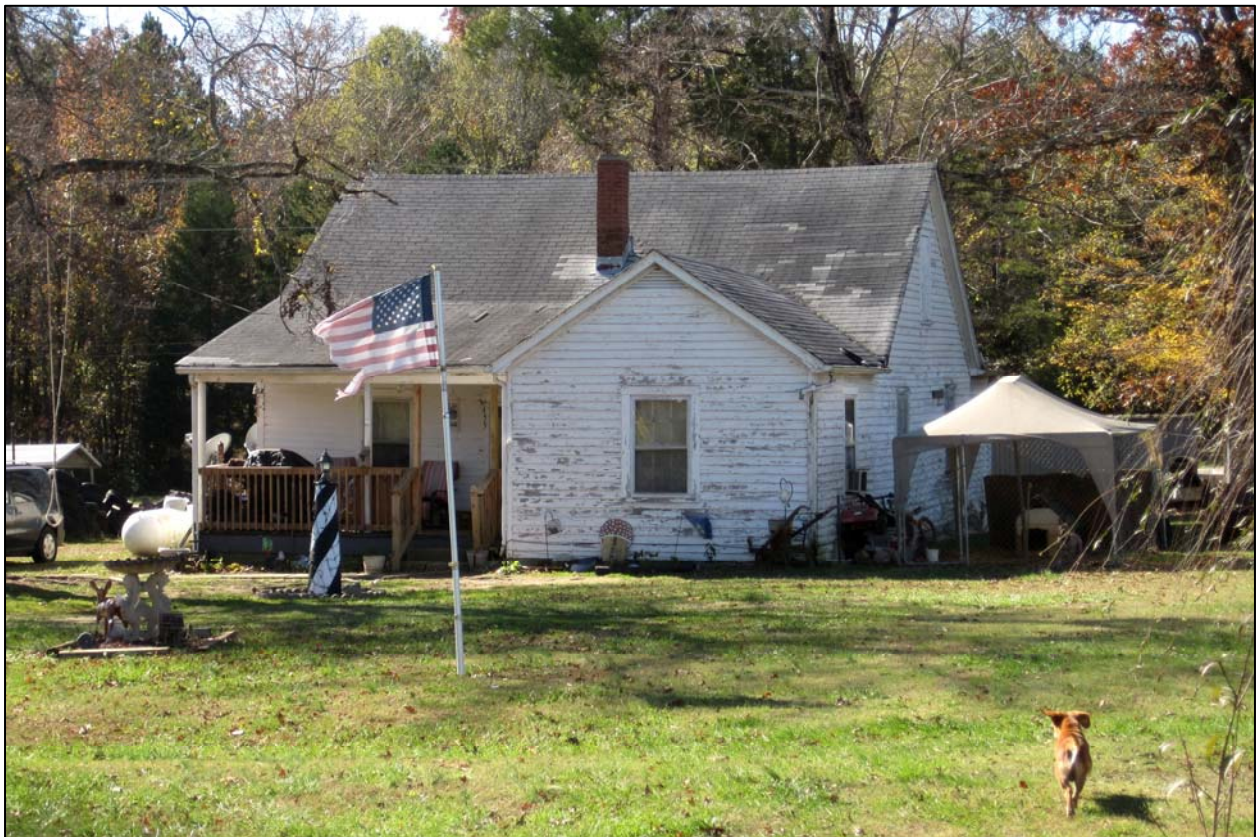
Figure 16. Single family residence at 9155 Grassy Creek Rd. Photos taken November 2012, facing west (top) and southwest (bottom).
