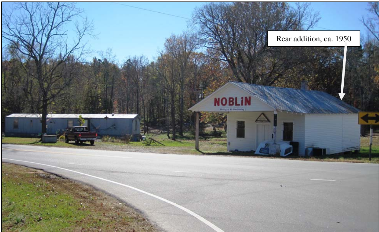
Figure 20. Noblin's Store. Photos taken November 2012, facing west (top) and south (bottom).
