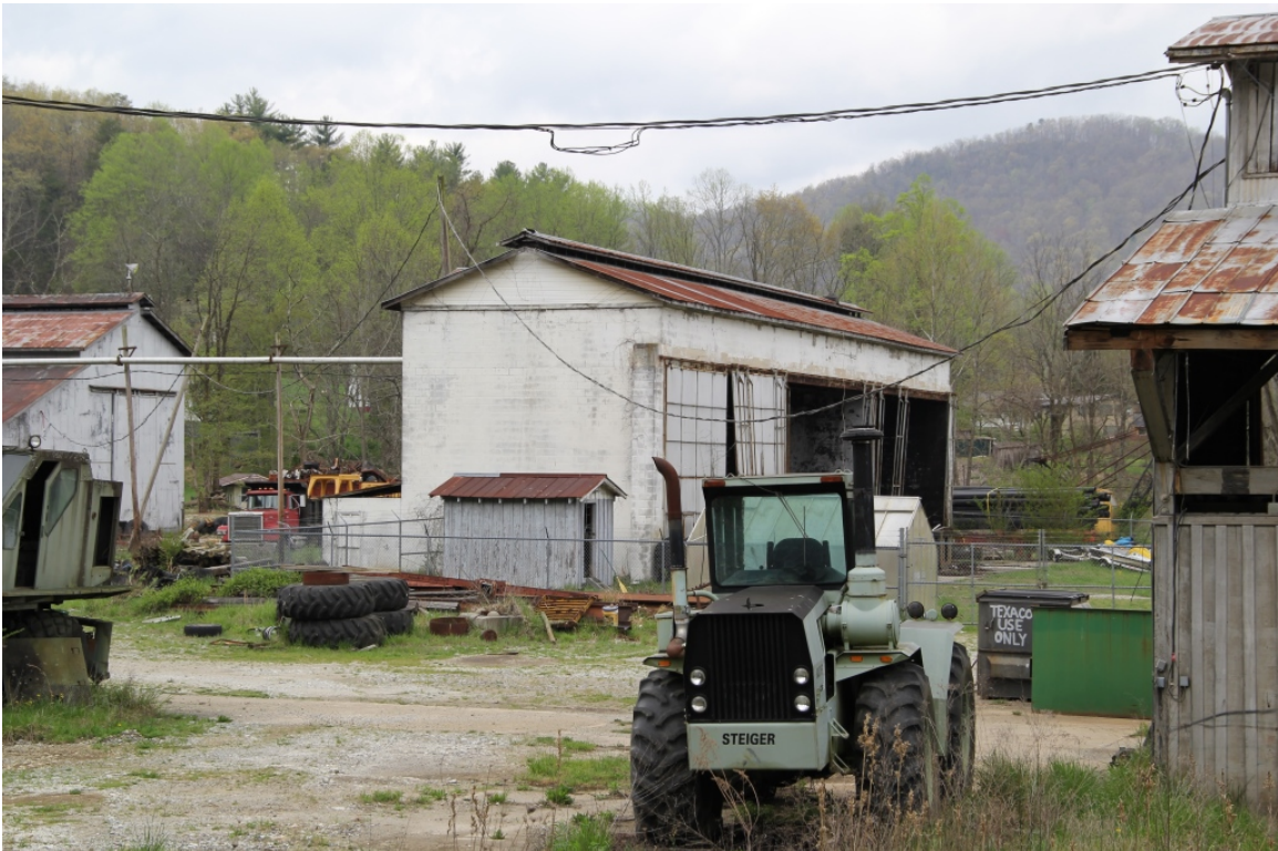
Dry Kiln, view to southwest; storage building in front of kiln
