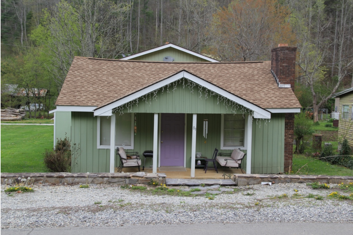
House, 89 Milltown Road, view to northeast
