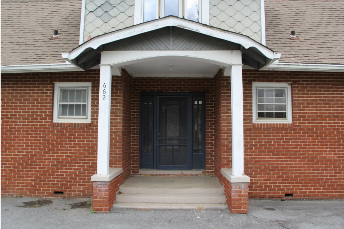
Bemis Company Office, entrance detail
