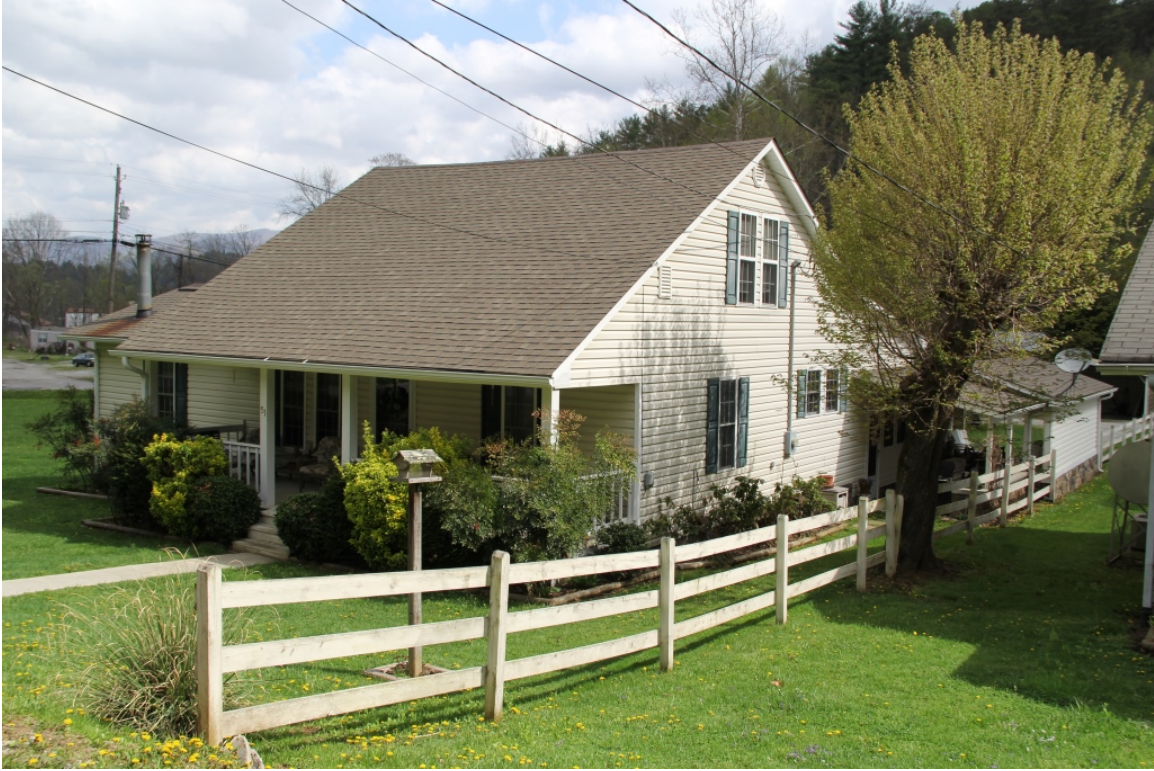
House, 51 Milltown Road, oblique front view to north
