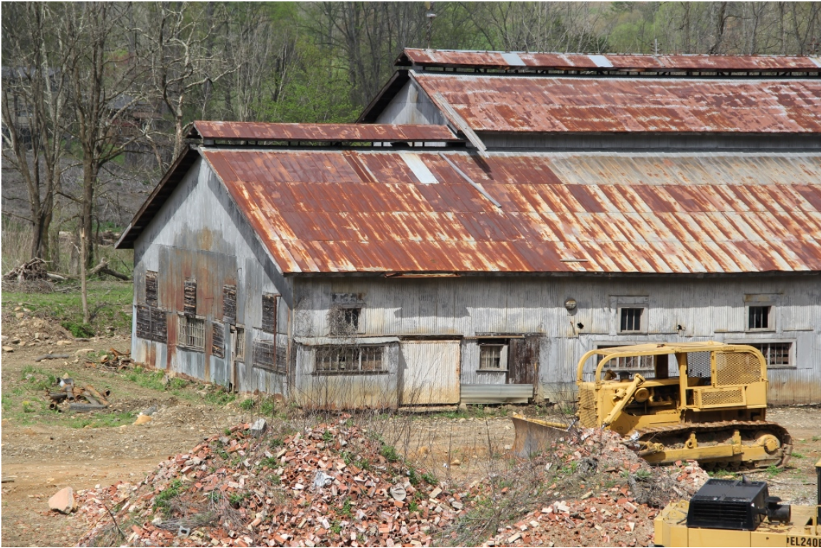
Shop (1927), overall view to northwest
