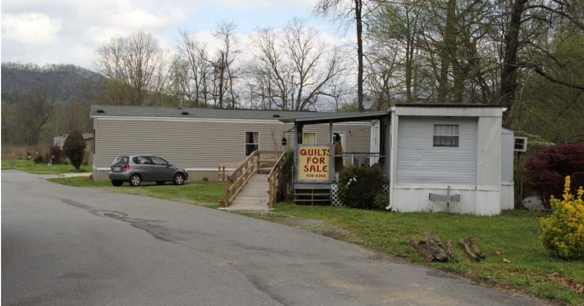
Mobile homes to east of Bemis Company Office, view north along driveway
