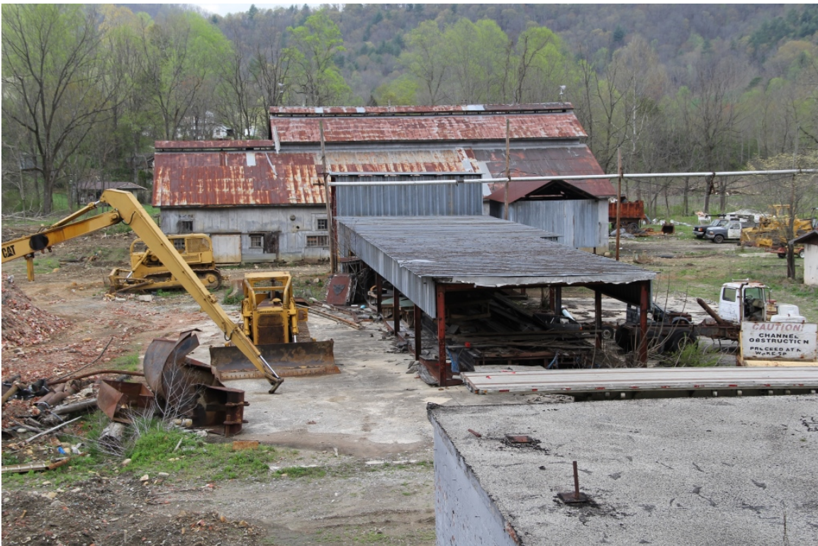
Remaining section of the saw mill, view to west
