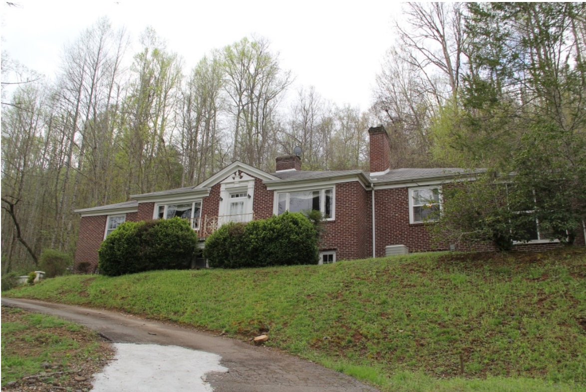
Wilson House, 4 Milltown Road, oblique front view to southwest
