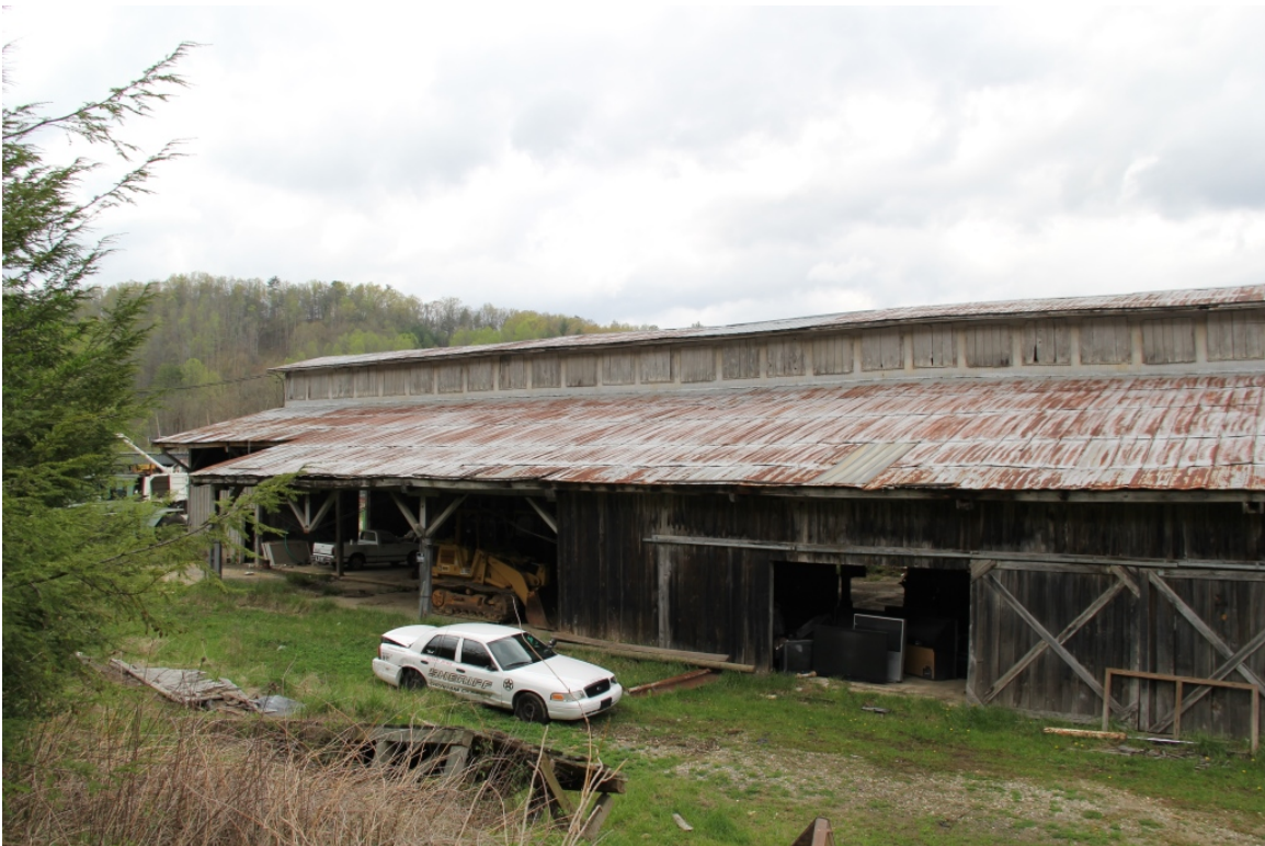
Shed, west elevation, view to southwest
