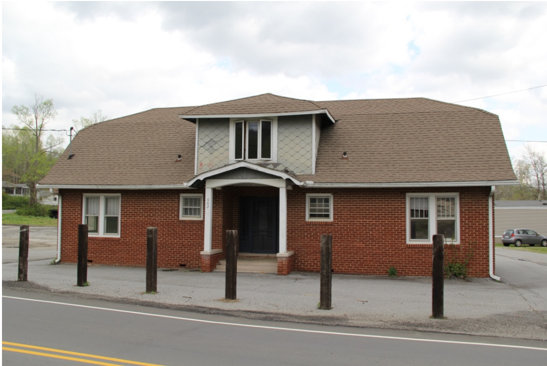
Bemis Company Office, 662 Snowbird Road, façade, view to northwest
