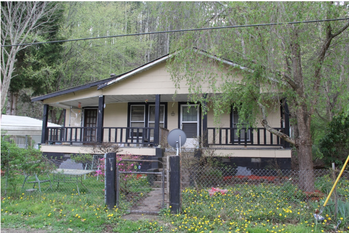
House, 118 Milltown Road, view to southwest
