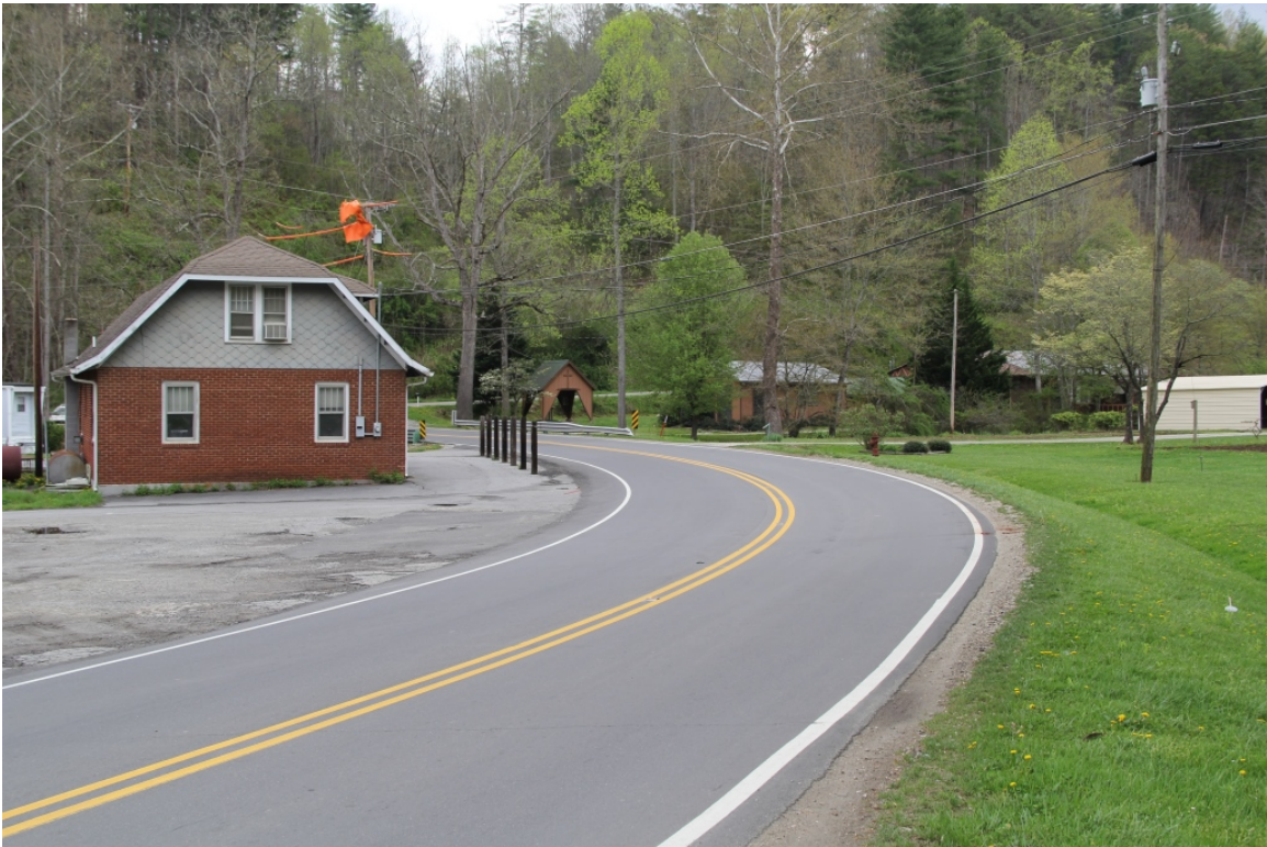
Bemis Company Office, west elevation, view to east along Snowbird Road
