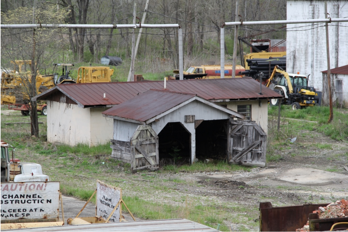
Garage (front) and Lounge (rear), overall view to northwest
