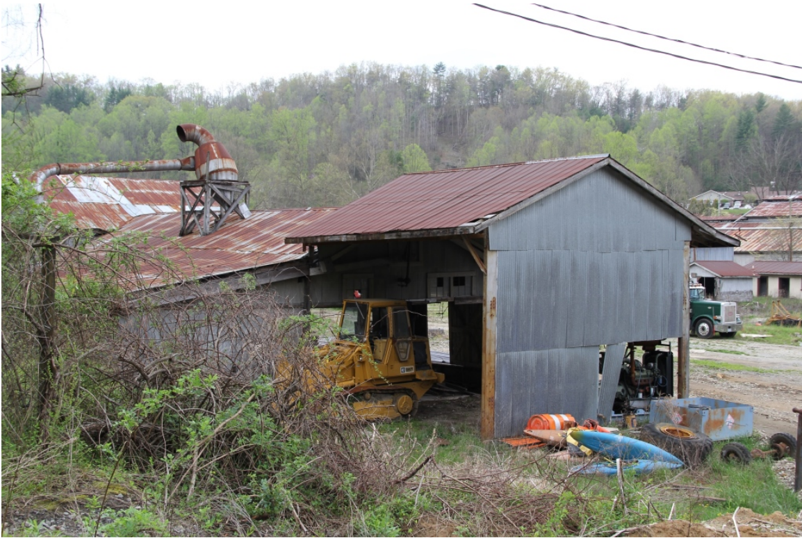
Planing mill, north end, oblique rear view to southwest
