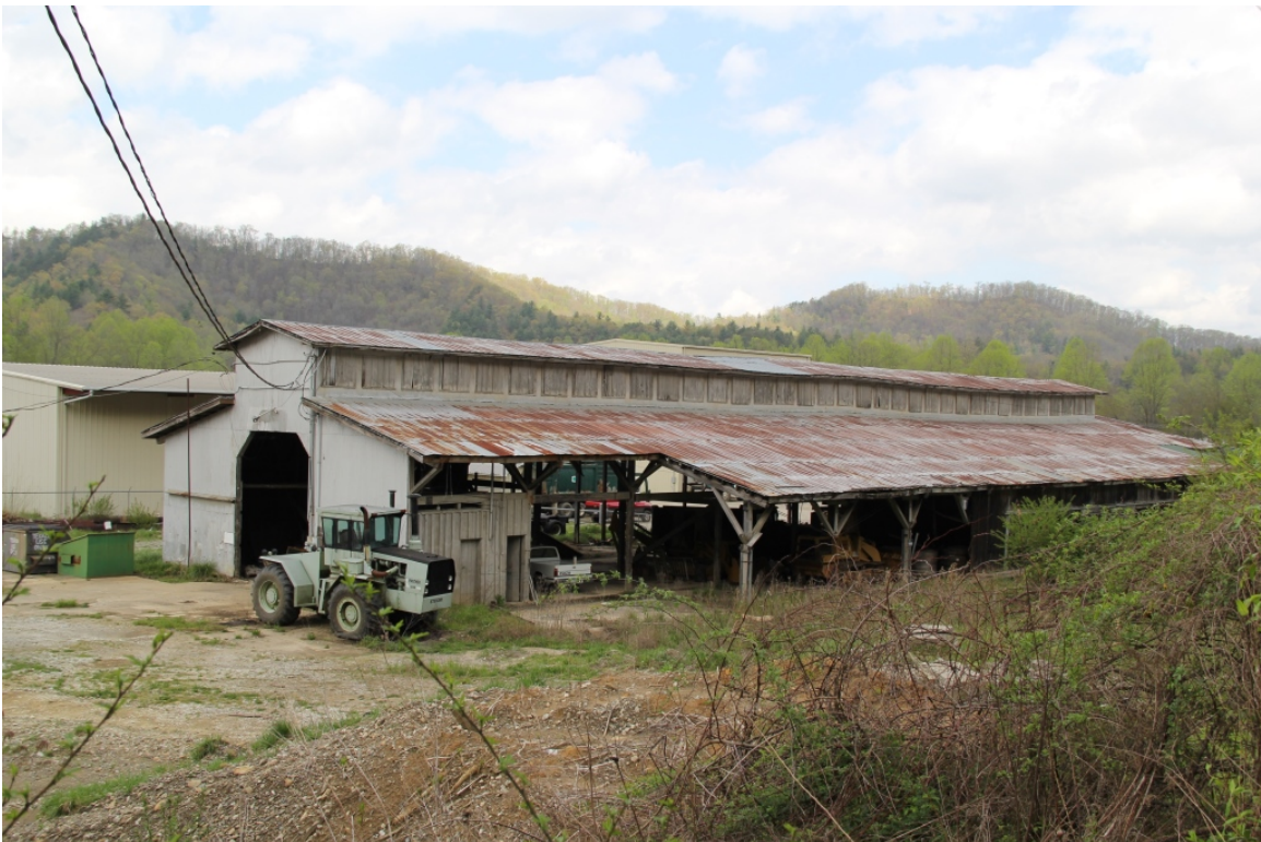
Shed, overall view to northwest
