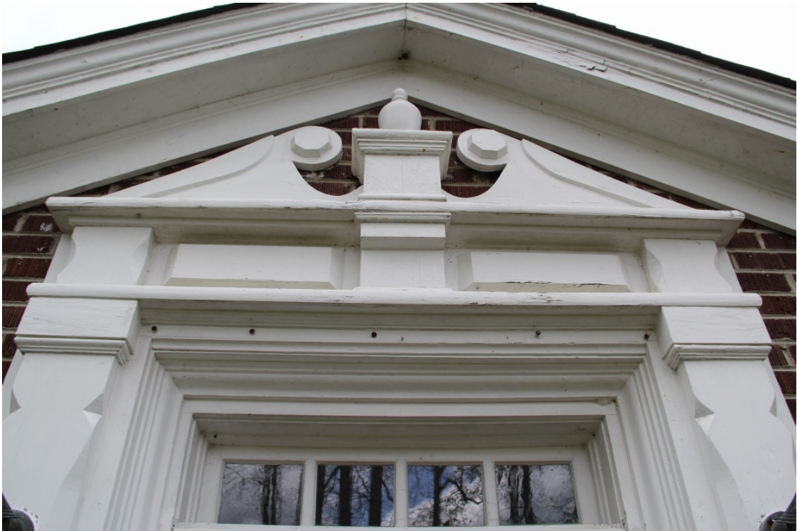
Wilson House, front entrance detail
