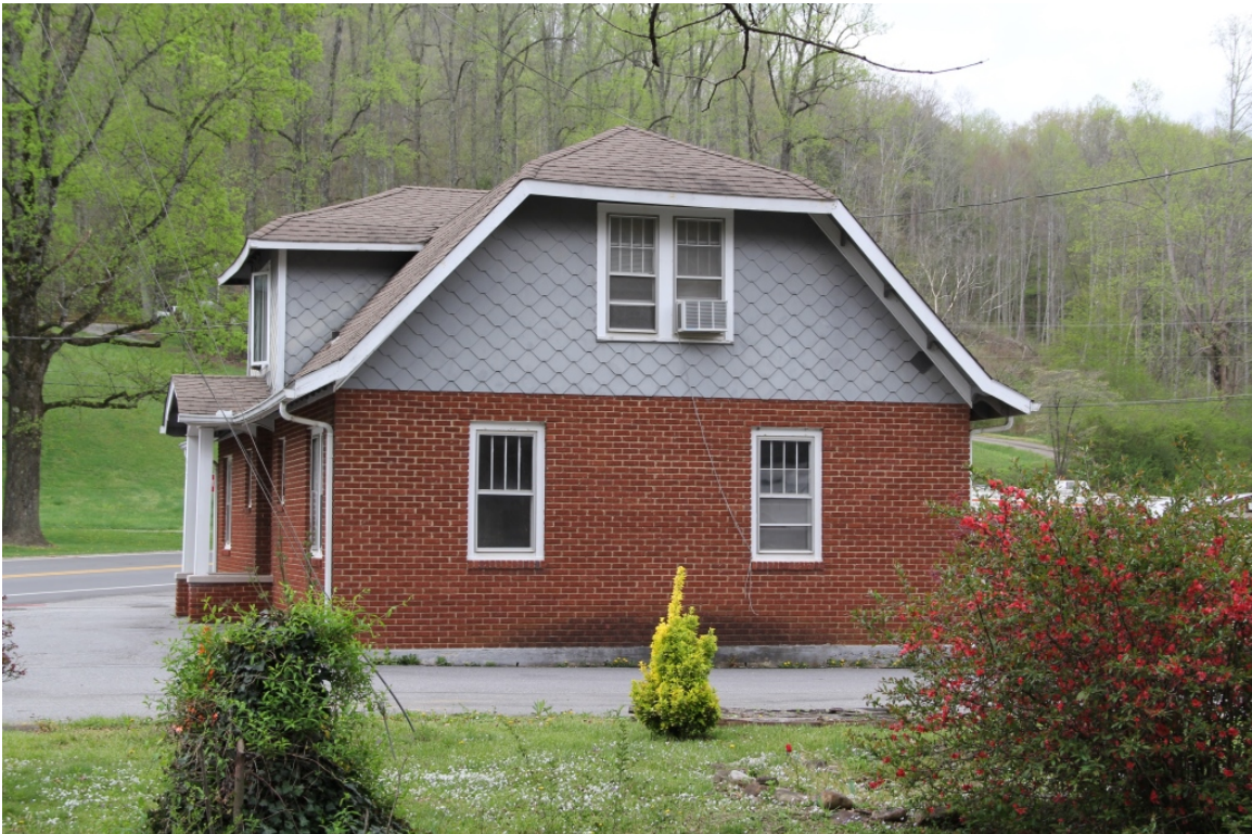
Bemis Company Office, east elevation, view to southwest
