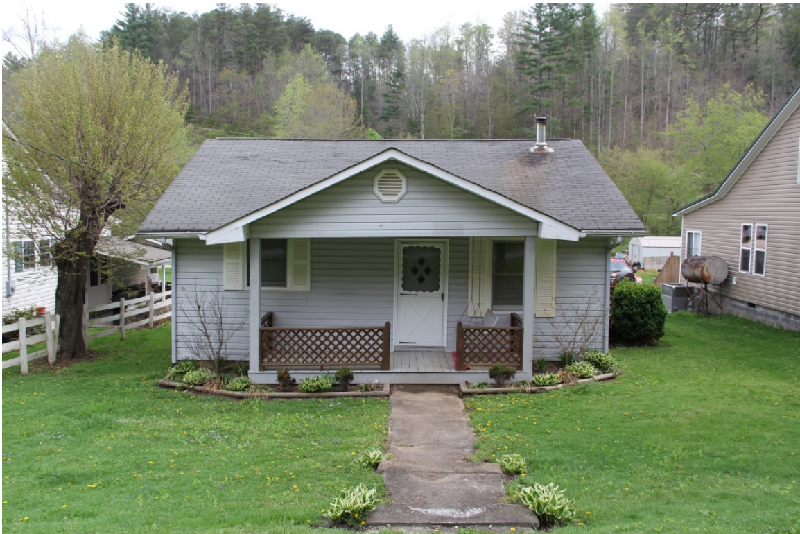
House, 61 Milltown Road, view to northeast
