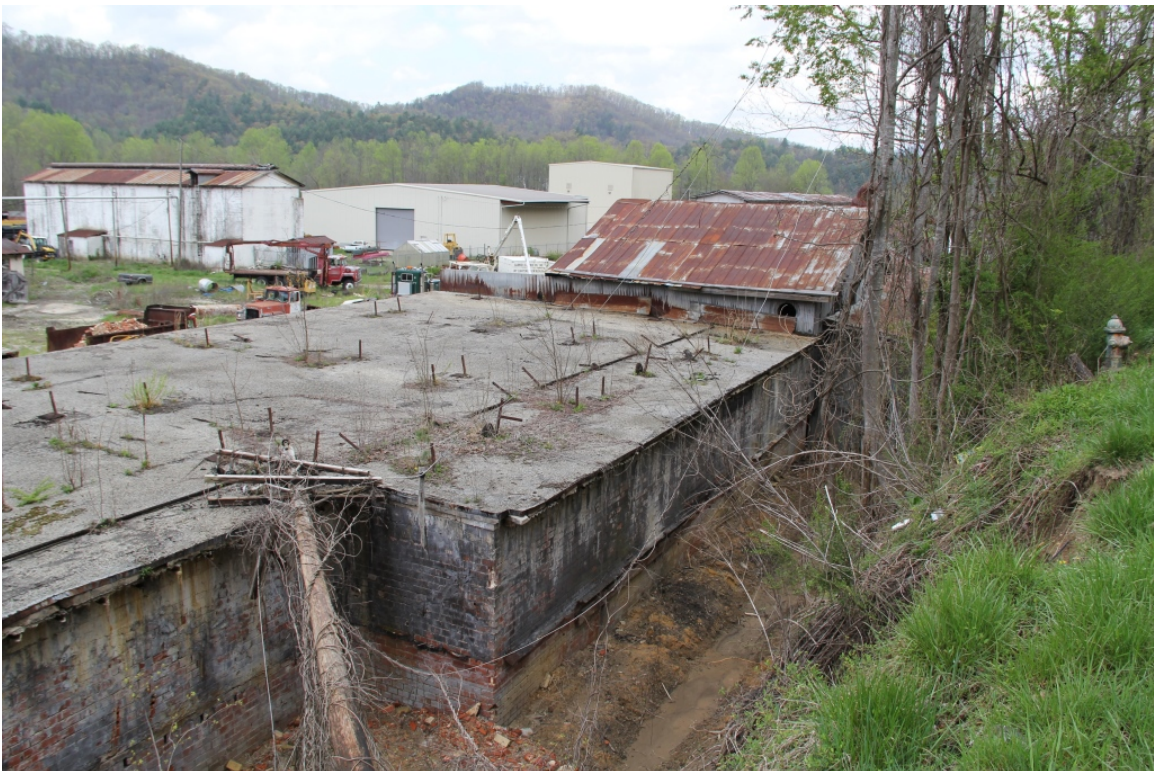
Planing mill, oblique rear view to northwest
