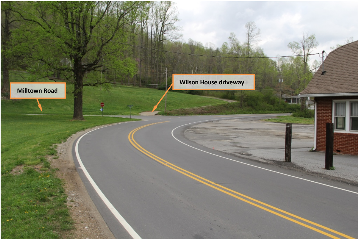
View northwest from Bridge No. 11 along Snowbird Road (NC 143B/SR 1127)
