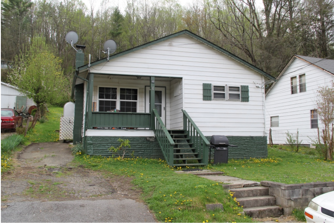
House, 80 Milltown Road, view to southwest
