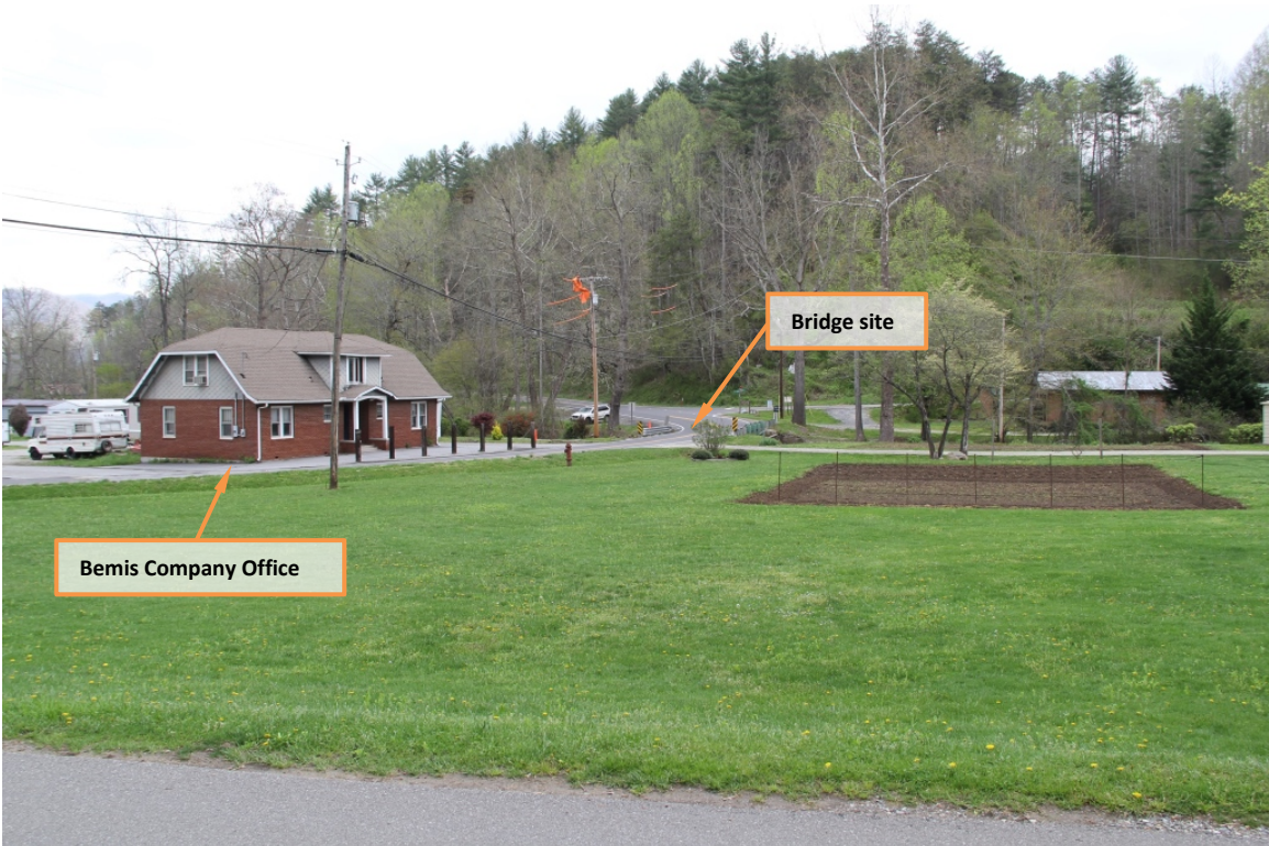
View northeast to Bridge No. 11 from Milltown Road (SR 1133)
