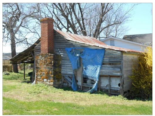
Figure 16. Outbuilding, view showing east gable end with stone chimney and replaced brick stack and north addition with shed roof, looking southwest.
