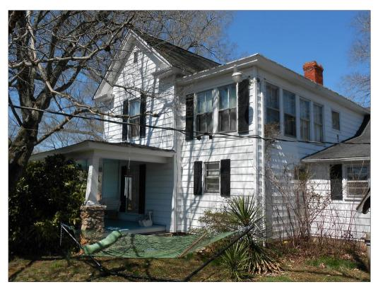
Figure 10. View of Isaac Terry House, rear elevation with 2-story rear section, looking northwest. The row of windows on the second story suggests a sleeping porch or sunroom. A portion of the gable-roofed rear ell with its later shed-roofed addition is visible on the right.
