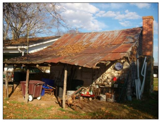
Figure 14. View of domestic outbuilding (possibly a kitchen/smokehouse converted to living quarters), south façade with later porch and east gable end chimney, looking northwest.
