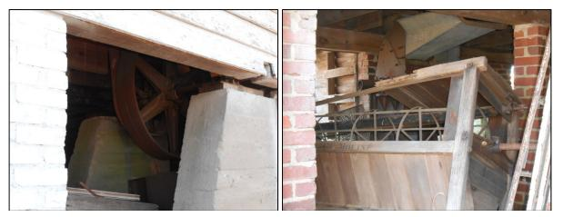
Figure 38. View of Clover Hill Corn Mill wheel (left) and chute (right), looking under building.
