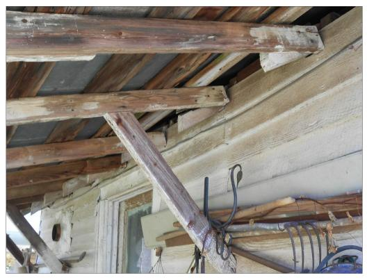
Figure 17. Outbuilding, view showing detail of braces attached to the south elevation and porch roof framing.
