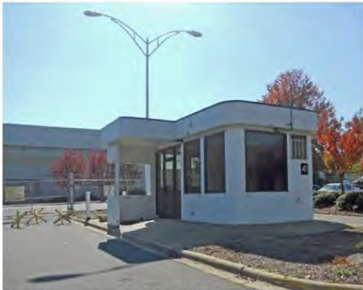
MK3160_CharlotteANGB_Bldg041_5-12_lp-02.jpg East and North façades
