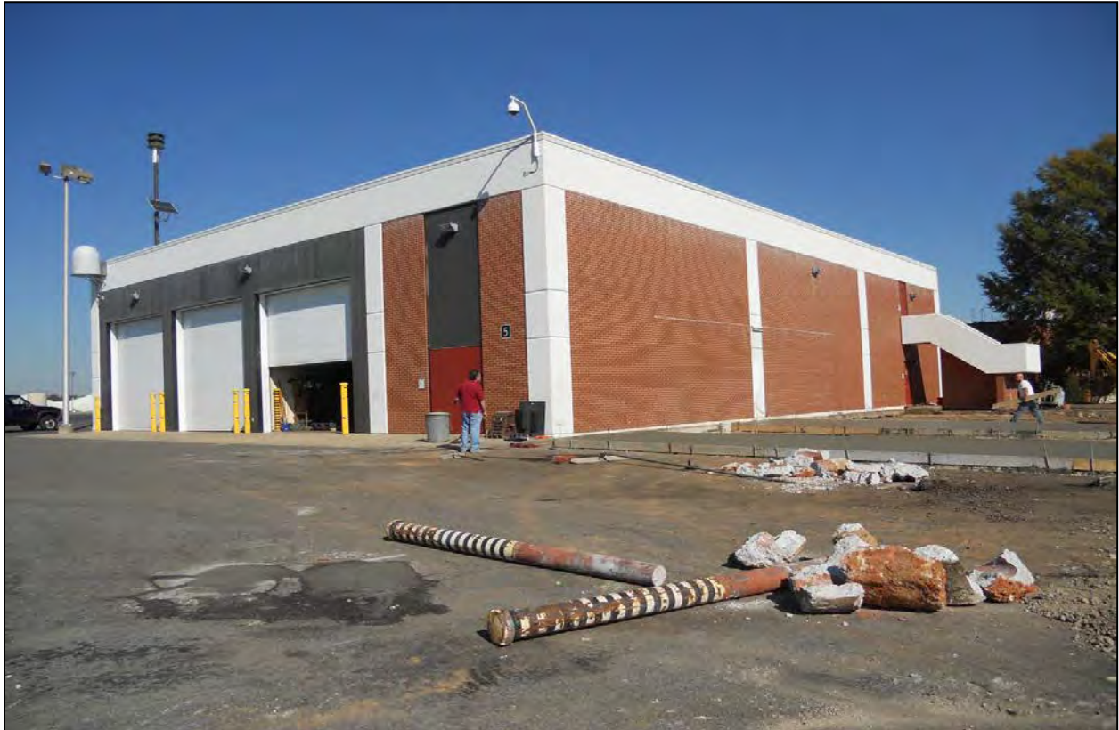
Figure 49. Building 5, West (Primary) and South Façades of Two-Story Block, View to Northeast.
