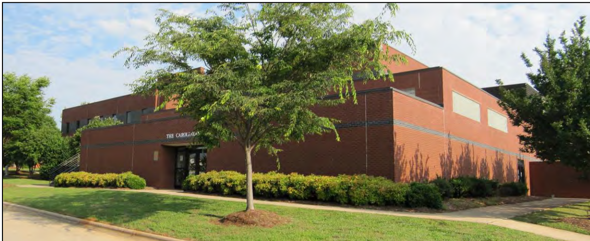
Figure 61. Building 45 South and East Façades, View to Northwest.
