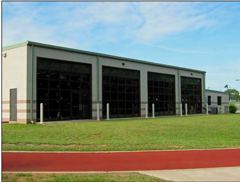
Figure 68. Building 69 North Façade, View to South.
