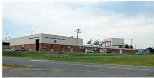
MK3157_CharlotteANGB_Bldg007_5-12_lp-01.jpg South and East façades
