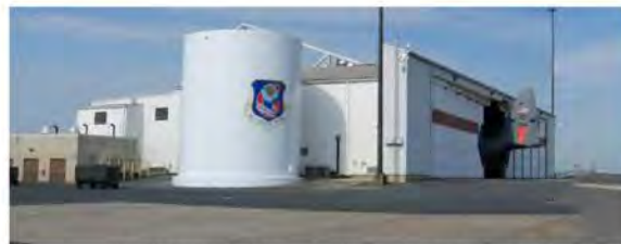
MK3155_CharlotteANGB_Bldg004_5-12_lp-01.jpg East and North façades
