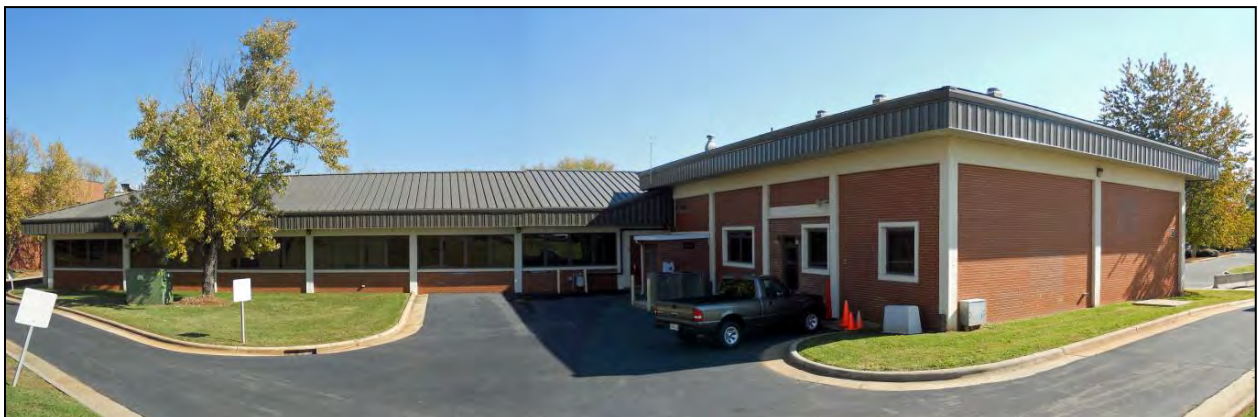
Figure 45. Building 2, West and North Façades, View to East.
