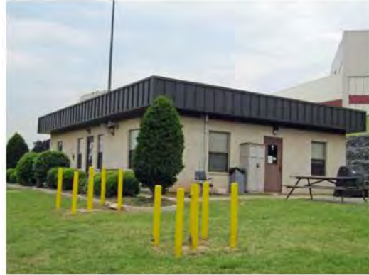
MK3158_CharlotteANGB_Bldg039_5-12_lp-02.jpg West and North façades
