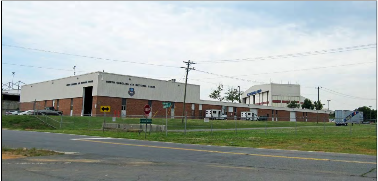
Figure 51. Building 7 South and East Façades, View to Northwest.
