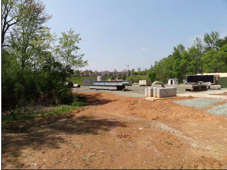
Figure 102. Stanly Area 4B, View Northwest.
