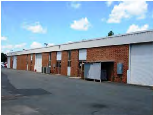
MK3157_CharlotteANGB_Bldg007_5-12_lp-02.jpg West façade
