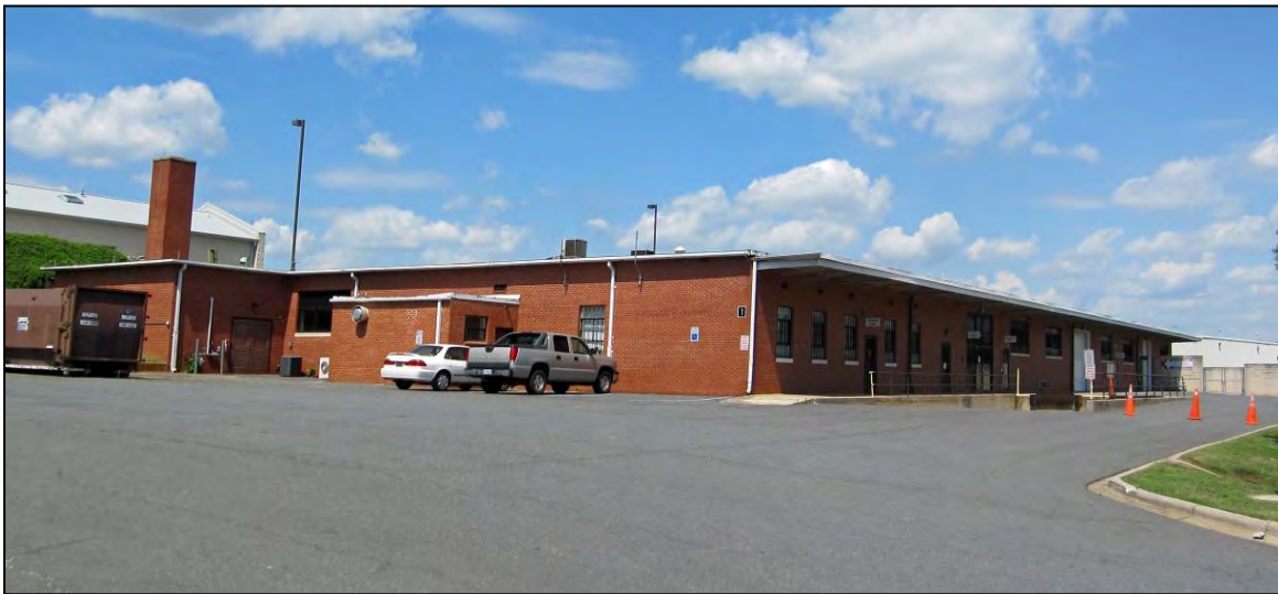
Figure 43. Building 1 West and South Façades, View to Northeast.
