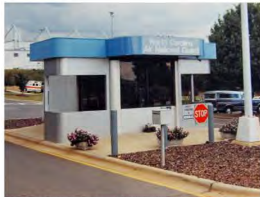
MK3160_CharlotteANGB_Bldg041_5-12_lp-03.jpg West and South facades in 1985 photograph
