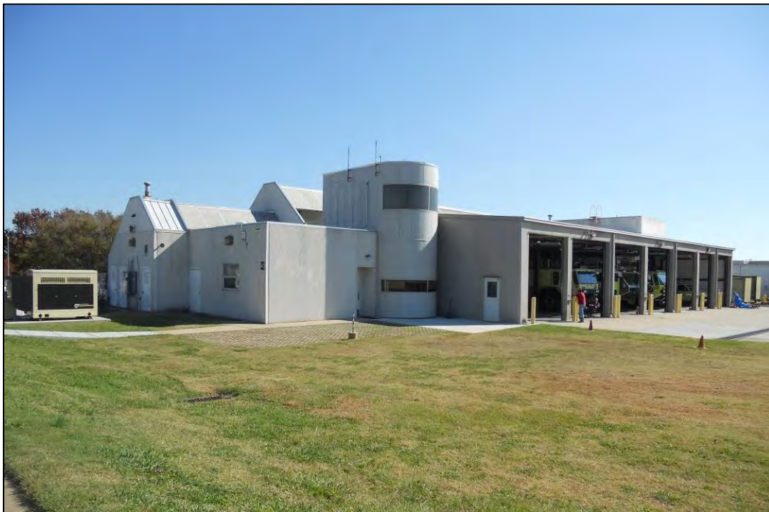
Figure 55. Building 40 North Façade and West Façade Oriented to the Airfield, View to Southeast.
