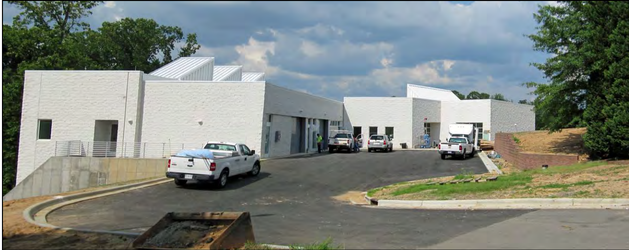
Figure 59. Building 43 Southwest and South Façades, View to East.
