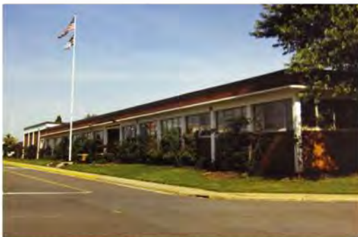
MK3153_CharlotteANGB_Bldg002_5-12_lp-03.jpg South and East façades in 1960 photograph
