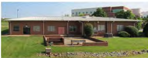
MK3165_CharlotteANGB_Bldg050_5-12_lp-02.jpg South façade
