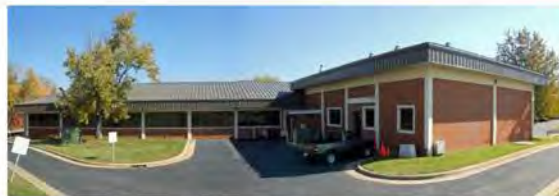
MK3153_CharlotteANGB_Bldg002_5-12_lp-02.jpg South and East façades
