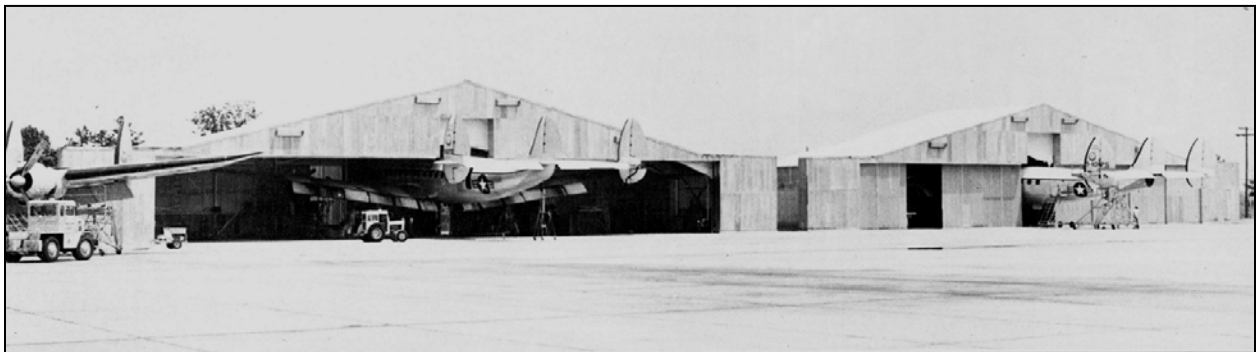
Figure 16. These NCANG C-121s Are Parked inside the Charlotte ANGB Hangars; One of the Hangars Was Building 22, Constructed in 1965 (Reid 1998:104).
