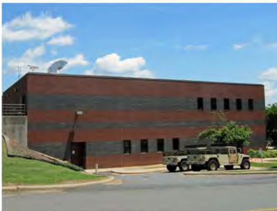
MK3162_CharlotteANGB_Bldg045_5-12_lp-03.jpg West façade
