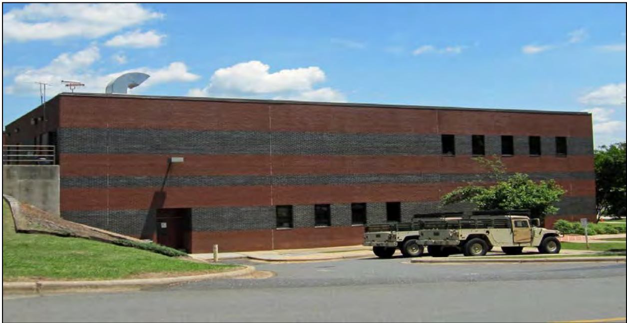
Figure 62. View to East of Building 45 West Façade.
