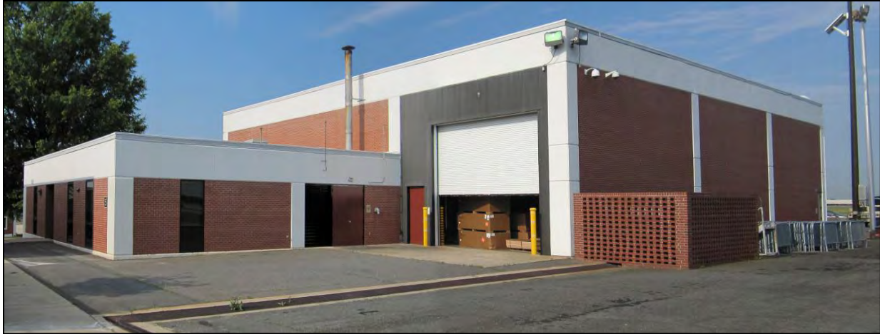
Figure 50. Building 5 East and North Facades, View to Southwest.
