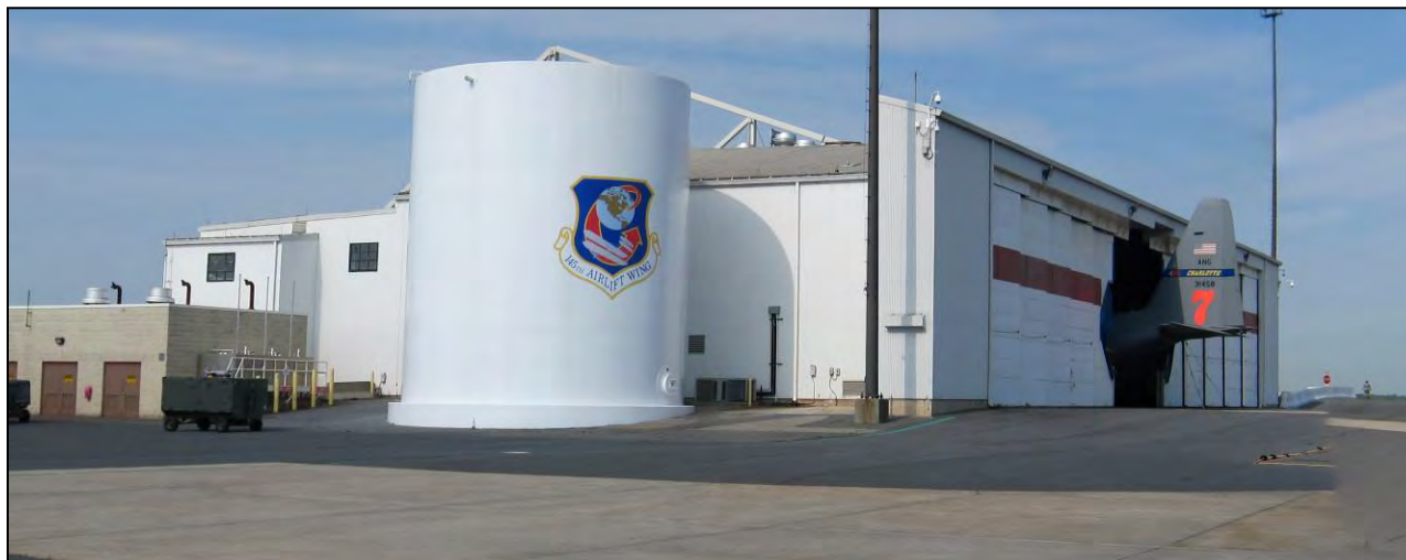
Figure 47. Building 4 East and North (Primary) Façades, View to Southwest. Building 137 is the tank containing fire suppression material.
