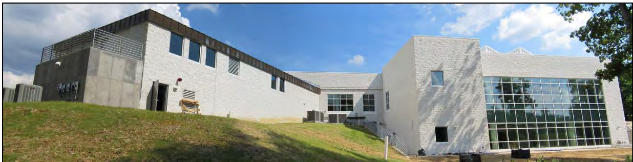
Figure 58. Building 43, View to South.
