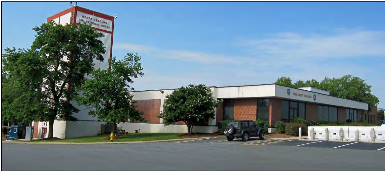
Figure 46. Building 3 East and North Façades, View to Southwest.
