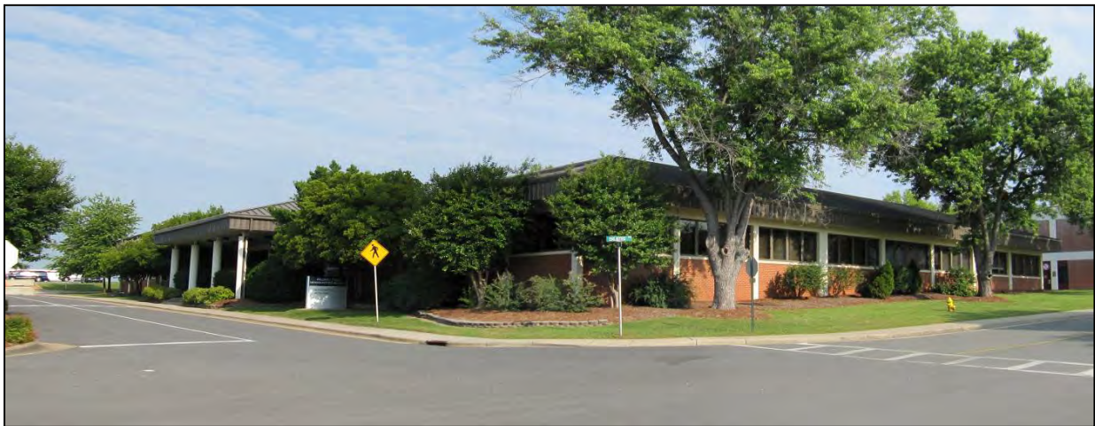
Figure 44. Building 2 South and East Façades, View to Northwest.
