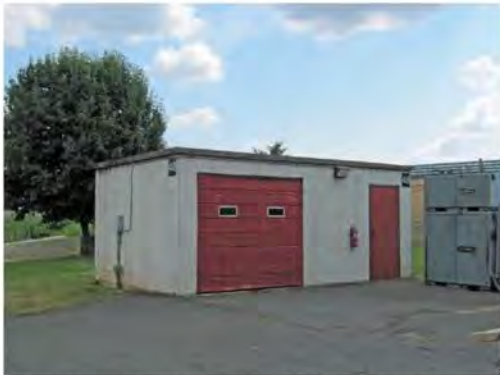
MK3163_CharlotteANGB_Bldg048_5-12_lp-01.jpg East and North façades
