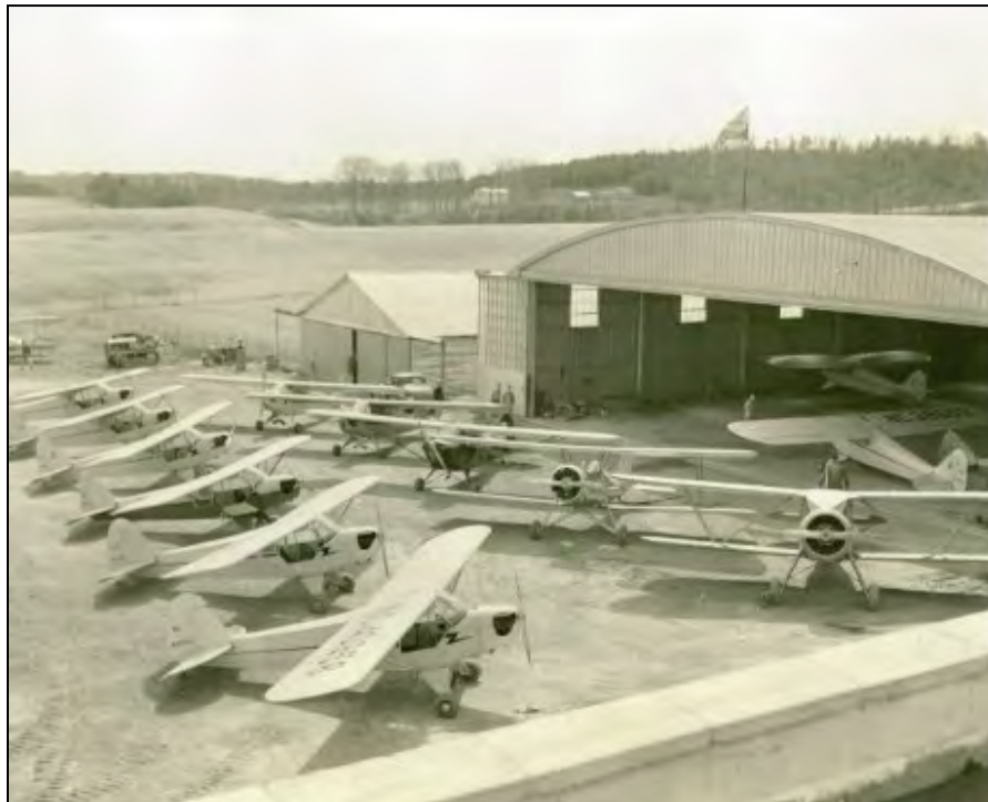
Figure 20. The Original Albemarle Airport Shortly after Its 1946 Construction (Courtesy of the Albemarle Charlottesville Historical Society).
