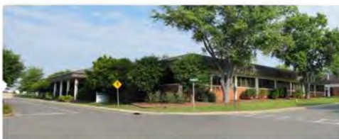
MK3153_CharlotteANGB_Bldg002_5-12_lp-01.jpg West and North façades
