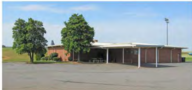
MK3165_CharlotteANGB_Bldg050_5-12_lp-01.jpg North and West façades
