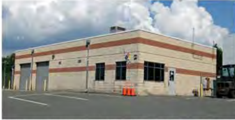
MK3164_CharlotteANGB_Bldg049_5-12_lp-01.jpg North and West façades
