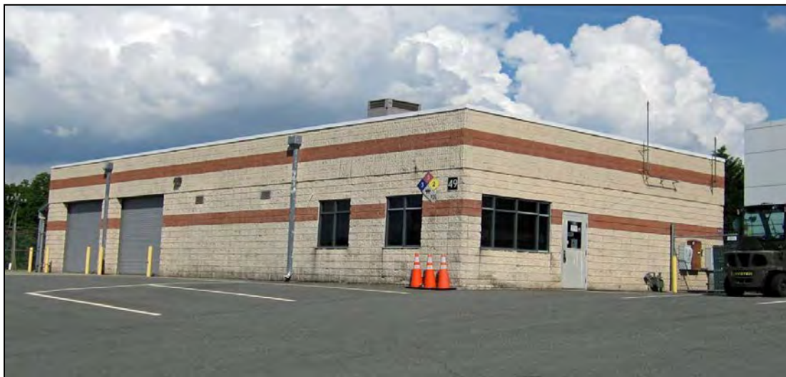
Figure 64. Building 49 North and West (Primary) Façades, View to the Southeast.
