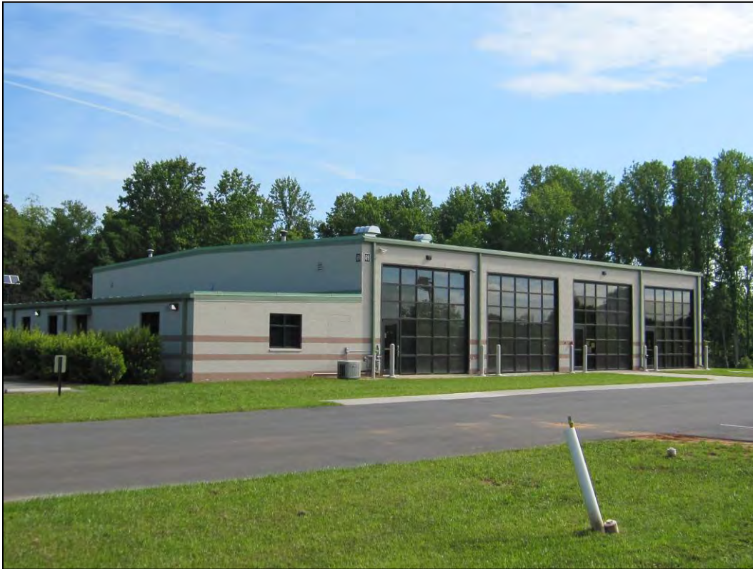
Figure 67. Building 69 West (Primary) and South Façades, View to Northeast.
