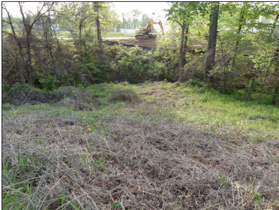
Figure 41. West Side of Charlotte Area 3, View East.
