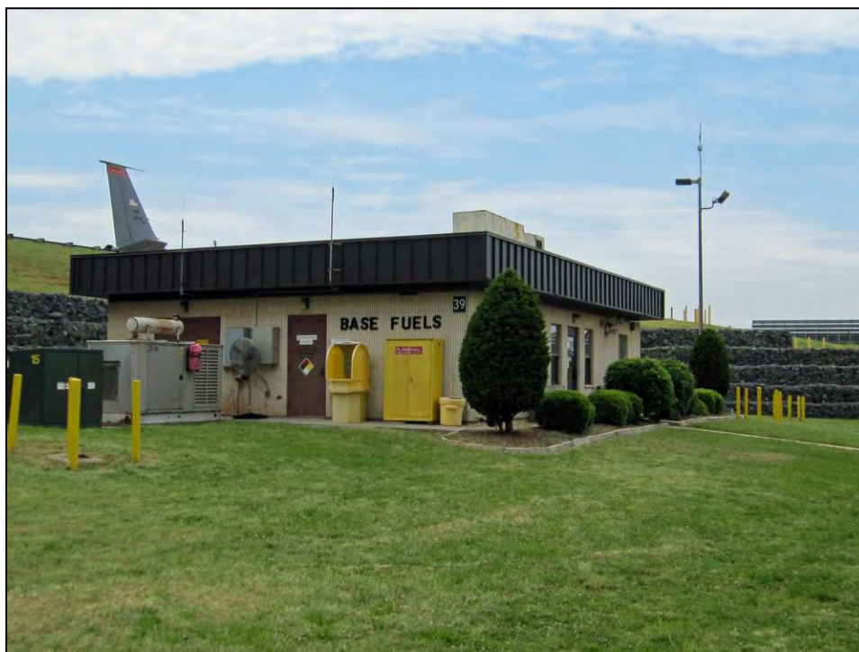
Figure 53. Building 39 East and North (Primary) Façades, View to Southwest.
