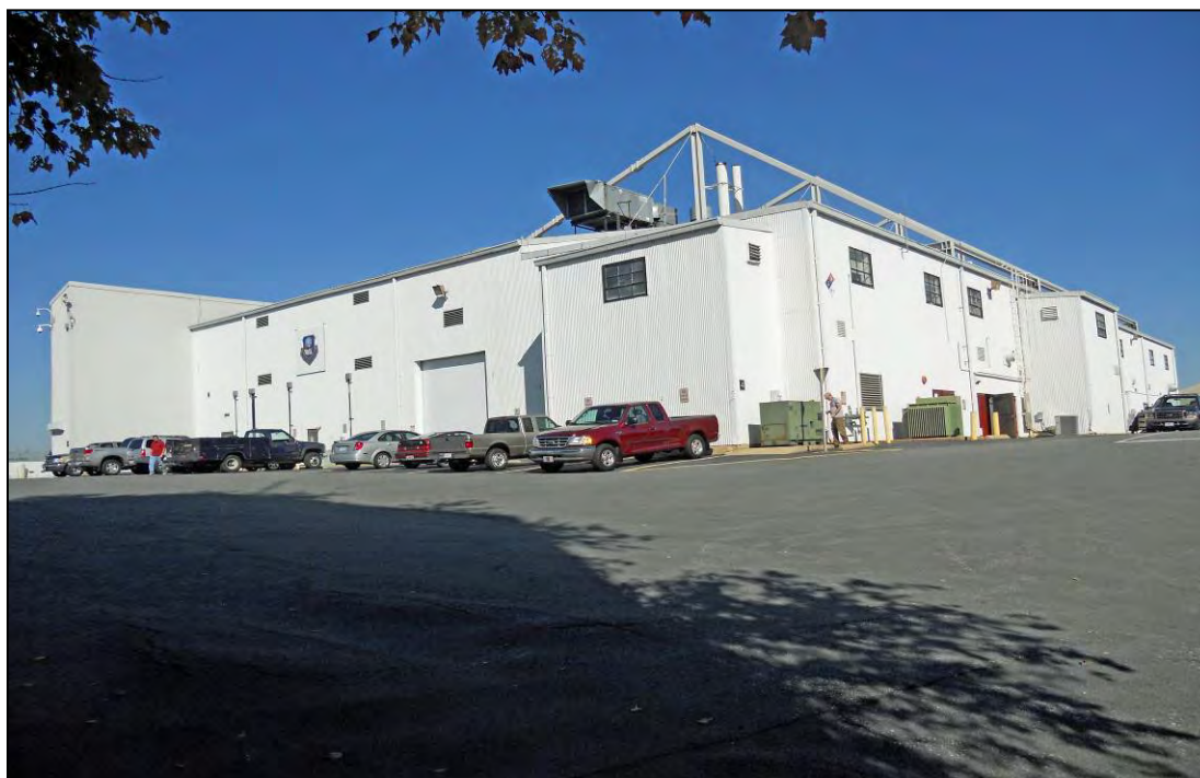
Figure 48. Building 4 West and South Façades, View to Northeast.
