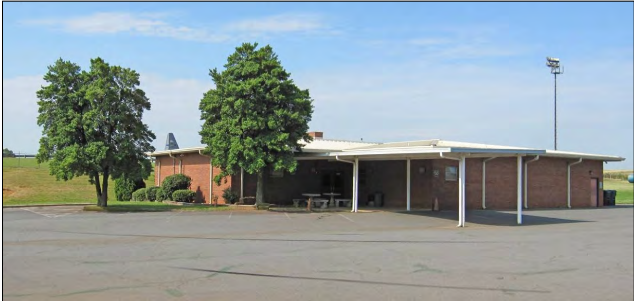
Figure 65. Building 50 North Primary Façade and East Façade.
