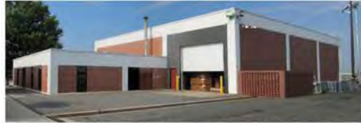
MK3156_CharlotteANGB_Bldg005_5-12_lp-02.jpg East and North façades
