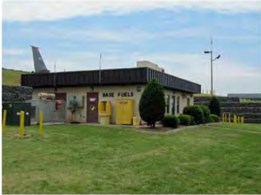
MK3158_CharlotteANGB_Bldg039_5-12_lp-01.jpg East and North façades
