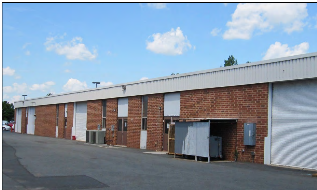
Figure 52. Building 7, West Façade of One-Story Block, View to Northeast.
