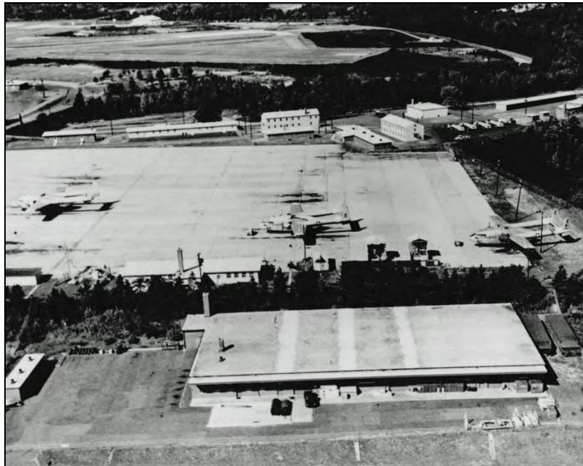
Figure 14. View to North, with Building 1 (1956) in the Foreground and Surplus Morris Field Army Buildings in the Background (NCANG Heritage Program 2012).
