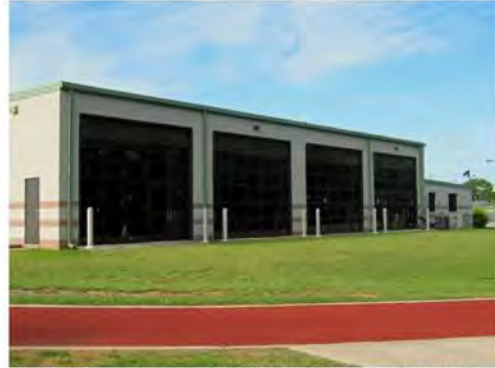
MK3166_CharlotteANGB_Bldg069_5-12_lp-02.jpg North facade
