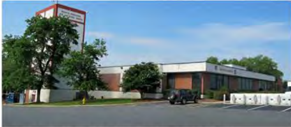
MK3154_CharlotteANGB_Bldg003_5-12_lp-01.jpg North and East façades
