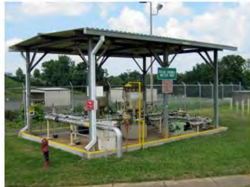
MK3167_CharlotteANGB_Bldg131_5-12_lp-01.jpg South and West façades
