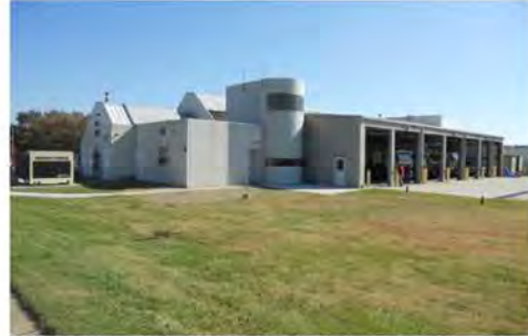
MK3159_CharlotteANGB_Bldg040_5-12_lp-02.jpg North and West façades
