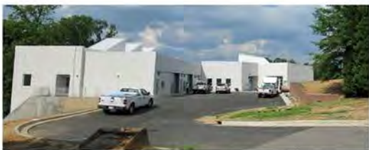
MK3161_CharlotteANGB_Bldg043_5-12_lp-03.jpg South and Southwest façades
