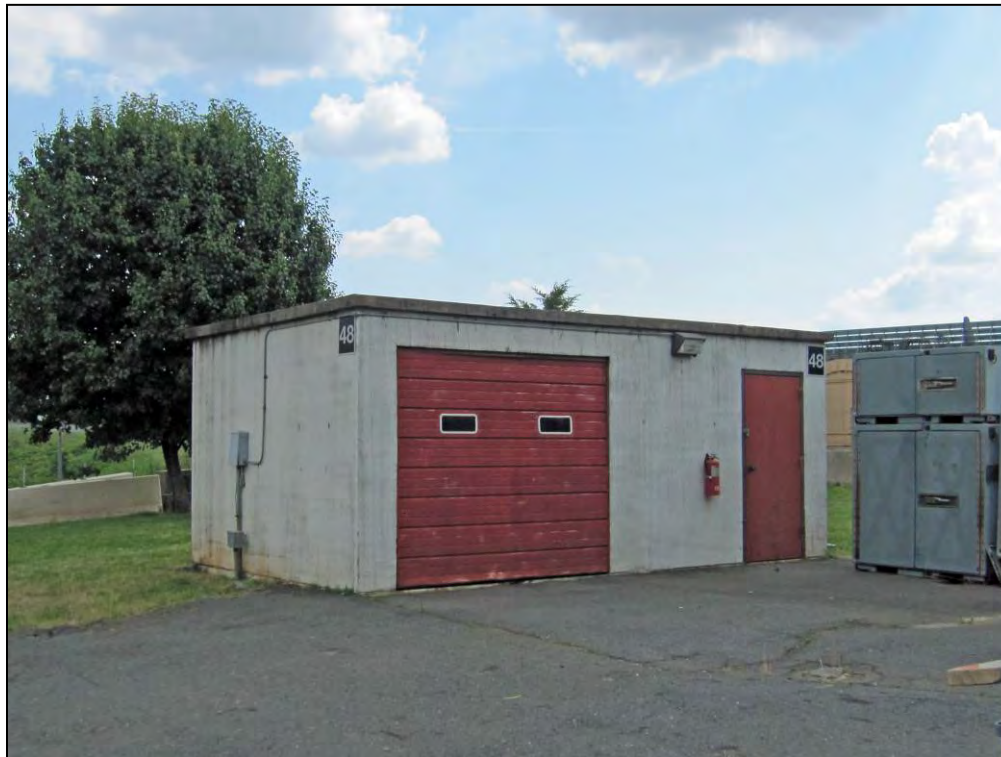
Figure 63. Building 48 North (Primary) and East Façades, View to Southwest.
