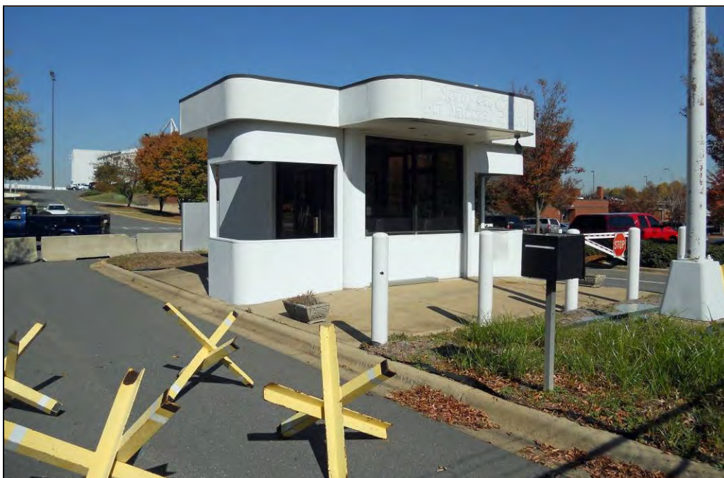
Figure 56. Building 41 West and South Façades, View to Northeast.
