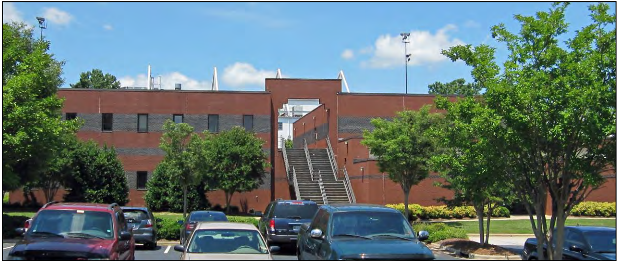
Figure 60. Building 45 South Façade and Brick Arch Leading to Interior Courtyard, View to North.
