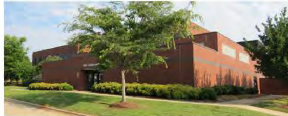
MK3162_CharlotteANGB_Bldg045_5-12_lp-02.jpg South and East façades
