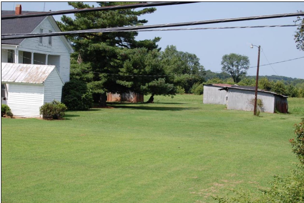
Campbell-Gray House and outbuildings looking SW from Regional Road S (Marvin Brown, August 2013)
