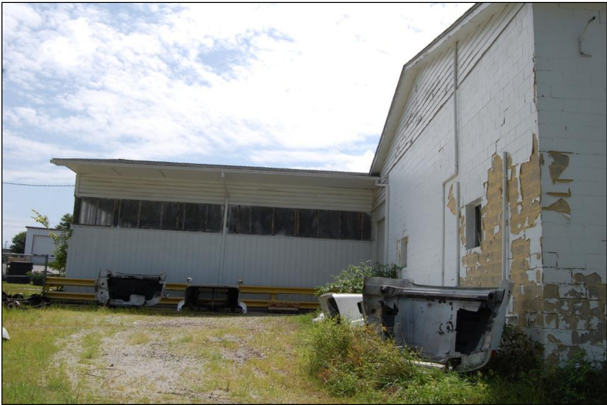
Additions to barn, looking SE (barn not visible)
