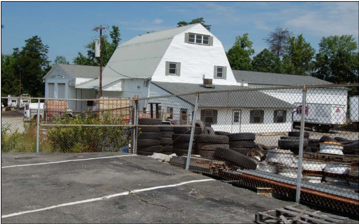
Barn and additions looking NW
