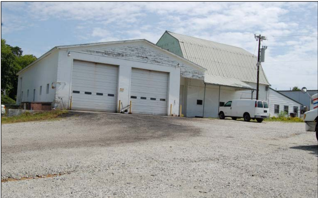
Barn and additions looking NE
