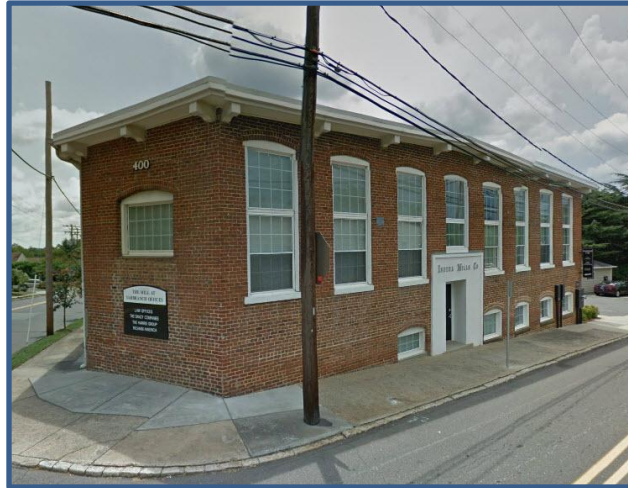
Figure 24. Property No. 70 – Indera Mills. Main mill building, looking southwest.
