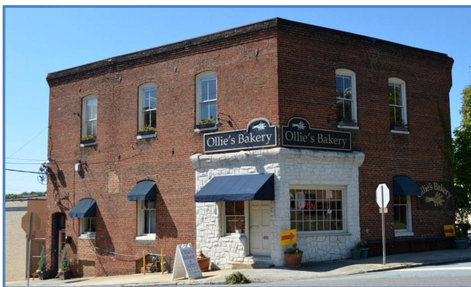
Figure 9. Property No. 76 - Commercial Building, 300 South Marshall Street, 1904. Northeast oblique. (HF)
