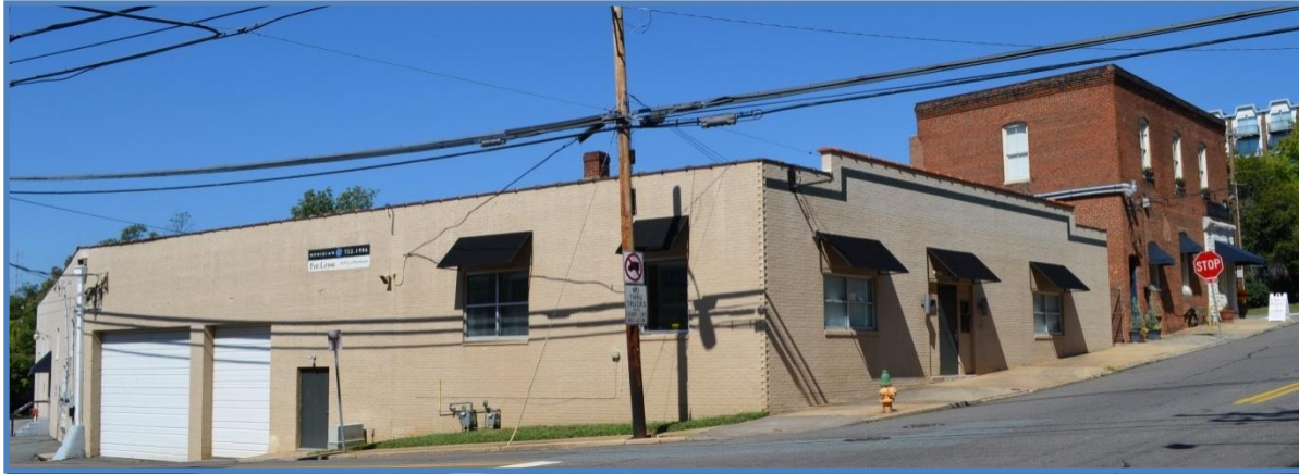
Figure 11. Property No. 77 - Commercial Building, 308 South Marshall Street, 1947. Southeast oblique. (HF)
