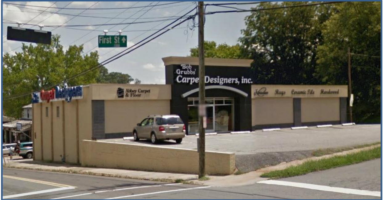
Figure 63. Property No. 134 – Commercial Building, 1168 West Fourth Street.
