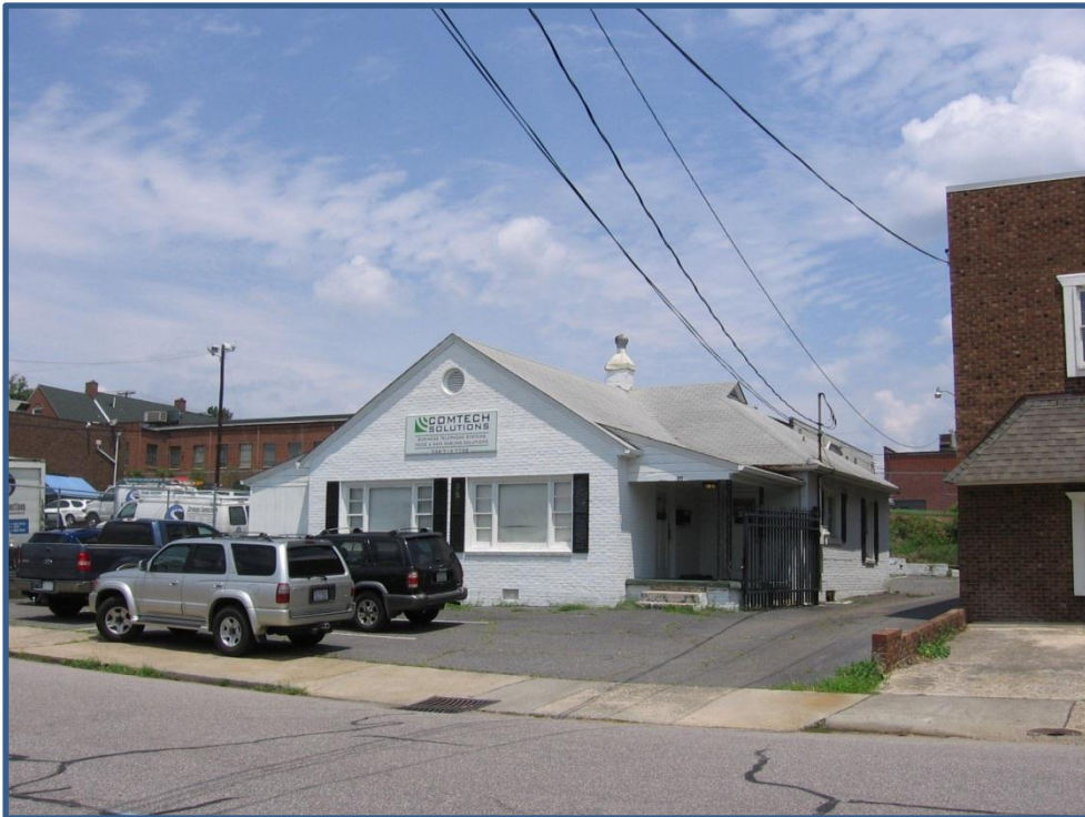
Figure 58. Property No. 129 – Commercial Building, 131-133 Fayette Street.
