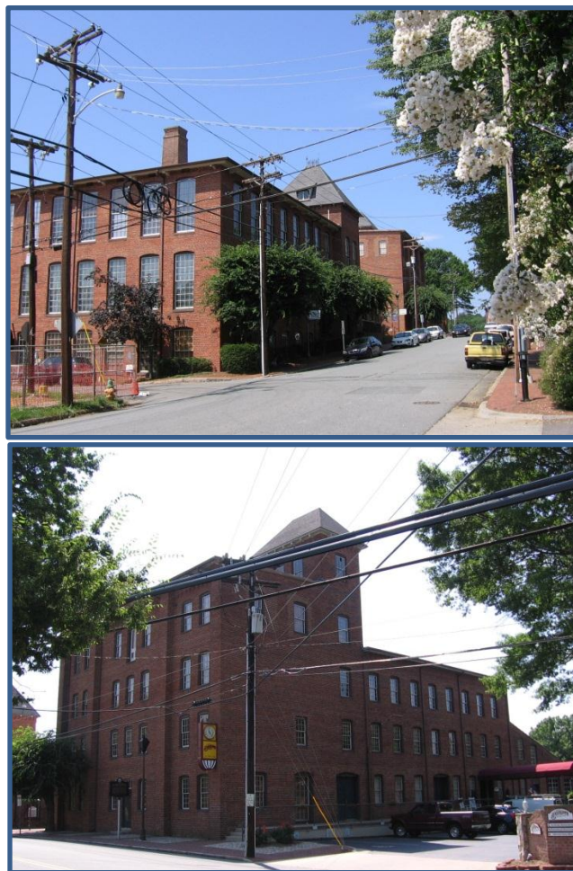
Figure 26. Property No. 81 – Arista Cotton Mill. Looking west along Brookstown Avenue (1880 building in foreground, above) and north and west elevations of the 1836 building (below).
