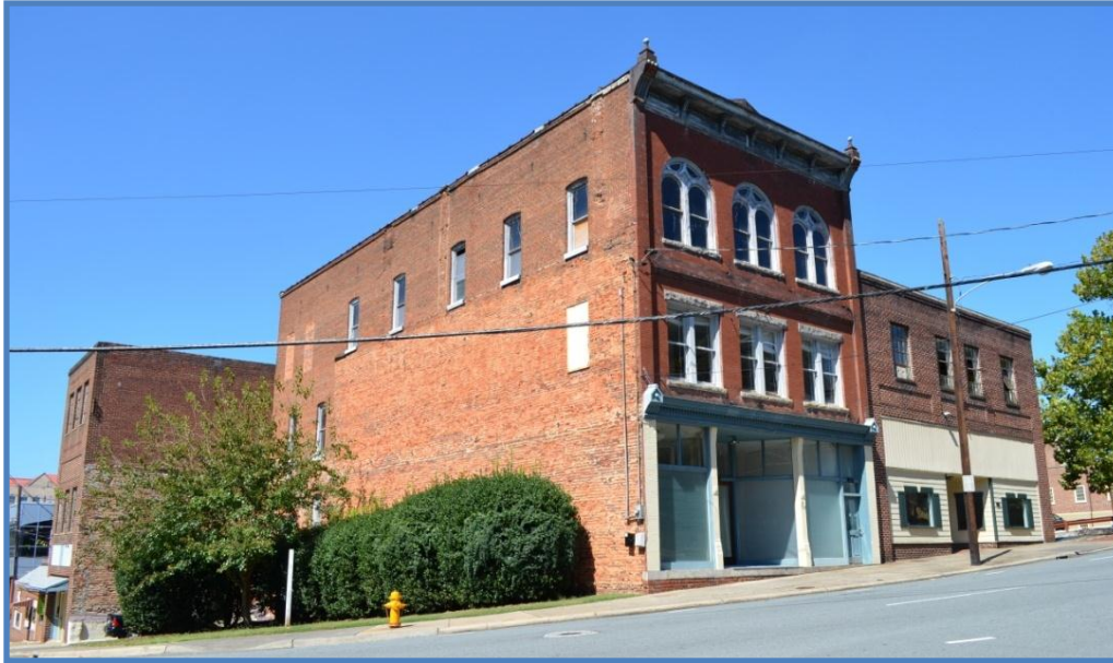
Figure 14. Brookstown Avenue and South Main Street intersection, looking northwest. Property No. 88 (326-328 South Main Street, at left) and Property No. 89 (330-332 South Main Street, at right) in the foreground. (HF)
