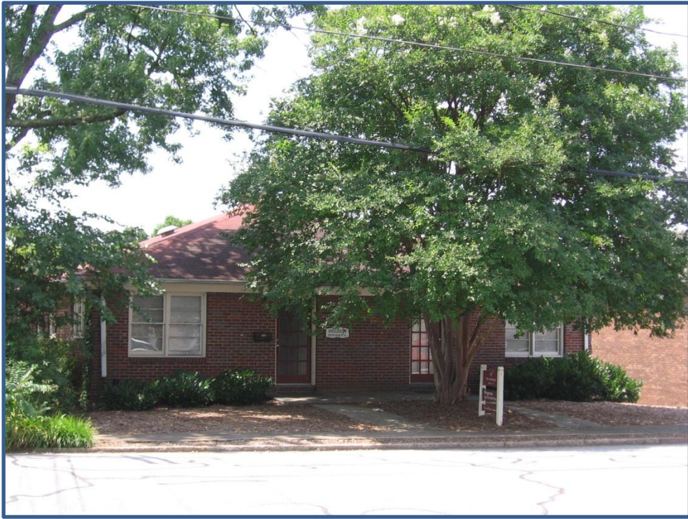
Figure 57. Property No. 128 – Commercial Building, 120-122 Fayette Street.
