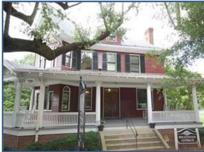
Figure 28. Property No. 82 – Brickenstein-Leinbach House. Main (east) elevation.
