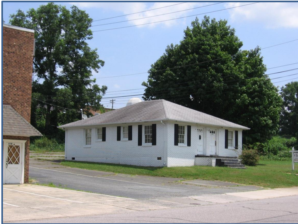
Figure 59. Property No. 130 – Commercial Building, 119-121 Fayette Street.
