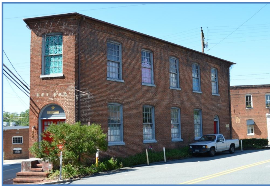
Figure 13. Property No. 78 - Fries Manufacturing and Power Company Transforming Station, 300 Brookstown Avenue, 1898. Northeast oblique. (HF)
