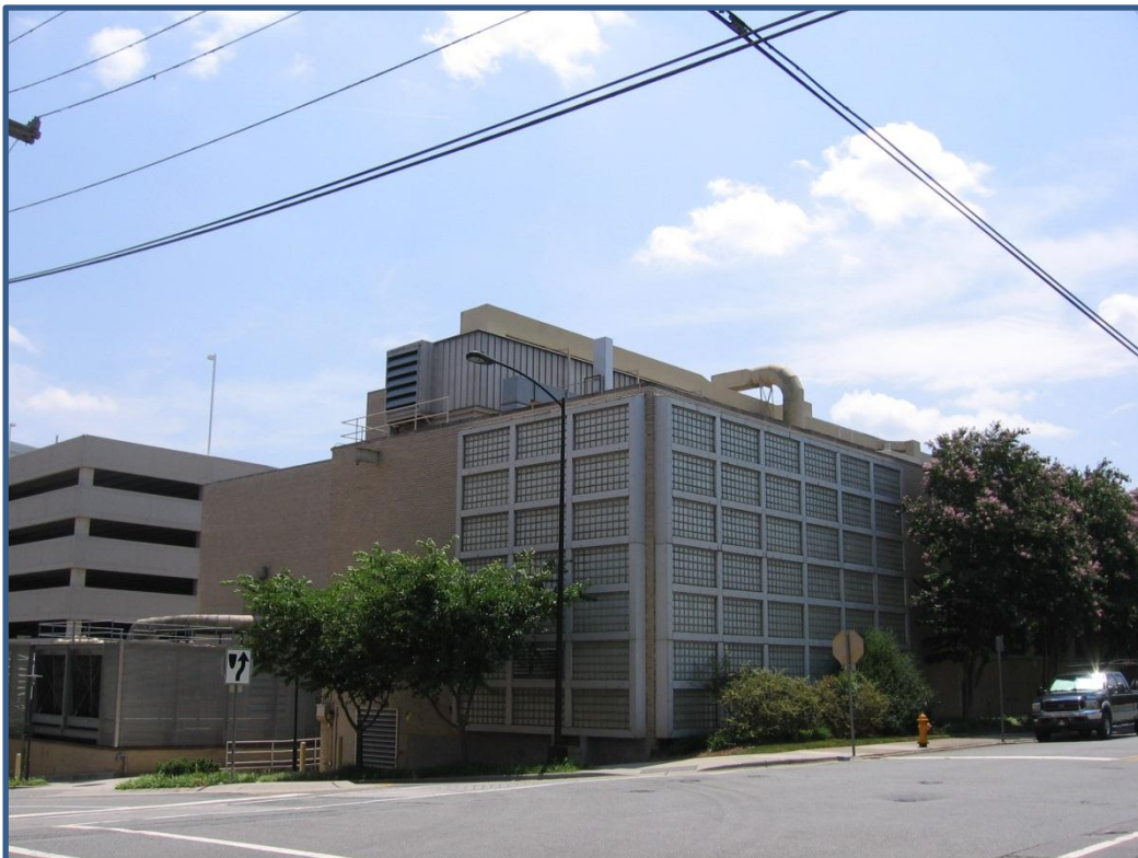
Figure 56. Property No. 127 - Commercial Building, 115 South Chestnut Street.
