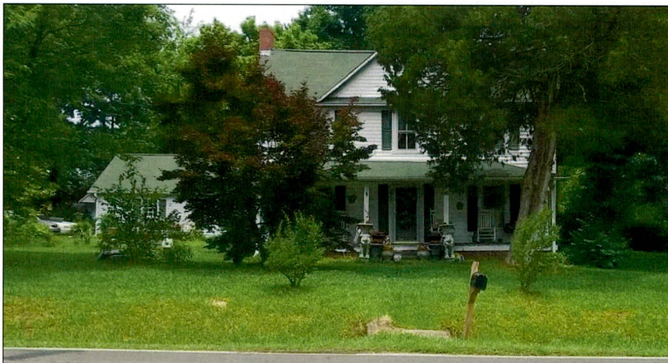
Photo 10: Façade or South Elevation, A.C. and Helon Council House.
