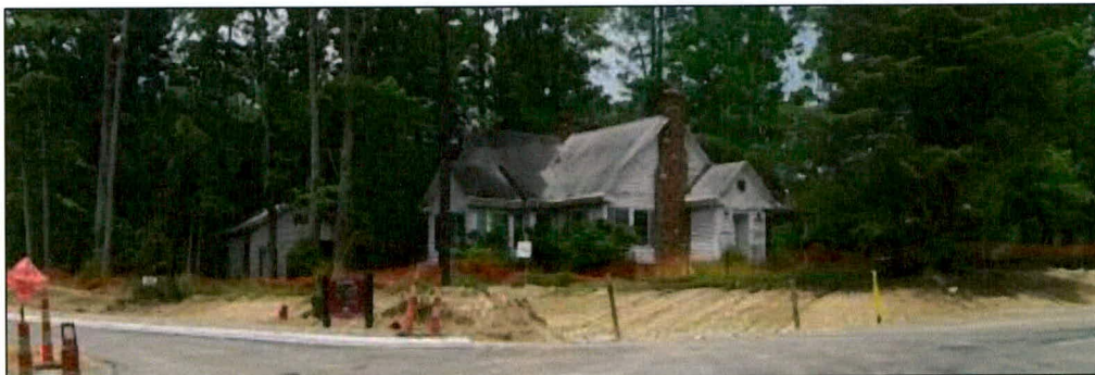
Photo 13: View of Kenneth and Reba Mills House, Looking Northwest.
