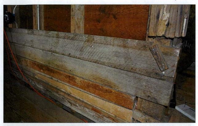
a. Original Circular Sawn Weatherboards on North Side, Now Inside Shed Addition
