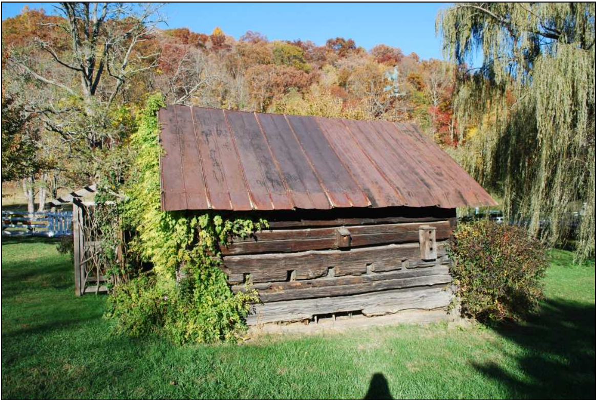
Log shed, looking north.
