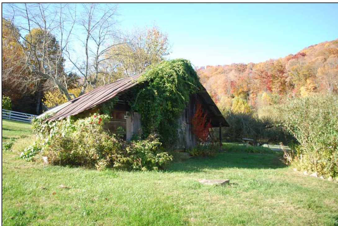
Frame shed west of house.
