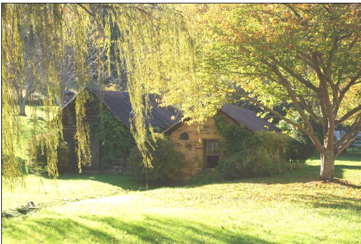
Log Shed and Stone Springhouse, looking west.
