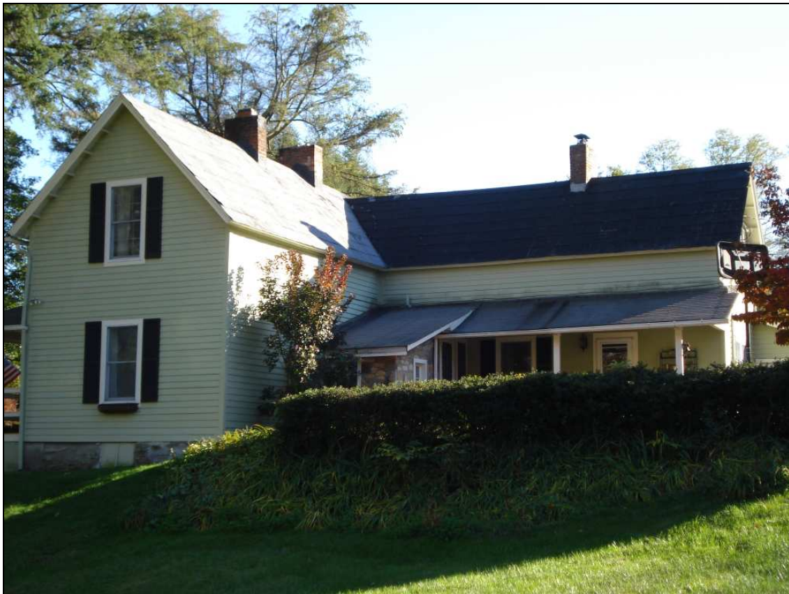
John A. Plott House, north elevation.
