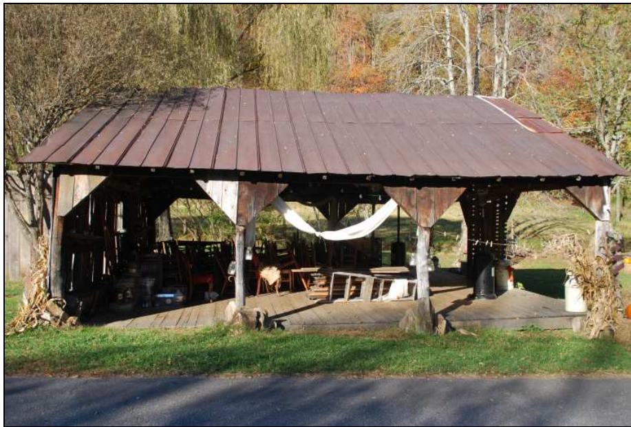
Corncrib, looking north.
