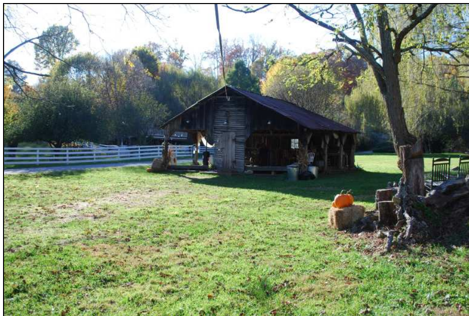
Corncrib, looking west.
