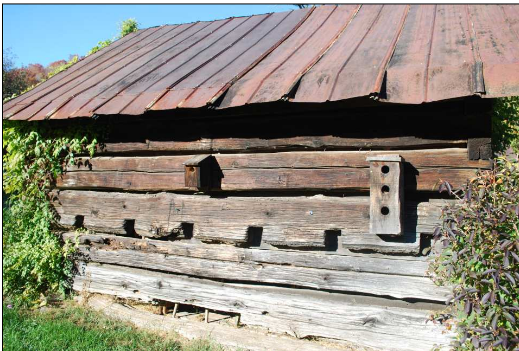
Detail of log shed, south elevation.
