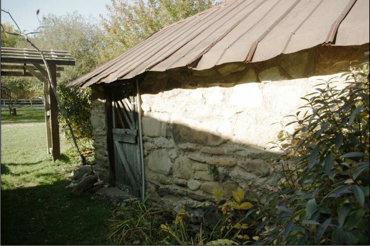
Entrance to Springhouse on south elevation.
