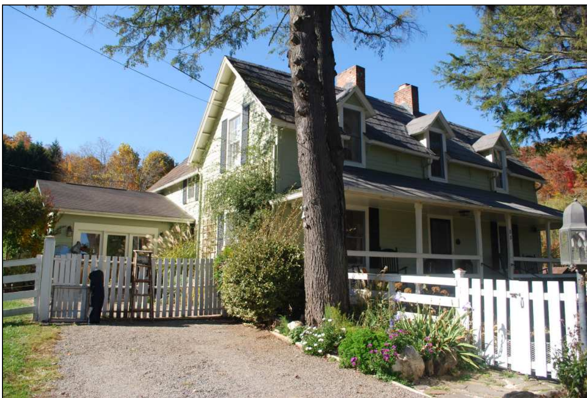
John A. Plott House, looking northwest.
