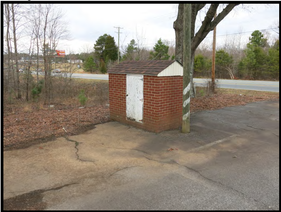
Figure 86: Berea Baptist Church (# 111),Well House (ca. 1961), Looking Northwest.
