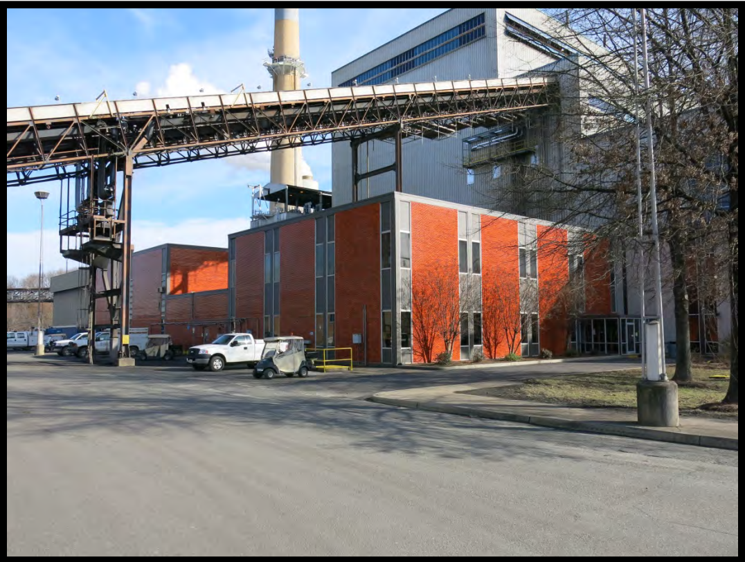
Figure 67: Marshall Steam Station (# 99), Office Building (No. 1), Looking Southeast.
