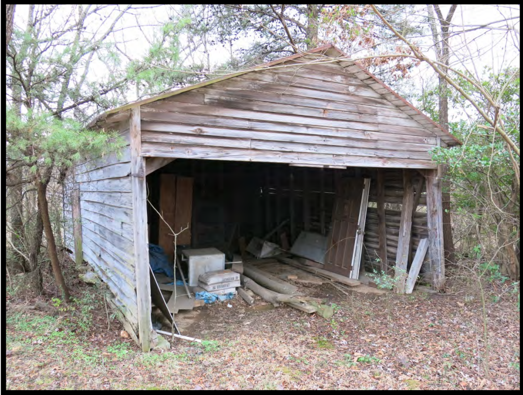
Figure 16: Sherrill-Gabriel House (# 63), Garage, Looking South.
