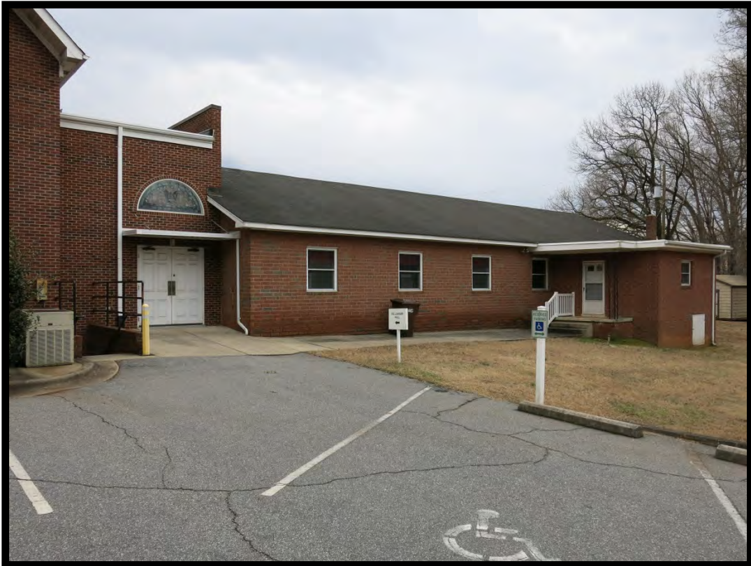
Figure 44: Rehobeth Methodist Church (#s 93 & 94), Fellowship Hall (ca. 1960), Looking Southeast.
