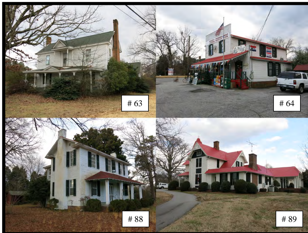
Figure 10: “Pivotal” Buildings of the Terrell Historic District.
