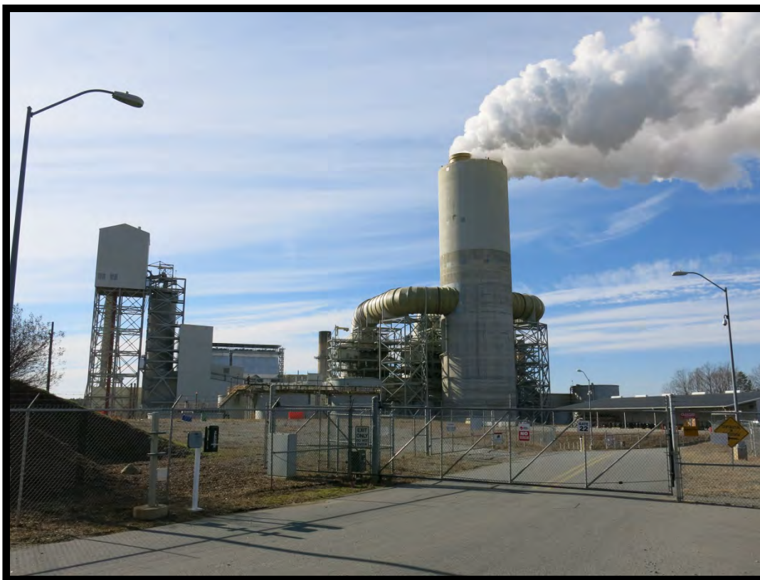
Figure 69: Marshall Steam Station (# 99), Scrubber Elements (No. 3), Looking West.
