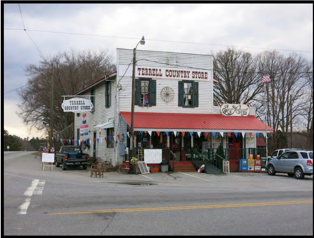
Figure 19: Connor Store and Post Office (# 64) (ca. 1891), Looking West.
