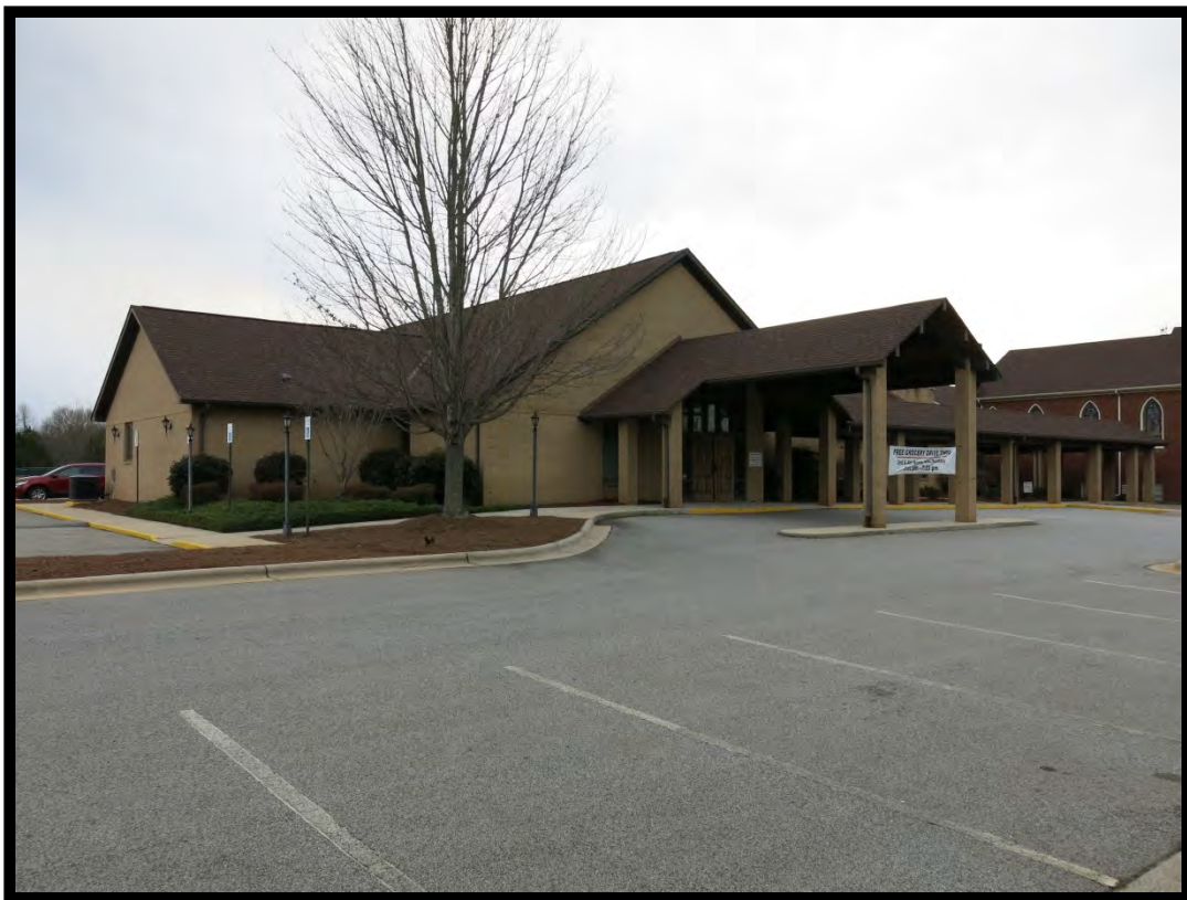
Figure 81: Berea Baptist Church (# 111), New Education Building & Fellowship Hall (ca. 1996), Looking Southwest.
