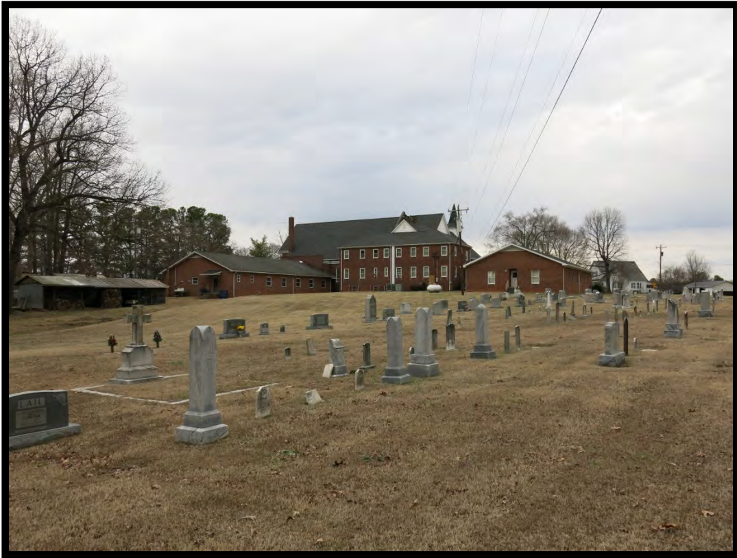
Figure 43: Rehobeth Methodist Church (#s 93 & 94) (1889, ca. 1955), Looking Northwest.
