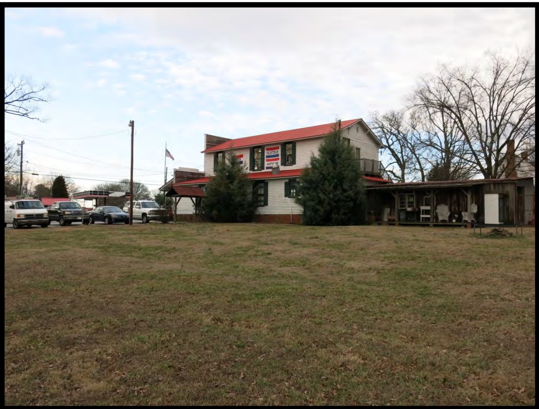
Figure 20: Connor Store and Post Office (# 64) (ca. 1891), Looking East.
