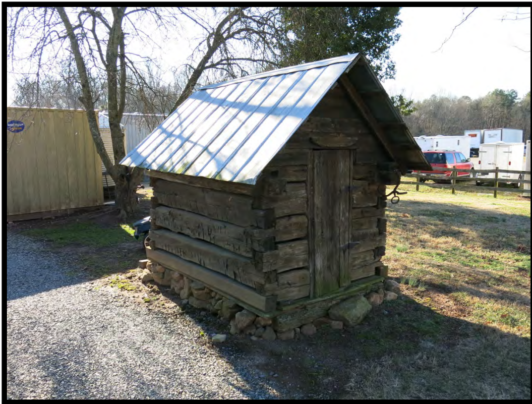
Figure 110: Johnson-Neel House (#123), Log Outbuilding (No. 7), Looking South.
