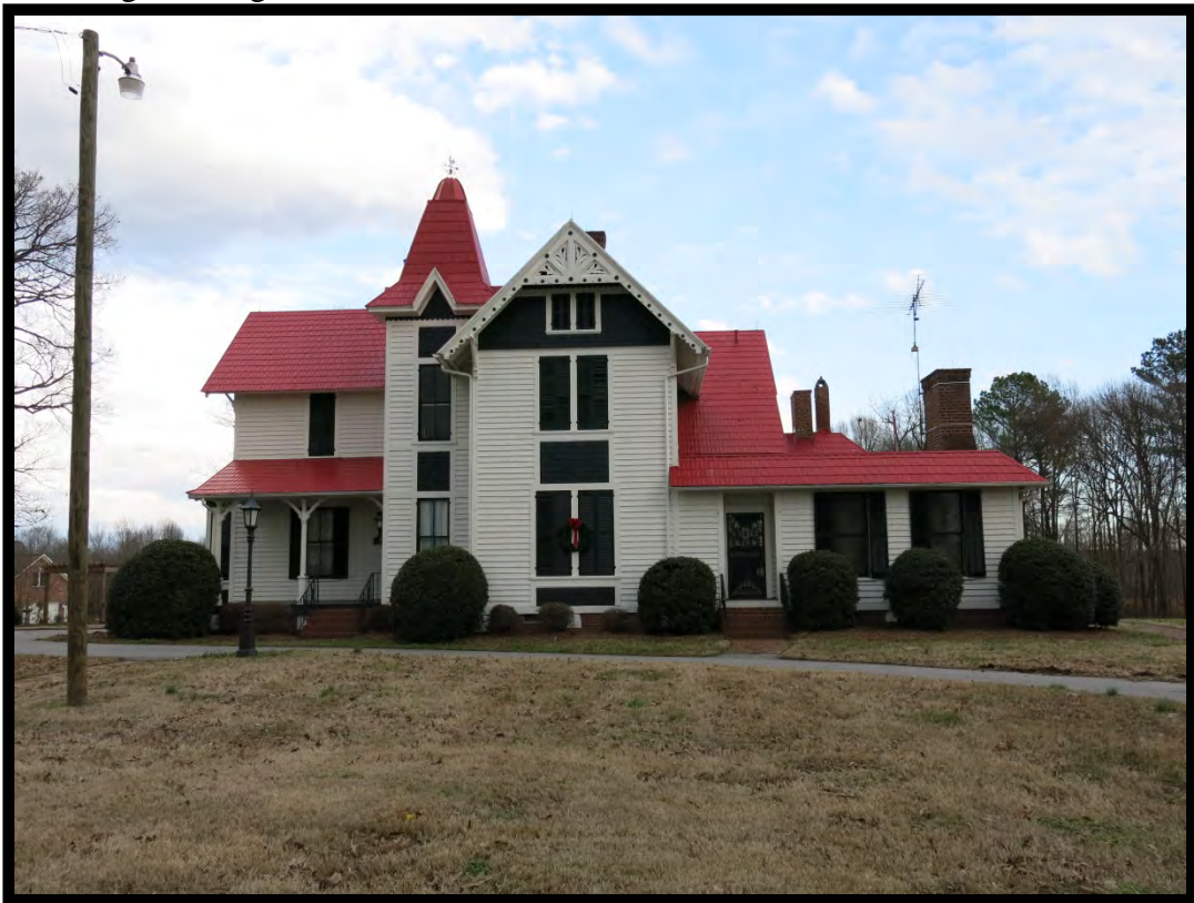
Figure 57: T. F. Connor House (# 89) with One-story Addition to the Right.
