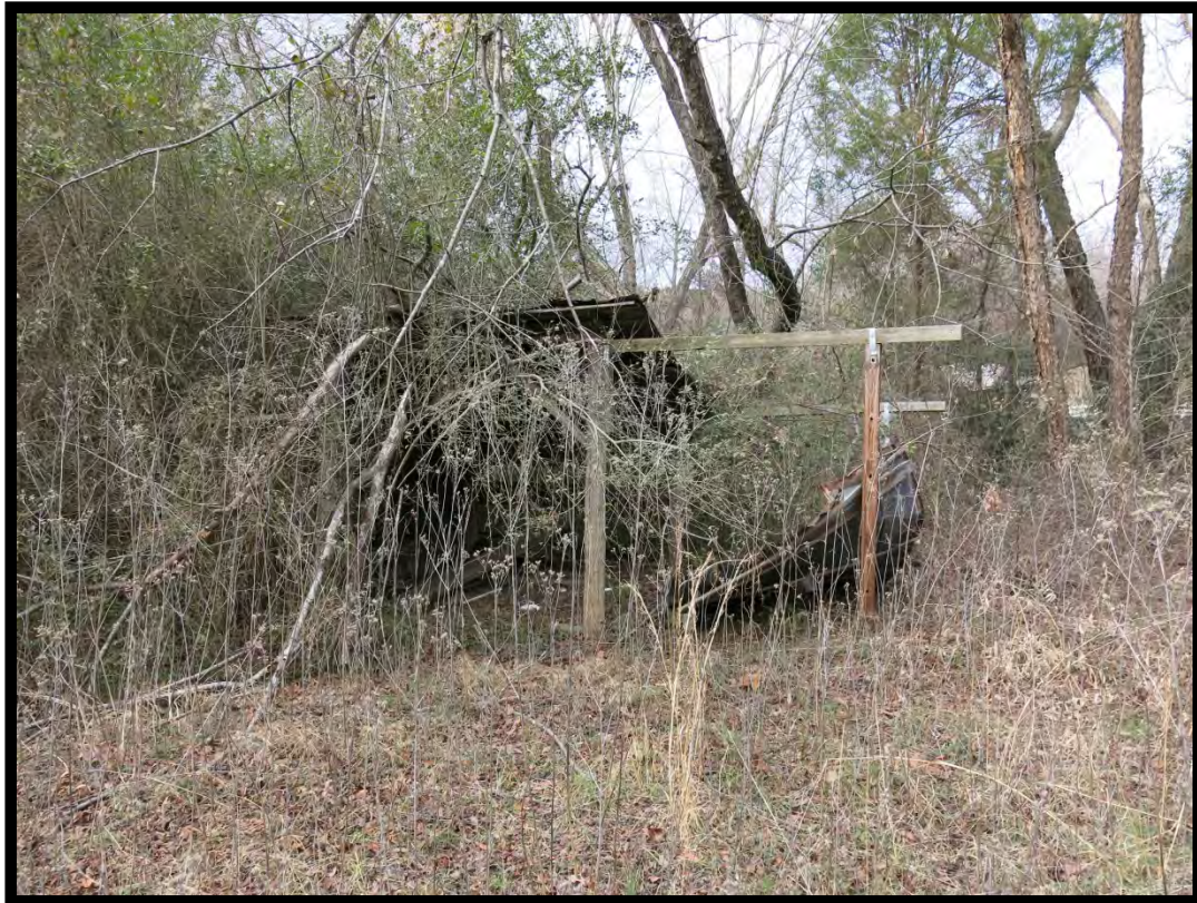
Figure 25: Jason Sherrill House (# 71/72), Shed, Looking North.
