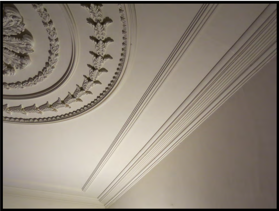
Figure 96: Johnson-Neel House (#123), Interior: Detail of Medallion and Molded Plaster Cornice in Northwest Room.
