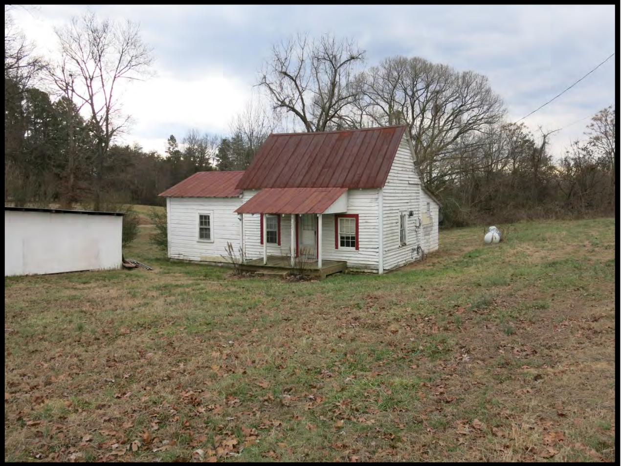
Figure 18: Sherrill-Gabriel House (# 63), R. E. Gabriel's carpenter shop (# 90), Looking Southwest.
