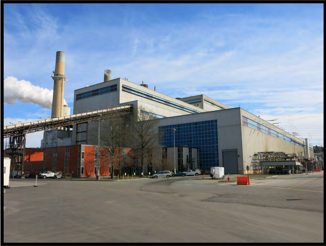
Figure 66: Marshall Steam Station (# 99), Main Building (No. 2), Looking Southeast.
