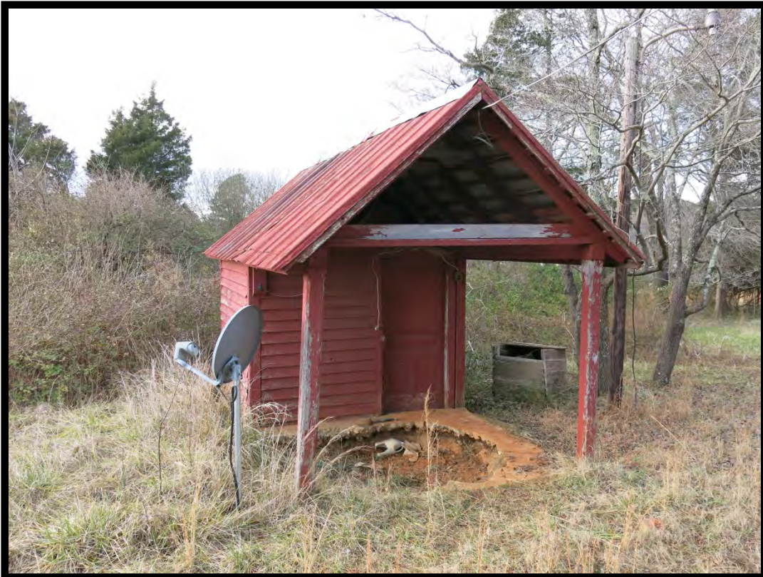
Figure 33: Coleman-Caldwell-Gabriel Farm (# 88), Well House, Looking Northwest.
