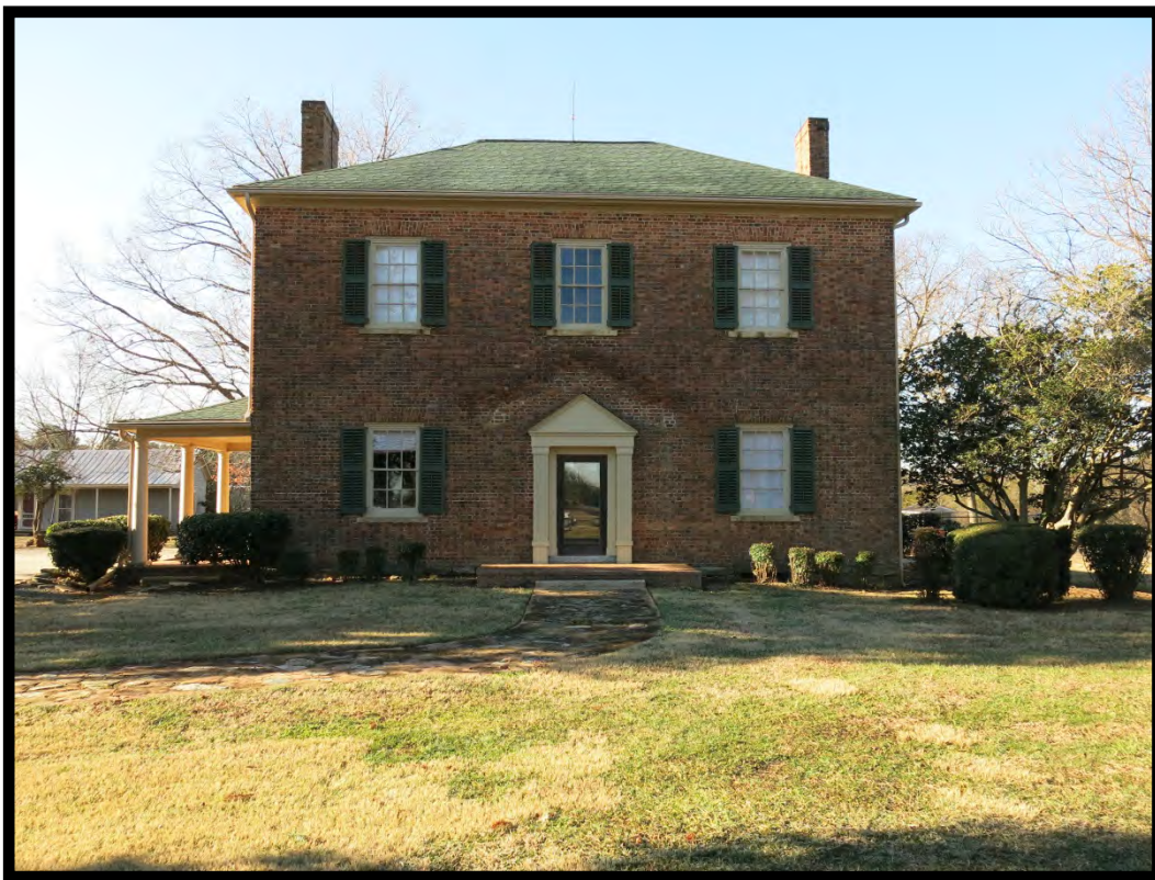
Figure 91: Johnson-Neel House (#123), Looking Southwest.
