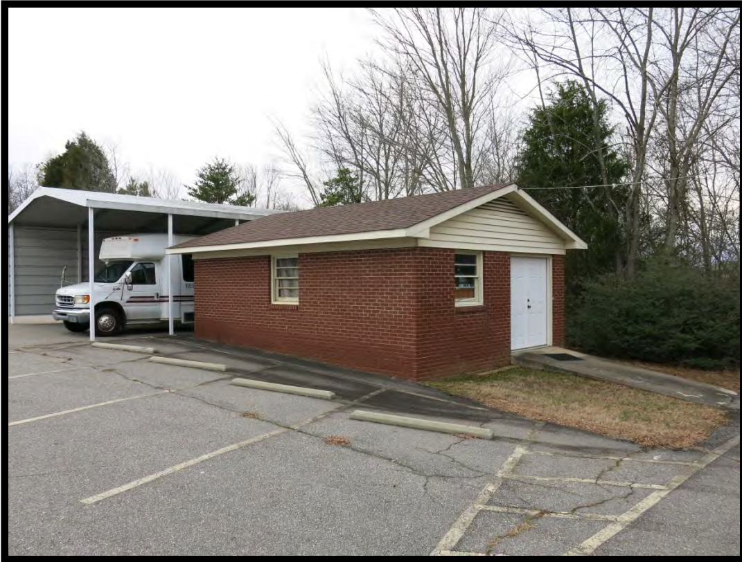
Figure 87: Berea Baptist Church (# 111),Garage/Workshop (ca. 1961) and Modern Carport (ca. 1990), Looking Southwest.
