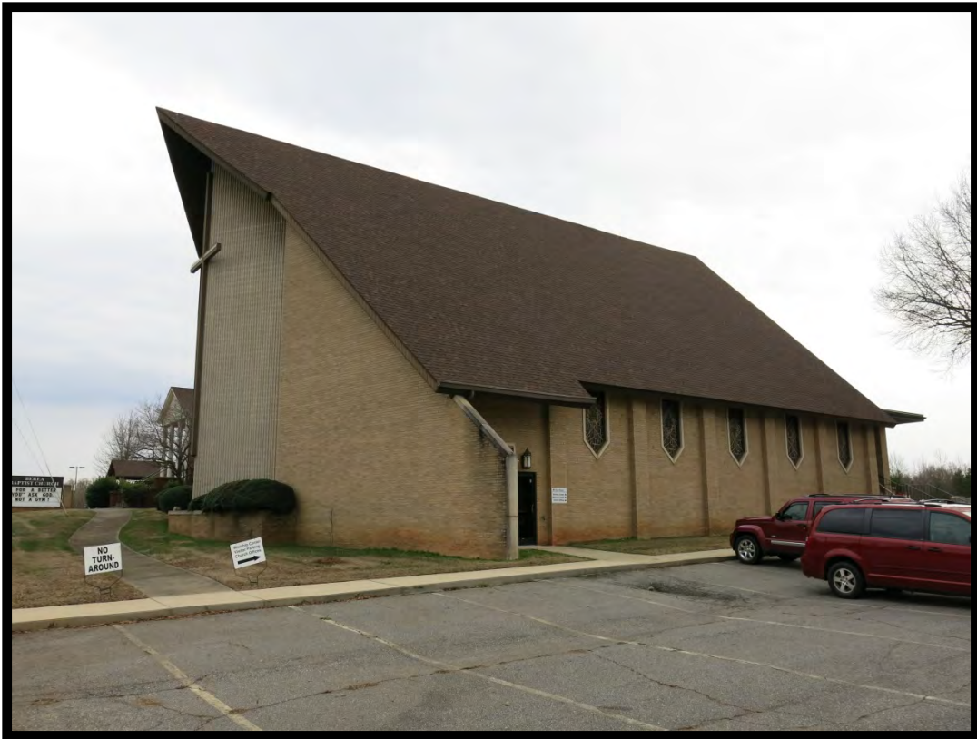
Figure 79: Berea Baptist Church (# 111), New Sanctuary (1979), Looking Southeast.
