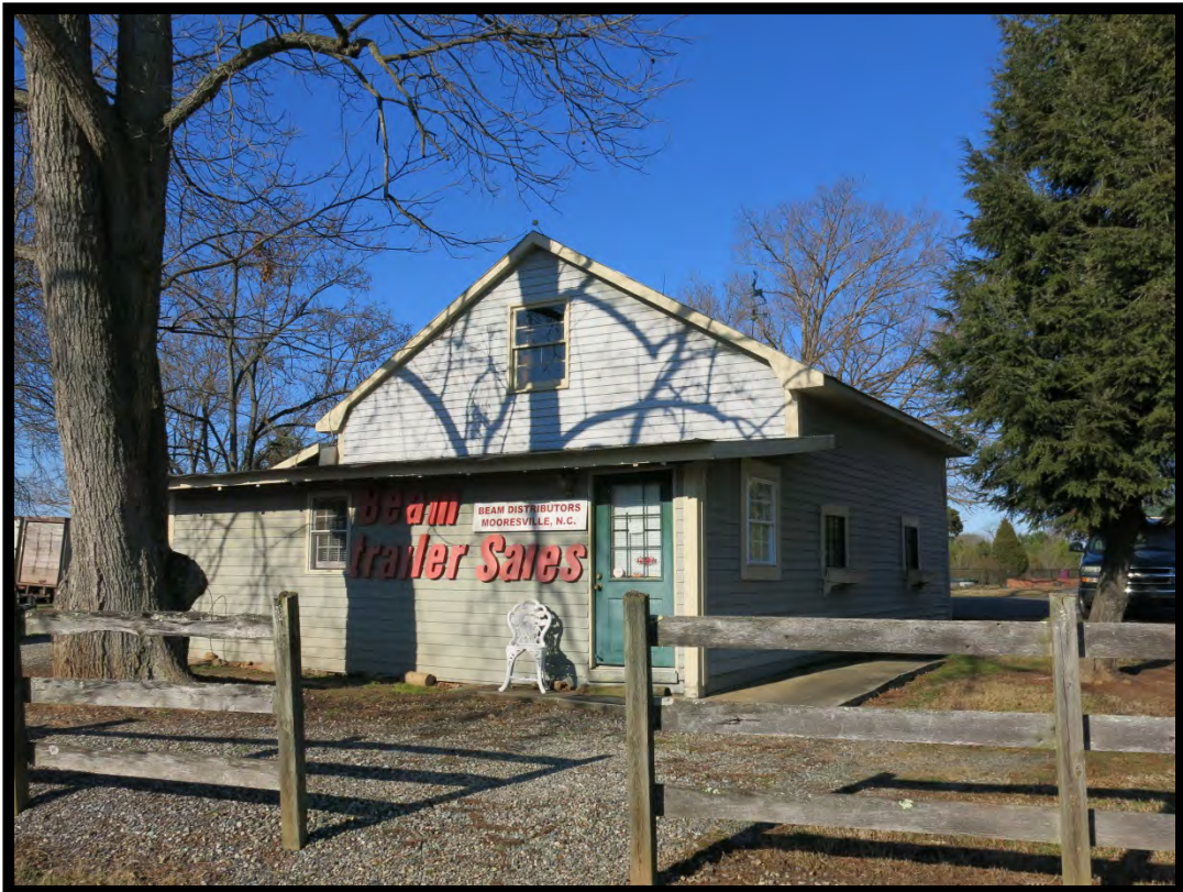
Figure 109: Johnson-Neel House (#123), Barn/Office (No. 8), Looking West.
