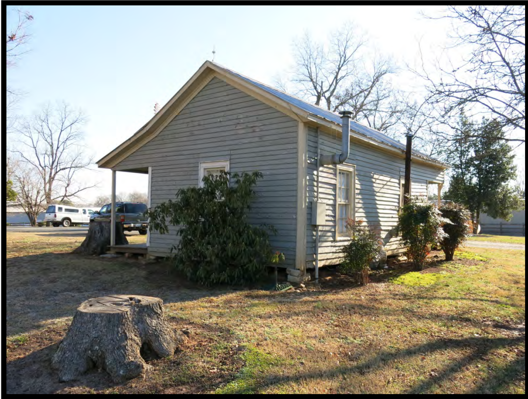
Figure 107: Johnson-Neel House (#123), Summer Kitchen, Looking East.
