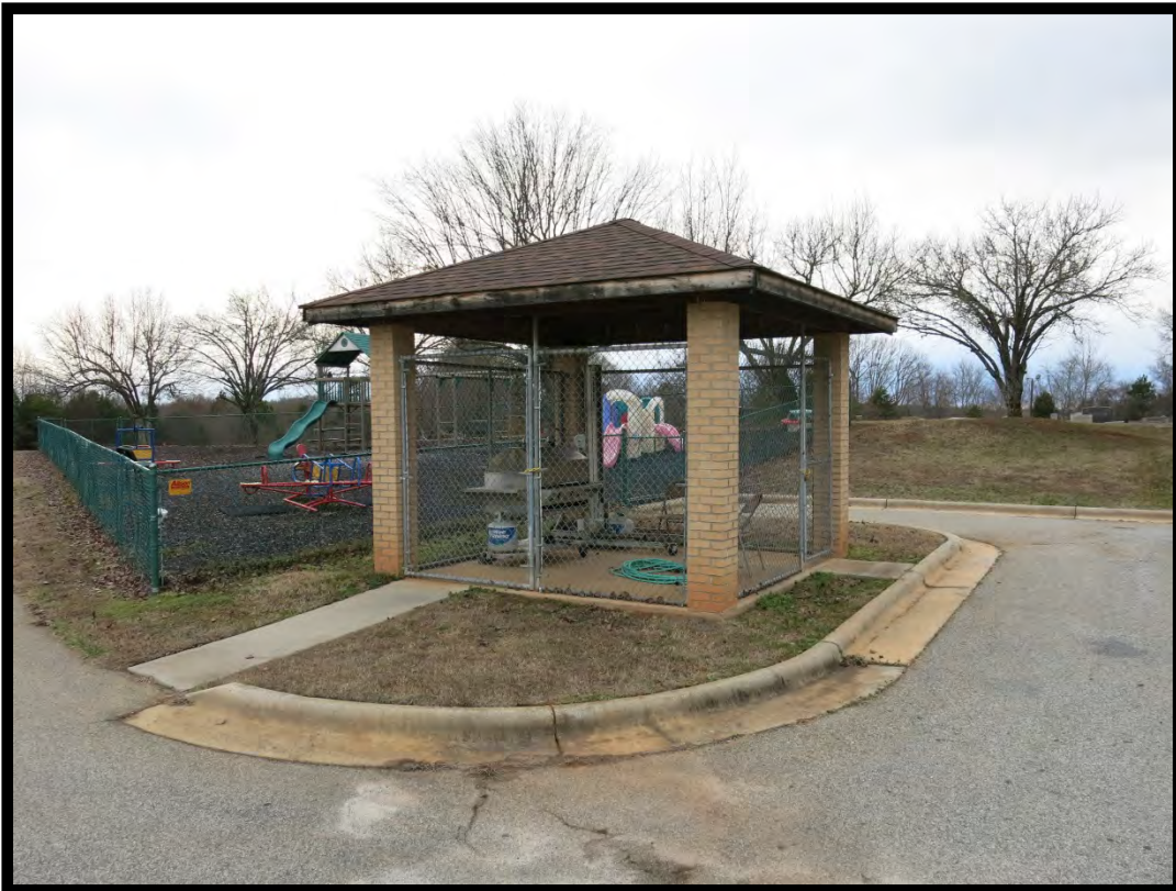
Figure 88: Berea Baptist Church (# 111), Picnic Shelter (ca. 1996), Looking Southwest.
