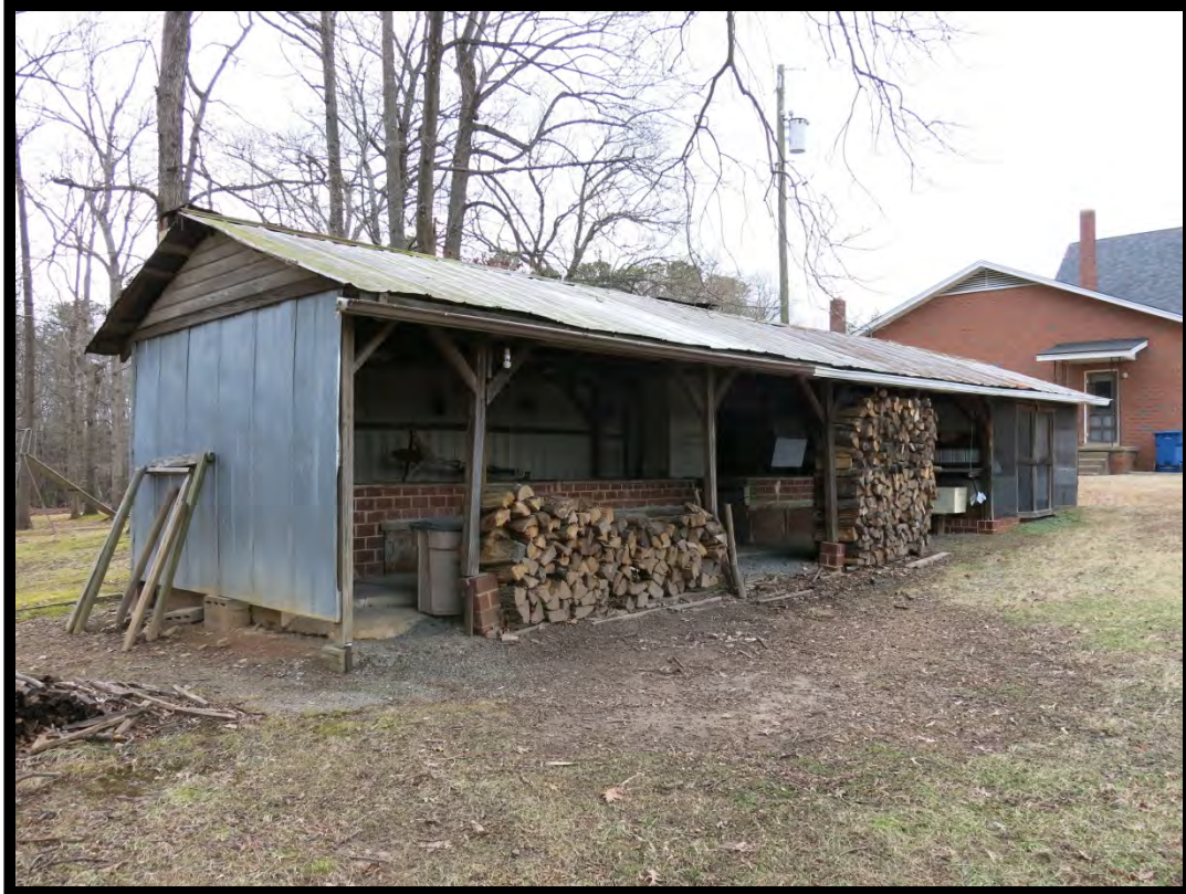
Figure 46: Rehobeth Methodist Church (#s 93 & 94), Picnic Shelter, Looking Northwest.
