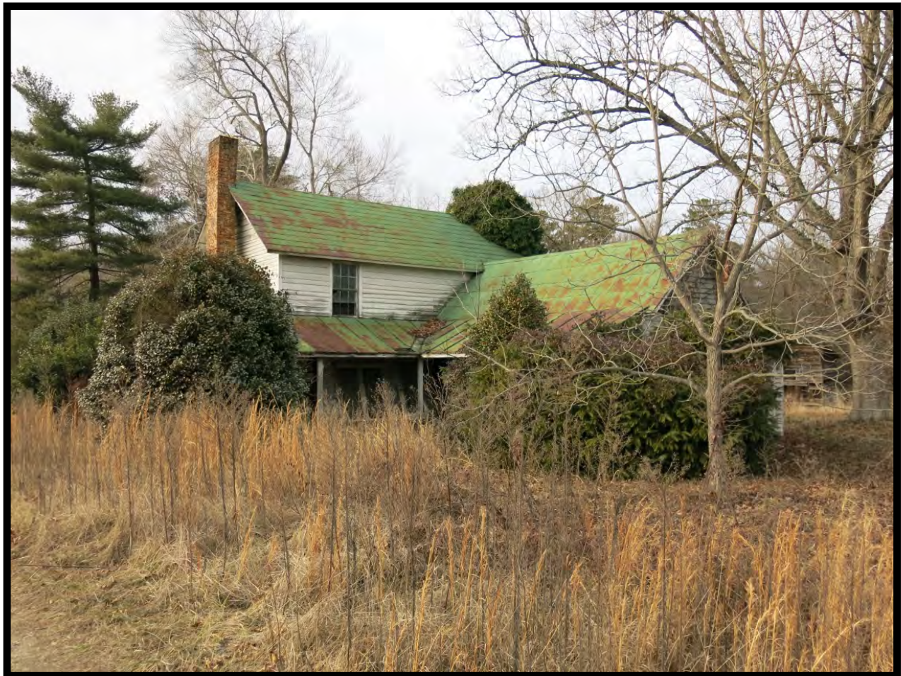
Figure 22: Jason Sherrill House (# 71/72) (ca. 1890 & 1930), Looking North.
