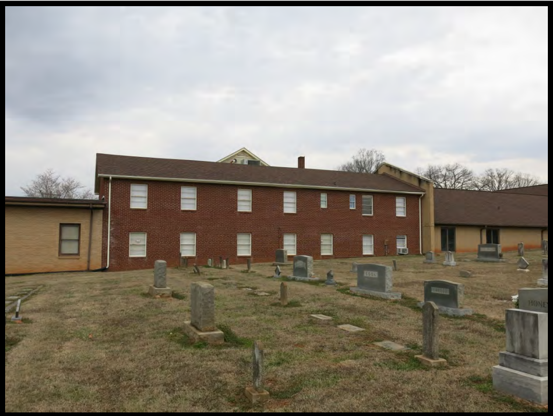
Figure 78: Berea Baptist Church (# 111), Sunday School/office wing, Looking Northeast.
