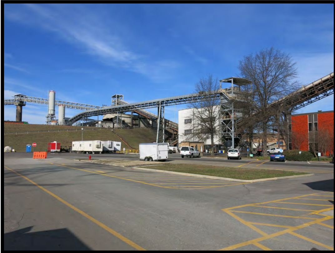
Figure 68: Marshall Steam Station (# 99), Coal Conveyor System Located Northwest of the Station, Looking North.
