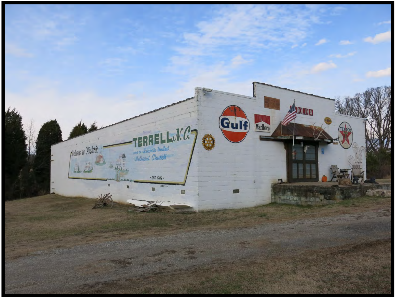
Figure 12: Cinderblock Warehouse (# 62) (ca. 1940), Looking Northeast.
