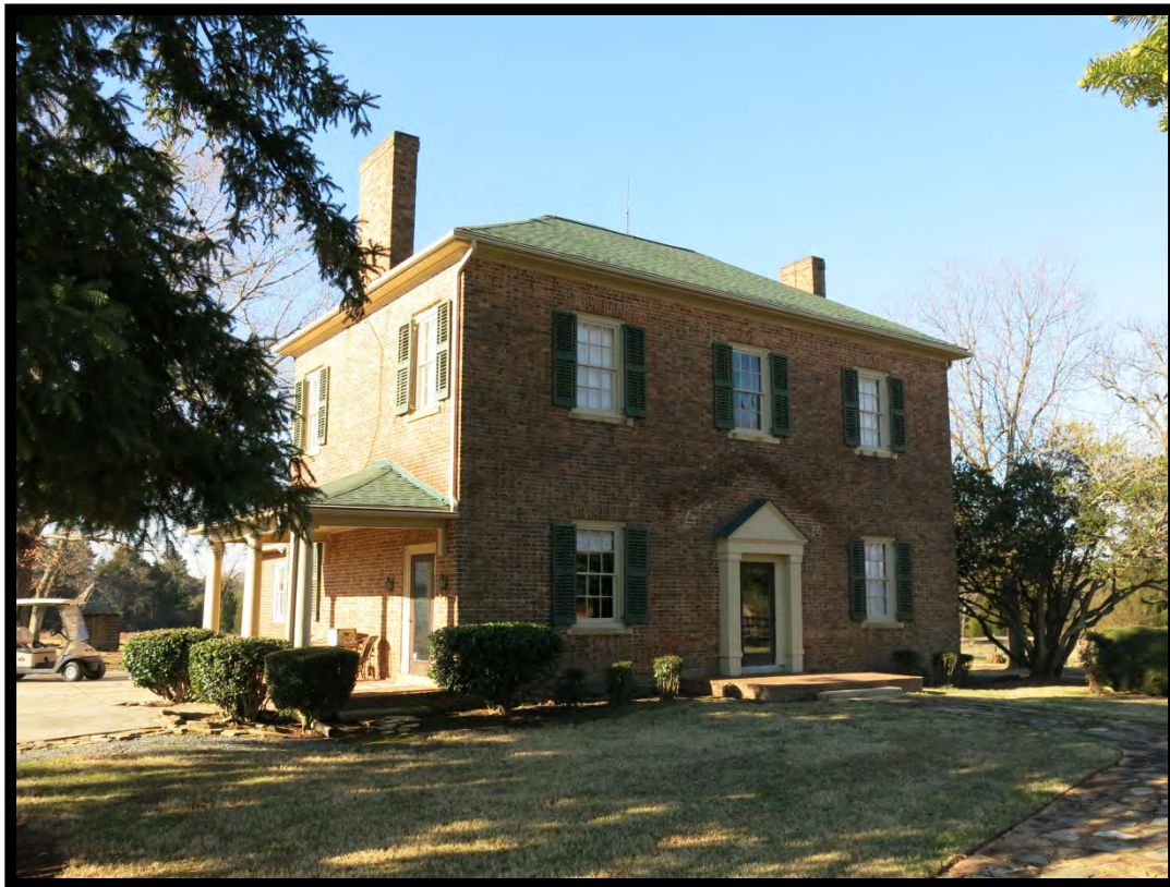
Figure 93: Johnson-Neel House (#123), Looking Southwest.
