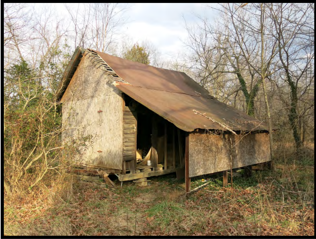
Figure 24: Jason Sherrill House (# 71/72), Former Kitchen, Looking Northeast.
