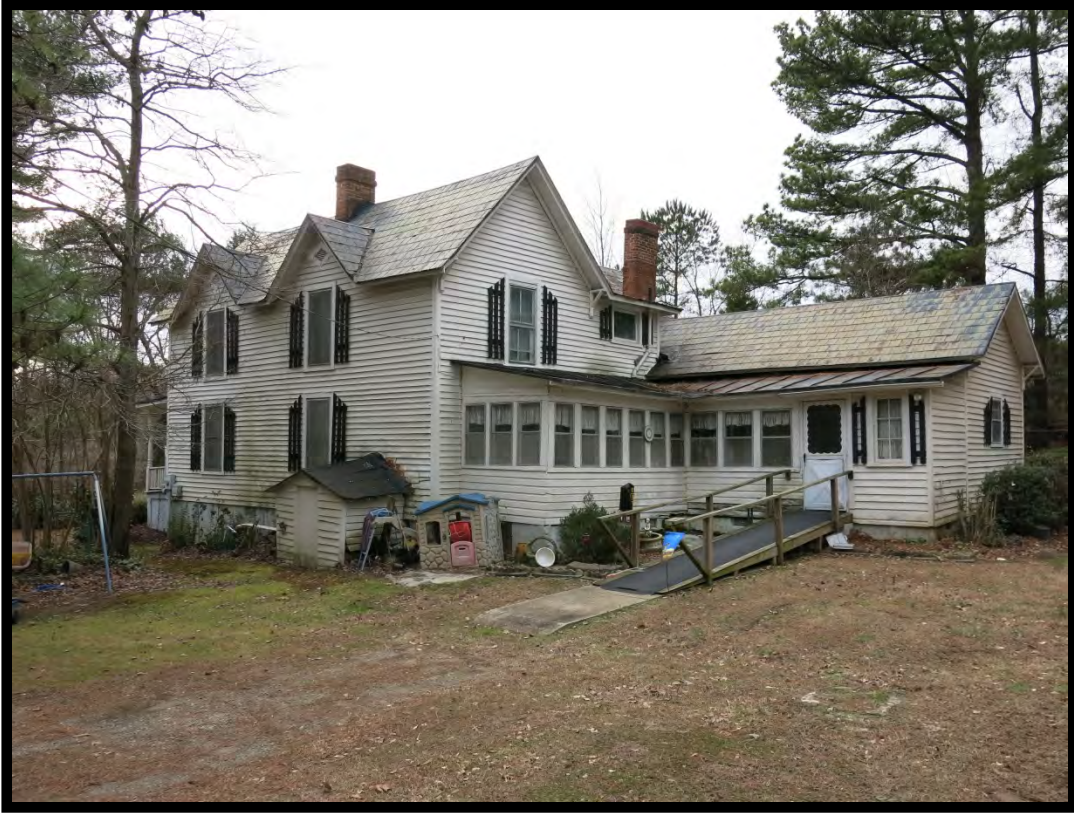
Figure 52: James Gillin House (# 98) (ca. 1908), Looking Southwest.
