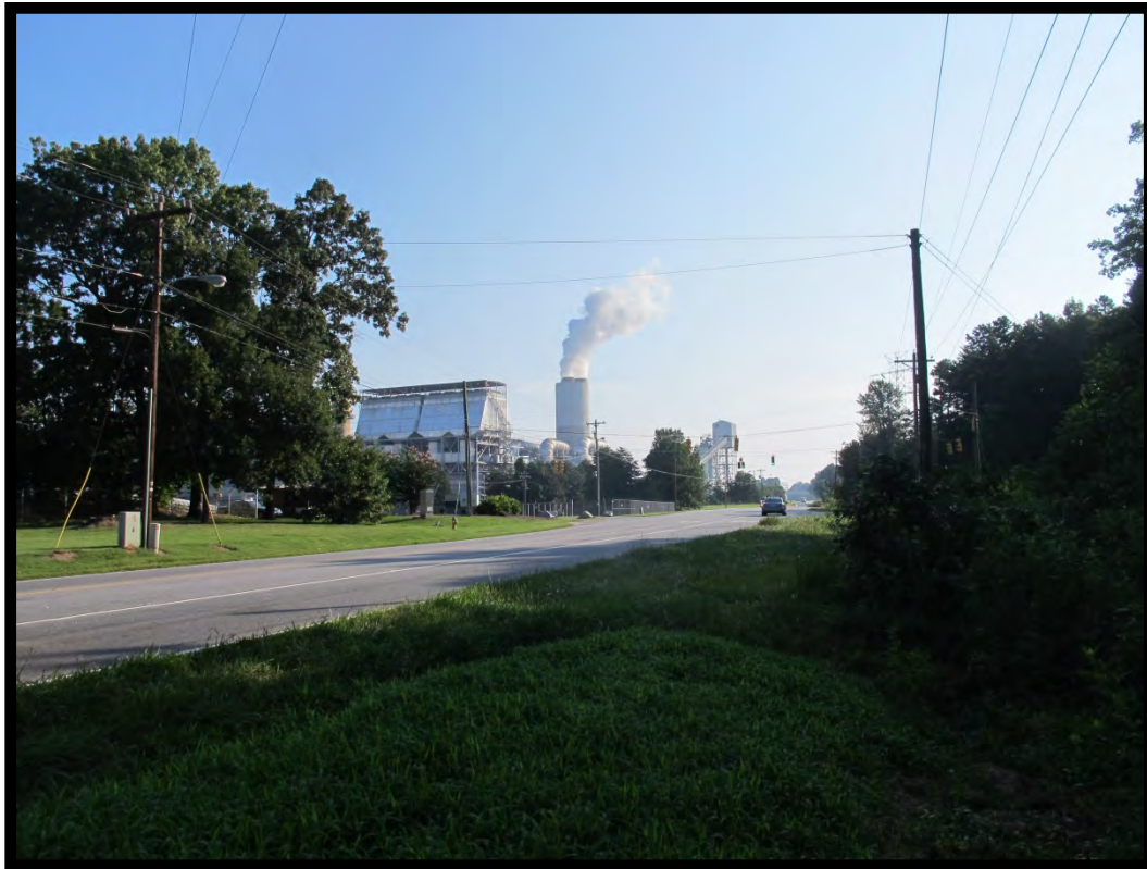
Figure 64: Marshall Steam Station (# 99), Looking Northeast.
