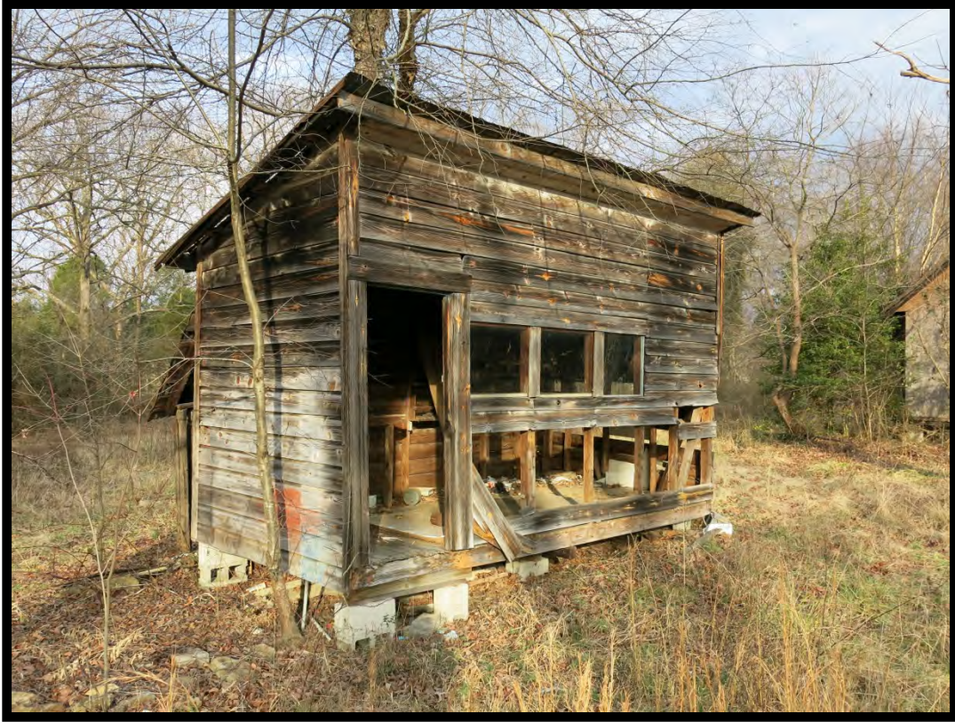
Figure 26: Jason Sherrill House (# 71/72), Chicken Coop, Looking Northeast.
