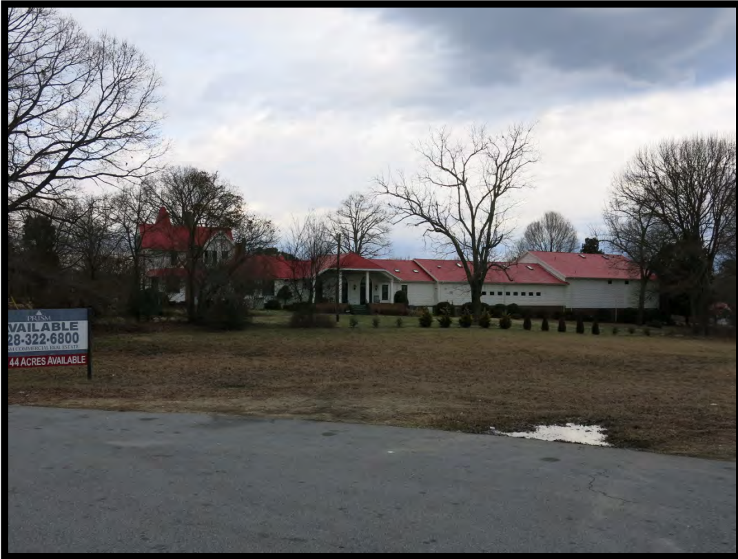
Figure 58: Addition to the T. F. Connor House (# 89), Looking North.
