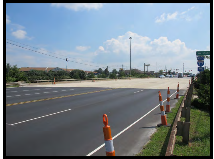
130 – Iredell County Bridge # 26 – 1967
