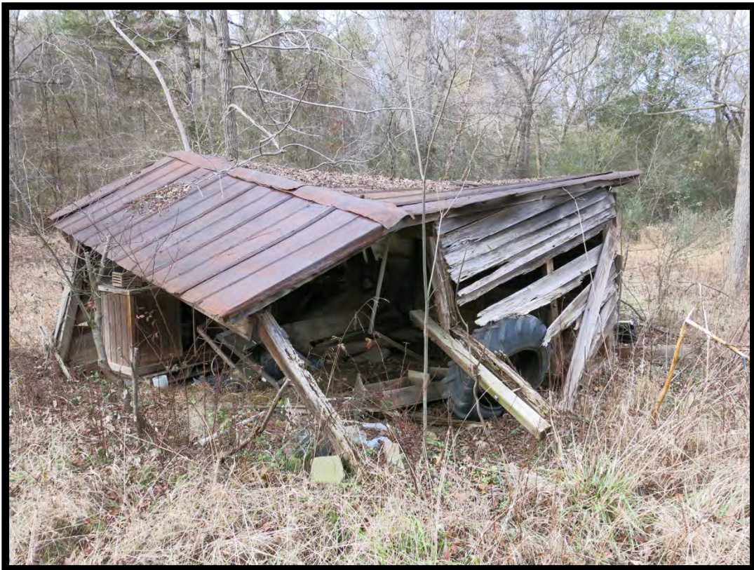
Figure 27: Jason Sherrill House (# 71/72), Wood Shed, Looking Northwest.
