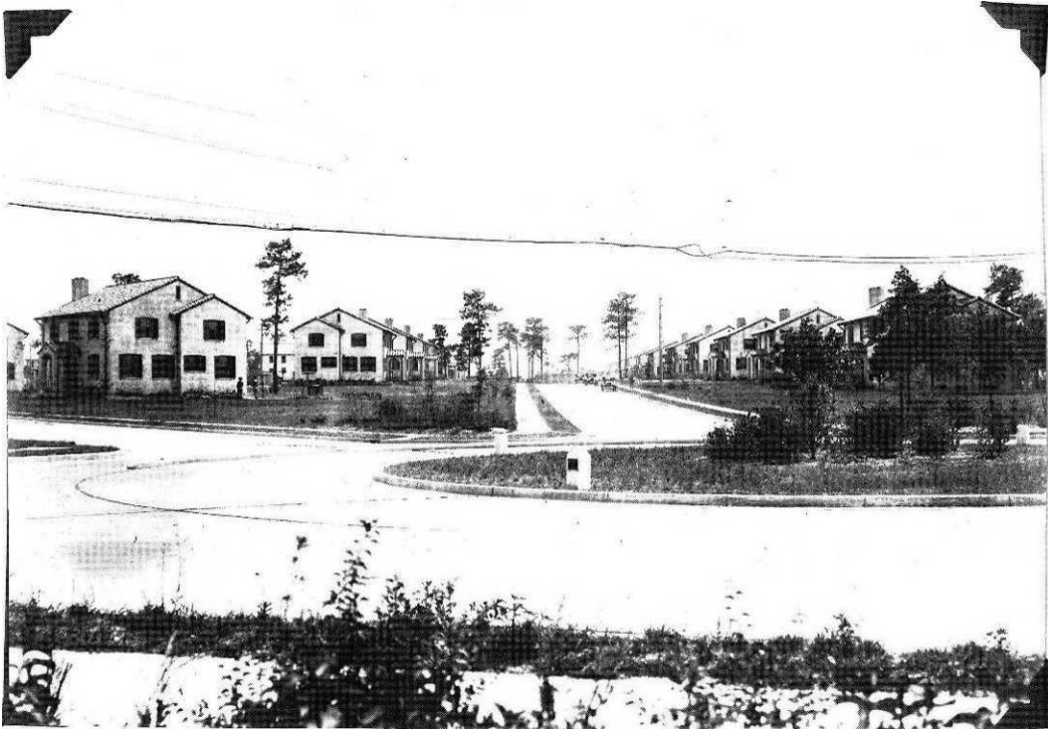
Figure 43. Field and company officers' quarters, looking south on Armistead Street, 1941 (Fort Bragg Cultural Resources).
