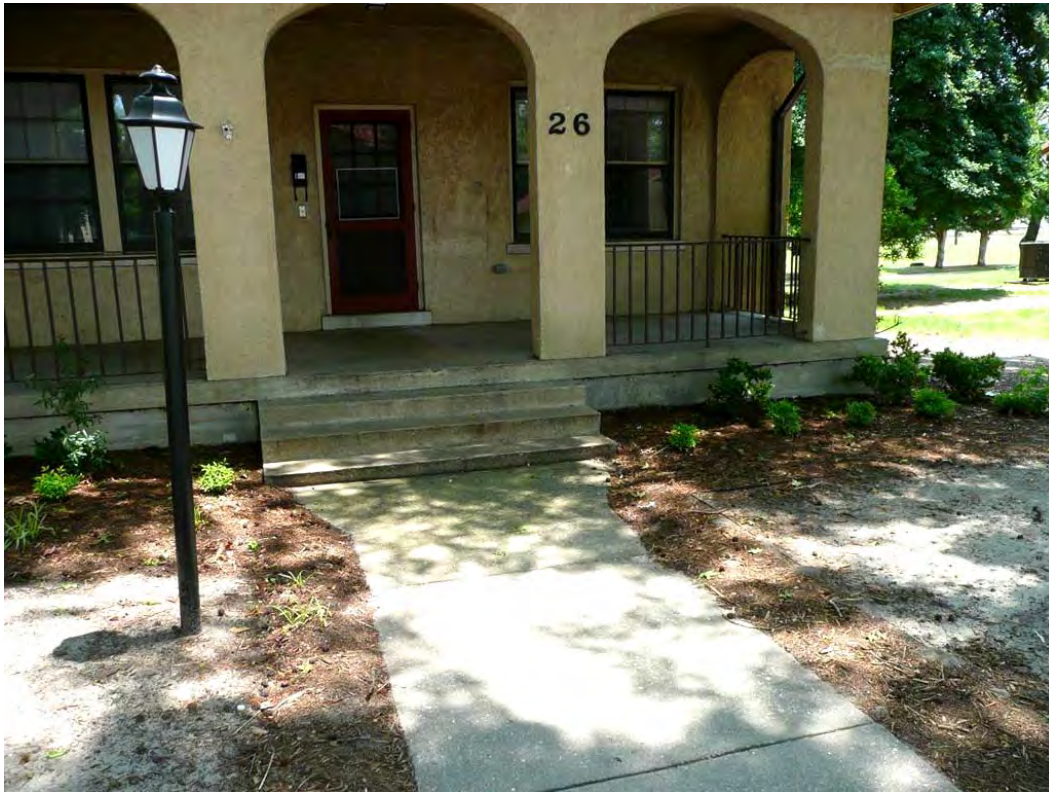
Figure 118. Bastogne Gables front plantings, 2009 (ERDC-CERL).
