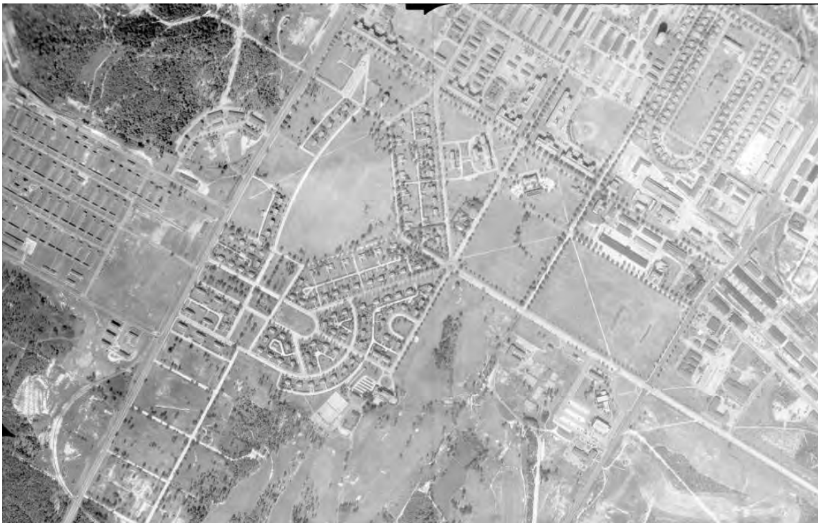
Figure 30. Aerial image of the OPHD, 1946 (Fort Bragg Cultural Resources).
