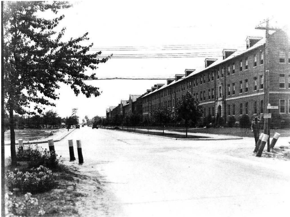
Figure 32. Street paving, combined curb and gutter, intersection of Randolph and Armistead, looking west, date unknown (NARA RG-77-391 Boxes 49-52).
