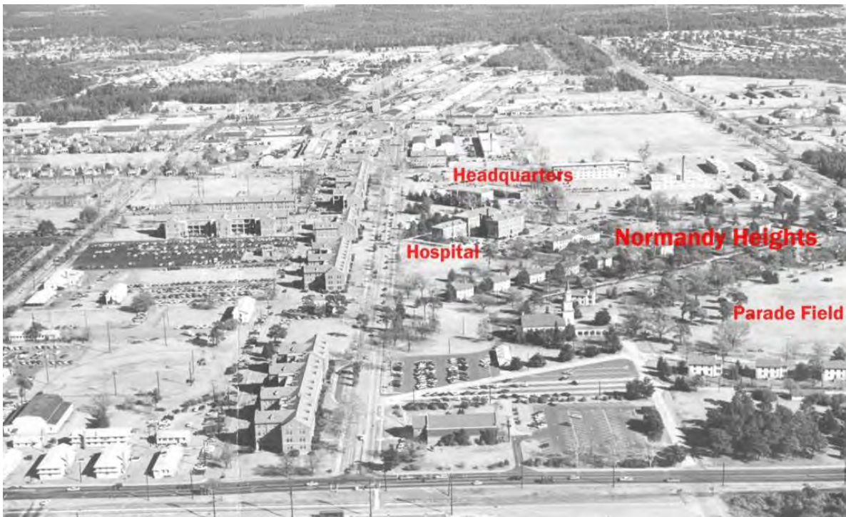
Figure 29. Relationship between Normandy Heights, the headquarters, and the hospital, 1968 aerial image looking east (Fort Bragg Cultural Resources).
