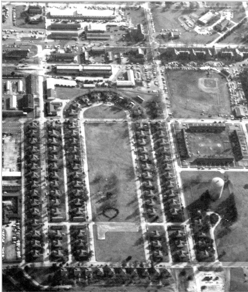
Figure 114. Aerial, looking south, of Bastogne Gables and Humphrey Plaza, 1968 (Fort Bragg Cultural Resources).
