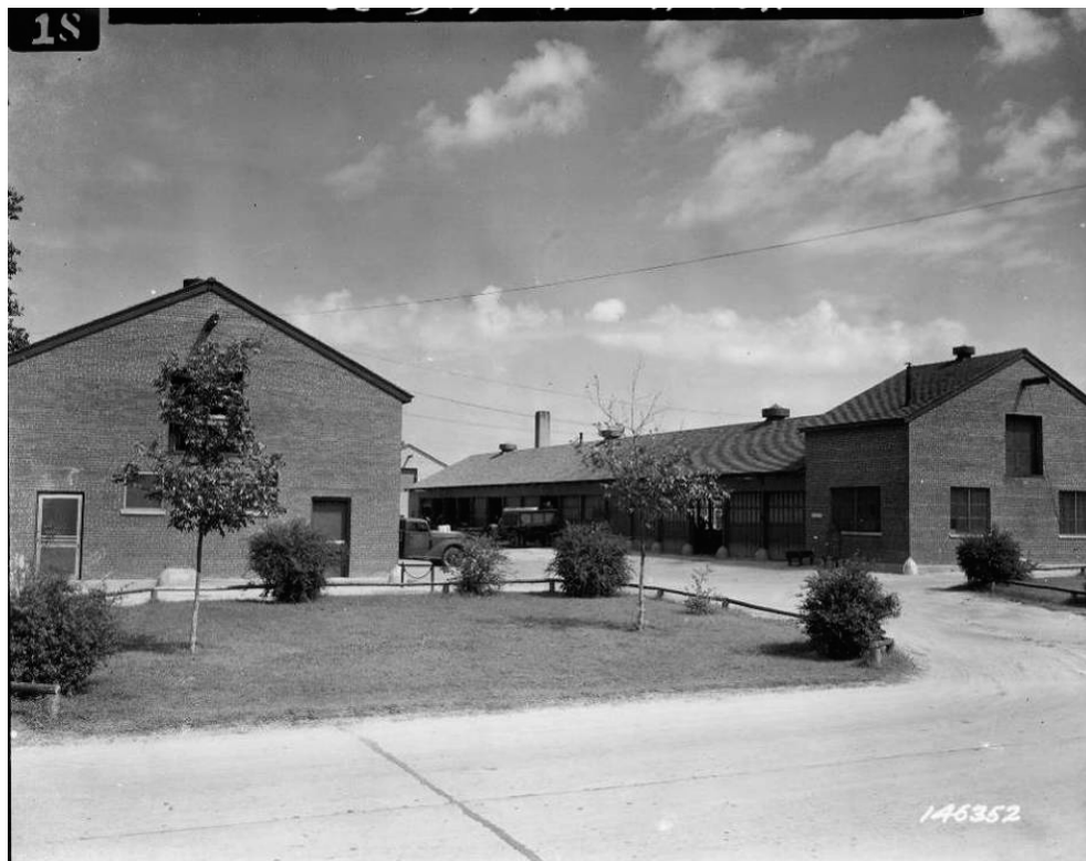
Figure 87. Former mule barns converted to the Motor Transport District, 1942 (NARA 111-SC box 92 146352).
