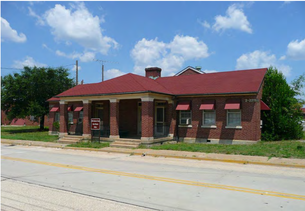
Figure 89. Former stable guard quarters now administrative space, 2009 (ERDC-CERL).
