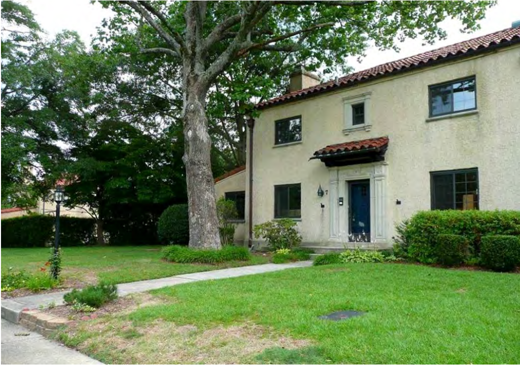
Figure 97. Normandy Heights duplex showing a variety of vegetation types, 2009 (ERDC-CERL).
