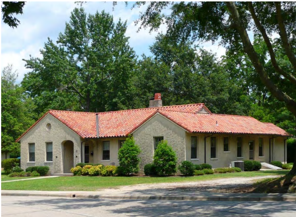
Figure 96. Normandy Heights ranch-style house type showing orderly foundation plantings, 2009 (ERDC-CERL).
