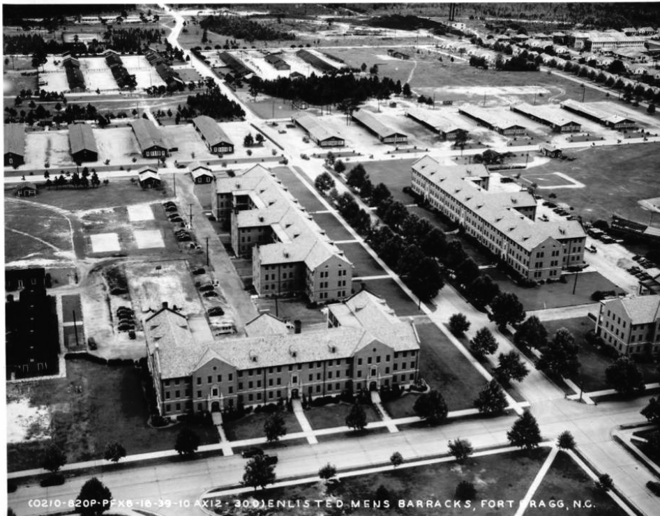
Figure 42. Aerial image of Enlisted Men's Barracks, 1939 (National Archives RG-342-FH-bx1060-B17348).
