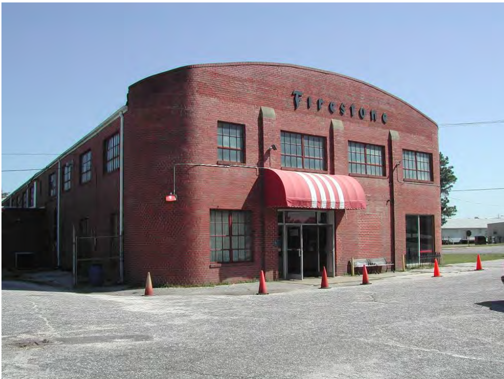
Figure 139. Former Firestone building in the industrial area, 2007 (Fort Bragg Cultural Resources).
