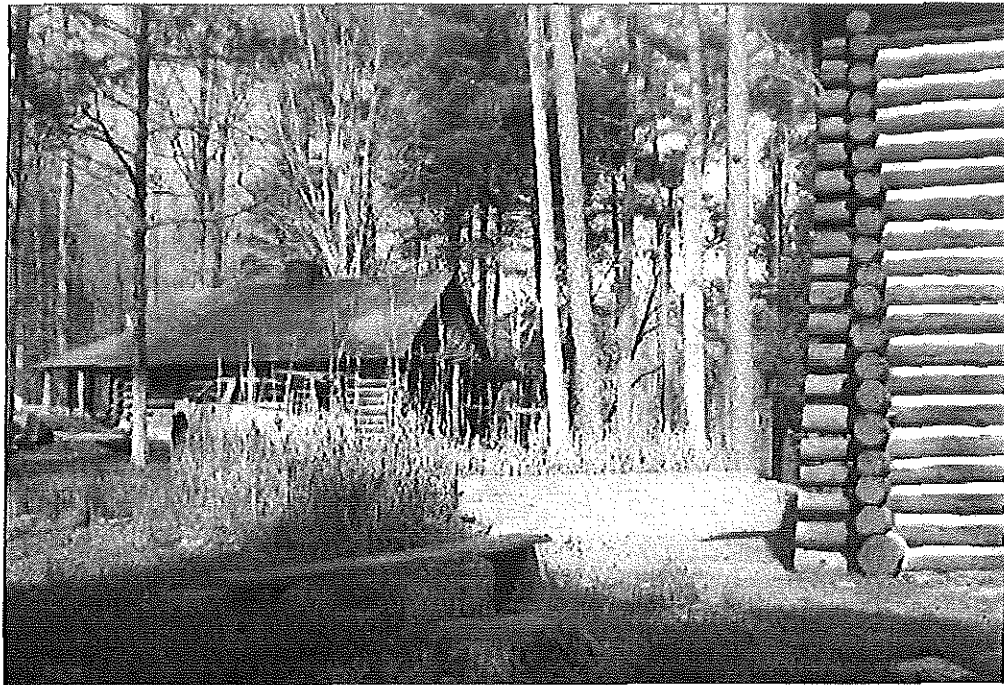
Figure 8: Hill Forest Residence Cottage no. 2, south and east elevations
