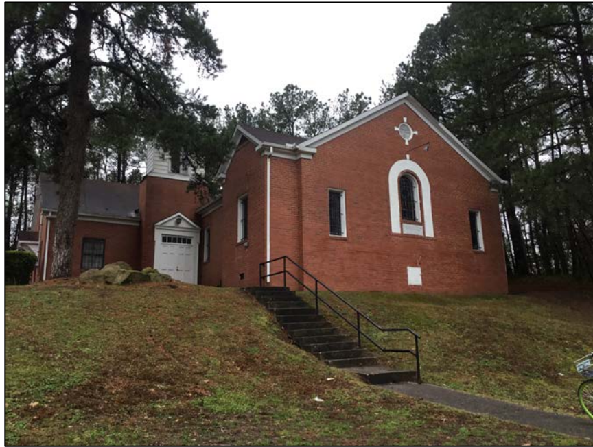
Figure 4-1. Asbury Temple United Methodist Church (DH 3964), view looking west from E. Lawson Street.
