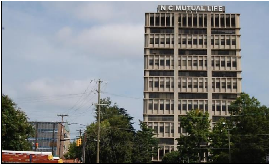
Figure 4-25. North Carolina Mutual Building (DH 2477)
