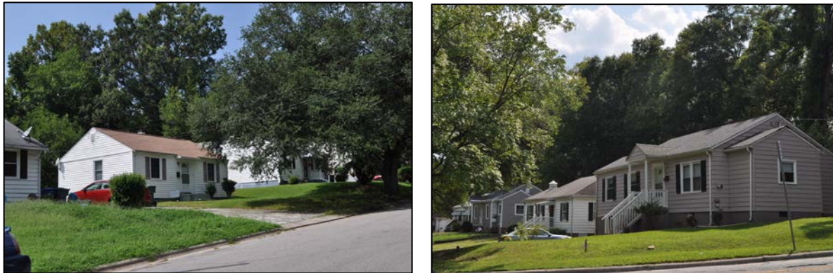
Figure 4-5. Views of the Glenview/Woodstock Neighborhood along Rosewood Street.
