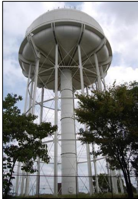
Figure 4-35. Durham Water Tower and Valve House (DH 3508)
