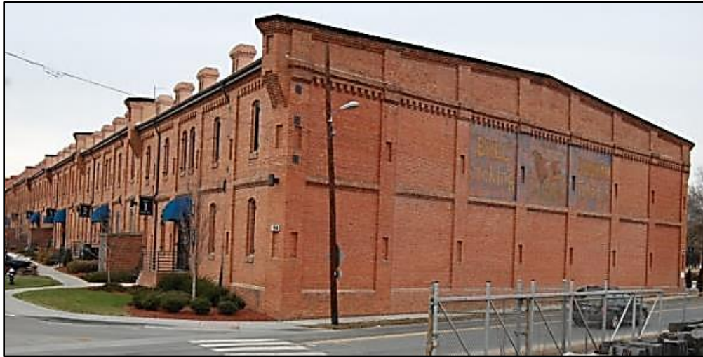
Figure 4-21. Smith Warehouse (DH 89)
