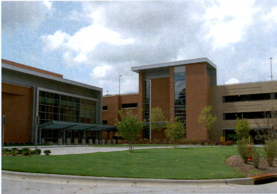
Plate 97. Modern North Carolina Correctional Facility West of Railroad Corridor (Excluded from Proposed National Register Boundary), Looking West.
