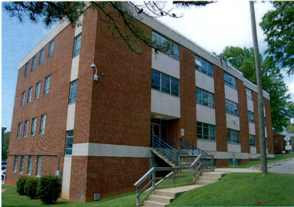
Plate 131. George W. Randall Administration Building, Side (East) and Rear (South) Elevations of Rear Wing, Looking Northwest.
