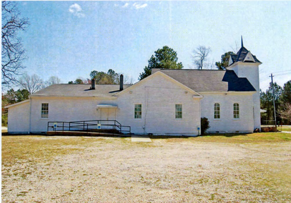
Plate 100. Auburn Christian Church, West Elevation, Looking East.
