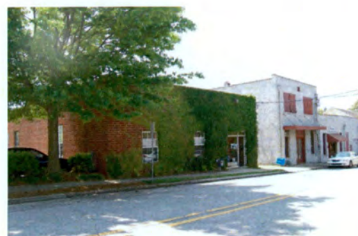
No. 42 Warehouse (PIN 1703384404), 731 West Hargett Street, Raleigh, Wake County
