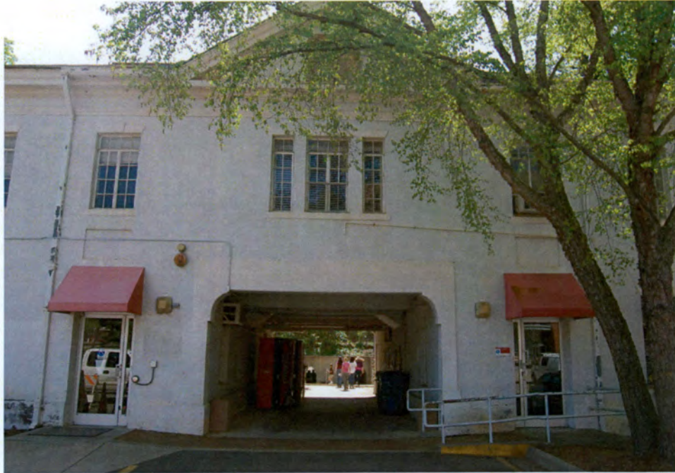
Plate 72. North Carolina State College Historic District, North Campus, Riddick Field House (Within APE), Looking South.
