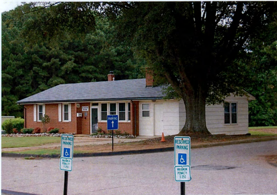
Plate 90. Governor Morehead School, Colored Department, Historic District, Principal's House (circa 1960), Looking Northwest.
