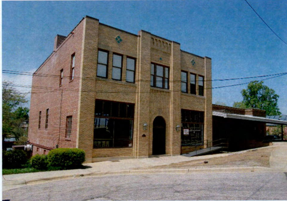
Plate 35. White Dairy Products Building, Façade (East Elevation) and Side (South) Elevation, Looking Northwest.
