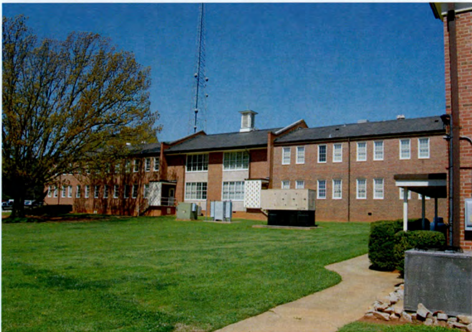
Plate 82. Governor Morehead School, Colored Department, Historic District, Deaf Girls' and Blind Girls' Cottages (circa 1930/circa 1960 Infill), Rear (South) Elevation, Looking North.
