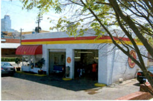
No. 8 Gas Station (PIN 1703489817), 501 West Morgan Street, Raleigh, Wake County
