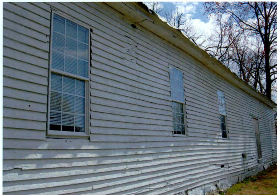
Plate 158. Watts Store and House, Side (West) Elevation of Store, New Windows.
