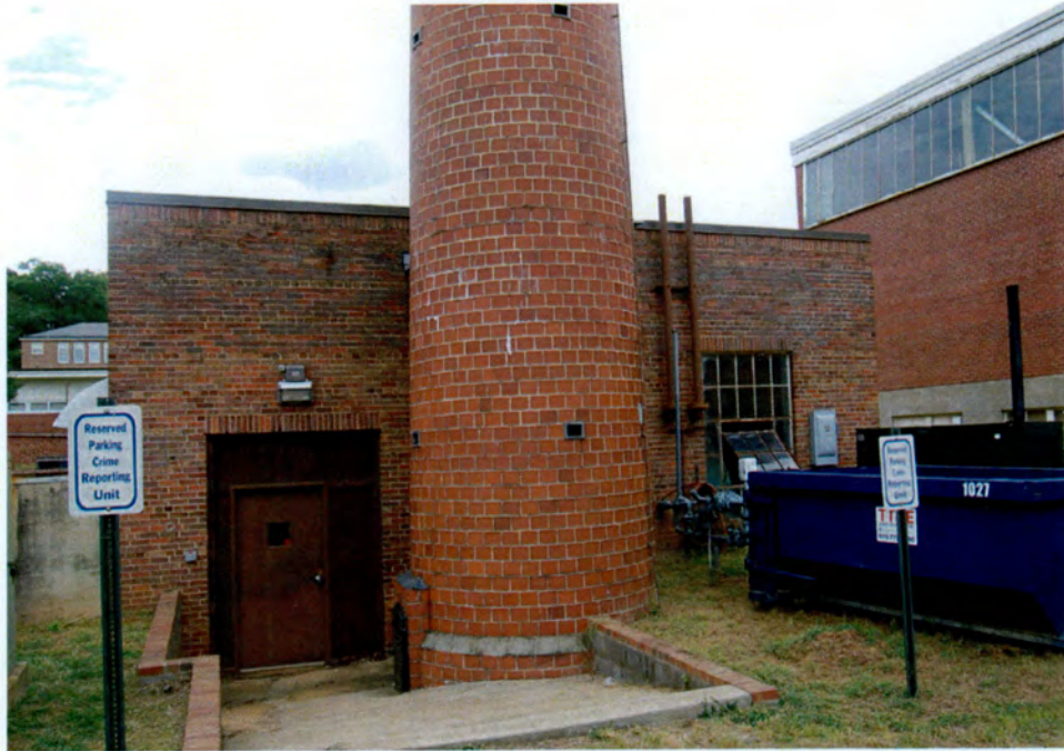
Plate 85. Governor Morehead School, Colored Department, Historic District, Heating Plant (circa 1930), West Elevation, Looking East.
