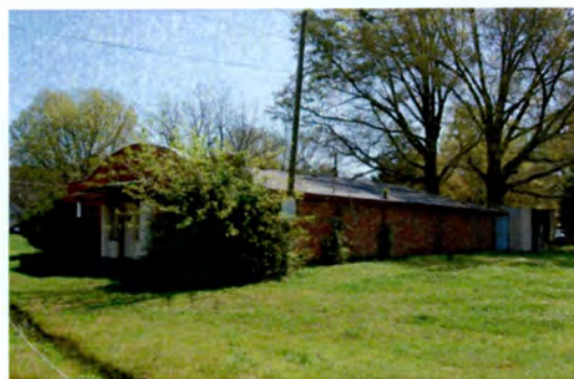
No. 59 House (PIN 1711165004), Other Building, 1331 East Garner Road, Garner, Wake County
