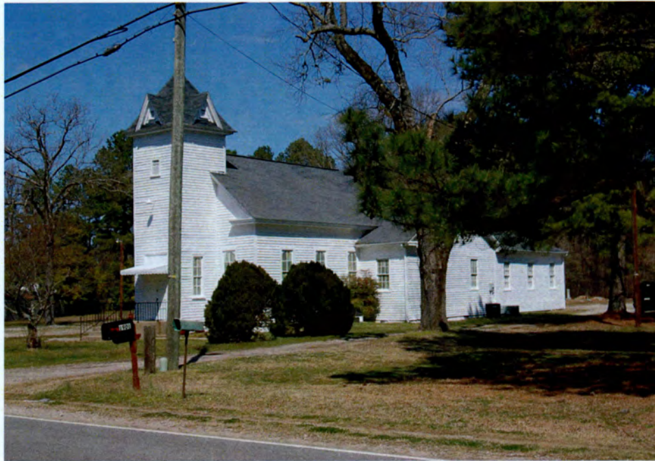
Plate 101. Auburn Christian Church, Front (South) and Side (East) Elevations, Looking Northwest.
