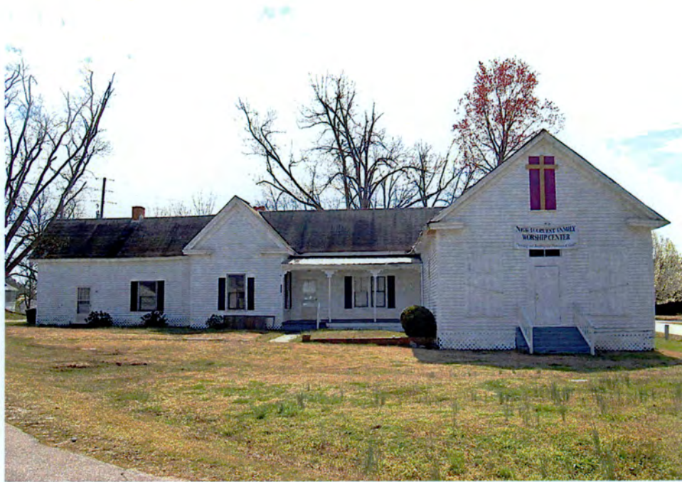
Plate 154. Watts Store and House, Overall View, Looking South.
