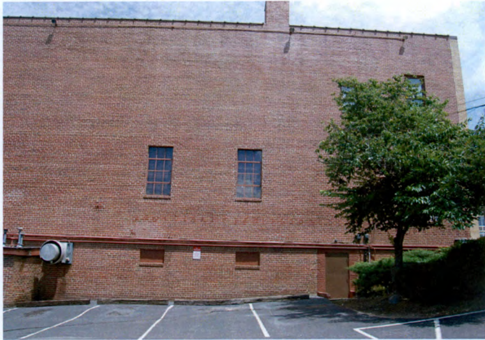
Plate 40. White Dairy Products Building, Side (South) Elevation, Looking North.
