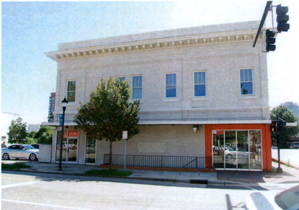
Plate 116. Commercial Block, Side (West) Elevation, Looking East.
