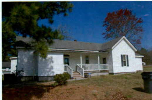
No. 87 House (PIN 1730177672), 2029 Auburn Road, Garner Vicinity, Wake County
