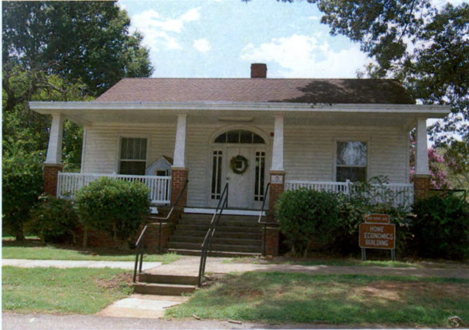
Plate 61. Governor Morehead School Historic District, Home Economics House, Looking West.
