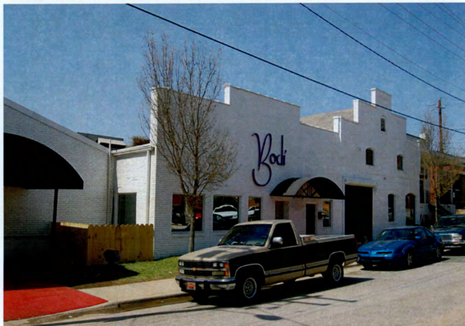
Plate 20. Depot Historic District, Proposed Amendment, Caveness Produce Company Warehouse (No. 17), on Left, and Swift Meat Company Warehouse No. 2 (No. 16), on Right, Looking Southwest.
