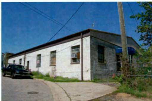
No. 32 Warehouse (PIN 1703473624), 324 Dupont Circle, Raleigh, Wake County
