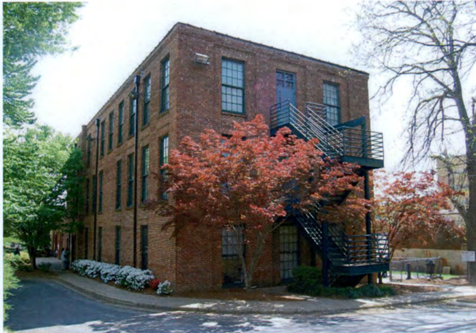
Plate 26. Raleigh Hosiery Company Building, Side (West) and Front (North) Elevations, Looking East.
