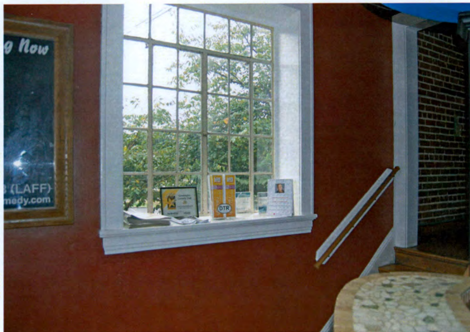
Plate 49. White Dairy Products Building, Interior, Former Receptionist's Office, Original Plaster Walls and Window Surround.
