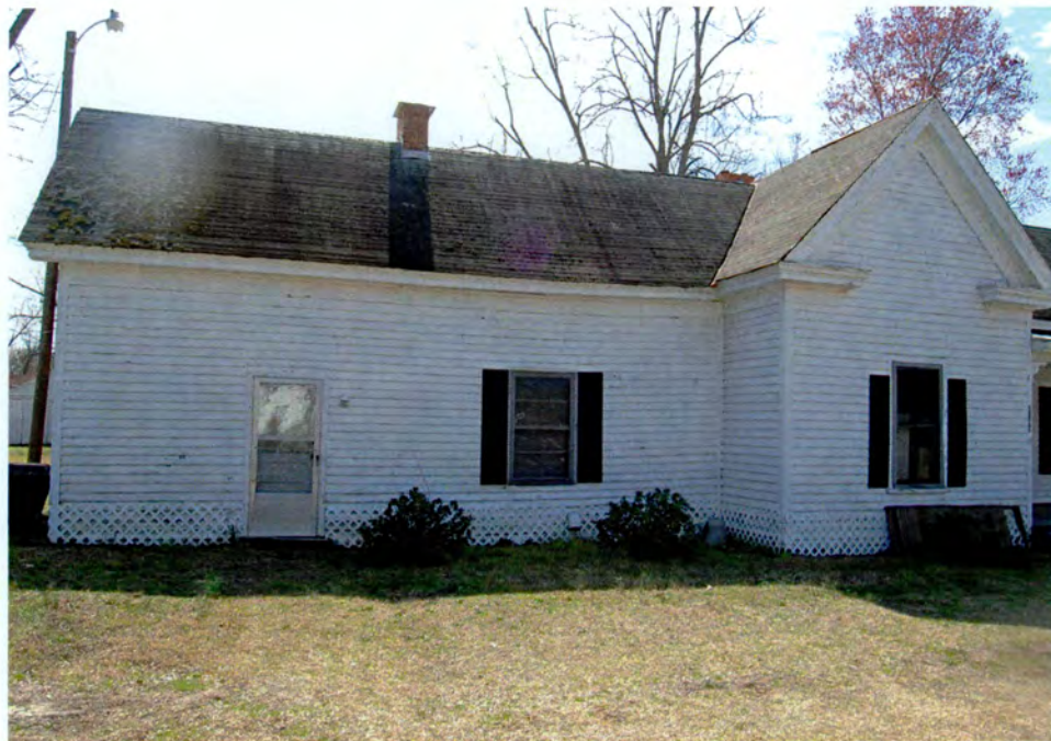
Plate 160. Watts Store and House, Front (North) Elevation of House and Late Nineteenth Century Wing, Looking South.
