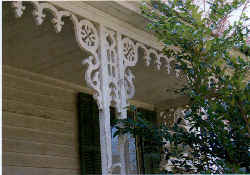
Plate 109. William Watts House, Porch Detail, Looking Southwest.
