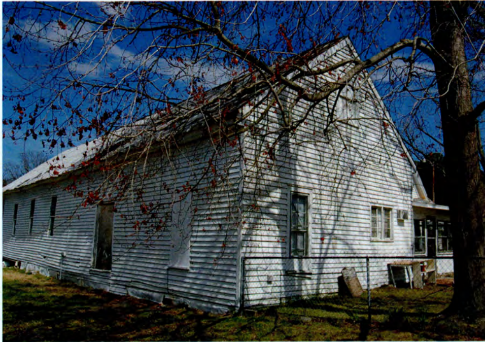
Plate 159. Watts Store and House, Side (West) and Rear (South) Elevations of Store, Looking South.
