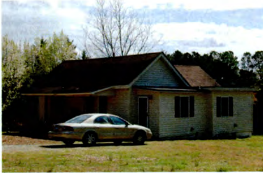
No. 80 House (PIN 1730264949), 2208 Auburn Road, Garner Vicinity, Wake County
