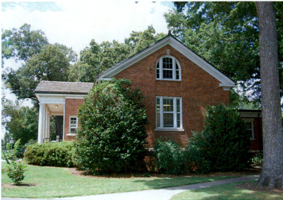
Plate 54. Governor Morehead School Historic District, Library (Within APE), Side (East) Elevation, Looking West.
