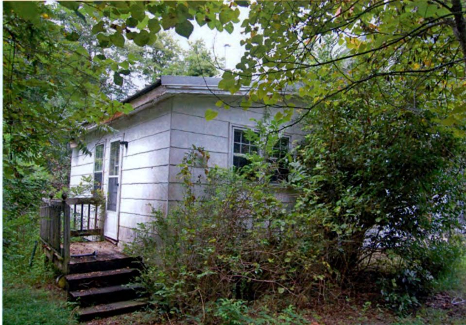
Plate 114. William Watts House, Rear Appendage, Looking West
