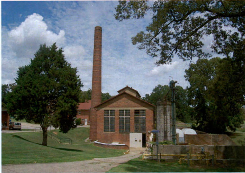
Plate 57. Governor Morehead School Historic District, Boiler Plant/Laundry, Looking North.
