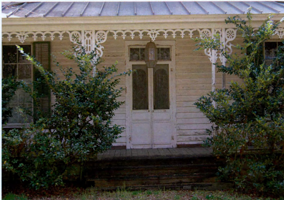
Plate 108. William Watts House, Entrance and Porch, Looking South.
