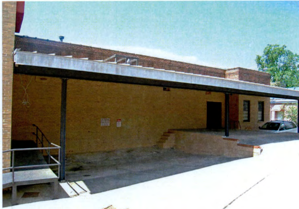
Plate 42. White Dairy Products Building, City Ice and Fuel Building, Attached to Side (North) Elevation of White Dairy Products Building, Looking Northwest.
