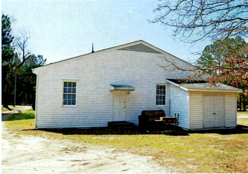
Plate 103. Auburn Christian Church, Rear (North) Elevation, Modern Rear Addition, Looking South.
