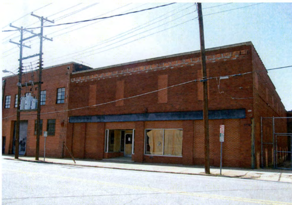
Plate 14. Depot Historic District, Proposed Amendment, Noland Company Building (No. 12), Looking West.
