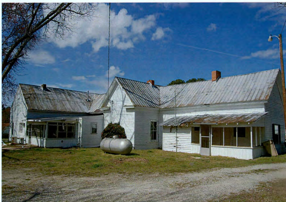
Plate 162. Watts Store and House, Rear (South) Elevations, Looking Northwest.
