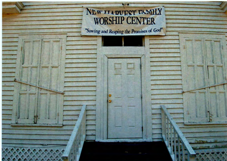
Plate 156. Watts Store and House, Store Façade (North Elevation), Looking South.
