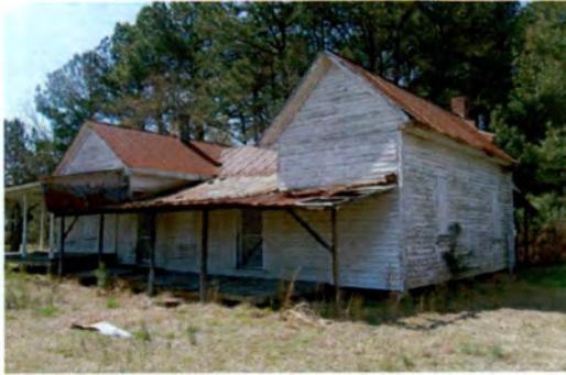
No. 66 House (WA0323) (PIN 1721900562), 0 East Garner Road, Garner Vicinity, Wake County
