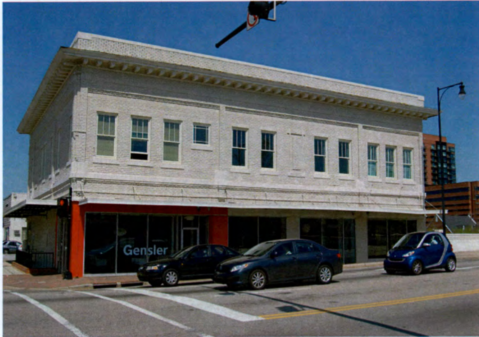
Plate 115. Commercial Block, Front (South) Elevation, Looking North.
