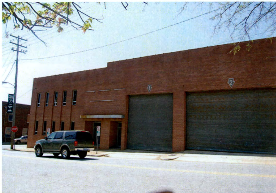
Plate 12. Depot Historic District, Proposed Amendment, Peden Steel Works (No. 10), Looking Southwest.
