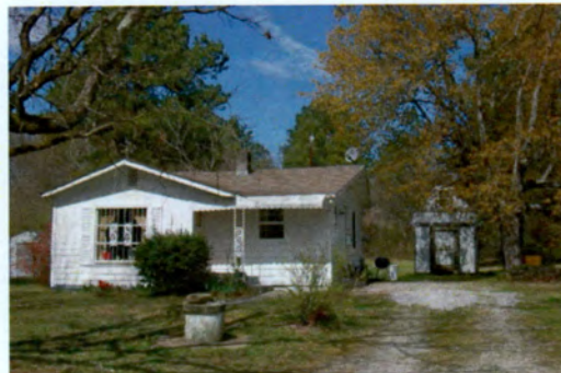
No. 88 House (PIN 1730276649), 2025 Auburn Road, Garner Vicinity, Wake County
