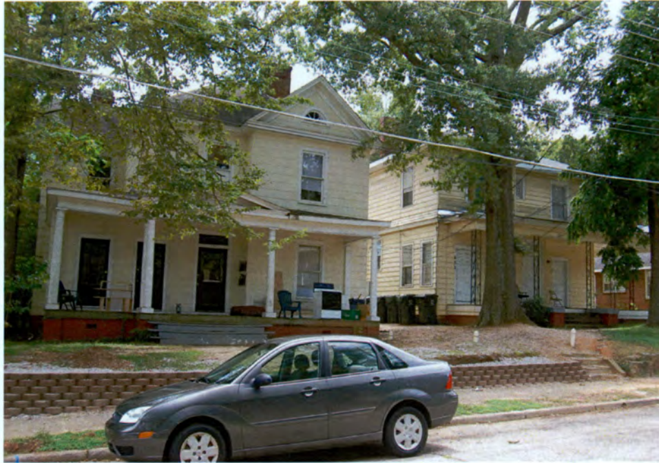
Plate 146. Park Avenue-Ashe Avenue Historic District, 207-211 Park Avenue, Looking East.
