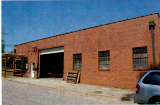
No. 34 Warehouse, (PIN 1703472722), 330 Dupont Circle, Raleigh, Wake County
