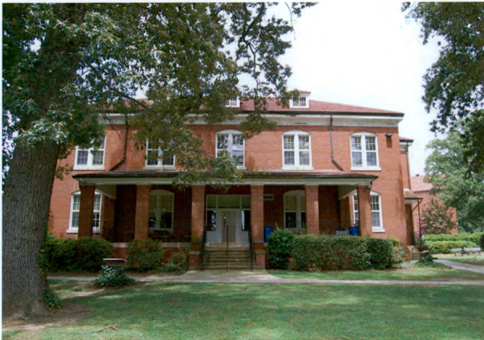
Plate 56. Governor Morehead School Historic District, Dormitory (Simpson Building), Looking North.
