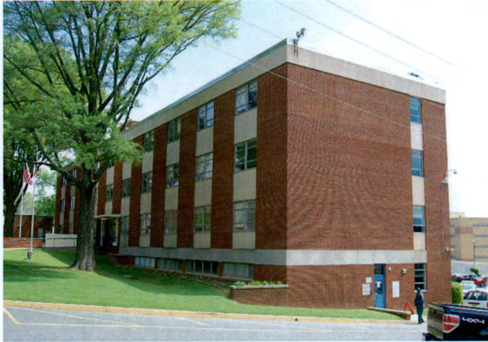
Plate 128. George W. Randall Administration Building, Front (North) and Side (West) Elevations, Looking East.
