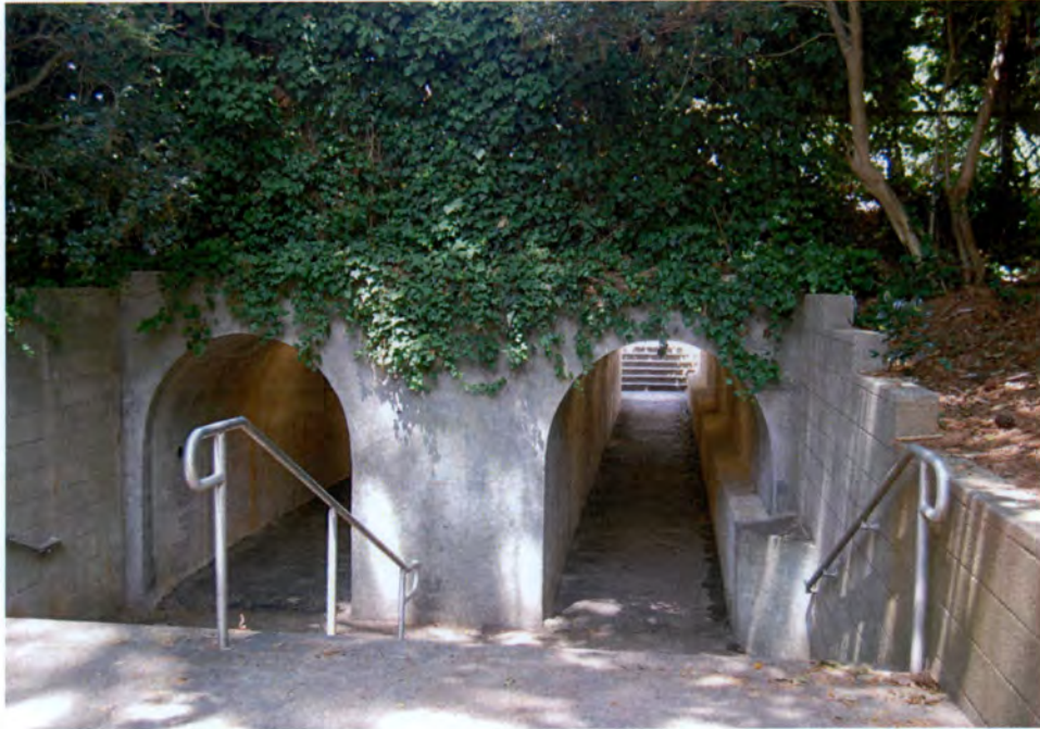
Plate 76. North Carolina State College Historic District, Pedestrian Tunnel (Within APE), Looking North.
