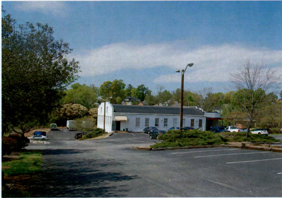
Plate 135. Martin Millwork Company-Woodworking Shop, Overall View, Looking Northwest.
