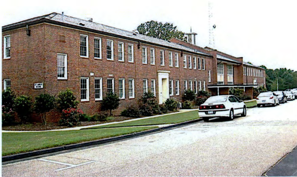
Plate 83. Governor Morehead School, Colored Department, Historic District, Deaf Girls' and Blind Girls' Cottages (circa 1930/circa 1960 Infill), Front (North) Elevation, Looking Southwest.
