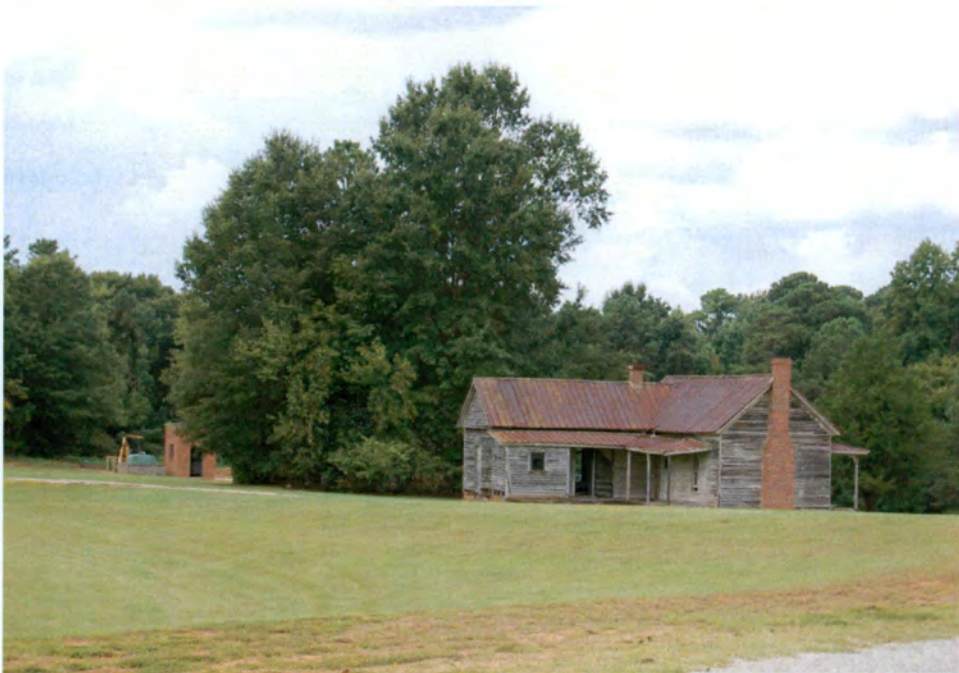
Plate 94. Governor Morehead School, Colored Department, Historic District, House for Agricultural Workers on Dairy Farm (circa 1900), Looking West toward Railroad Corridor.
