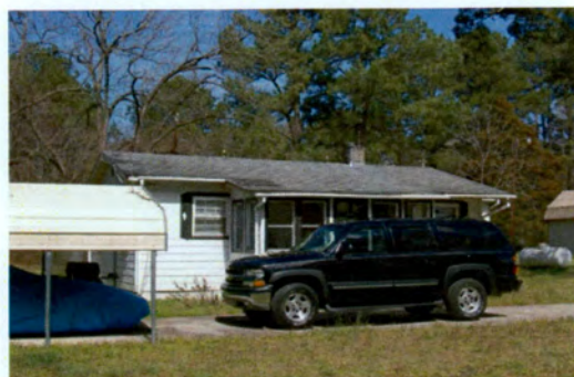
No. 89 House (PIN 1730175657), 2021 Auburn Road, Garner Vicinity, Wake County
