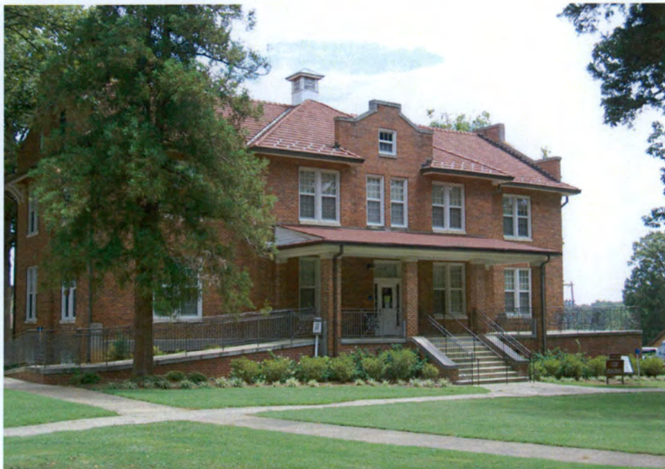
Plate 58. Governor Morehead School Historic District, Dormitory (Cox Building), Looking East.
