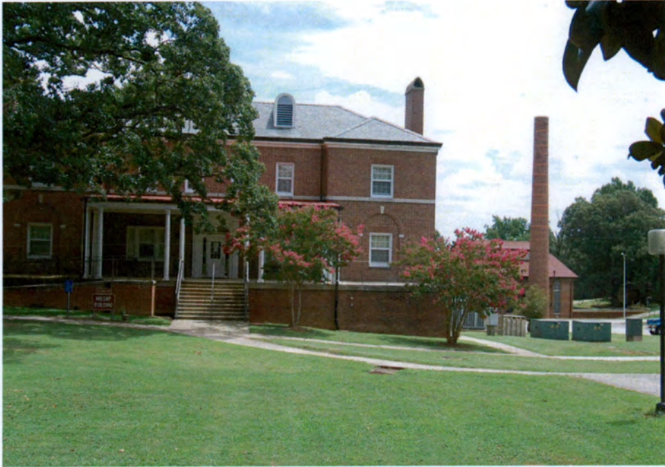
Plate 59. Governor Morehead School, Dormitory (Milsap Building), Looking South towards Boiler Plant/Laundry.
