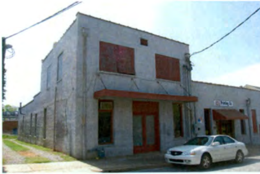
No. 43 Warehouse (PIN 1703383445), 733 West Hargett Street, Raleigh, Wake County
