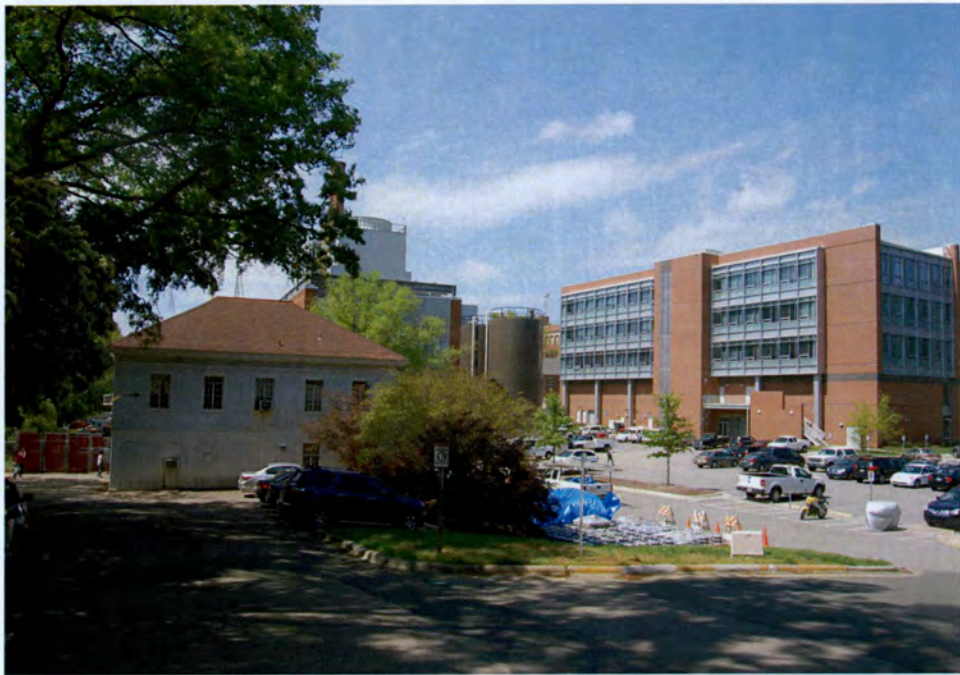
Plate 71. North Carolina State College Historic District, Riddick Field House (Left) (Within APE), Looking West.
