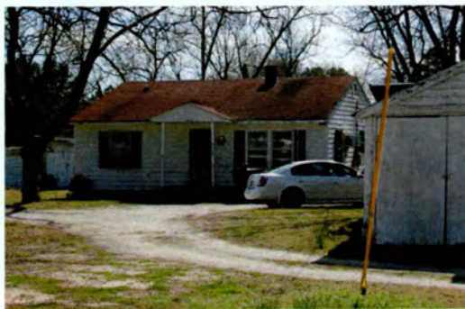
No. 84 House (PIN 1730271142), 2106 Auburn Road, Garner Vicinity, Wake County
