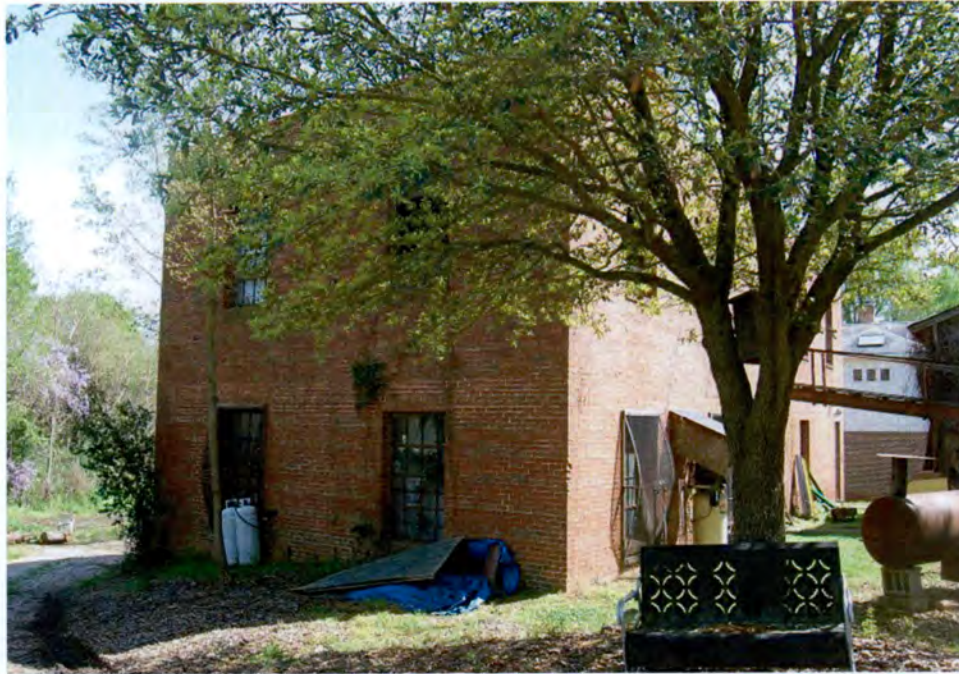
Plate 25. Boylan Heights Historic District, Warehouse (No. 37), 303 Kinsey Street (Within APE), Looking Southeast.
