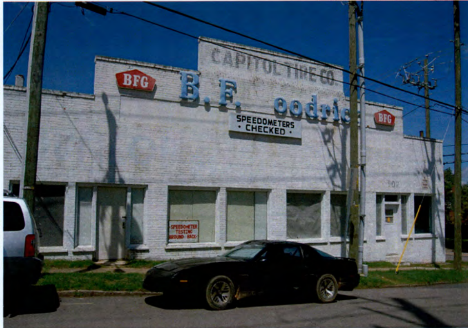
Plate 121. Old Fourth Ward Historic District, Warehouse (No. 31), 518 South West Street (Within the APE), Looking West.
