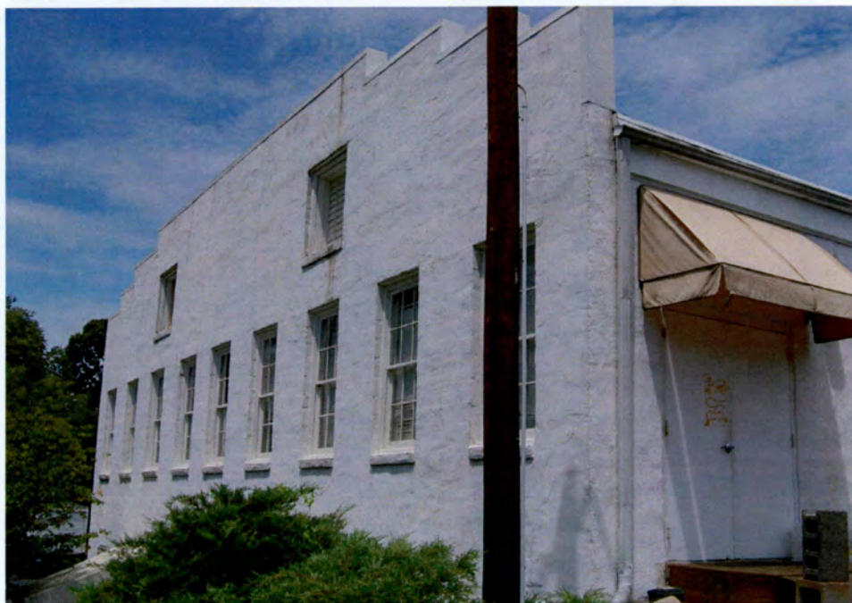
Plate 138. Martin Millwork Company-Woodworking Shop, Rear (South) Elevation, Looking Northwest.
