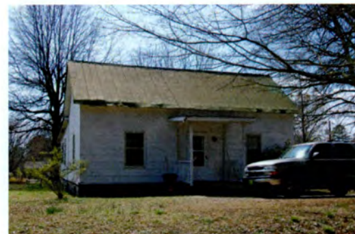
No. 79 House (PIN 1730267832) 2300 Auburn Road, Garner Vicinity, Wake County
