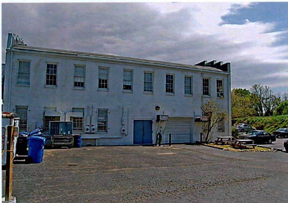
Plate 137. Martin Millwork Company-Woodworking Shop, Side (West) Elevation, Looking East.
