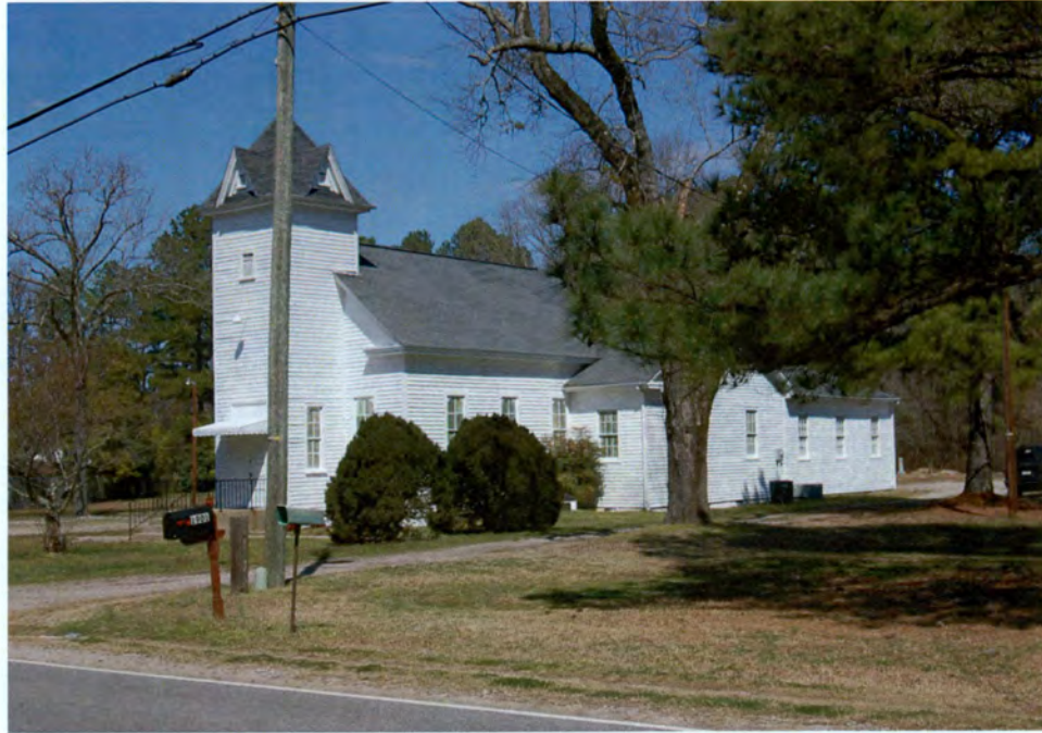
Plate 172. Auburn, Auburn Christian Church (No. 71), Looking Northwest.
