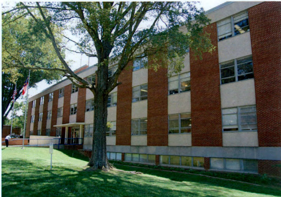
Plate 129. George W. Randall Administration Building, Front (North) Elevation, Looking Southeast.
