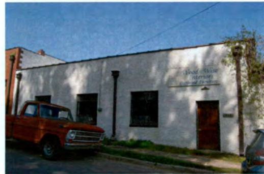
No. 33 Warehouse (PIN 1703472668), 328 Dupont Circle, Raleigh, Wake County
