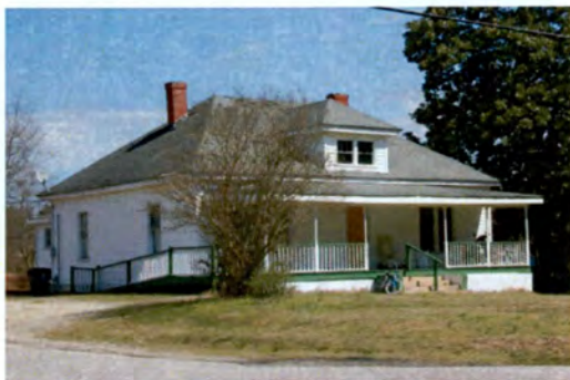
No. 70 House (PIN 1730094147), 1801 East Garner Road, Garner Vicinity, Wake County
