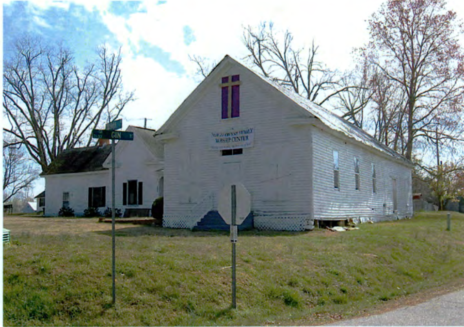
Plate 157. Watts Store and House, Store and House Façades (North Elevations), Side (West) Elevation of Store, Looking Southeast.
