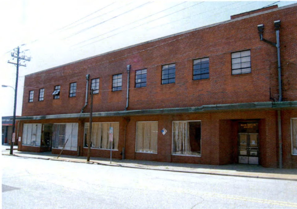
Plate 16. Depot Historic District, Proposed Amendment, Dillon Supply Company Warehouse (No. 13), Looking Southwest.
