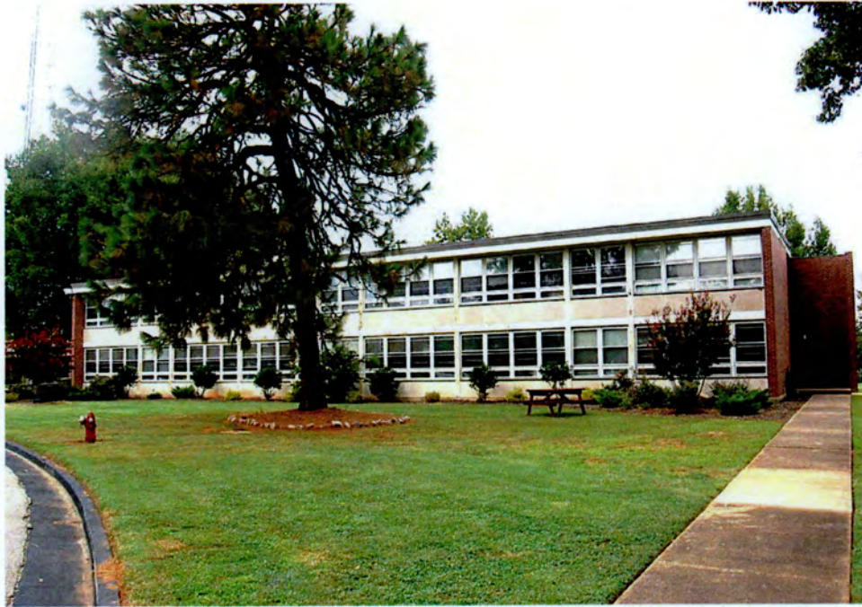
Plate 87. Governor Morehead School, Colored Department, Historic District, William Young Cottage (Girls' Dormitory) (circa 1960), South Elevation, Looking North.
