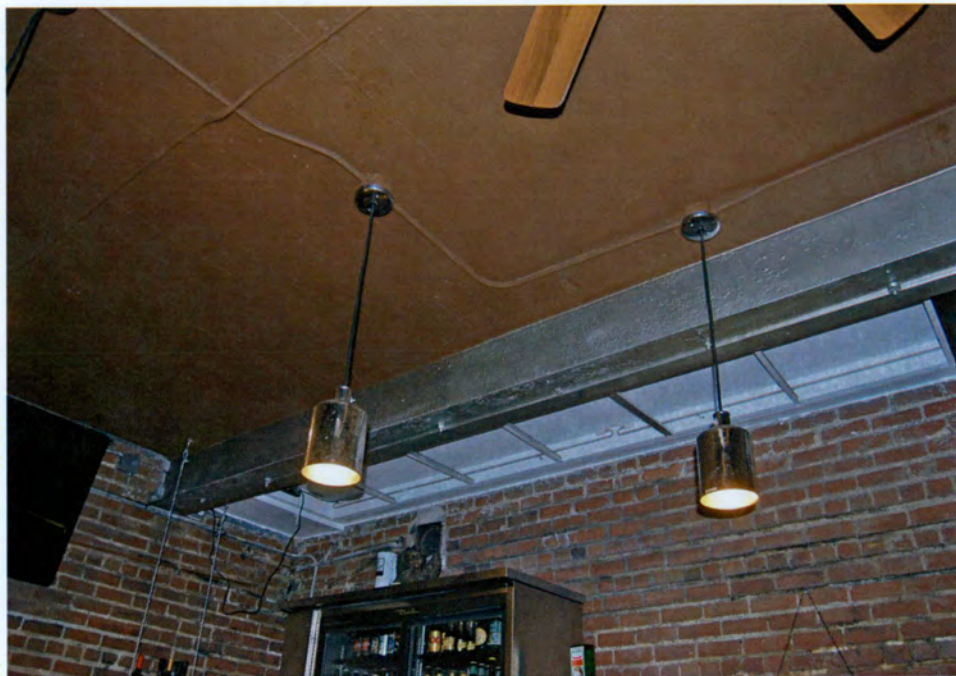
Plate 48. White Dairy Products Building, Interior, Basement, Ceiling Beam.
