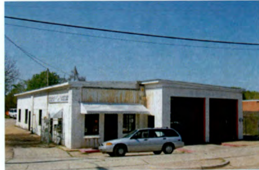
No. 38 Garage (PIN 1703377957), 234 South Boylan Avenue, Raleigh, Wake County
