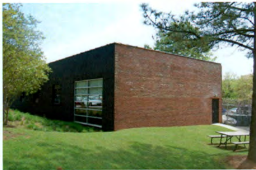
No. 46 Warehouse (PIN 1703287689), 819 West Hargett Street, Raleigh, Wake County
