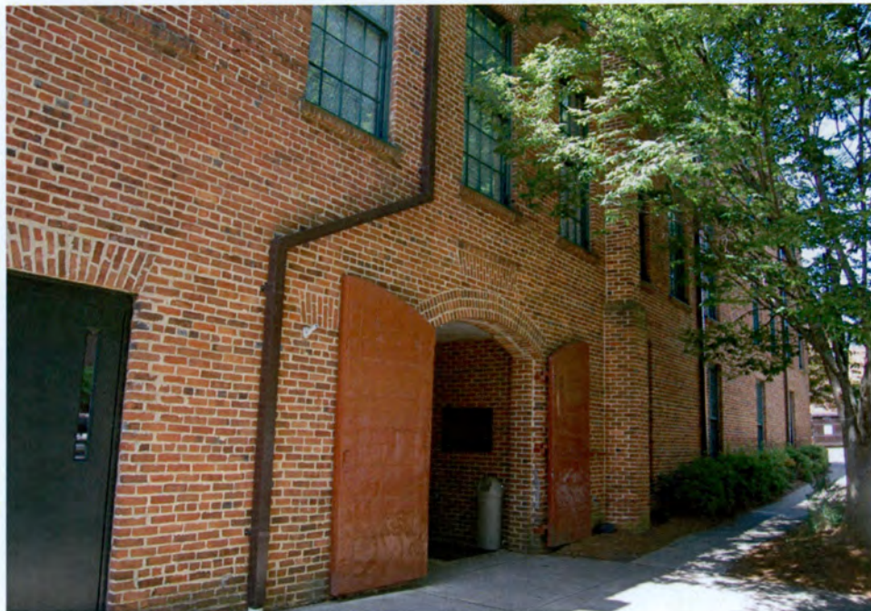
Plate 27. Raleigh Hosiery Company Building, Front (North) Elevation, Looking Southwest.
