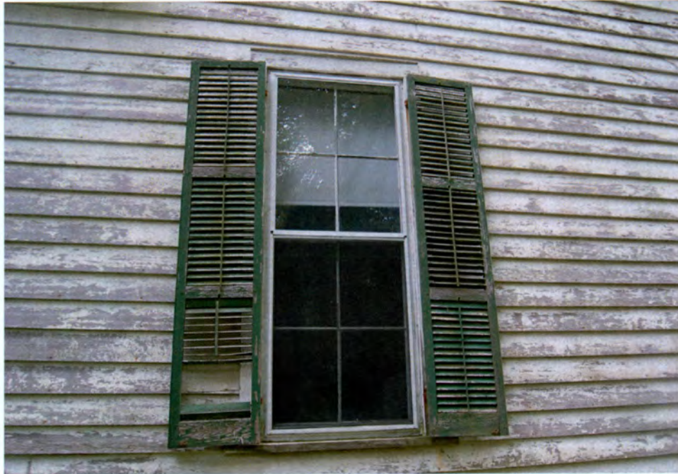
Plate 113. William Watts House, Window, Side (West) Elevation, Looking East.
