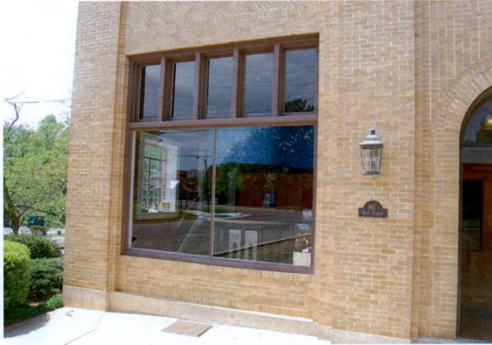
Plate 38. White Dairy Products Building, Façade, First-Story Window, Looking Southwest.
