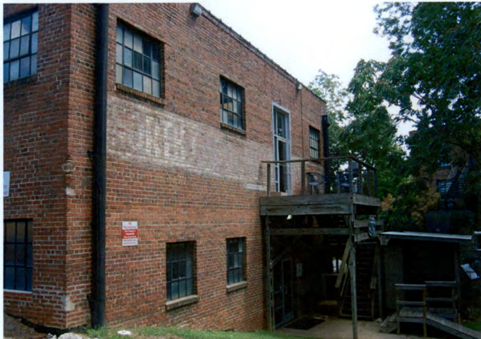
Plate 34. North Carolina School Book Depository, Rear (South) Elevation, Looking Northeast.
