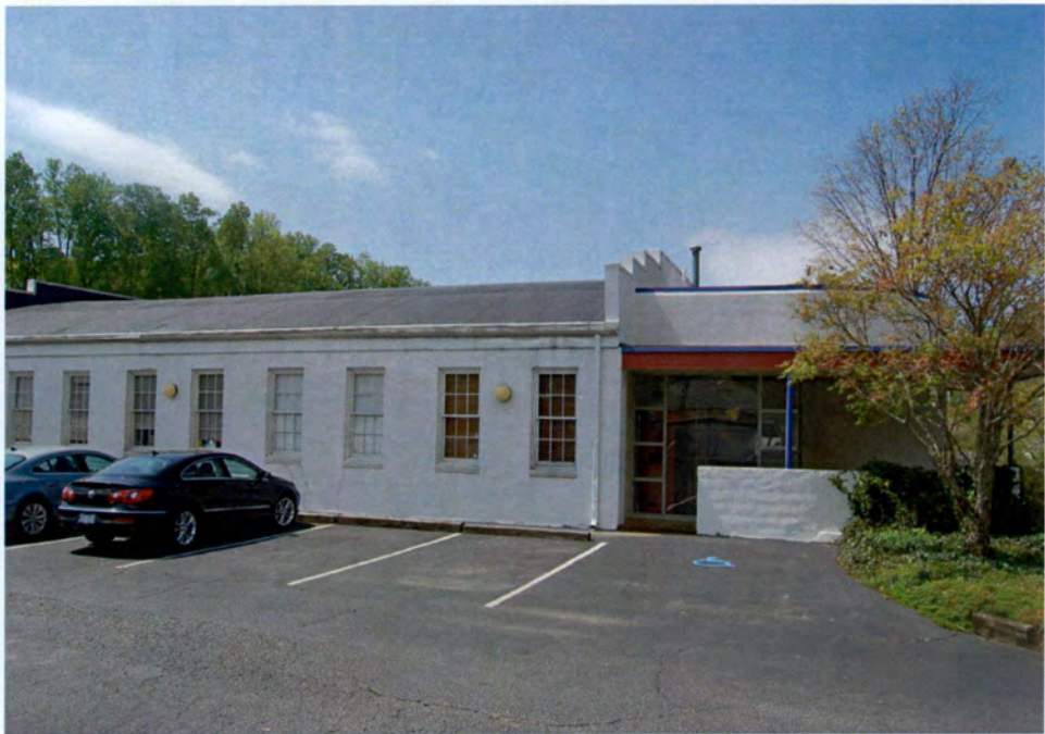
Plate 136. Martin Millwork Company-Woodworking Shop, Side (East) Elevation and Modern Entrance Addition, Looking West.
