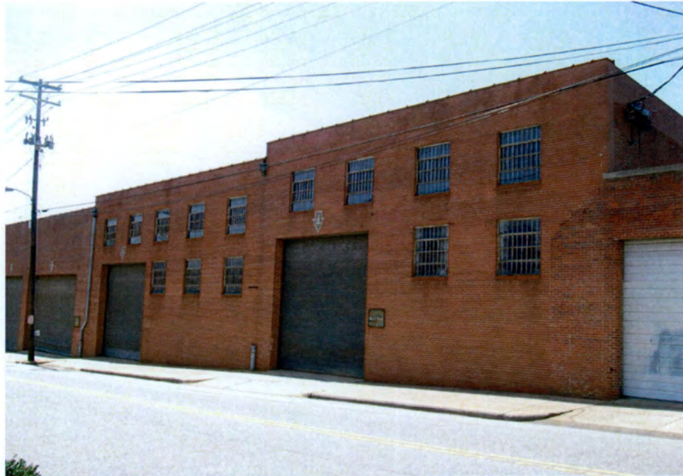
Plate 11. Depot Historic District, Proposed Amendment, Peden Steel Works (No. 10), Looking Southwest.
