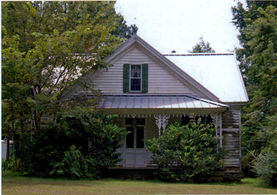
Plate 107. William Watts House, Façade (North Elevation), Looking South.
