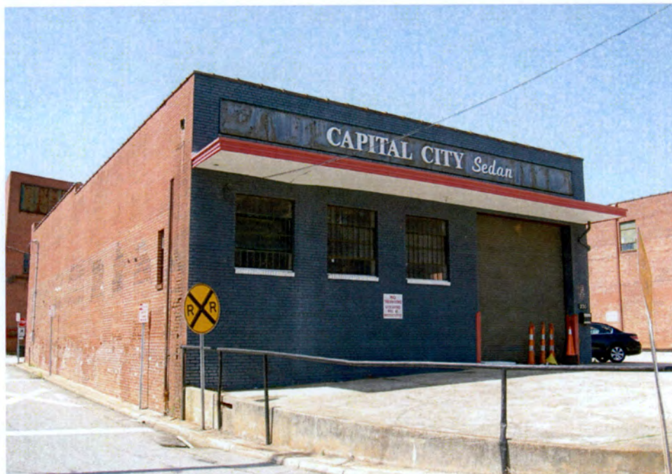
Plate 17. Depot Historic District, Proposed Amendment, Capital Feed and Grocery Company Building (No. 14), Looking Northwest.
