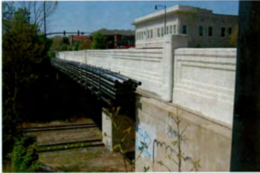
No. 2 Bridge No. 910528, Hillsborough Street, Raleigh, Wake County
