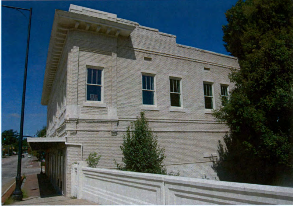
Plate 117. Commercial Block, Side (East) Elevation, Looking West.
