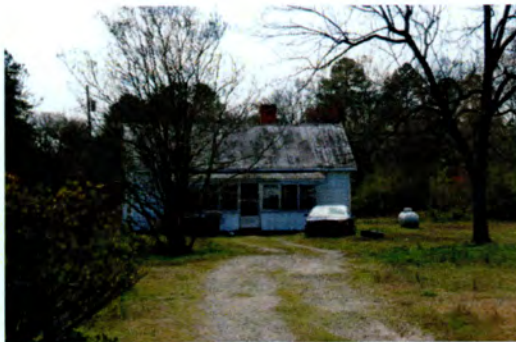
No. 82 House (PIN 1730271142), 2110 Auburn Road, Garner Vicinity, Wake County
