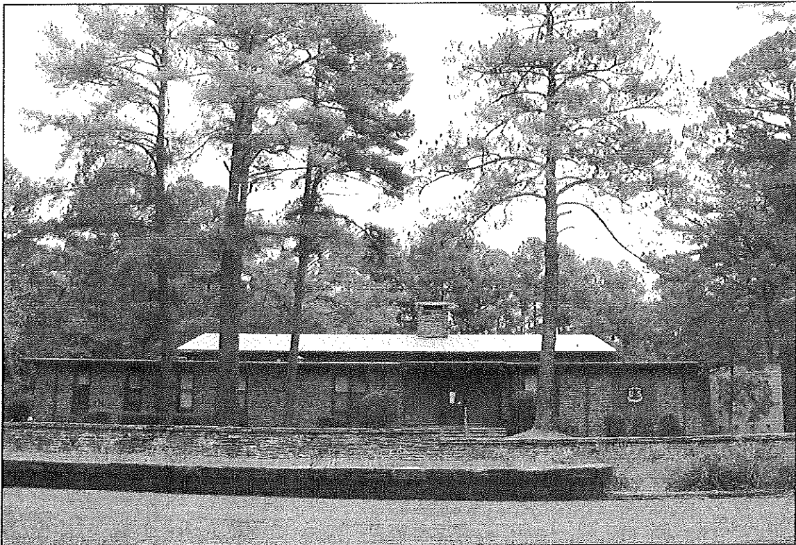
Figure 7.3. DH 3502: Main Laboratory Building, façade, looking northeast.
