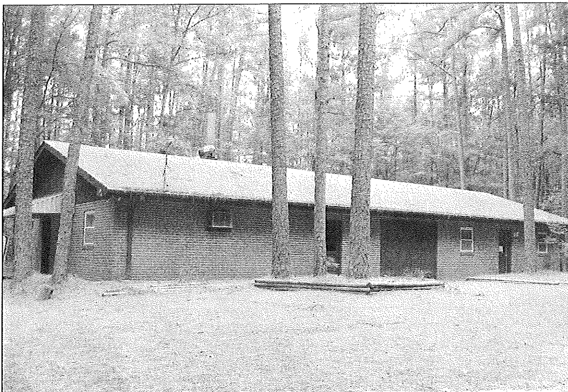
Figure 7.22. DH 3504: Annex, façade and northeast elevation, looking south.
