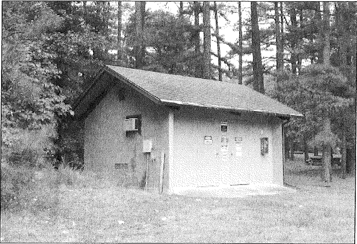
Figure 7.25. New Chemical Storage Building.
