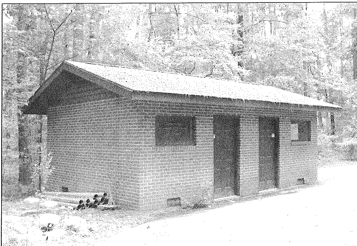
Figure 7.23. DH 3505: Old Chemical Storage Building, façade and northeast elevation, looking south.
