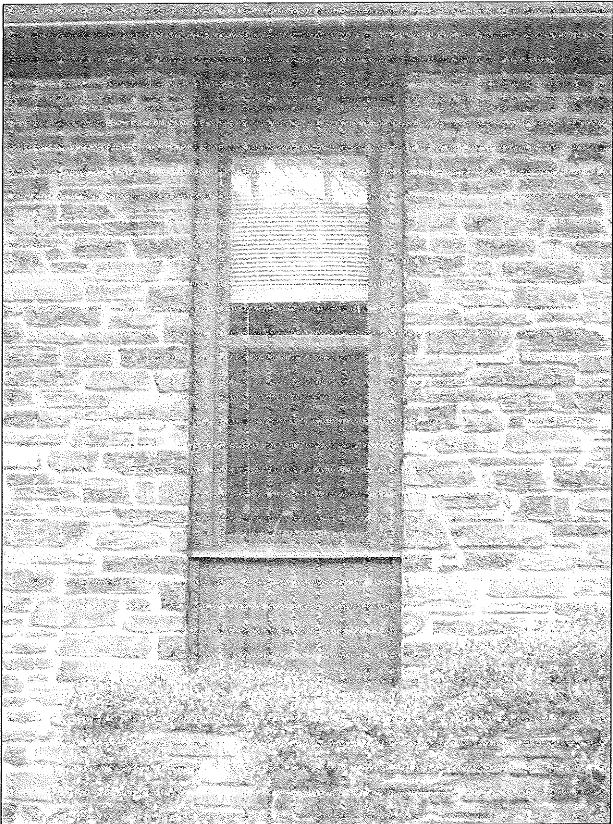
Figure 7.9. DH 3502: Main Laboratory Building, window and stone detail, looking northeast.
