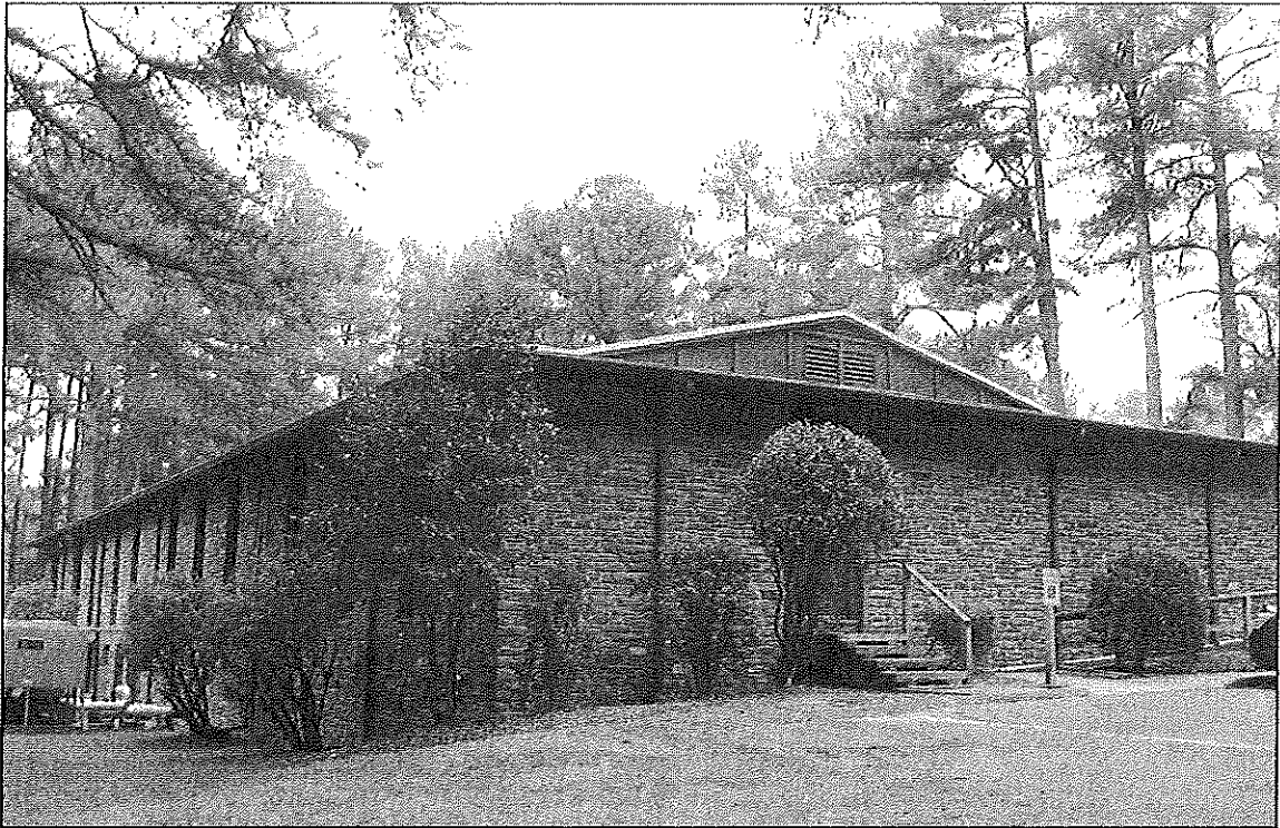
Figure 7.4. DH 3502: Main Laboratory Building, northwest (side) and northeast (rear) elevations, looking southeast.
