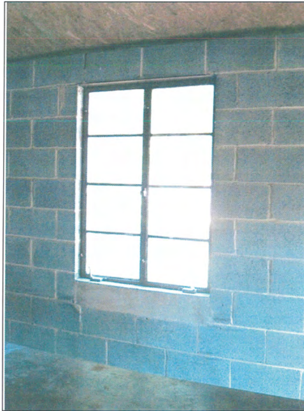
Figure 5.15. Detail of interior window in building 3503.
