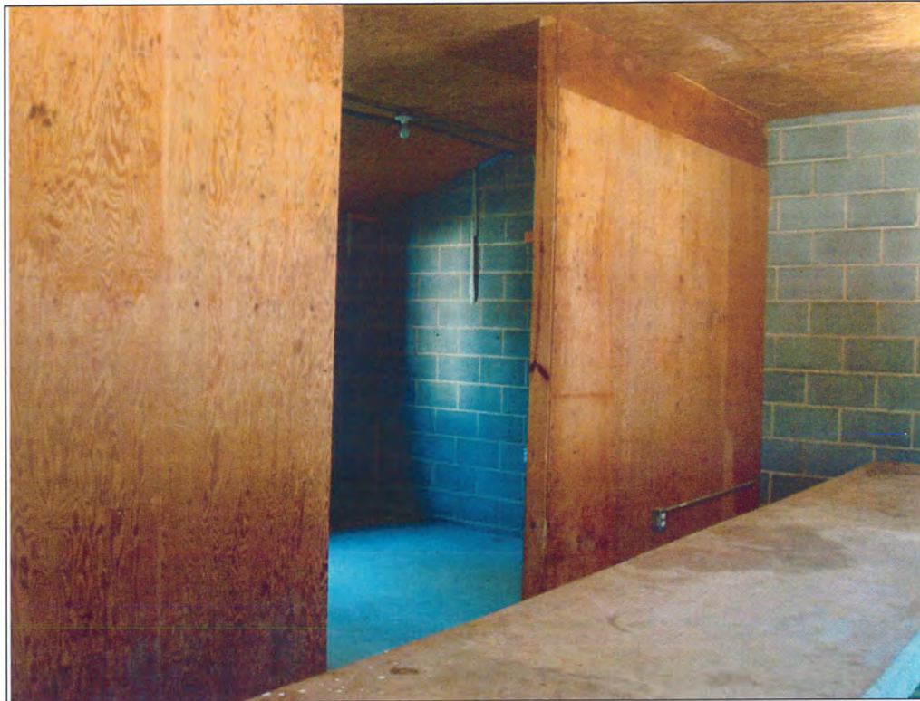
Figure 5.31. Interior of 3703, showing plywood divider.
