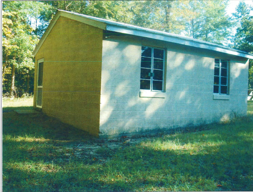
Figure 5.13. Oblique exterior view of building 3503 showing the north and east elevations.
