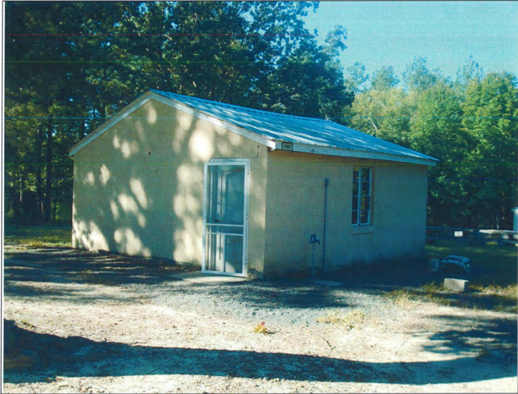
Figure 5.10. Oblique view of building 3502, north and east elevations.
