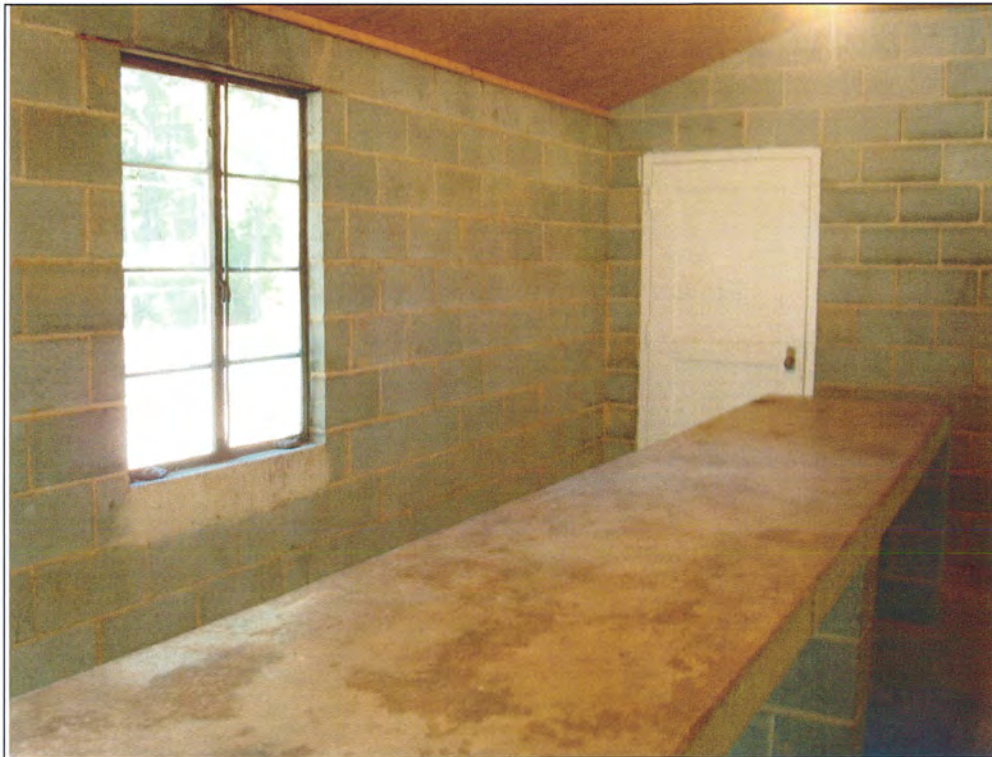
Figure 23. Interior of Building 3701.
