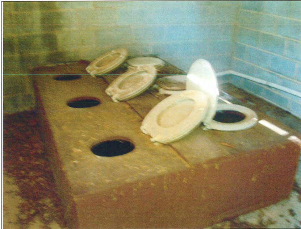
Figure 5.18. Male Latrine in Building 3505.
