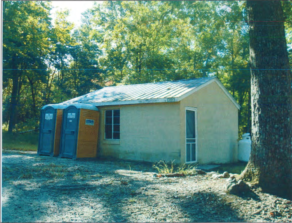
Figure 5.4. West and south elevations of Building 3501.
