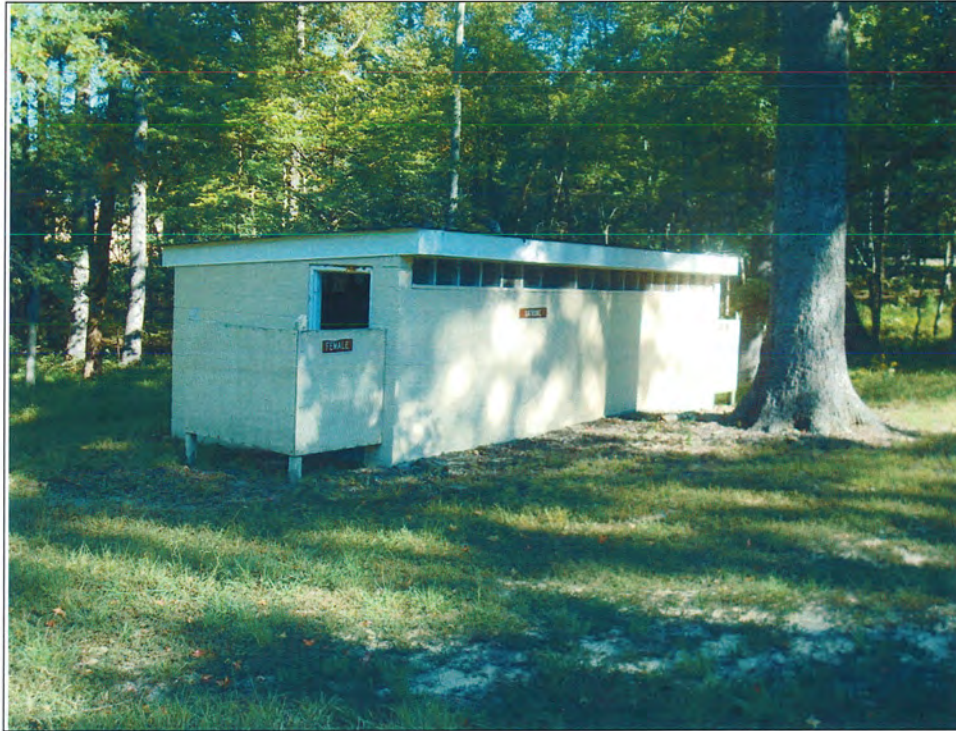
Figure 5.16. Oblique view of the Building 3505 showing the west and south elevations.
