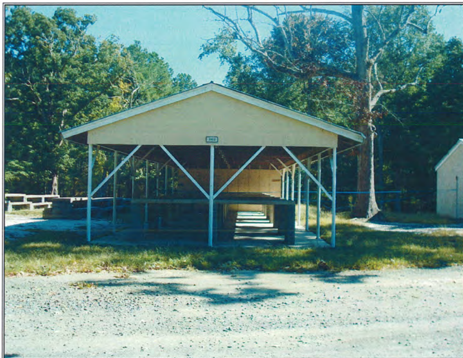
Figure 5.27. Building 3702, showing tables under overhang.
