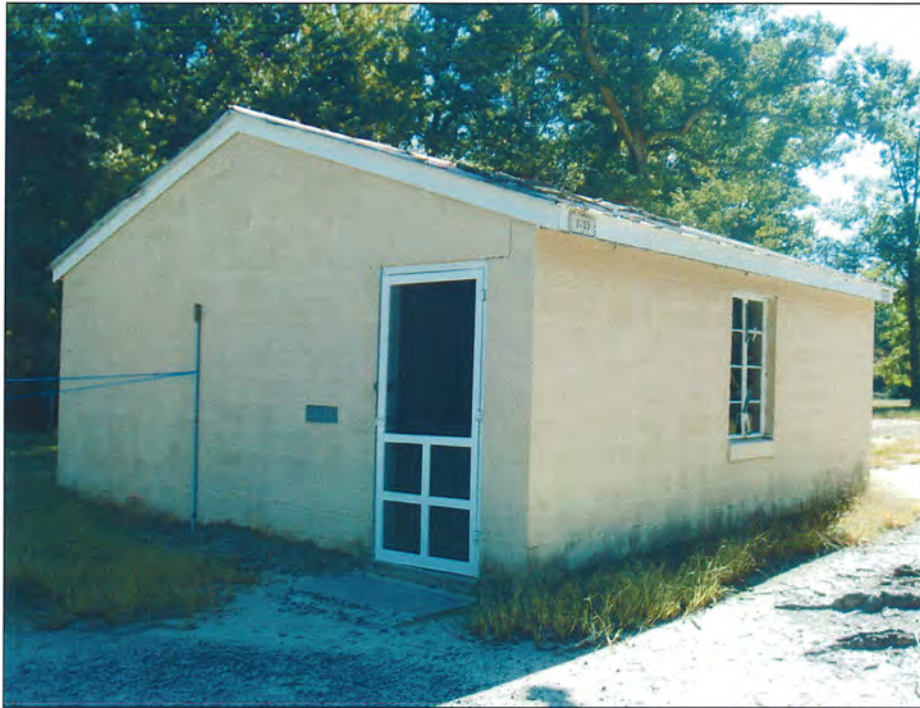
Figure 5.30. Exterior of Building 3703 oblique view of north and east elevations.
