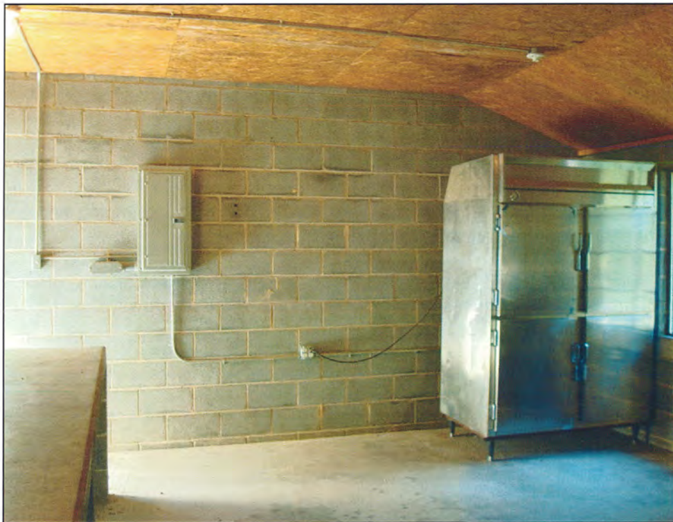
Figure 5.5. The poured concrete counter in Building 3501, which is duplicated in the other kitchens documented in this survey.
