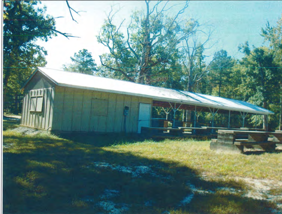
Figure 5.26. South and east elevations of Building 3702.
