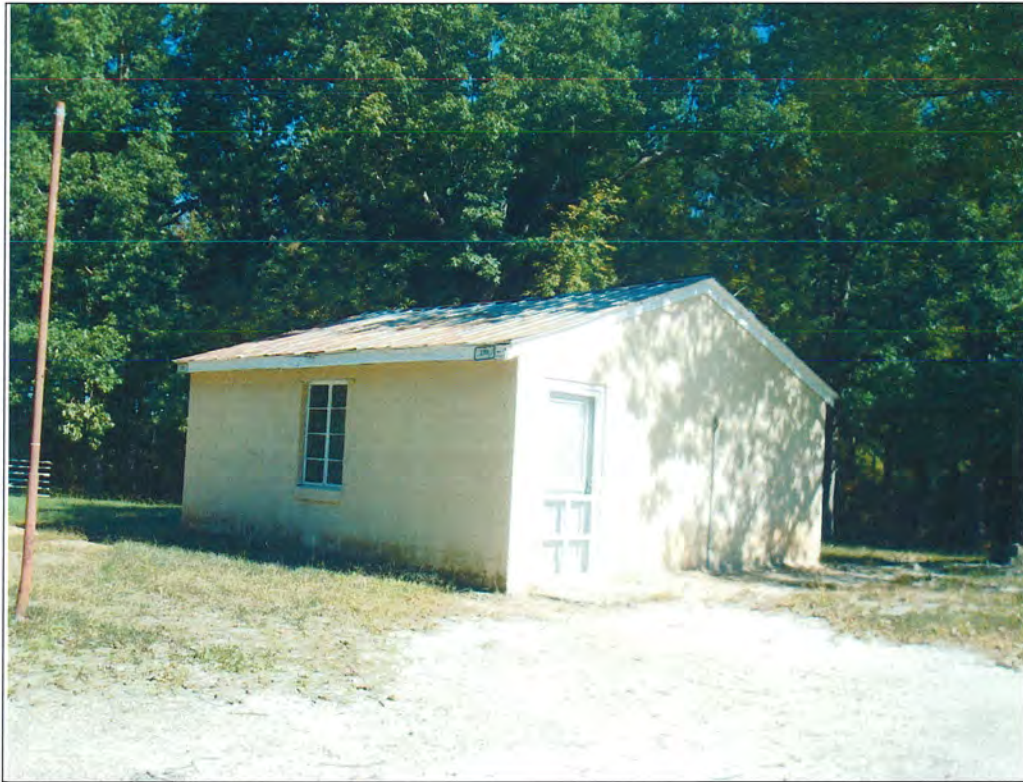
Figure 5.22. Oblique view of west and north elevations of Building 3701.
