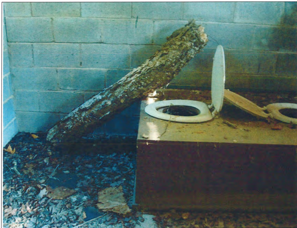
Figure 5.17. Female latrine in Building 3505.
