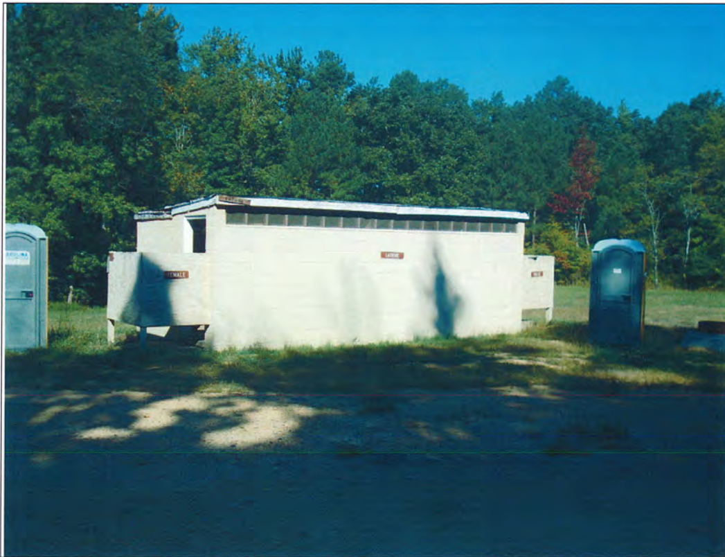
Figure 5.32. East elevation of Building 3704.
